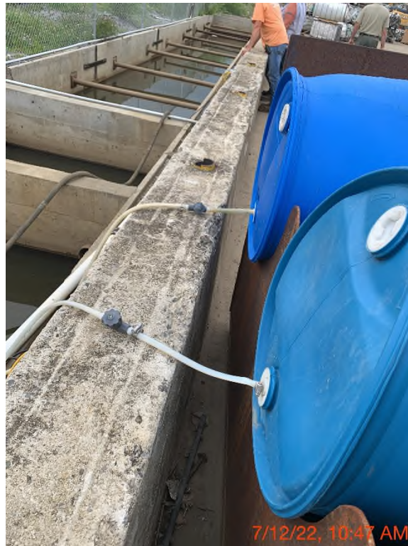
7/12/2022 Improper secondary containment for drums and hoses.
