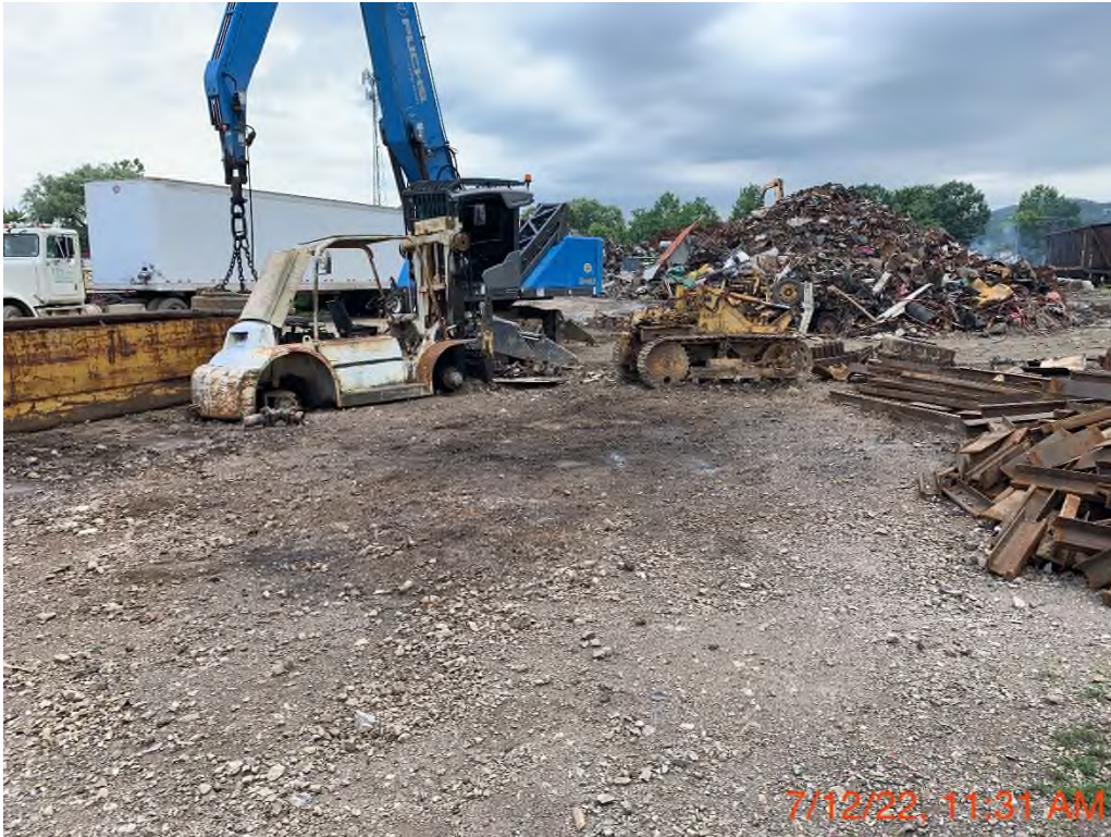
7/12/2022 Staining near the metal cutting area.
