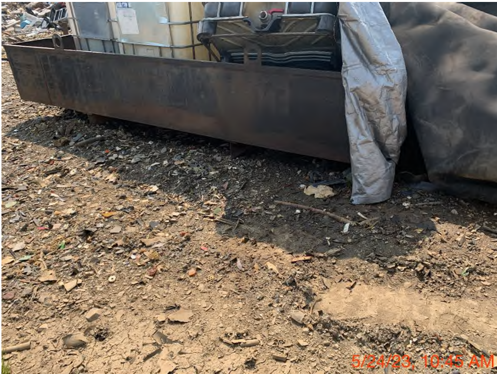
5/24/2023 There was staining on the ground around secondary containment.
