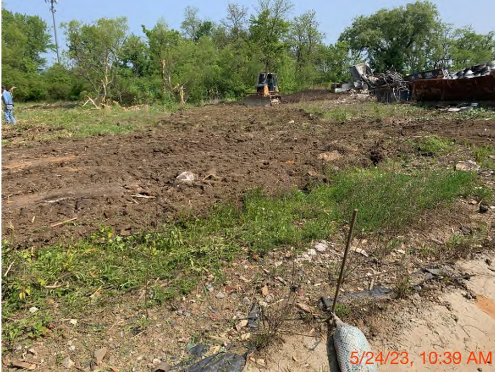
5/24/2023 There was heavy equipment filling in the “wetland” area.
