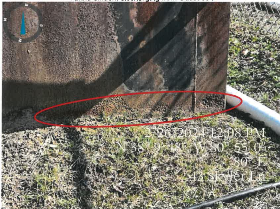
Corrosion/pitting
