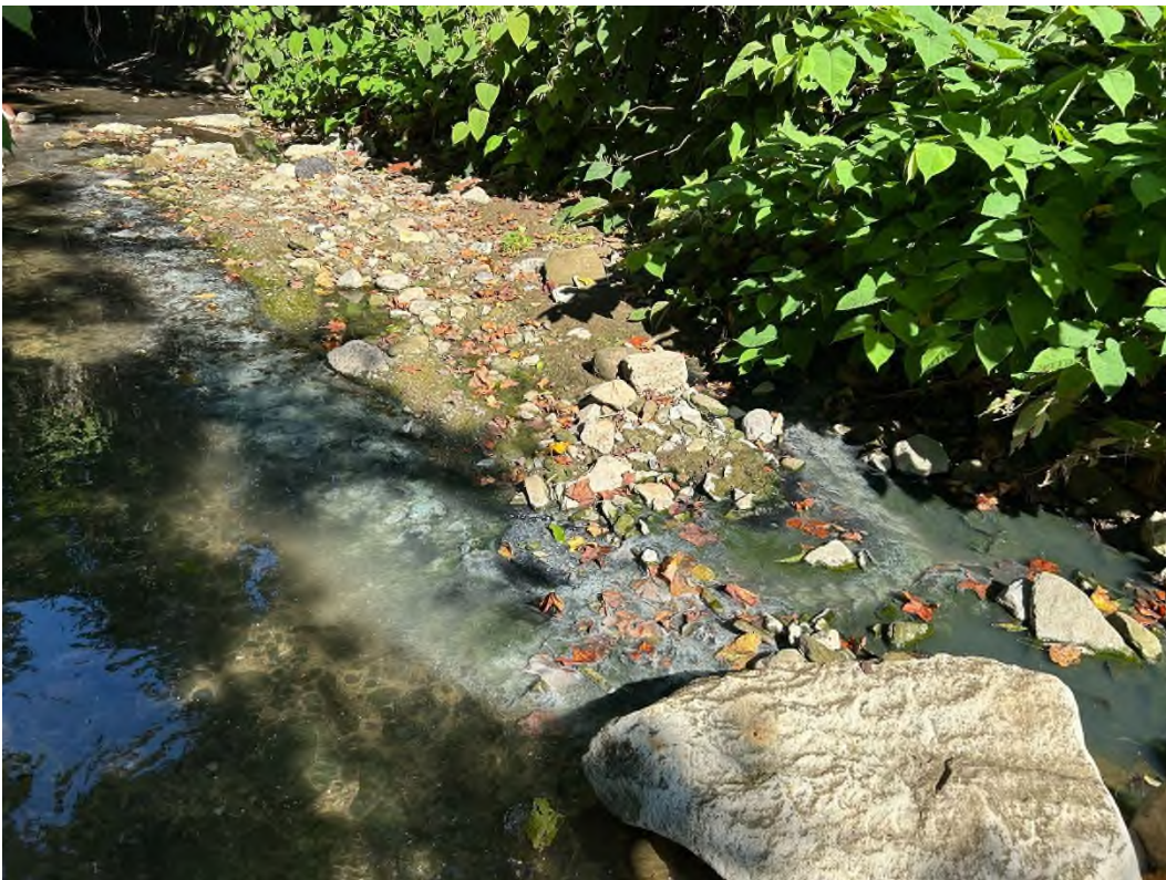
8/26/2025 - IMG_6022 Dry weather discharge from Outfall C003, causing a sludge bank in waters of the State.
