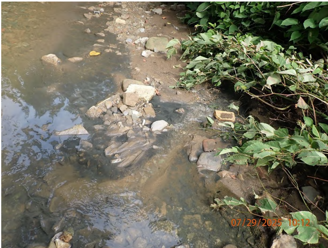
7/29/2025 - P7292029 - Outlet C003 discharging in dry weather, causing a sludge bank in waters of the State.
