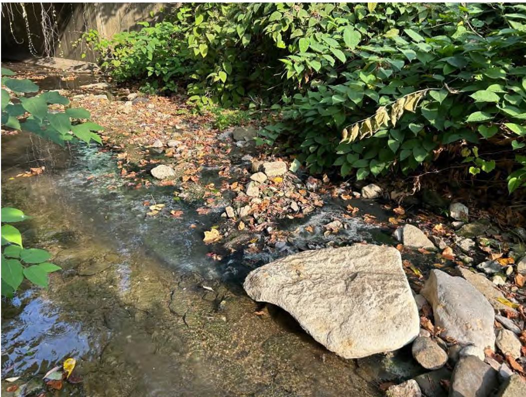
9/22/2025 - IMG_6103 Dry weather overflow from Outfall C003, causing a sludge blanket in waters of the State.
