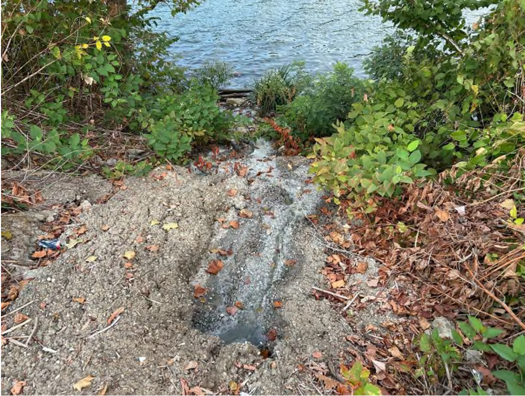
9/22/2025 - IMG_6101 Dry weather overflow from Outfall C002.
