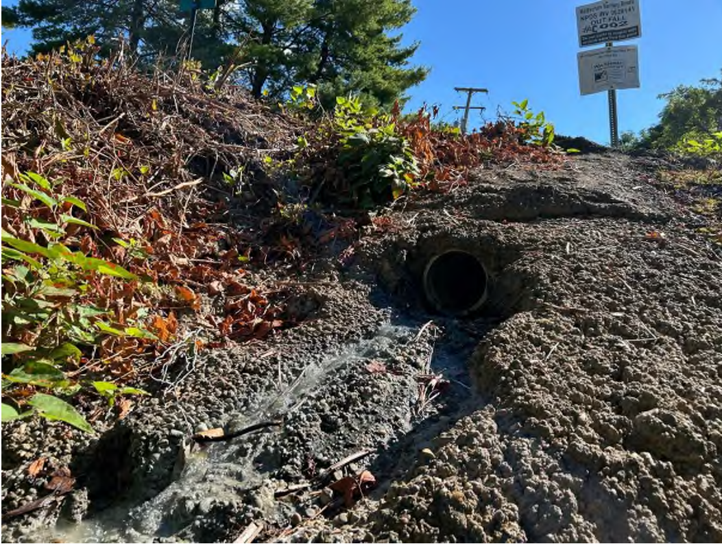
8/26/2025 - IMG_6025 Dry weather discharge from Outfall C002
