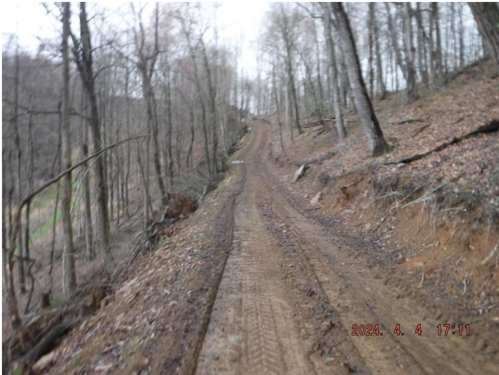
Photo # DSCF4145: Proposed access road on sheet 1 lacks stabilization and BMPs.
