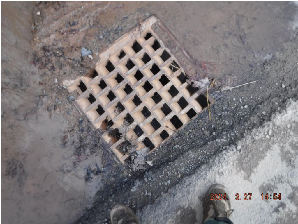
Photo # DSCF3444: Drop inlet protection missing from drop inlet B1.
