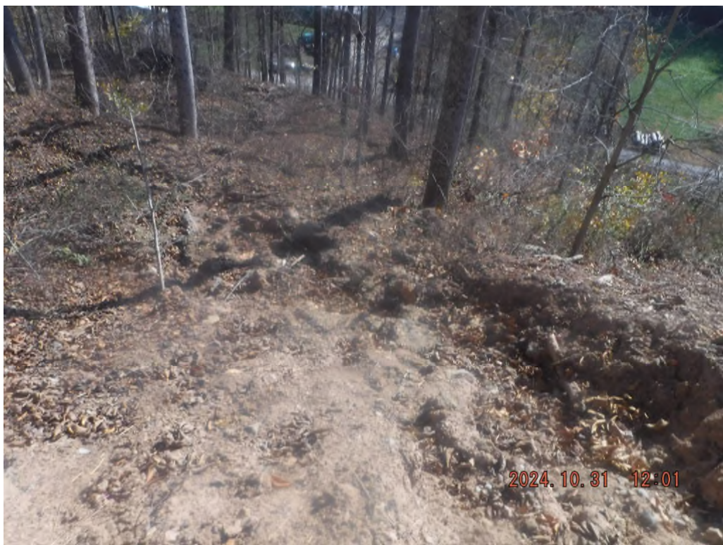
Photo # DSCF0036: Sediment offsite adjacent to the waterbar outlet at station 77+50.
