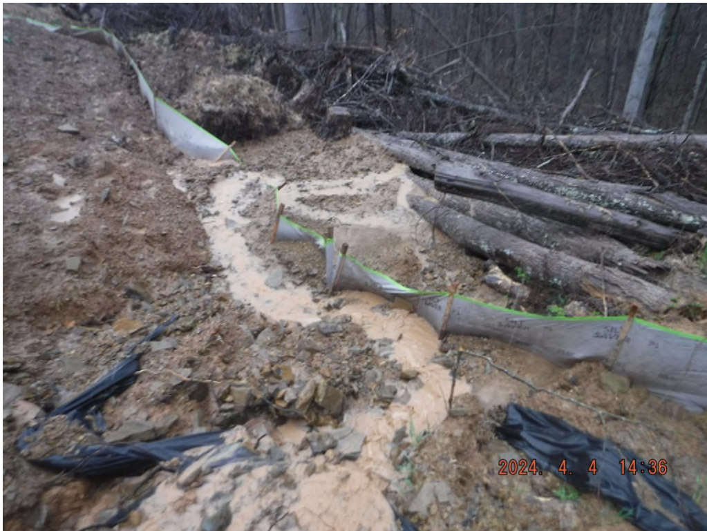
Photo # DSCF3942: BMPs lacking maintenance and sediment laden water leaving the ROW at or near N 39° 31.0460', W 80° 31.0529'.
