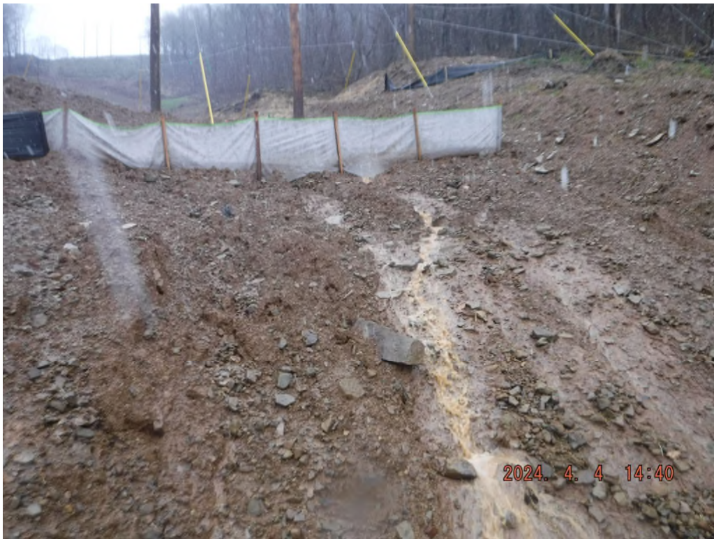
Photo # DSCF3952: BMPs lack maintenance (undercut) at station 110+00.
