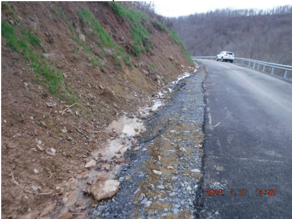
Photo # DSCF3340: Rock checks missing in roadside ditch near station 36+00.
