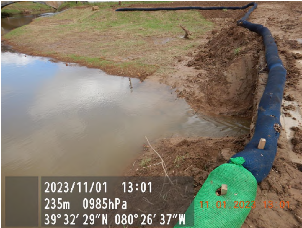
Conditions not allowable as sediment deposit on bottom of Warrior Fork ( 39° 32 '29"N, 80° 26' 37"W).
