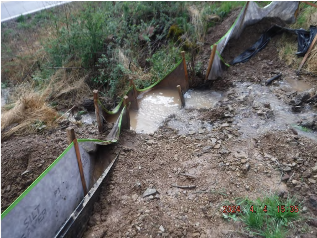
Photo # DSCF4003: Sediment deposits creating conditions not allowable in UNT Glade Fork at or near N 39° 30.5966', W 80° 29.8266'.
