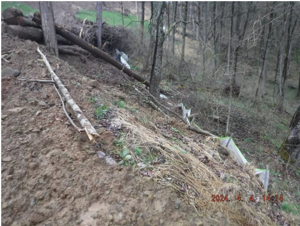
Photo # DSCF3902: Silt fence lacks maintenance at or near N 39° 31.0547', W 80° 30.8078.
