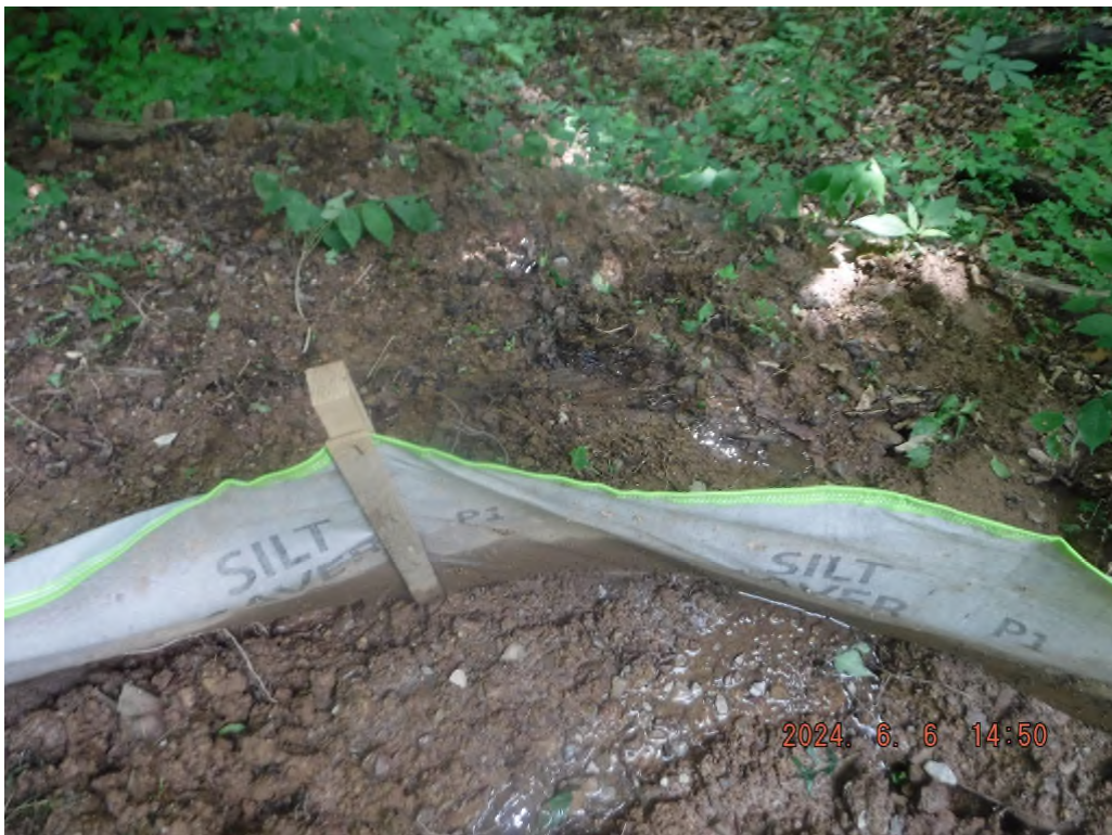
Photo # DSCF5521: Sediment laden water leaving the existing access road found on drawing sheet 2 of the approved SWPPP.
