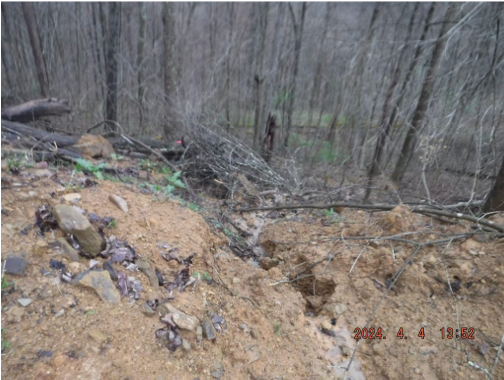
Photo # DSCF3870: Sediment laden water leaving the existing access road on sheets 2 and 3 from Pickenpaw Rd. at or near N 39° 30.9827', W 80° 30.5636'.
