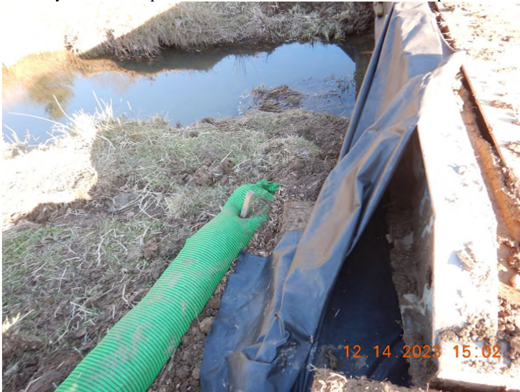
Perimeter controls were not tied to the bridge correctly, creating bypasses in the controls.
