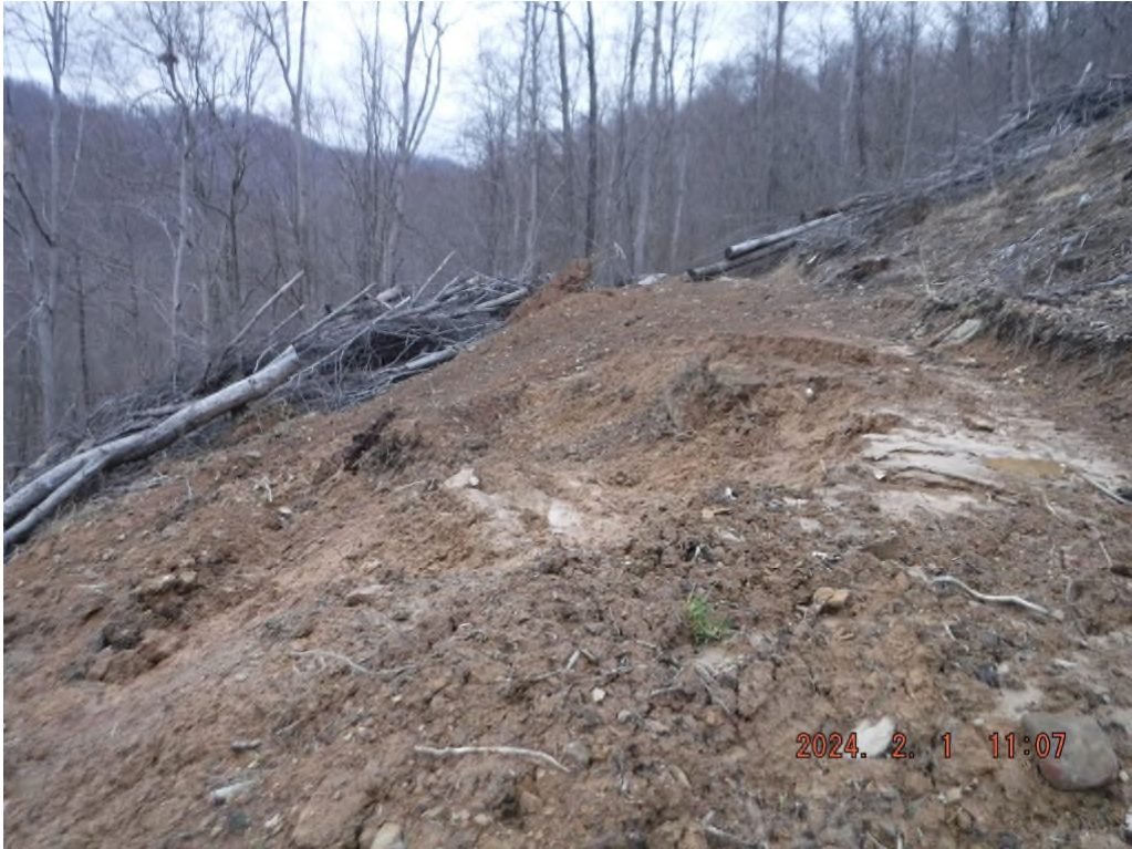
Photo # DSCF1572: Slip in disturbed area off LOD at or near station 145+00.
