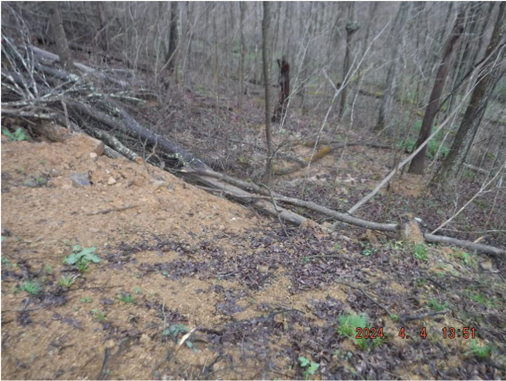
Photo # DSCF3867: Sediment laden water leaving the existing access road on sheets 2 and 3 from Pickenpaw Rd. at or near N 39° 30.9805', W 80° 30.5575'.
