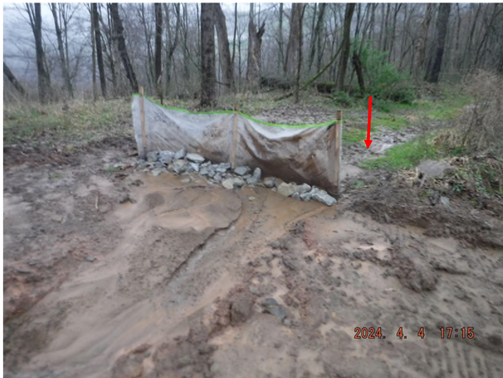
Photo # DSCF4153: Sediment laden water leaving the proposed access road on sheet 1 at or near N 39° 30.4346', W 80° 29.3473'.
