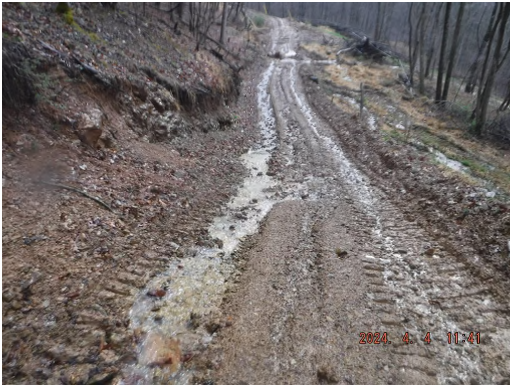
Photo # DSCF3727: Proposed access road on drawing sheet 3 of the approved SWPPP lacks stabilization and BMPs.
