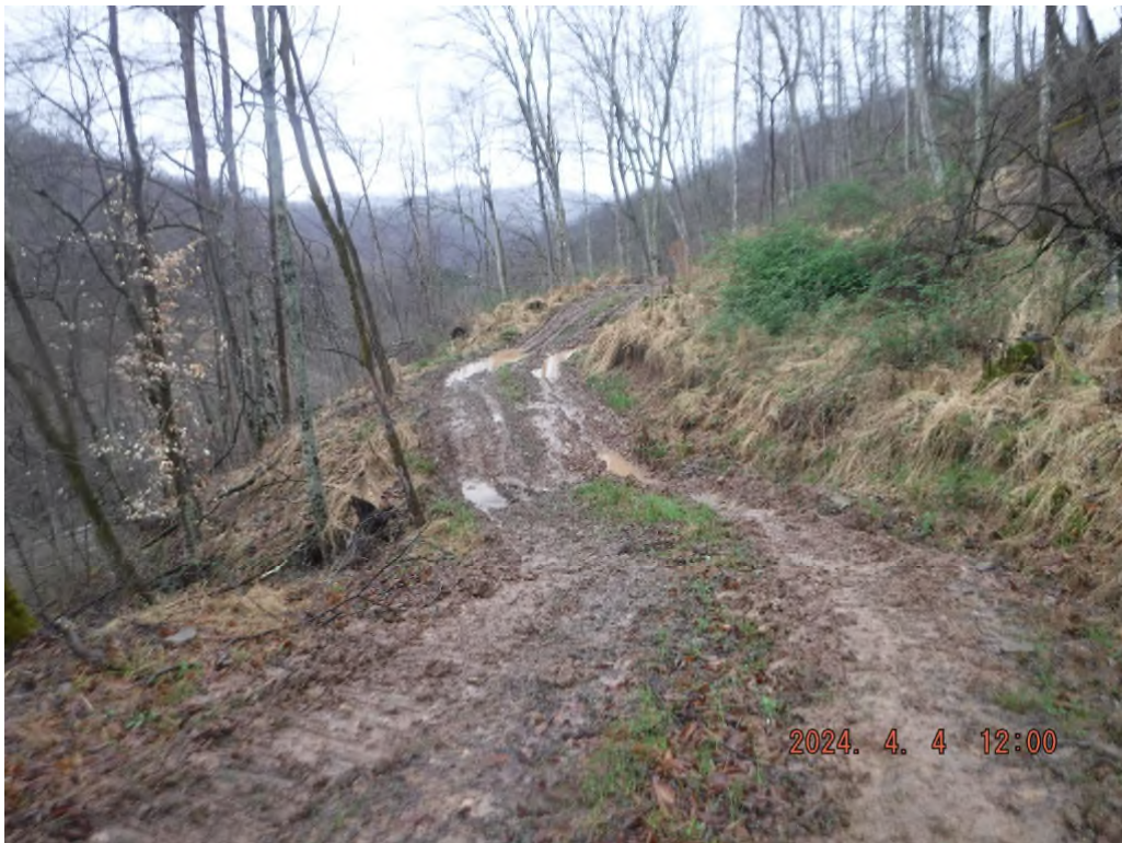
Photo # DSCF3774: Unpermitted access road at or near N 39° 31.0736', W 80° 30.3038' that lacks stabilization and BMPs.
