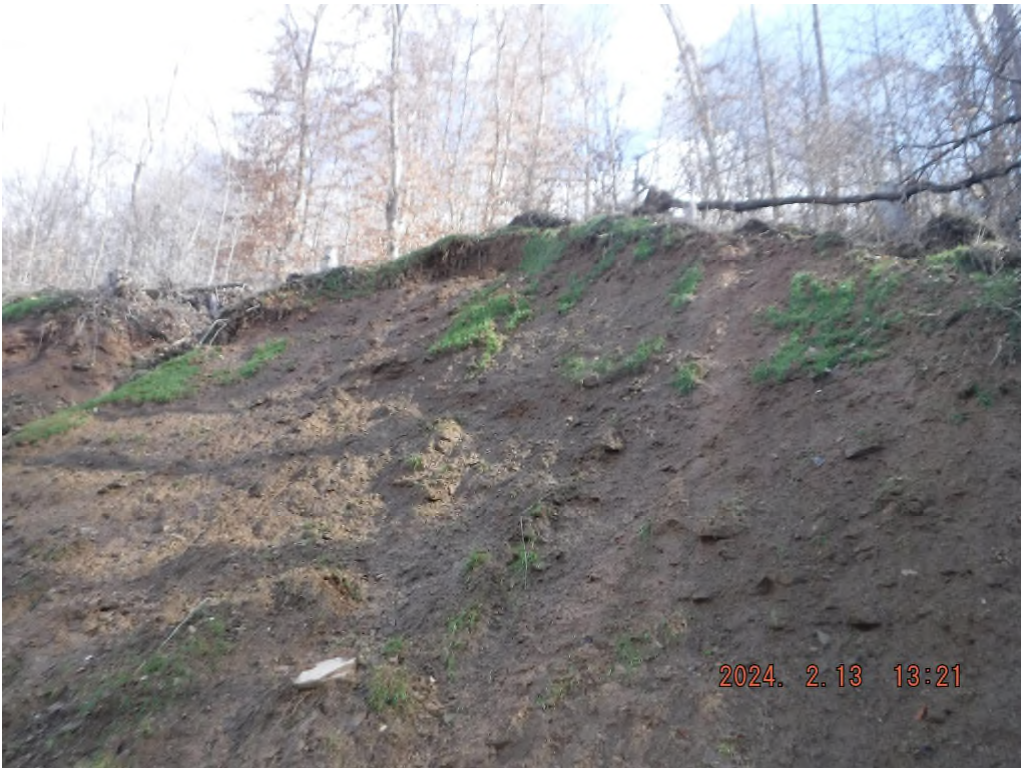
Photo # DSCF2119: Slope above the inlet lacking inlet protection at station 20+00.
