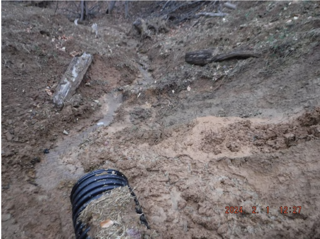
Photo # DSCF1700: Sediment off LOD leading to a UNT near station 110+00.
