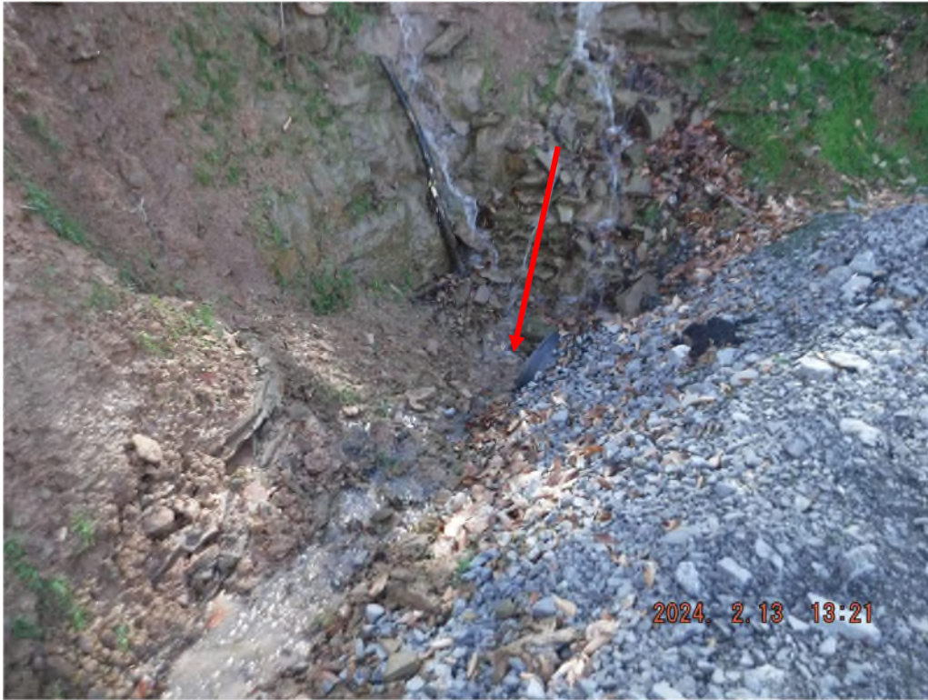
Photo # DSCF2118: No inlet protection at or near station 20+00.
