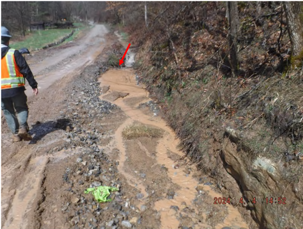
Photo # DSCF3981: Sediment laden water from unpermitted access road at station 115+00 entering a culvert (red arrow) along Buck Run Rd.
