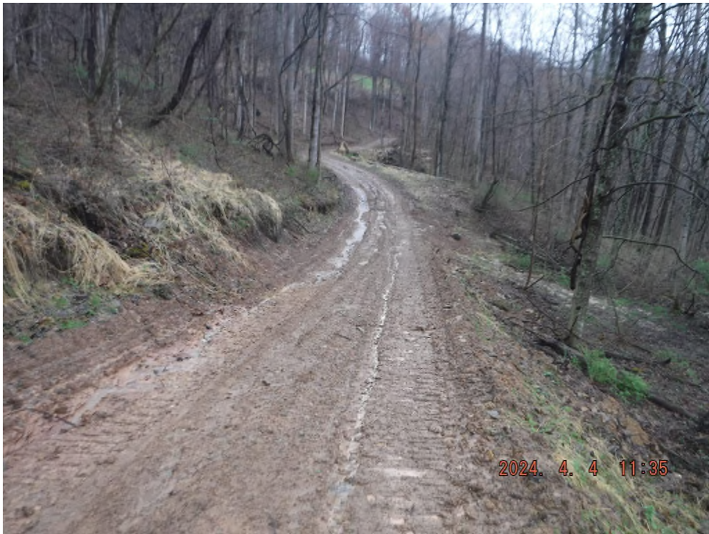
Photo # DSCF3700: Proposed access road on drawing sheet 3 of the approved SWPPP lacks stabilization and BMPs.
