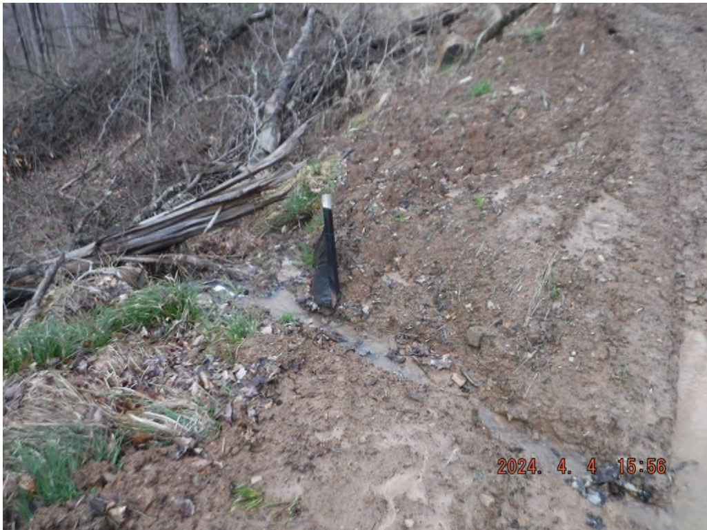
Photo # DSCF4040: Sediment laden water leaving the proposed access road on drawing sheet 2 at or near N 39° 30.8158', W 80° 29.8998'. Note lack of maintenance on the incorrect silt fence.
