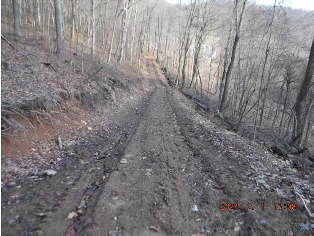
Photo # DSCF1889: Proposed access road on drawing Sheet 1 lacks stabilization.
