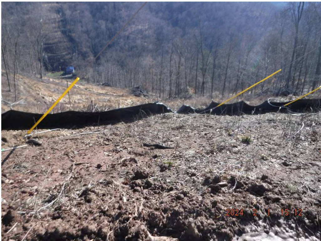
Photo # DSCF1830: Incorrect BMPs installed which lack maintenance at or near station 47+00. The SWPPP calls for BSRF or super silt fence.
