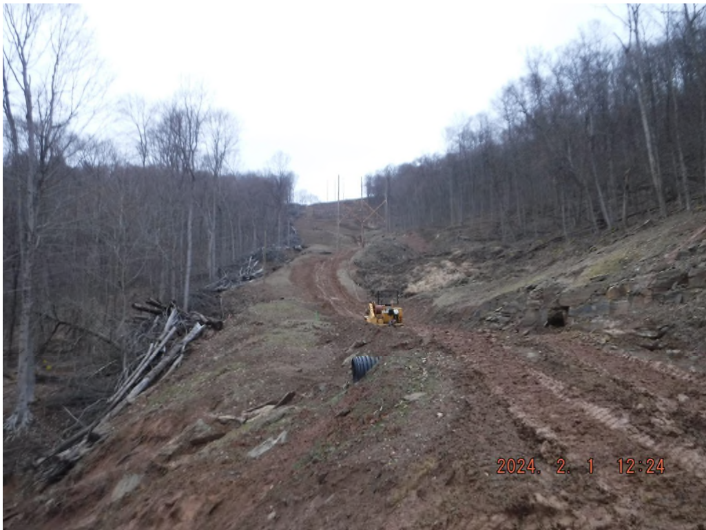
Photo # DSCF1694: Unpermitted disturbance off the LOD in the powerline ROW between stations 112+00 and 100+00. No BMPs installed.
