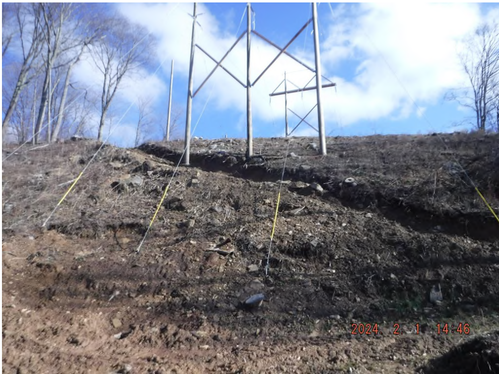
Photo # DSCF1798: Area missing BMPs (BSRF or super silt fence) at or near station 63+00.
