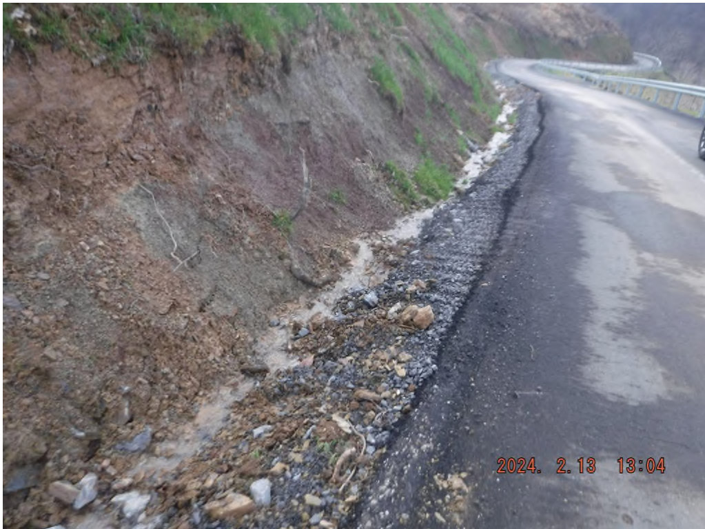
Photo # DSCF2067: Area between stations 30+00 and 32+00 that lacks rock check dams.
