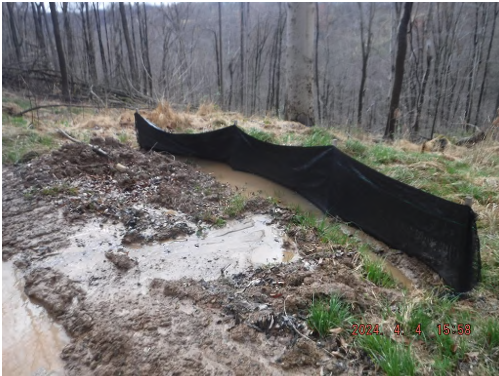
Photo #DSCF4045: Incorrect silt fence along the proposed access road on drawing sheet 2 of the approved SWPPP.
