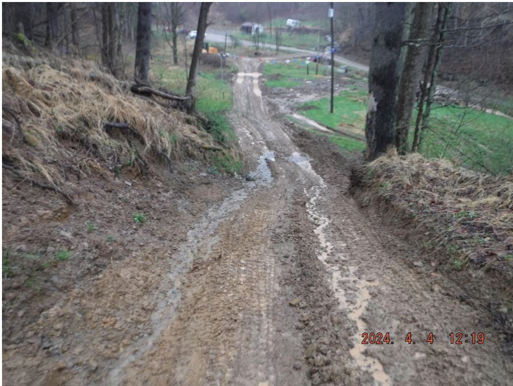
Photo # DSCF3812: Unpermitted access road to Buck Run that lacks stabilization and BMPs.
