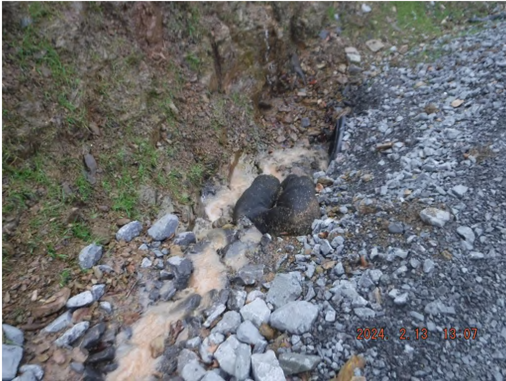
Photo # DSCF2076: Inlet protection lacks maintenance at or near station 29+20.
