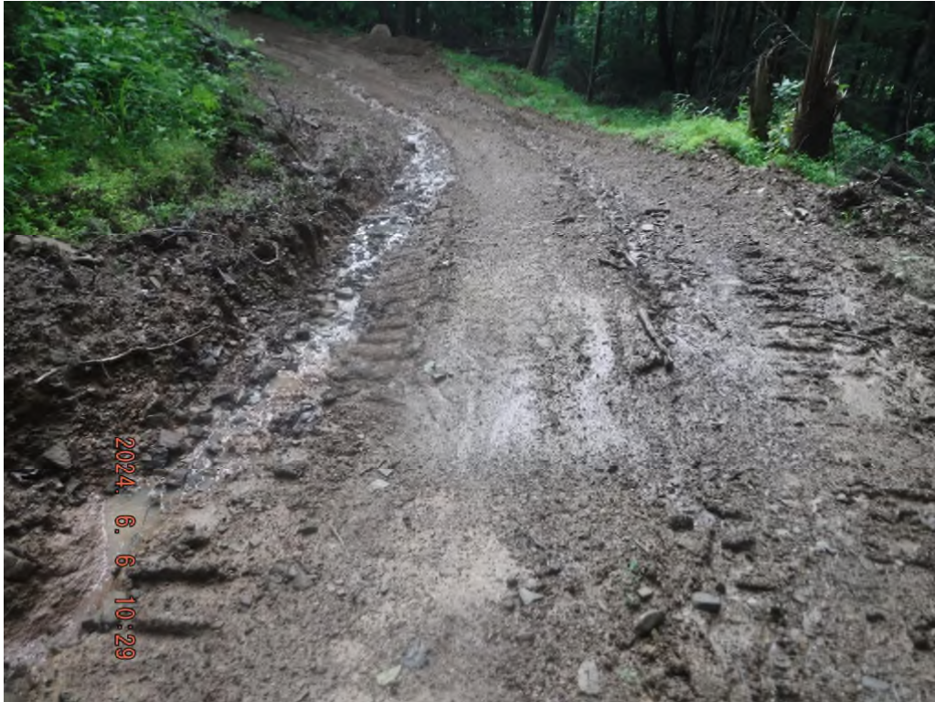
Photo # DSCF5217: Erosion rilling starting on the proposed access road found on sheets 3 and 4 of the SWPPP drawings.
