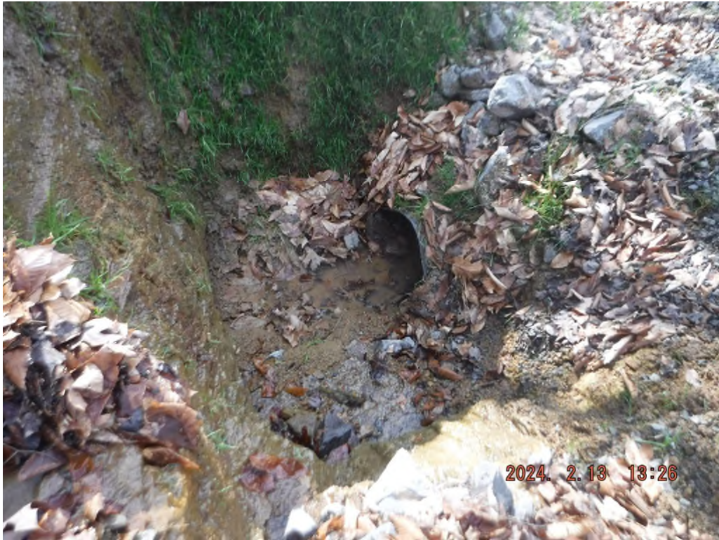
Photo # DSCF2128: No inlet protection present at or near station 15+50.
