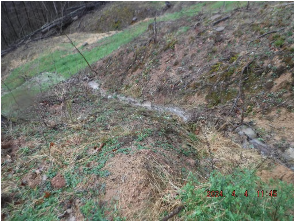
Photo # DSCF3737: Sediment laden water leaving from the ROW between stations 120+00 and 125+00 at or near N 39° 30.9457', W 80° 31.4481'.
