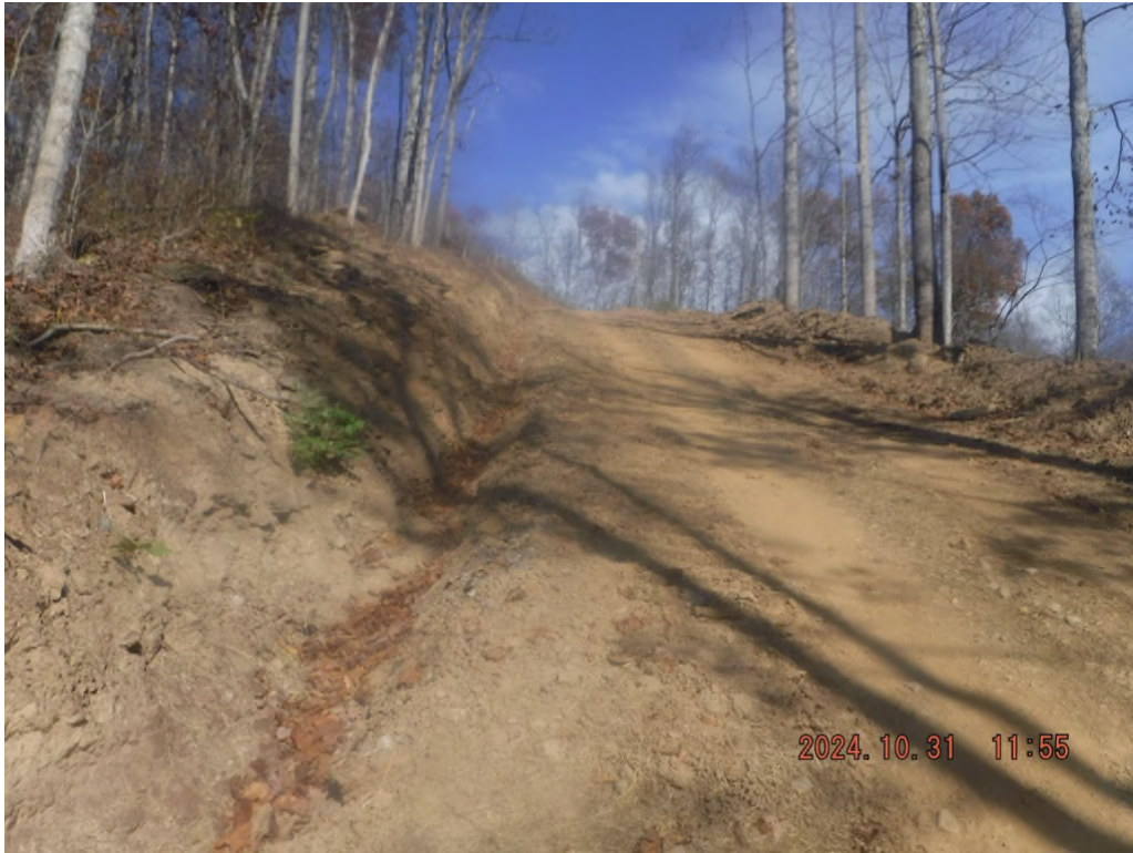
Photo # DSCF0026: Access road beginning at station 75+00 from Pickenpaw Rd. lacks water bars/cross culverts, ditch checks, and a graveled surface as outlined on the detail sheet (sheet 3.0) of the approved SWPPP drawing.
