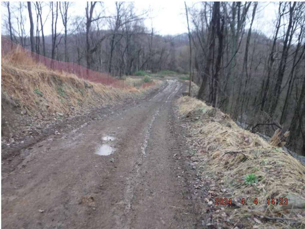
Photo # DSCF3913: Unpermitted access road between Buck Run Rd. and Pickenpaw Rd. at or near N 39° 31.0950', W 80° 30.9033' that lacks stabilization and BMPs.
