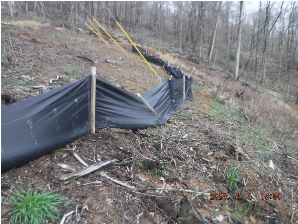
Photo # DSCF4030: Incorrect BMPs installed at station 48+00 at or near N 39° 30.7266', W 80° 29.9277'.
