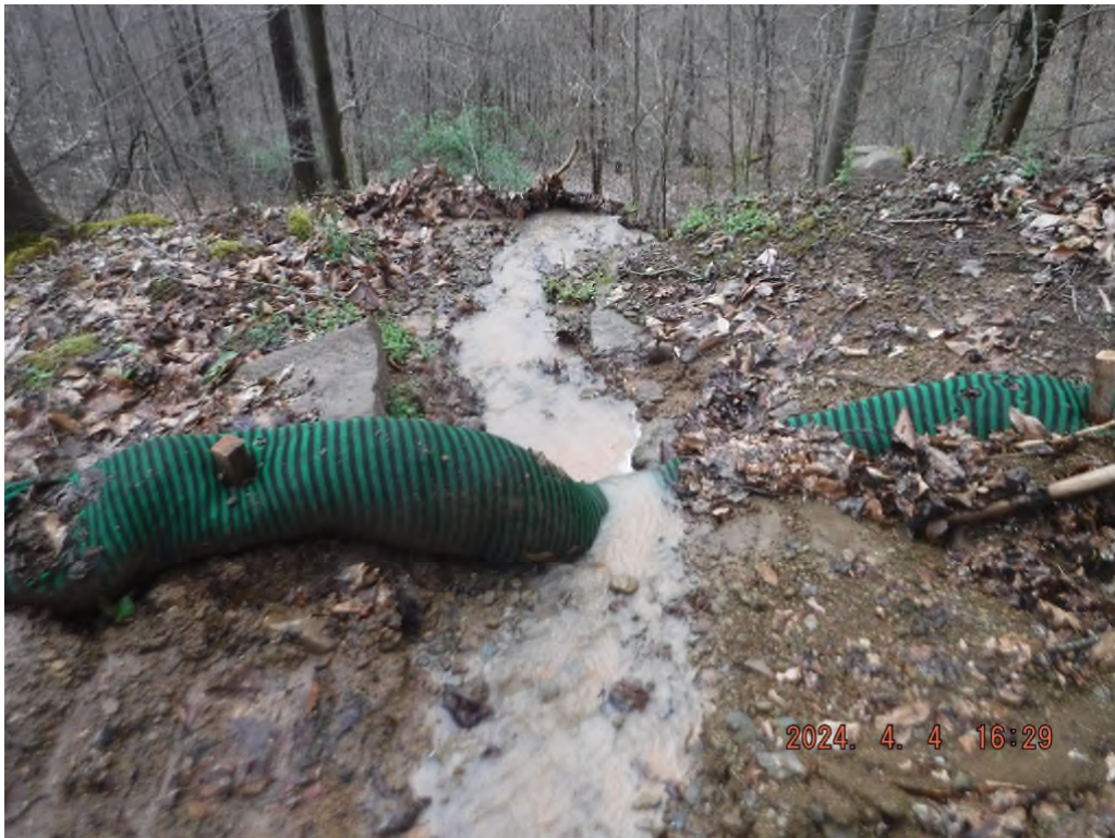
Photo # DSCF4111: Sediment laden water leaving the existing access road on sheet 2 at or near N 39° 30.5328', W 80° 30.4918'.
