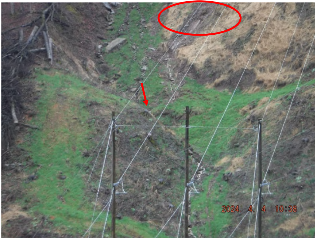
Photo # DSCF3640: Slip (circled) and material (arrow) entering UNT Price Run at or near N 39° 30.7218', W 80° 31.9736'.
