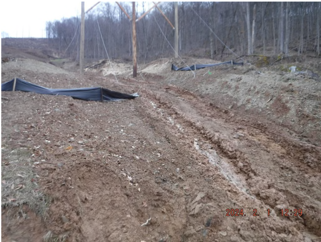
Photo # DSCF1704: BMPs at or near station 110+00 lacked maintenance and are not the BMPs detailed in the SWPPP.
