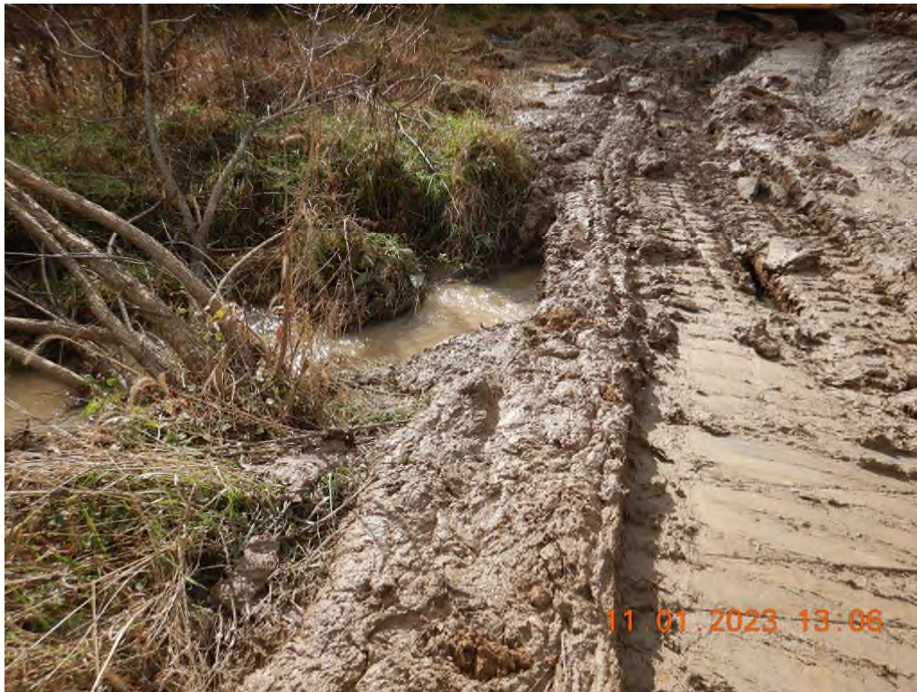
Air bridge over Buffalo Creek in the middle of the project with no controls in place.
