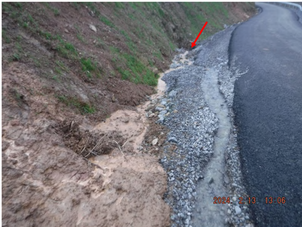
Photo # DSCF2075: Slip in ditch A-6 at or near station 29+25. Inlet for culvert to ephemeral 8 denoted by red arrow.
