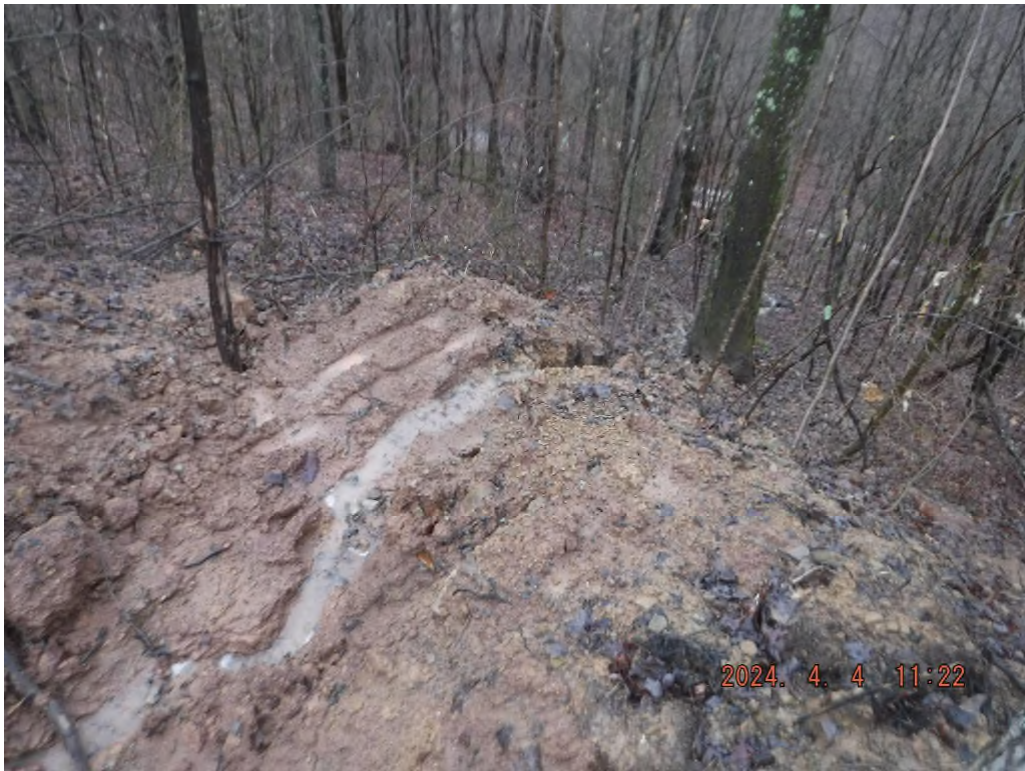
Photo # DSCF3681: Sediment laden water leaving unpermitted access road at or near N 39° 30.7677', W 80° 31.7202'.
