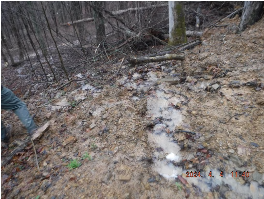
Photo # DSCF3725: Sediment laden water leaving the proposed access road on sheet 3 at or near N 39° 30.9749', W 80° 31.5214'.
