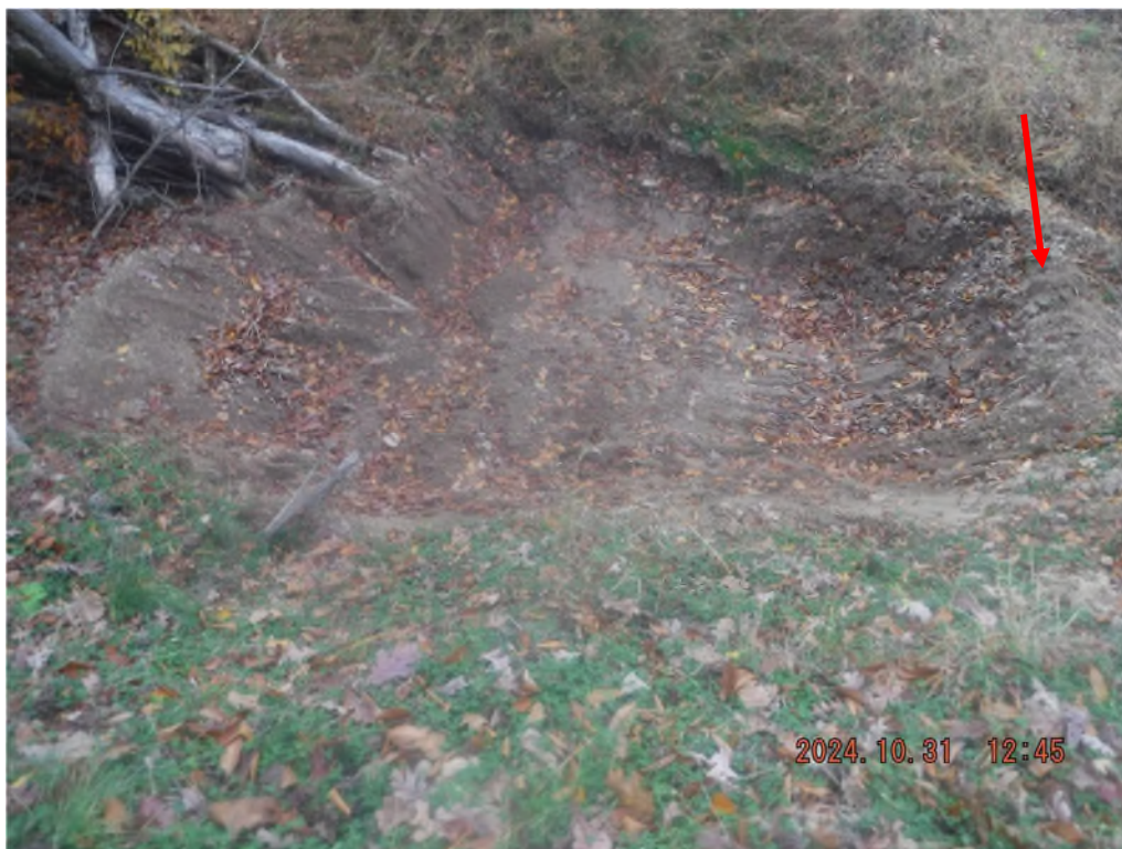
Photo # DSCF0077: Sediment deposit (red arrow) from digging a large sump in UNT Buck Run at or near 39° 31 '01.2"N 80° 31' 11.8"W.
