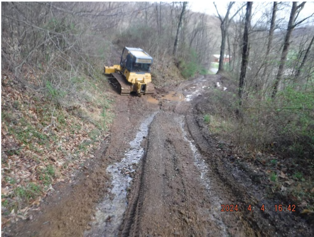
Photo # DSCF4137: Existing access road on sheet 2 lacks stabilization and BMPs.
