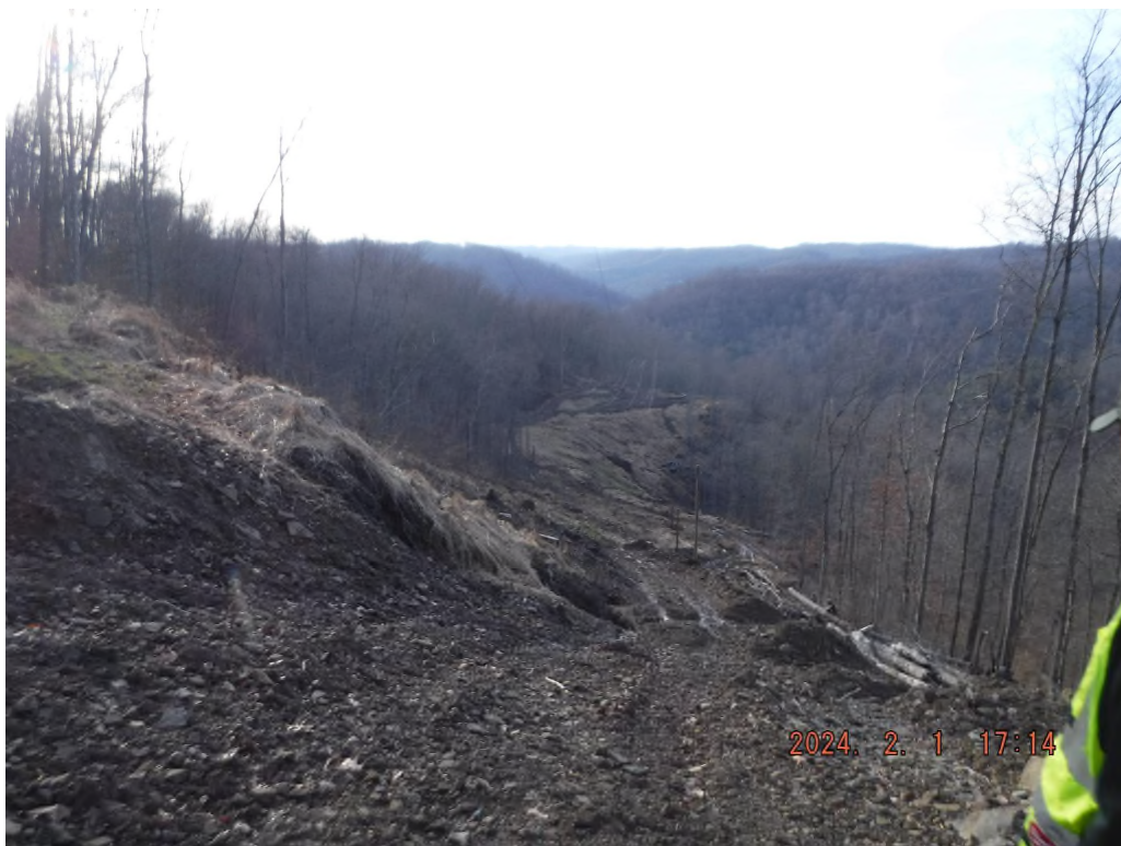
Photo # DSCF1894: Disturbed area outside of the LOD between station 12+00 and 25+00
