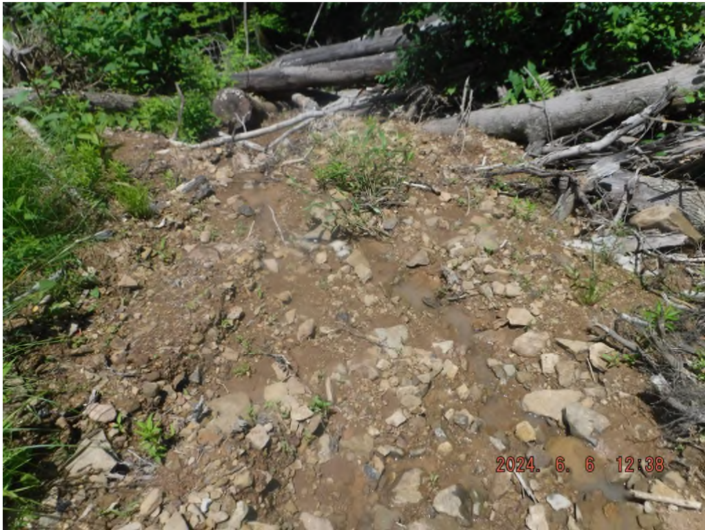
Photo # DSCF5366: Sediment laden water leaving the site near station 104+50 at or near N 39° 31.0509', W 80° 31.0313'.
