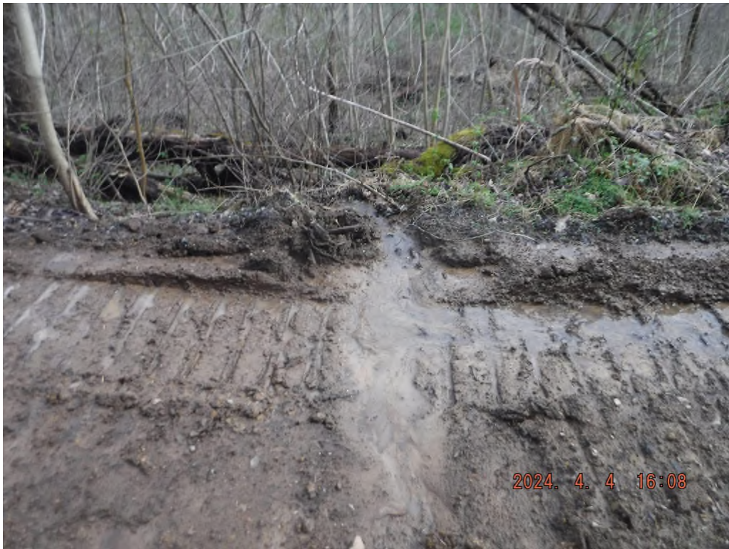
Photo # DSCF4067: Sediment laden water leaving the proposed access road on drawing sheet 2 at or near N 39° 30.8552', W 80° 30.1391'.
