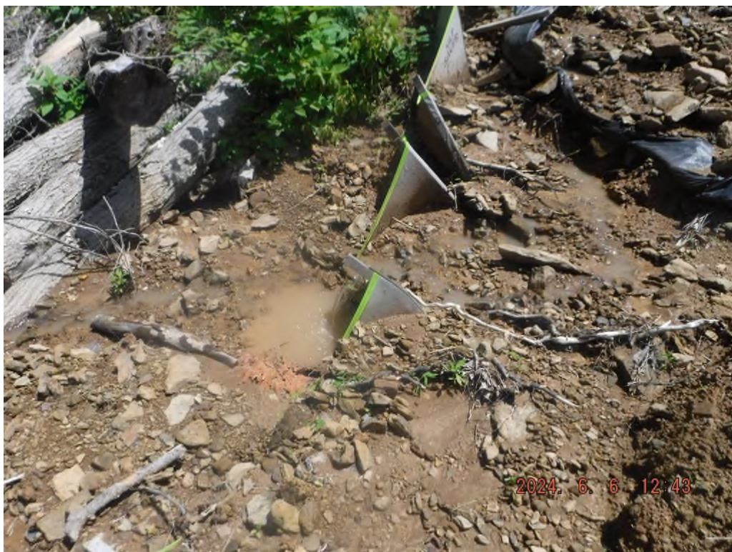
Photo # DSCF5374: silt fence lacks maintenance and sediment laden water leaving the site at station 110+00 at or near N 39° 31.0430', W 80° 31.0574'.
