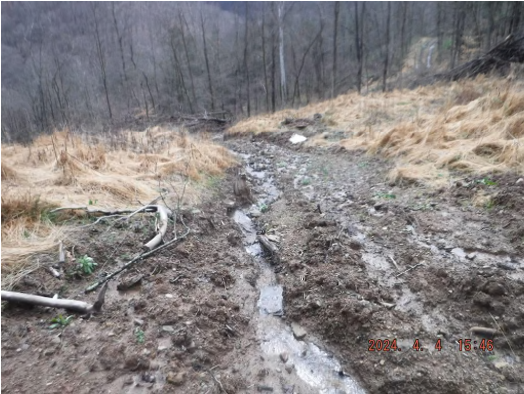
Photo # DSCF4024: Disturbed travel lane in ROW between stations 40+00 and 47+00. No BMPs installed.
