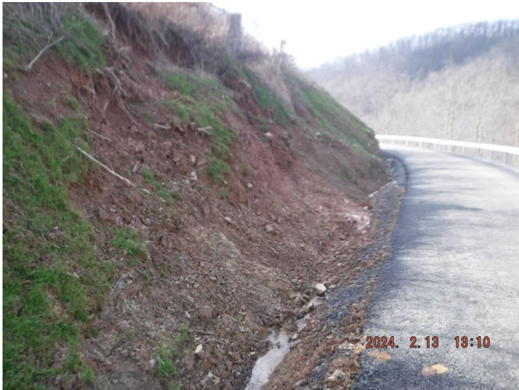
Photo # DSCF2087: Fill material in ditch near station 28+00.
