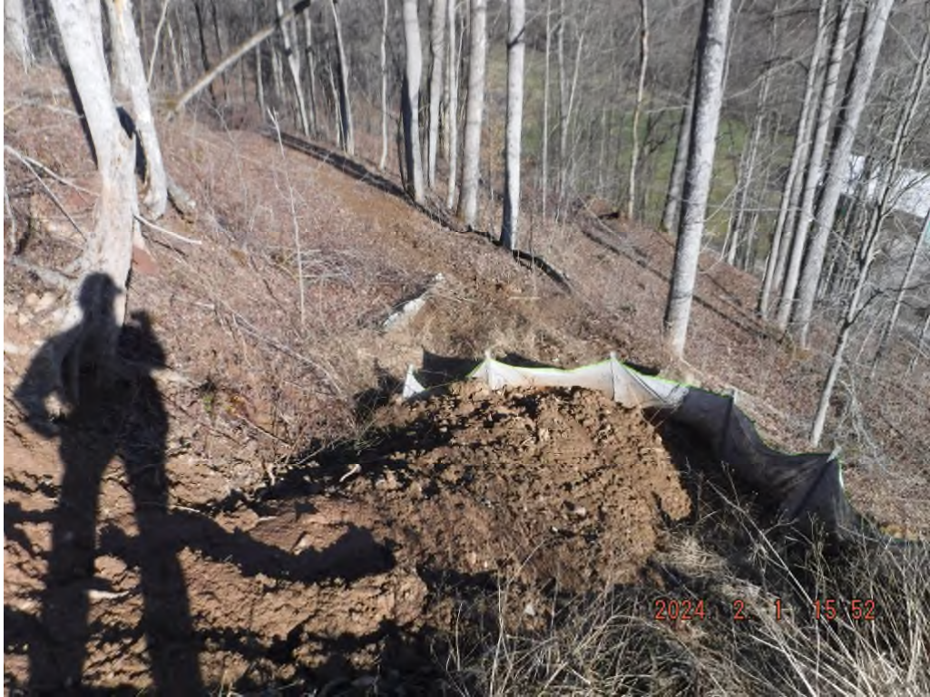
Photo # DSCF1861: BMPs lack maintenance between stations 75+00 and 80+00.
