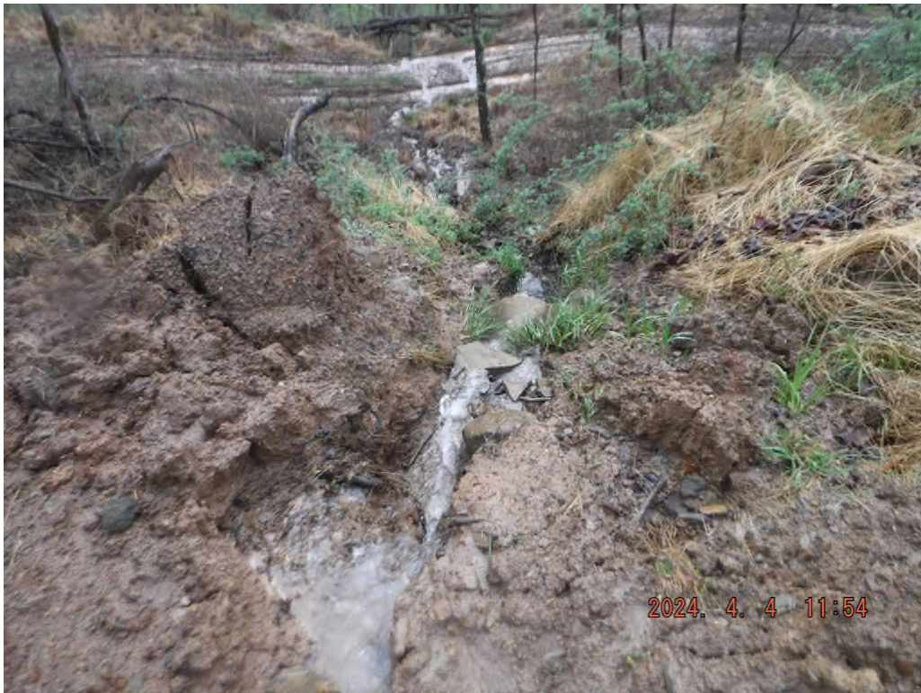
Photo # DSCF3757: Sediment laden water leaving the unpermitted access road to Buck Run Rd. at or near N 39° 31.0243', W 80° 31.3335'.
