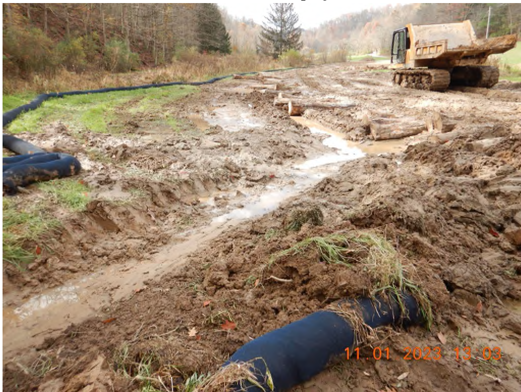
A diversion ditch was cut directly into Buffalo Creek with no erosion sediment controls in place.
