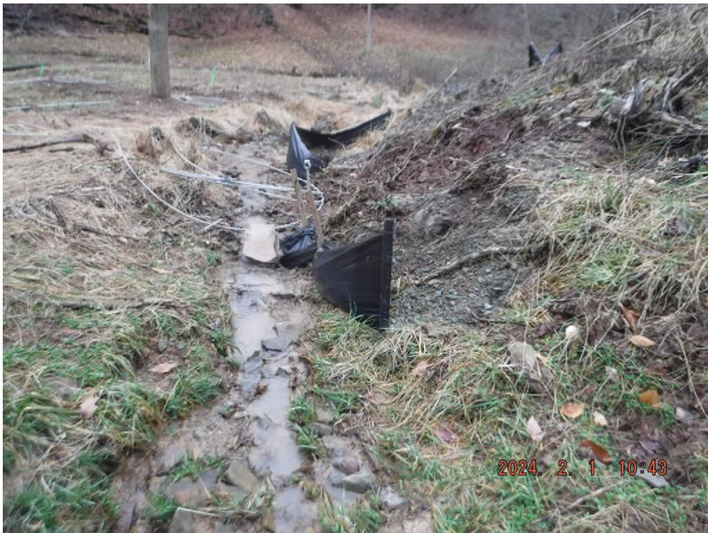
Photo # DSCF1531: Sediment laden water and non-maintained BMPs. The BMPs are not installed as detailed in the SWPP.
