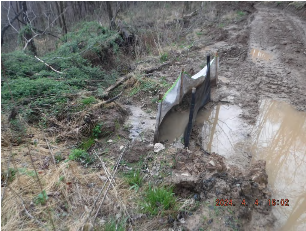
Photo # DSCF4056: Sediment laden water leaving the proposed access road on drawing sheet 2 at or near N 39° 30.9030', W 80° 29.9669'.
