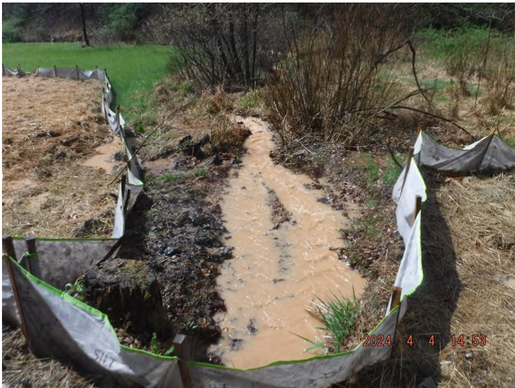
Photo # DSCF3983: Sediment laden water exiting culvert on Buck Run Rd. in UNT Buck Run.
