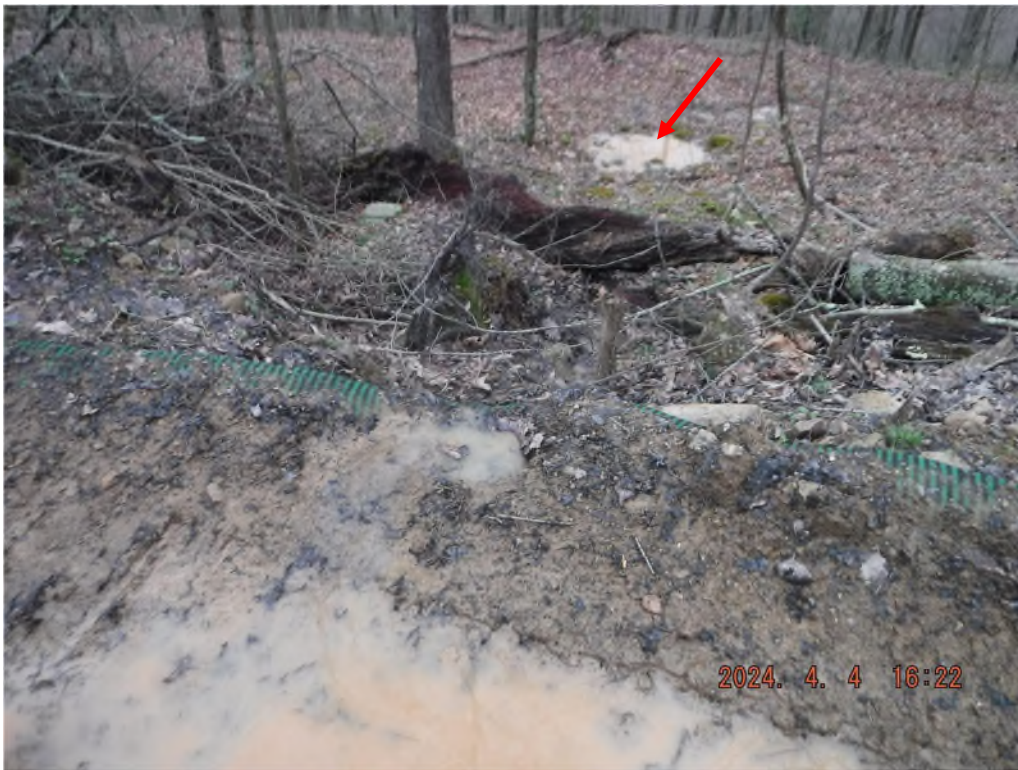
Photo # DSCF4102: Sediment laden water leaving the existing access road on sheet 2 at or near N 39° 30.6554', W 80° 30.3161'
