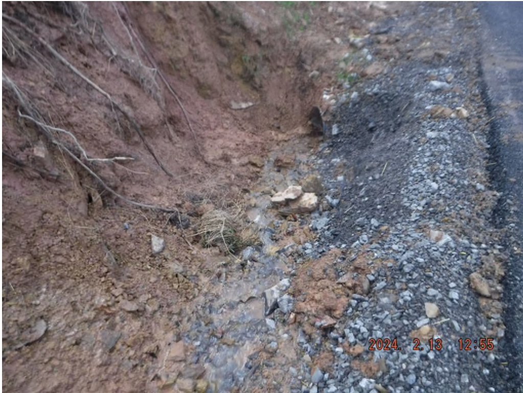
Photo # DSCF2042: No inlet protection present at the culvert inlet for Ephemeral 11 at or near station 37+00.
