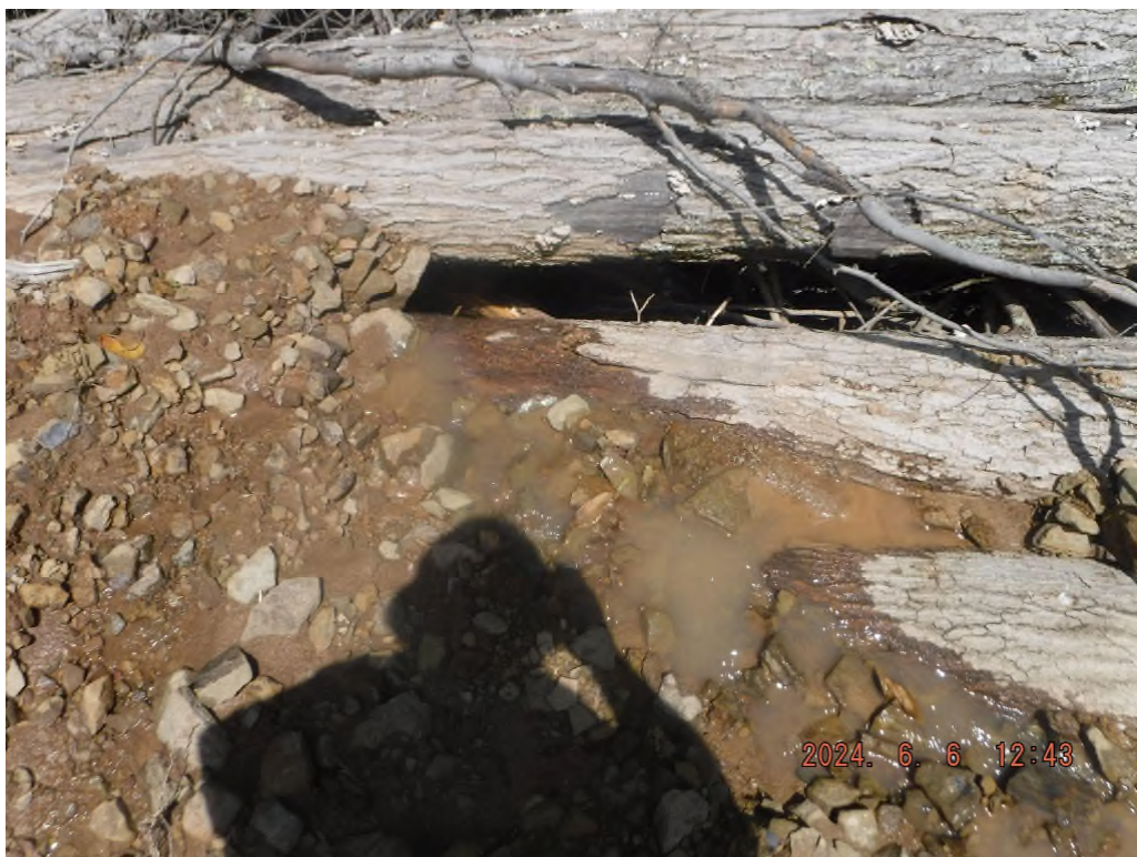
Photo # DSCF5377: Sediment laden water leaving the site at station 110+00 at or near N 39° 31.0430', W 80° 31.0574'.
