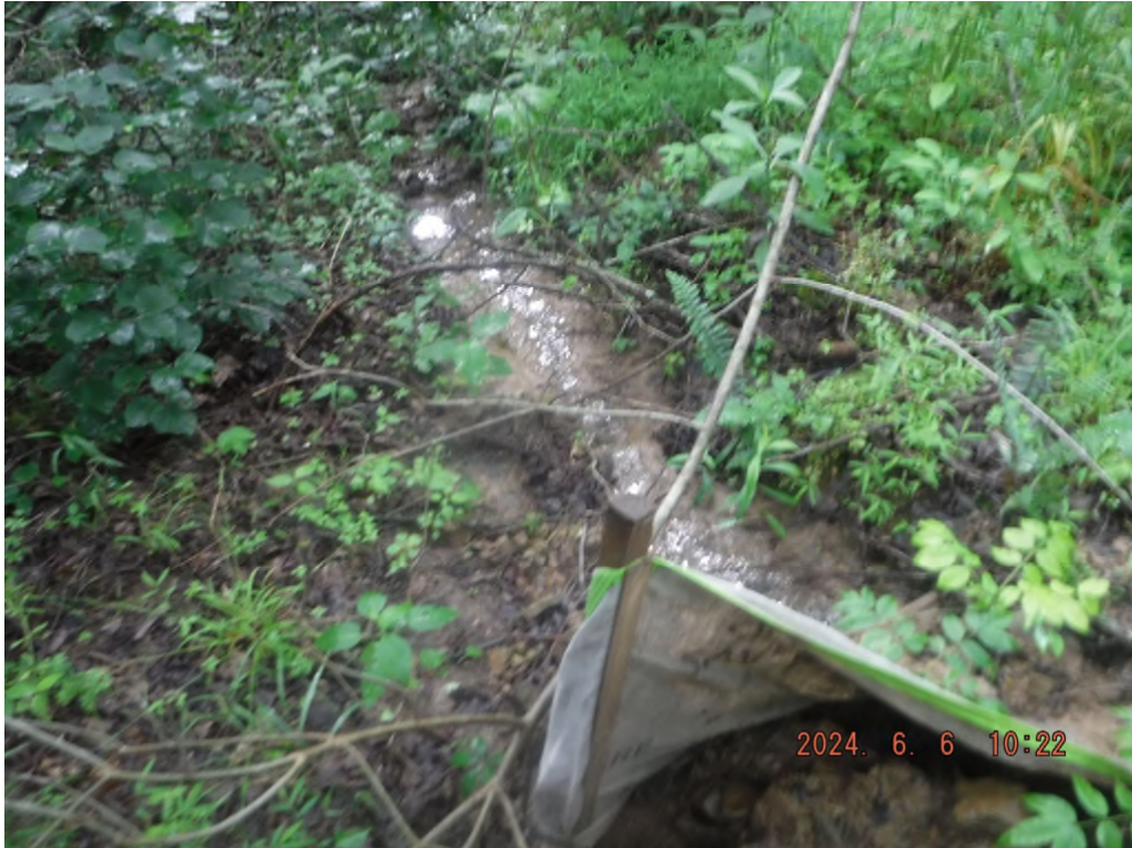
Photo # DSCF5189: Sediment laden water leaving the proposed access road found on sheets 3 and 4 of the approved SWPPP drawings.
