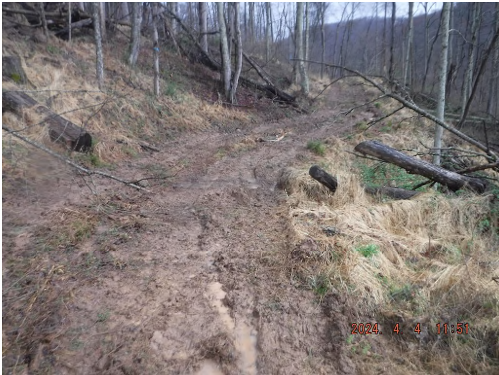
Photo # DSCF3744: Unpermitted access road at or near N 39° 30.9806', W 80° 31.3774' that leads down to Buck Run Rd. and lacks stabilization and BMPs.
