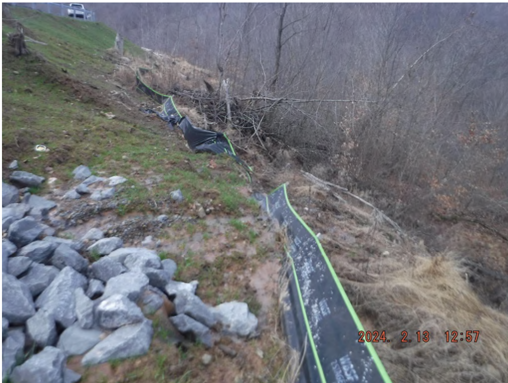
Photo # DSCF2052: Silt fence lacks maintenance below stormwater discharge point 11.
