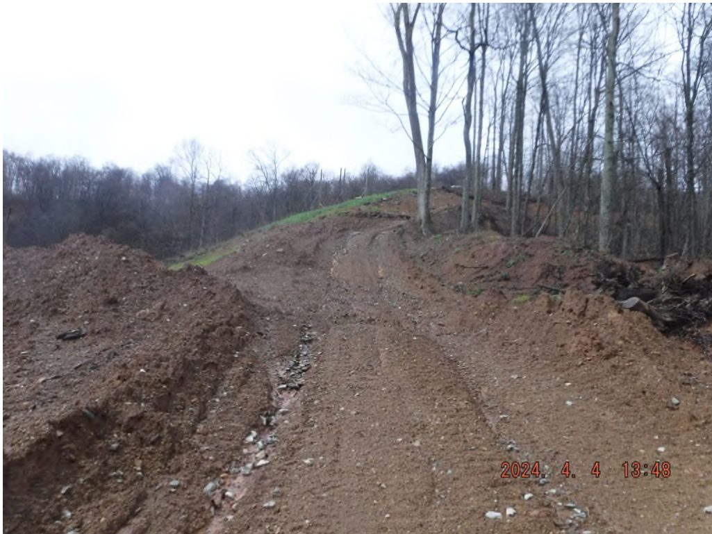
Photo # DSCF3858: Existing access road on sheets 2 and 3 from Pickenpaw Rd. lacks stabilization and BMPs.
