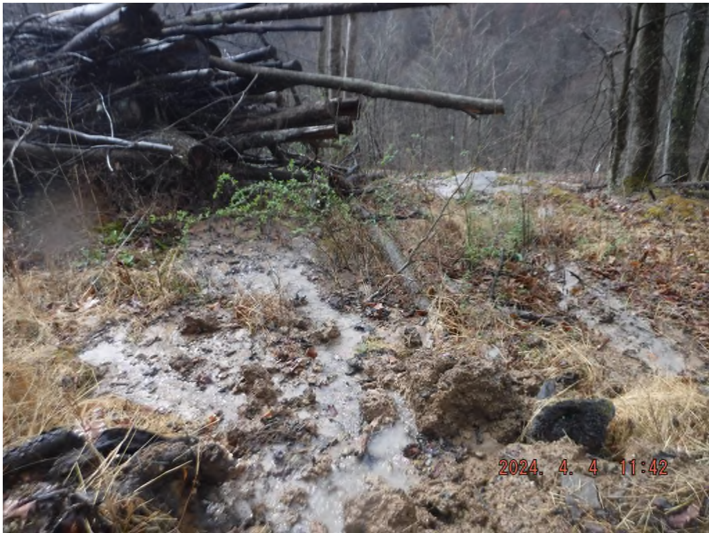
Photo # DSCF3730: Sediment laden water leaving the proposed access road on sheet 3 at or near N 39° 30.9694', W 80° 31.4477'.
