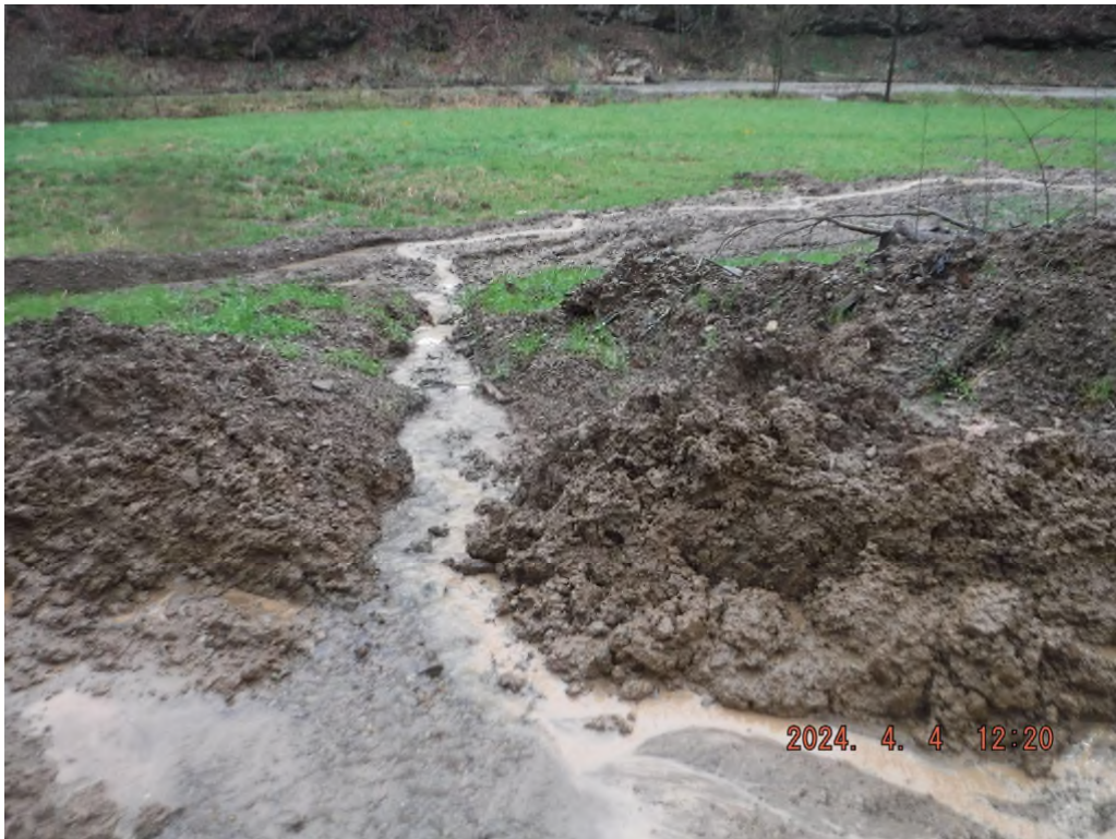
Photo # DSCF3813: Sediment laden water leaving the unpermitted access road to Buck Run.
