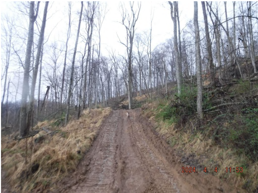
Photo # DSCF3751: Unpermitted access road at or near N 39° 30.9806', W 80° 31.3774' that leads down to Buck Run Rd. and lacks stabilization and BMPs.
