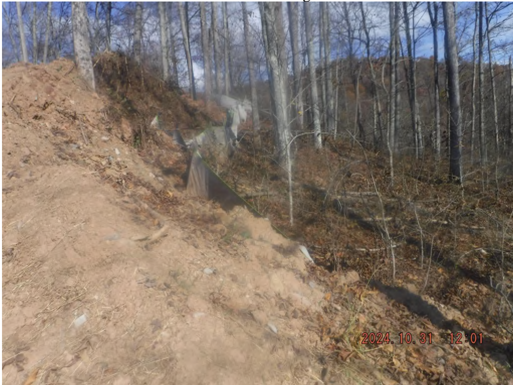
Photo # DSCF0034: Silt fence lacks maintenance between stations 75+00 and 80+00.
