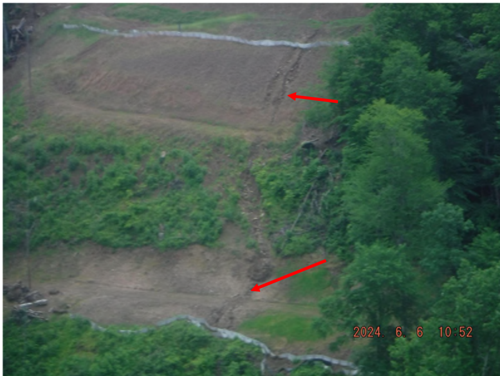
Photo # DSCF5252: Erosion rilling on the ROW between stations 115+00 and 110+00.
