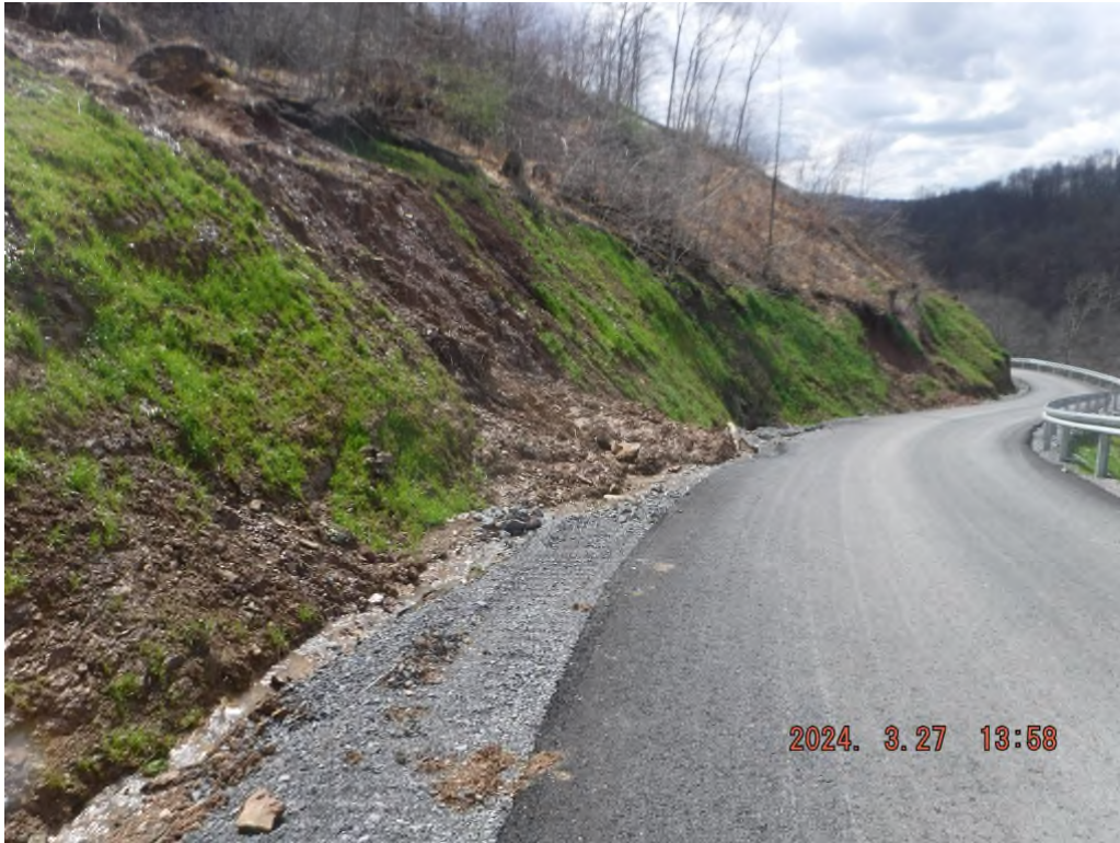
Photo # DSCF3352: Slip in roadside ditch at or near N 39° 30.7076', W 80° 32.7174'.
