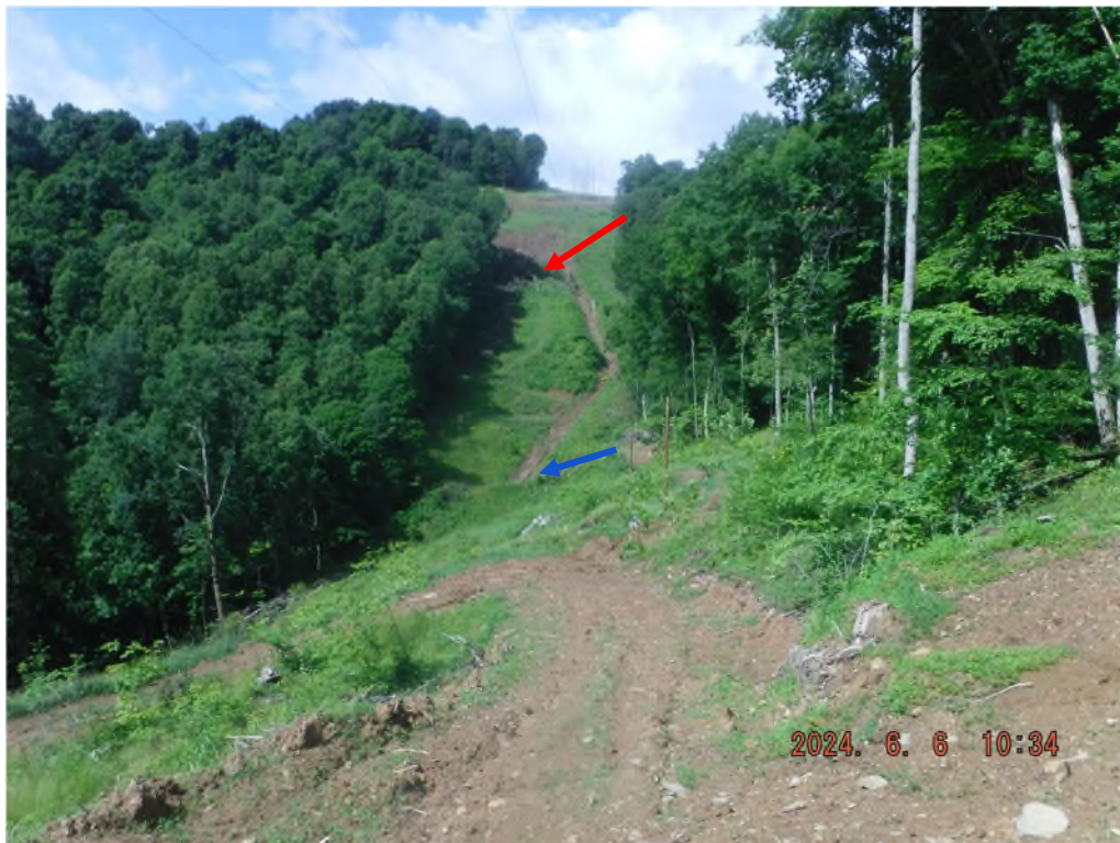
Photo # DSCF5226: Slip (red arrow) on the ROW that settled at the bottom of the slope at or near N 39° 30.9039', W 80° 31.5246' in UNT Buck Run.
