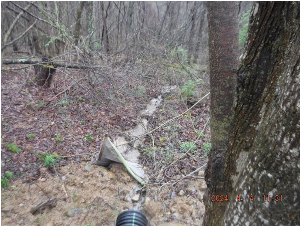
Photo # DSCF3694: Sediment laden water leaving the proposed access road on sheet 3 at or near N 39° 30.8977', W 80° 31.6754'.
