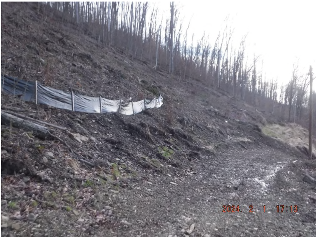
Photo # DSCF1892: Installed BMPs are not installed as detailed in the SWPPP at or near station 12+00.
