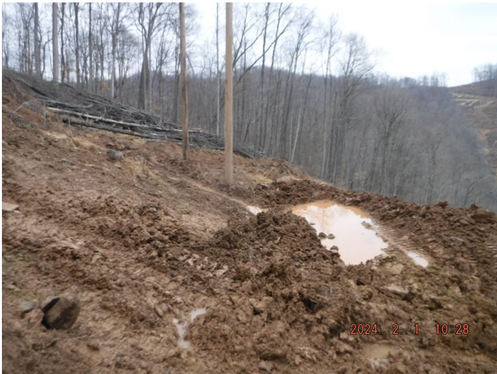
Photo # DSCF1501: Area at or near station 165+00 that is missing BMPs (BSRF or super silt fence).
