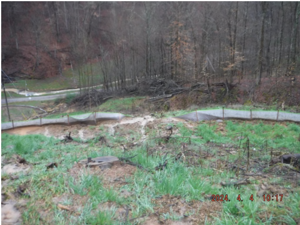
Photo # DSCF3605: BMPs lack maintenance at or near station 157+00.
