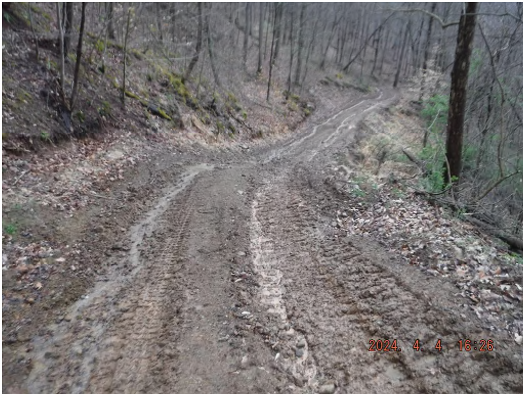
Photo # DSCF4106: Existing access road on sheet 2 lacks stabilization and BMPs.
