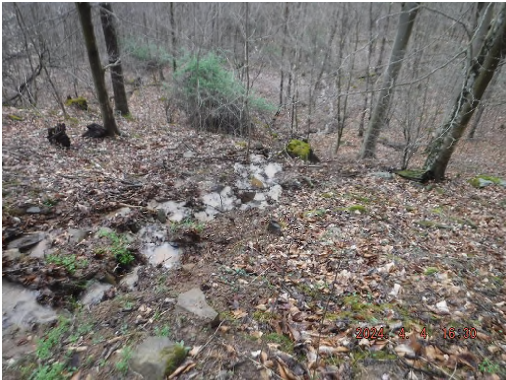
Photo # DSCF4112:Sediment laden water leaving the existing access road on sheet 2 at or near N 39° 30.5328', W 80° 30.4918'.
