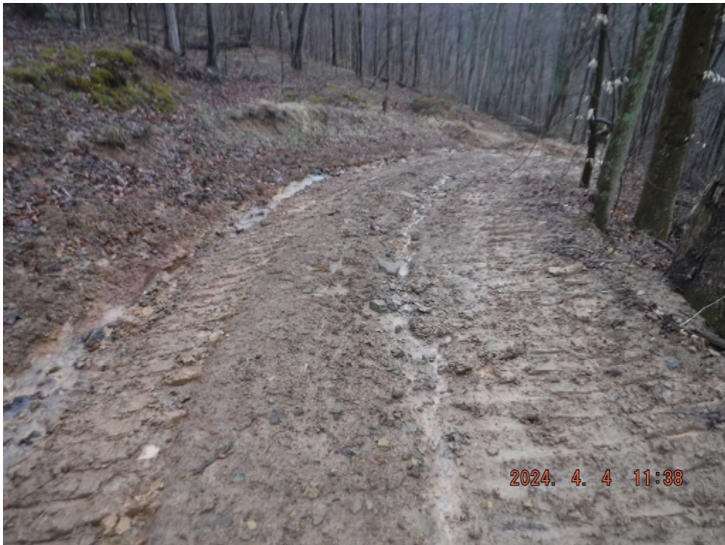
Photo # DSCF3714: Proposed access road on drawing sheet 3 of the approved SWPPP lacks stabilization and BMPs.
