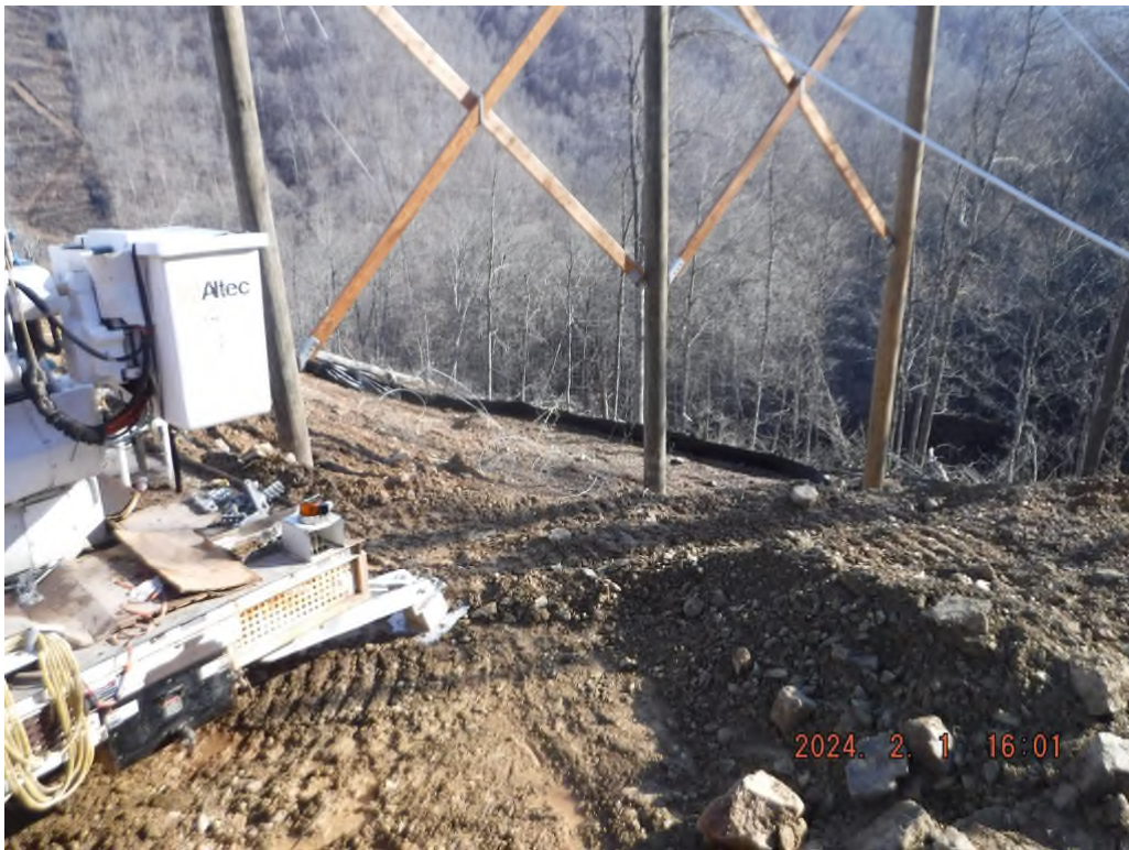
Photo # DSCF1877: BMPs are not installed as detailed in the SWPPP at or near station 80+00.
