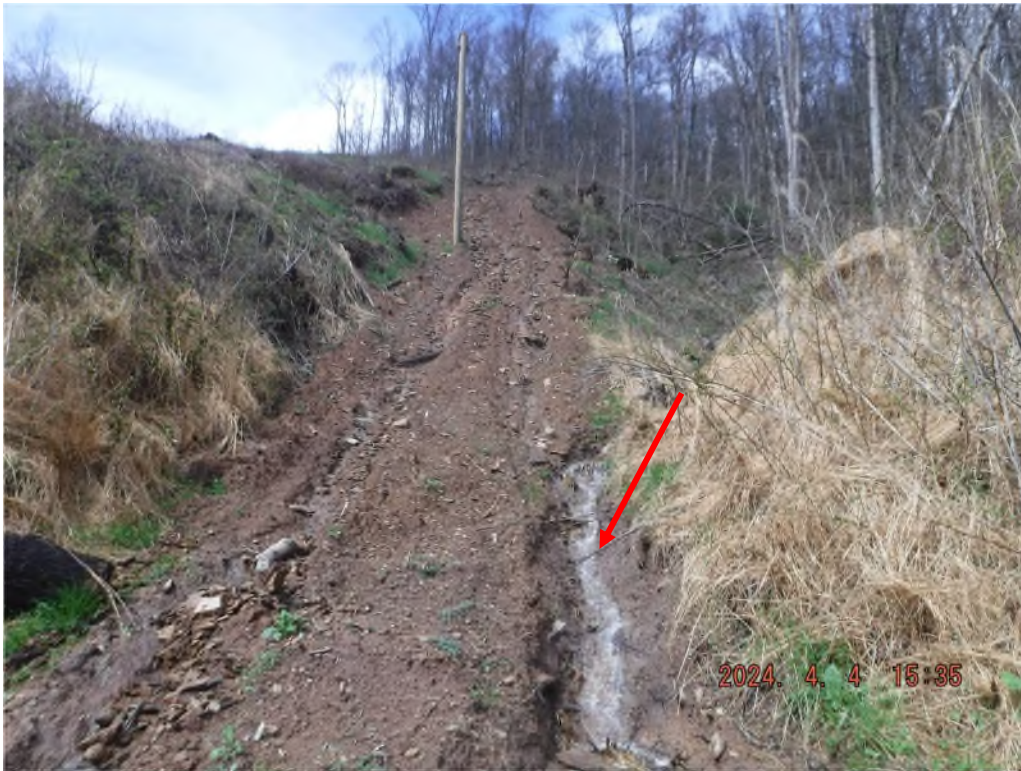
Photo # DSCF4004: Travel lane on disturbed ROW off LOD at station 39+00 with no BMPs. UNT Glade Fork noted by red arrow.
