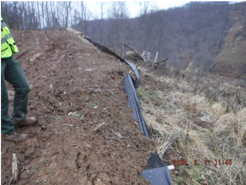
Photo # DSCF1632: Silt fence lacks maintenance at or near station 123+00 and is not the BMP (BSRF or super silt fence) described in the SWPPP.
