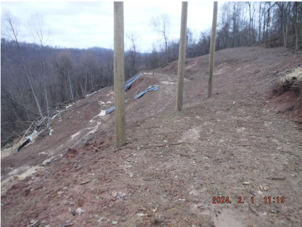
Photo # DSCF1595: Area that is missing BMPs (BSRF or super silt fence) at or near station 137+00.
