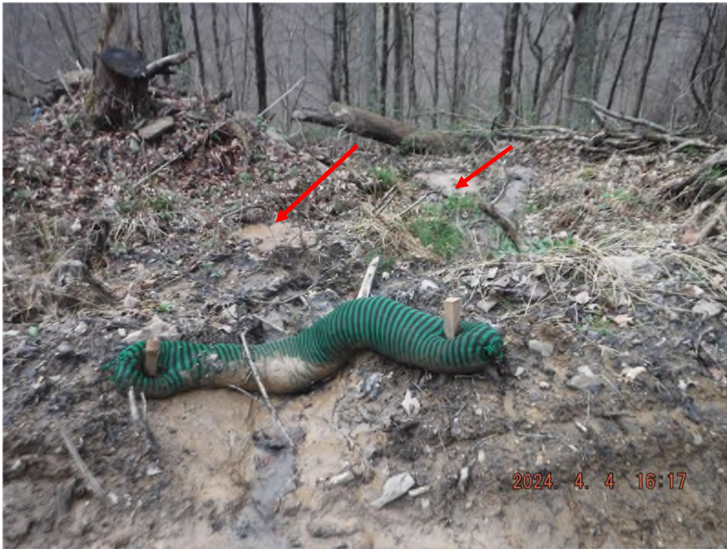
PHoto # DSCF4090: Sediment laden water leaving the existing access road on sheet 2 at or near N 39° 30.7948', W 80° 30.2454'.
