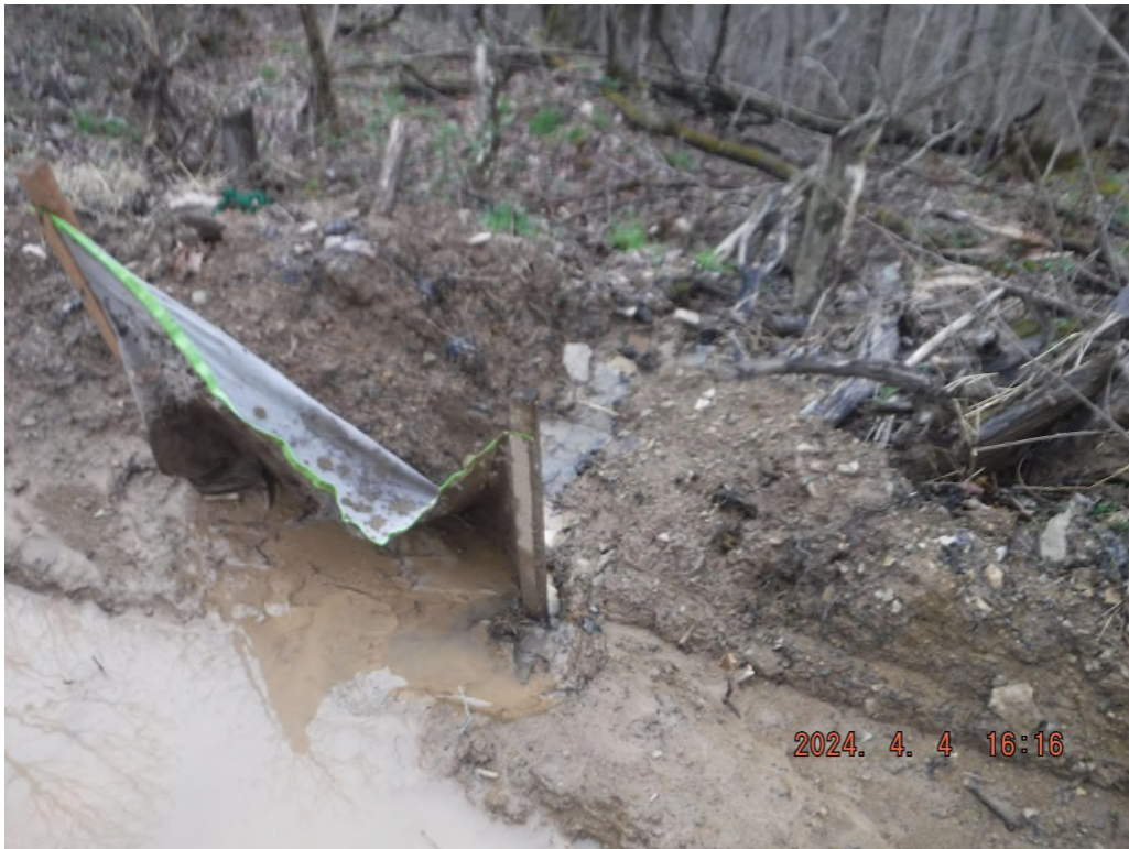
Photo # DSCF4084: Sediment laden water leaving the existing access road on sheet 2 at or near N 39° 30.8219', W 80° 30.2317'.
