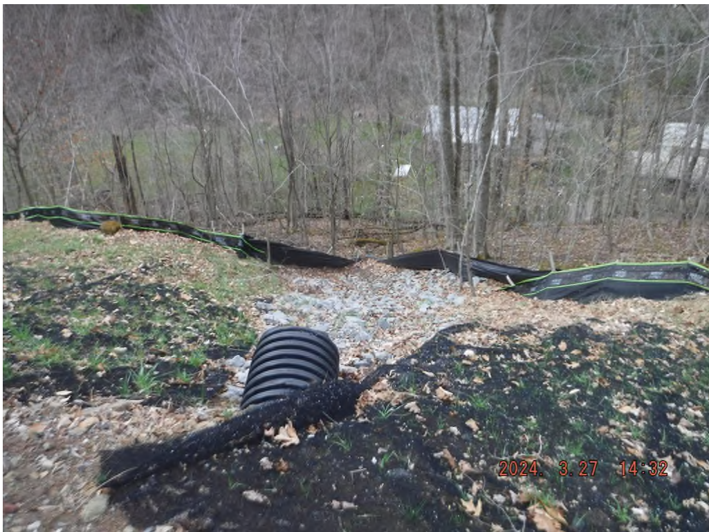
Photo # DSCF3407: Incorrect silt fence installed below discharge point 7 at station 15+50 lacks maintenance.
