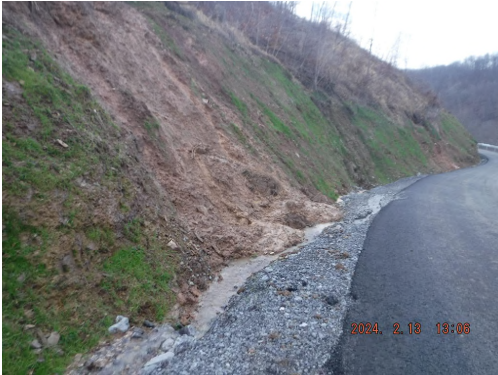
Photo # DSCF2074: Slip in ditch A-6 at or near station 29+25.
