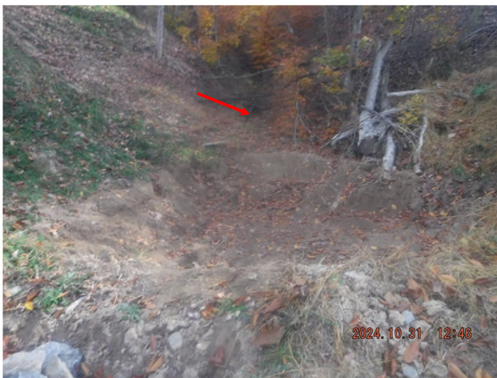
Photo # DSCF0080: Sediment deposit in UNT Buck Run from digging a large sump at or near 39° 31 '01.2"N 80° 31' 11.8"W. Original stream channel labeled with red arrow.
