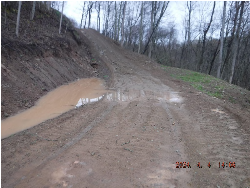
Photo # DSCF3891: Existing access road on sheets 2 and 3 from Pickenpaw Rd. lacks stabilization and BMPs.
