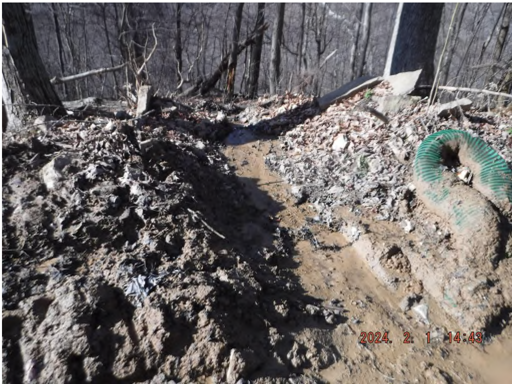
Photo # DSCF1789: Sediment laden water leaving the unstabilized existing access road found on Sheet 2 of the drawings in the SWPPP.
