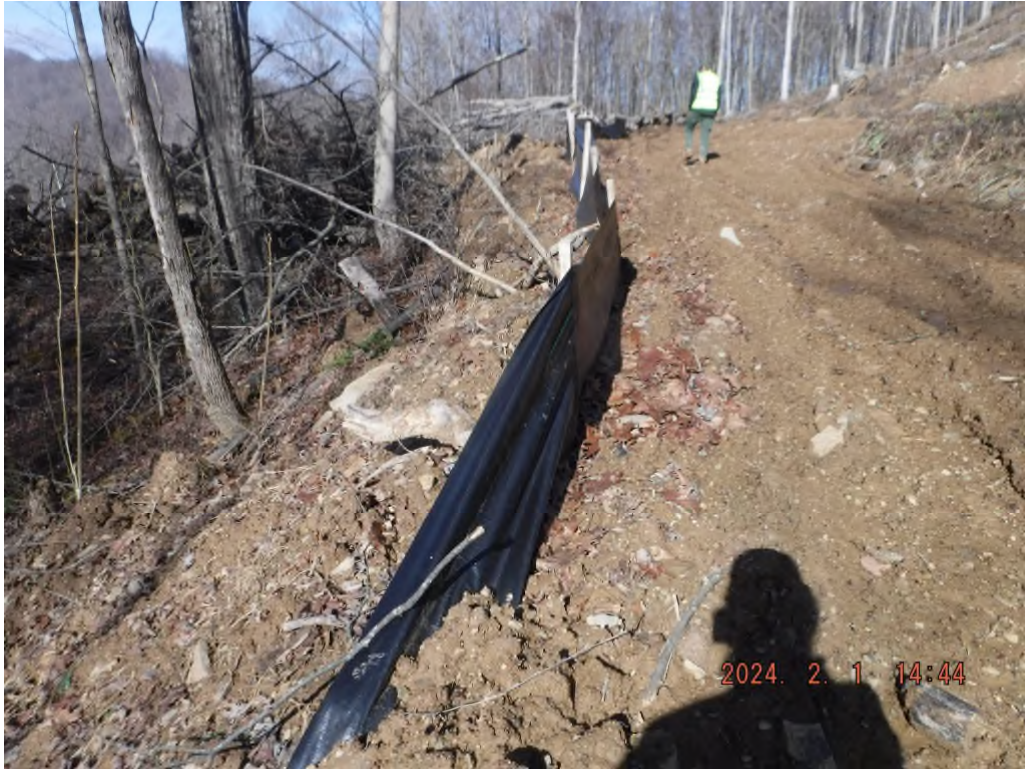
Photo # DSCF1792: Incorrect BMPs installed at or near station 63+00. The SWPPP calls for BSRF or super silt fence.
