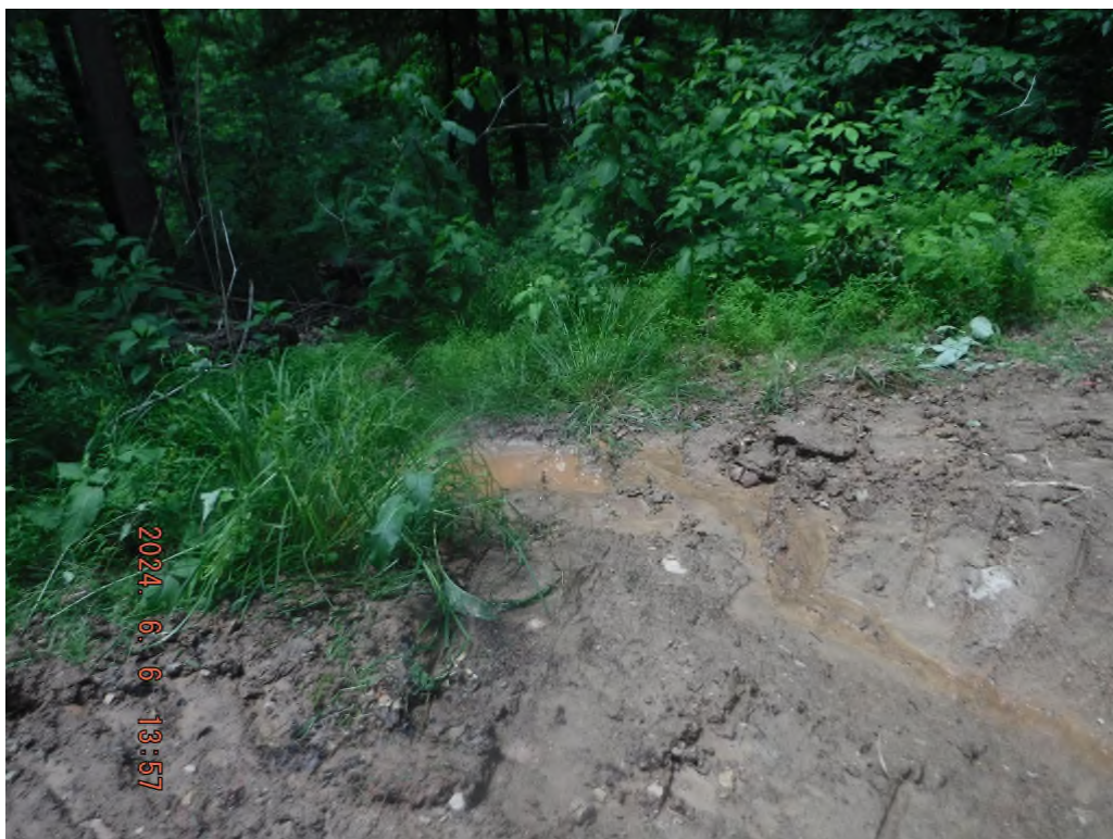
Photo # DSCF5451: Sediment laden water leaving the proposed access road found on drawing sheets 1 and 2 of the approved SWPPP.
