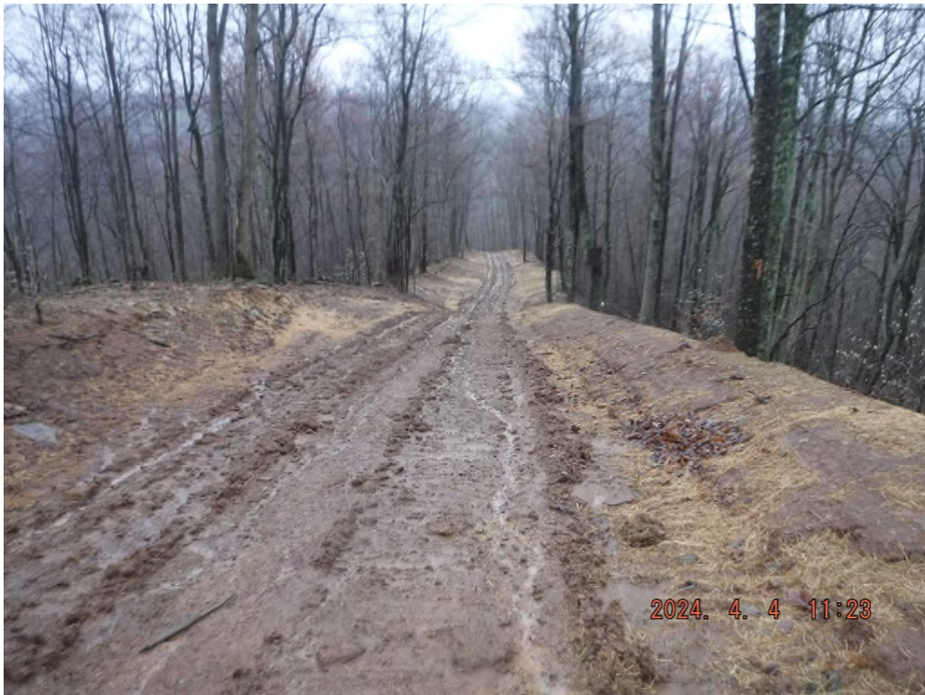
Photo # DSCF3684: Unpermitted access road that starts at ROW at or near N 39° 30.8187', W 80° 31.6944' with no BMPs or stabilization.
