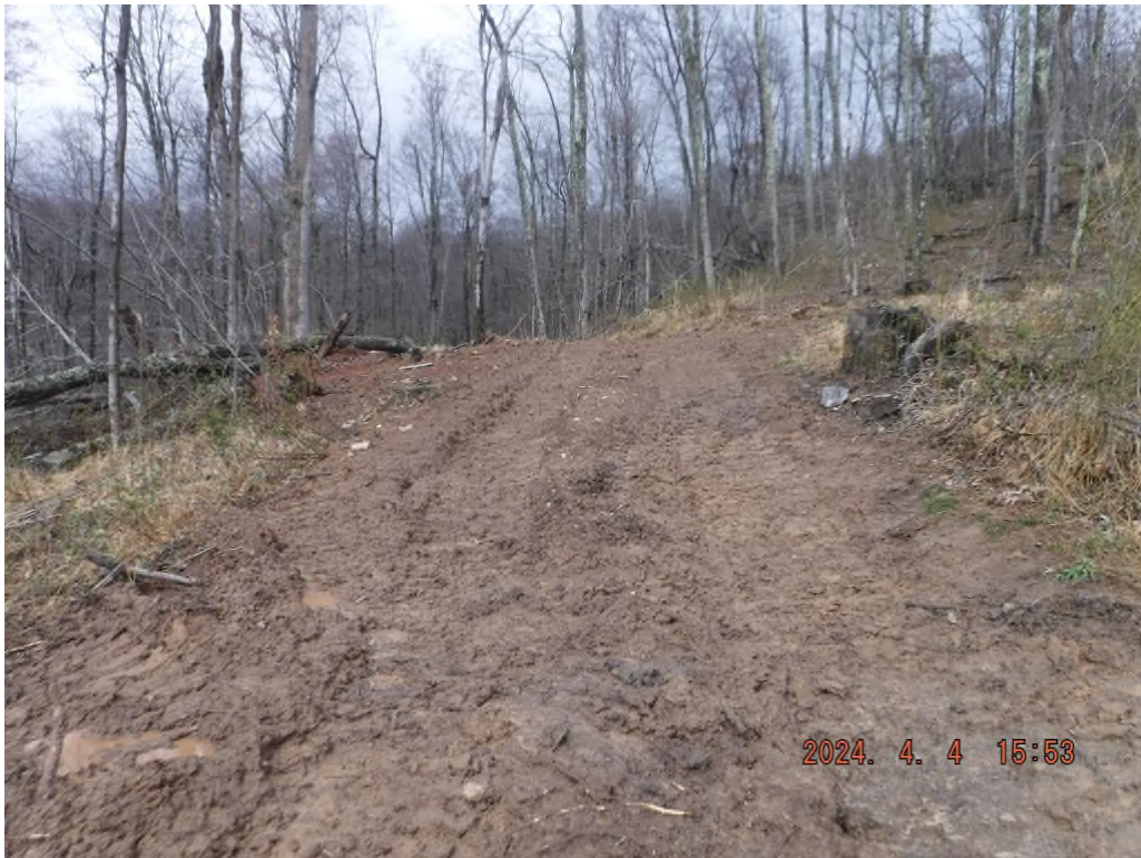
Photo # DSCF4034: Proposed access road on drawing sheet 2 lacks stabilization and BMPs.
