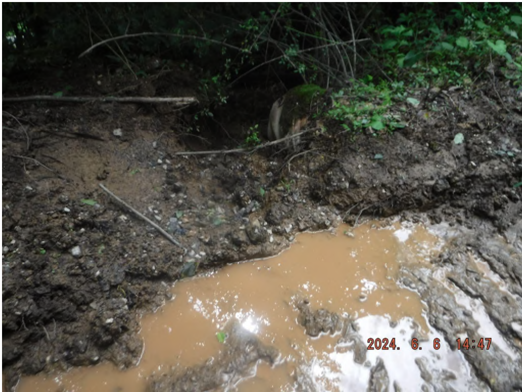
Photo # DSCF5515: Sediment laden water leaving the existing access road found on drawing sheet 2 of the approved SWPPP.
