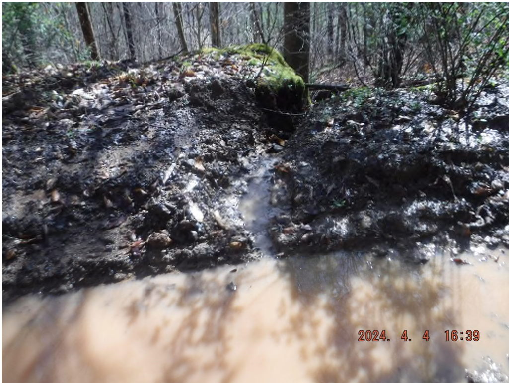
Photo # DSCF4131: Sediment laden water leaving the existing access road on sheet 2 at or near N 39° 30.3899', W 80° 30.4622'.
