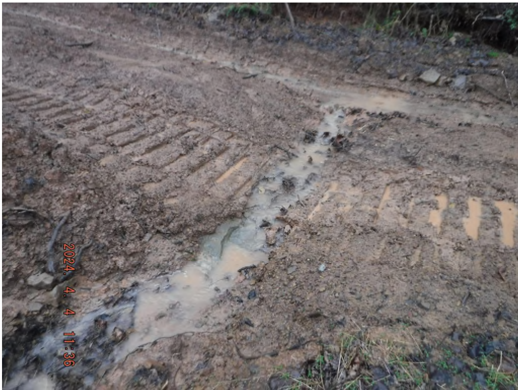
Photo # DSCF3704: Source of sediment laden water leaving the proposed access road on sheet 3 at or near N 39° 30.9789', W 80° 31.6173'.
