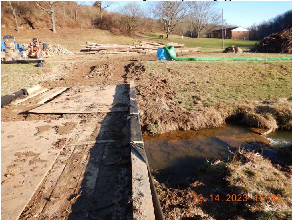
Approximately 30 feet of unprotected area close to Warrior Fork lacked perimeter controls.
