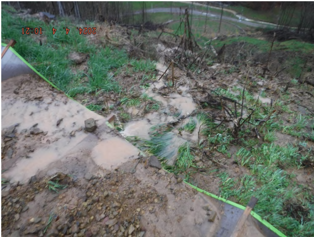
Photo # DSCF3612: BMPs lack maintenance near station 155+00.
