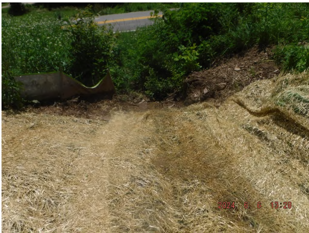
Photo # DSCF5429: Sediment deposits and straw matting in UNT Glade Fork at or near N 39° 30.6051', W 80° 29.8265'.
