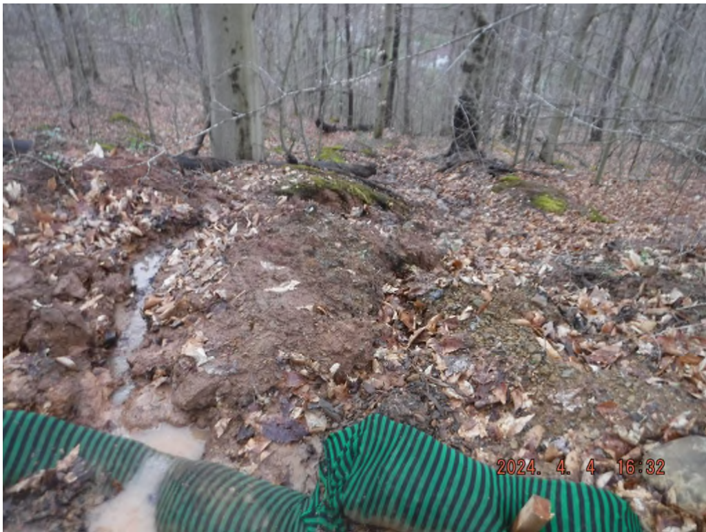
Photo # DSCF4117:Sediment laden water leaving the existing access road on sheet 2 at or near N 39° 30.5143', W 80° 30.5347'.
