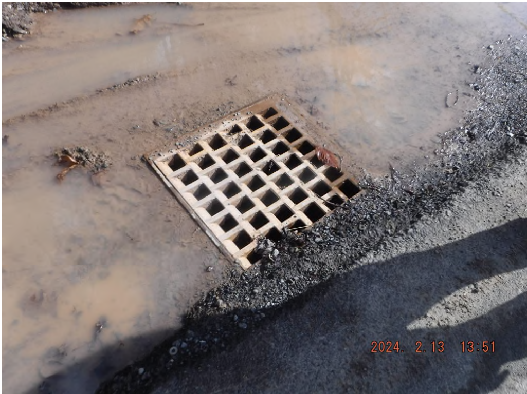
Photo # DSCF2155: No inlet protection at drop inlet B3.
