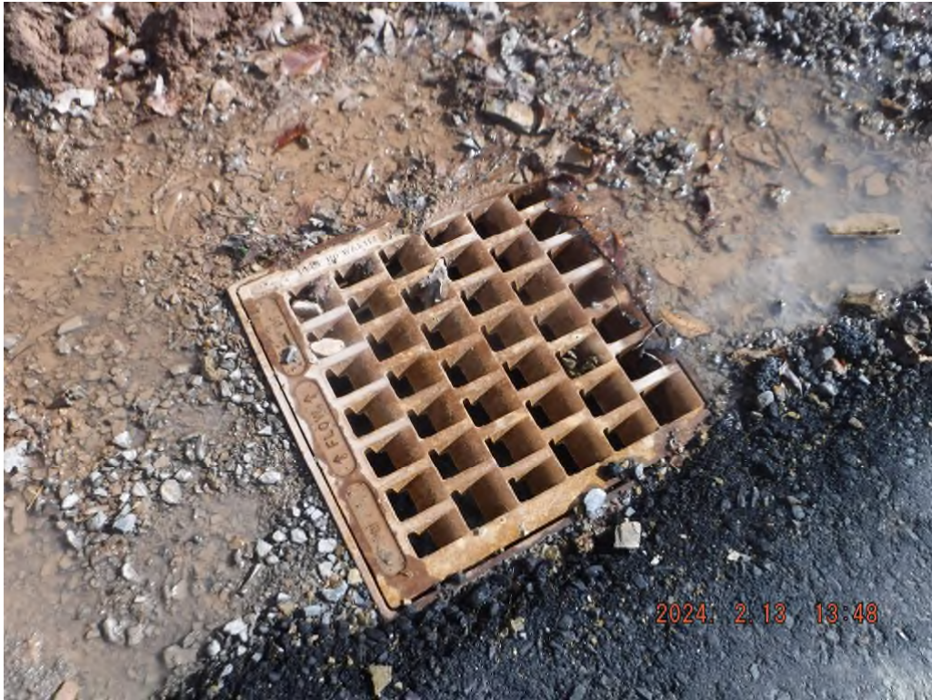
Photo # DSCF2153: No inlet protection at drop inlet B4.
