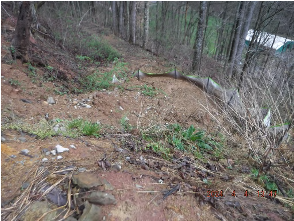
Photo # DSCF3857: Silt fence lacks maintenance at or near N 39° 30.9564', W 80° 30.5013'.
