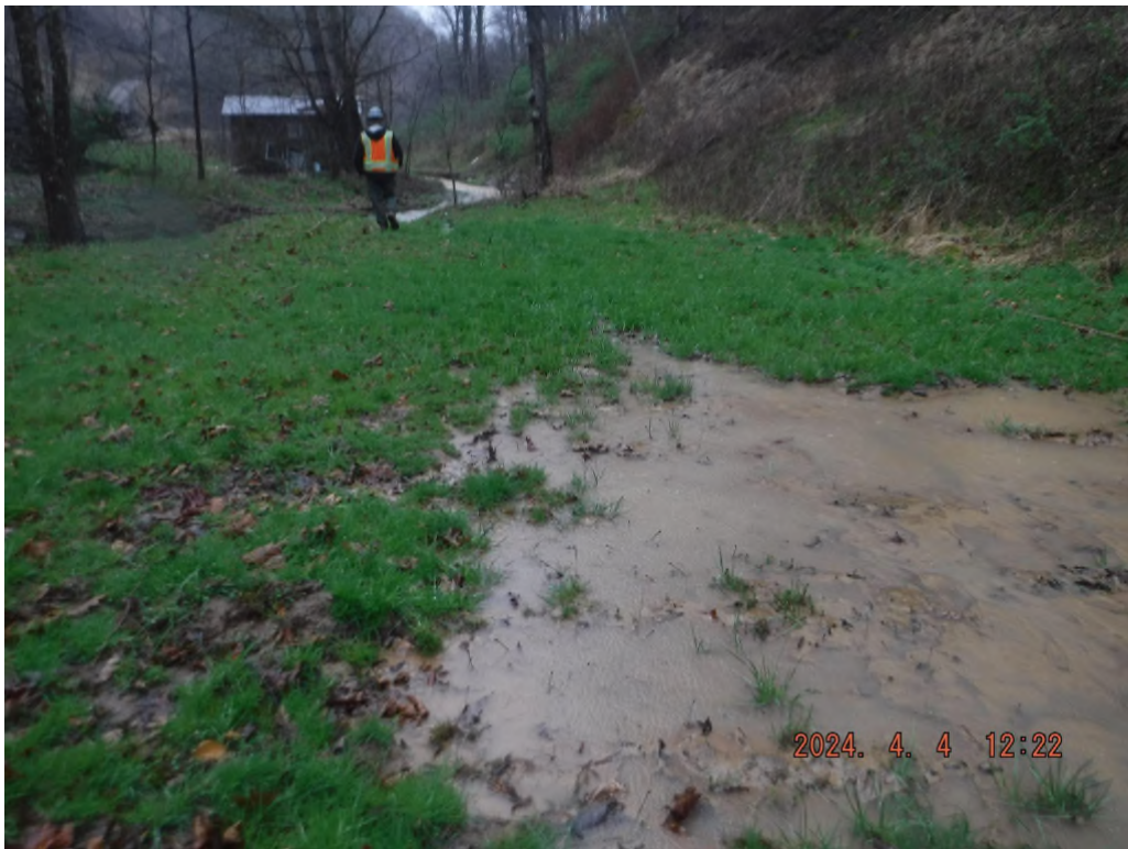
Photo # DSCF3821: Sediment laden water from the unpermitted access road to Buck Run flowing toward Buck run.
