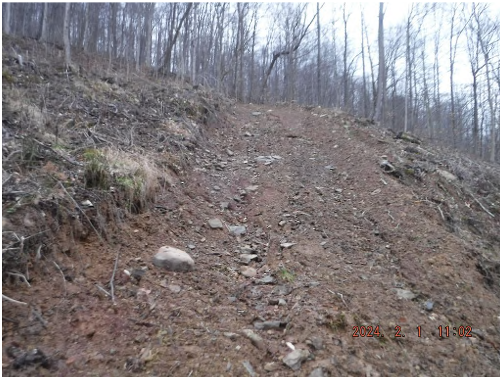
Photo # DSCF1566: Disturbed travel lane off LOD between stations 137+00 and 150+00.
