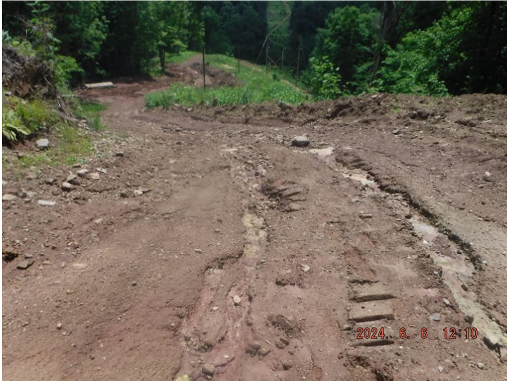
Photo # DSCF5324: Erosion rilling on the existing access road between stations 75+00 and 100+00.
