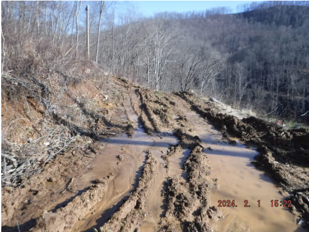
Photo # DSCF1843: Disturbed area outside of the permitted LOD between stations 47+00 and 38+00.
