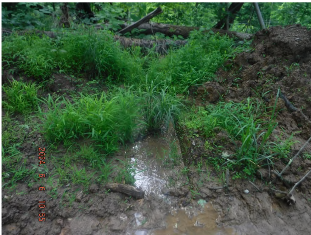
Photo # DSCF5258: Sediment laden water leaving the unpermitted access road to buck run that begins at or near N 39° 30.9806', W 80° 31.3774'.
