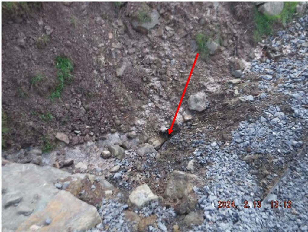
Photo# DSCF2093: No inlet protection at the culvert inlet (red arrow) at station 25+00.
