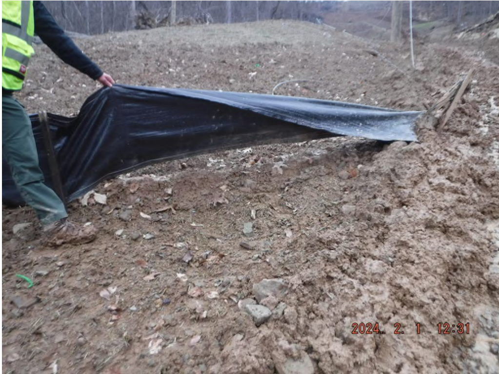
Photo # DSCF1707: Improperly installed silt fence, which is not the BMP detailed in the SWPPP.
