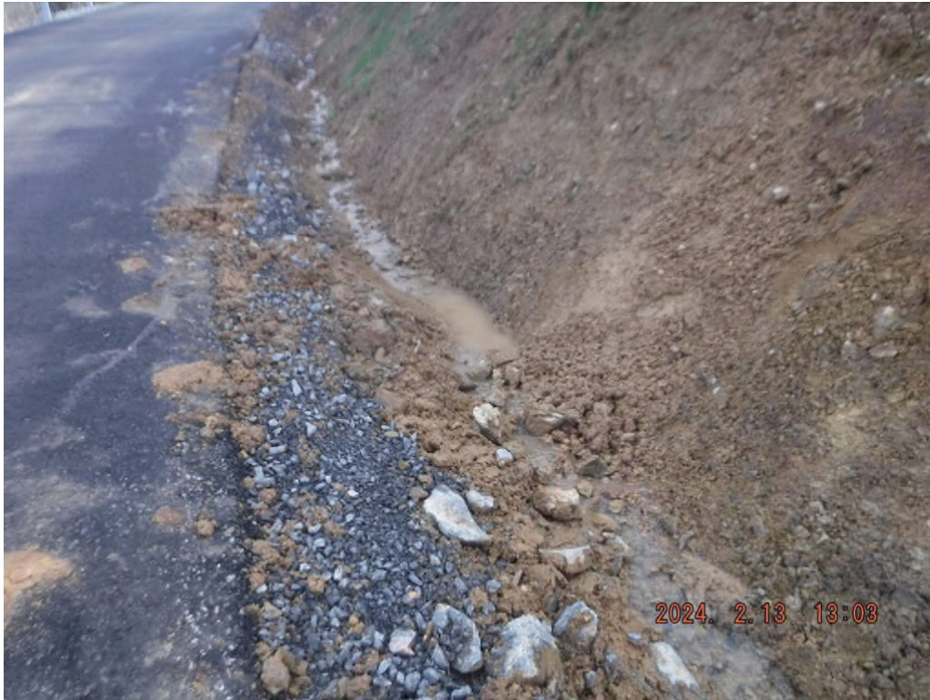
Photo # DSCF2065: Area between station 35+00 and 37+00 that lacks rock check dams.
