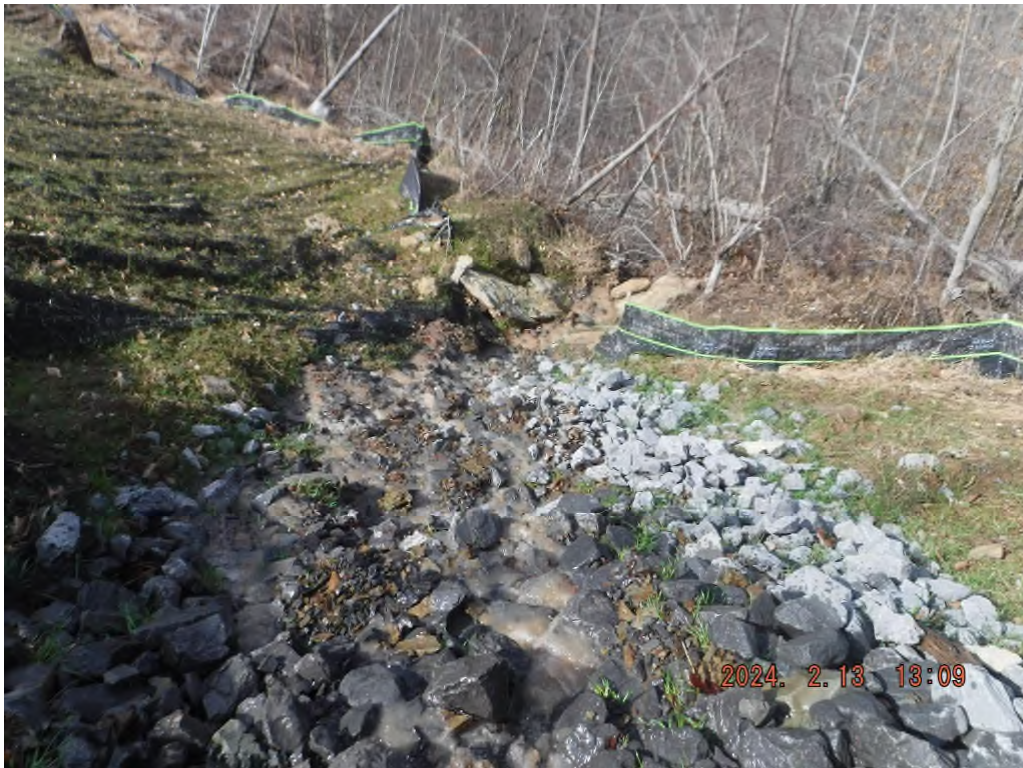
Photo # DSCF2082: Stormwater discharge point 10 at or near station 29+00. Silt fence lacks maintenance leading into ephemeral 8.
