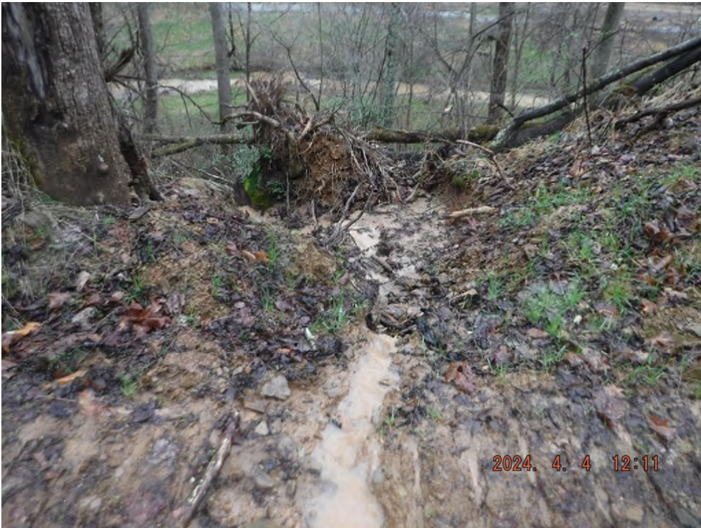
Photo # DSCF3800: Sediment laden water leaving the unpermitted access road near N 39° 31.1366', W 80° 31.2743' at or near N 39° 31.0703', W 80° 31.2682'.
