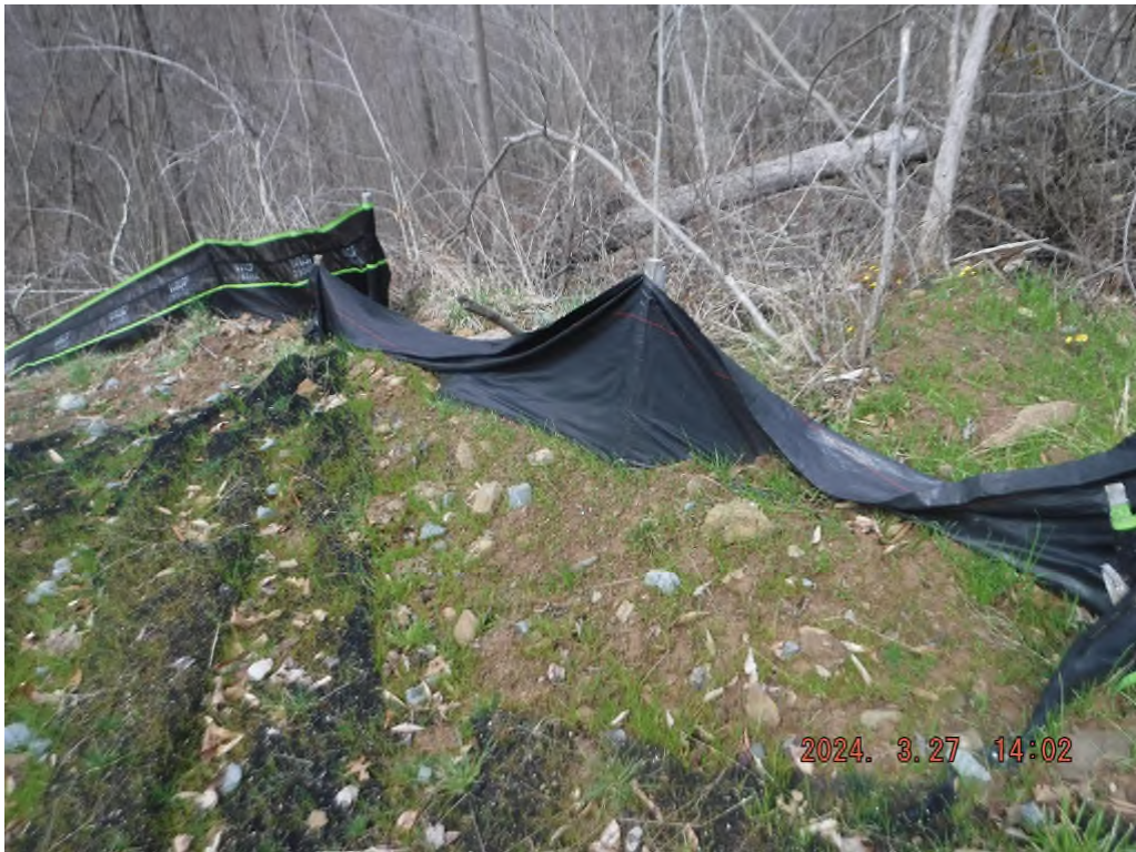
Photo # DSCF3361: Incorrect silt fence installed at station 29+50.
