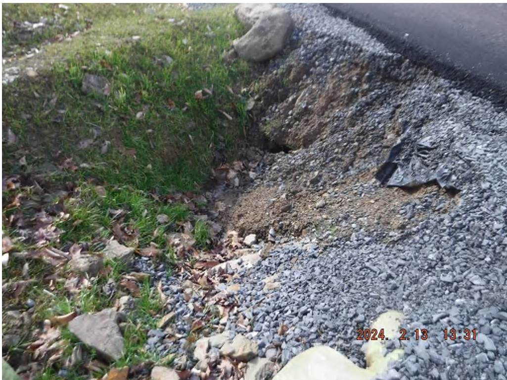
Photo # DSCF2139: No inlet protection at or near 14+50.
