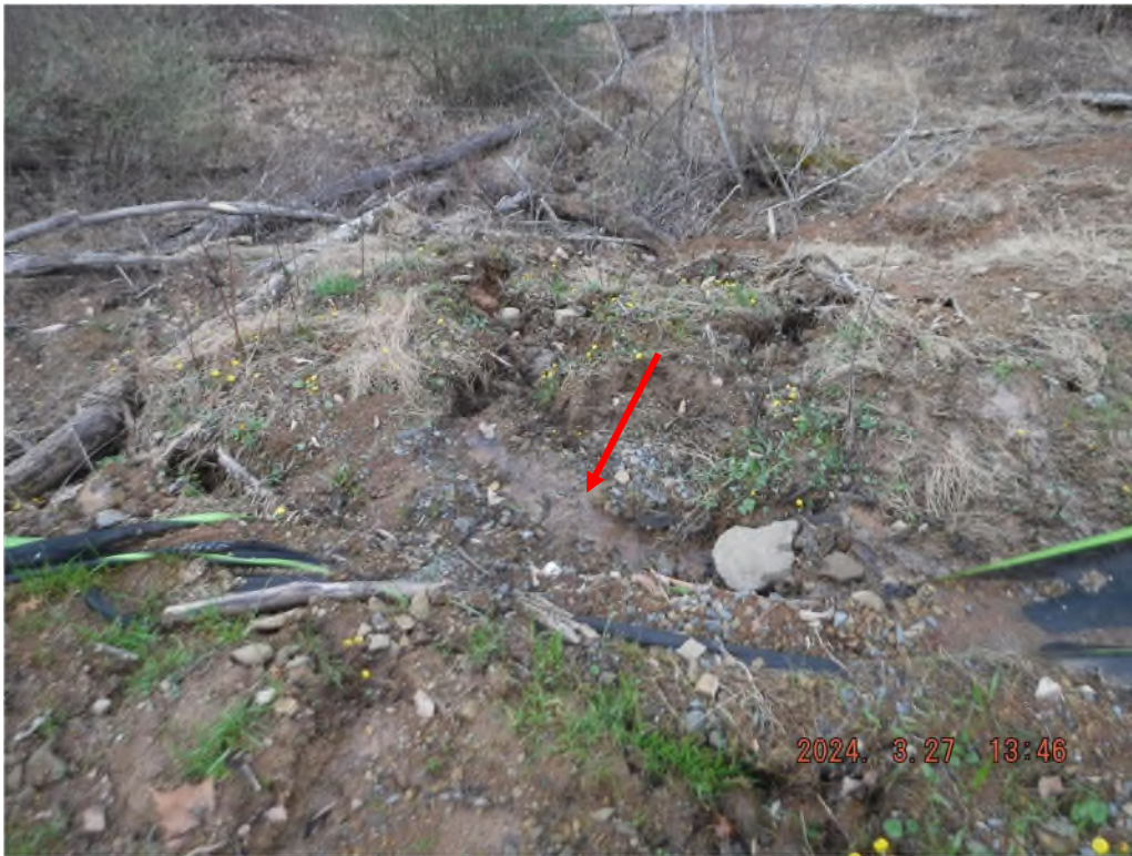
Photo # DSCF3329: Sediment laden water leaving the site from discharge point 11 at station 37+00, and silt fence lacks maintenance.
