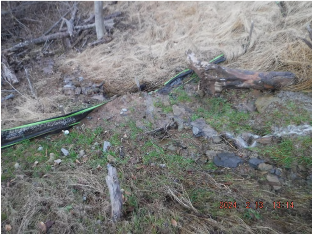
Photo # DSCF2096: Silt fence lacks maintenance below the culvert outlet at station 25+00.
