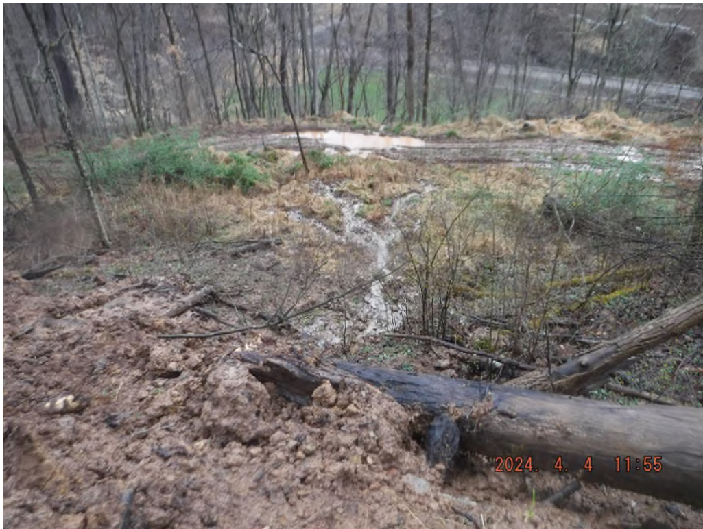
Photo # DSCF3761: Sediment laden water leaving the unpermitted access road to Buck Run Rd. at or near N 39° 31.8484', W 80° 31.3387'.
