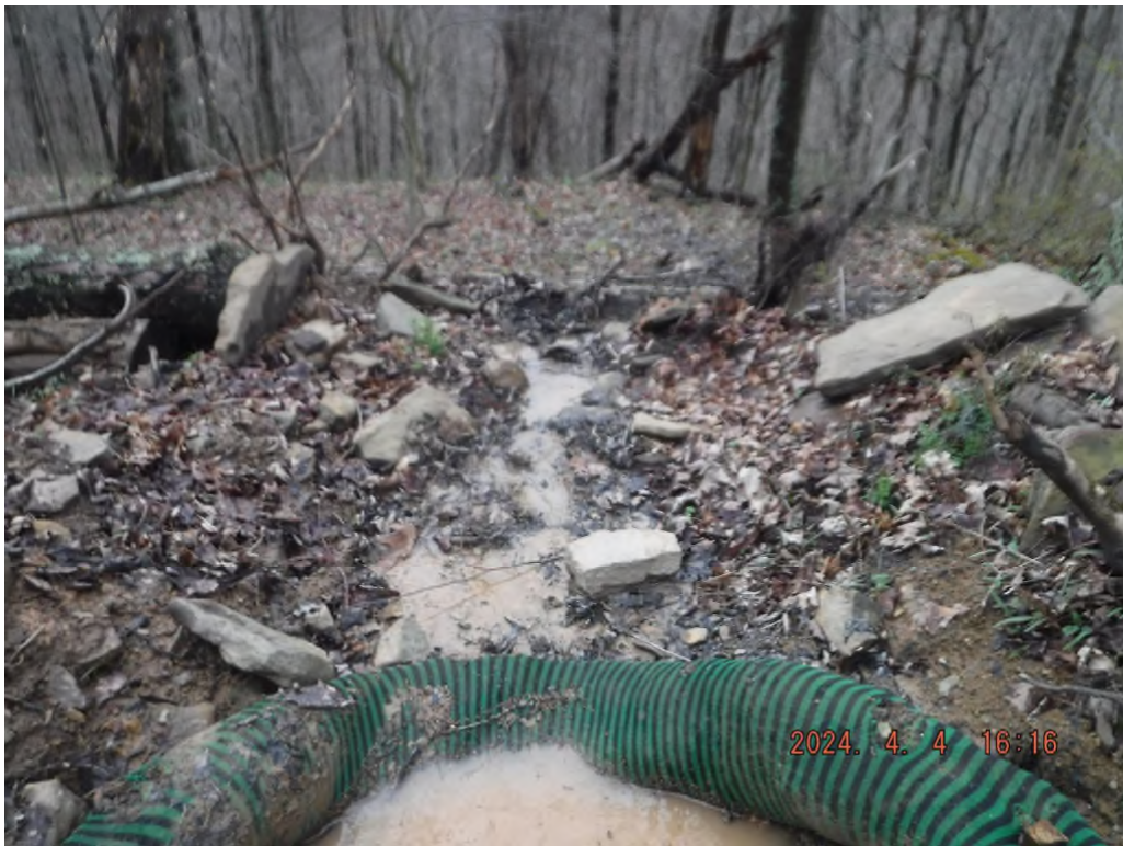
Photo # DSCF4088: Sediment laden water leaving the existing access road on sheet 2 at or near N 39° 30.8112', W 80° 30.2427'.
