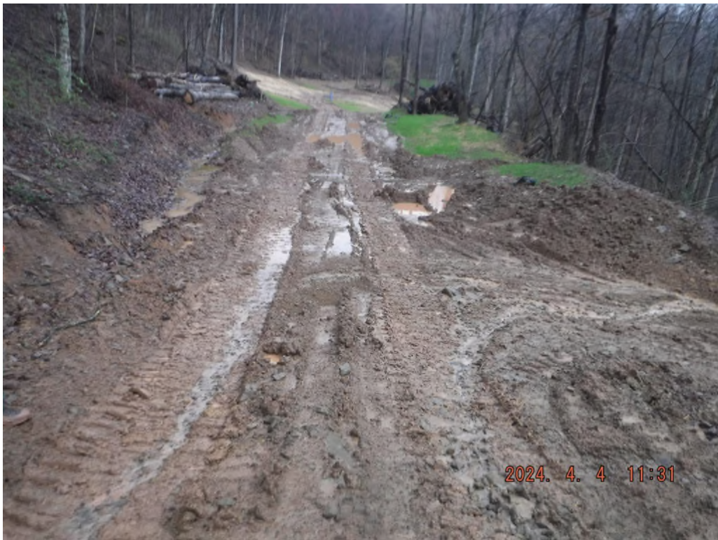
Photo # DSCF3690: Proposed access road on drawing sheet 3 of the SWPPP lacks stabilization.
