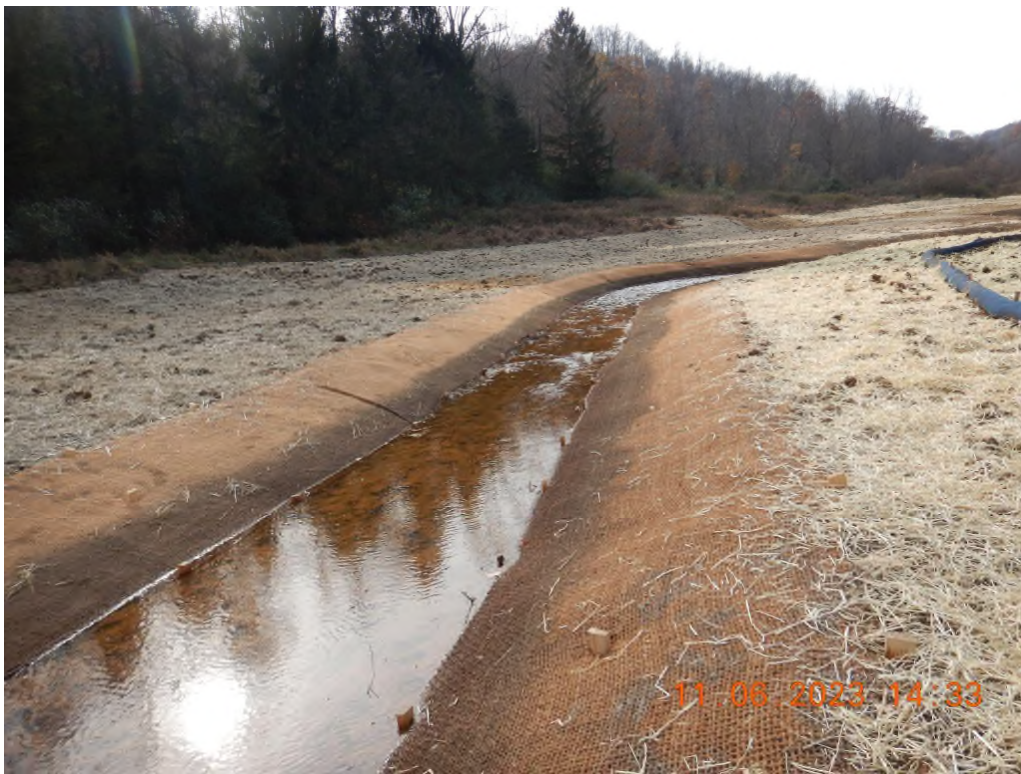
Area above active work area where water is clear in Buffalo Creek. Missing perimeter controls along the edge of the stream.
