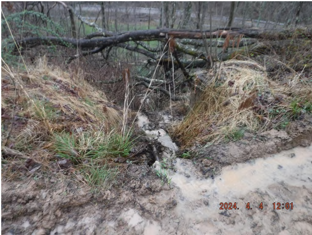
Photo # DSCF3783: Sediment laden water leaving the unpermitted access road at N 39° 31.0736', W 80° 30.3038' at or near N 39° 31.0187', W 80° 31.3165'.
