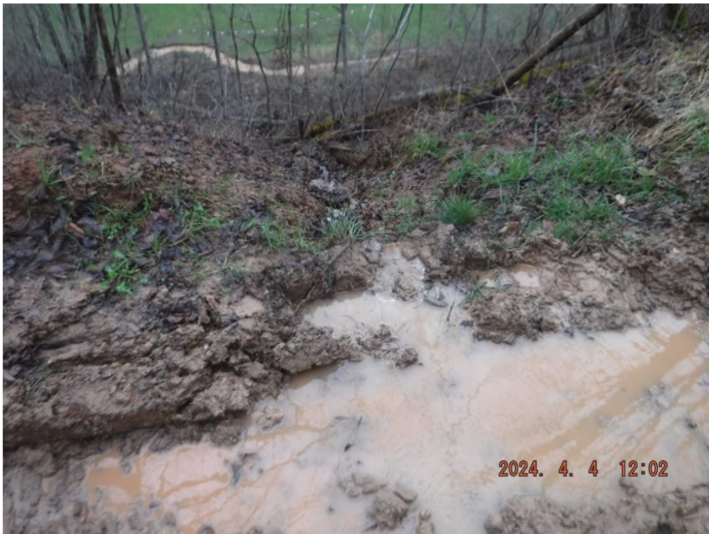
Photo # DSCF3785: Sediment laden water leaving the unpermitted access road at N 39° 31.0736', W 80° 30.3038' at or near N 39° 31.0050', W 80° 31.3265'.
