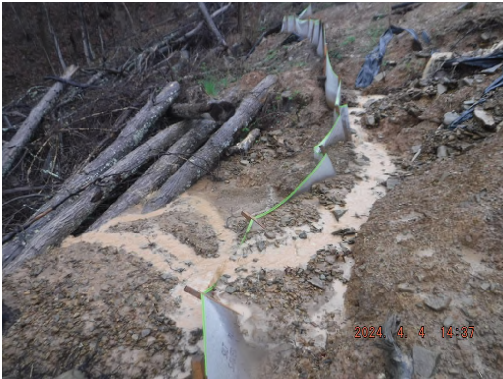
Photo # DSCF3945: BMPs lacking maintenance and sediment laden water leaving the ROW at or near N 39° 31.0460', W 80° 31.0529'.
