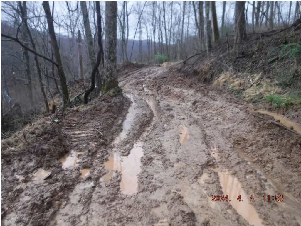
Photo # DSCF3762: Unpermitted access road at or near N 39° 30.9806', W 80° 31.3774' that leads down to Buck Run Rd. and lacks stabilization and BMPs.
