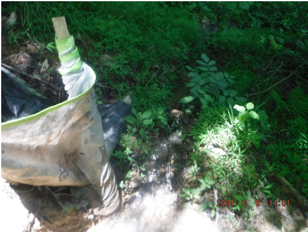
Photo # DSCF5464: Sediment laden water leaving the proposed access road found on drawing sheets 1 and 2 of the approved SWPPP.
