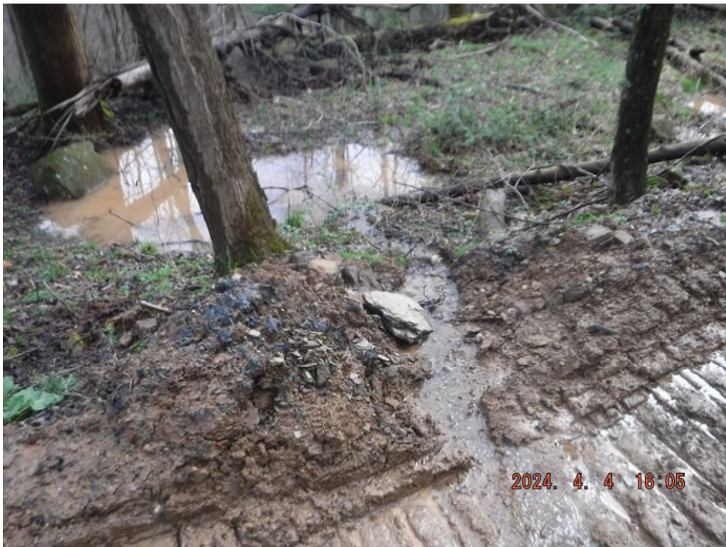
Photo # DSCF4061: Sediment laden water leaving the proposed access road on drawing sheet 2 at or near N 39° 30.8934', W 80° 30.0364'.
