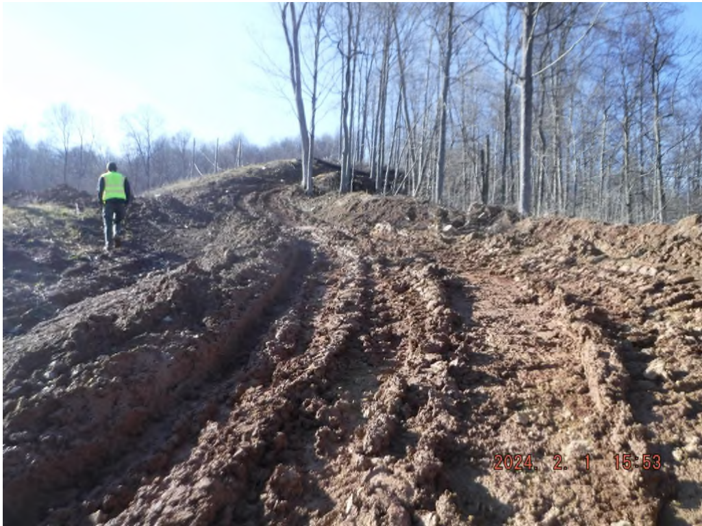
Photo # DSCF1863: Disturbed area outside of LOD between stations 75+00 and 80+00.
