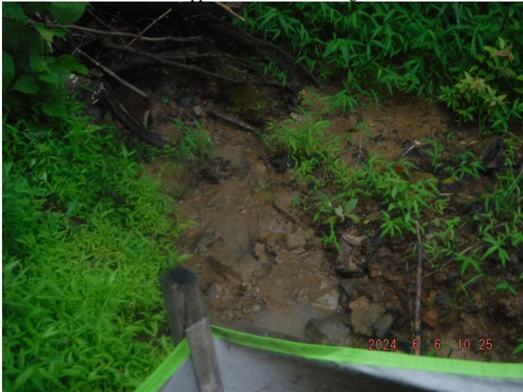
Photo # DSCF5201: Sediment laden water leaving the proposed access road found on sheets 3 and 4 of the approved SWPPP drawings.
