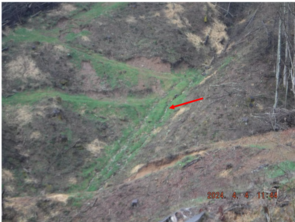
Photo # DSCF3733: Erosion in the travel lane off LOD in the ROW between stations 130+00 and 135+00.
