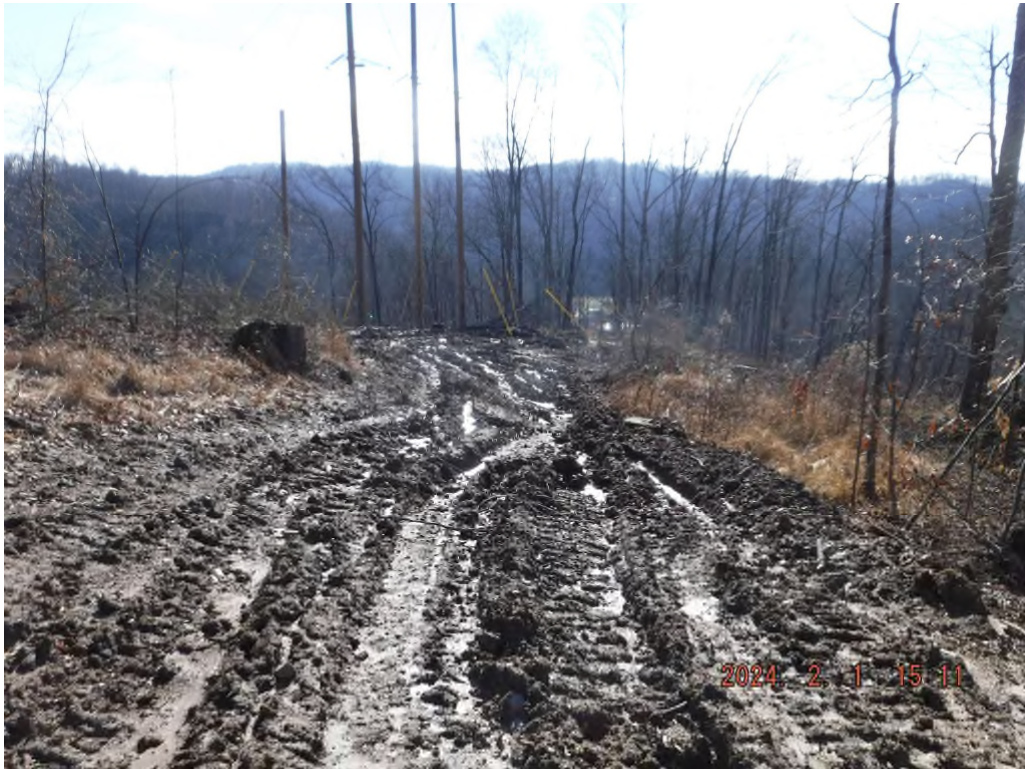
Photo # DSCF1828: Proposed access road found on Sheet 2 of the drawings in the SWPPP lacks stabilization.
