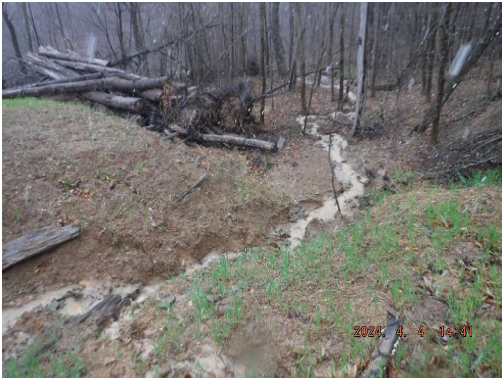
Photo # DSCF3955: Sediment laden water leaving the ROW at or near N 39° 31.0306', W 80° 31.1208'.
