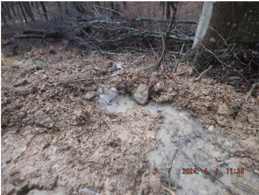
Photo # DSCF3718: Sediment laden water leaving the proposed access road on sheet 3 at or near N 39° 30.9891', W 80° 31.5432'.
