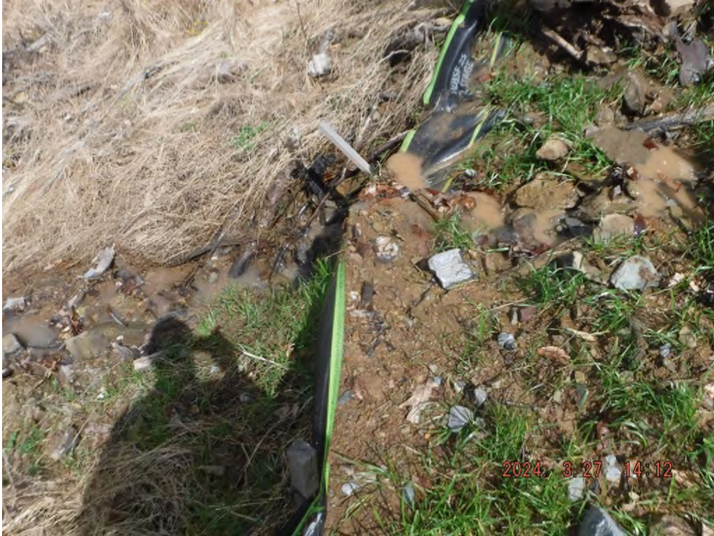
Photo # DSCF3382: Sediment laden water leaving at station 25+00
