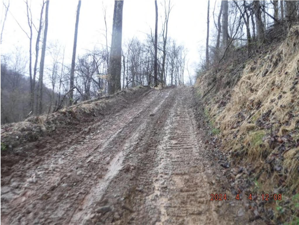
Photo # DSCF3793: Unpermitted access road to Buck Run that lacks stabilization and BMPs.
