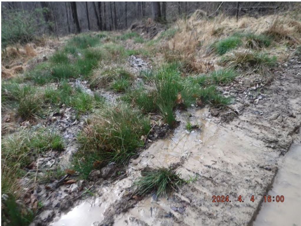
Photo # DSCF4049: Sediment laden water leaving the proposed access road on drawing sheet 2 at or near N 39° 30.8884', W 80° 29.9053'.
