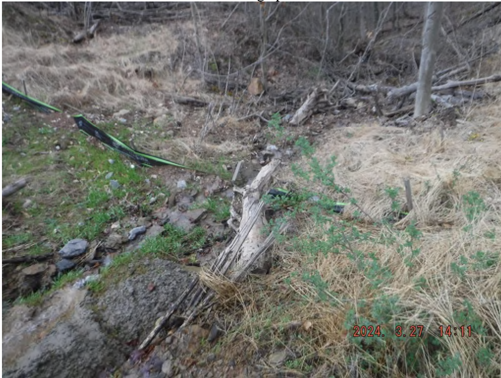
Photo # DSCF3380: BMPs lack maintenance at station 25+00.
