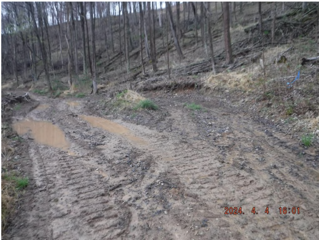
Photo # DSCF4054: Proposed access road on drawing sheet 2 lacks stabilization and BMPs.
