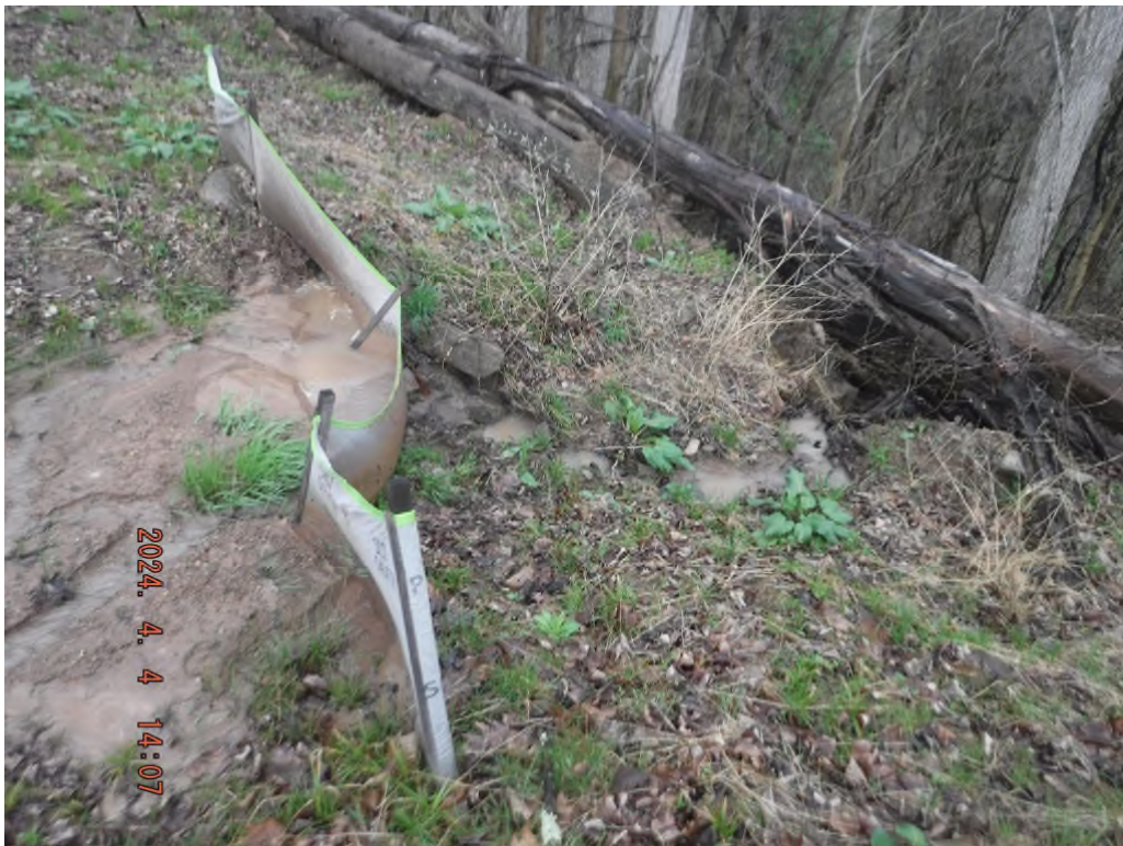
Photo # DSCF3896: Sediment laden water leaving the existing access road on sheets 2 and 3 from Pickenpaw Rd. at or near N 39° 31.0252', W 80° 30.7007'.
