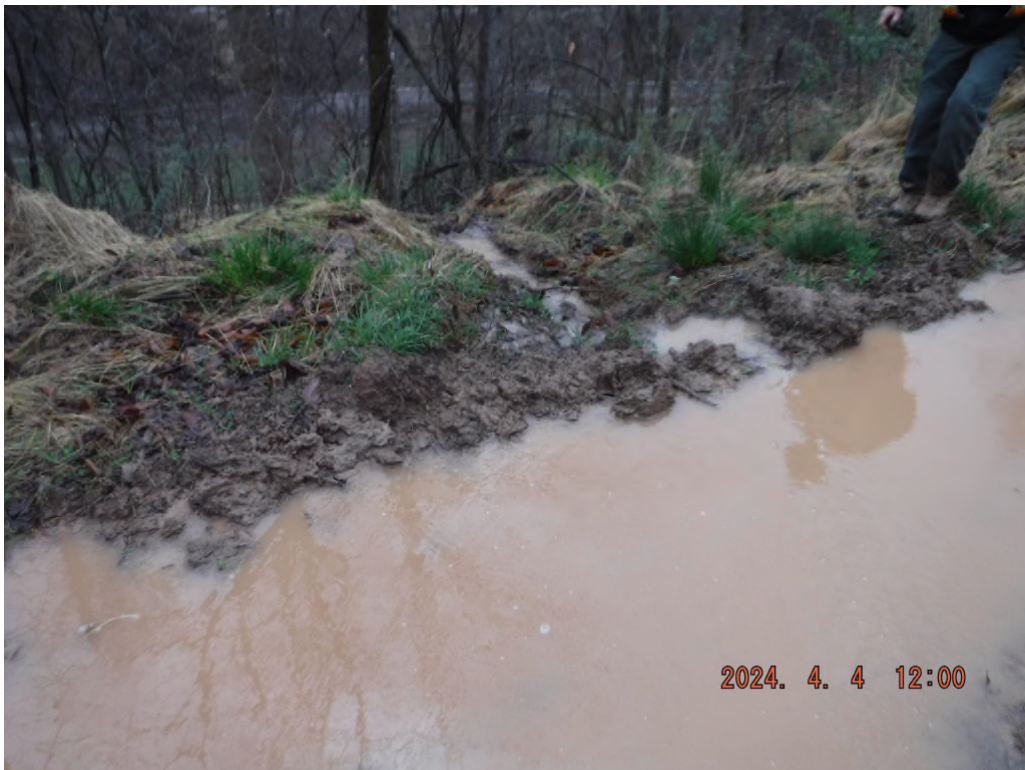
Photo # DSCF3779: Sediment laden water leaving the unpermitted access road at N 39° 31.0736', W 80° 30.3038' at or near N 39° 31.0373', W 80° 31.3126'.
