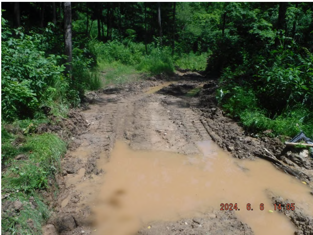
Photo # DSCF5468: Proposed access road found on sheets 1 and 2 of the approved SWPPP is unstabilized.
