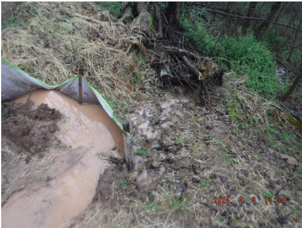
Photo # DSCF3699: Sediment laden water leaving the proposed access road on sheet 3 at or near N 39° 30.9685', W 80° 31.6435'.
