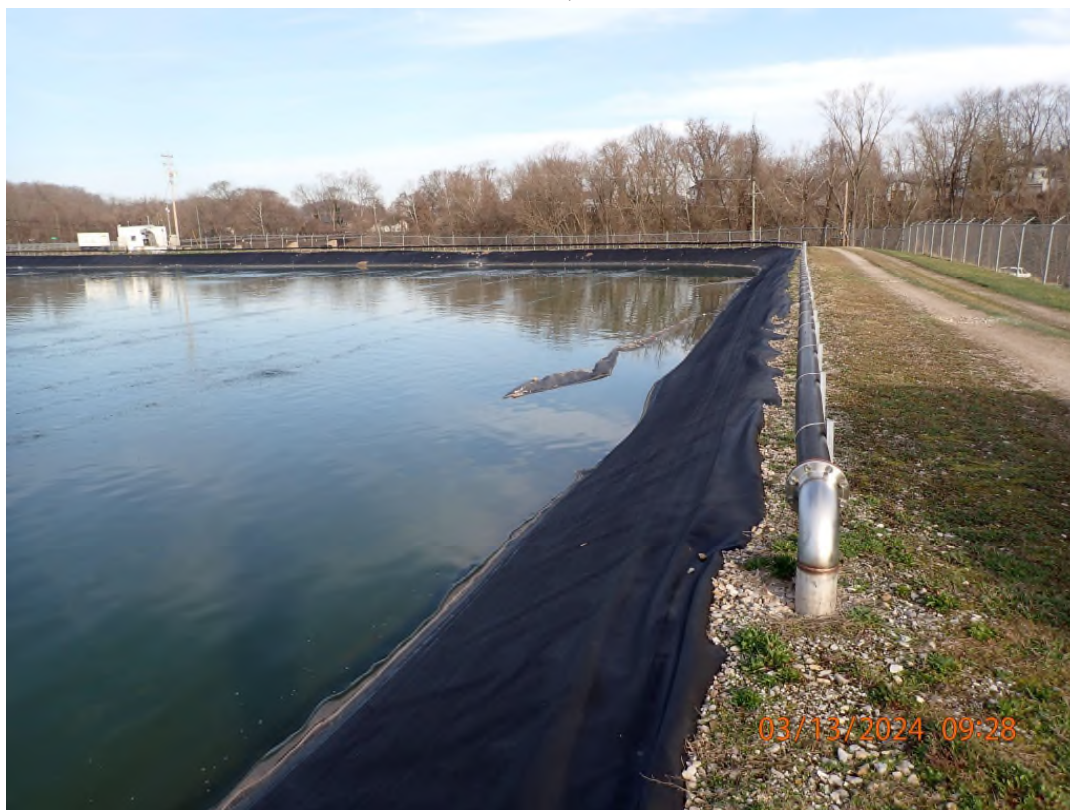
P3130651 - Floating Liner Section in Pond 1
