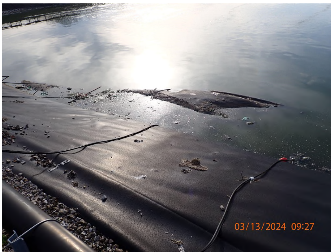
P3130650 - Another Floating Liner Section in Pond 1
