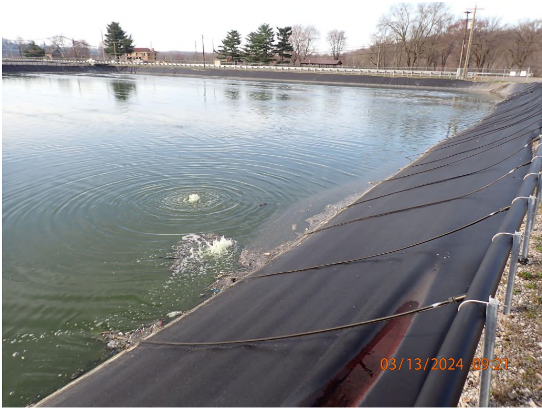
P3130643 - Broken Air Lines in Pond 1
