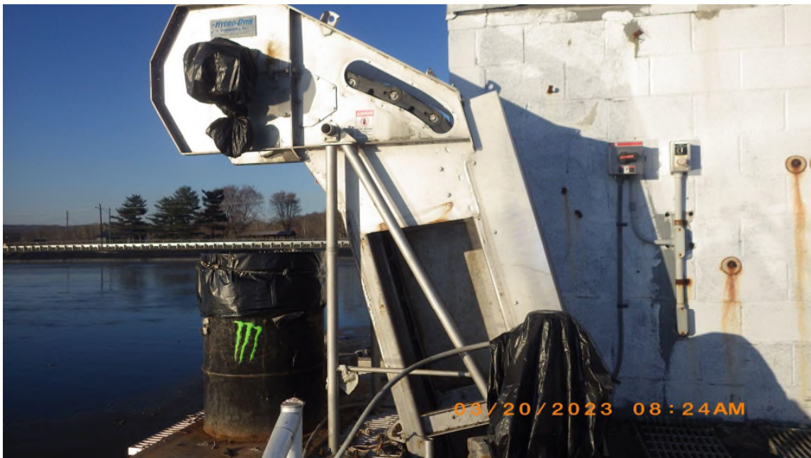
Nonoperational Automatic Bar Screen
