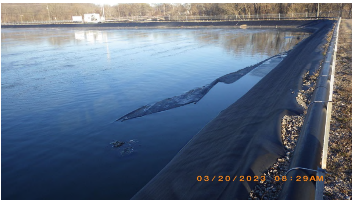
Floating Baffle Curtain in Cell 1
