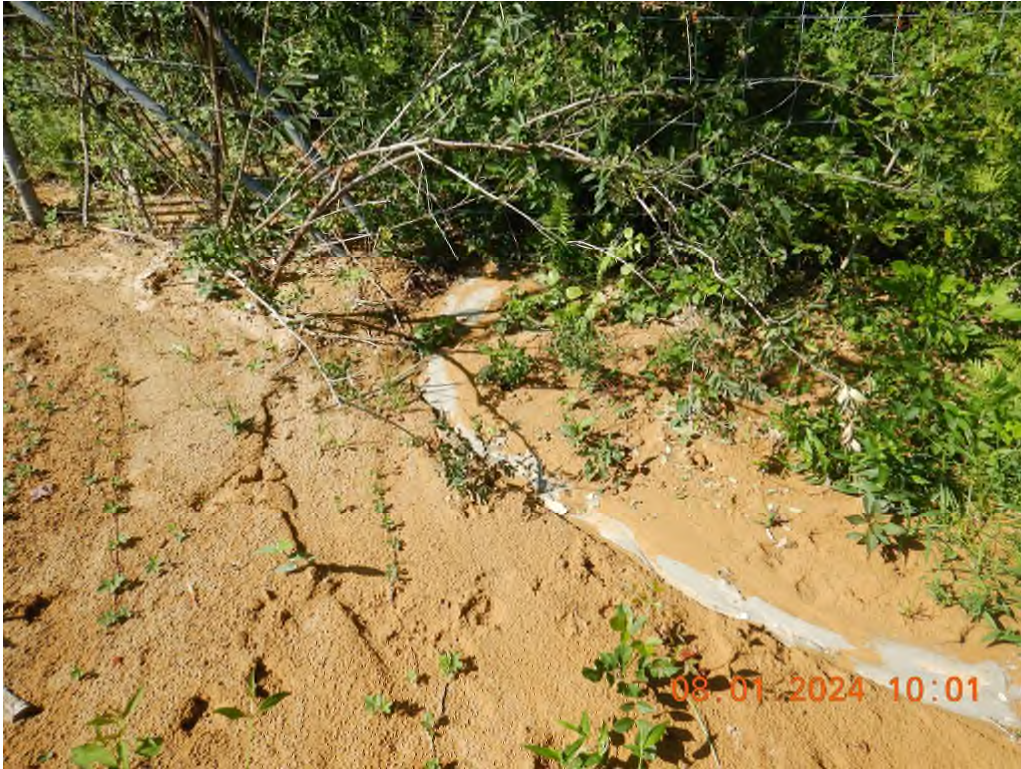
Concrete washout discharge beyond the property boundary.
