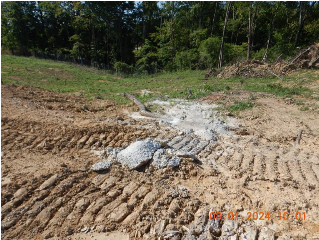
Concrete washout that had discharged directly onto the ground.
