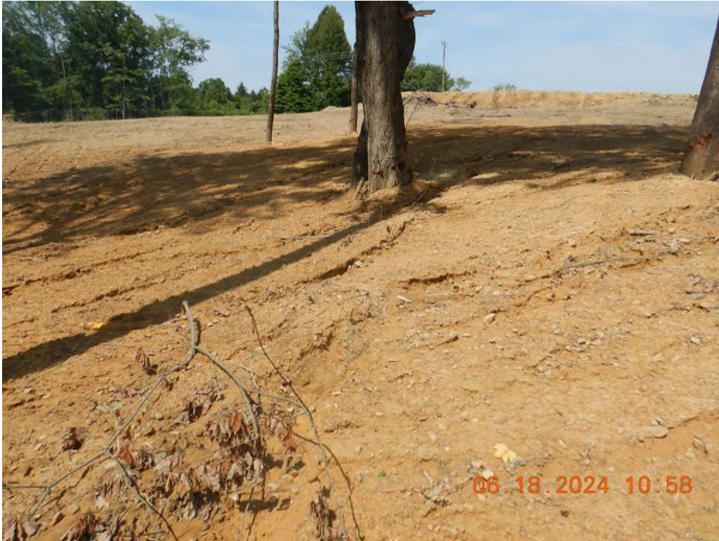
Erosion rills that formed due to a lack of stabilization.
