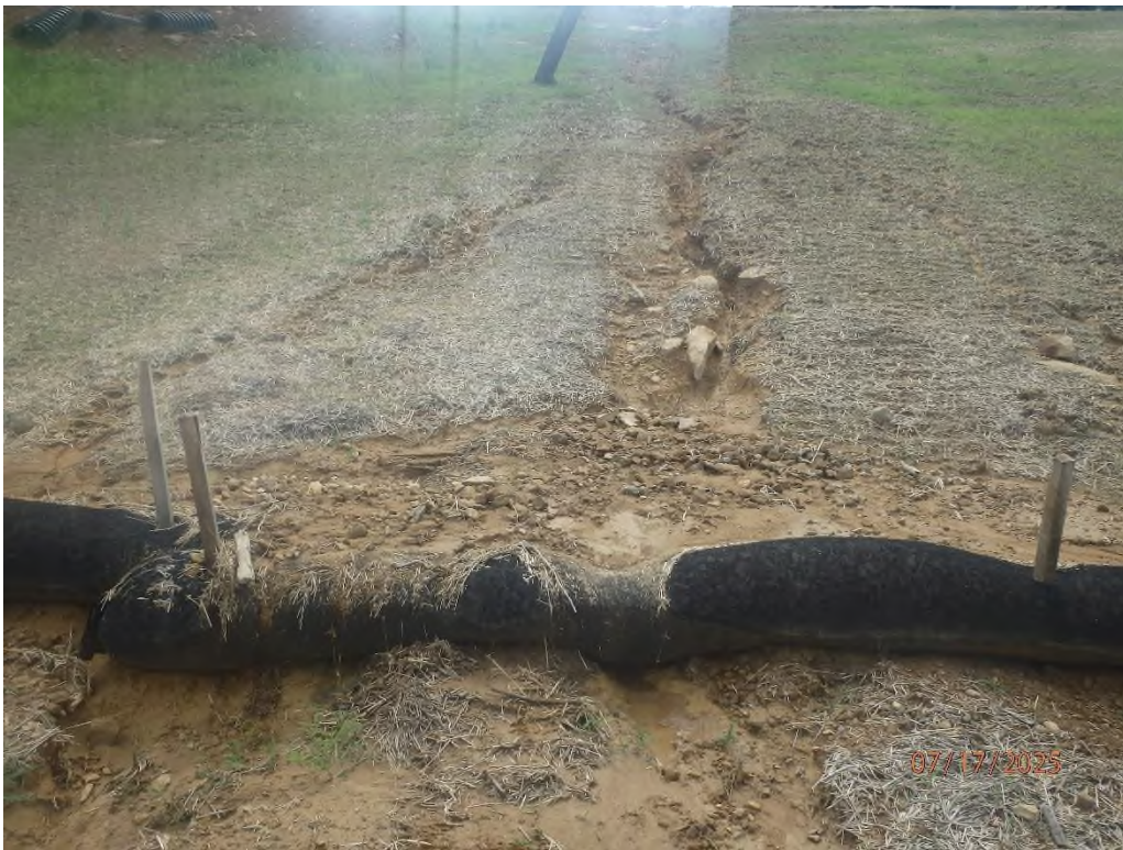
Fill slope erosion, unmaintained BMPs, and sediment laden water bypass in the western portion of the project.
