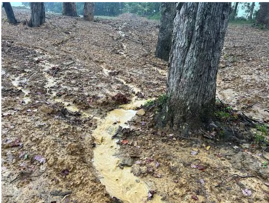
Overview of disturbance in the area of the complaint. Sediment laden water discharges with no BMPs in place.
