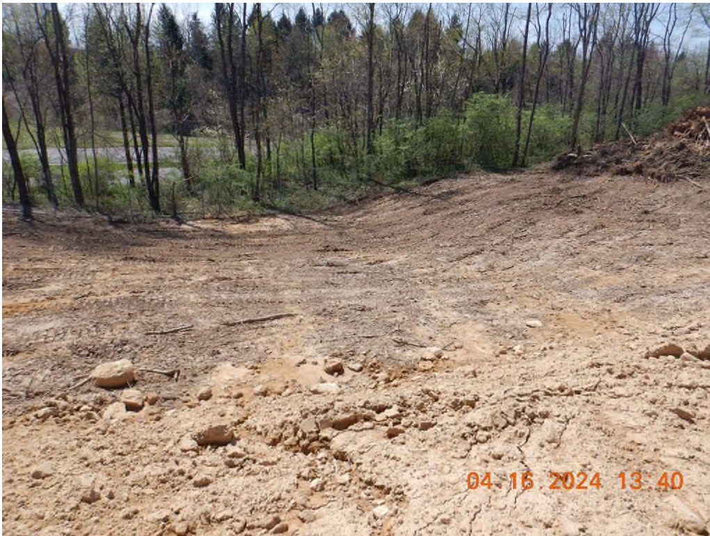
Erosion and sediment controls were not installed at the time of inspection.
