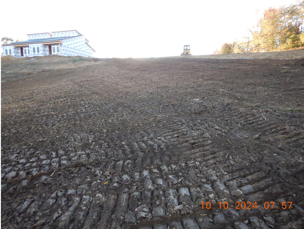
Failure to implement temporary stabilization on the western portion of the site.
