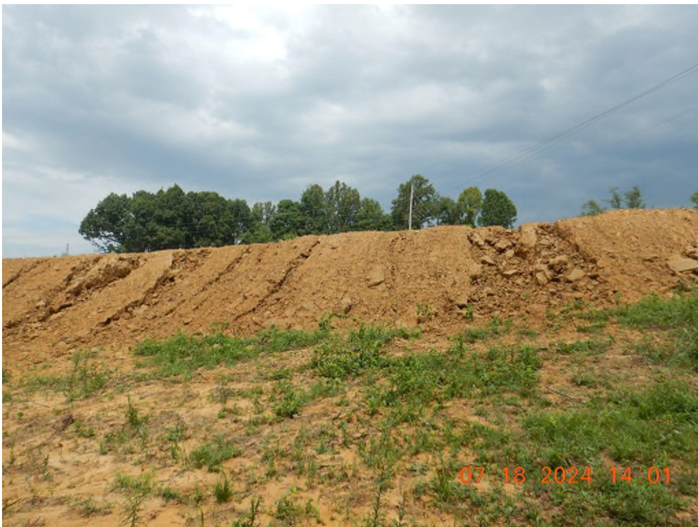
The erosion rills on the fill slope of the pad continue to worsen.
