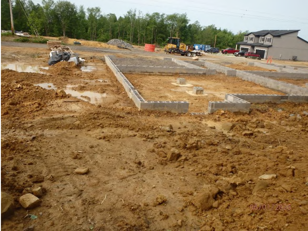
Backfilling of foundations and changes to the adjacent stockpiles, in violation of Order 10314.
