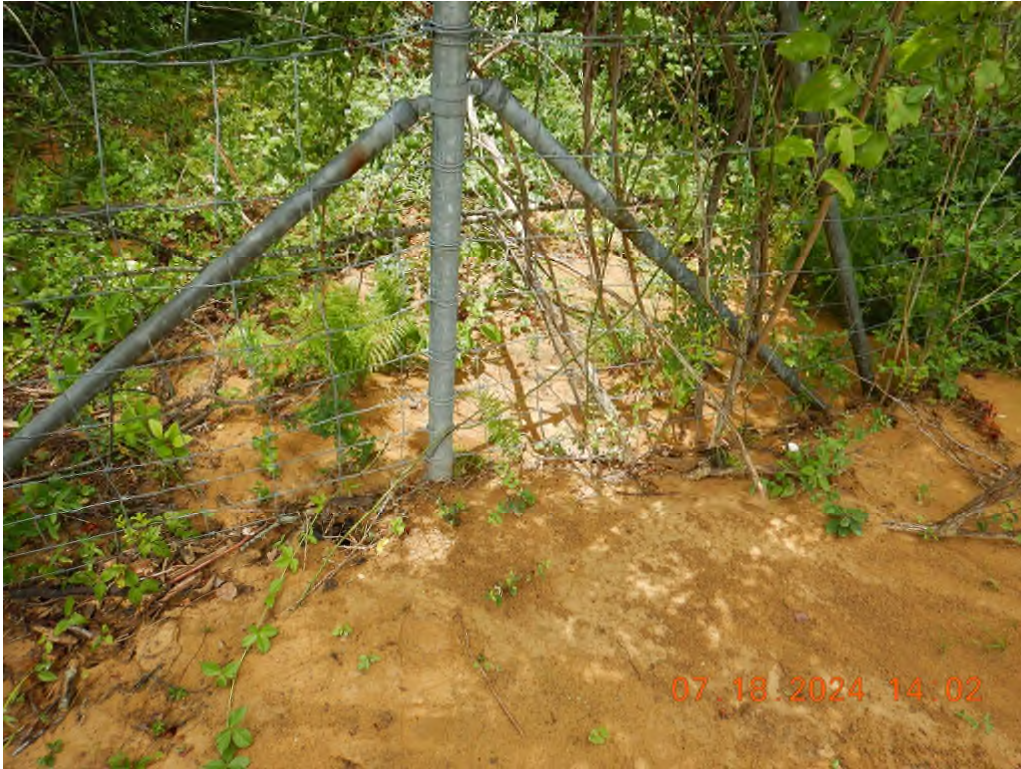
The sediment from the eroded fill slope is discharging across the fence line towards US Route 33.
