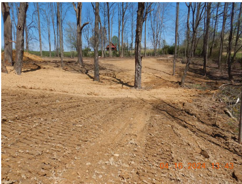
A small ephemeral stream (UNT of Sand Run) that was dozed over leaving sediment deposits within the stream channel.
