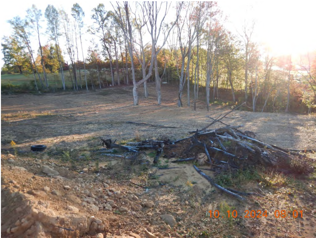
Failure to implement temporary stabilization on the eastern portion of the site.
