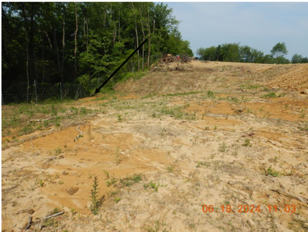
The erosion from photo 8 was causing sediment to discharge at a low spot on the south side of the project.
