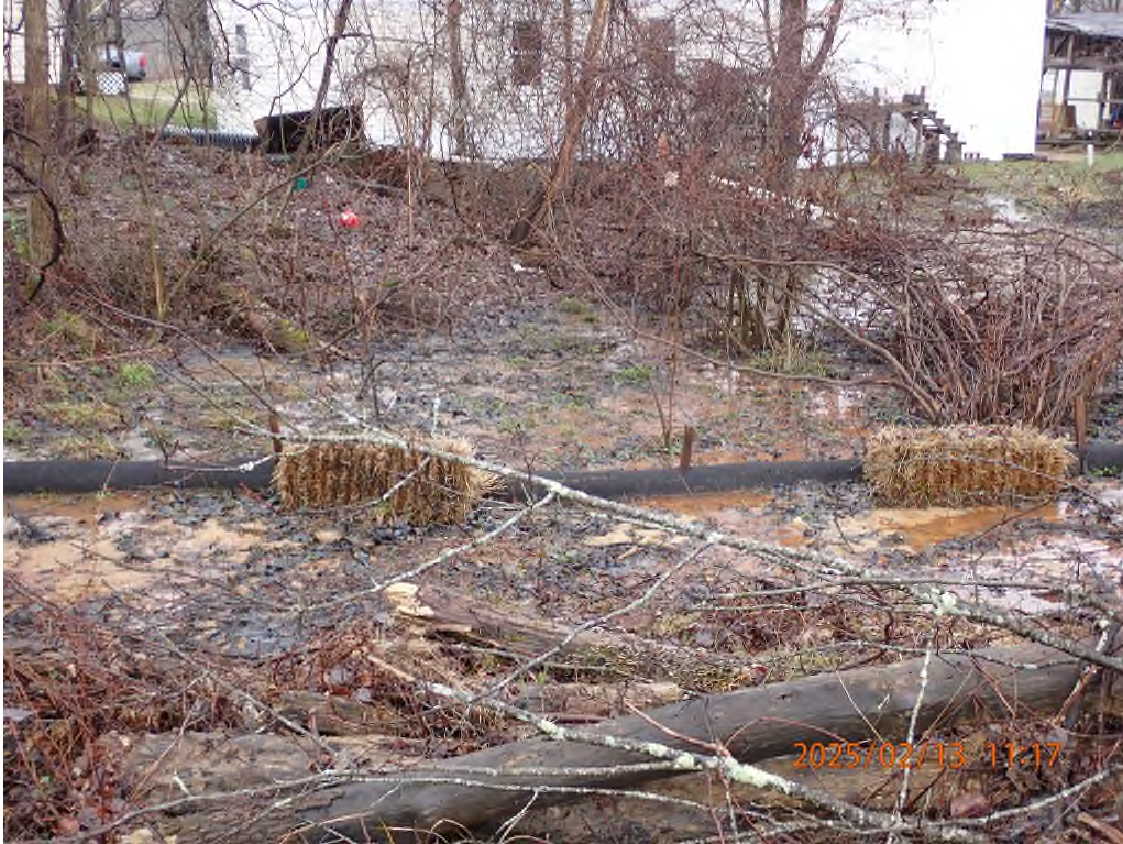
Sediment and sediment laden water discharging off the unpermitted site.
