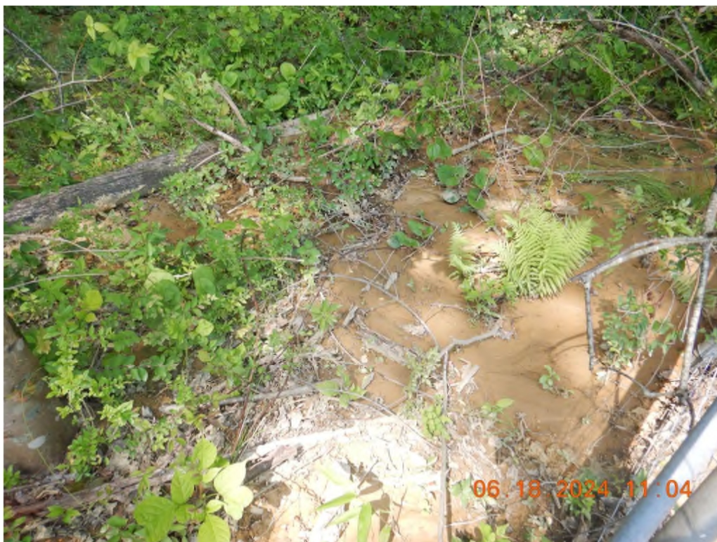
Sediment that was deposited beyond the fence line shown in the previous photograph.
