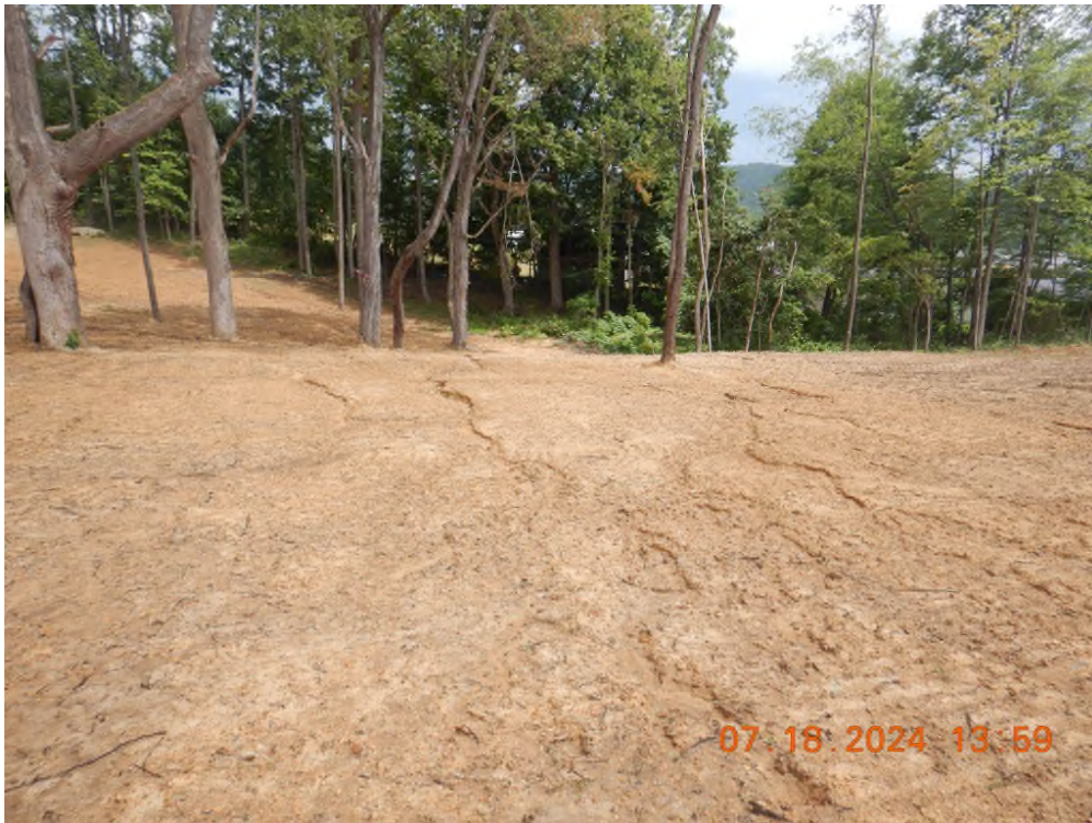
Erosion rills on the eastern side of the project continue to worsen, causing sediment to discharge into ephemeral UNT of Sand Run.
