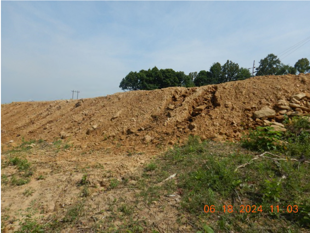
The fill slopes for the pad were eroding away.
