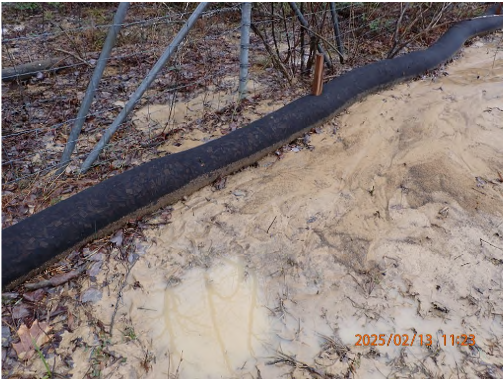
Sediment and sediment laden water discharging off the unpermitted site due to lack of maintenance.
