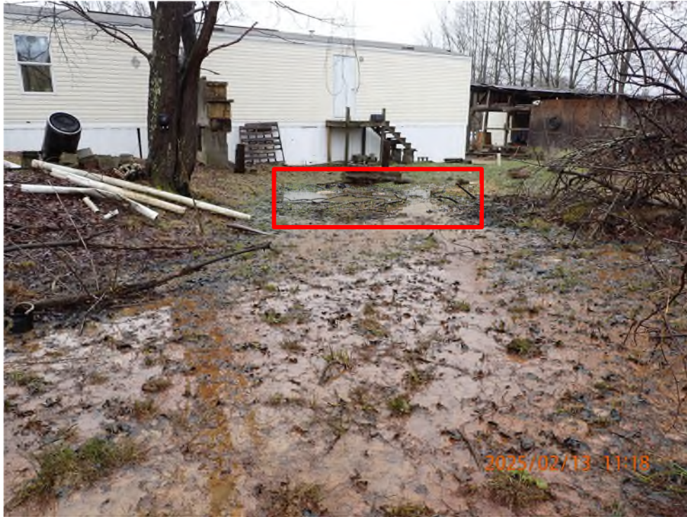
Sediment and sediment laden water discharging toward the existing culvert that discharges into the UNT of Sand Run.
