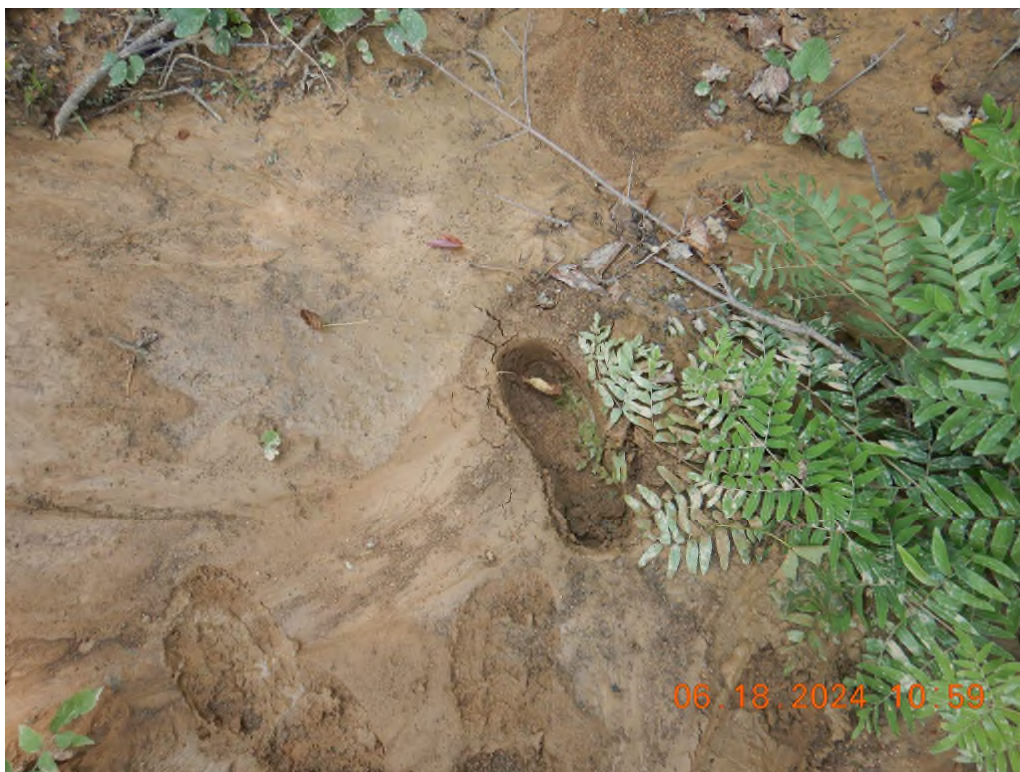
Example of sediment deposits at a low spot on the eastern side of the project. This sediment trail leads to an ephemeral stream (UNT of Sand Run).
