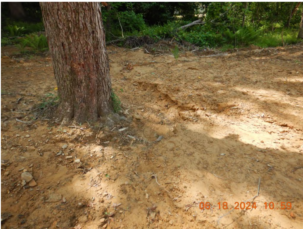
The erosion rills shown in the previous photograph have resulted in large amounts of sediment being carried off-site.
