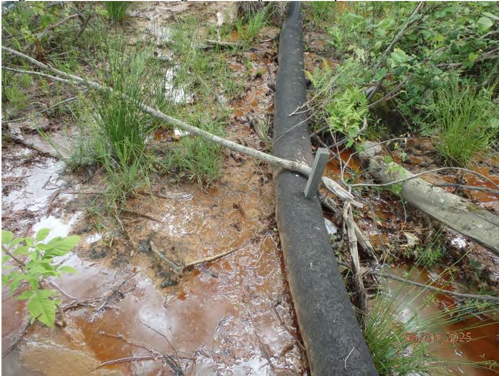
Perimeter control in the eastern portion of the project where sediment laden water bypassed due to the lack of maintenance.
