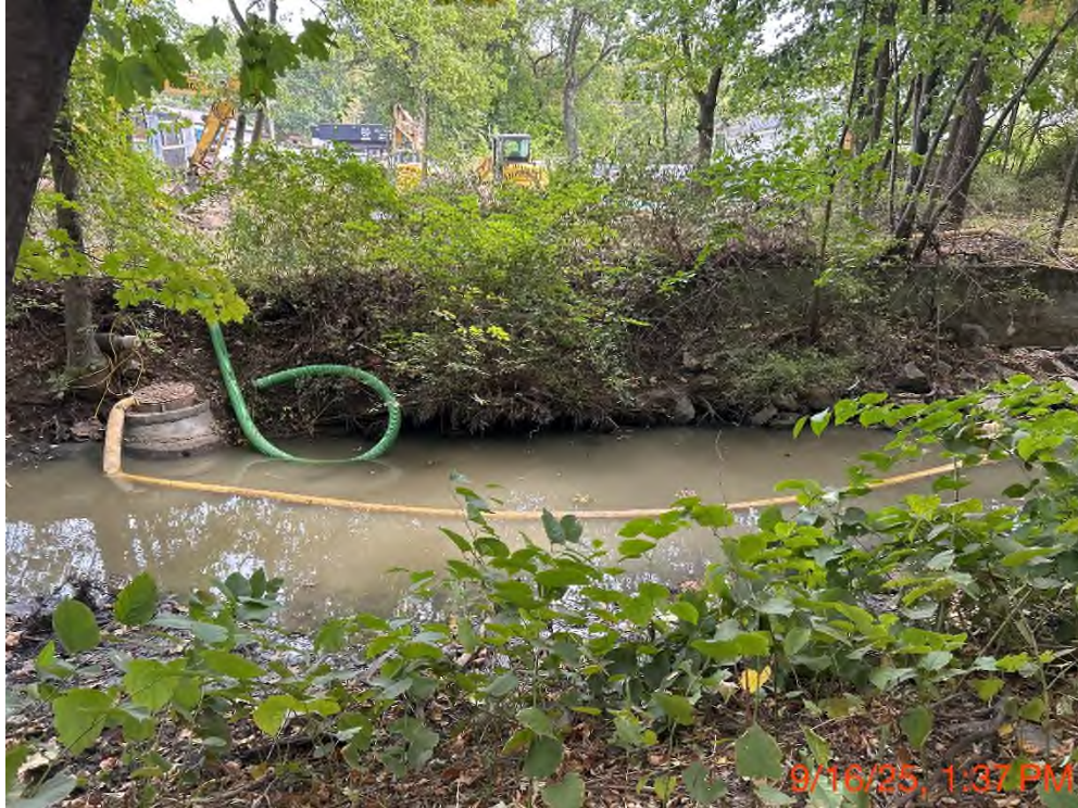
The sewer pump-around.
