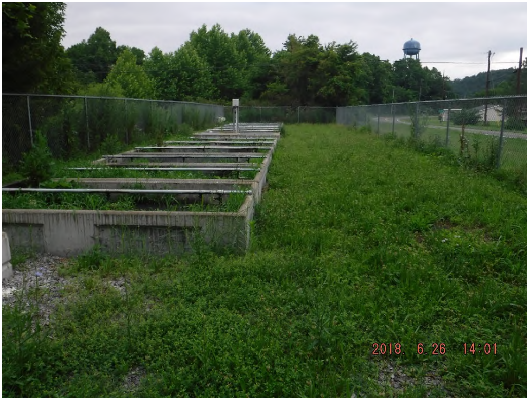
6/26/18- Sand filters with overgrown vegetation
