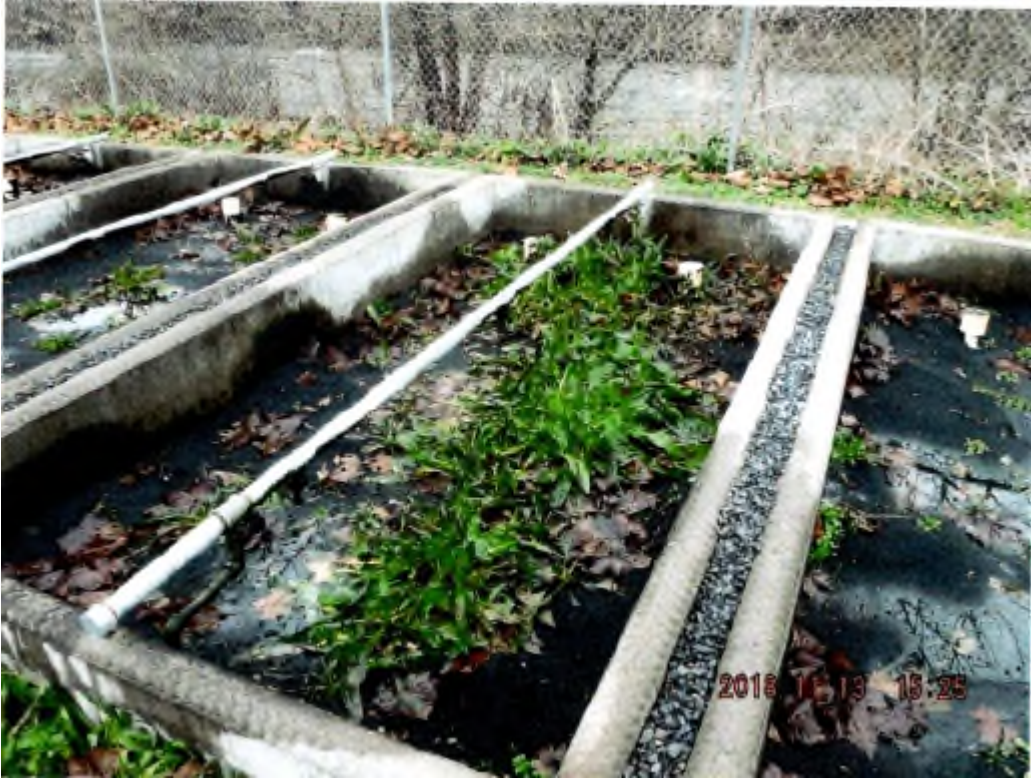
11/13/18- Sand filters with vegetation
