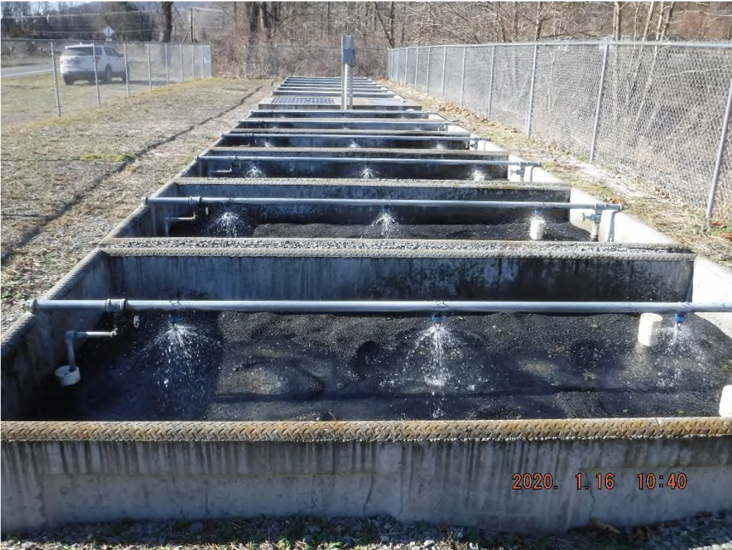
1/16/20- Wastewater entering the sand filters
