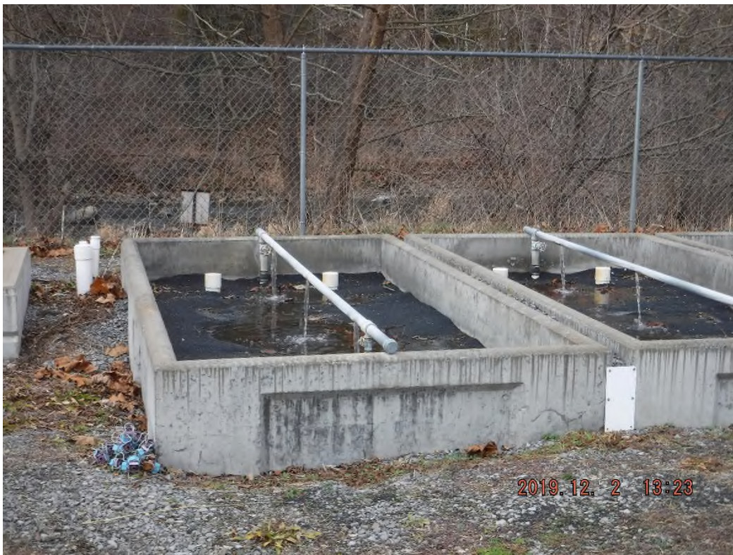
12/02/19- Wastewater entering the sand filters
