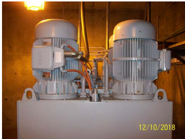
Electric Pump Motors Mounted on Reinforced Tank Top
