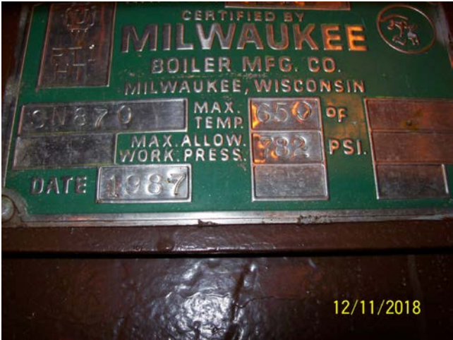
Tank Manufacture Plate
