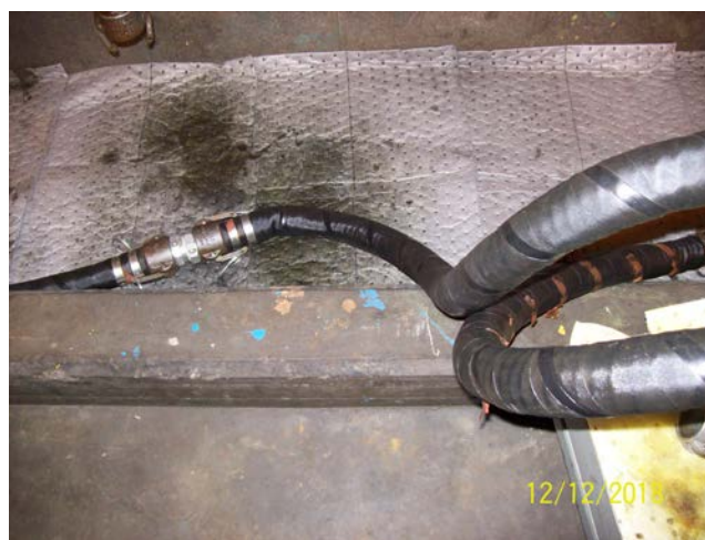
Discharge & Filling Station Containment
