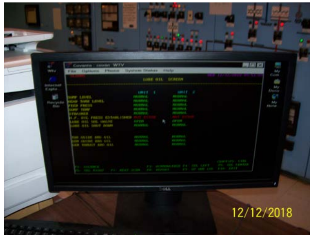
Tank Remote Level Monitor Control Room
