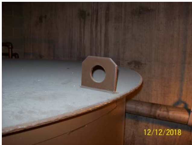
Tank Roof Welded To Shell & Lifting Lug
