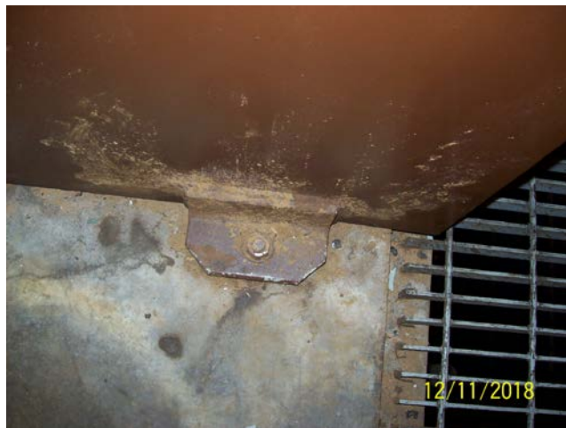
Containment Catch Basin To Basement
