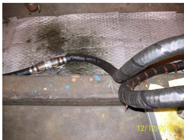
Discharge & Filling Station Containment
