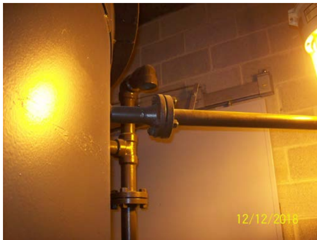
Tank Atmospheric Vent
