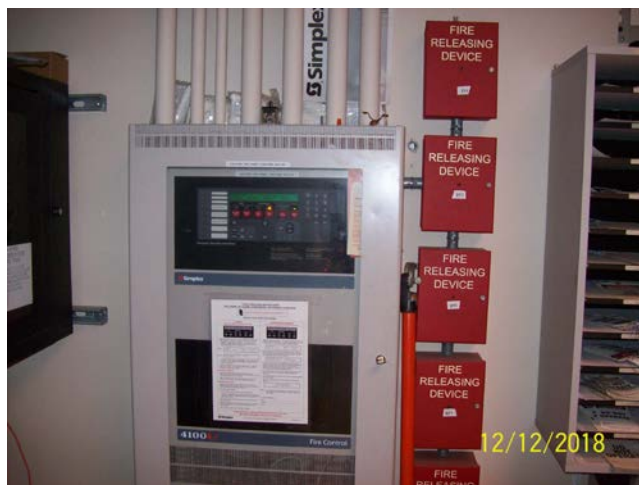
Lube Room Fire Monitoring In Control Room
