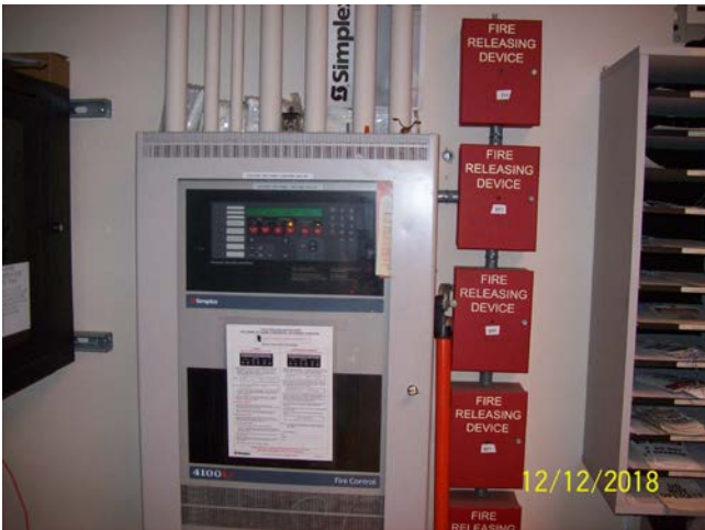
Lube Room Fire Monitoring In Control Room
