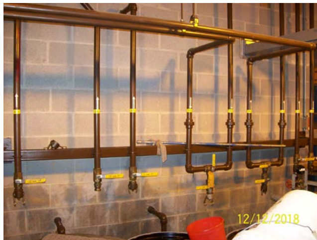
Lube Tanks Filling Station
