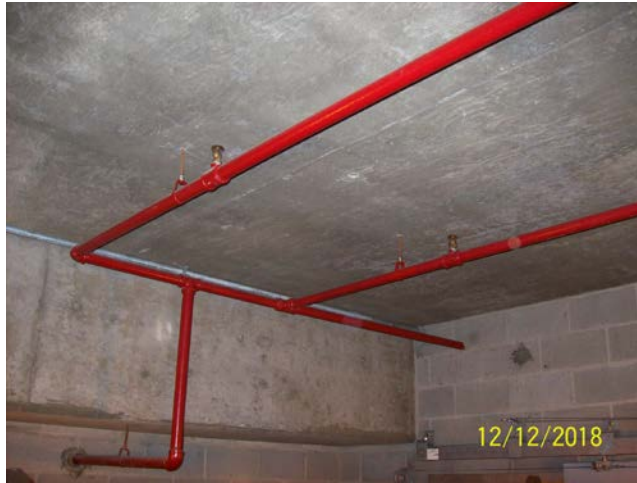
Lube Room Fire System
