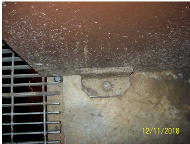
Foundation – Concrete Pad & Anchor Bolt
