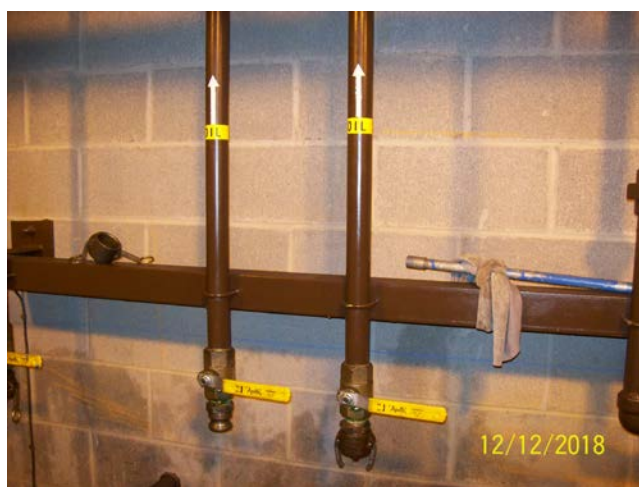
Tank Fill Station
