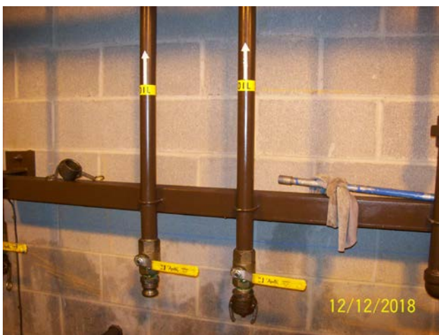
Tank Fill Station
