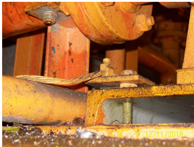
Tank Ground Strap
