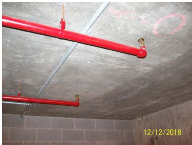
Lube Room Fire System
