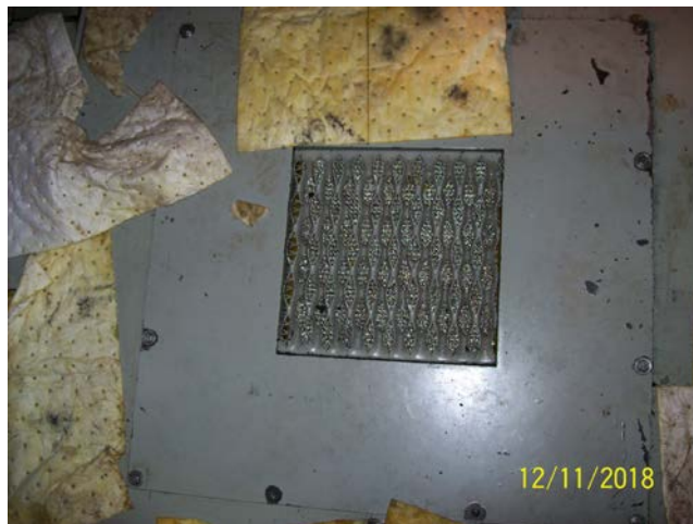
Tank Inspection Manway
