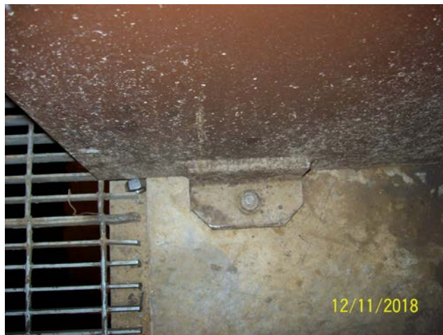
Containment Catch Basin To Basement
