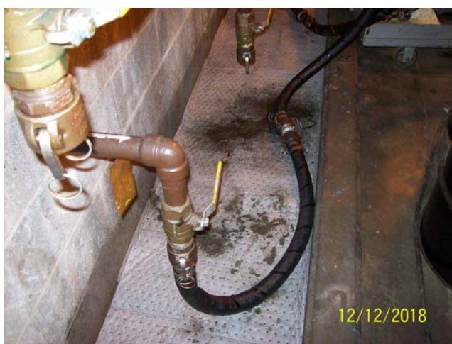
Discharge & Filling Station Containment
