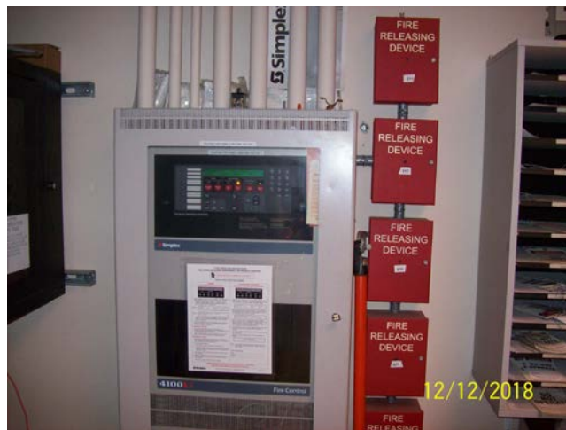
Tank Remote Fire Monitoring System Control Room
