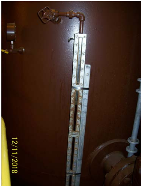
Tank Level Indicator Gauge
