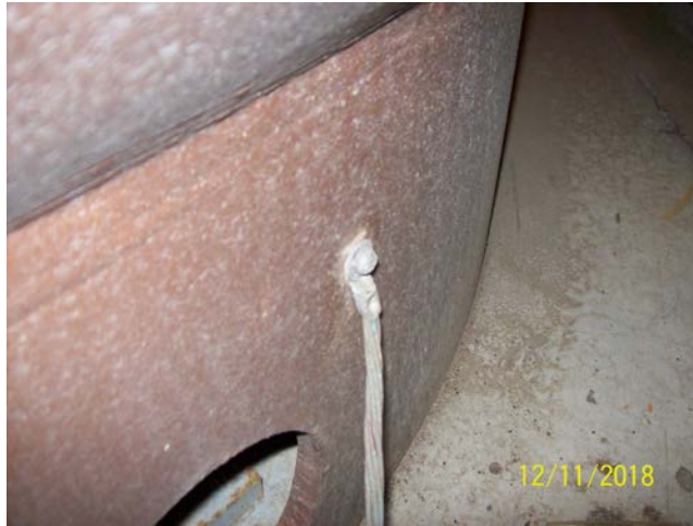
Tank Ground Strap
