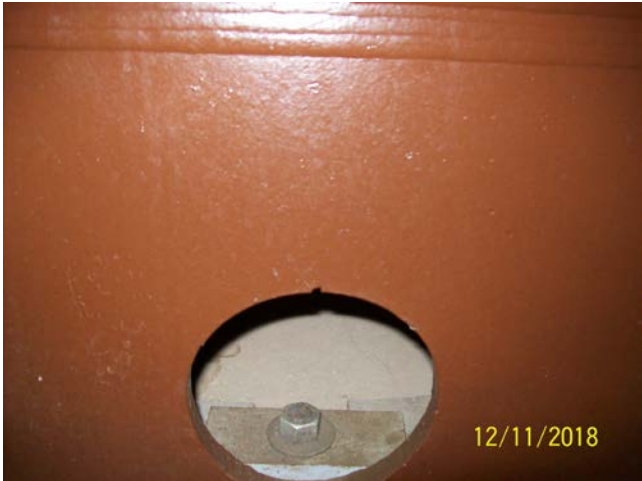
Tank Anchor Plates
