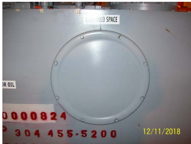
1 of Two Tank Inspection & Entry Man-holes 18"
