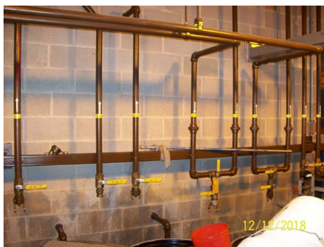
Lube Tanks Filling Station
