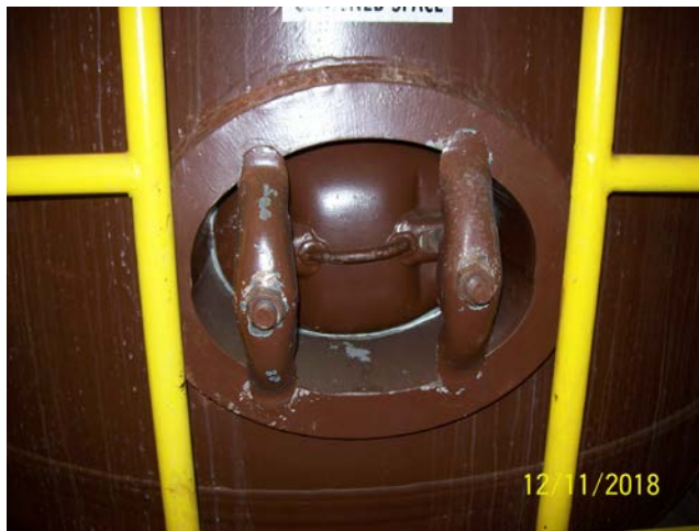
Tank Inspection Manway
