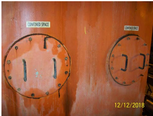
Tank Inspection Manways
