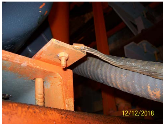
Tank Ground Strap
