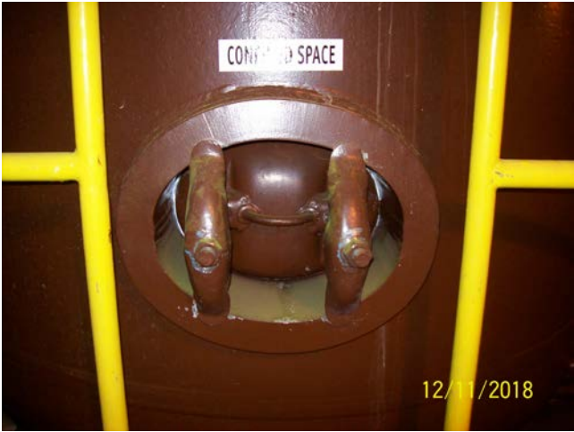
Tank Inspection Manway
