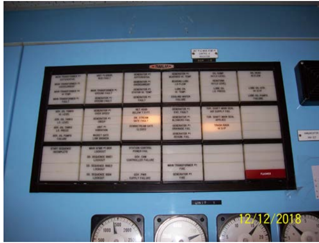
Tank Remote Level Monitor Control Room
