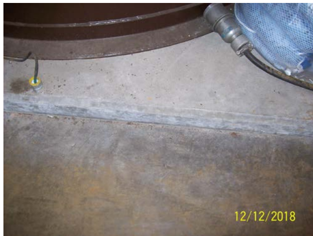
Tank Foundation & Ground Rod
