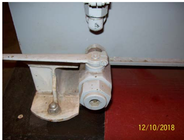
Tank Anchor Bolt and Drain Valve
