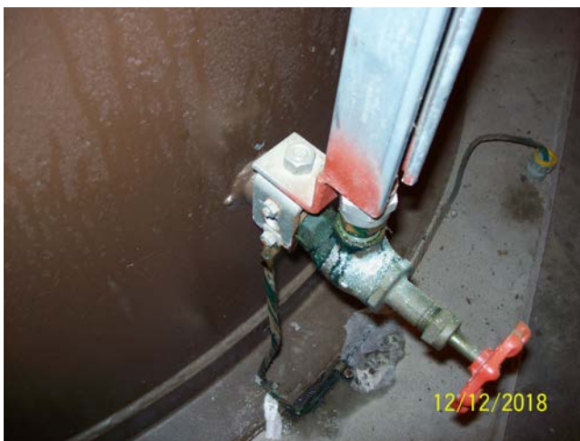
Tank Ground Strap
