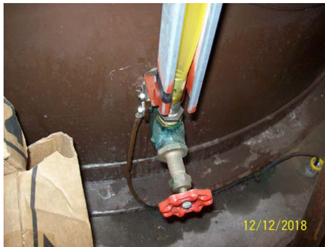
Tank Ground Strap
