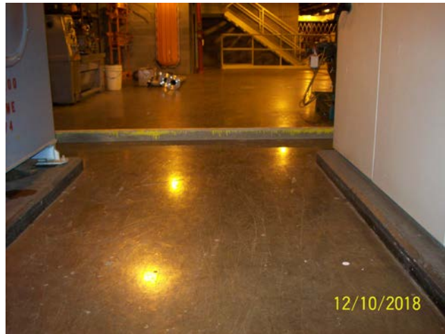
Concrete Containment Dike
