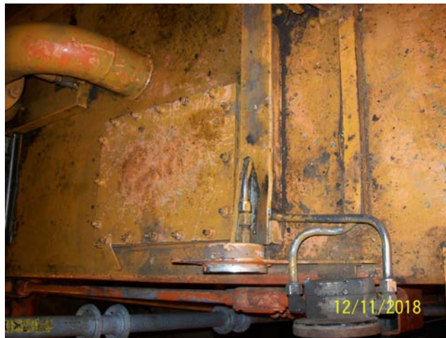
Tank Inspection Port
