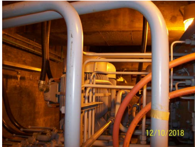
Tank Fill & Vent Piping 3”
