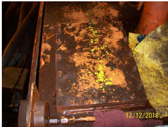
Tank Inspection Port
