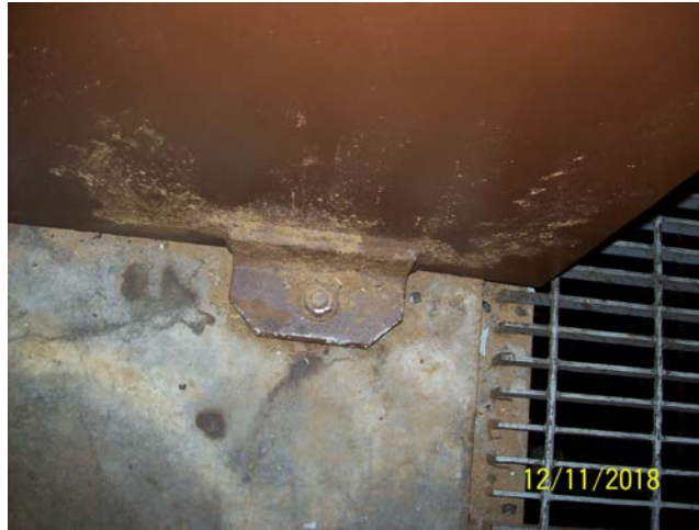
Tank Anchor Bolt and Drain Valve
