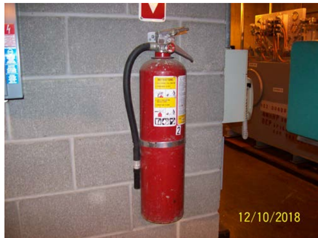
Tank Area Hand Held Fire Extinguisher
