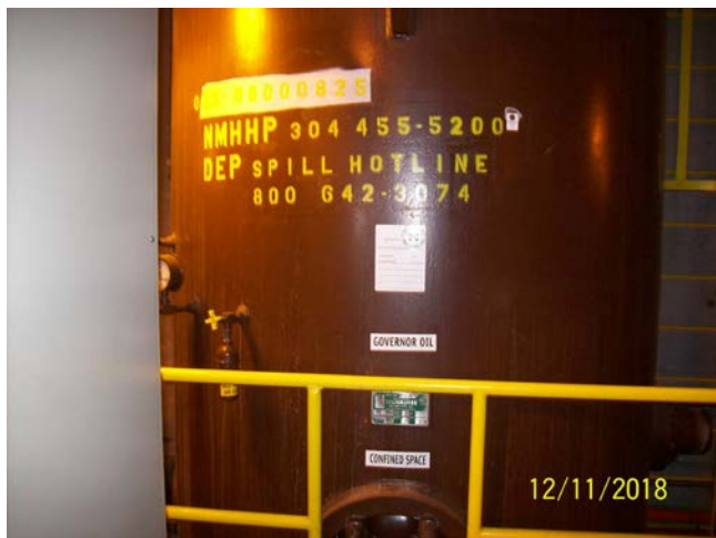
Tank Id & Emergency Contacts
