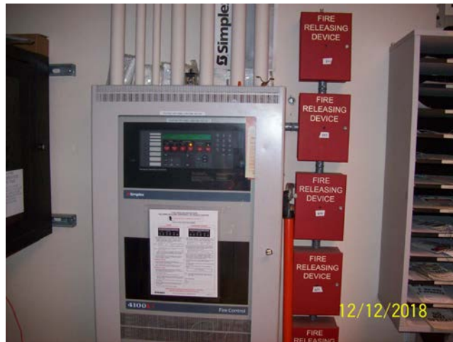
Tank Remote Fire Monitoring System Control Room
