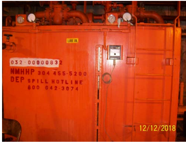
Tank Identification & Emergency Contact Numbers
