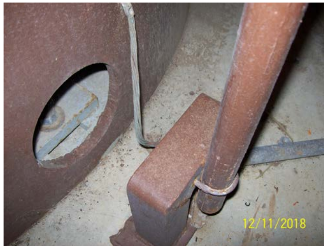
Tank Anchor Plates
