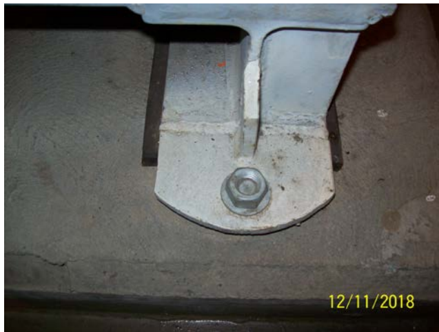
Foundation – Concrete Pad & Anchor Bolt
