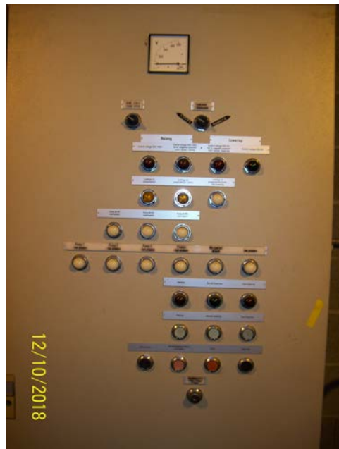
Pumps Motor Control Panel
