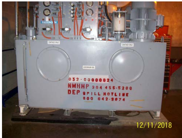
Tank Identification & Emergency Contact Numbers
