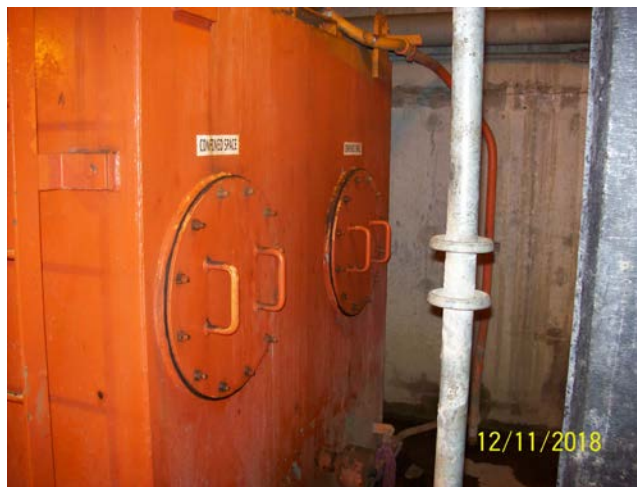
Tank Inspection Manways
