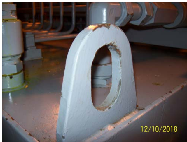
One of Five Lifting Lugs
