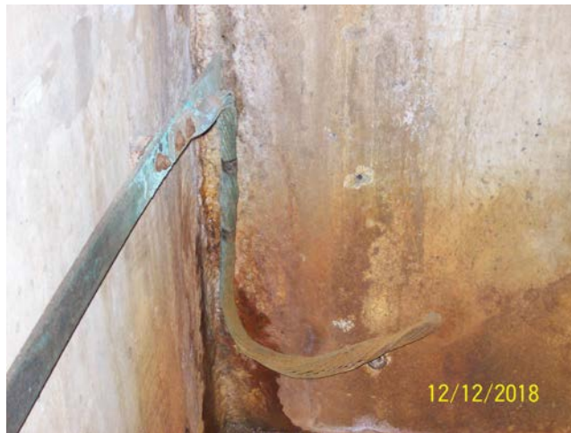
Tank Ground Bar
