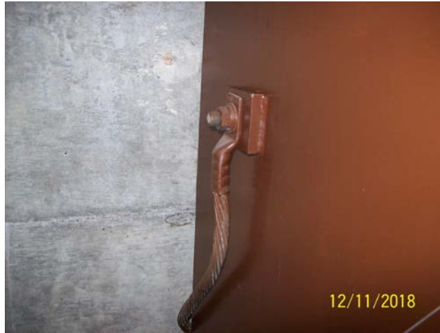
Tank Ground Strap and Anchor Bolt
