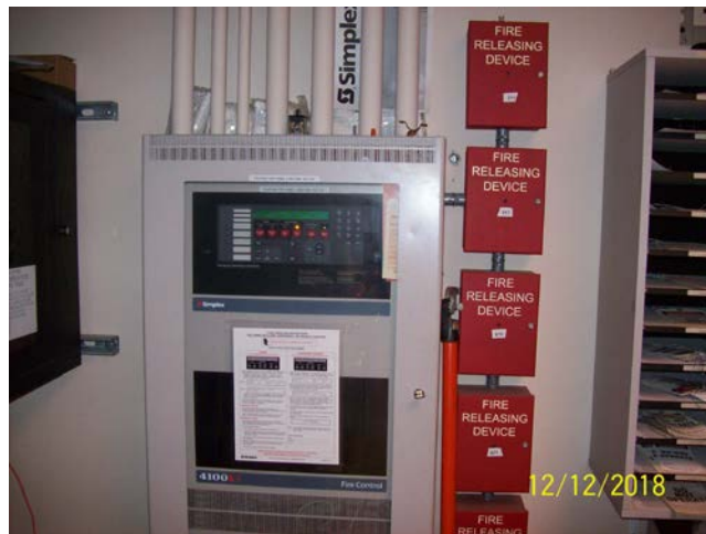
Tank Remote Fire Monitoring System Control Room
