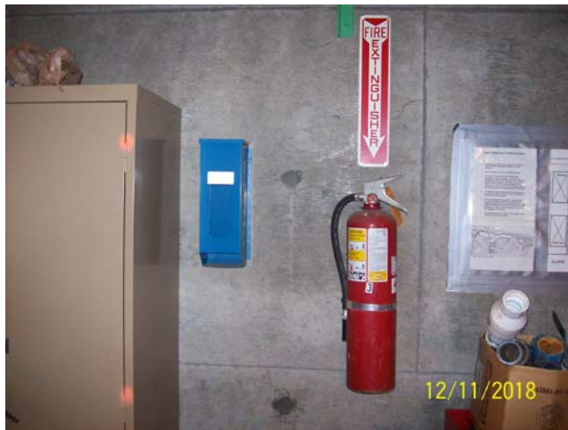
Tank Area Han Held Fire Extinguisher
