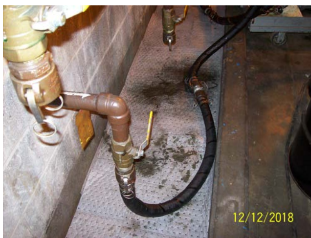
Discharge & Filling Station Containment
