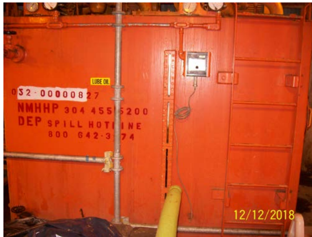
Tank Identification & Emergency Contact Numbers
