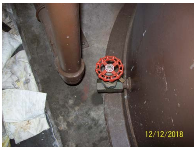
Tank Drain Line
