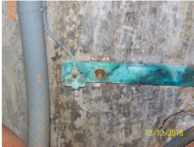
Tank Ground Bar
