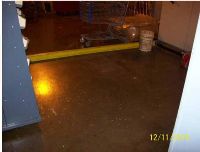
Concrete Containment Dike
