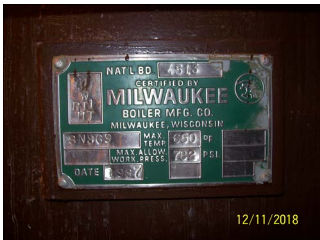
Tank Manufacture Plate
