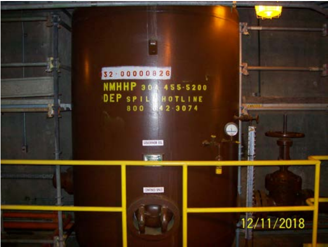
Tank Id & Emergency Contacts
