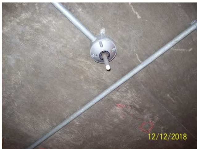
Lube Room Heat Sensor
