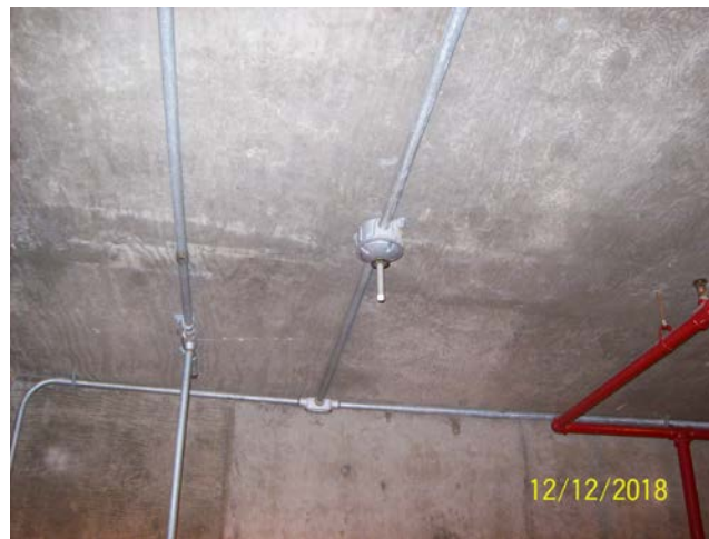
Lube Room Heat Sensor
