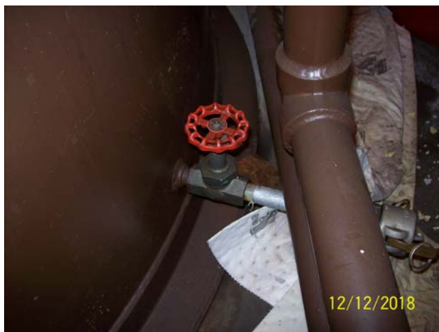
2" Discharge Line & Tank Drain Line
