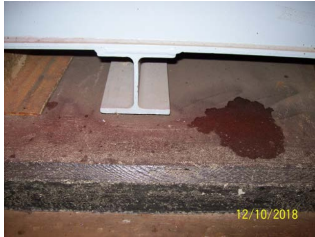
One of Four Tank I Beam Tank Supports
