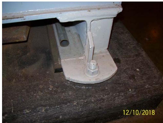
Foundation – Concrete Pad & Anchor Bolt
