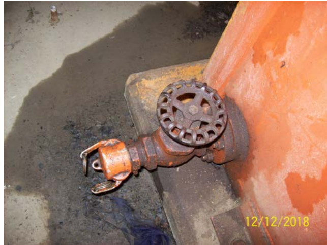
Tank Anchor Bolt and Drain Valve
