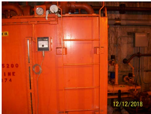
Ladder Tank Top Access
