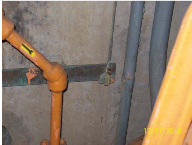
Tank Ground Strap
