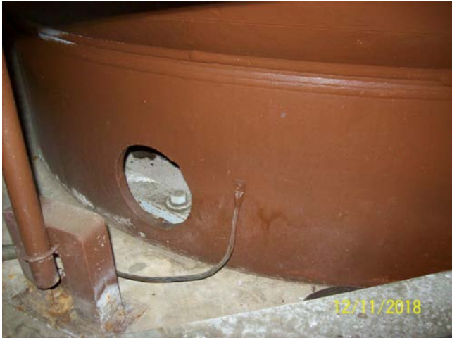
Tank Ground Strap
