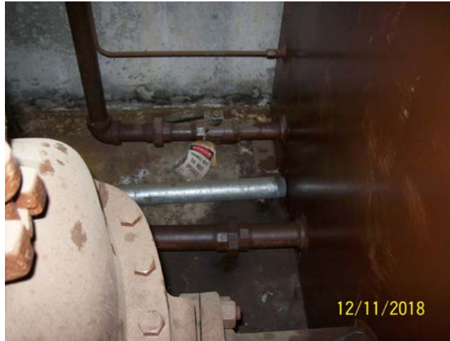
Tank Anchor Bolt
