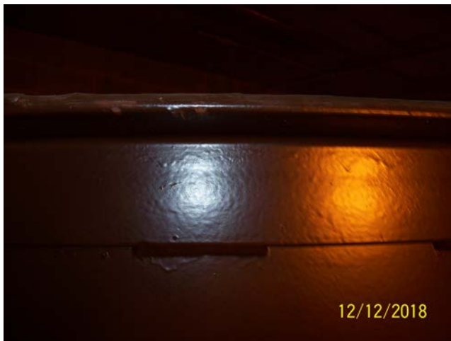
Tank Roof Welded To Shell
