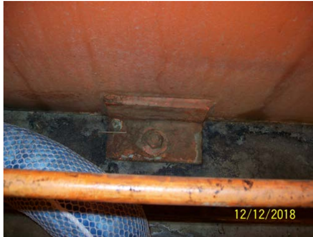
Tank Anchor Bolt
