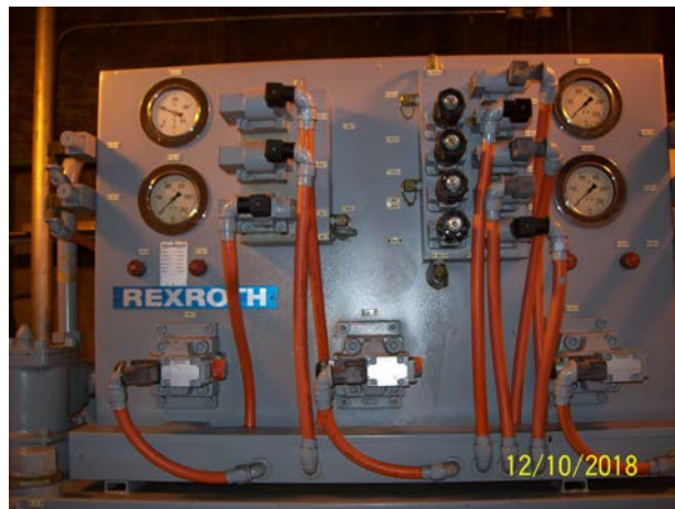
Oil Issue Control Panel
