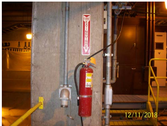
Hand Held Fire Extinguisher
