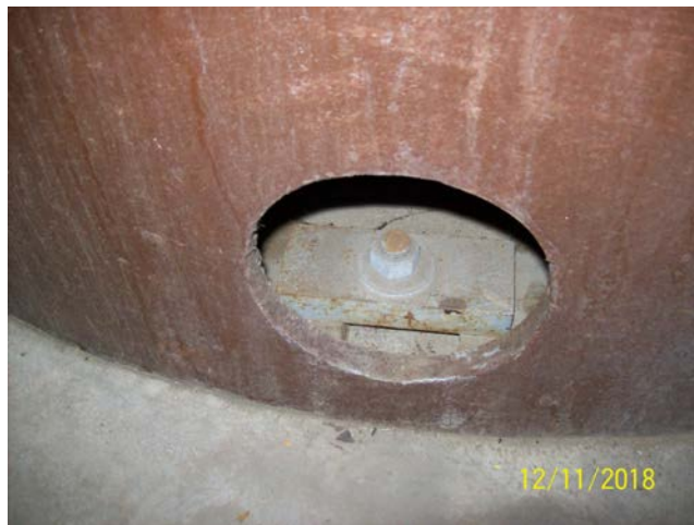
Tank Anchor Plates
