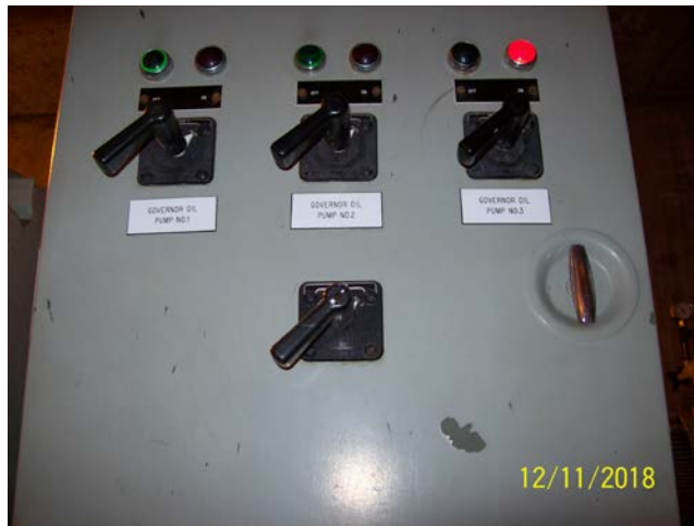
Oil Pump Controllers
