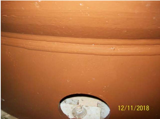
Tank Anchor Plates
