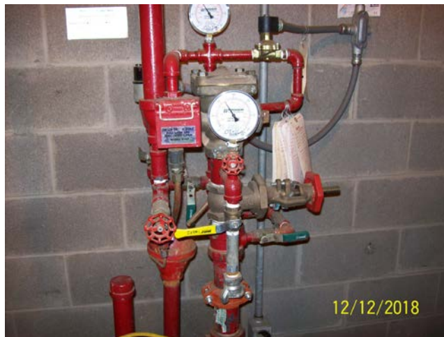
Lube Room Fire Protection
