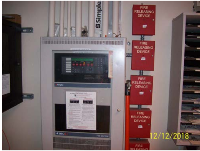
Lube Room Fire Monitoring In Control Room
