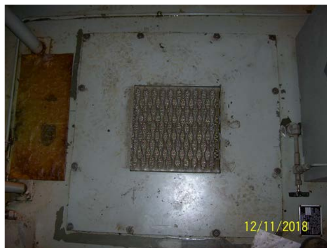
Tank Inspection Manway
