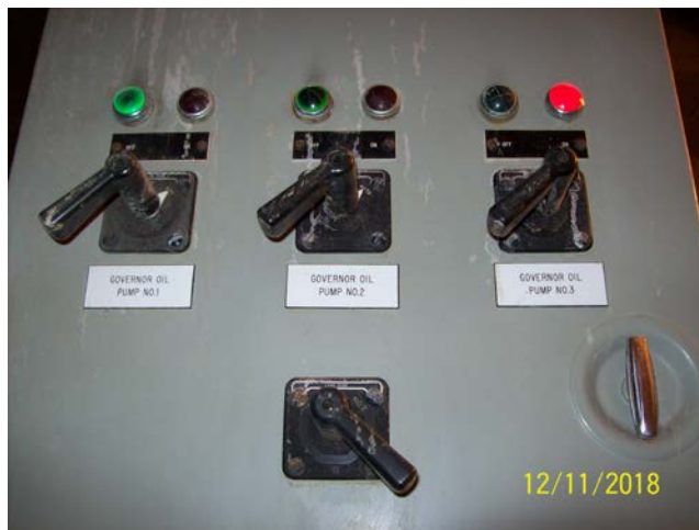
Oil Pump Controllers
