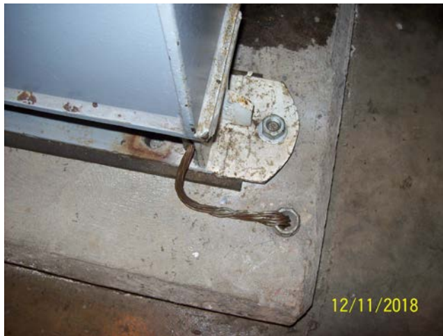
Tank Ground Strap and Anchor Bolt
