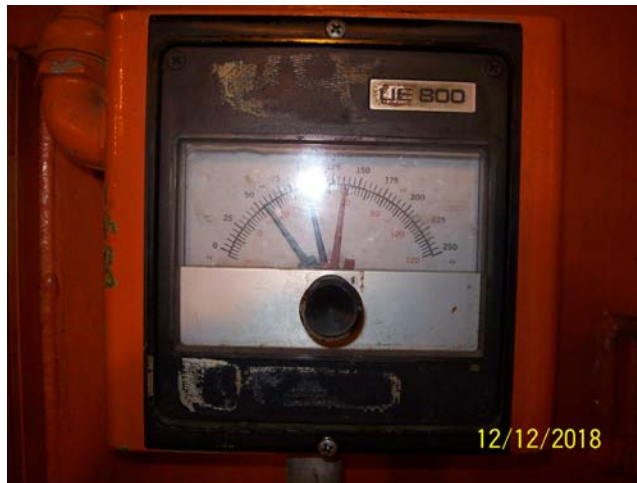
Tank Temperature Control
