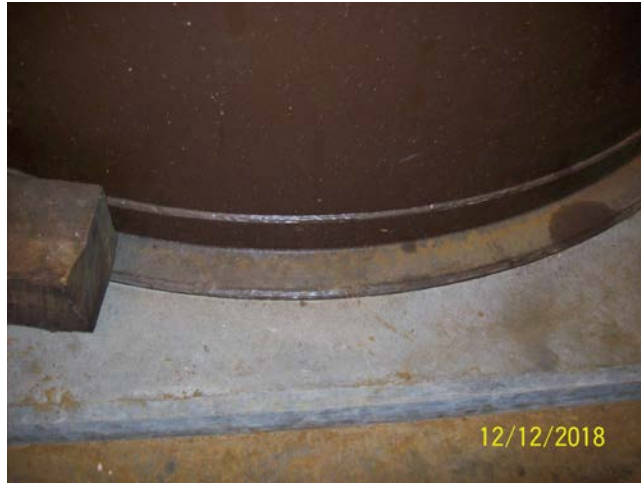
Tank Foundation & Tank Bottom Chime
