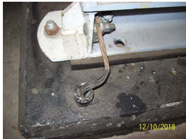
Tank Ground Strap
