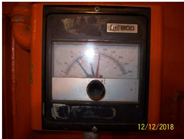
Tank Temperature Control
