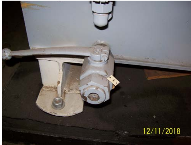
Tank Anchor Bolt and Drain Valve
