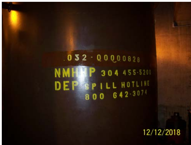
Tank Id & Emergency Contacts
