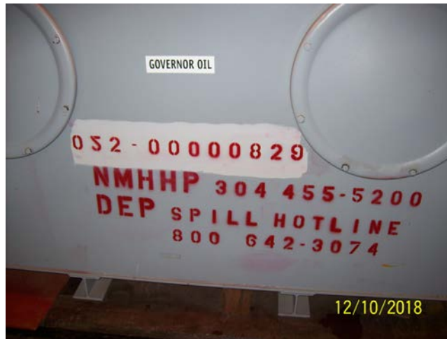
Tank Identification & Emergency Contact Numbers
