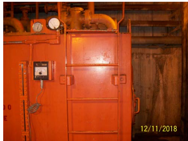
Ladder To Tank Top Access
