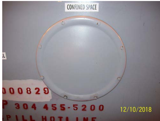
1 of Two Tank Inspection & Entry Man-holes 18”
