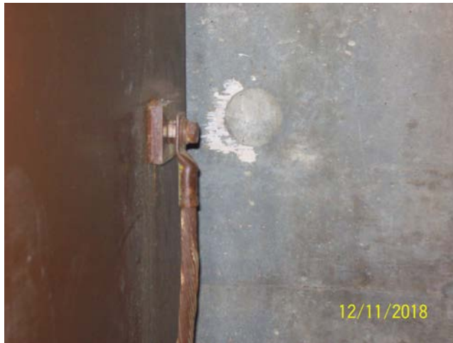
Tank Ground Strap
