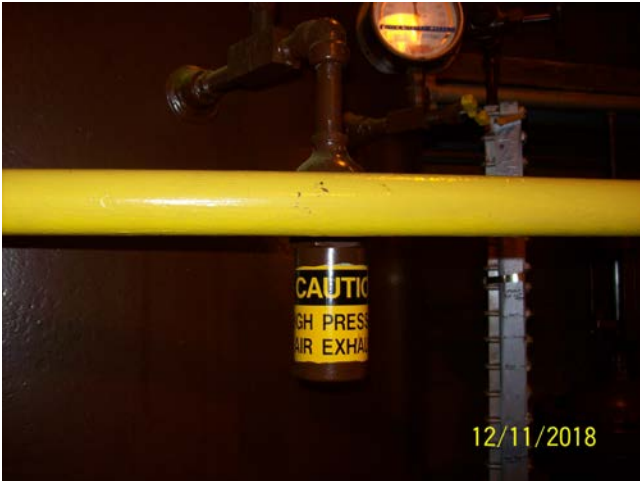
Tank High Pressure Air Exhaust
