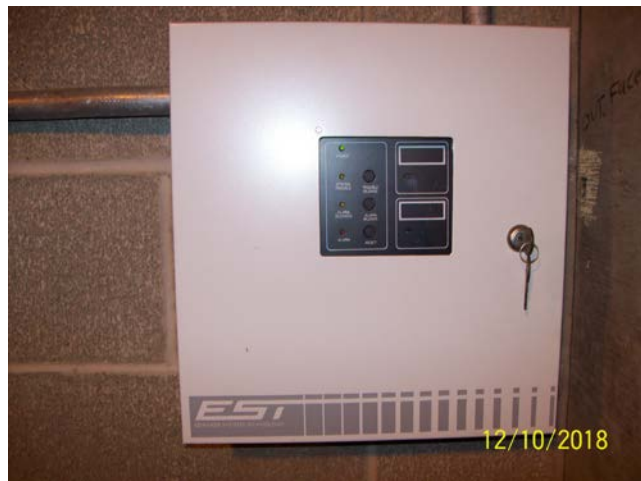
Tank Fire Control Panel Monitored From Control Room
