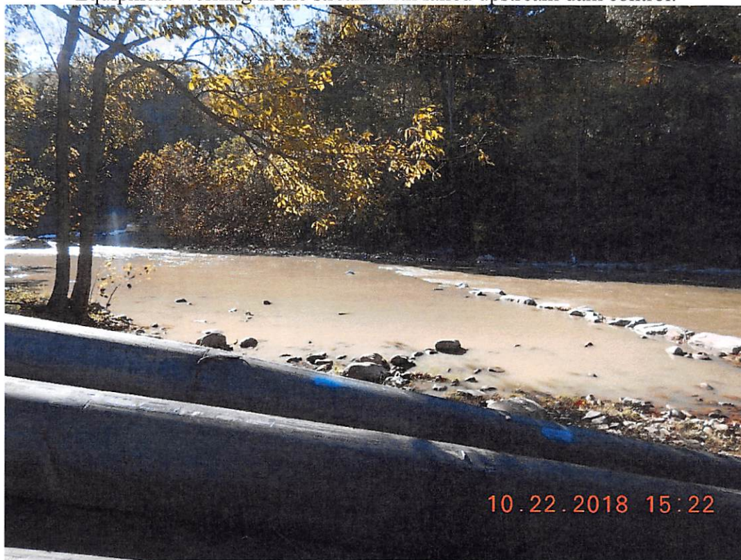
CNA and sediment laden water between the upstream dam and the discharge lines.
