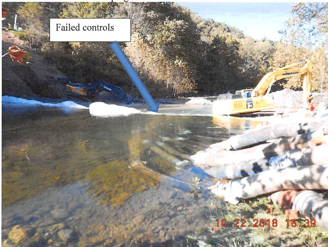
Approximately 20 intake lines pictured above upstream dam. Upstream dam control failed.
