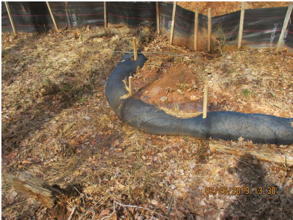
Waterbar terminus at station #6752+00. Evidence of concentrated flow due to control being undermined and erosion occurring between devices.
