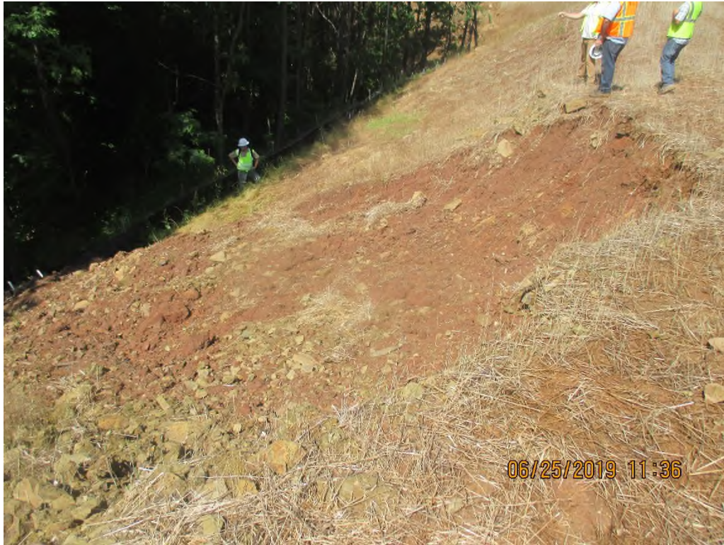
Slip area next to waterbar terminating onto slope at station No. 5355+67.
