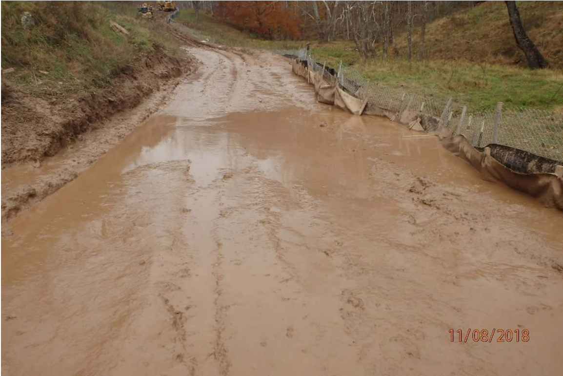
ARDO08.5 showing concentration of mud in a low area adjacent to the receiving stream due to a lack of upslope ditching to handle run-on stormwater and poor maintenance.
