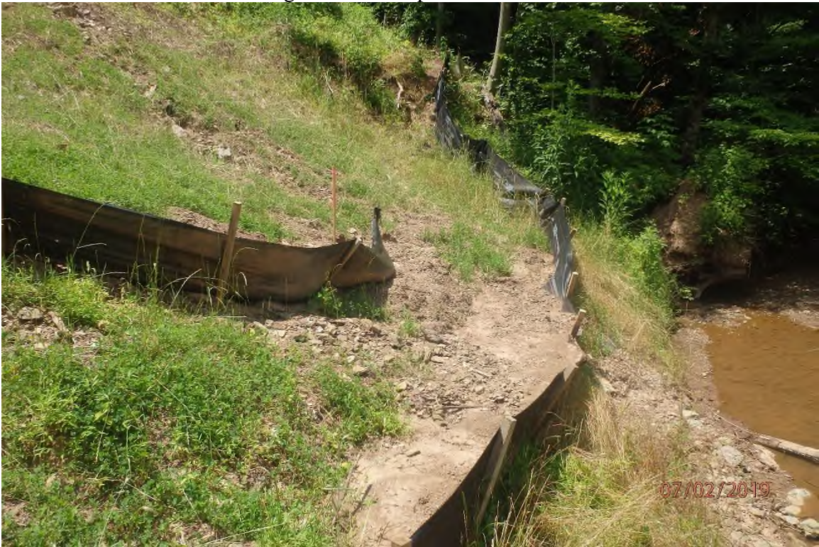
Erosion gullies that run from the top of the slope to the bottom of the slope adjacent to UNT Left Fork of Arnolds Creek (SDOG040) due to poor maintenance of installed water bars. Concentrated flow stormwater is overwhelming the installed perimeter controls at the base of the hill.
