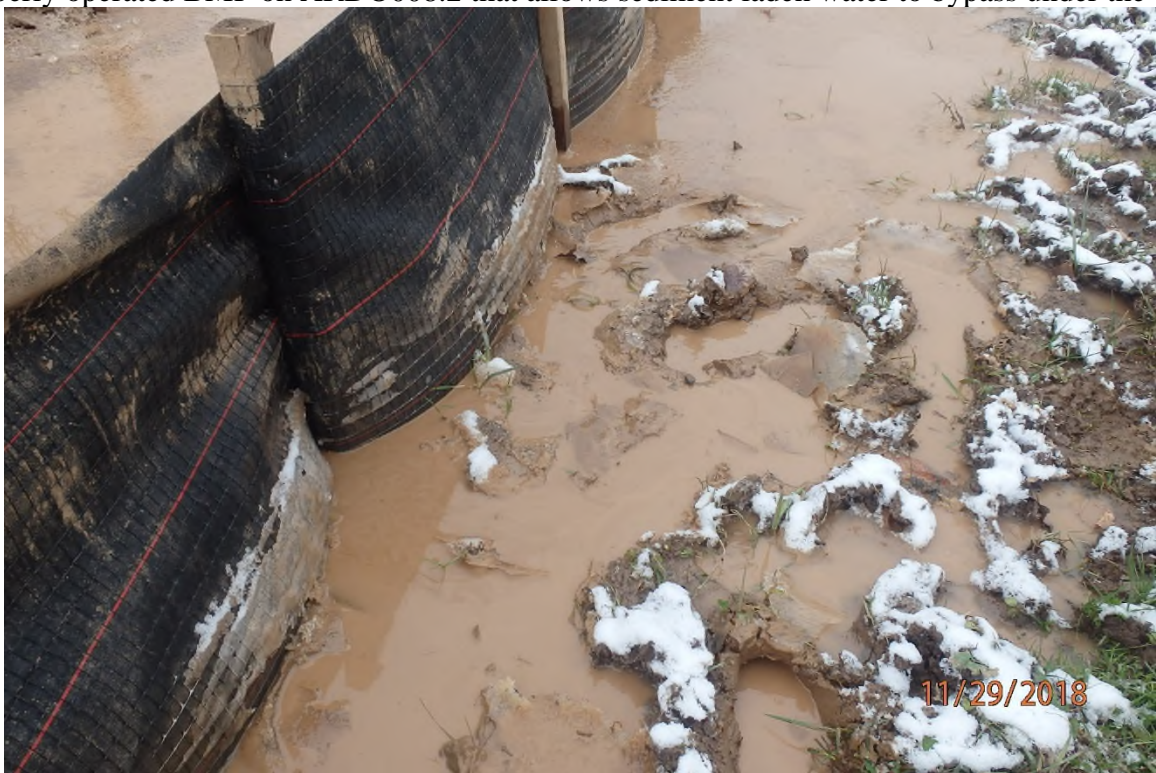
Improperly operated BMP on ARDO008.2 that allows sediment laden water to bypass under the device.
