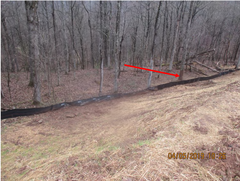
Area where past slip had occurred near station #6795+40. Arrow depicts stain lines on trees from slip. Slope had sediment being deposited behind controls.
