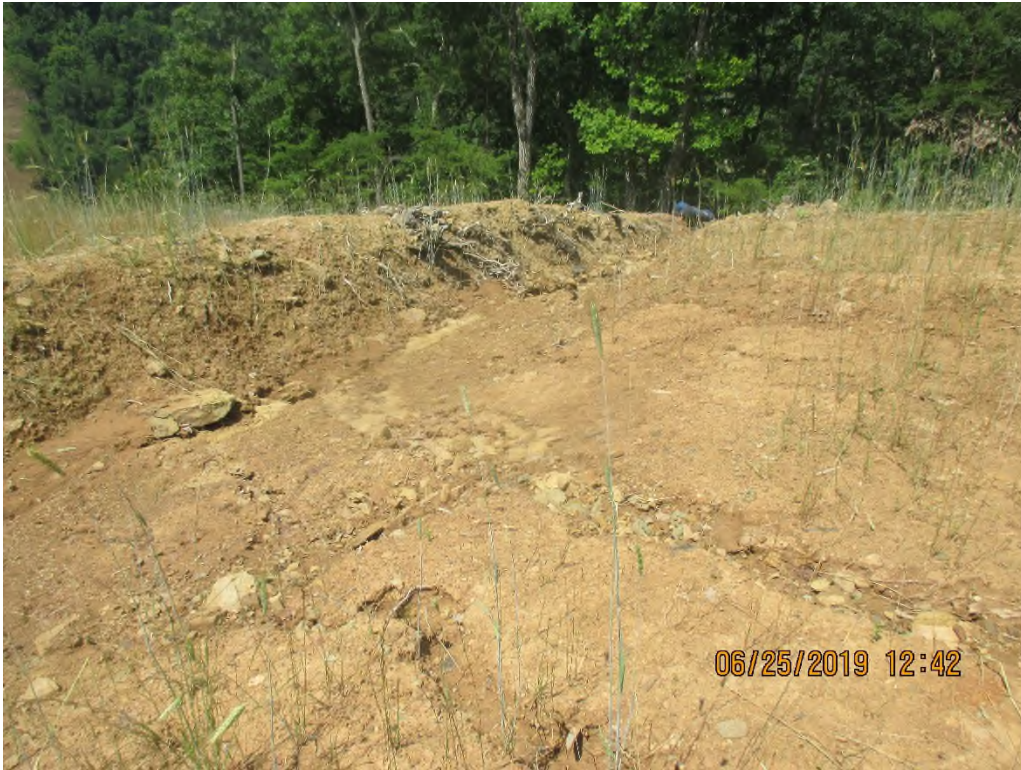
Erosion occurring on slope above waterbar at station No. 5396+00
