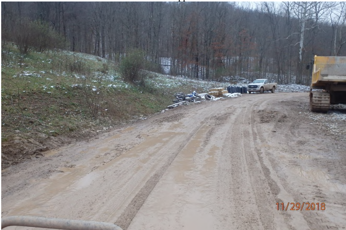
ARDO009.3 showing an unstable road surface that requires construction activity with no BMPs in place as indicated in the approved SWPPP.
