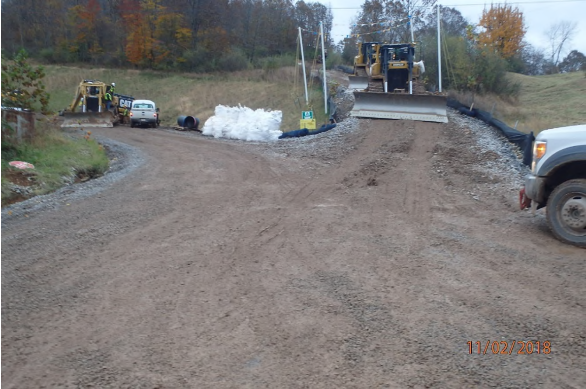
AR-20 (ARDO-001.5) showing an unstable construction entrance that is causing track-out onto the public road.
