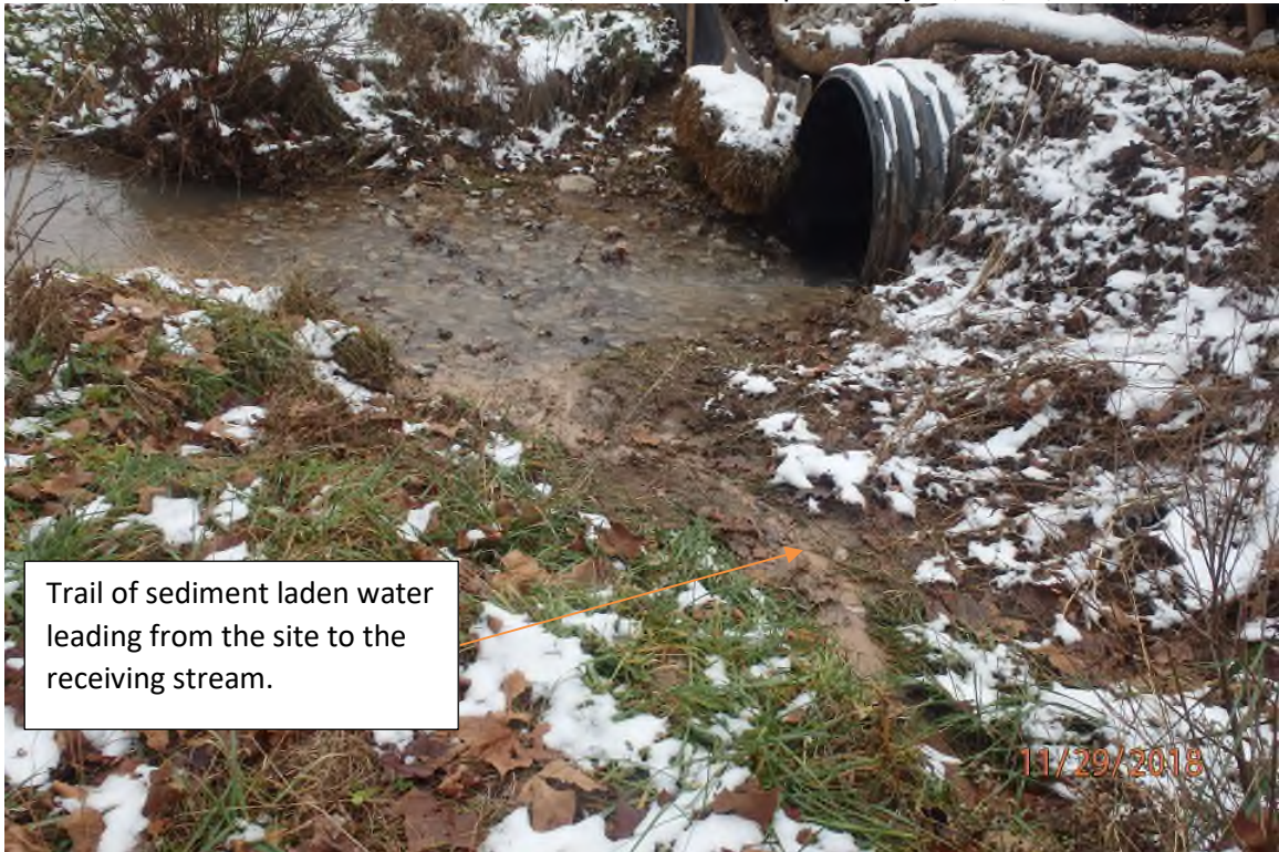
Trail of sediment laden water leading to the receiving stream from the previously pictured BMP on ARDO008.2.
