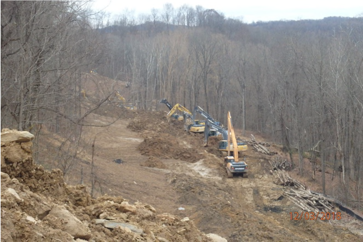
Work being conducted to mitigate the slip associated with spill report number 09-83236 (A).
