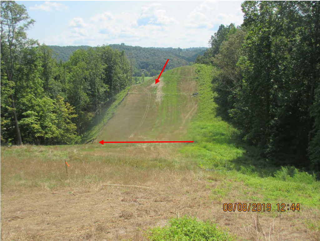
Near station No. 8772+72 facing South. Arrow depicts slip area and drainage point in between slopes leading to overwhelmed perimeter controls.
