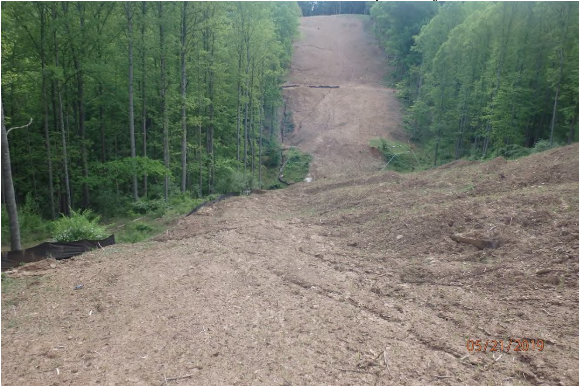
Unmaintained water bars in the Taylor Drain watershed and the associated fill slope erosion.
