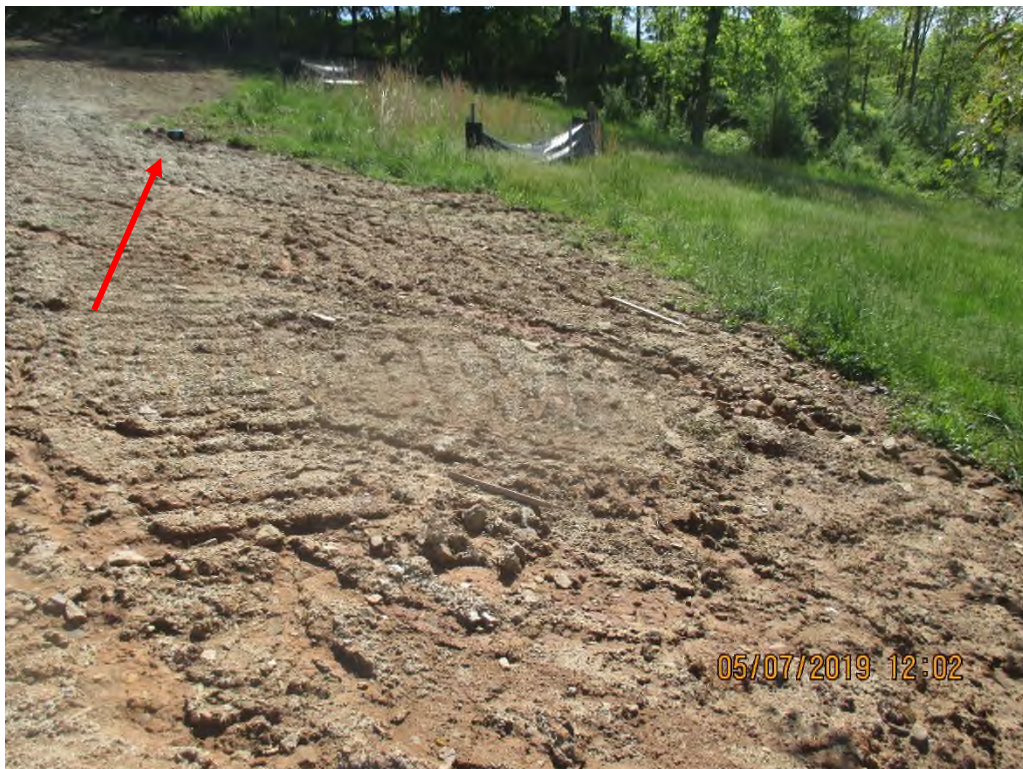
Downslope of slope drain outlet on west slope above LOD. Arrow depicts slope drain. Erosion present on slope, depositing sediment into and through perimeter controls.
