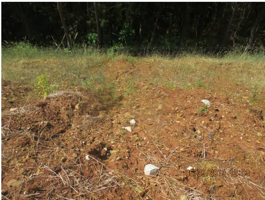
Erosion occurring on slope next to topsoil pile near station No. 5355+67.
