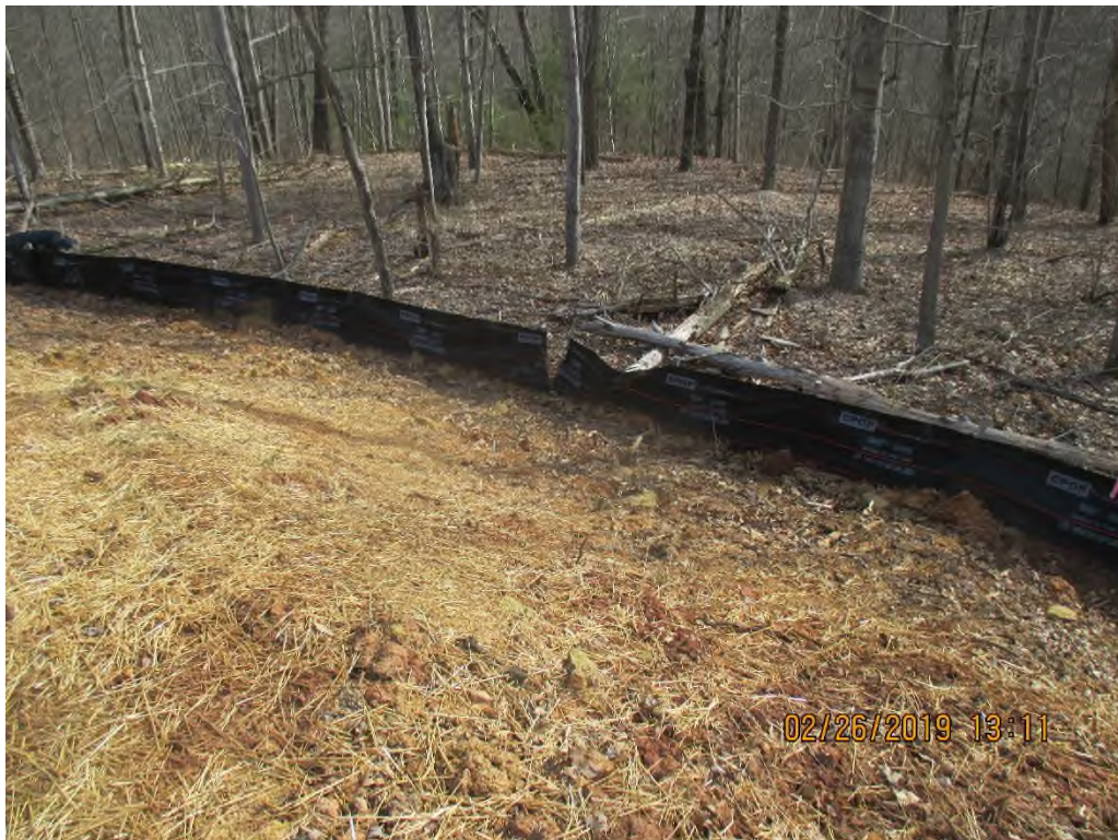
Ripped silt fence on downslope perimeter near station #6766+60
