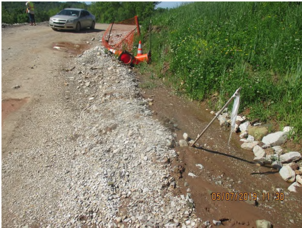
Sediment deposited in ditch downslope of erosion observed on South slope of compressor station pad.
