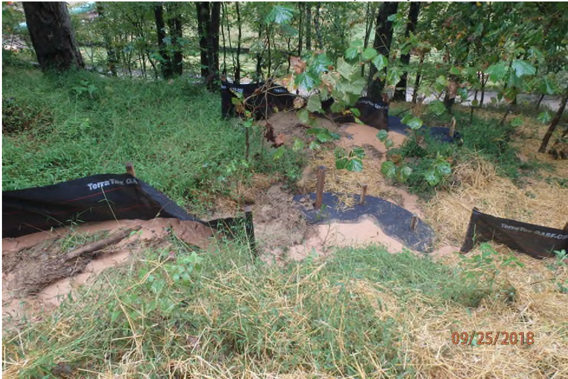
Installed BMPs adjacent to ARDO002.8 that are not being properly operated or maintained and are allowing sediment laden water to bypass the devices.
