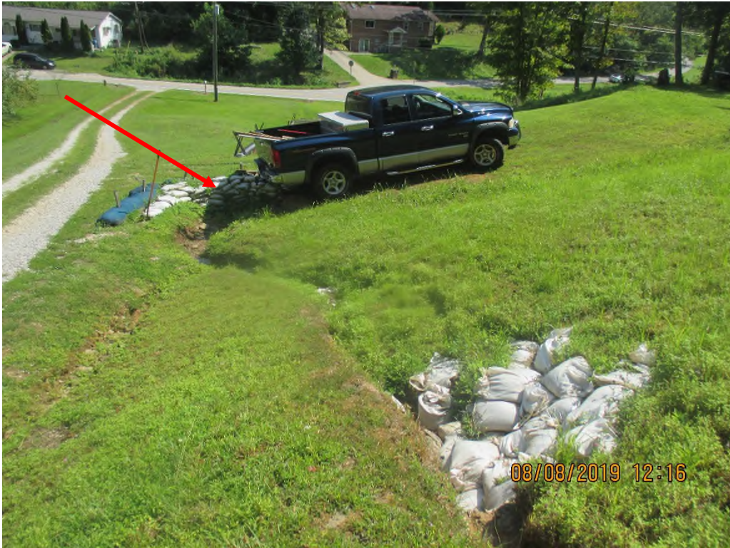
Sandbags installed to stabilize ditch. Arrow depicts where slope drain inlet was located.
