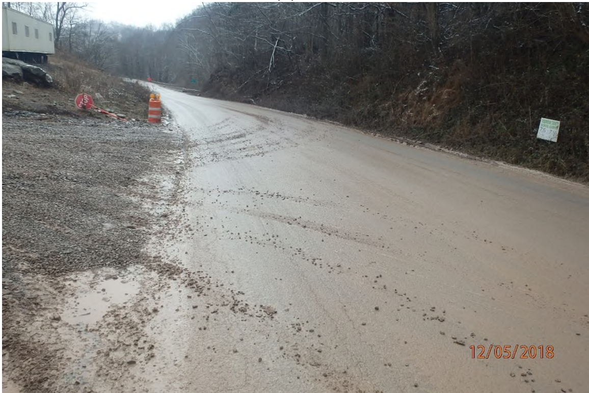
The construction access road to WV 18 showing the ineffectiveness of the construction entrance at preventing track-out onto the public roadway.
