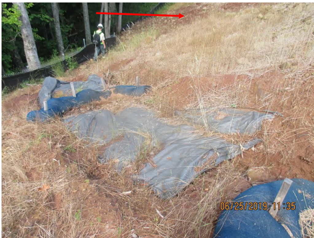
Controls below waterbar outlet terminating onto fill slope causing erosion on slope at station No. 5355+67. Arrow depicts slip area next to outlet.
