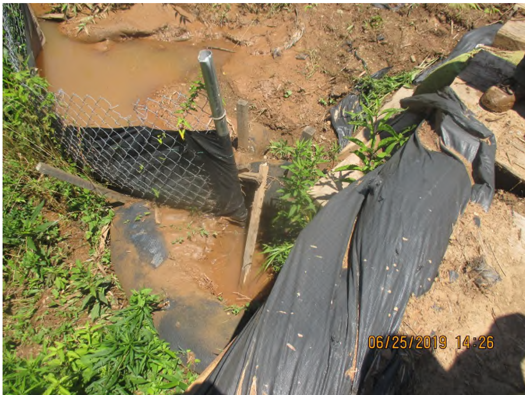
Controls overwhelmed with sediment at bridge crossing (North side) of Stream SROC 029 near station No. 5638+46.
