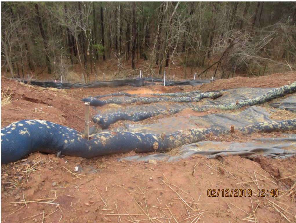
Waterbar outlet at station 5376+00
