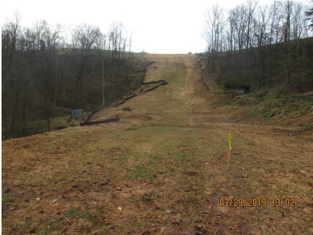
Section of ROW with multiple slips near station #5180+43.
