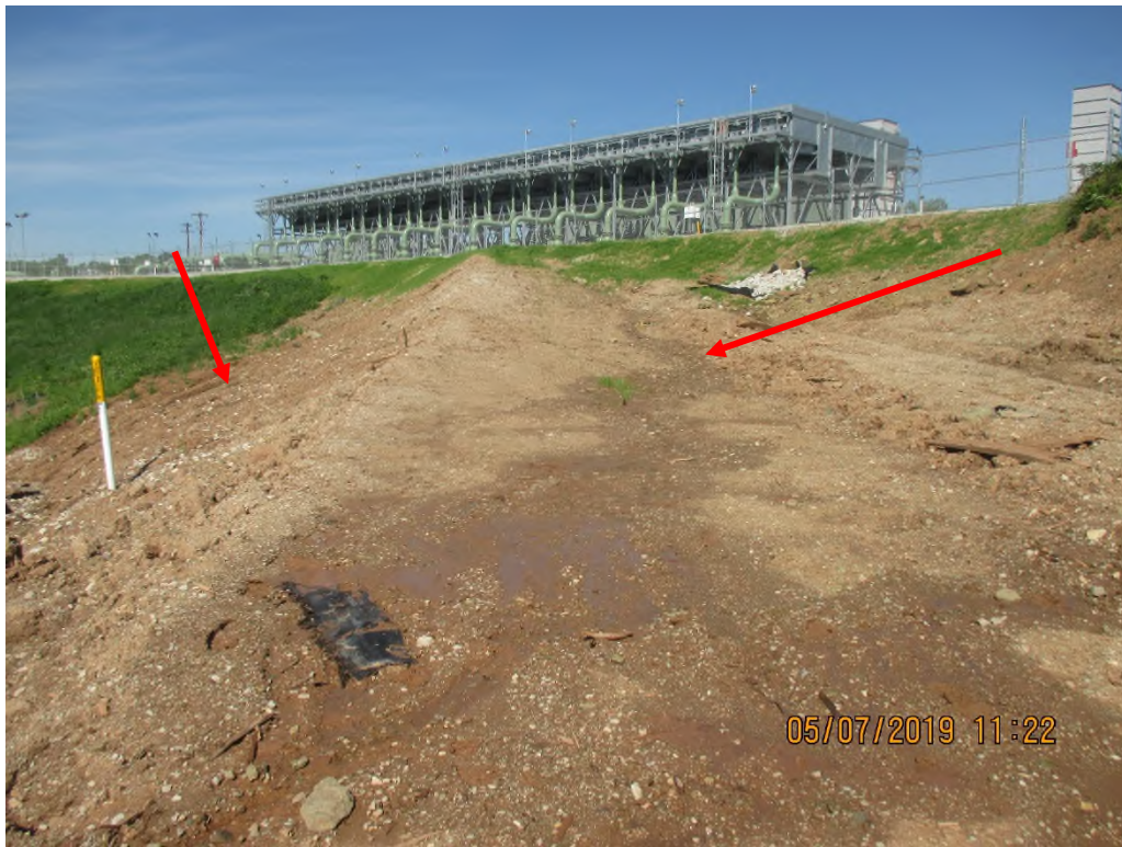
View facing upslope at South slope. Arrows depict swale outlet and erosion occurring from run-off from pad.
