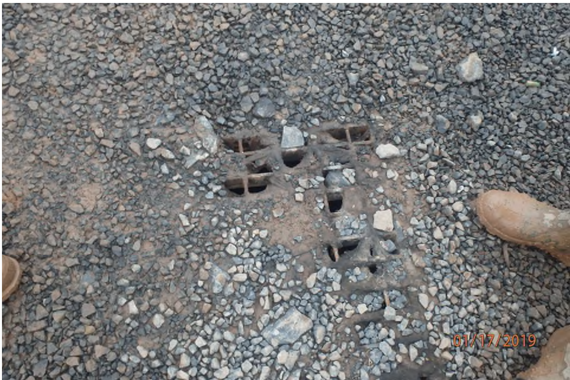
Drop inlet protection in need of maintenance.
