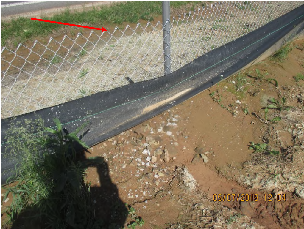
Super silt fence with sediment deposited above, below, and into roadside ditch. Arrow depicts off-site sediment deposits.
