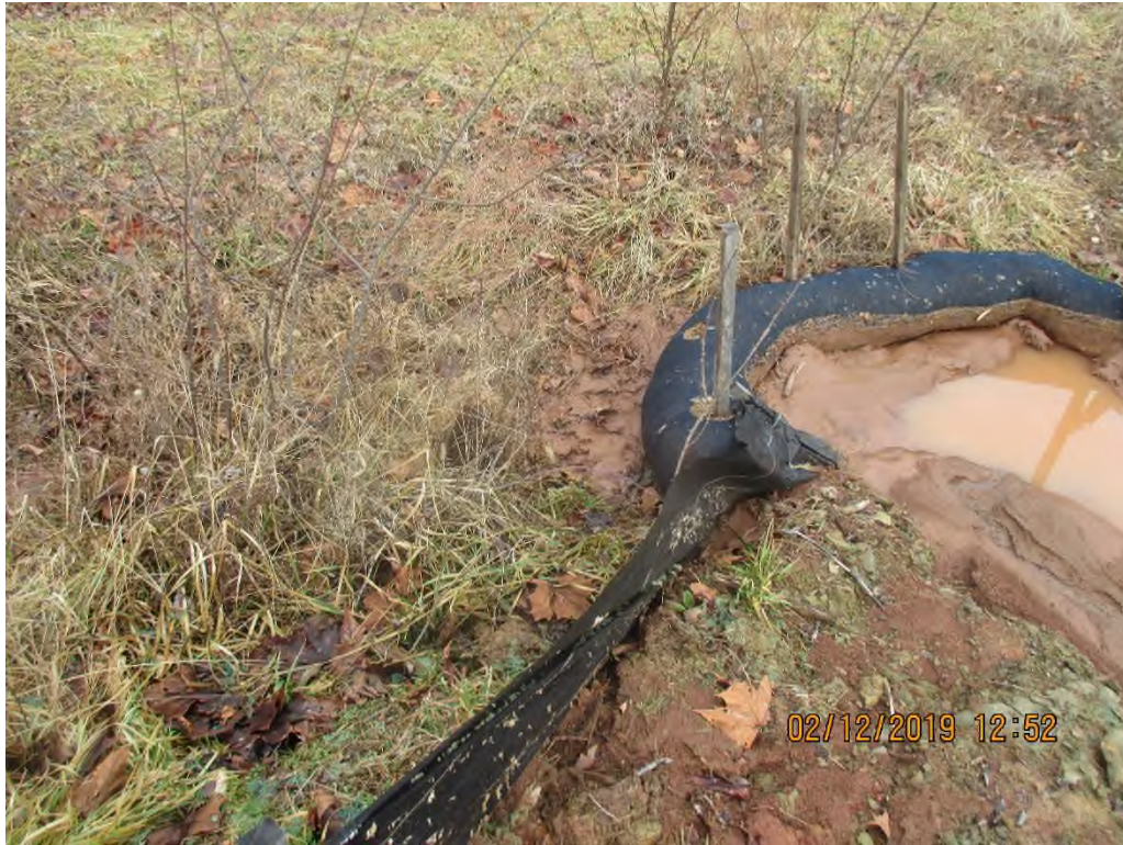
Perimeter control near station 5388+00
