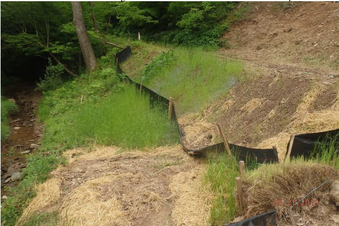
Unmaintained BMP in the UNT S. Fork of Hughes River watershed.
