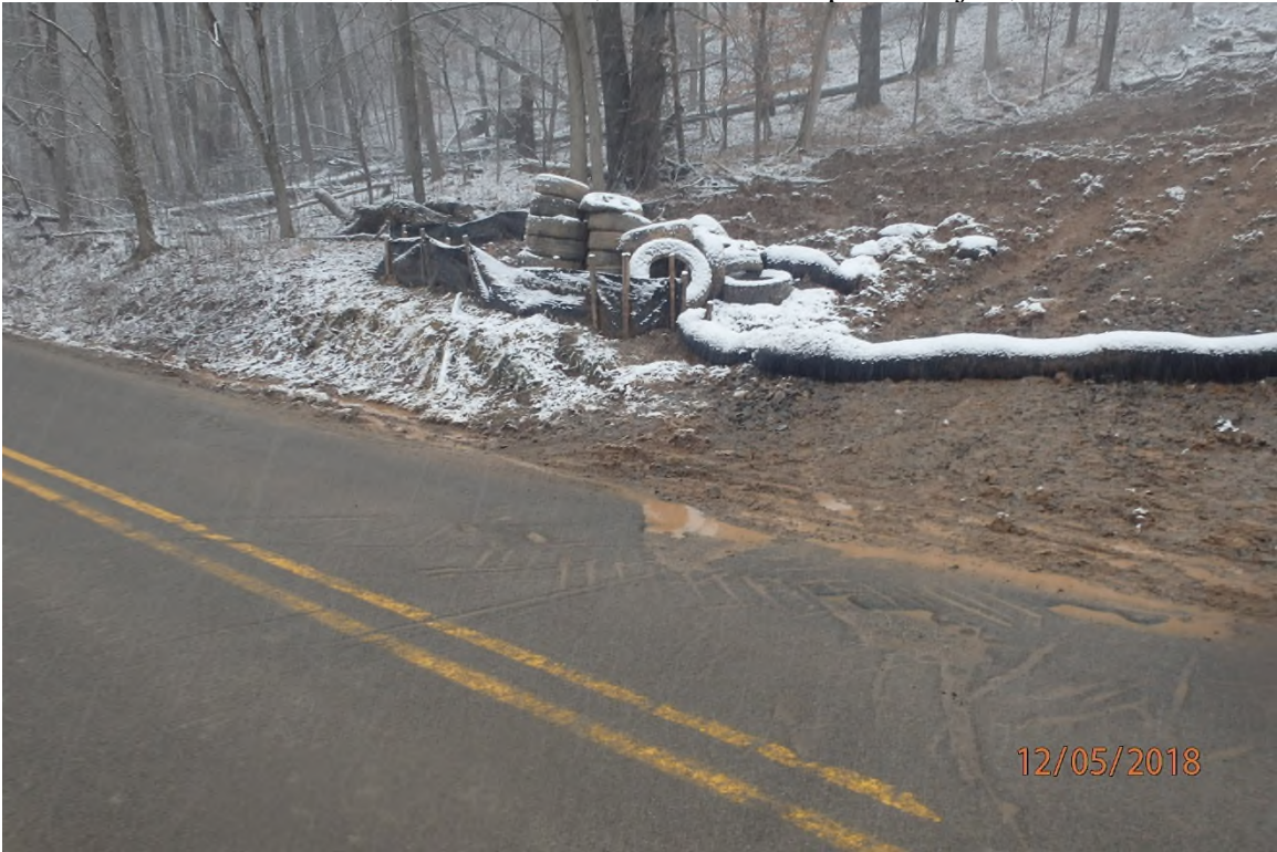
ARDO002.9 showing improperly installed perimeter control that allows sediment laden water to bypass under the device.
