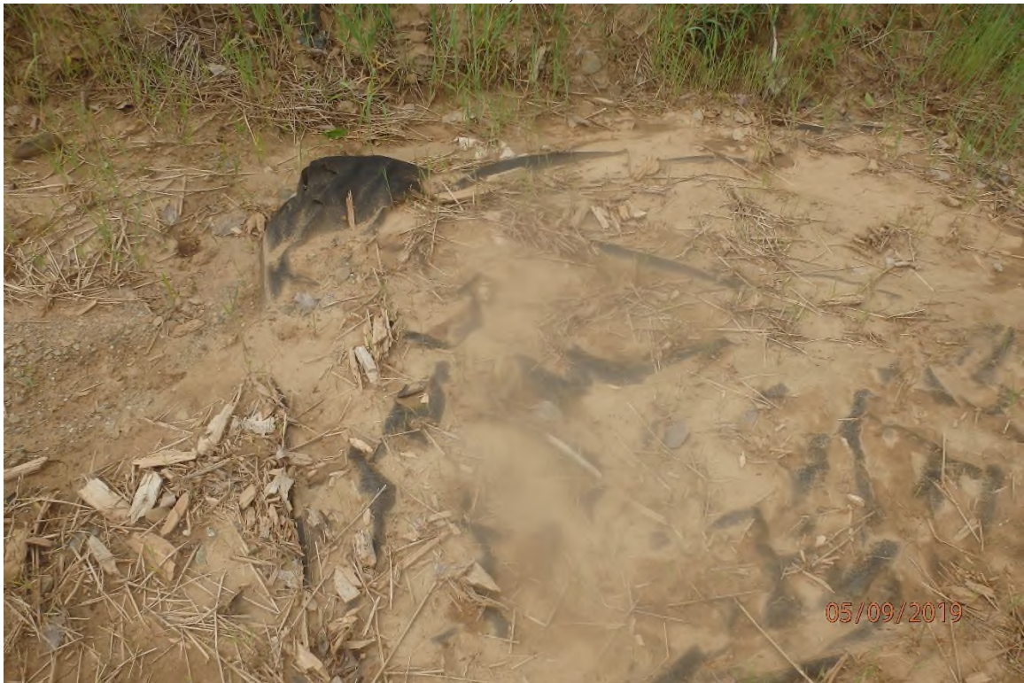
Discarded dewatering bag on the project.
