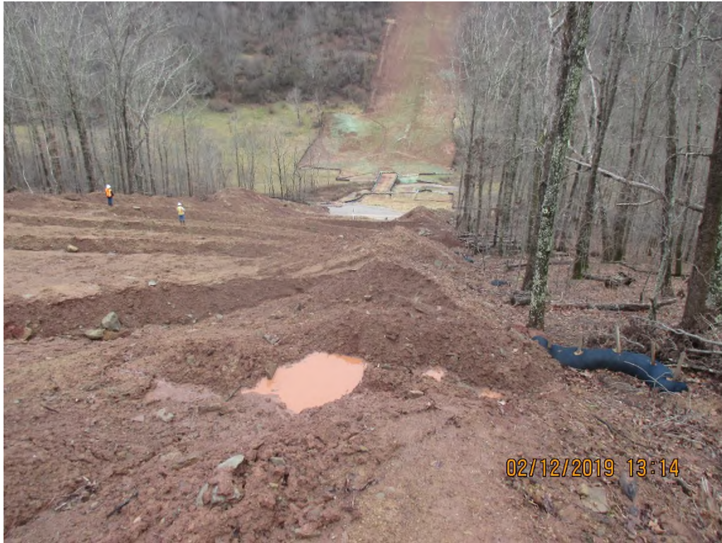
Waterbar outlets near station #5398+00 facing South
