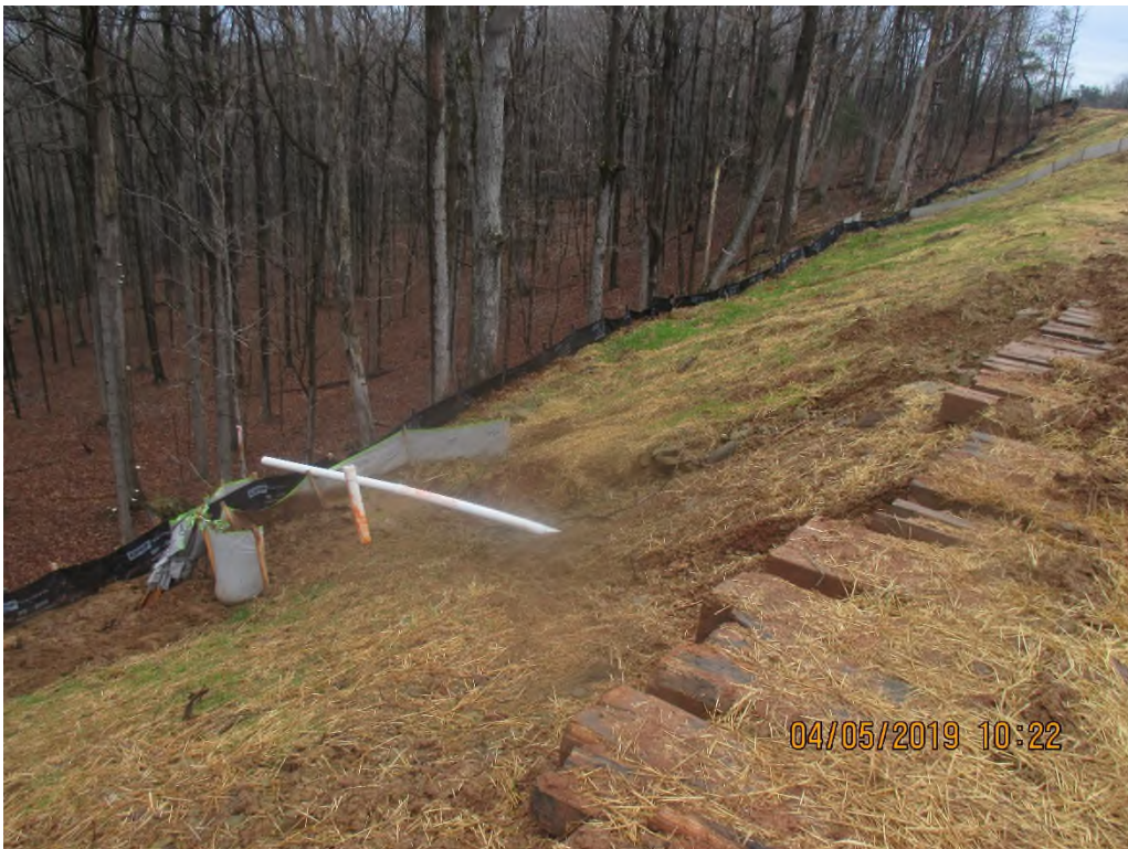
Pipe slope drain outlet near station #6781+55.
