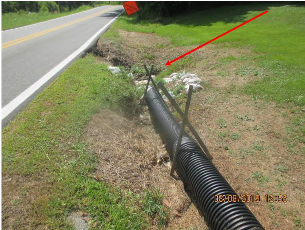
Slope drain outlet above culvert that conveys under Charles Creek Road.
