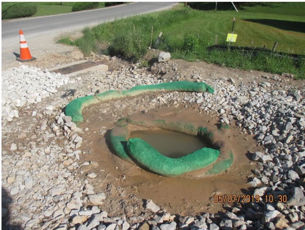
Drop inlet outlet and roadside drain outlets facing toward Route 21 and roadside ditch.
