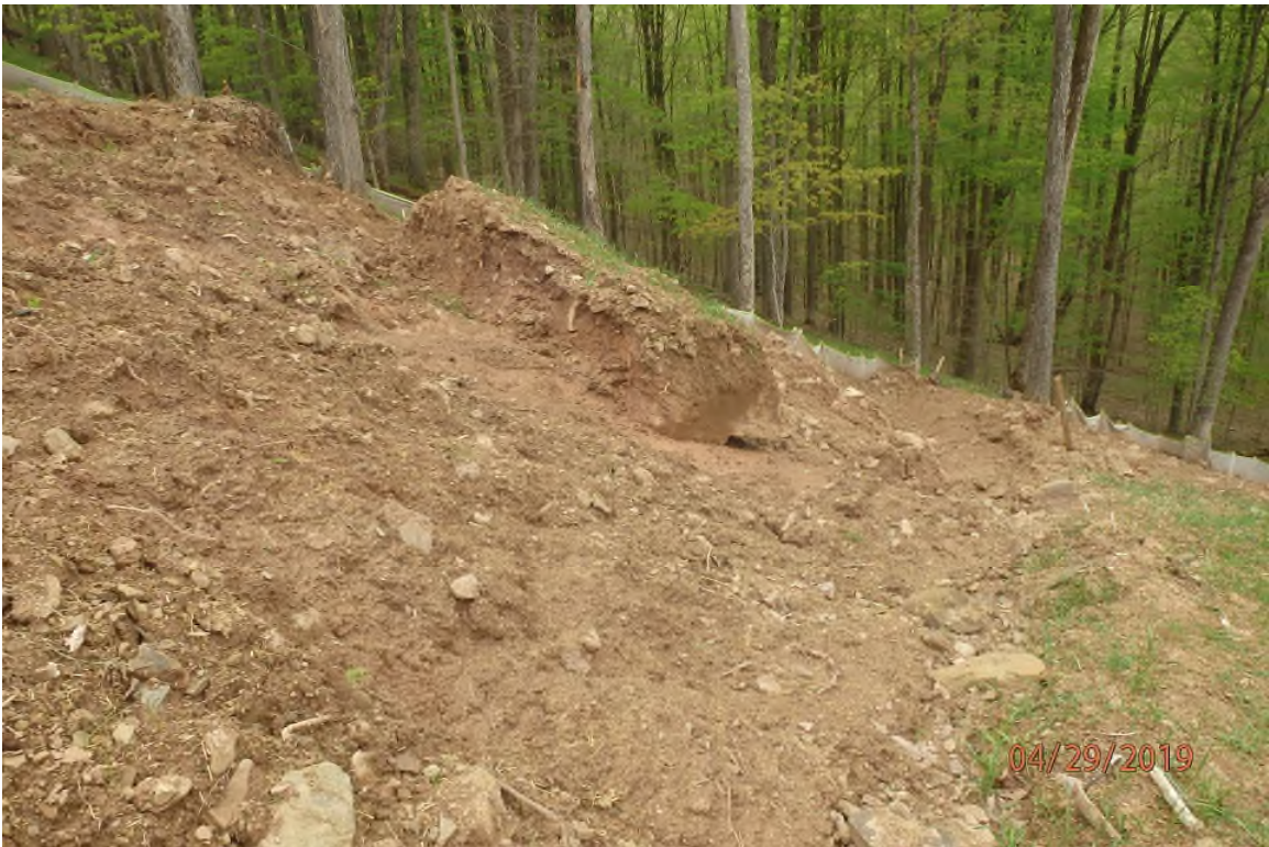
Overview of slip adjacent to 2227+50.
