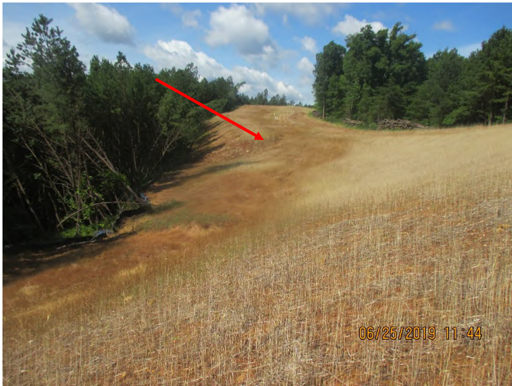
Past slip area with sediment deposited against super silt fence near station No. 5355+67. Arrow depicts where erosion was occurring on slope.
