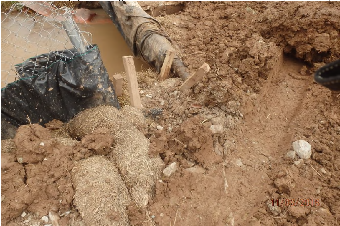
Unmaintained equipment bridge BMP in the Bluestone Creek watershed (SDOG0055).
