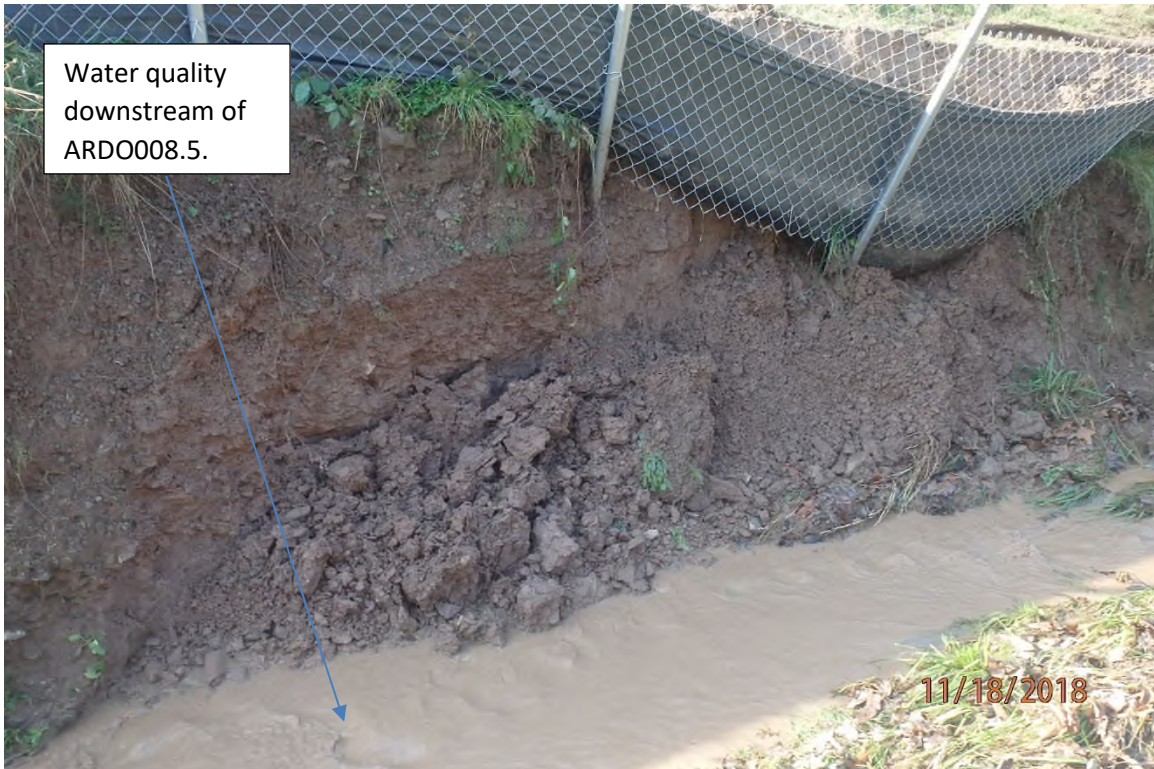
Third installed BMP failed and caused CNA deposits in UNT Georgescamp Run (39°15.182' X 80° 44.033').
