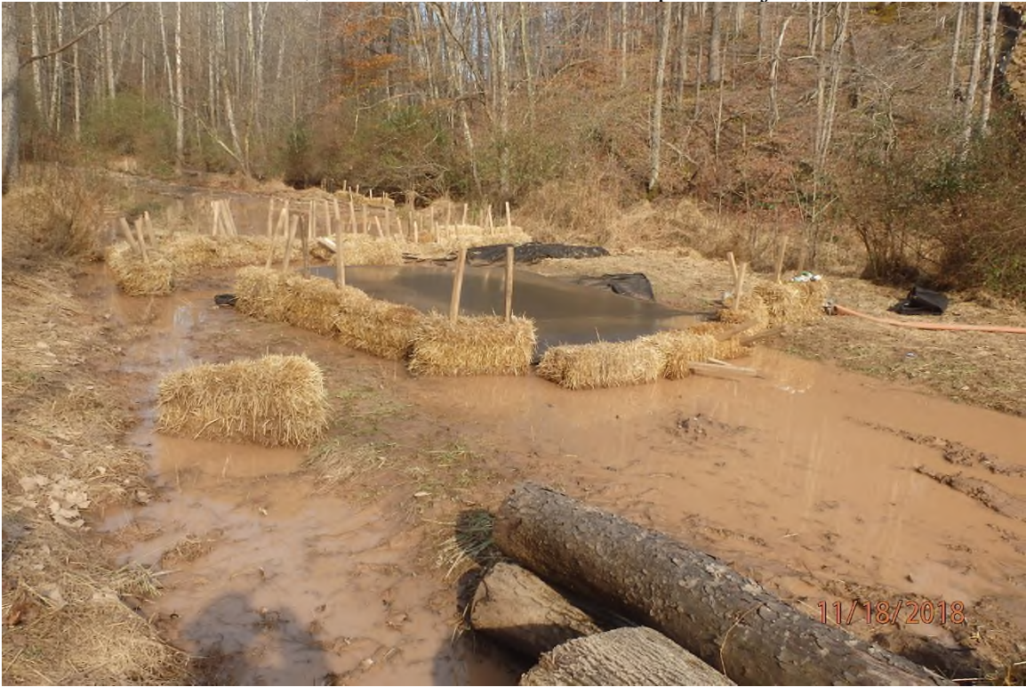
Dewatering bag associated with pipe trench dewatering adjacent to the SDOG536 stream crossing.
