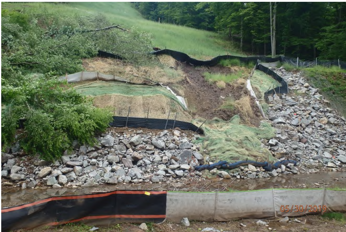
Overview of the slip associated with spill report #-09-90266 (A) showing the need for maintenance to the installed BMPs.
