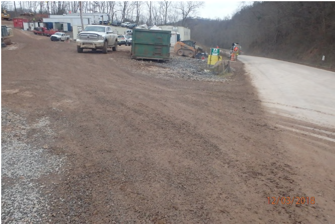
The construction access road to WV 18 showing the lack of a stable construction entrance and the associated track-out onto the public roadway.
