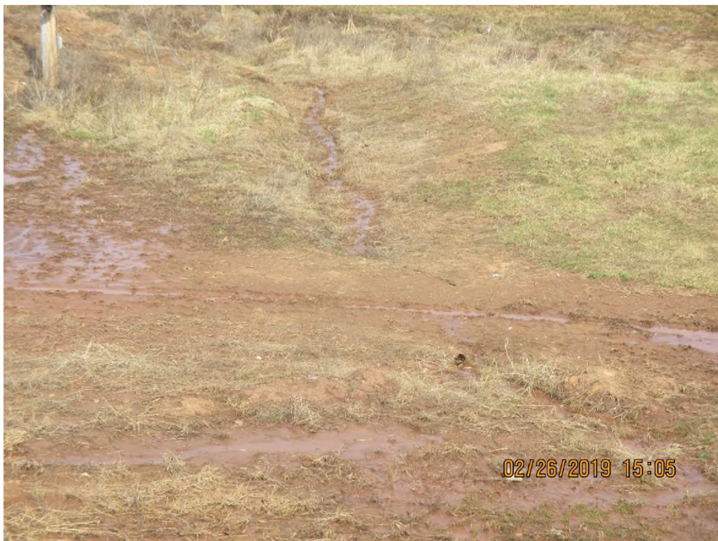
Downslope of station #6702+30. Culvert installed under additional workspace. No controls installed in this area.
