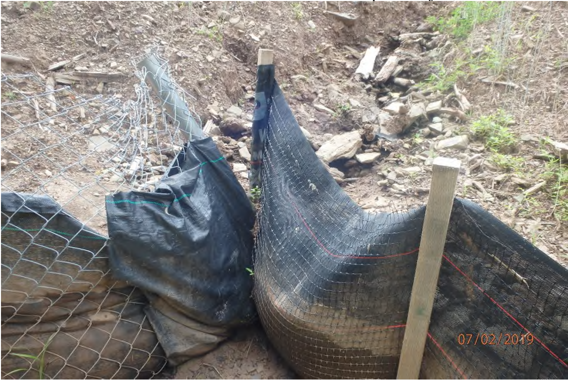
Improperly installed perimeter controls adjacent to 3214+00 that are inundated with sediment and in need of maintenance as a result of the previously pictured deficiency.
