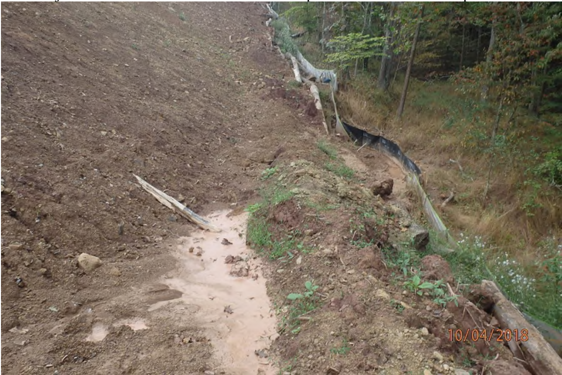
BMP adjacent to SDOI 008. Offsite sediment deposits and CNA downslope of the BMP.
