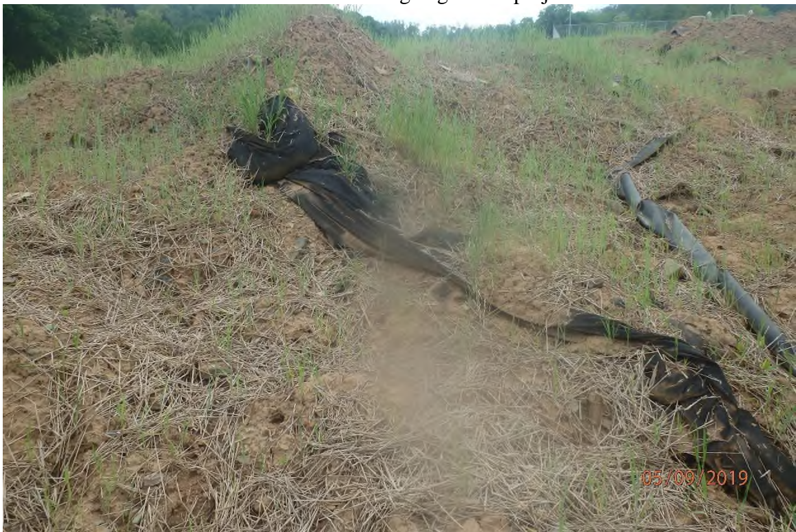
Solid waste in the soil stockpile.
