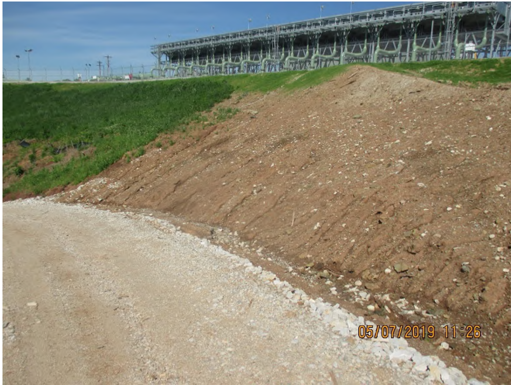
Erosion rills occurring on unprotected south slope above ditch that conveys under access road and toward perimeter of project.
