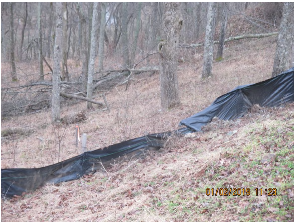
Silt fence along south slope parameter needing maintenance.
