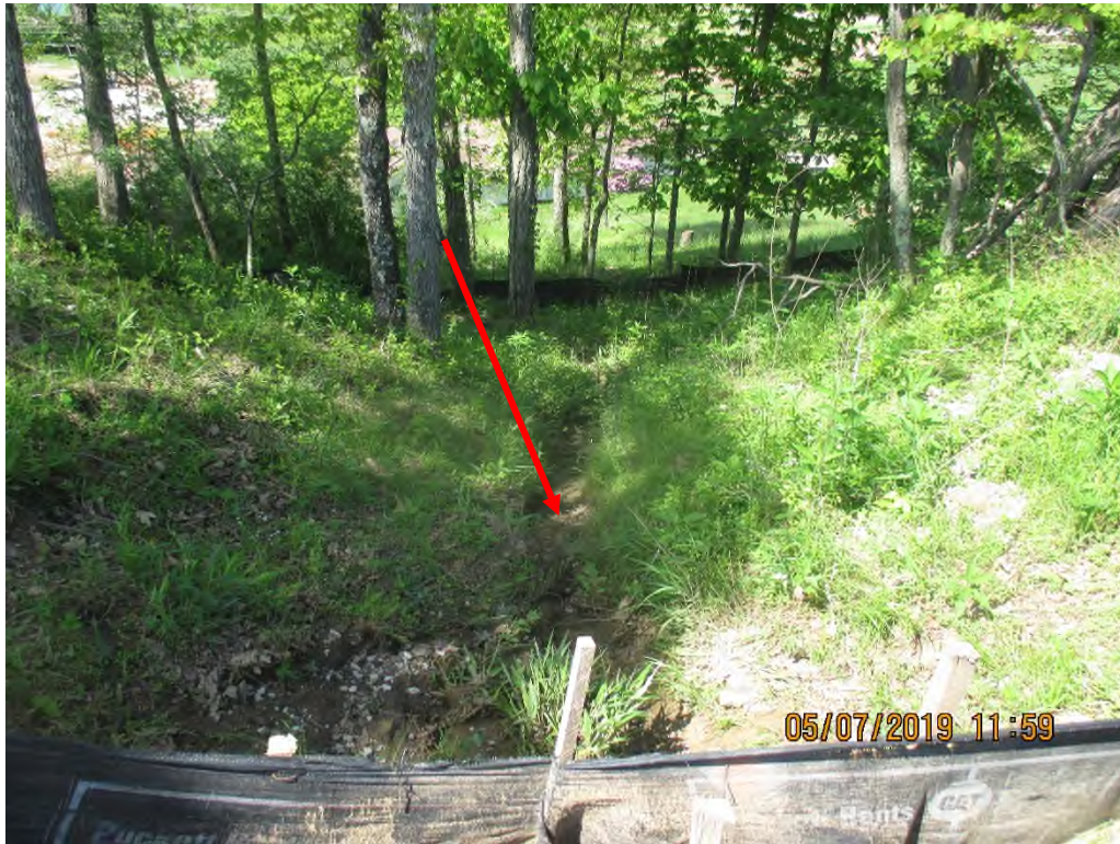
Below perimeter controls and silt fence that is not trenched-in on West Slope. Erosion gully forming downslope of controls.
