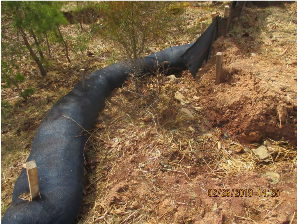
Waterbar terminus at station #6730+05. Erosion occurring above terminus.
