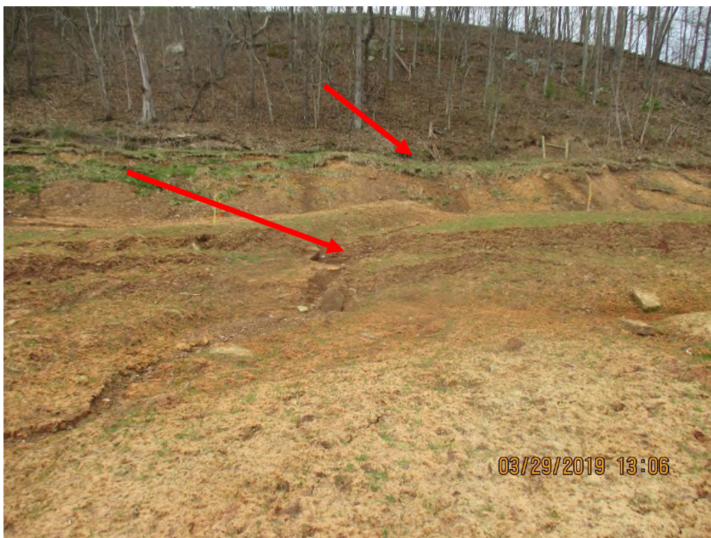
Standing in front of downslope controls facing slips. Arrow depicts slips occurring above and below where the pipeline is located.
