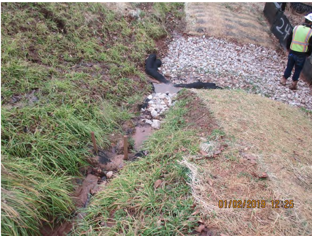
Diversion ditch flowing into discharge point at silt fence 24.
