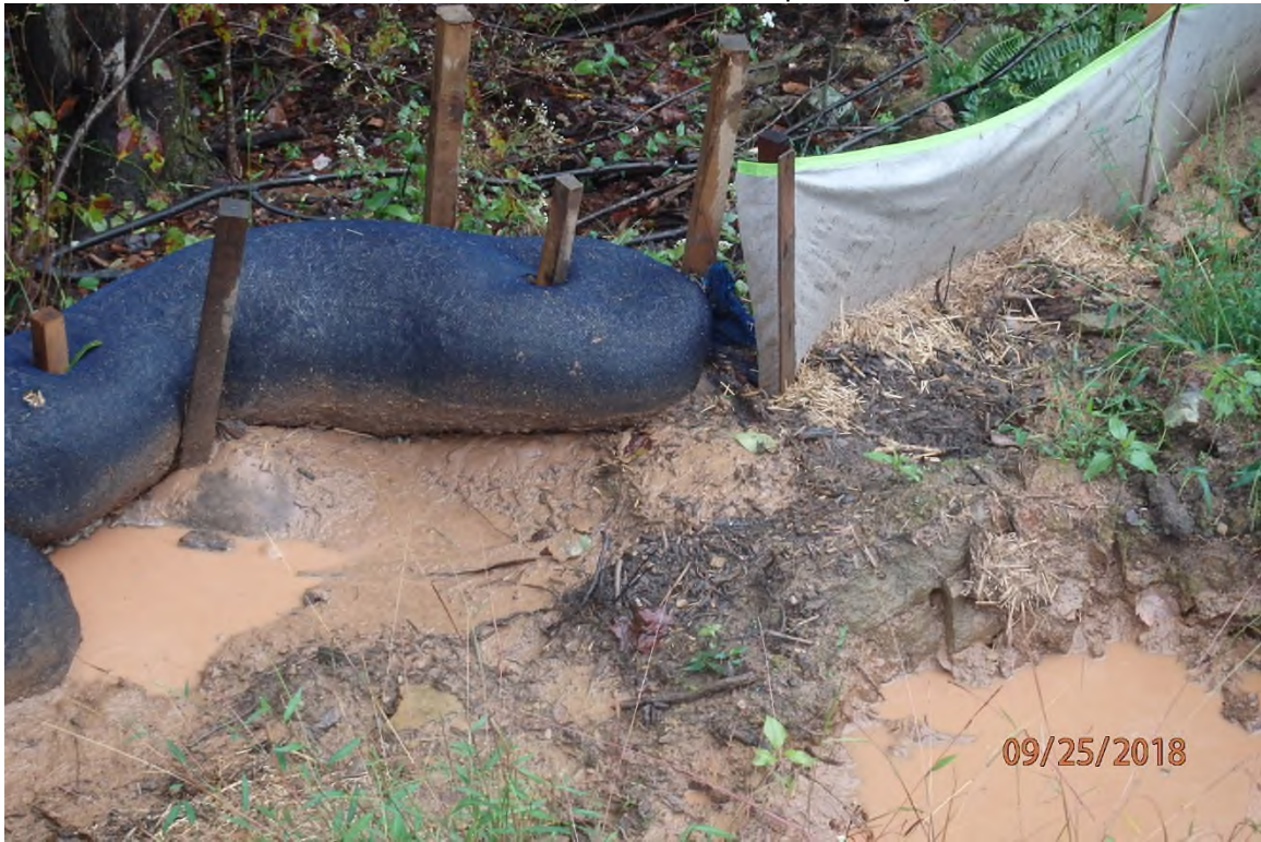
Improperly operated water bar terminus BMP adjacent to 2255+00.
