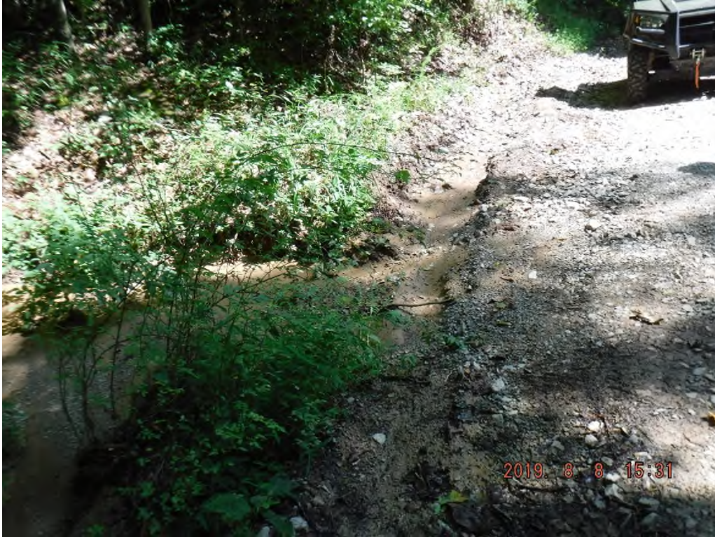
East ditchline at ROW filled with sediment from runoff.
