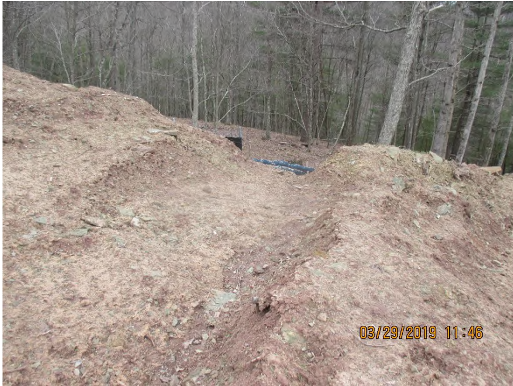
Waterbar terminus above stream SWIF-057 near station #5163+50
