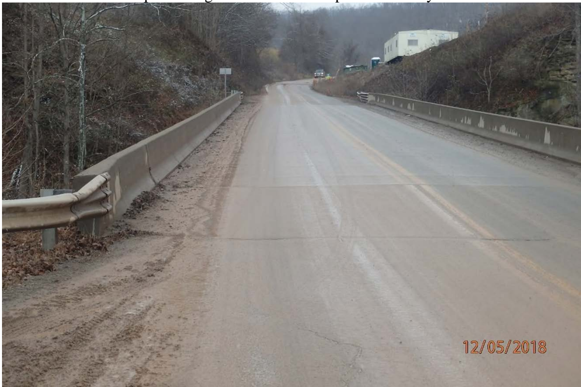
WV 18 showing track-out and slick film of mud on the public roadway that originates from project.
