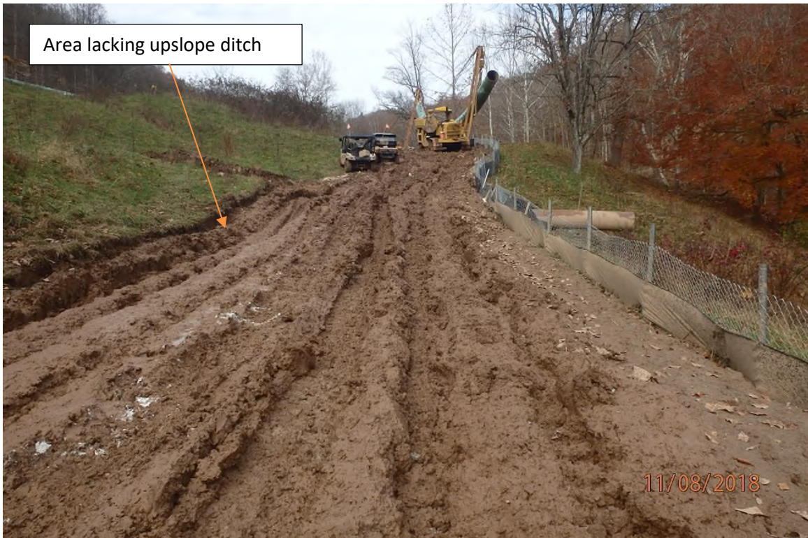
ARDO08.5 showing a lack of upslope ditches to collect run-on stormwater as indicated in the approved SWPPP.
