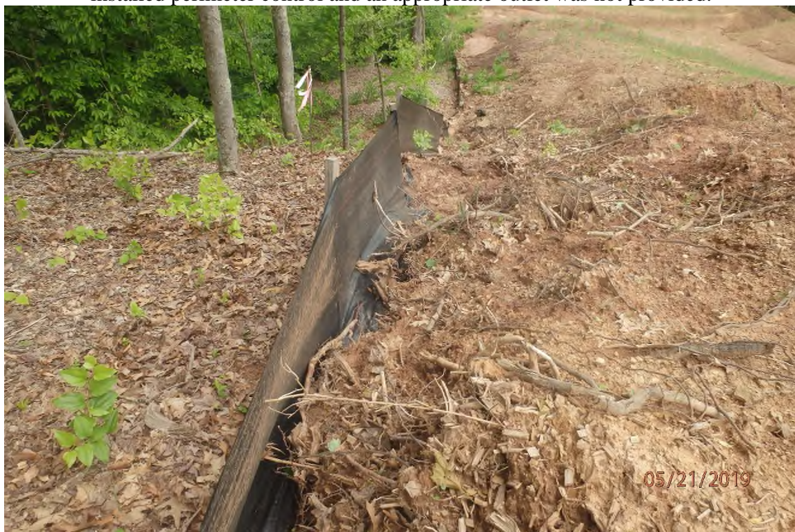
Concentrated flow area along the installed perimeter control downslope of the above pictured BMP.
