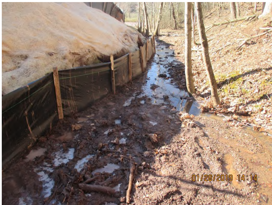
Area where slipped material was removed from Stream SJAG316.
