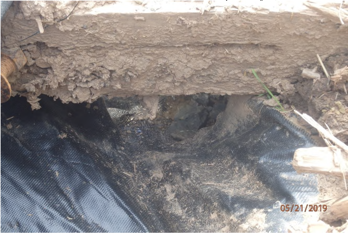
Unmaintained timber mat equipment BMP at the Taylor Drain crossing (SDON837).
