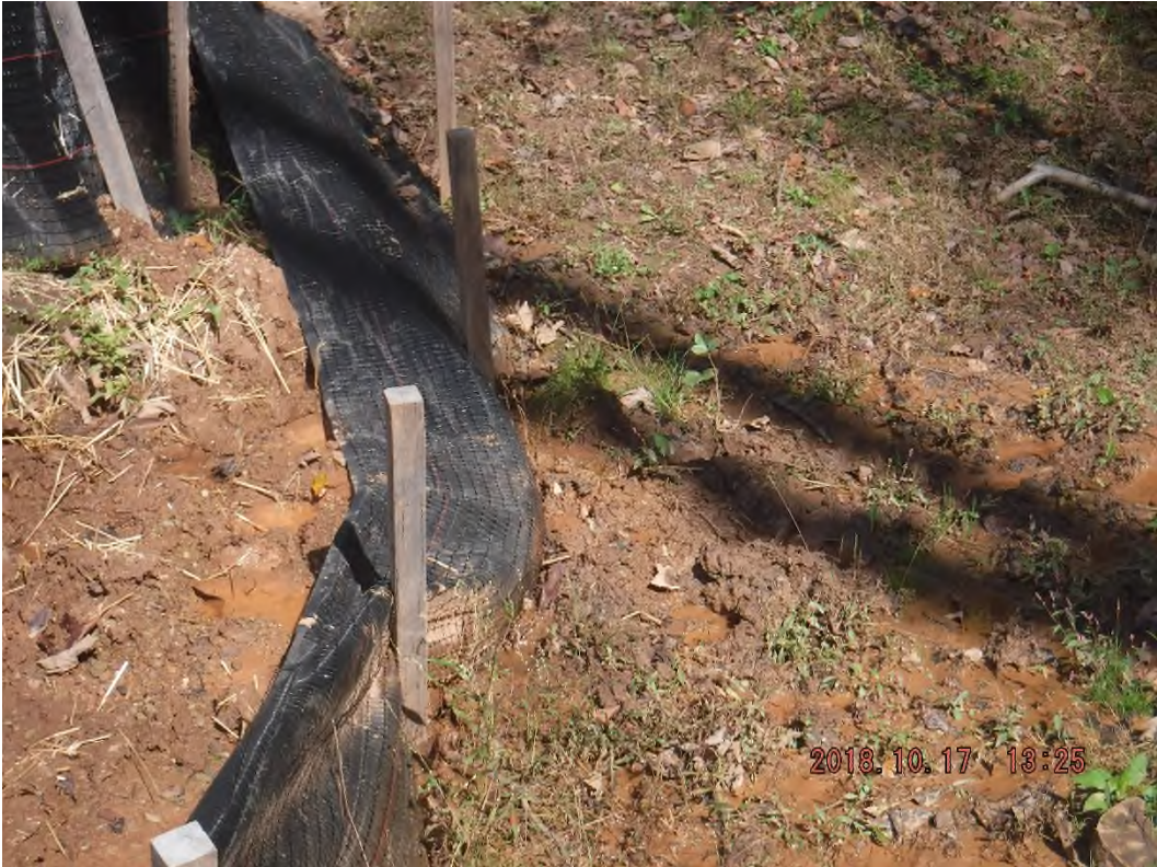
Silt fence in disrepair directly above crossing at Station 6705+00.
