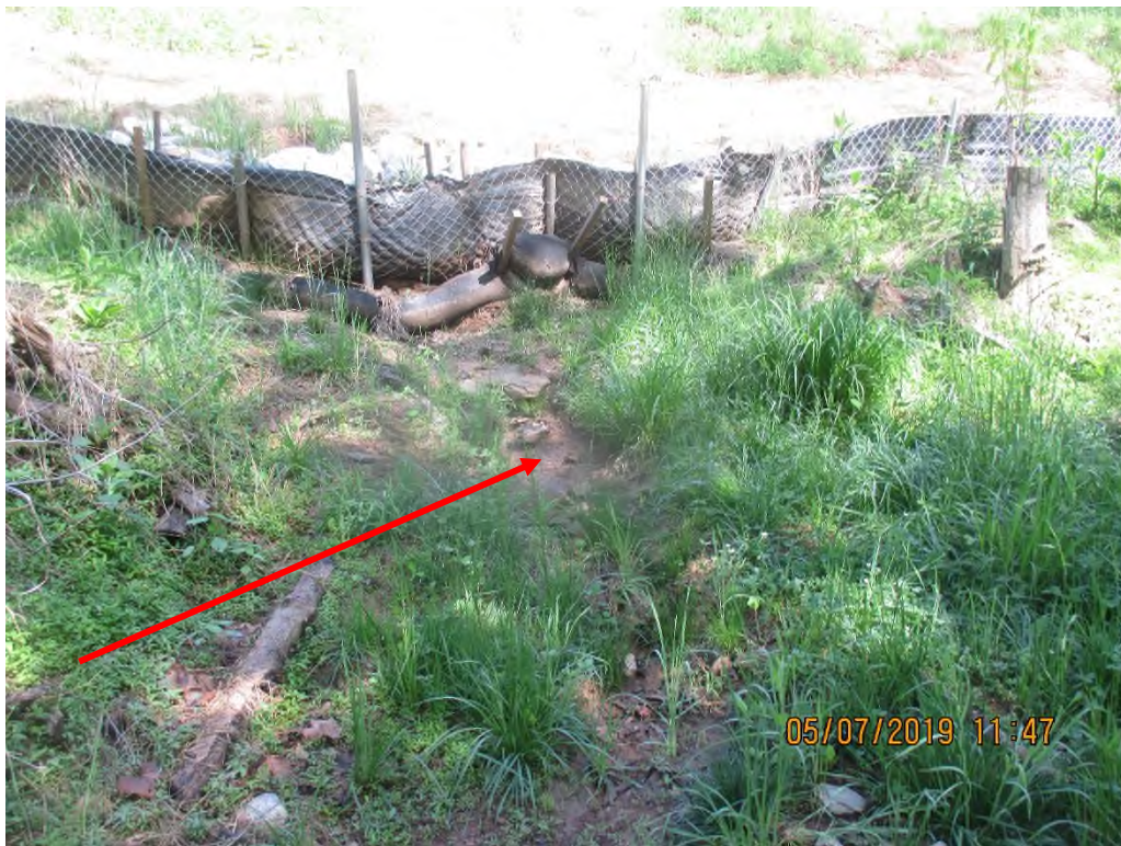
Downslope of perimeter controls on south west slope of project LOD. Arrow depicts evidence that sediment laden water had flowed past controls.
