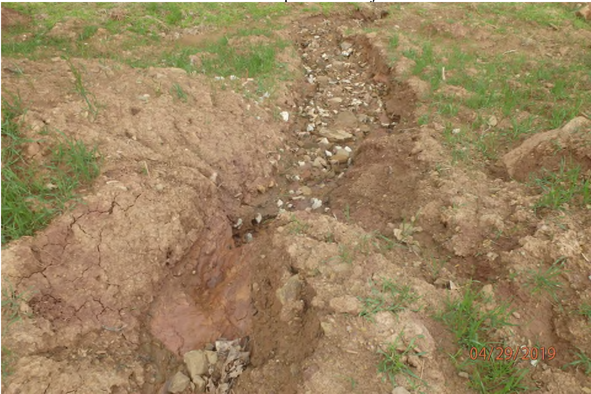
Water bar outlet with fill slope erosion adjacent to 2265+00.
