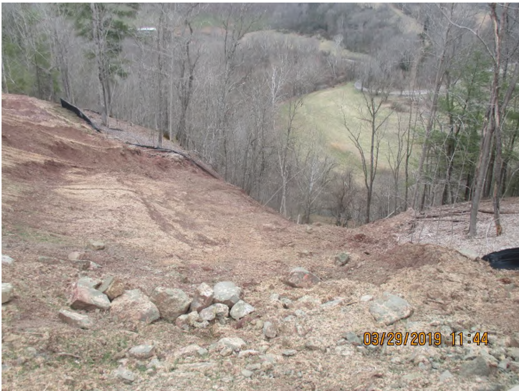
Slip on slope above stream SWIF-057 near station #5163+50
