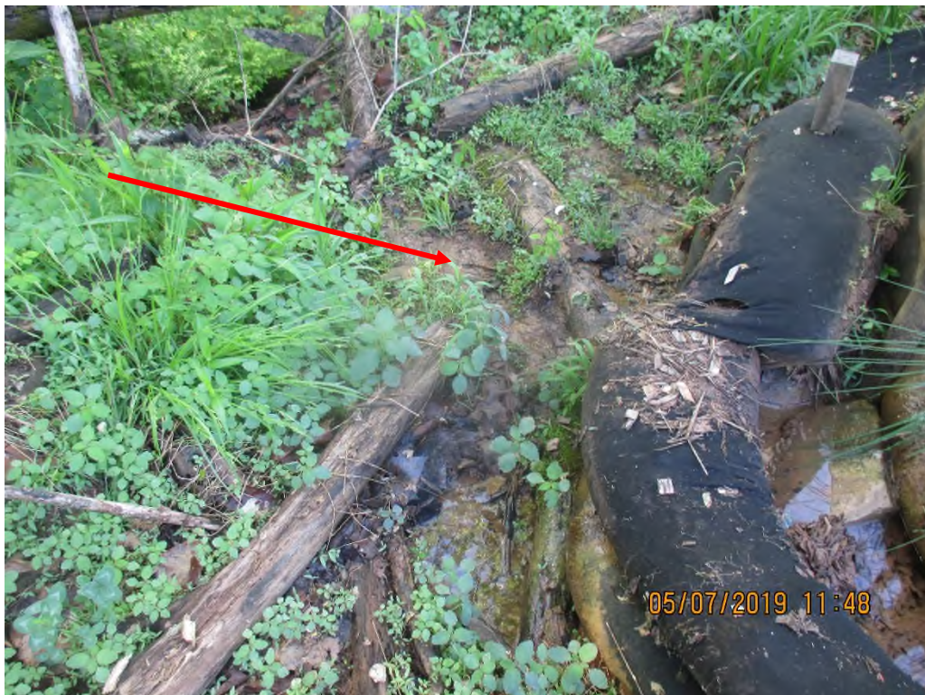
Perimeter controls on south west slope of project LOD. Arrow depicts evidence that sediment laden water had flowed past controls.
