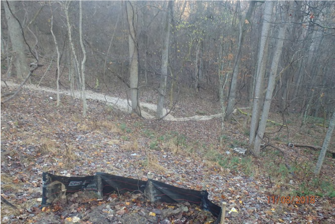
Slip and associated mud flow adjacent to 2822+00.
