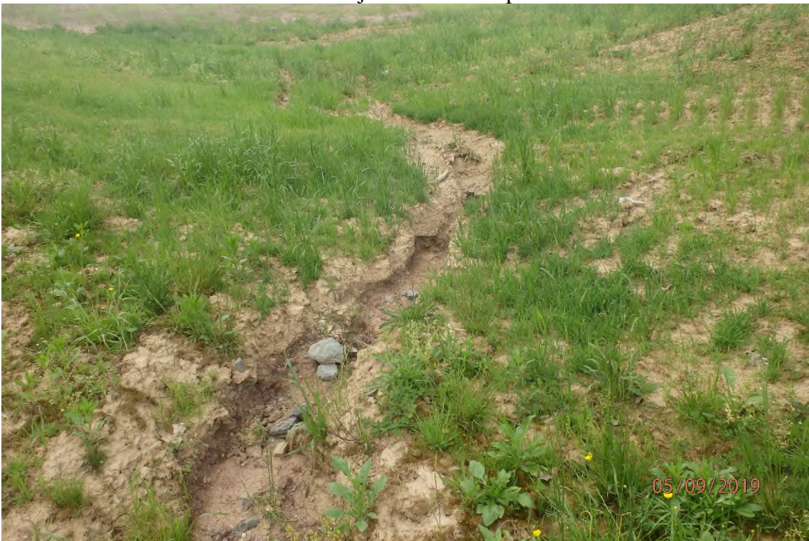
Concentrated flow stormwater being directed over an unprotected fill slope and associated fill slope erosion adjacent to the fill pad.
