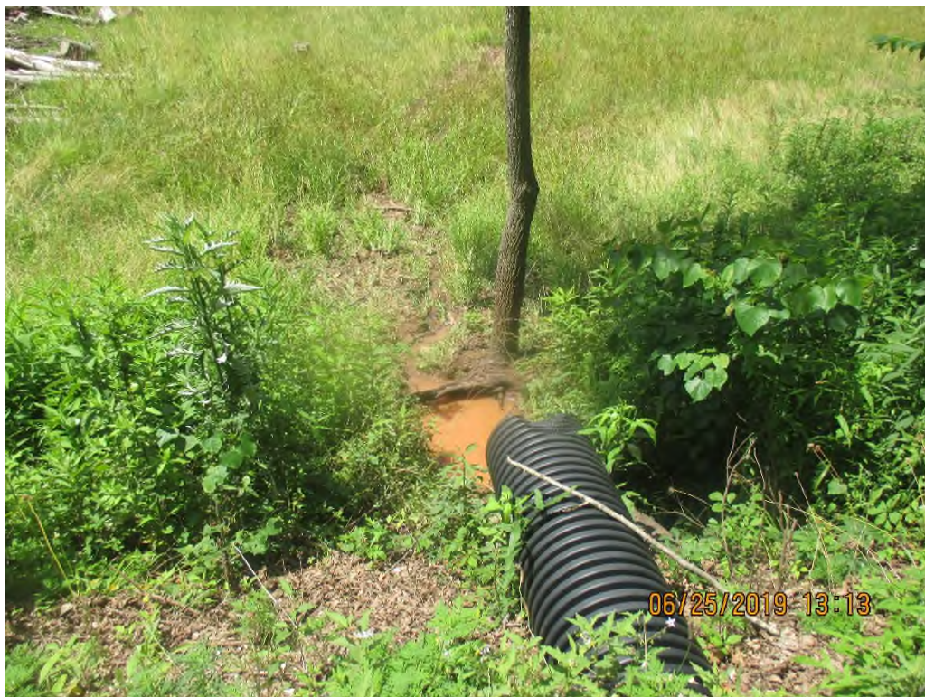
Culvert outlet downslope of MXP RPW along Munchausen Road.
