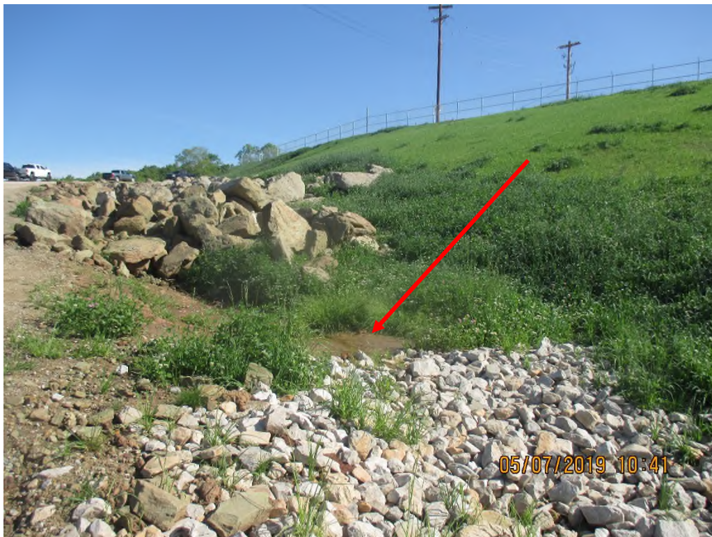
Rock placed in depression at base of West slope. Sediment present above smaller rock lined diversion.
