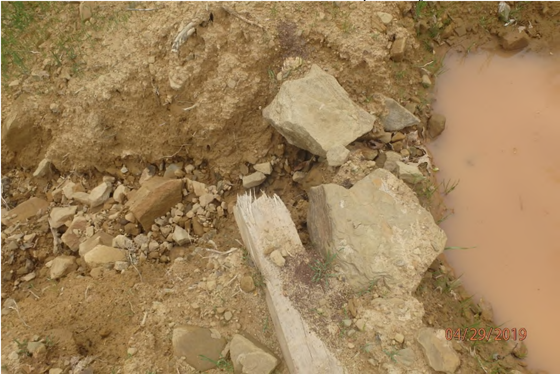
Water bar outlet with fill slope erosion adjacent to 2268+00.
