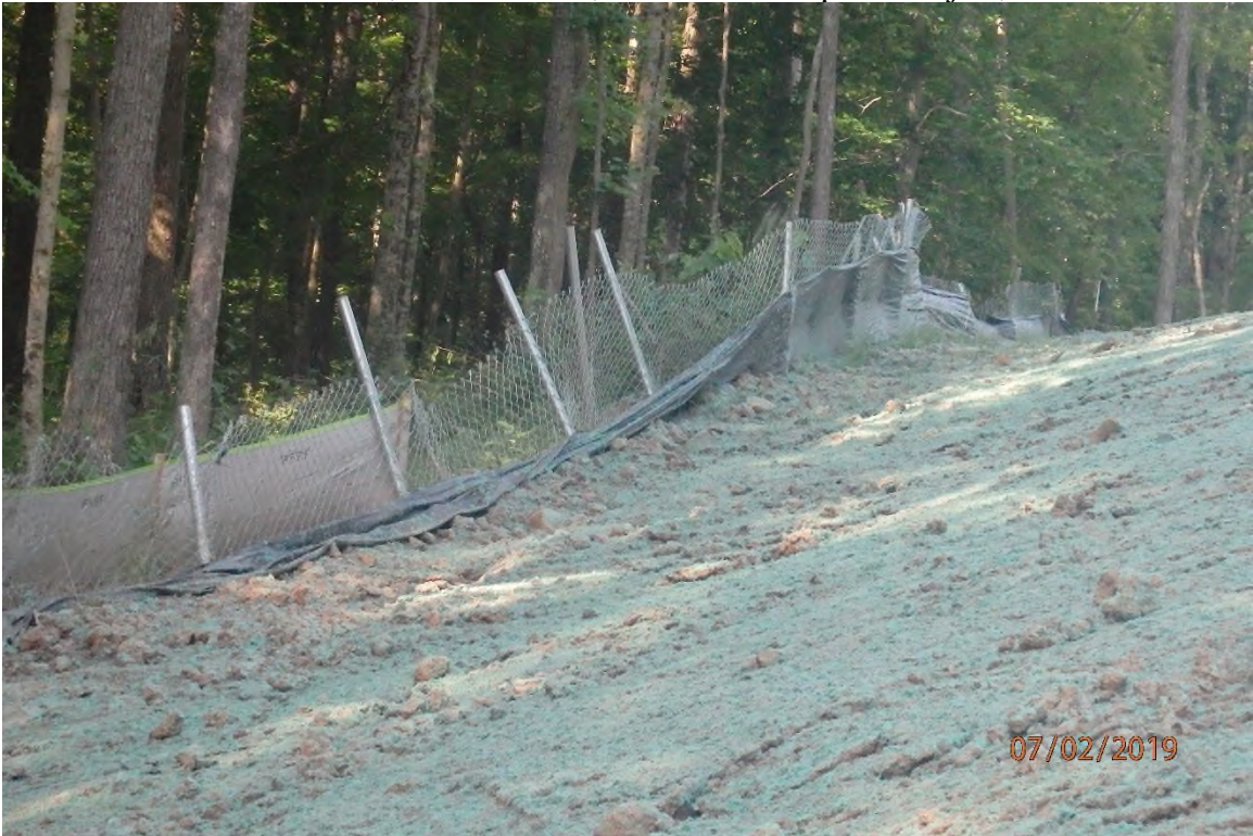
Perimeter control in need of maintenance in the Sugar Run watershed.
