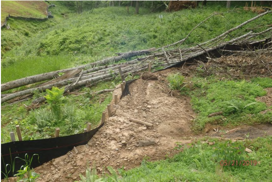
Perimeter control adjacent to UNT Sugar Run that is inundated with sediment as a result of the previously pictured water bar failures upslope.
