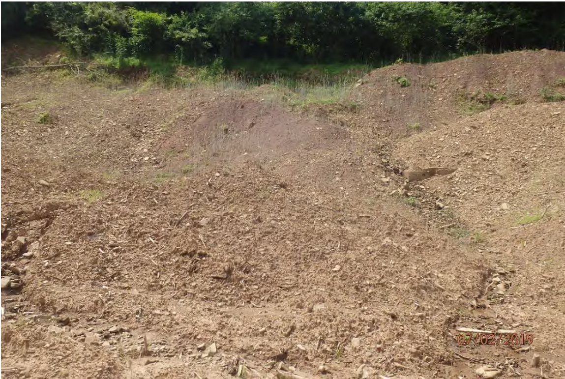
Project area adjacent to 3214+00 showing erosion gullies associated with concentrated flow run on stormwater. The approved SWPPP does not address this situation and the plan has not been modified in this area.
