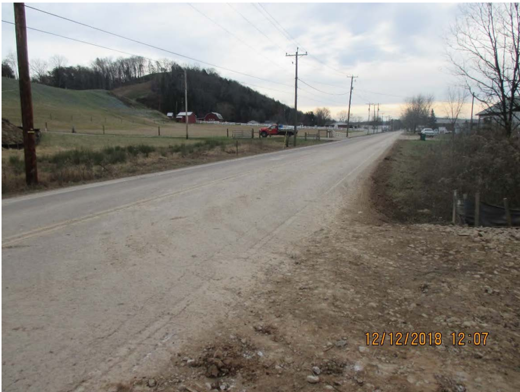
The MXP ROW crossing with Route 62, facing East toward contractor yard.
