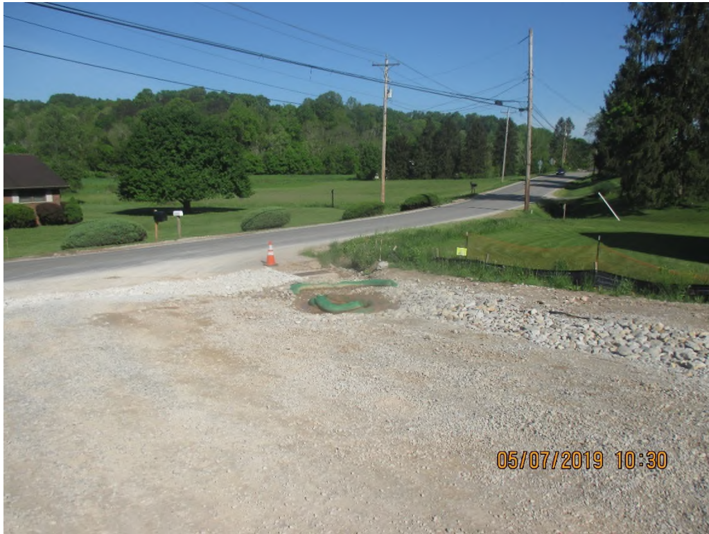
Facing downslope at construction entrance toward outlets for roadside drain and drop inlet. These outlets convey into UNT of Grasslick Run.
