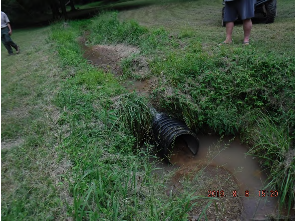
Culvert on west side showing sediment deposits from ROW runoff.
