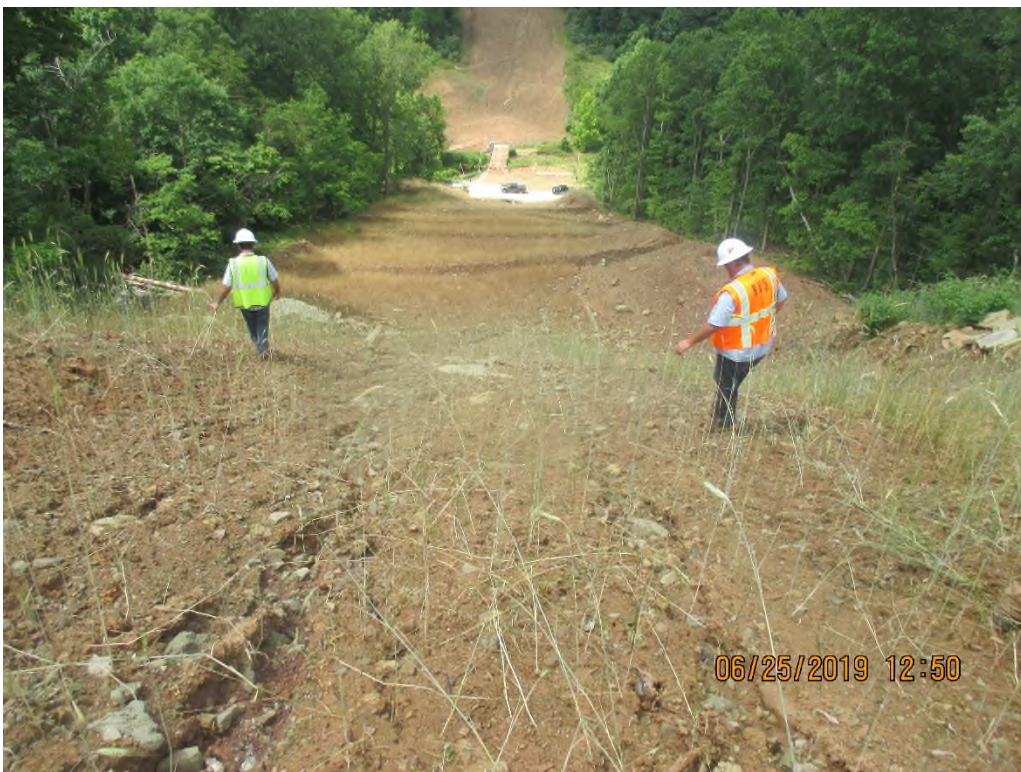
South of station No. 5396+00, downslope towards Munchausen Road Crossing.
