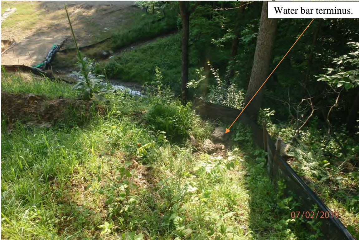
Sheet flow silt fence placed in a concentrated flow area at the terminus of a water bar in the Sugar Run watershed.
