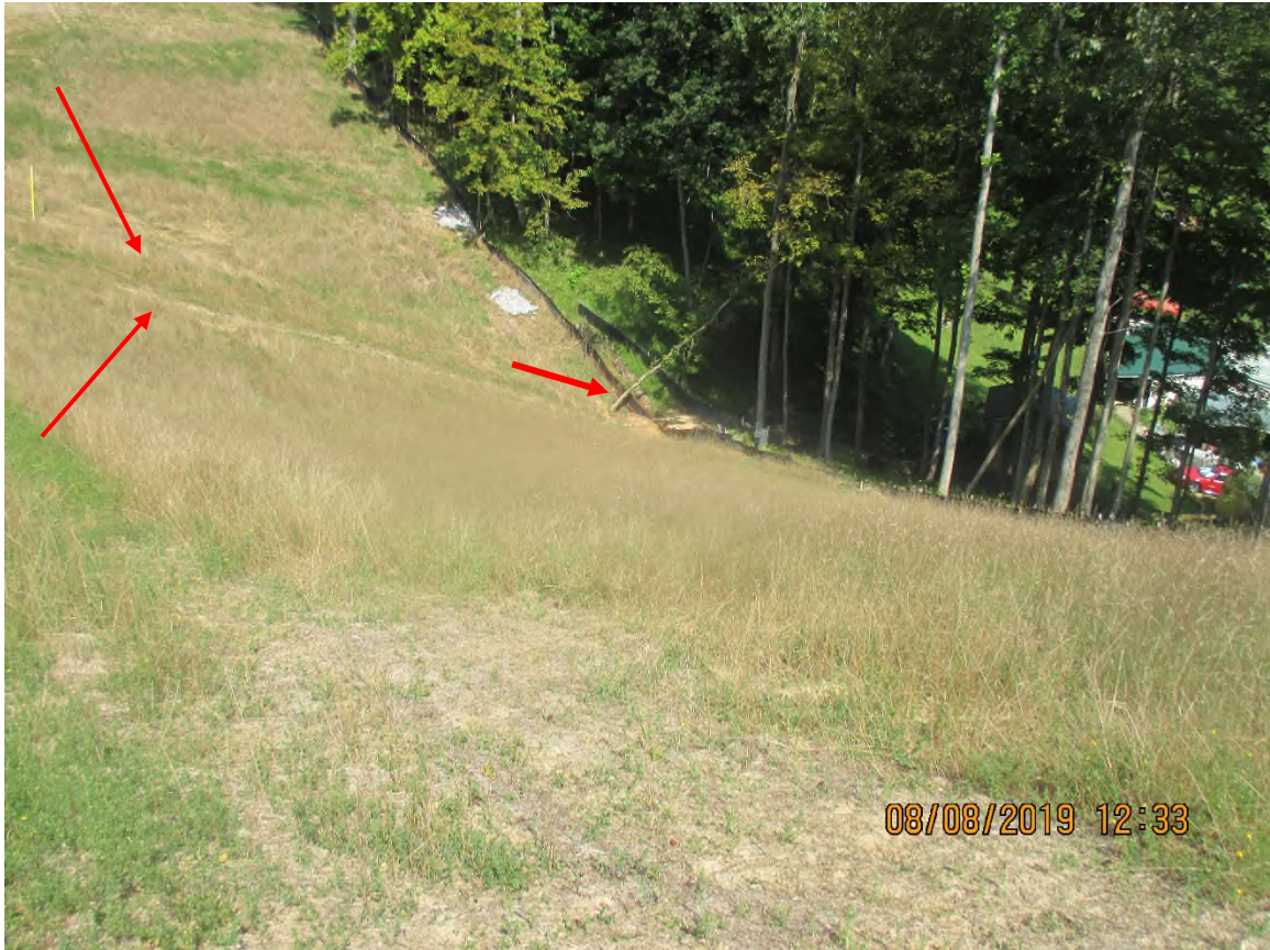
Drainage area between the two slopes facing North. Arrow depicts where erosion was occurring and overwhelming perimeter controls.
