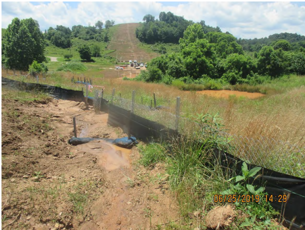
Facing South towards Stream SROC 029 at station No. 5638+46 below waterbar with erosion present on slope.
