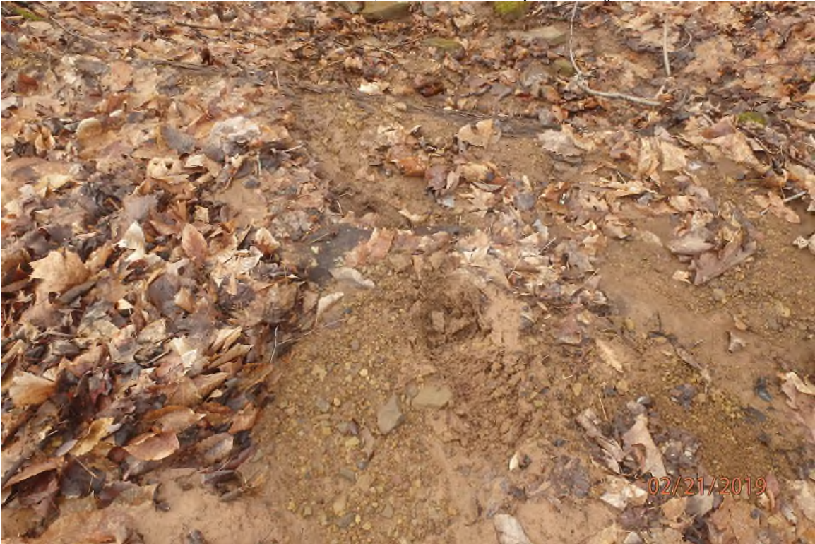
Offsite sediment trail leading to the receiving stream from the previously pictured improperly installed perimeter control.
