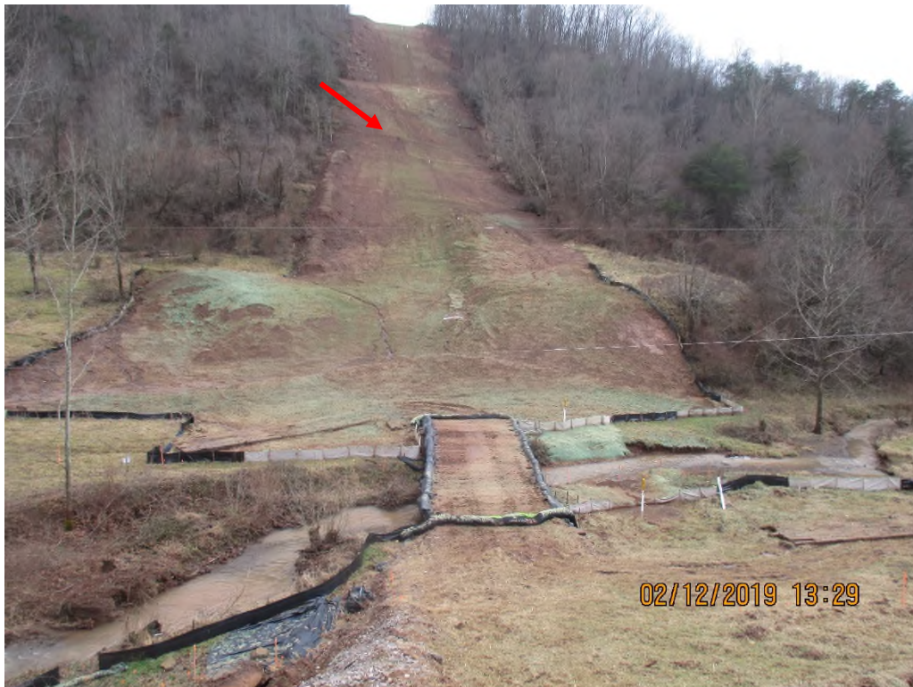
Munchausen Road crossing at station #5407+07 facing South at Stream SWIH-001. Arrow depicts waterbar being eroded due to concentrated runoff upslope
