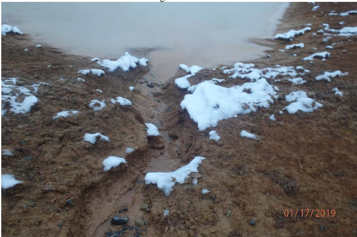
Basin 1 inlet showing the lack of a stabilized inlet.
