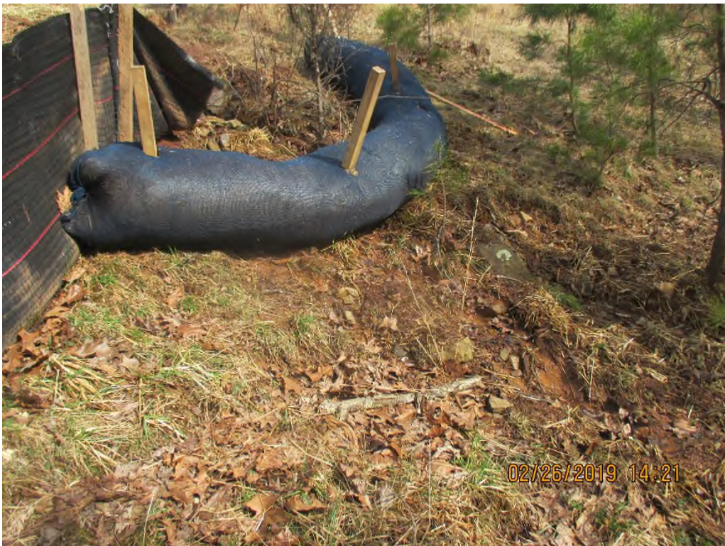
Waterbar terminus at station #6730+05. Compost filter sock undermined and evidence of sediment deposits past LOD.
