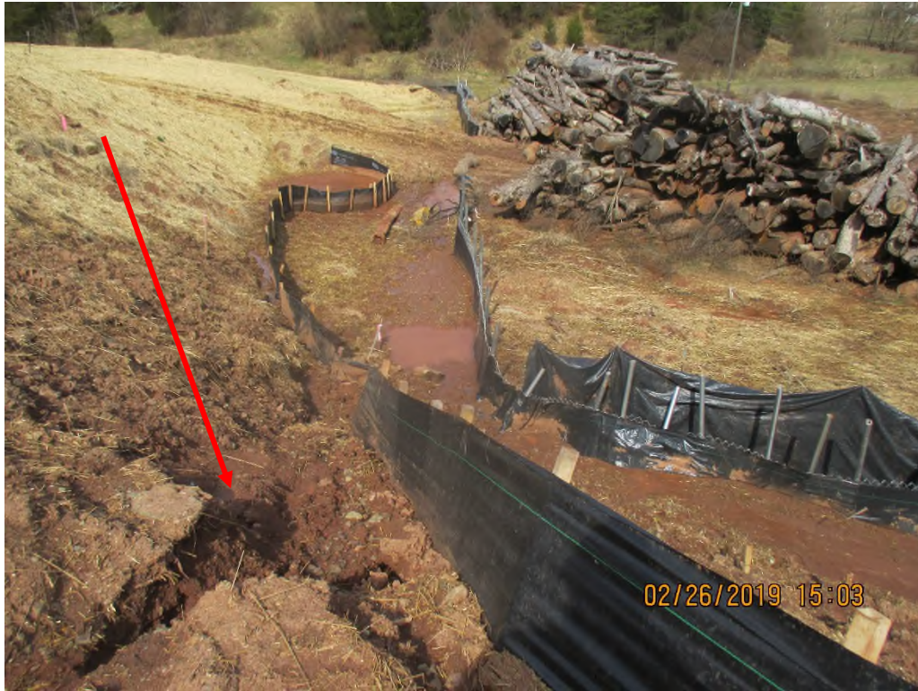
Slope near station #6720+60 facing downslope. Erosion occurring from run-on flowing across ROW.
