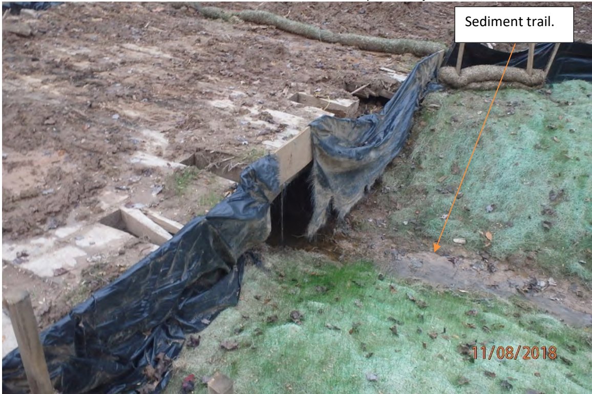
Equipment bridge BMP in need of maintenance at Taylor Drain (SDOG071) crossing.
