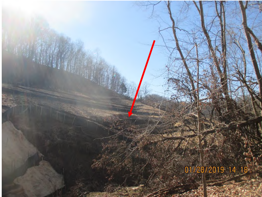
Area upslope of Stream SJAG316 where slips have reoccurred. This area has slipped approximately 2 vertical feet.
