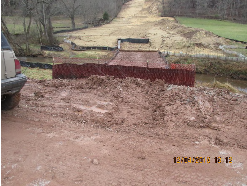
Facing South at MXP ROW entrance at Station Number 6880+41.
