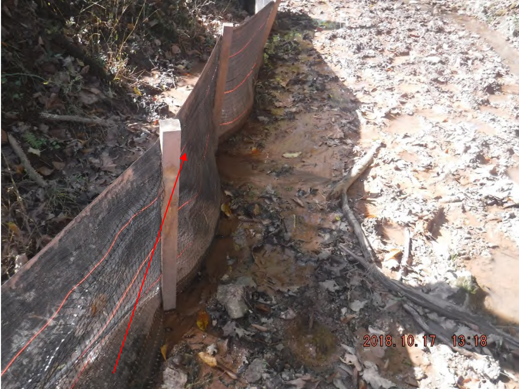
Sediment deposits in stream leading to the farm pond below.
