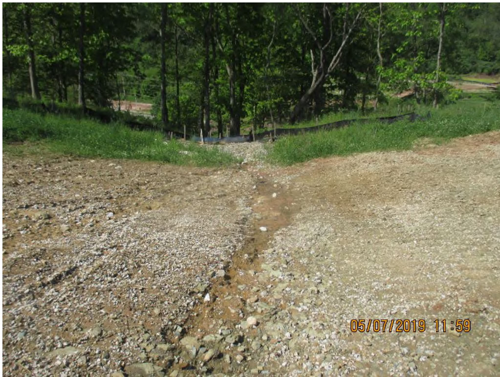
Erosion occurring on slope above perimeter controls on West slope.
