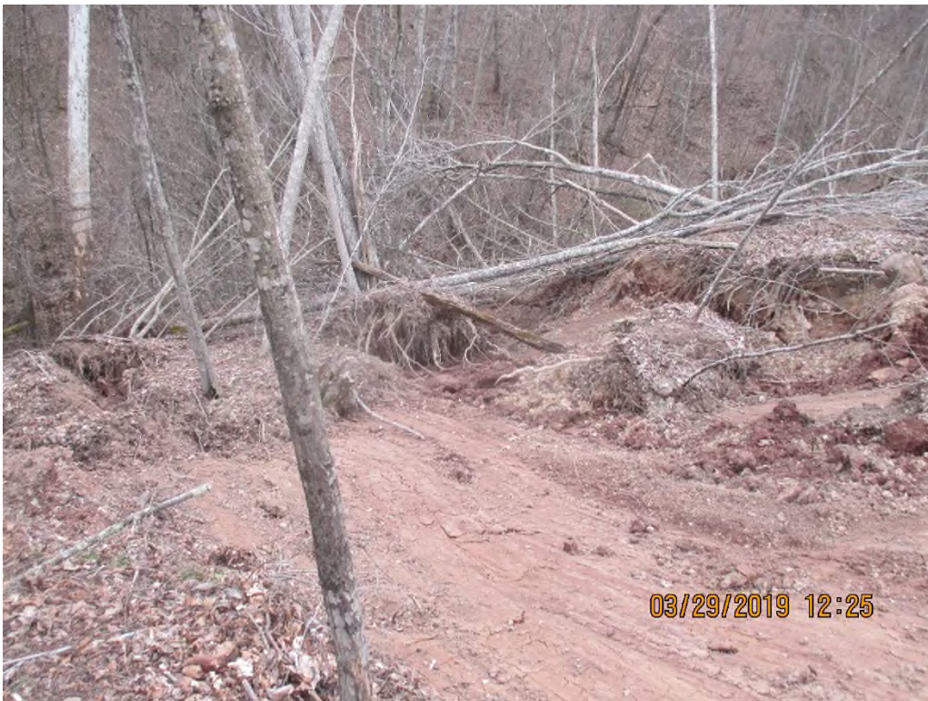
Station #5163+50 facing downslope toward material that slipped into Stream SWIF-057
