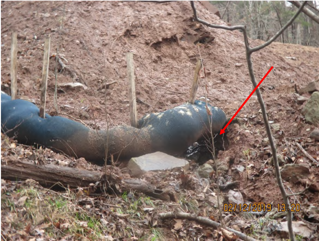
Waterbar Outlet #2 near station #5398+00 facing upslope. Arrow shows undermined CFS.
