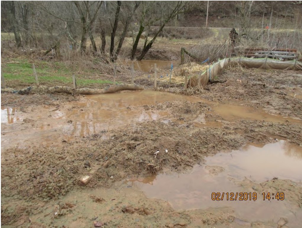
North Side stream SROC-030 facing South at controls
