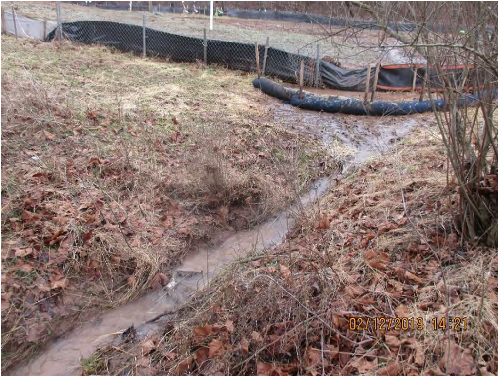
Near station 5453+84 facing upslope at controls
