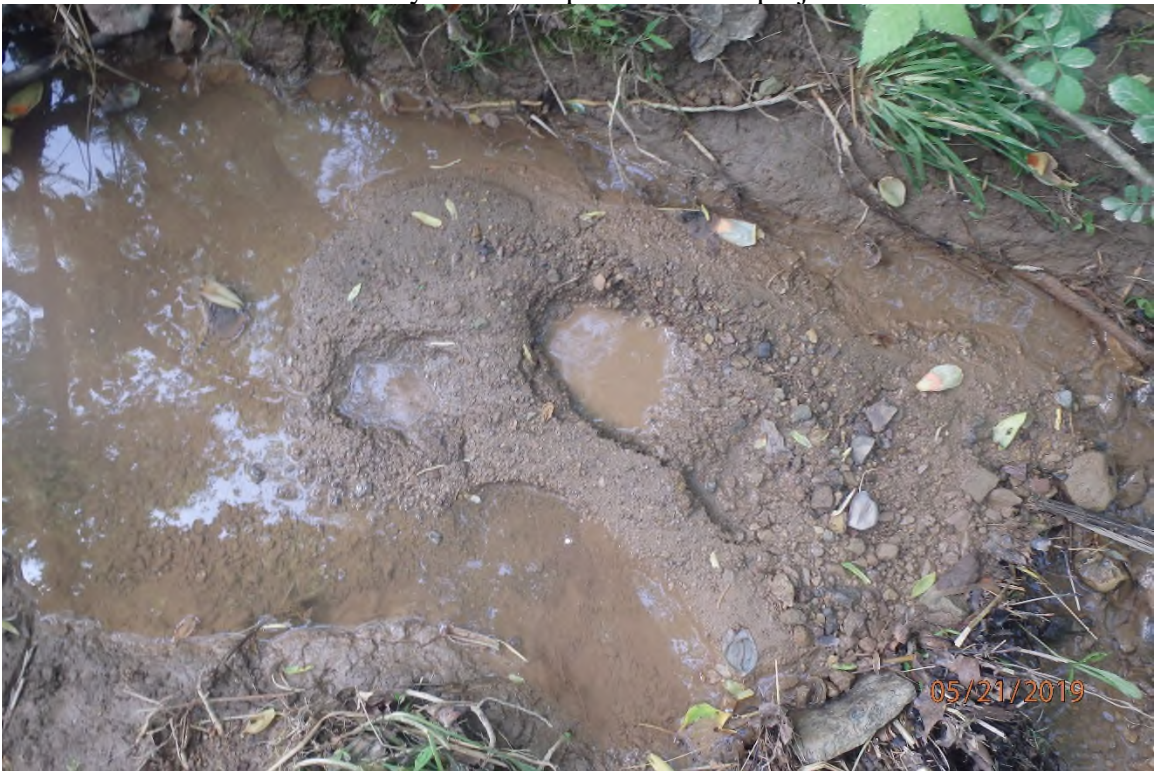
CNA deposits in in UNT Taylor Drain (39° 11.391' X 80° 50.386') as a result of the previously pictured deficiencies from a failure to install water bars.
