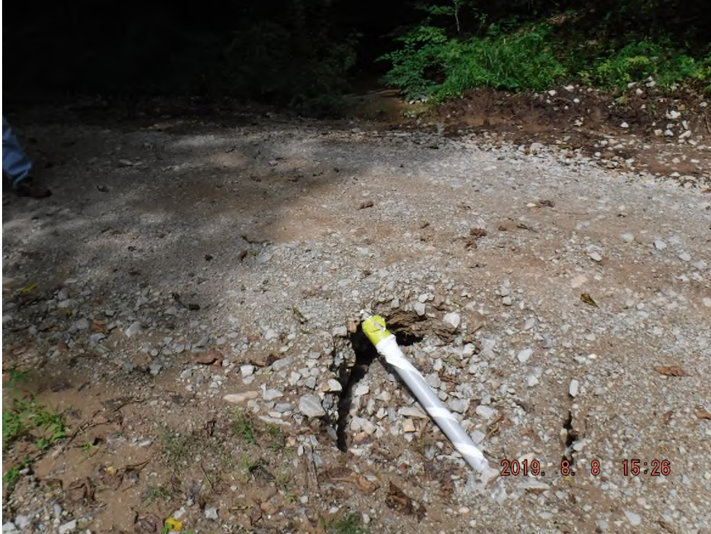
Runoff undermined the road, causing the slip.
