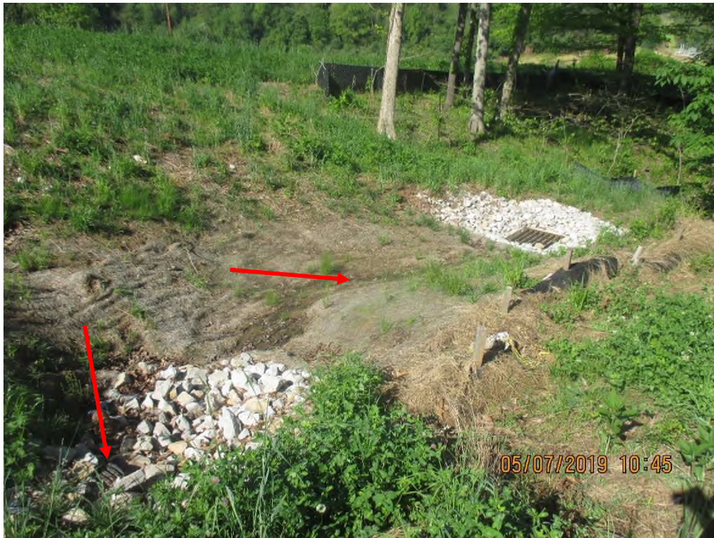
Rock check at drop inlet's outlet, upslope of drop inlet above ephemeral stream. Arrow depicts outlet pipe and erosion between rock checks and inlet.
