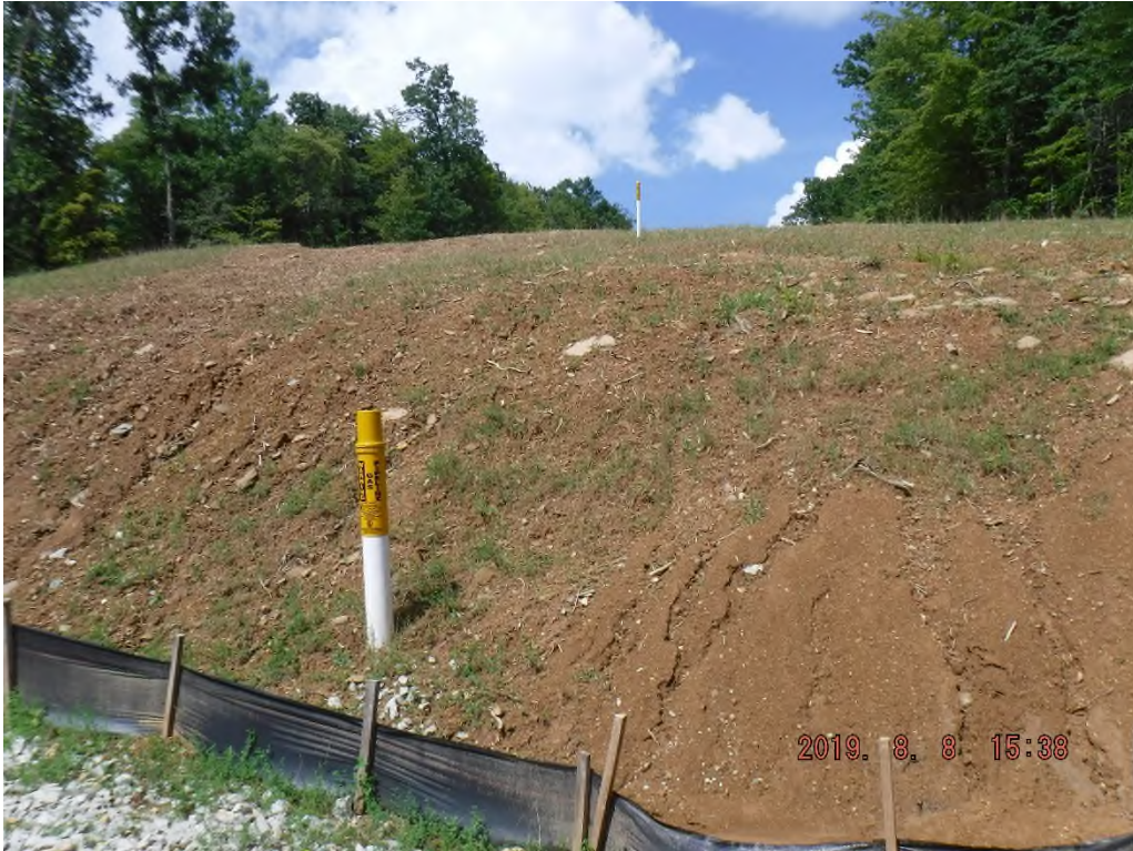
Erosion gullies on fill slope.
