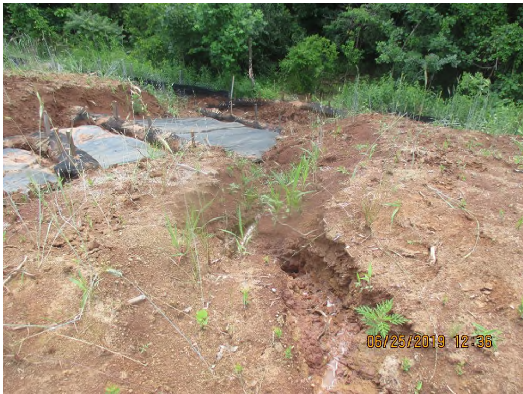
Waterbar outlet controls on slope south of ARWI 024 near station 5372+00. Perimeter controls overwhelmed with sediment. Erosion occurring under and next to Geotech fabric.
