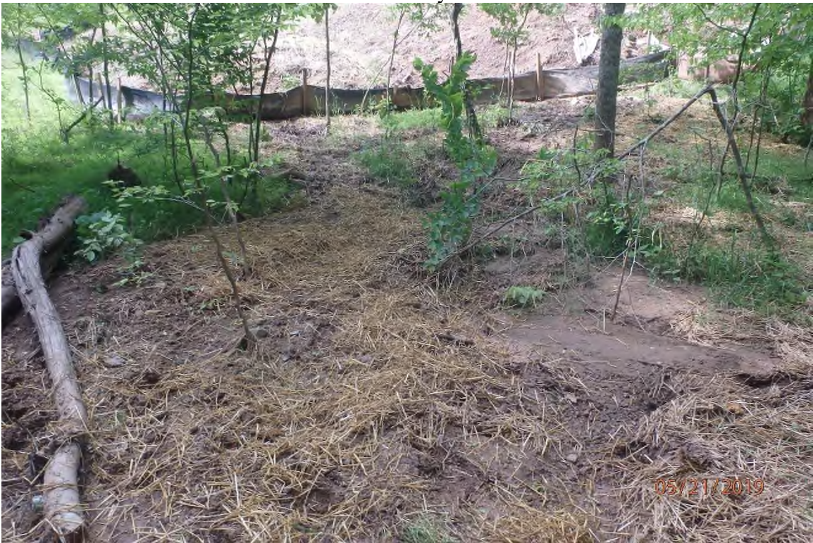
Unmaintained BMP in the Tylor Drain watershed and the sediment trail that leads to the receiving stream.
