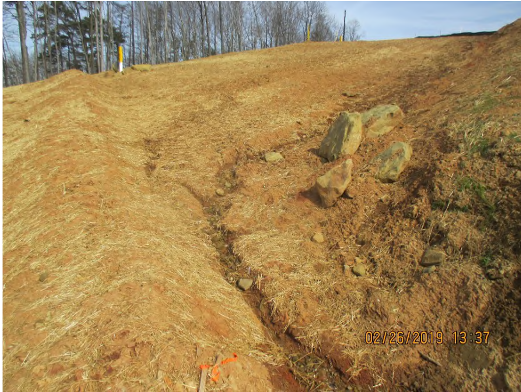
Waterbar terminus at station #6753+94. Evidence of concentrated flow due to erosion occurring along the slope.
