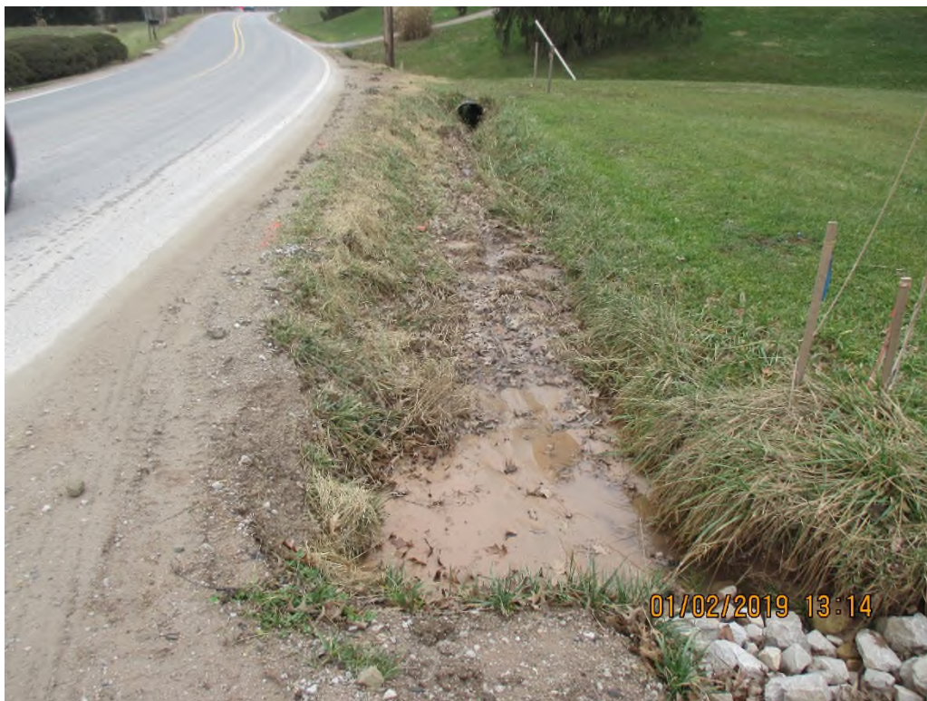
Off-site sediment deposits present in roadside ditch along route 21.
