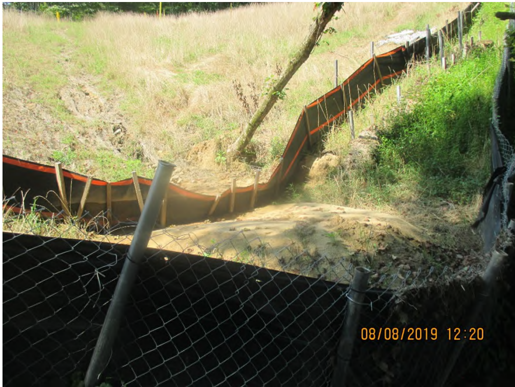
Perimeter controls overwhelmed with sediment due to erosion on slopes near station No. 8772+72.
