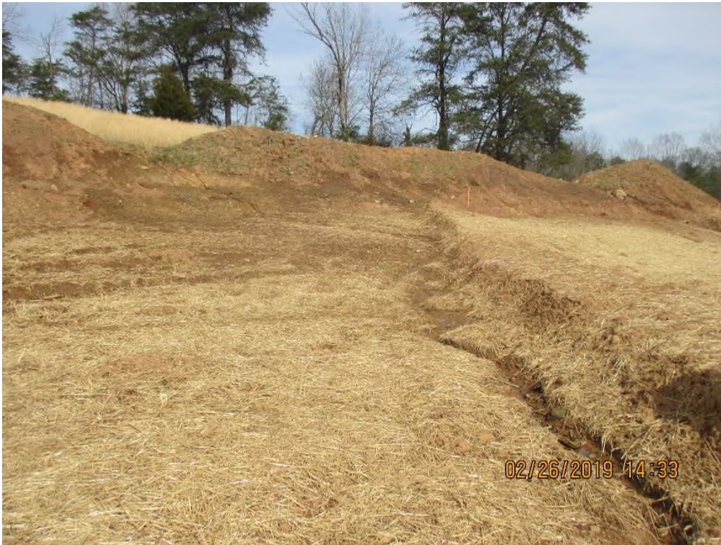
Seep near waterbar causing erosion in waterbar.
