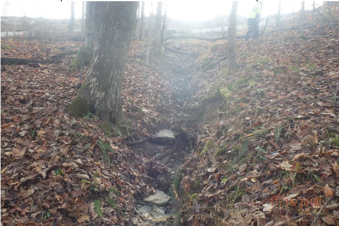
Unmaintained perimeter control and associated offsite sediment deposits near 2815+00.
