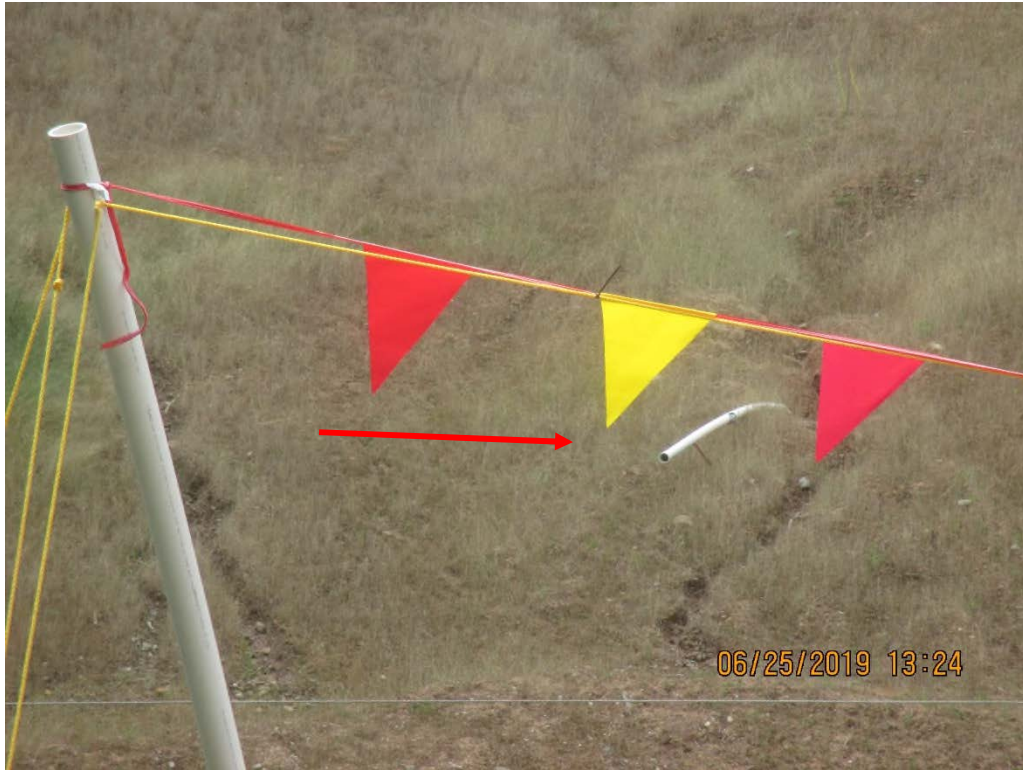
Across from Munchausen road crossing adjacent slope. Pipe trench drain terminating onto unprotected slope.
