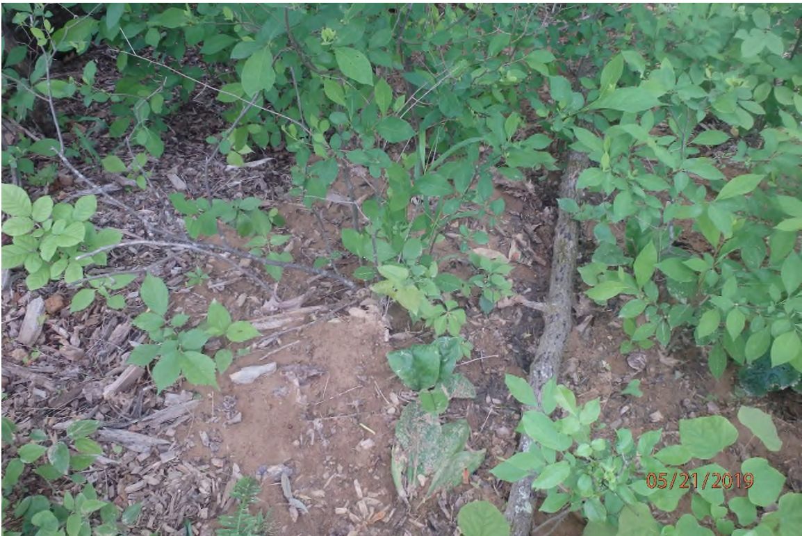
Area adjacent to 3314+00 where the approved SWPPP does not indicate the need for perimeter controls and the plan has proved inadequate. Offsite sediment deposits documented in lower photo.
