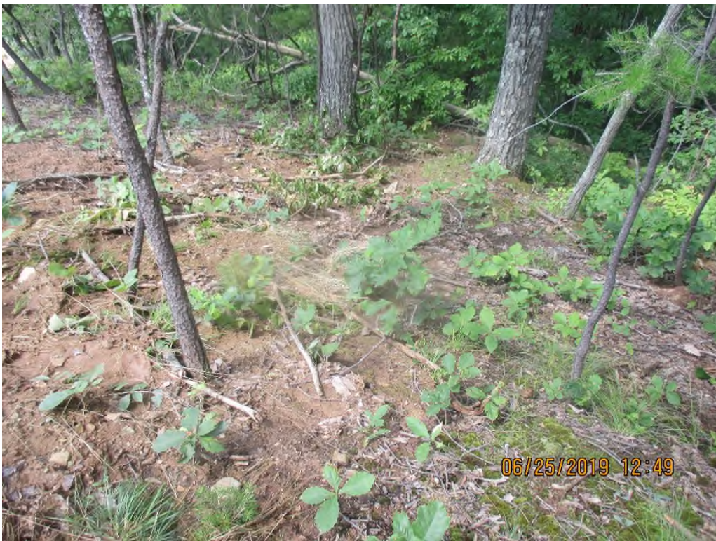
South of Station No. 5396+00. Downslope of overwhelmed Waterbar outlet controls with sediment deposits past LOD.
