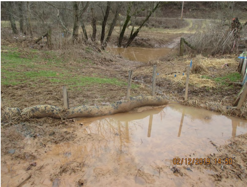
SLW leaving site upslope of Stream SROC-030
