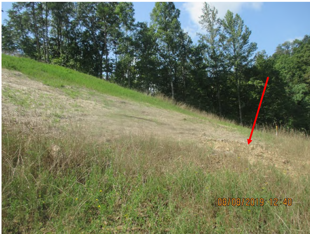
Area where curlex had been added to stabilize slope. Soil was slipping from under the curlex and being transported downslope towards perimeter controls. Arrow depicts slipped material.
