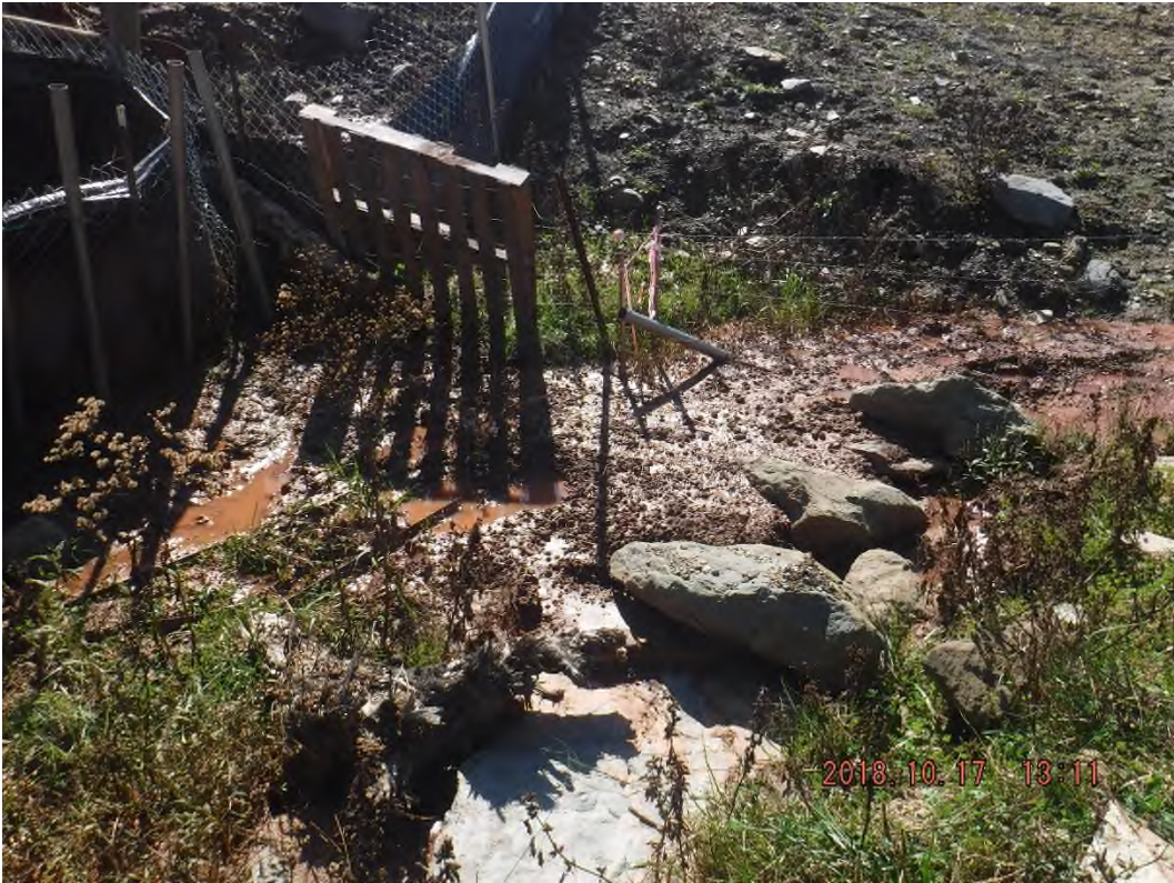
Sediment directly below silt fence.
