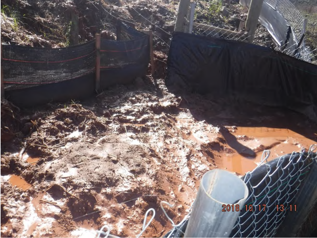
Sediment collected inside silt fence.
