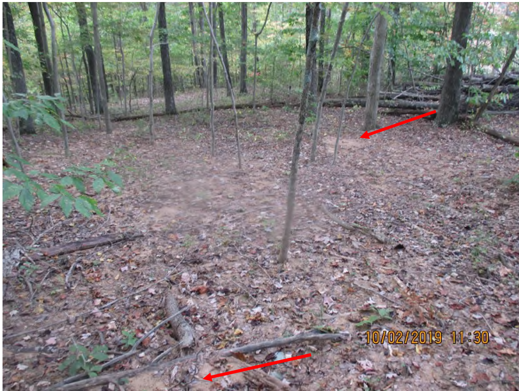
Sediment deposits observed past the LOD downslope from where gully erosion was occurring, and no waterbar outlet or perimeter controls were observed. Arrow depicts sediment deposits observed.
