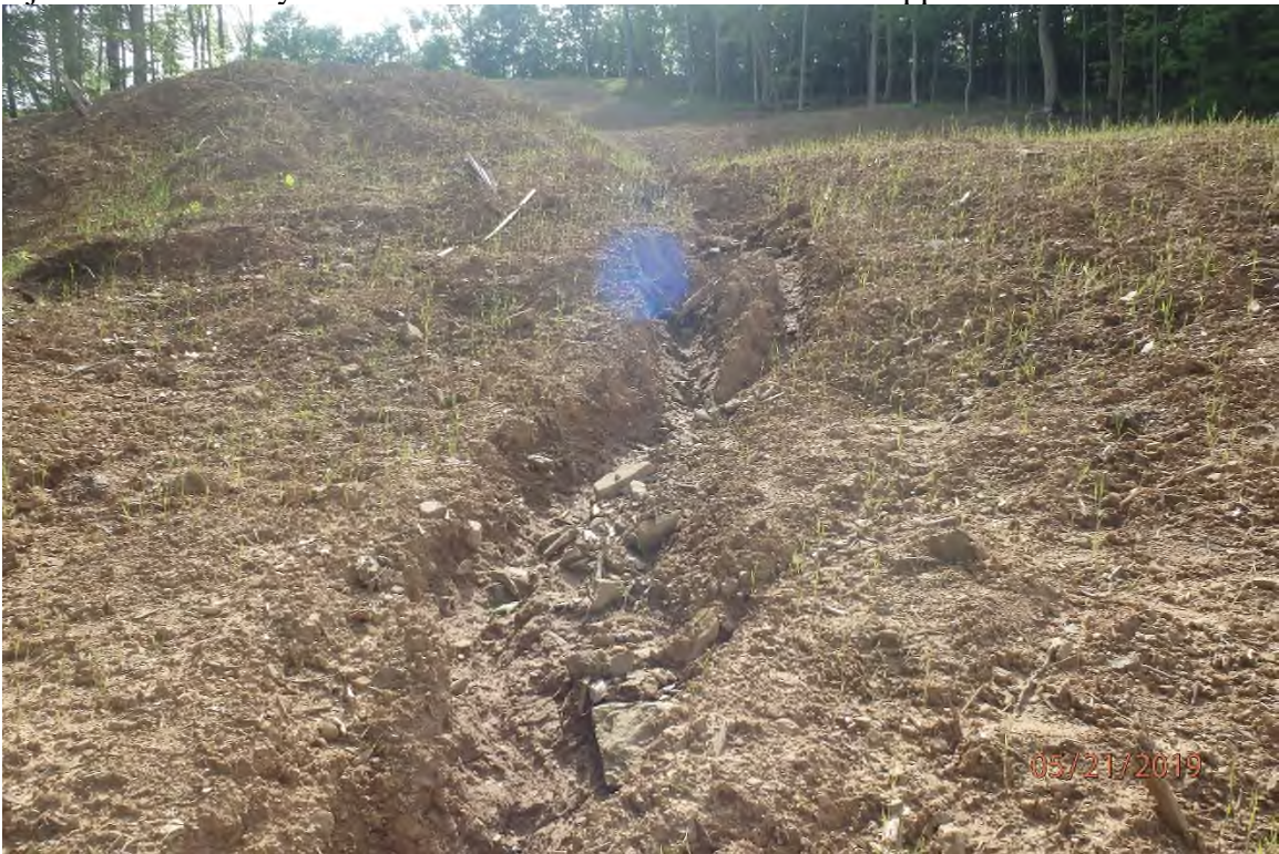
Fill slope erosion as a result of the above pictured deficiency.
