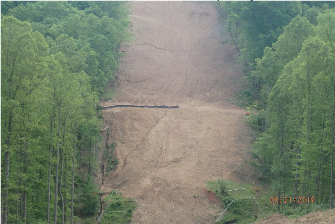
Slope adjacent to UNT Taylor Drain where water bars that are in the approved SWPPP are not in place.
