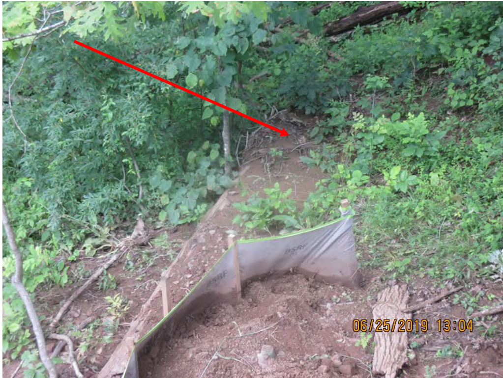
South of Station No. 5396+00. Sediment being deposited past log piles beyond LOD.
