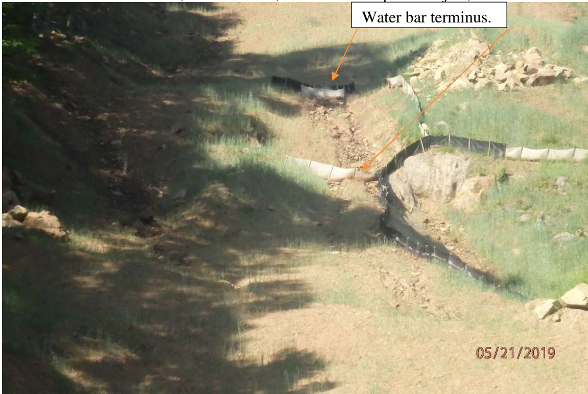
Improperly installed water bars in the UNT Georgescamp Run watershed.
