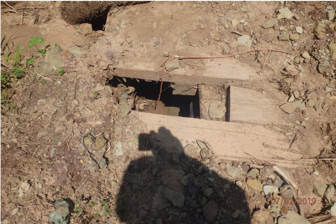
The installed timber mat bridge at the UNT Left Fork of Arnolds Creek (SDOG040) crossing showing the need for maintenance.
