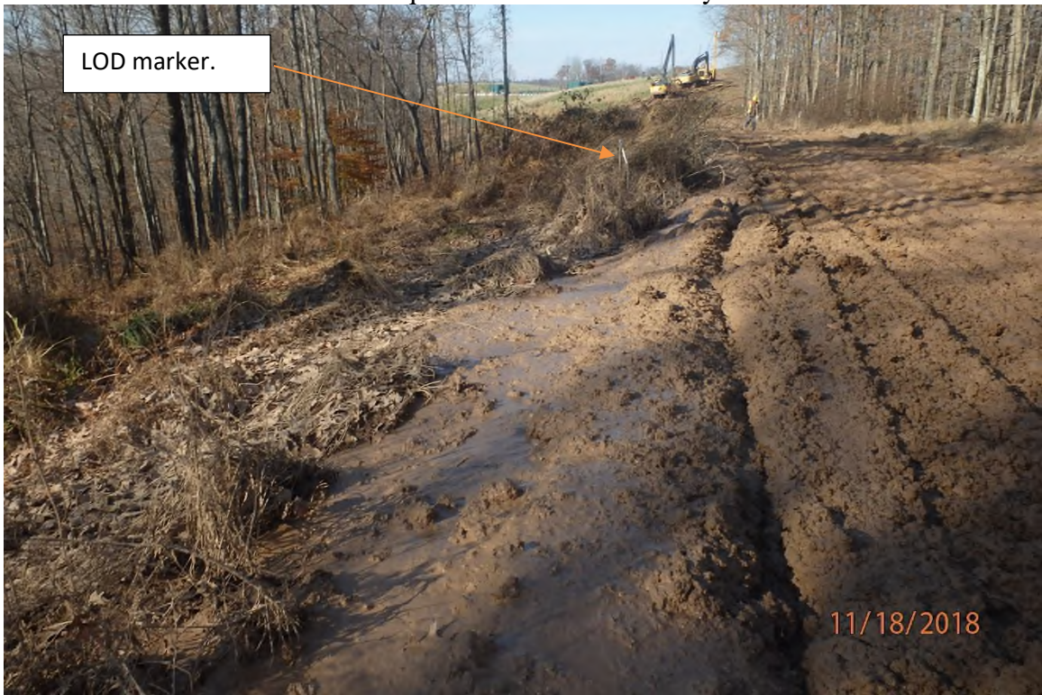
ARDO008.4 showing the lack of a graveled surface and the lack of perimeter controls, even though the road requires construction activity.
