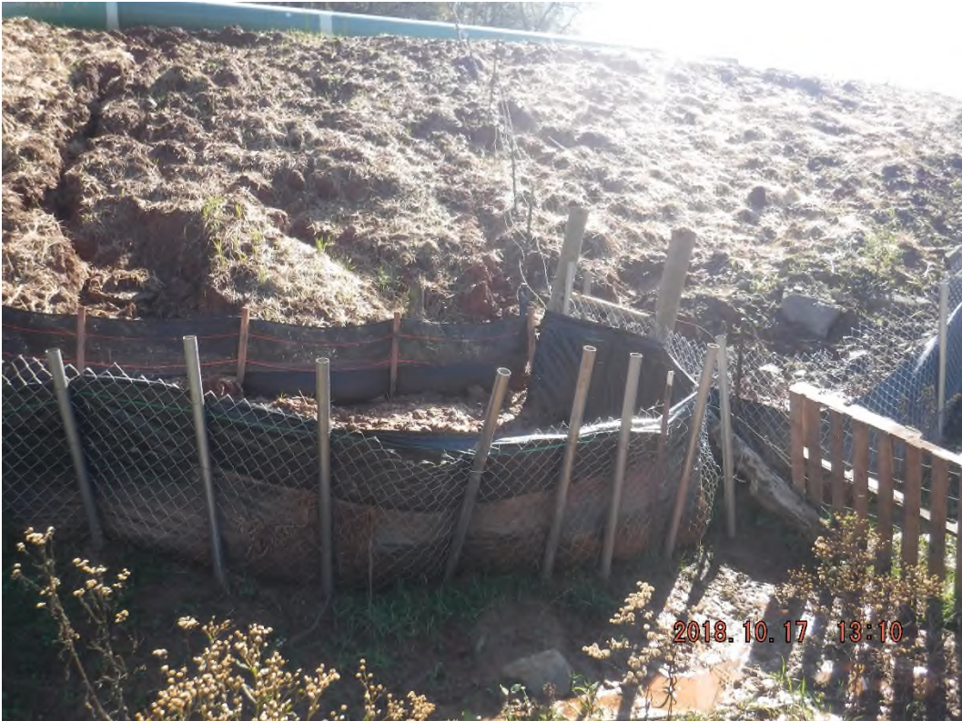
Super silt fence adjacent to the farm pond.
