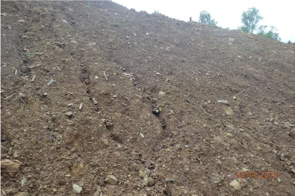
Fill slope erosion near 2065+00. The area has been idle for a long period of time and lacks temporary stabilization.
