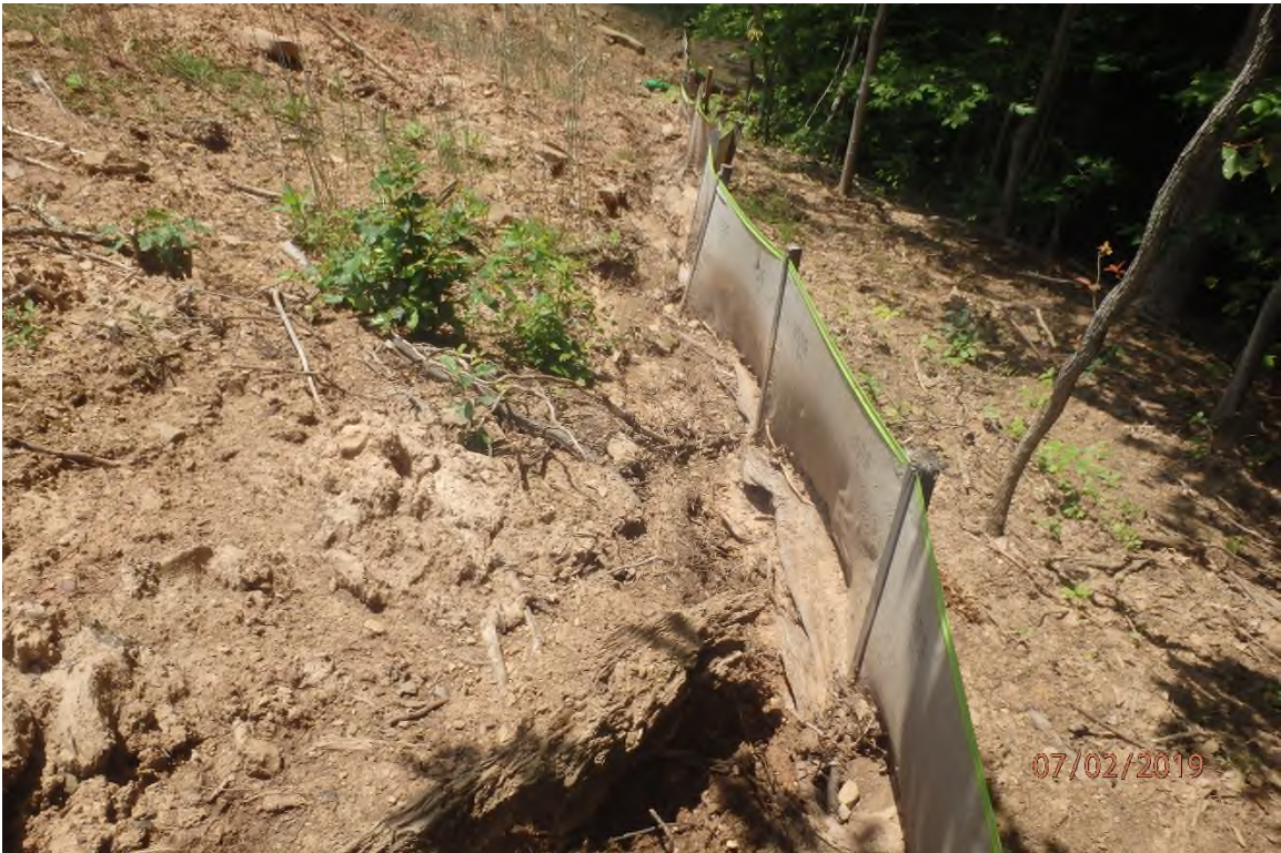
Fill slope erosion along the installed silt fence trench as a result of the above pictured deficiency.
