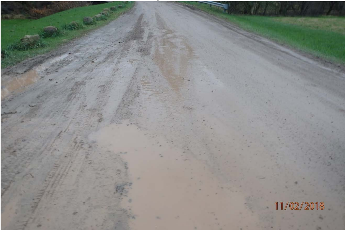
Mud on CR 5 (Riggins Run Road) that originates from AR-20 (ARDO-001.5).
