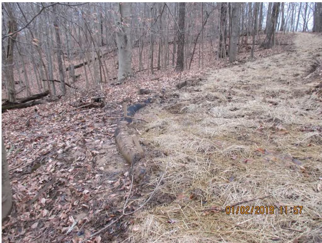
Access road with BMP being overwhelmed and needing maintained or enhanced.
