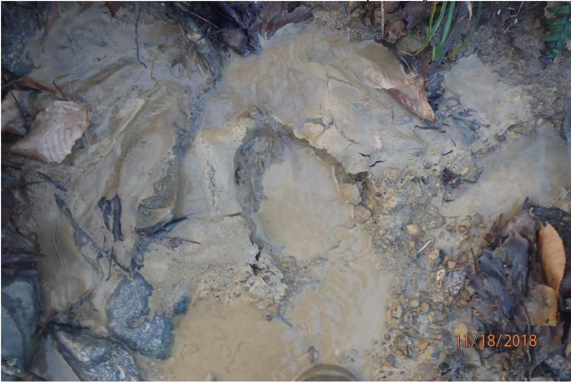
CNA deposits in UNT Bluestone Creek (39° 14.761' X 80° 45.019') near 2815+00 due to poor maintenance of perimeter control.
