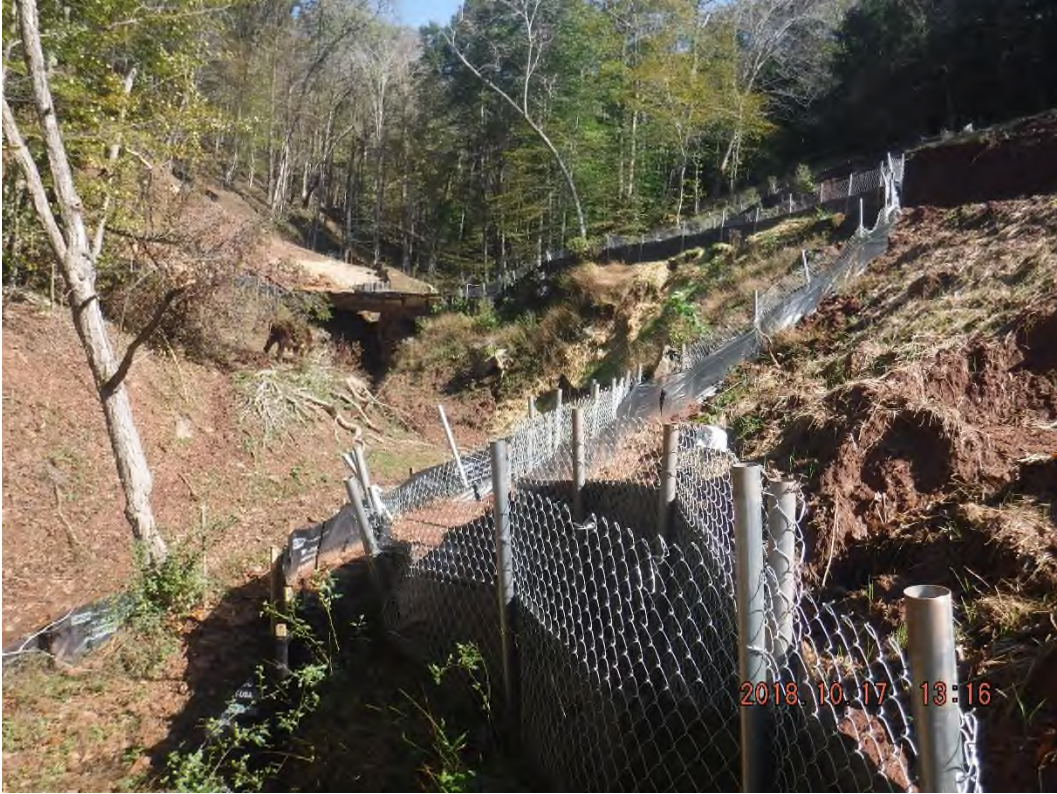
The crossing at Station 6705+00.
