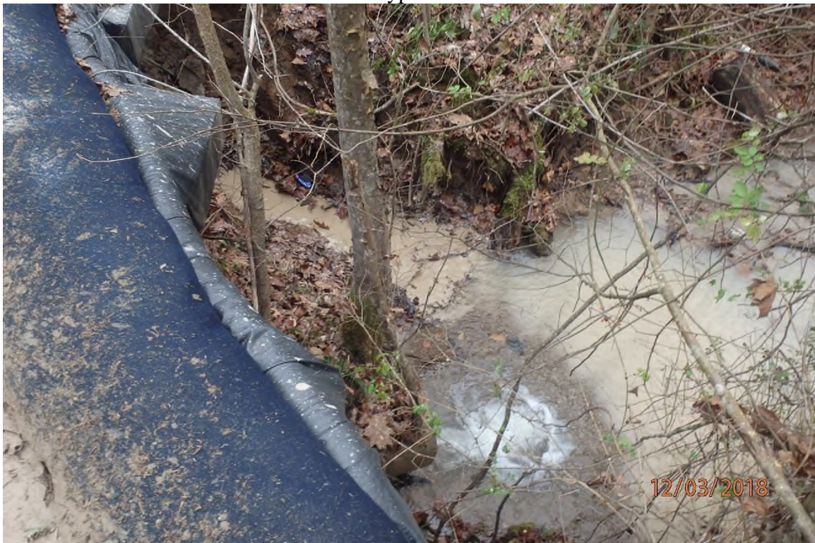
Offsite sediment deposits and CNA in UNT Douglascamp Run as a result of sediment laden water bypassing the equipment bridge BMP due to poor maintenance.
