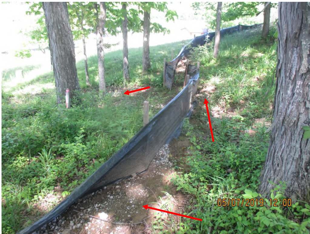
Downslope of erosion gully. Sediment deposited behind controls and being transported along perimeter controls and past LOD.
