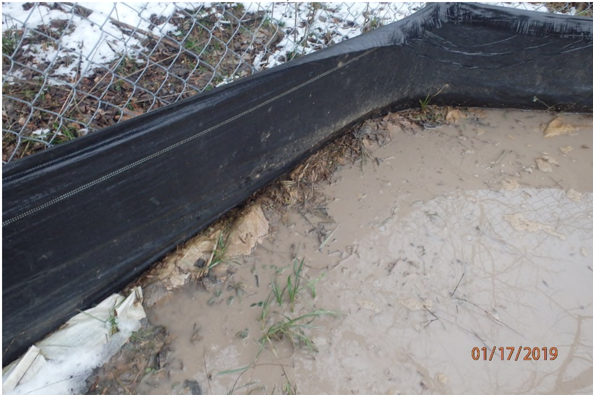
Improperly installed silt fence in the eastern portion of the project.
