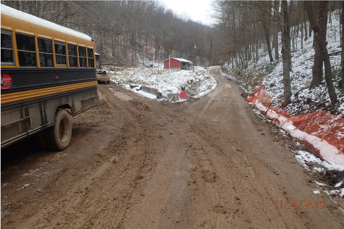
ARDO002.41 (Ralphs Run Access) showing the lack of a stable construction entrance and track-out onto the public road (paved surface).
