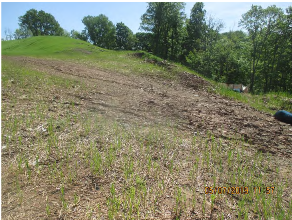
Area of unstabilized slope with erosion occurring on western side of project.
