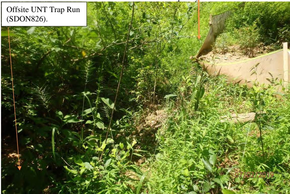
Perimeter controls downslope of the previously pictured deficiency in the Trap Run watershed that has become inundated with sediment as a result of poorly installed water bars. Area where sediment laden water is leaving the site is pictured.
