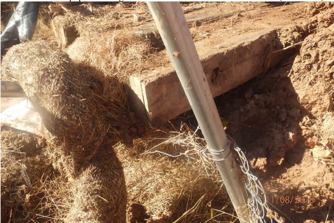
Unmaintained equipment bridge BMP in the Bluestone Creek watershed (SDOI205).
