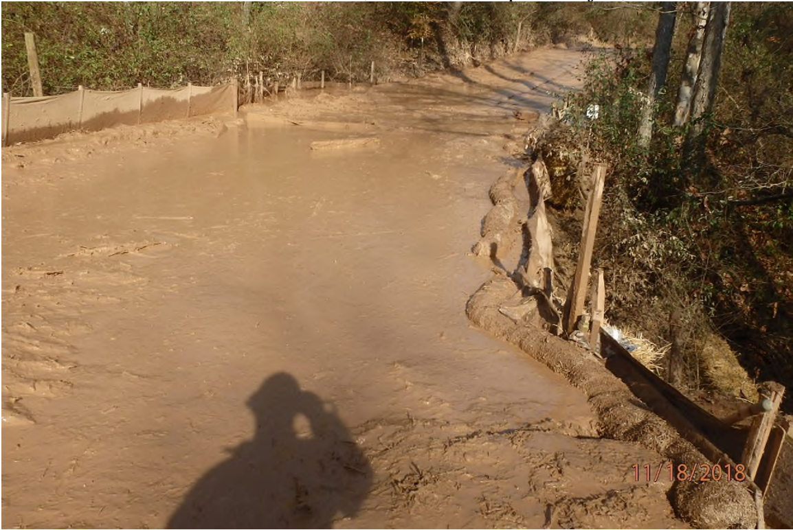
UNT Bluestone Creek equipment crossing on ARDO009.3 showing overwhelmed BMPs due to the lack of drainage indicated on the approved SWPPP.
