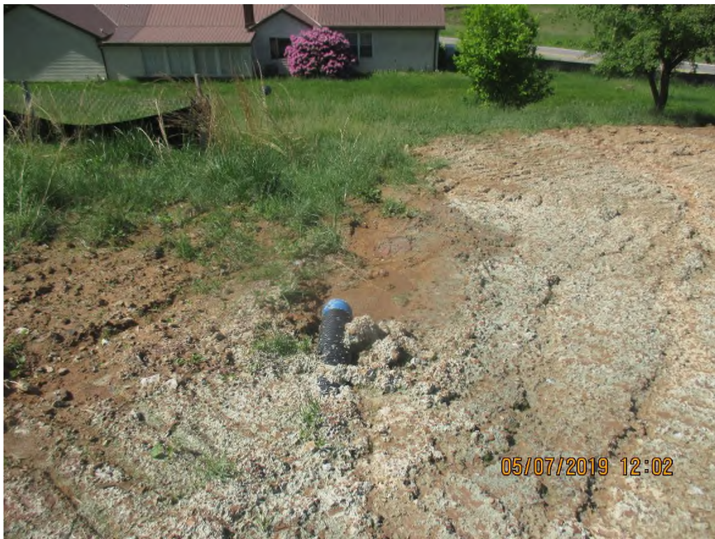
Slope drain outlet terminating onto slope above vegetated buffer.
