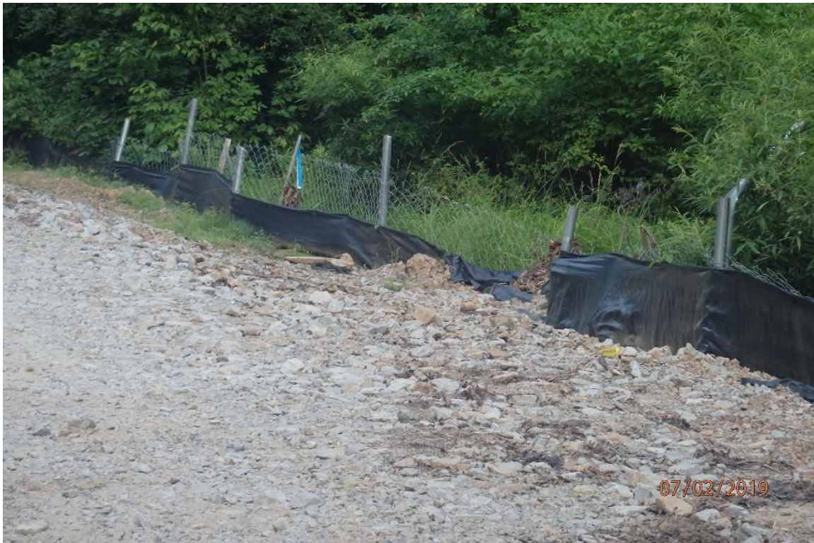
Perimeter control in need of maintenance at ARDO016.
