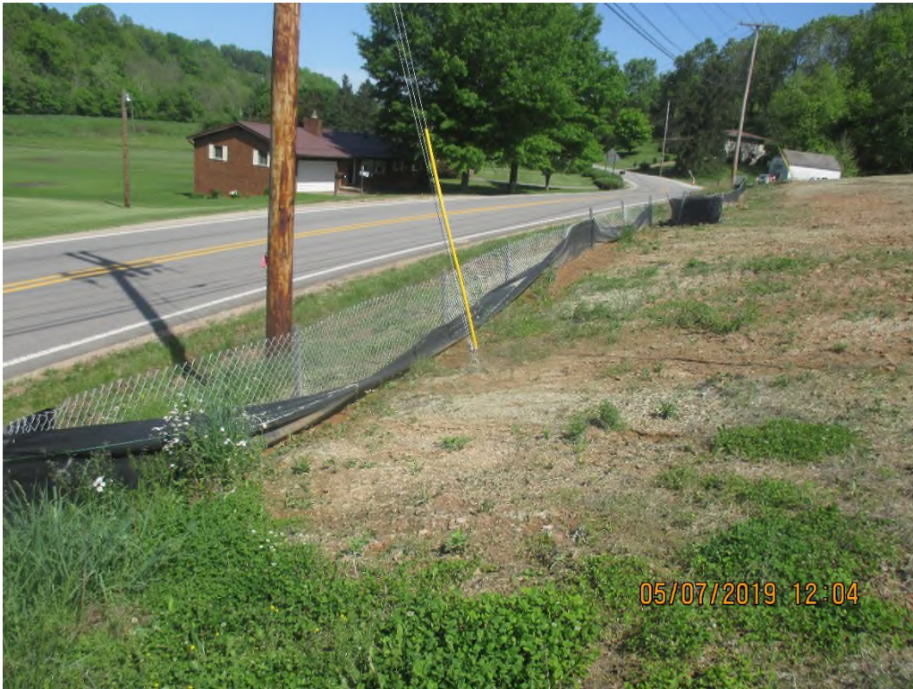
Downslope of slope drain outlet on west slope above LOD. Erosion present on slope, depositing sediment into and through perimeter controls. Super silt fence not maintained.
