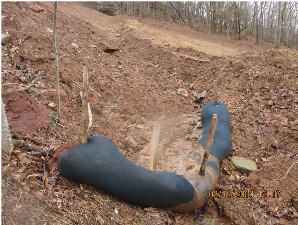
Waterbar Outlet #1 near station #5398+00 facing upslope
