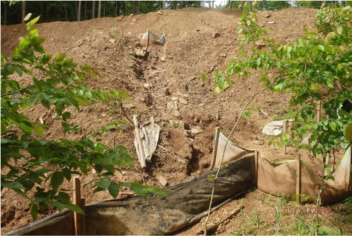
Unmaintained BMP in the Tylor Drain watershed.
