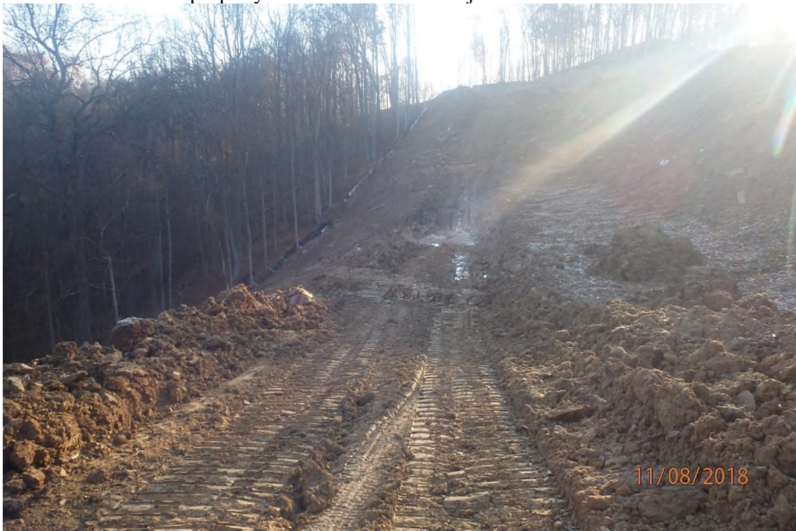
Improperly installed water bars adjacent to 2822+00.
