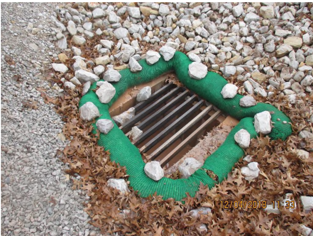
Drop inlet where sediment laden water was entering from pressure wash station.
