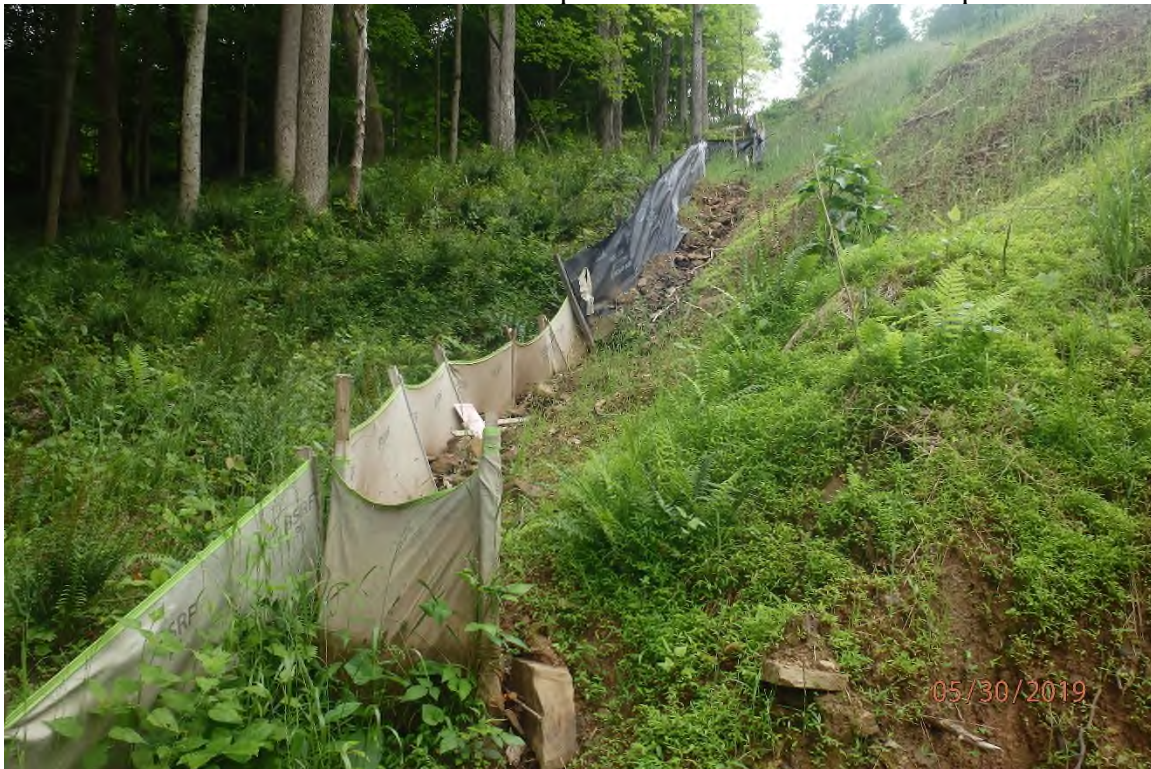
Close up view of the above pictured deficiency.
