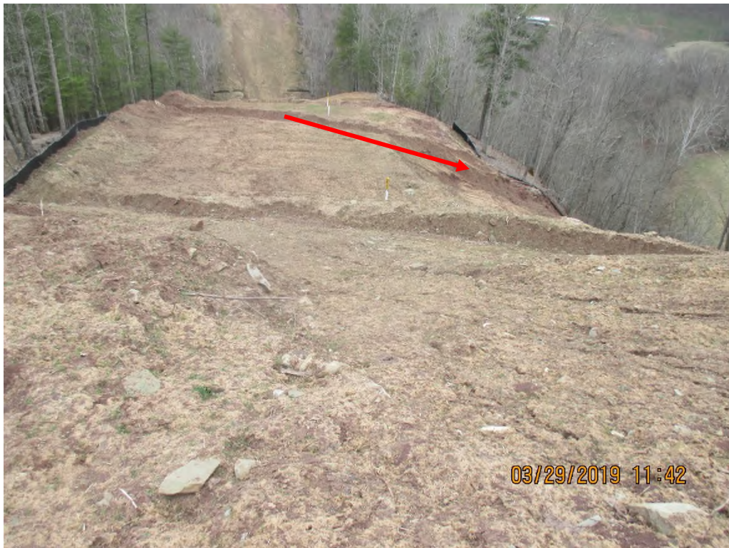
ROW facing South above Stream SWIF-057 near station #5163+50. Arrow depicts additional slipped area of slope above stream.
