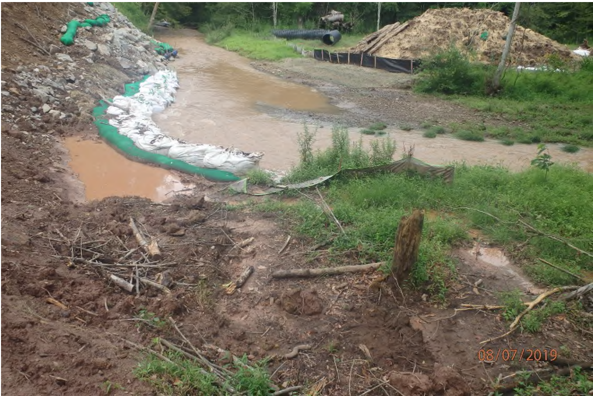
Perimeter controls at the slip repair site showing the need for maintenance.
