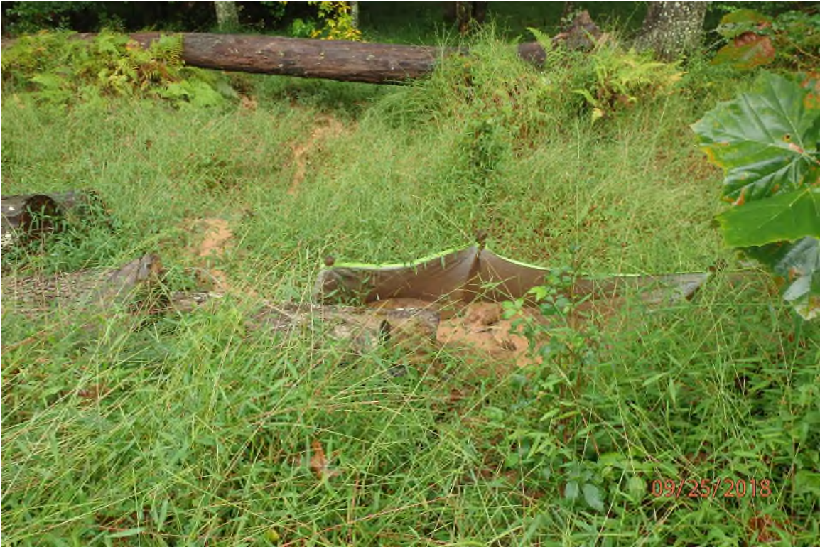
Sediment and diesel laden water bypassing a perimeter control.
