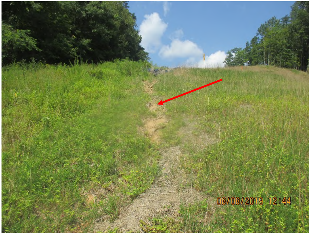
Facing upslope towards waterbar outlet controls. Arrow depicts erosion caused by outlet control failure.
