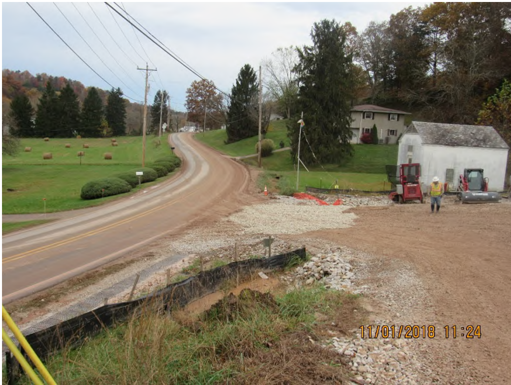
Rt 21 and construction entrance.
