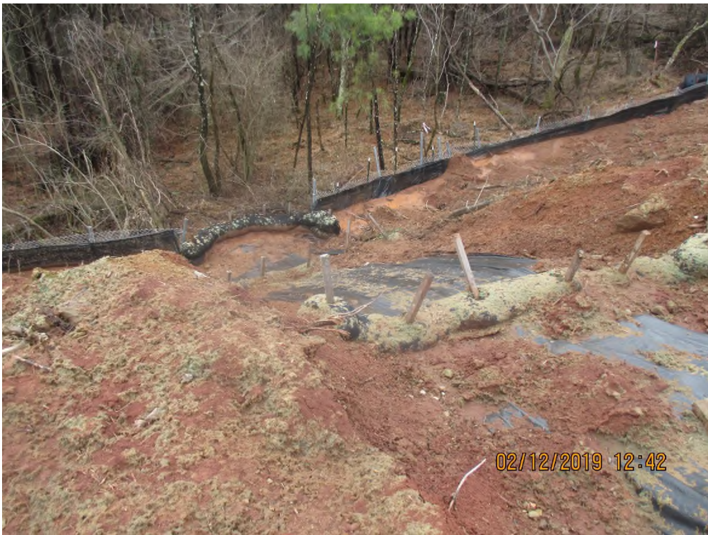
Waterbar outlet near station 5376+00.
