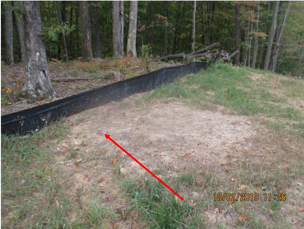
Waterbar terminating into perimeter controls near station No. 3380+84. Sediment being deposited against controls. Arrow depicts waterbar flow.
