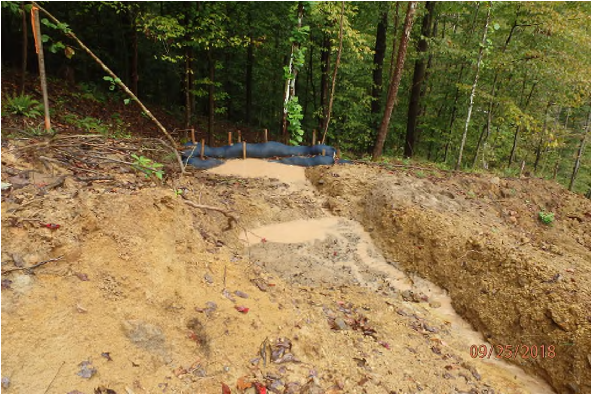
Water bar terminus BMP adjacent to 2275+00 allowing sediment laden water to bypass under the device.
