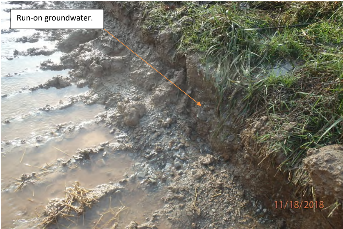
Run-on groundwater on ARDO008.5 that is running into the road surface contrary to the approved SWPPP.
