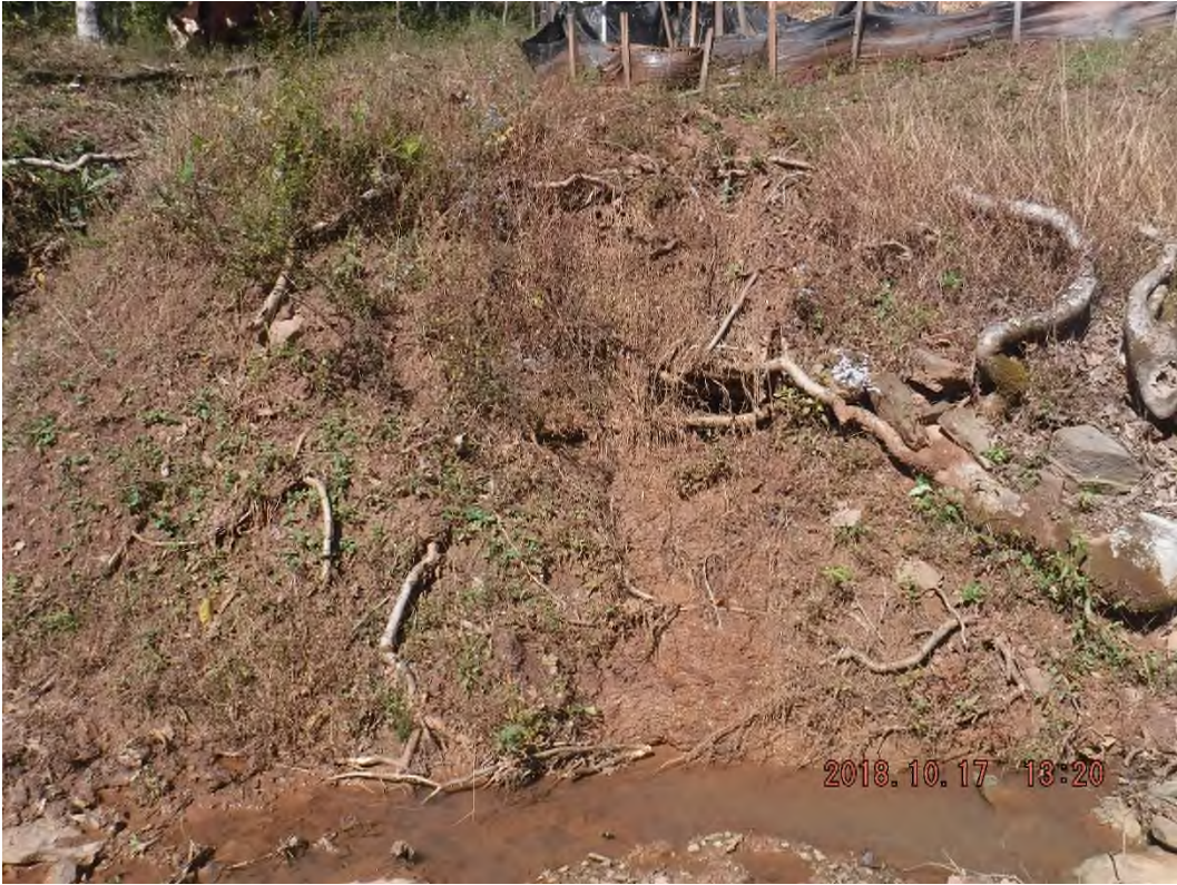
Evidence of a discharge of sediment laden water from silt fence above.
