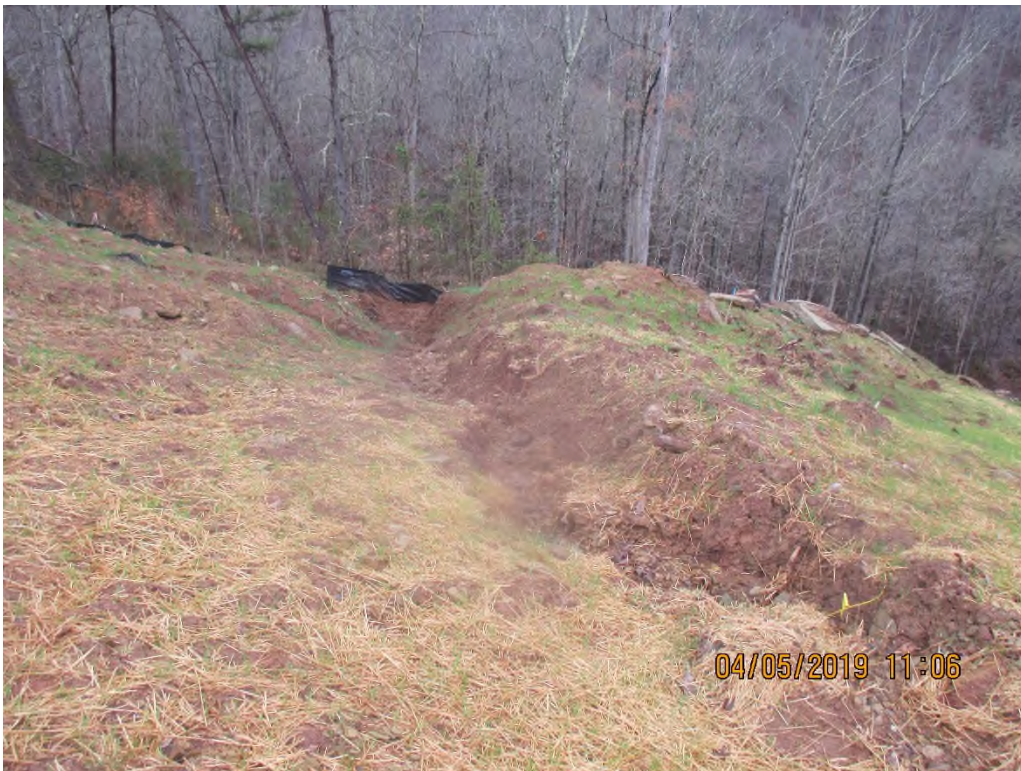
Waterbar near station #6810+00. Erosion present in waterbar and slope at terminus.
