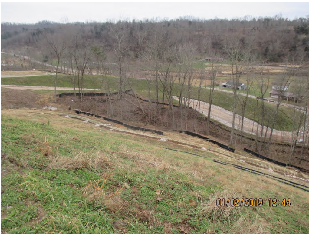
Western side of project facing toward Route 21 and construction entrance.
