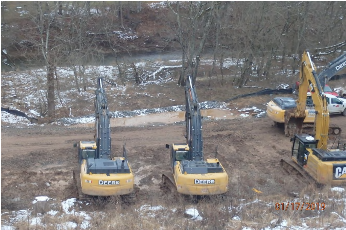
Overview of the area where the proposed basin (Basin 2) was to be constructed.
