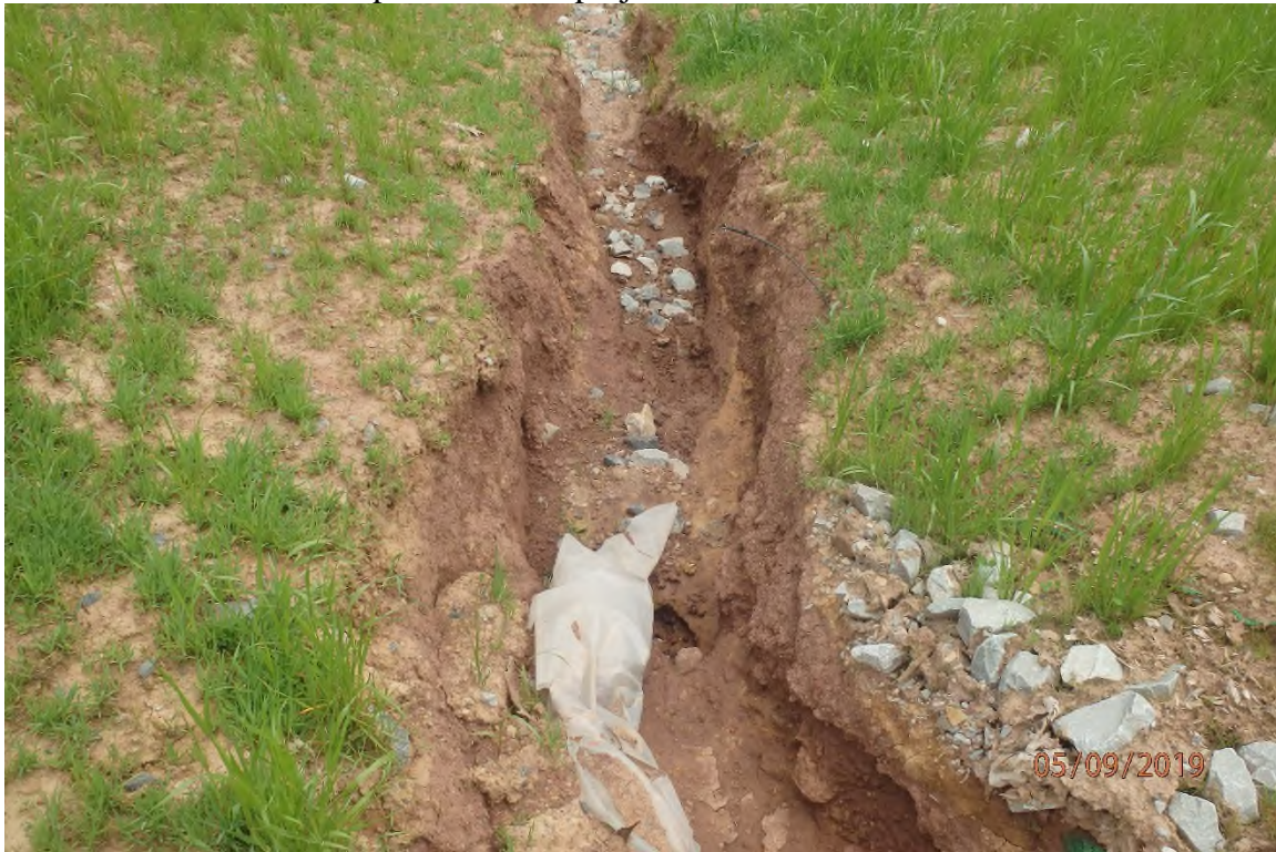
Diversion in the southern portion of the project that is eroded and in need of maintenance.
