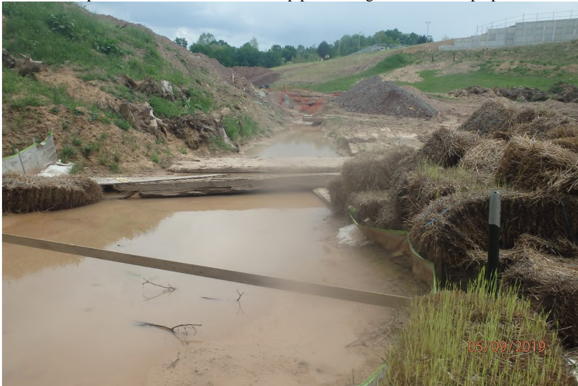
Diversion carrying stormwater from the basin outlet to the makeshift treatment structure.
