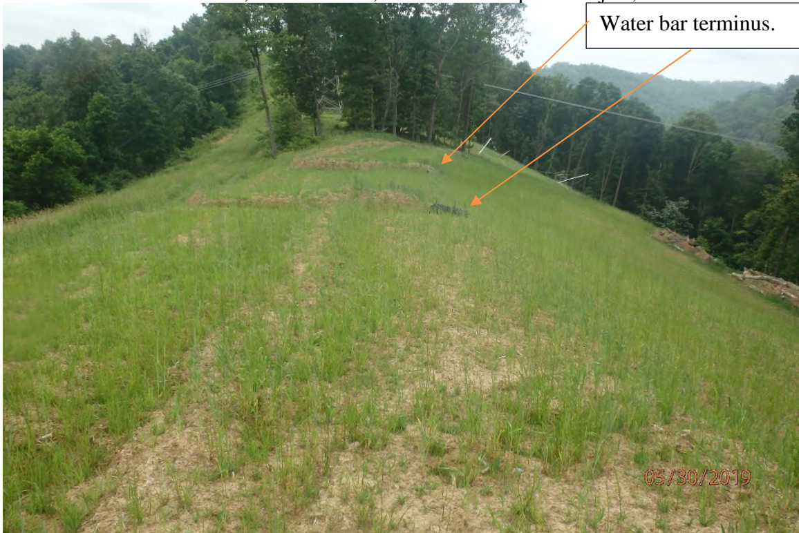
Improperly installed water bars in the Englands Run watershed.
