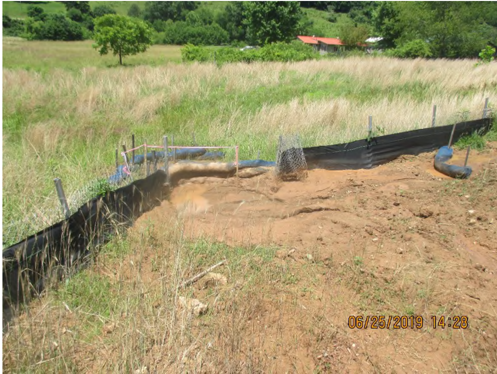
Perimeter controls at station No. 5638+46.
