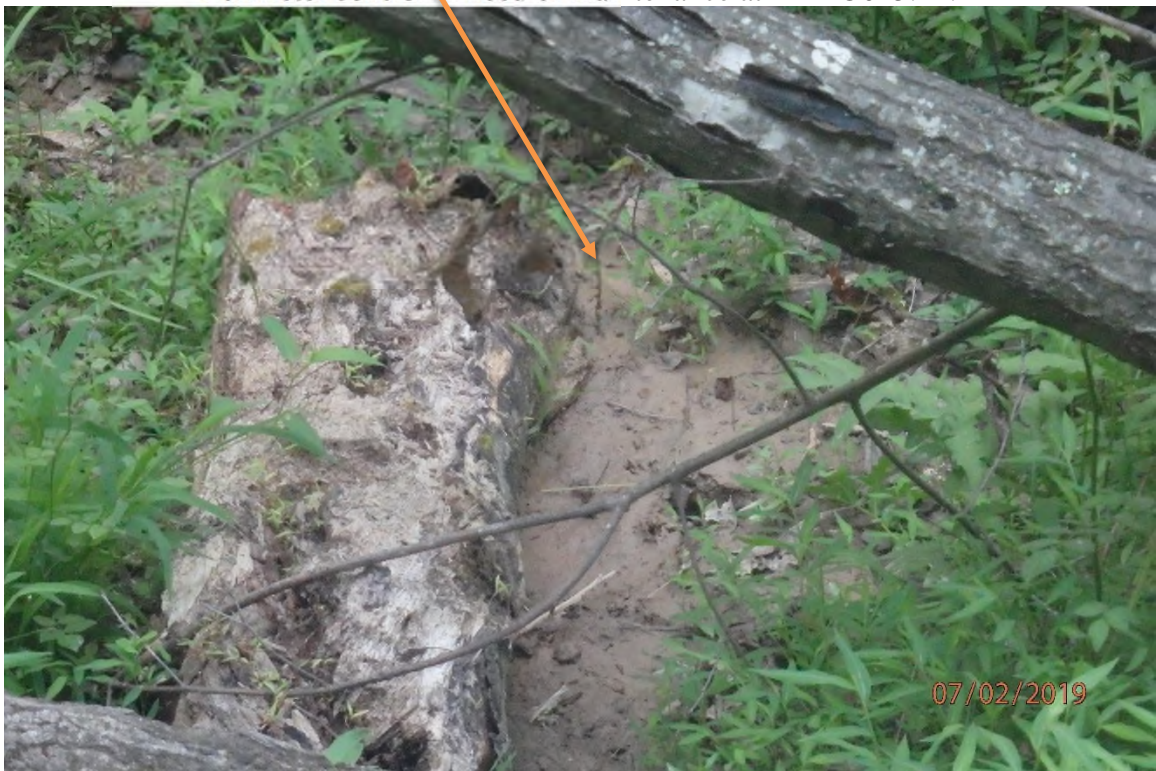
Offsite sediment deposits as a result of the above pictured deficiency.
