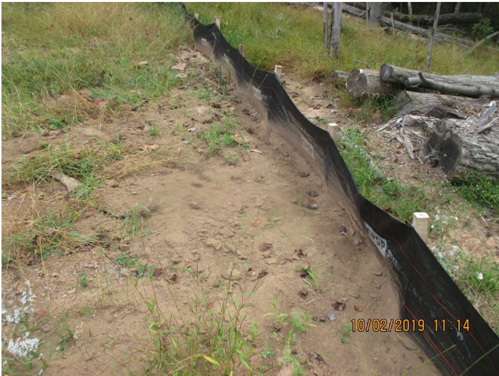
Downslope of gully erosion occurring on slope. Sediment deposited behind and past controls near station No. 3368+00.
