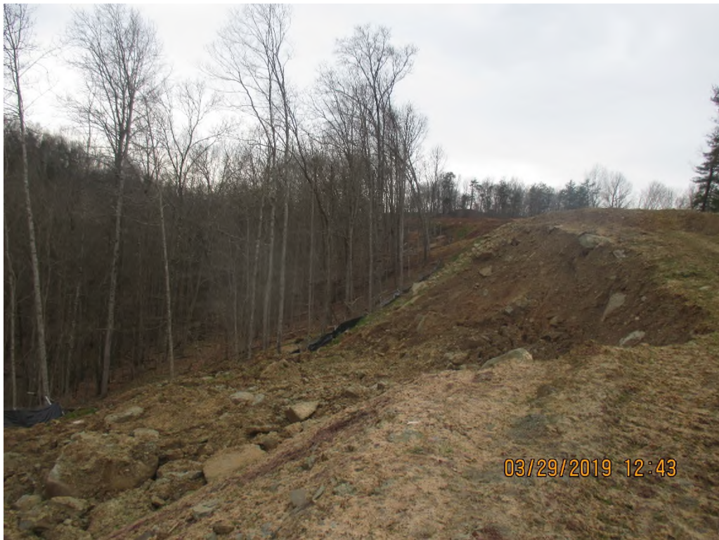
Slip at station #5168+80 facing South. Sediment deposited past LOD
