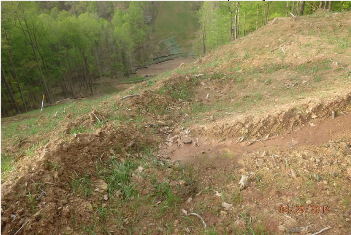
Improperly installed water bar with varying angles that is installed with a height less than 16" adjacent to 2226+50.
