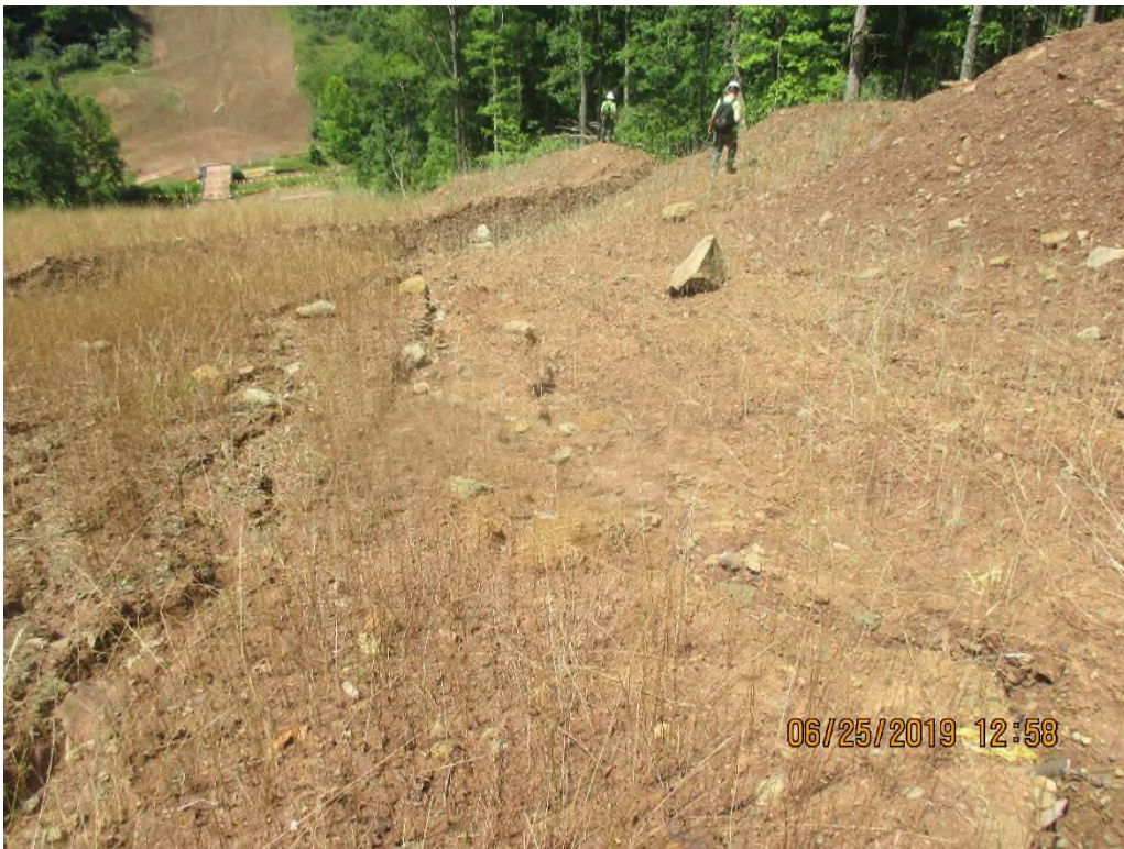
South of Station No. 5396+00. Erosion on slope above Munchausen Road Crossing leading towards waterbar and perimeter controls.
