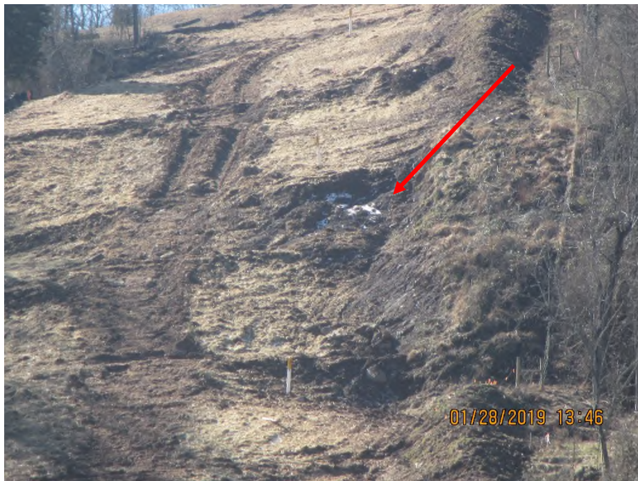
Section of ROW above Shamblin Run where topsoil pile had slipped, and material was deposited into waterbar.
