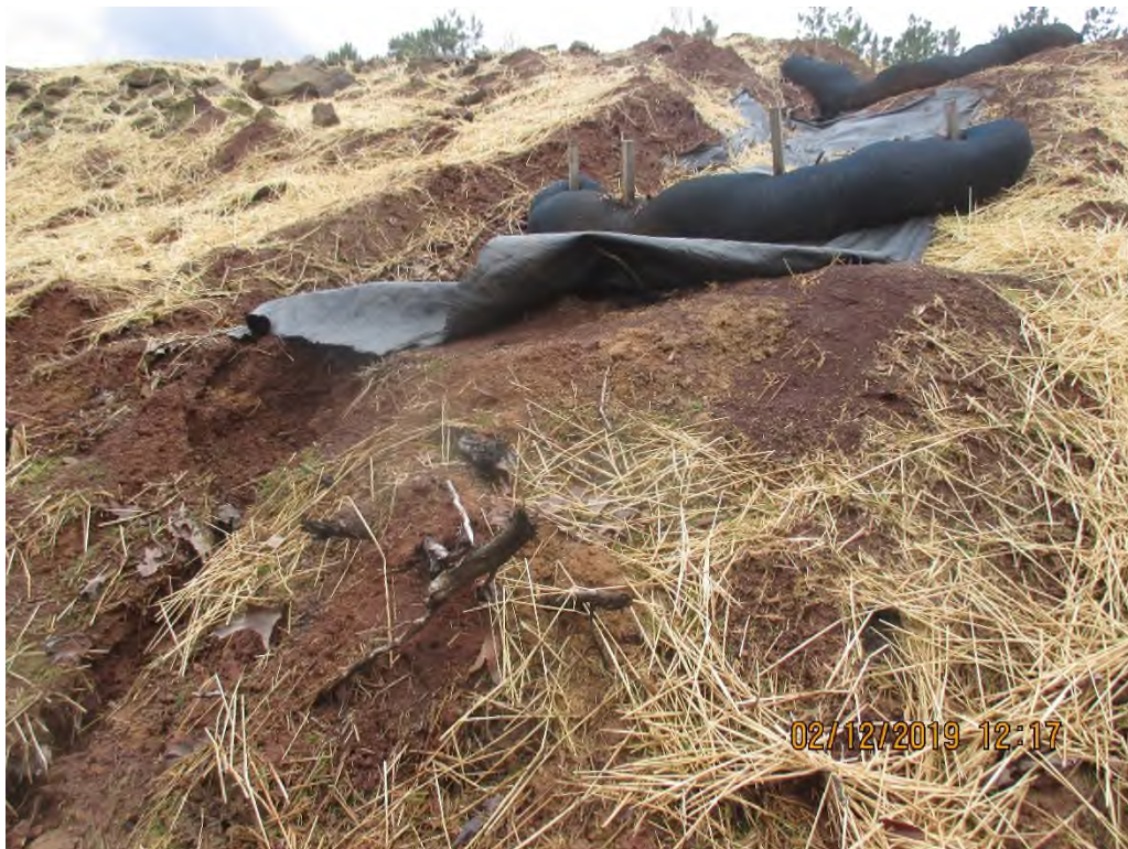
Waterbar terminus at station #5359+00 facing upslope
