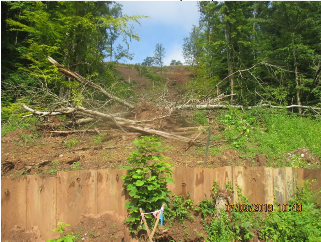
Upslope toward MXP ROW at Sulu Road toward ongoing slip at station No. 7347+00.
