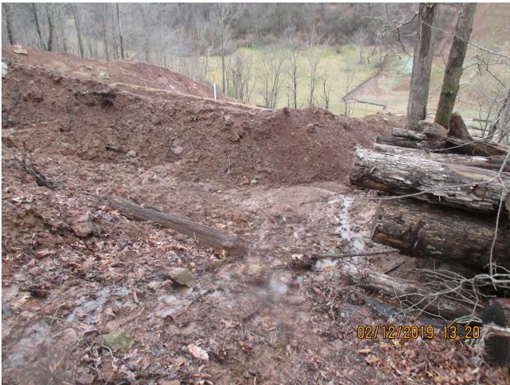
Off site sediment deposits present and SLW flowing past controls above log pile near station 5400+00
