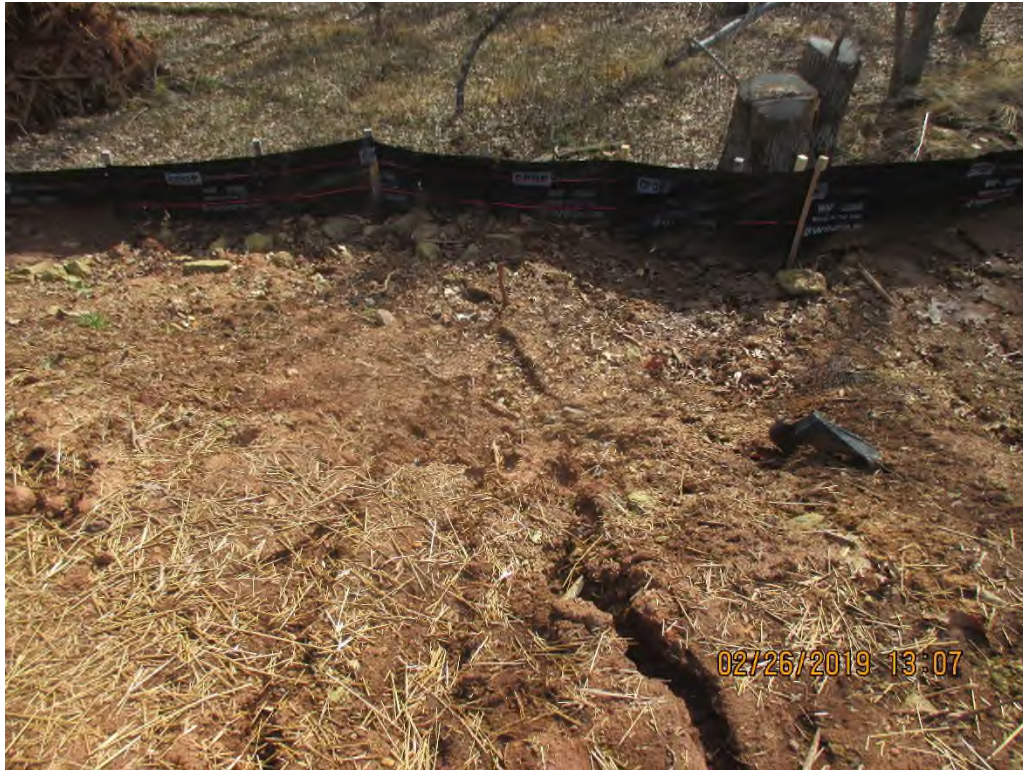
Erosion on slope above perimeter control at station #6766+60. Silt fence had multiple holes.
