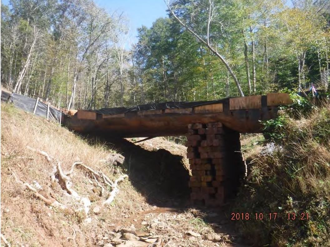
Crossing at Station 6705+00.
