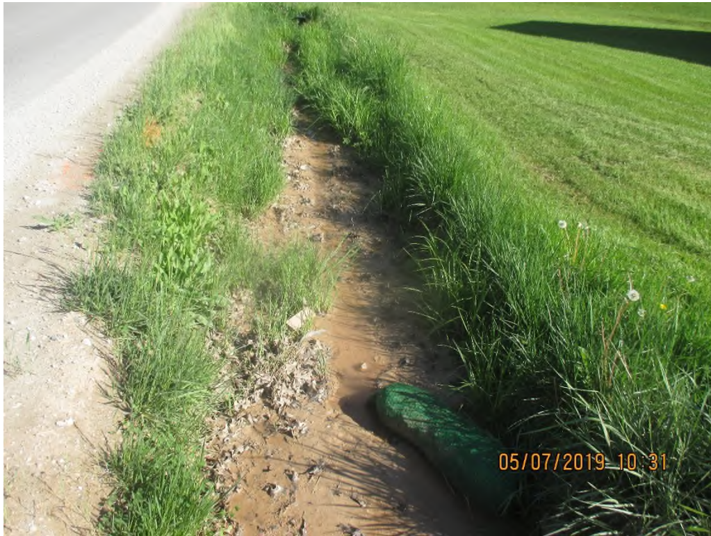
Roadside ditch below roadside drain and drop inlet outlets. Sediment present in ditch that conveys to UNT of Grasslick Run.
