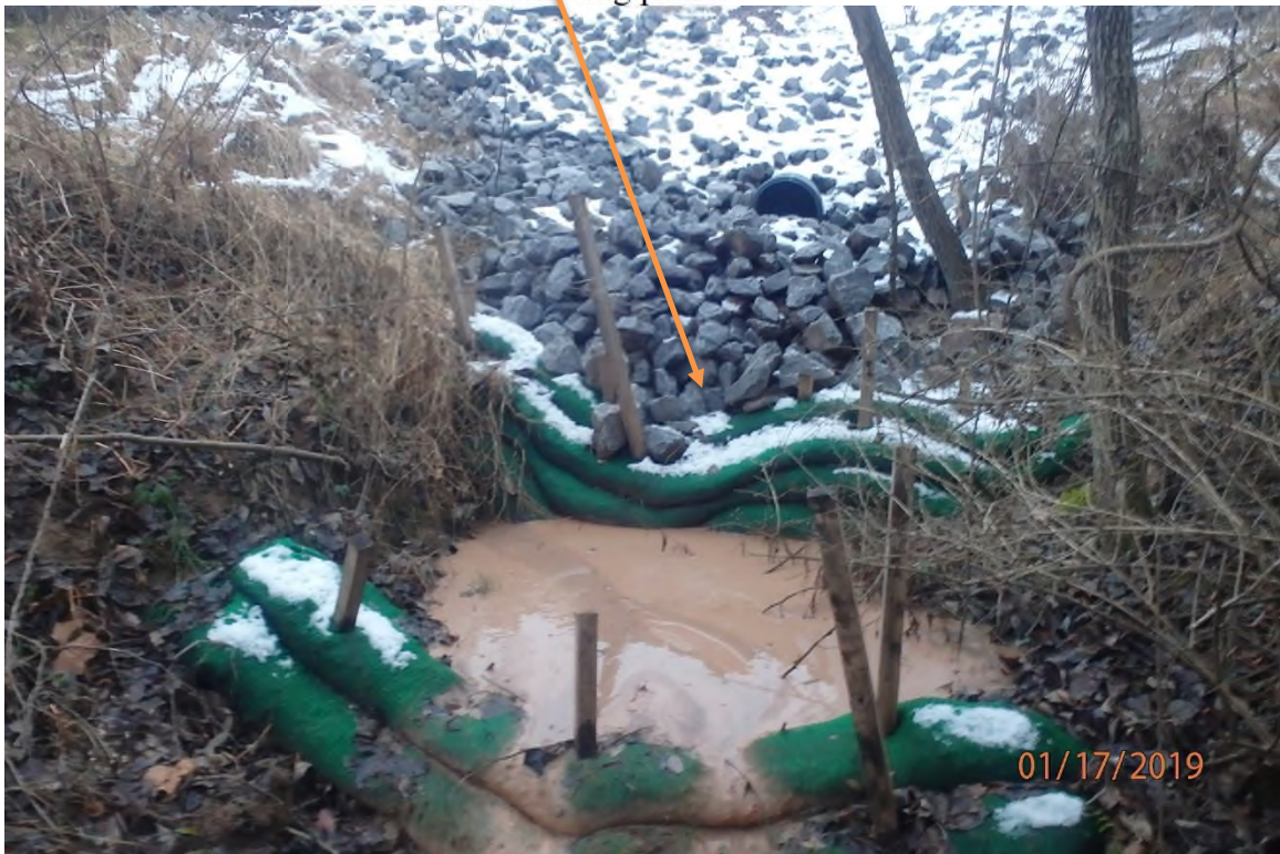
Installed BMPs downslope of truck wash.
