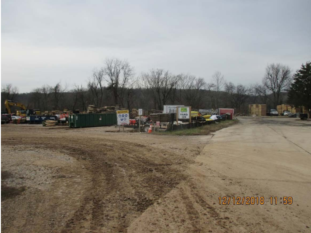
Tracking occurring from contractor yard onto access road that leads to Route 62.
