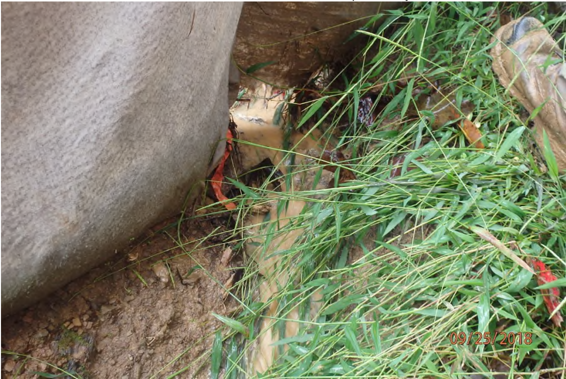
Stormwater bypass of perimeter control adjacent to 2260+00 due to poor maintenance.
