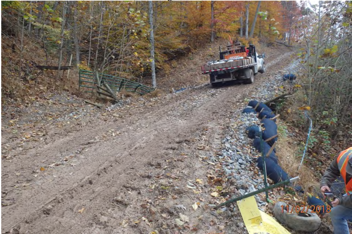
AR – 17 (ARDO002.8) showing an unstable construction entrance.
