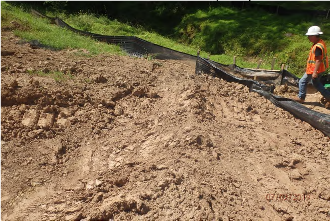
Improperly installed water bar in the Taylor Drain watershed. Water bar terminates prior to the installed perimeter control (sheet flow silt fence in concentrated flow area).
