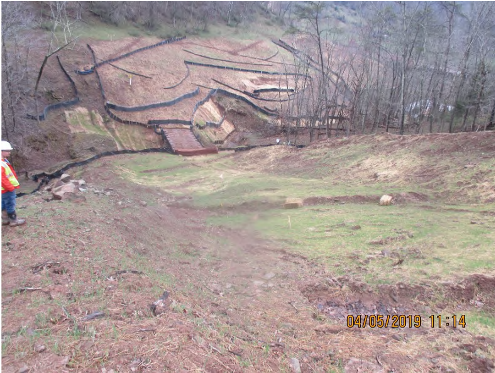
Waterbar above stream SJAG-316 terminating into topsoil pile. Erosion occurring below waterbar on ROW due to concentrated flow overtopping the waterbar at the terminus and running downslope along topsoil pile.
