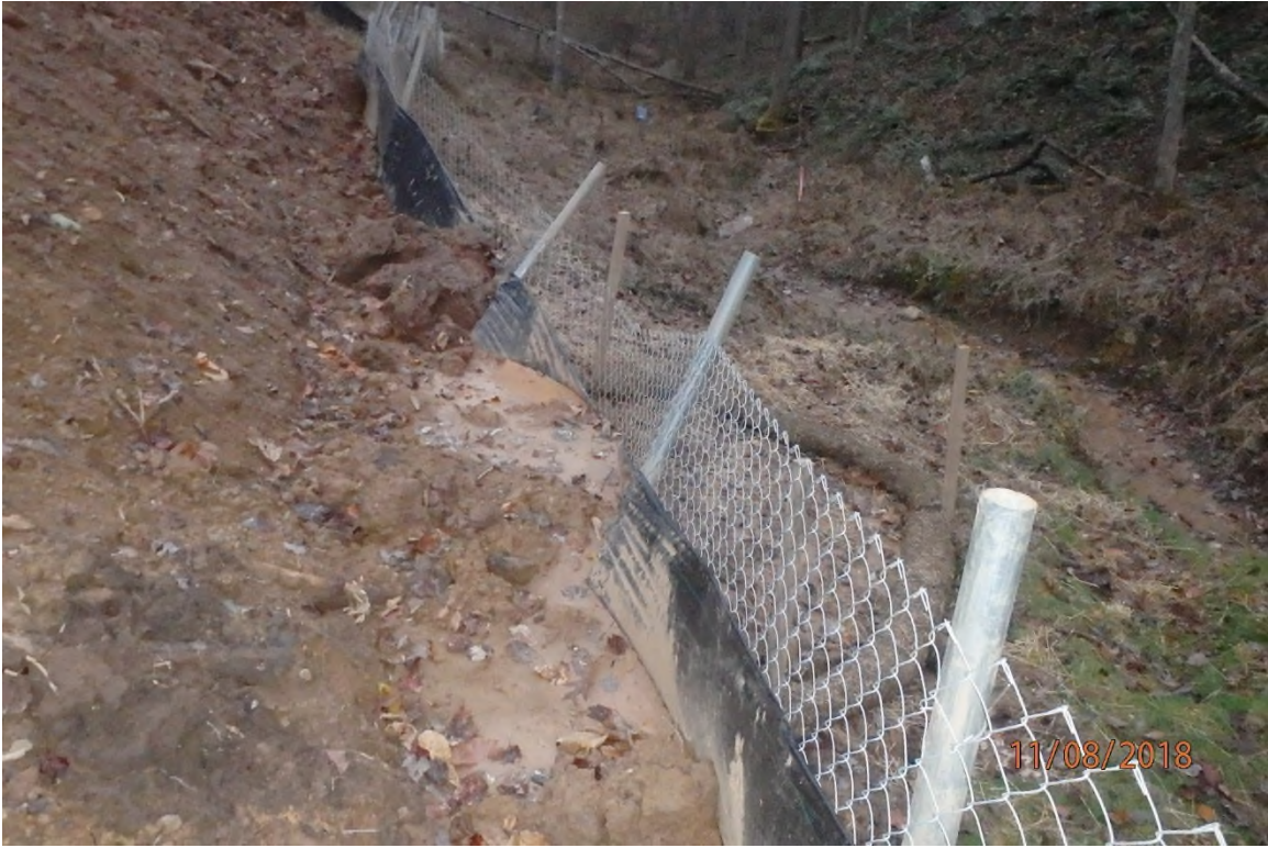
BMP in need of maintenance that caused offsite CNA deposits in UNT Sugar Run (SDOH008) (39°11.070' X 80°51.112').
