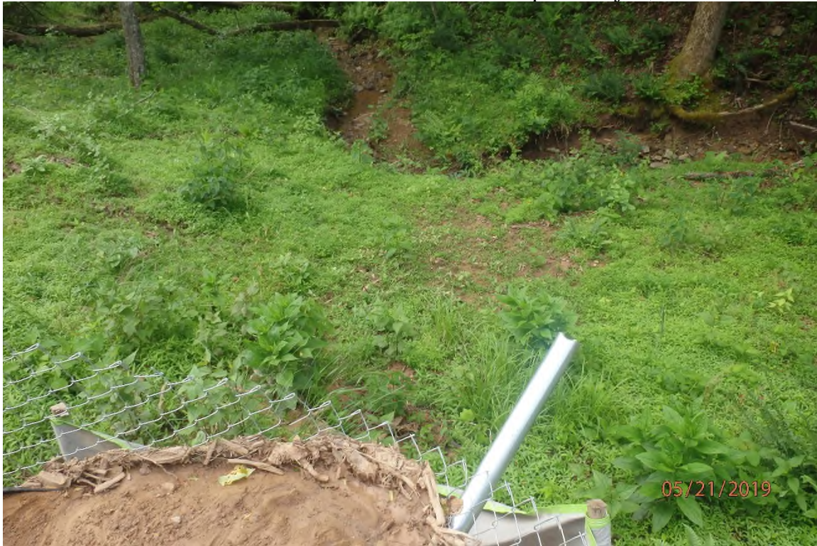
Unmaintained BMP in the UNT Sugar Run watershed and the sediment trail that leads to the receiving stream.
