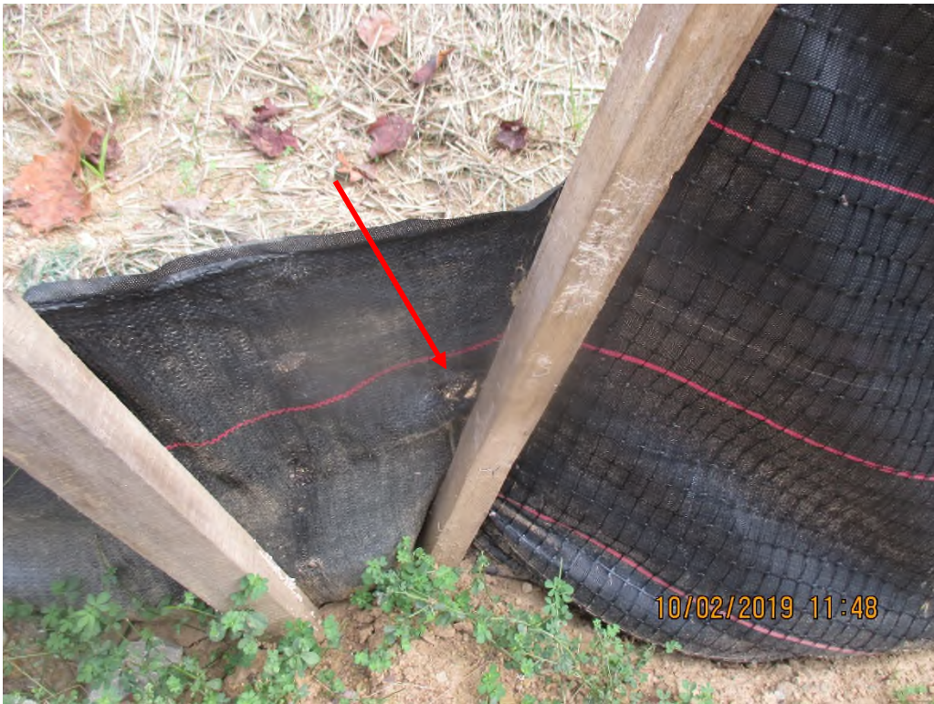
Perimeter controls along CR 22/1 near station No. 3380+84 with sediment deposits behind and past controls. Hole present in silt fence.
