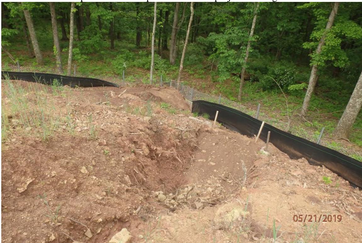
Improperly installed water bar in the Jims Run watershed. Water bar outlet discharges inside of the installed perimeter control and an appropriate outlet was not provided.
