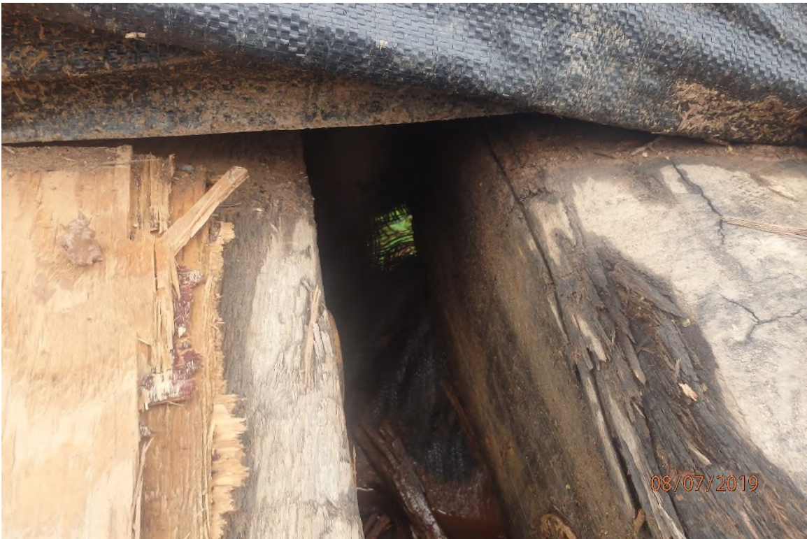
Installed timber mat equipment bridge at UNT Riggins Run (SDOG902) showing the need for maintenance.
