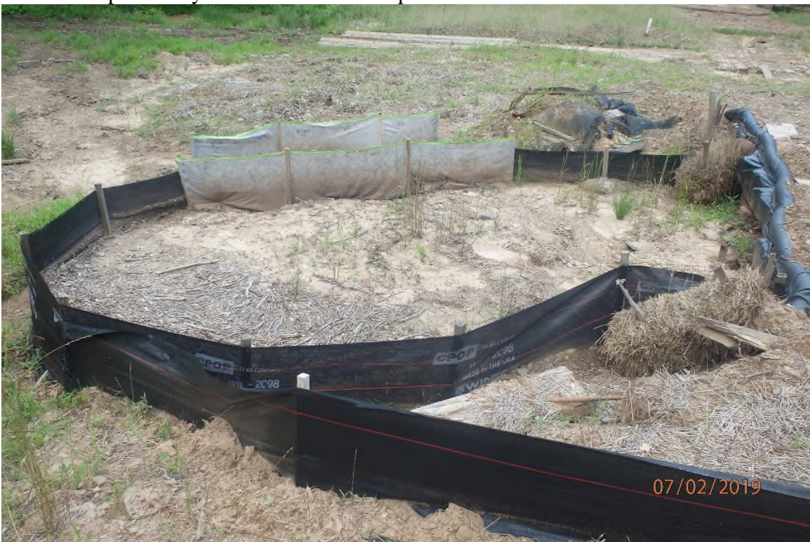
Project area adjacent to 2965+00 showing perimeter controls installed to protect the delineated UNT Left Fork of Arnolds Creek (SDOG057). The pictured accumulated instream sediment deposits originate from the previously documented CNA deposits in SDOG056 & SDOG057.
