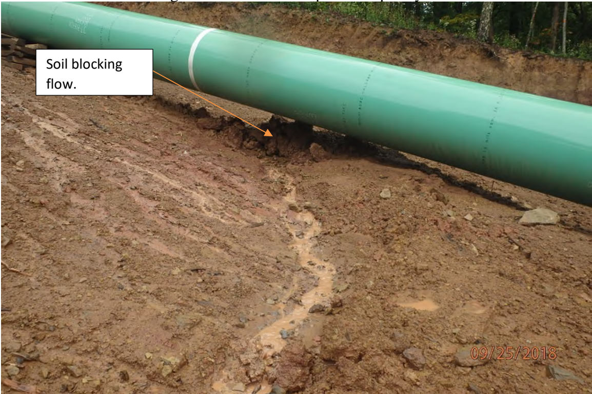
Poorly maintained water bar.
