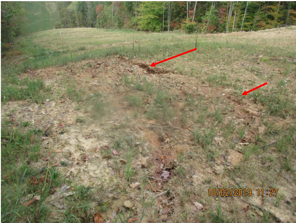
Gully erosion present between waterbars near station No. 3380+84. No waterbar outlet or perimeter controls observed.
