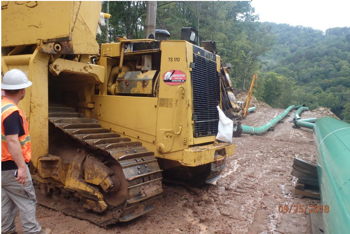
Piece of equipment that was leaking diesel fuel onto the ground.
