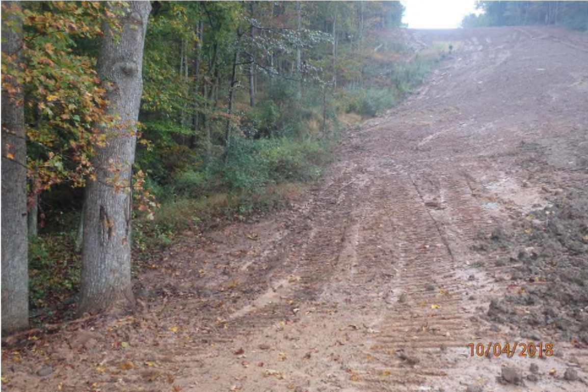
Project area near 2019+00 showing a lack of perimeter silt fence as indicated in the approved SWPPP.
