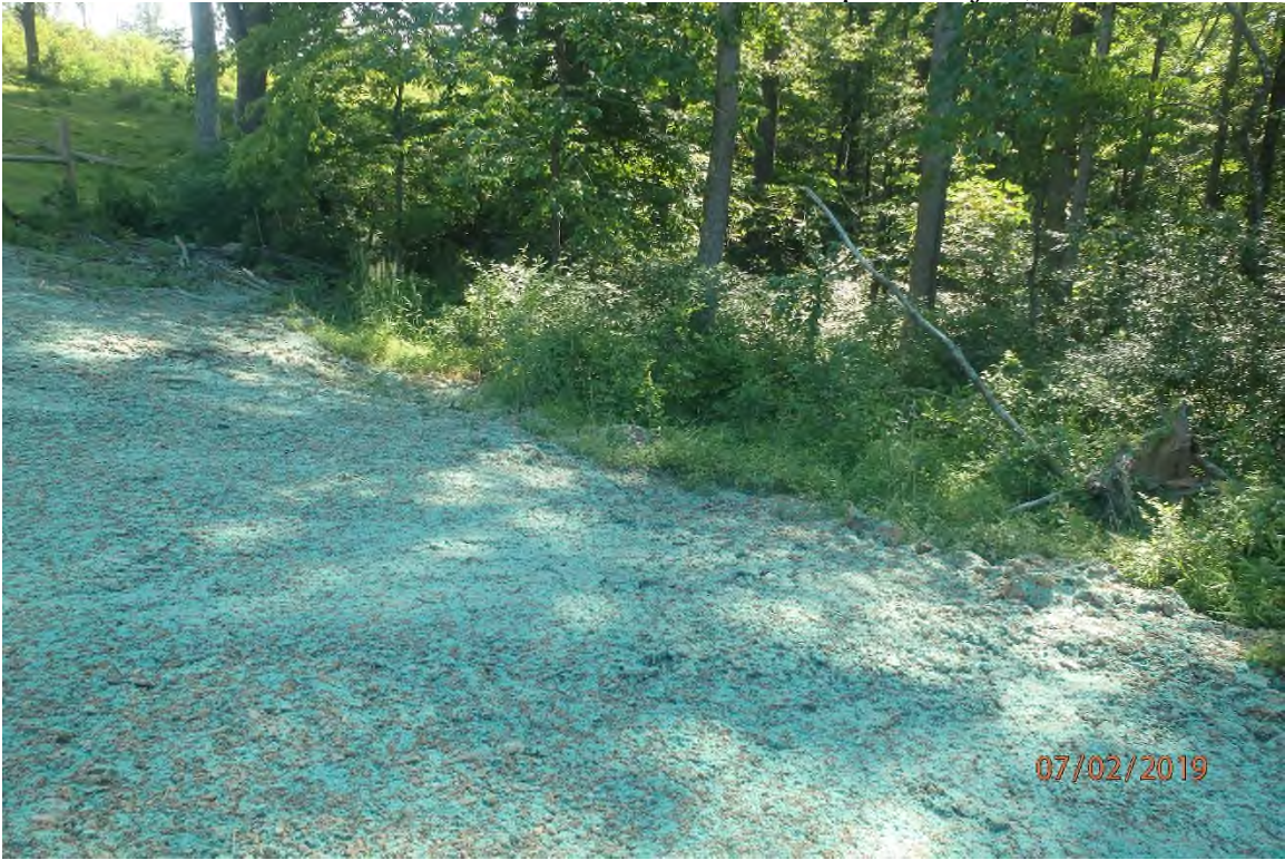
Area adjacent to 3314+00 where the approved SWPPP does not indicate the need for perimeter controls and the SWPPP has proved inadequate.
