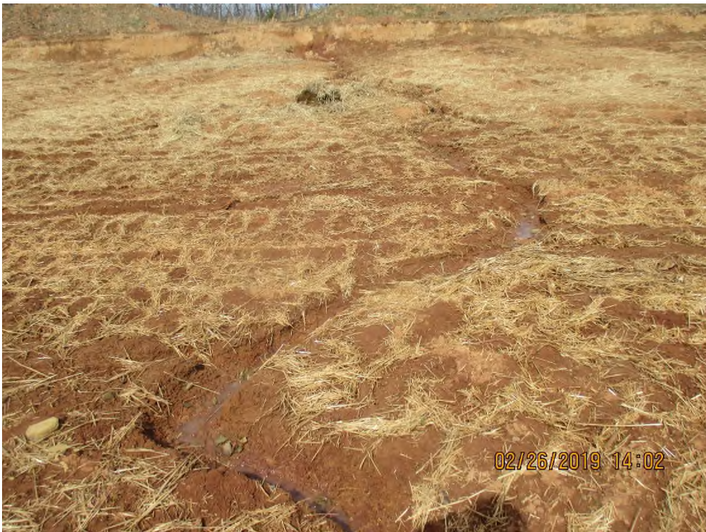
Near station #6620+00 (per SWPPP). Seep intersecting ROW and causing erosion.
