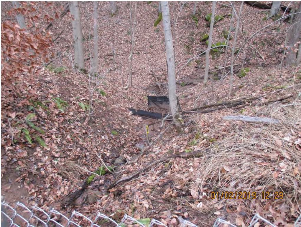
Discharge point (silt fence 23) on North slope that flows into UNT of Grasslick Creek.
