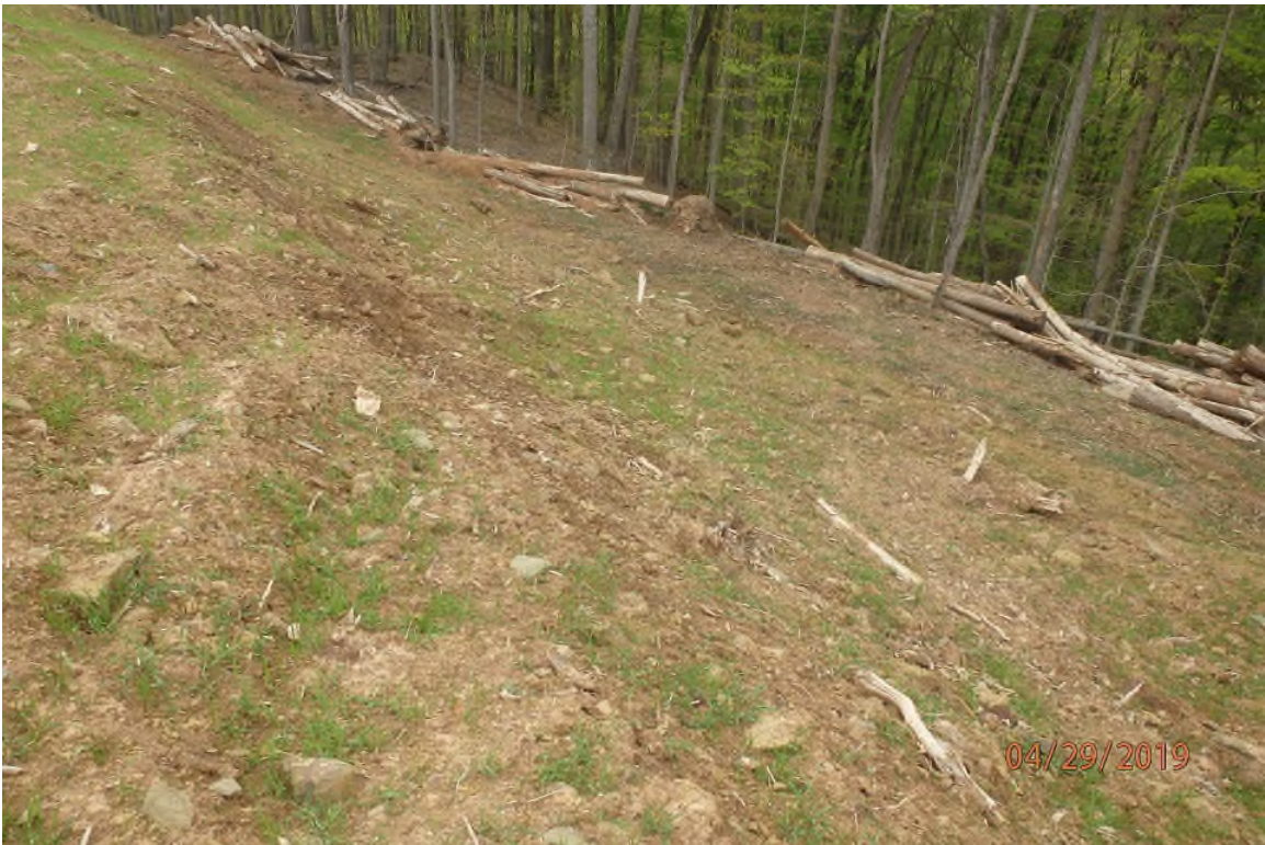
Project area adjacent to 2229+00 showing the need for perimeter controls where the approved SWPPP does not indicate the need.
