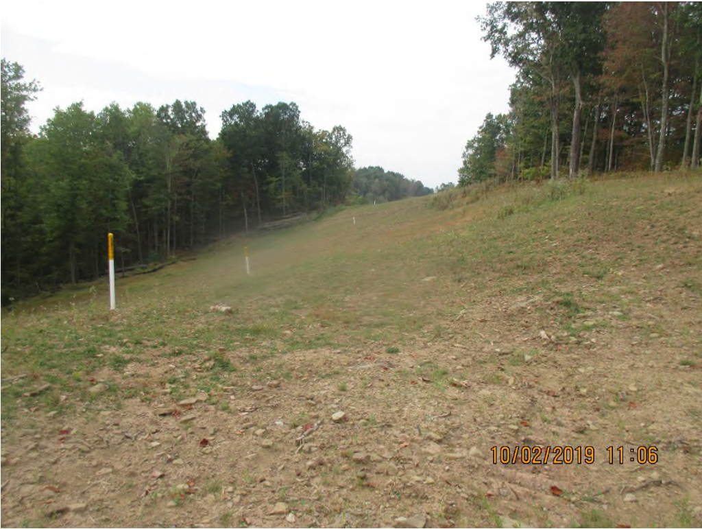
Standing near station No. 3368+00 facing south at MXP ROW.
