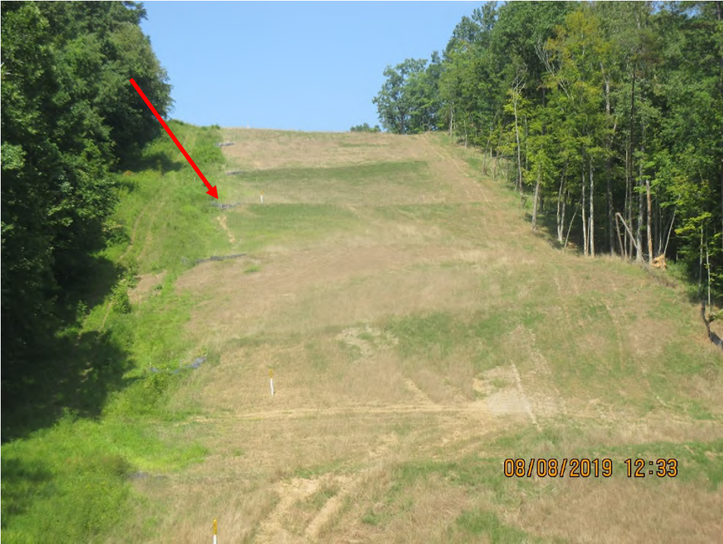
Adjacent slope facing North. Arrow depicts waterbar outlet control failure causing erosion on slope.
