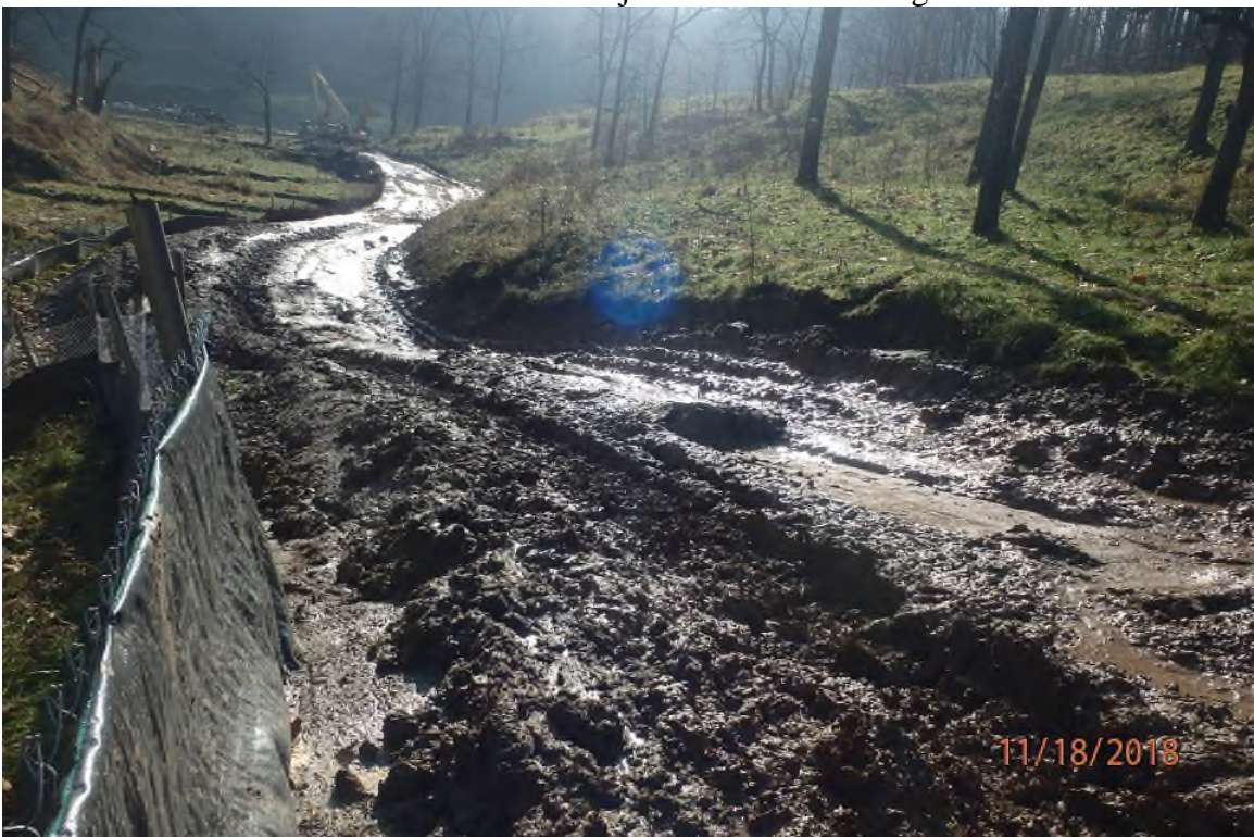
ARDO008.5 showing the lack of a graveled surface and the lack of adequate drainage.
