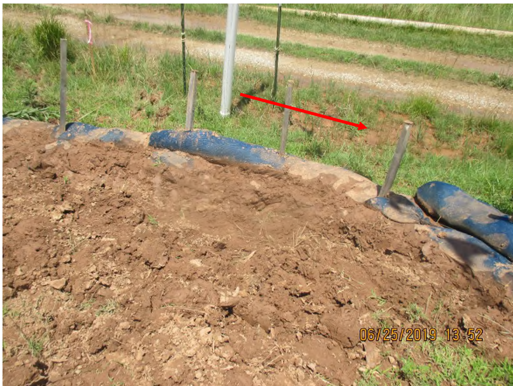
Middle Fork Road Crossing at station No. 5643+50 above stream SRUA 005 facing perimeter controls downslope of where Waterbars were eroded. Controls not maintained, with sediment deposits past LOD.
