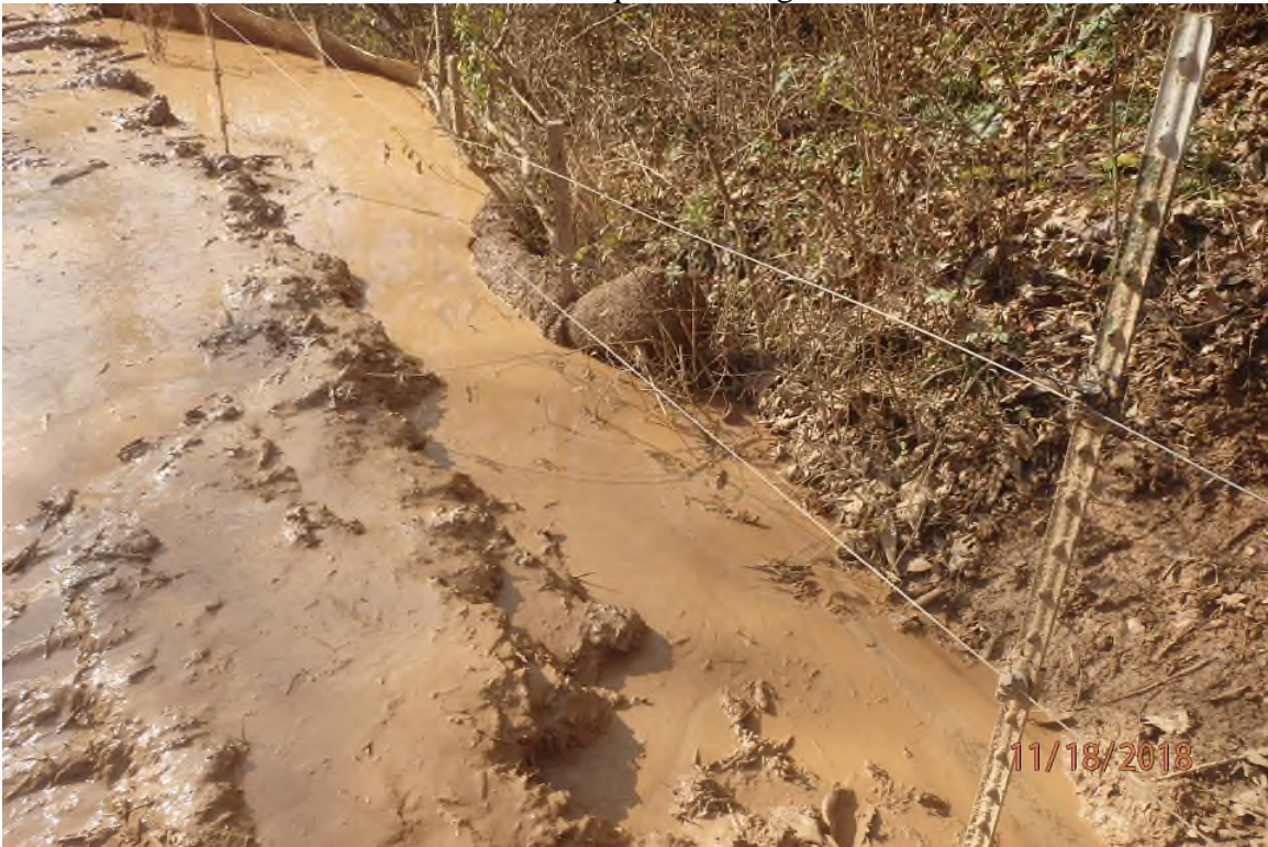
ARDO009.3 showing stormwater in an upslope ditch that is overflowing onto the road surface due to the lack of adequate drainage.
