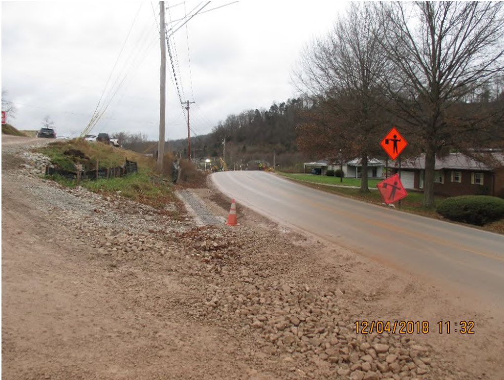
Facing South on route 21 at compressor station entrance.
