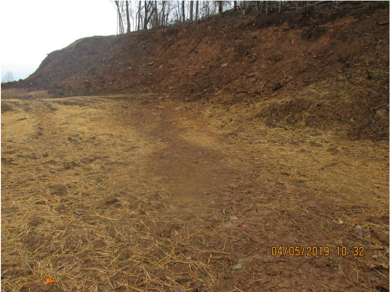
Downslope of slip occurring above ROW at station #6792+40. Scouring of temporary stabilization occurring.
