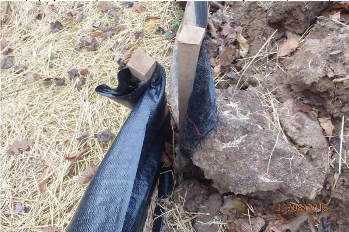
Improperly installed perimeter control adjacent to UNT Taylor Drain (SDOH012).
