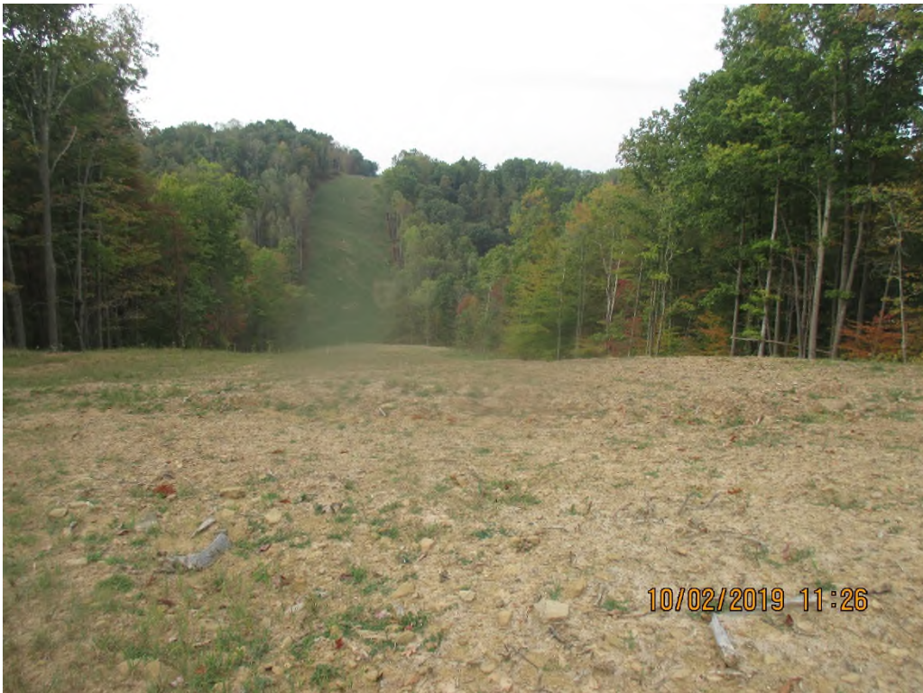
Facing south toward Bear Run and (CR 22/1) near station No. 3380+84. ROW not stabilized.
