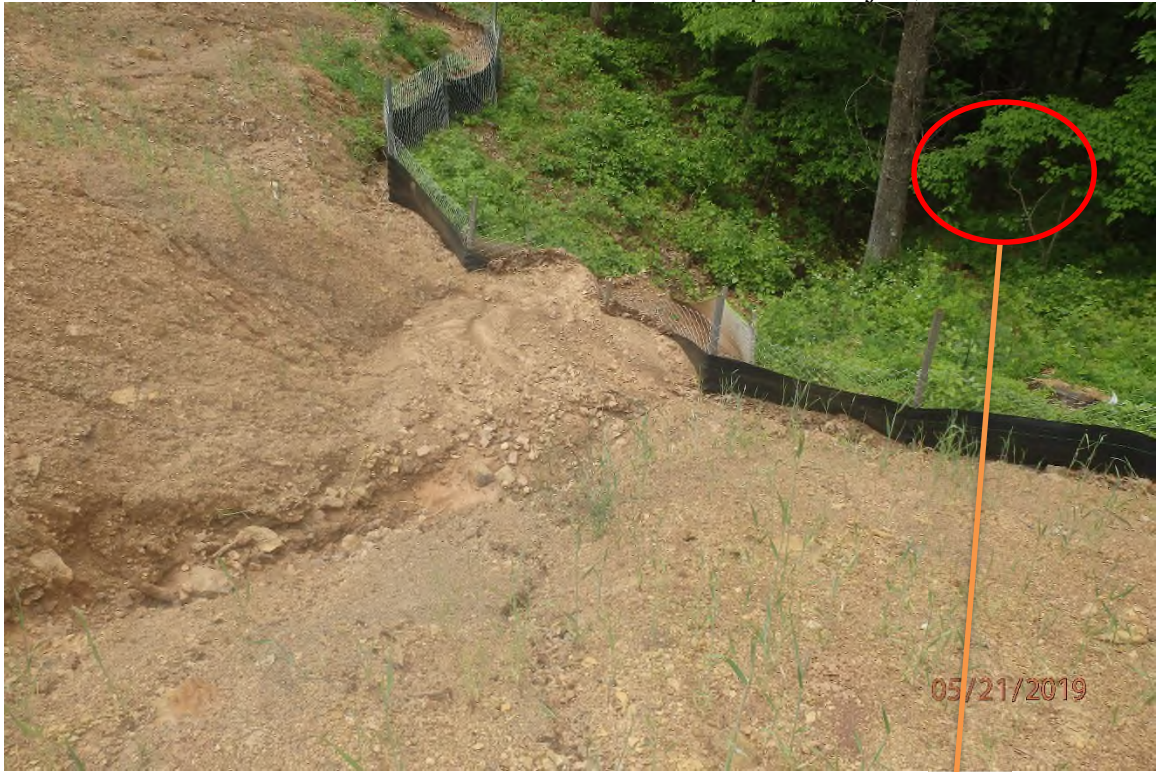
Unmaintained BMP in the UNT Trap Run watershed.
