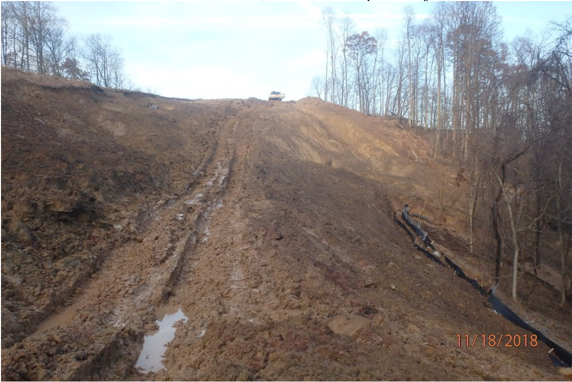
Overview of slip near 2822+00.
