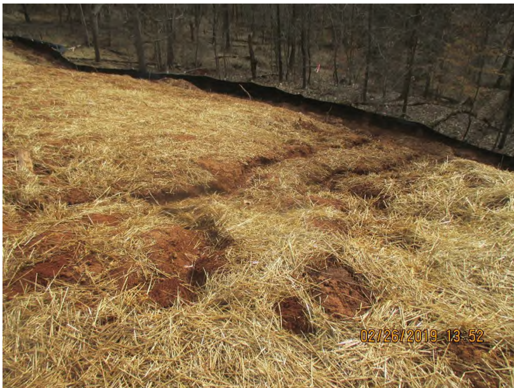
Run-on from adjacent field flowing across ROW and creating rill/gully erosion on slope near station #6742+60.
