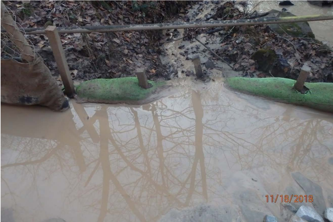
BMPS adjacent to Georgescamp Run that are overwhelmed due to the lack of drainage on the access road, causing sediment laden stormwater to bypass the devices.
