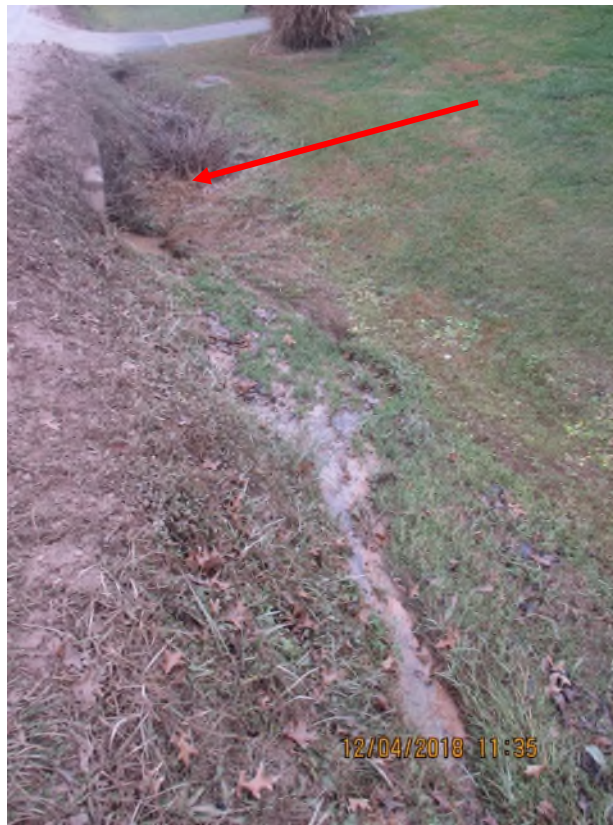
Sediment laden water entering ephemeral stream that crosses under route 21. Arrow shows culvert that crosses under Route 21.
