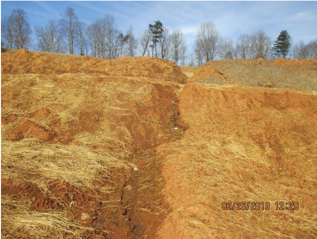
Seep causing gully erosion on slope near station #6781+00, flowing into waterbar.
