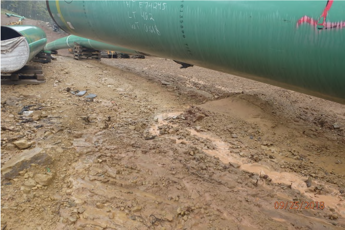
Concentrated flow being directed over fill slope due to poorly maintained water bars.
