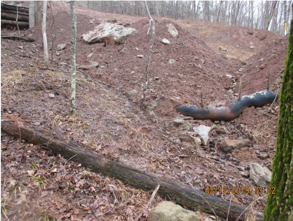
Waterbar outlet downslope of log pile near station 5400+00.
