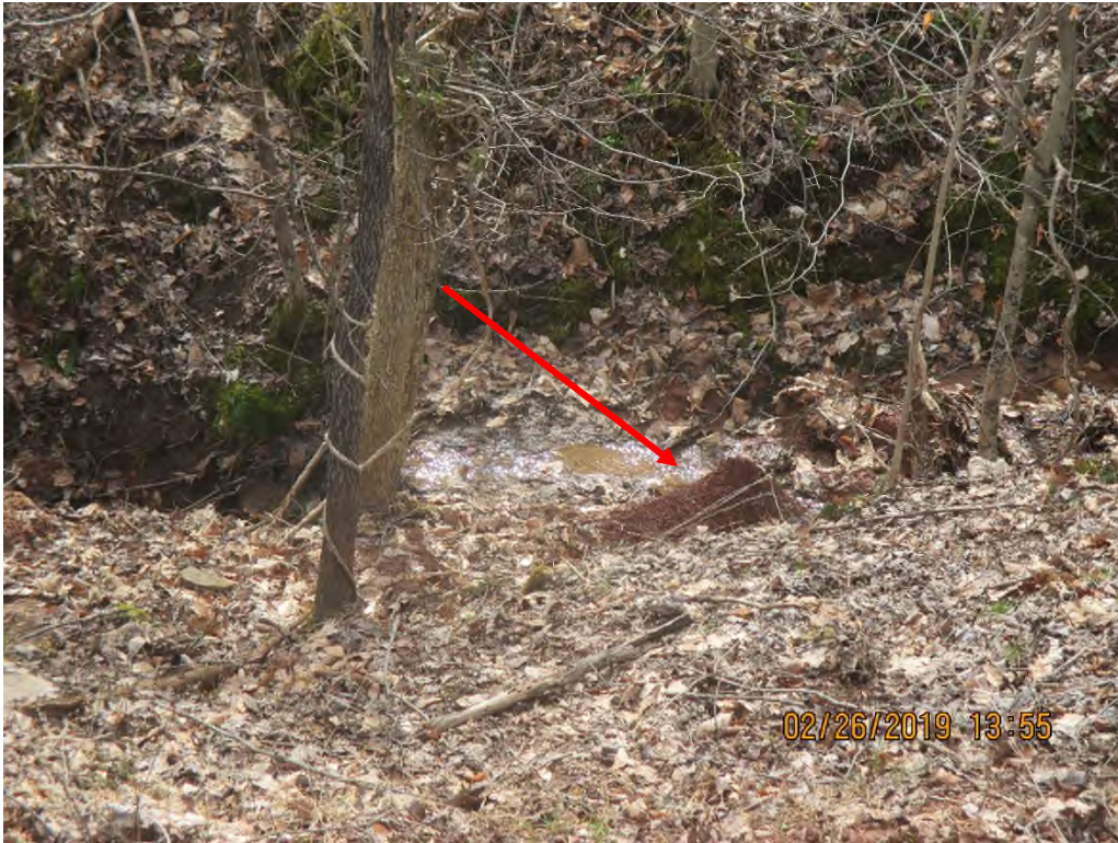
Near station #6742+60. Sediment being deposited past perimeter control and present in stream SJAA-040
