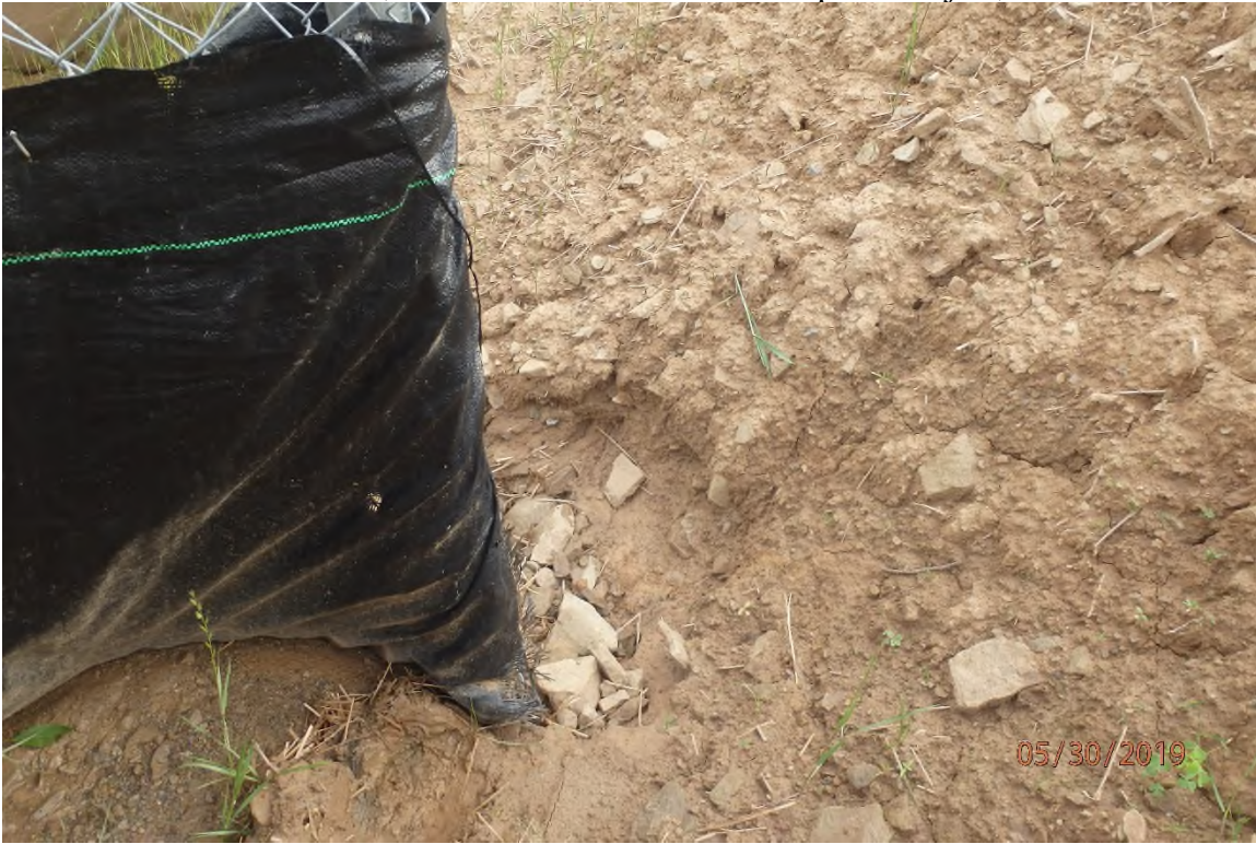
Water bar terminus adjacent to 2591+00 showing the area where concentrated flow is directed over the unprotected fill slope.
