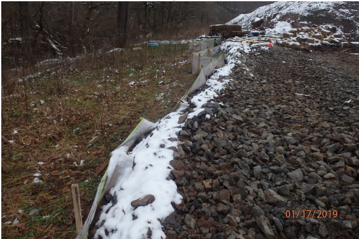
Perimeter silt fence in need of maintenance.
