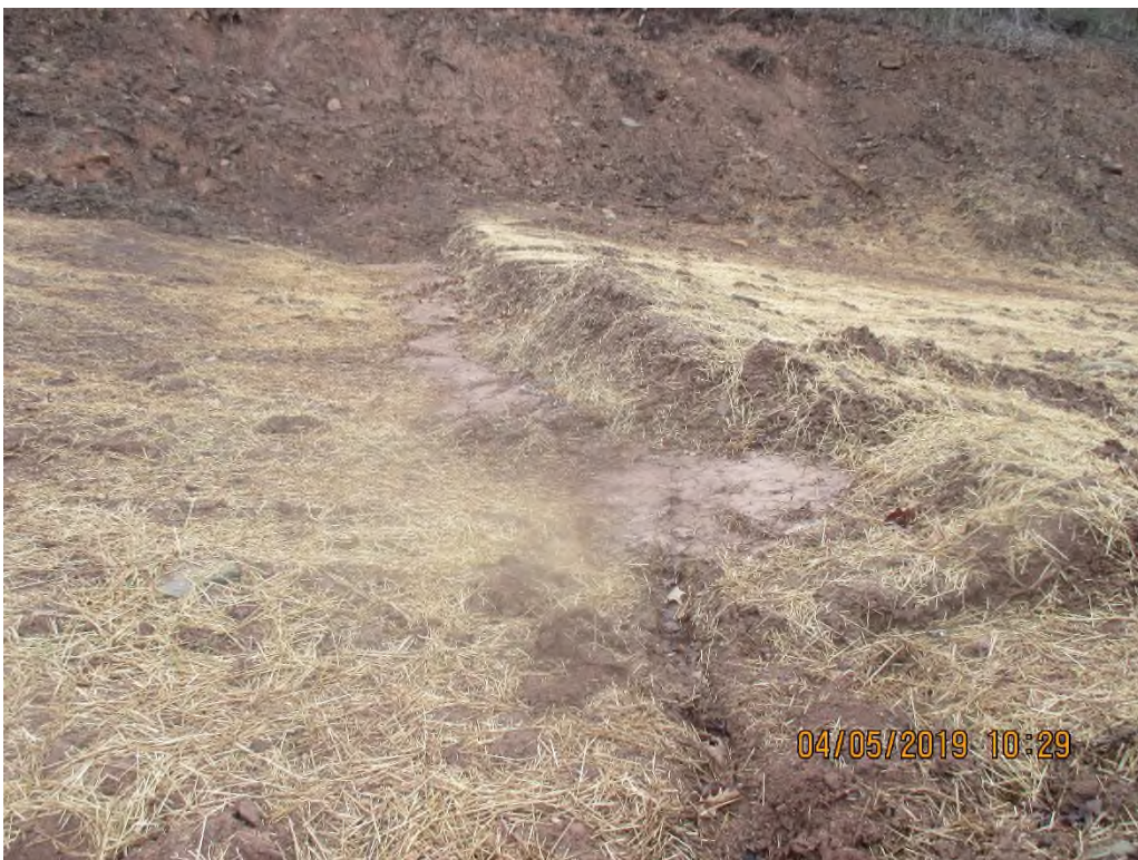
Waterbar with ponding present. Sediment from topsoil pile slipping into waterbar near station #6795+55.
