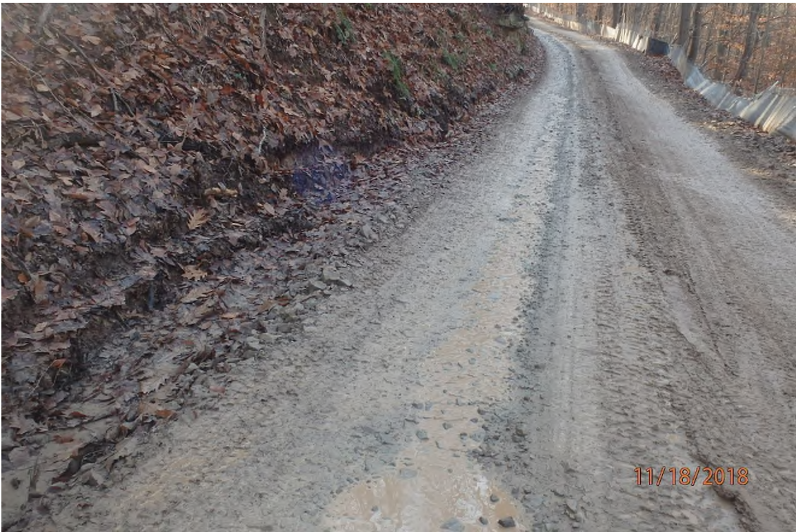
ARDO008.2 showing stormwater flowing downslope in ruts on the road surface due to the lack of adequate drainage.
