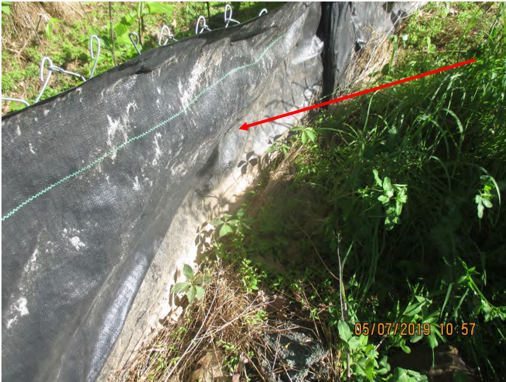
Super silt fence installed at base of North slope below compressor station pad. Arrow depicts hole in fence.
