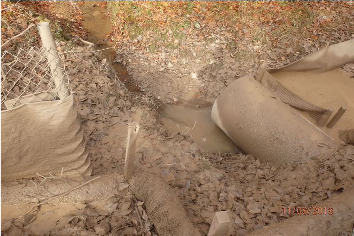
ARDO008.2 showing improperly installed controls and failure to follow SWPPP, resulting in CNA.
