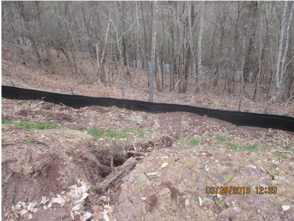
Erosion on fill slope with sediment being deposited against perimeter controls near station #5162+60
