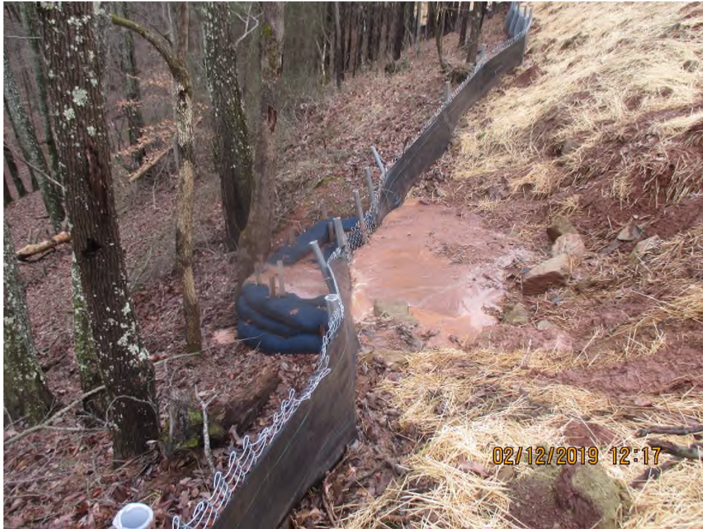
Perimeter control at station #5359+00
