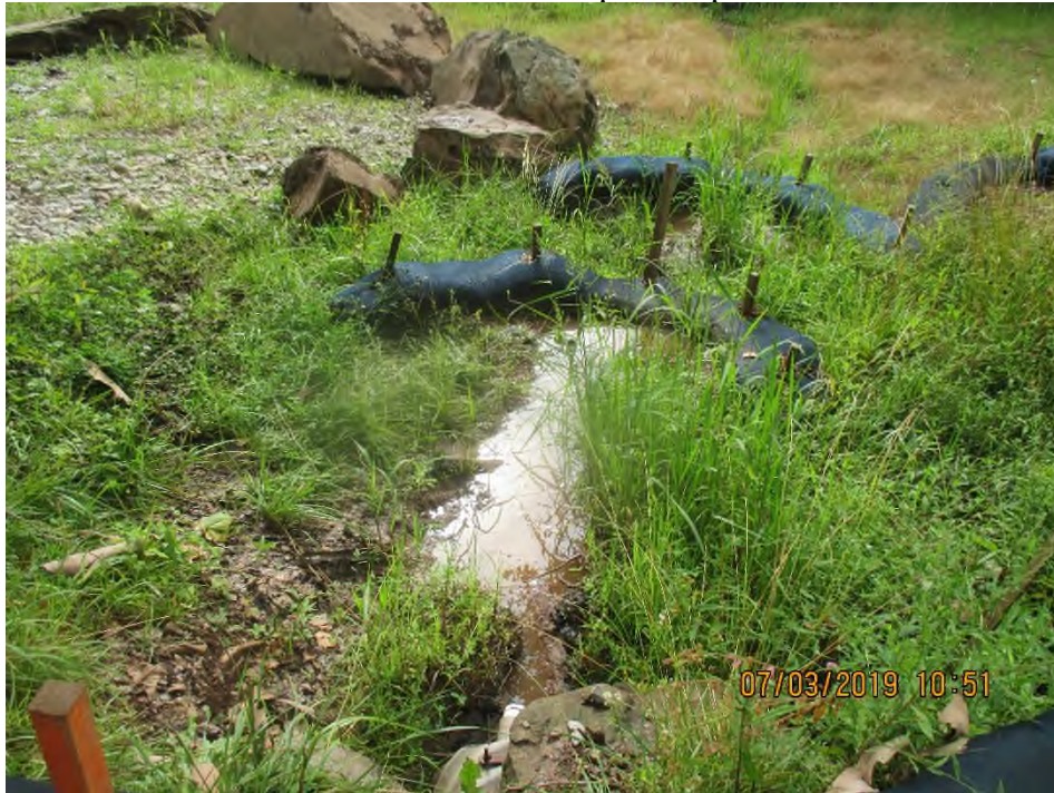
Second culvert outlet that covers under Sulu road and was receiving sediment laden water from ditch line impacted by slip.
