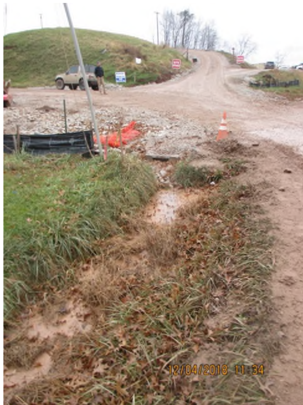
Facing toward drop inlet and sediment trap that was overflowing into ditch.
