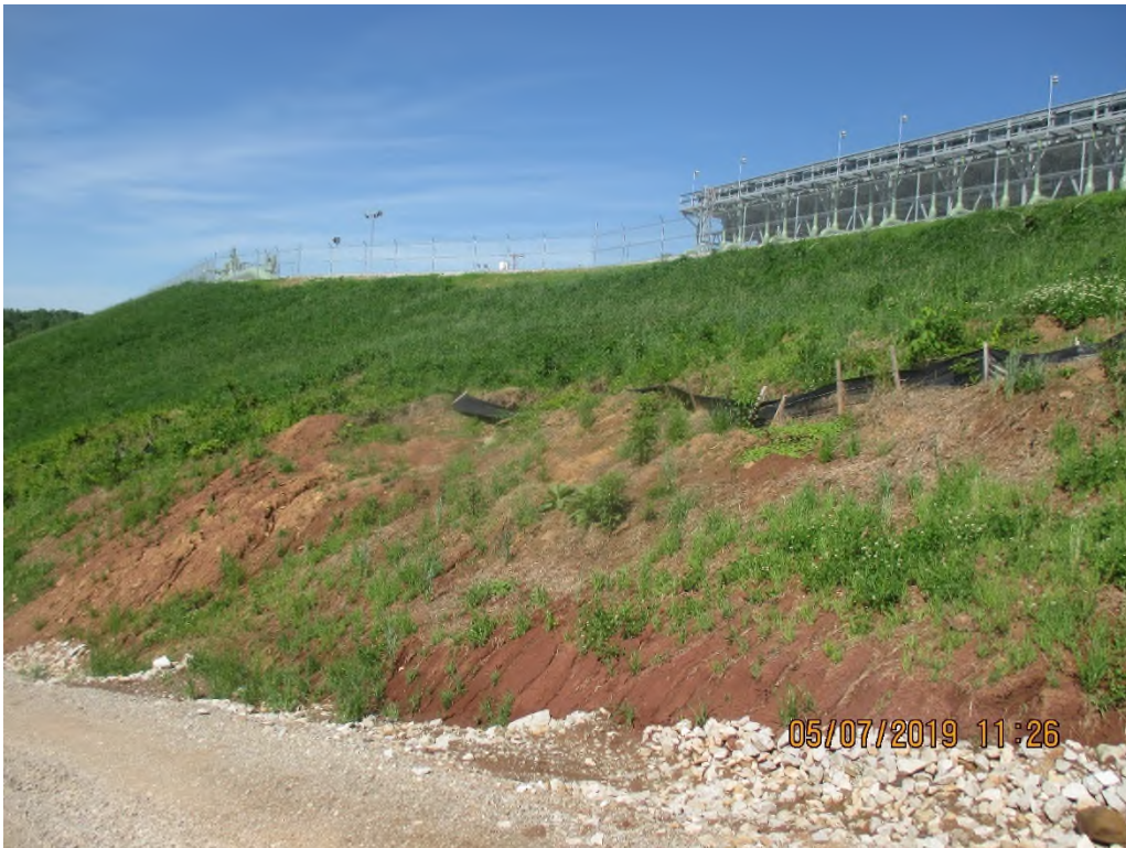
Ditch line along access road below erosion that was taking place along south slope of compressor station pad. Unstabilized portion of slope above ditch and culvert inlet.
