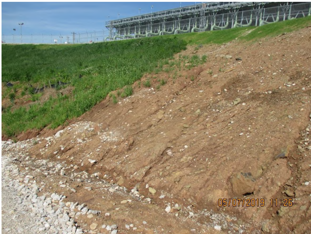
Erosion on south slope above ditch that conveys toward perimeter of project.
