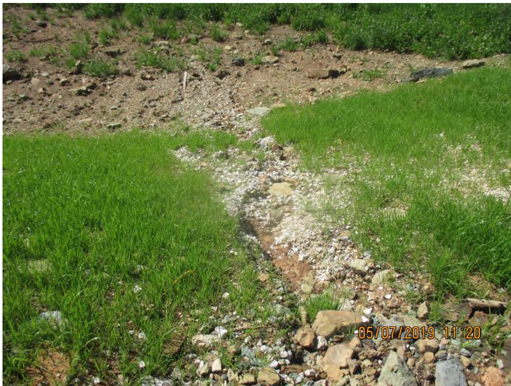
Erosion occurring adjacent to diversion swale outlet. Run-off from pad eroding fill slope on south side of pad.
