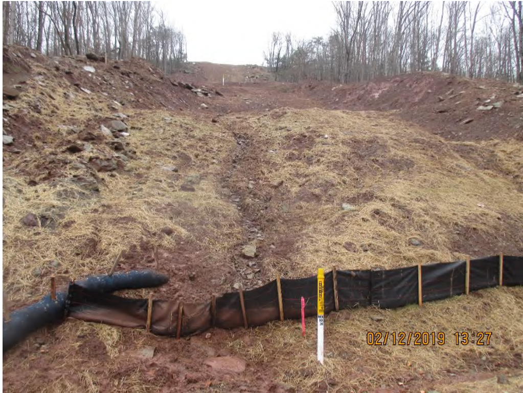
Facing North upslope at Munchausen Road crossing station #5407+07
