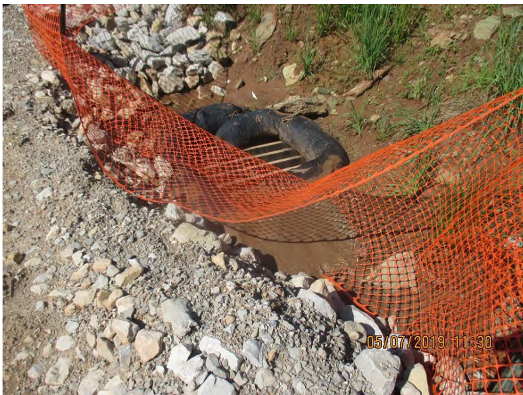
Culvert inlet on South side of compressor station slope conveying under access road. Sediment deposits present in drop inlet.
