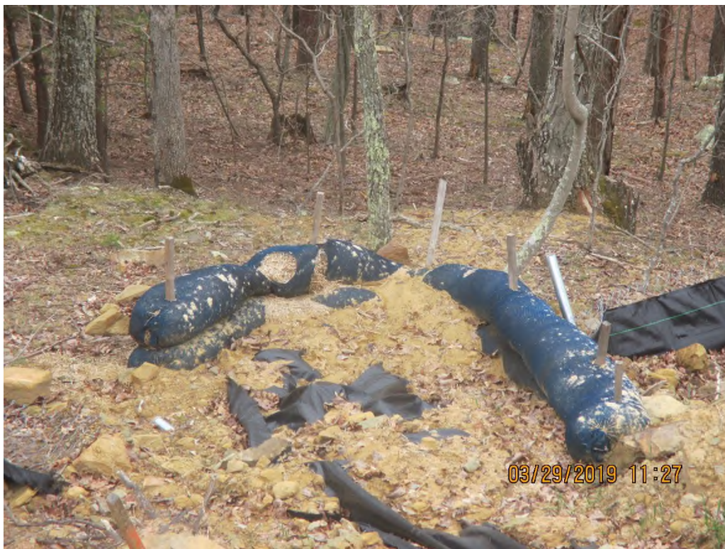
Perimeter controls being overwhelmed with sediment downslope of waterbar terminus near station #5148+00. Sediment deposits were present past controls and LOD.
