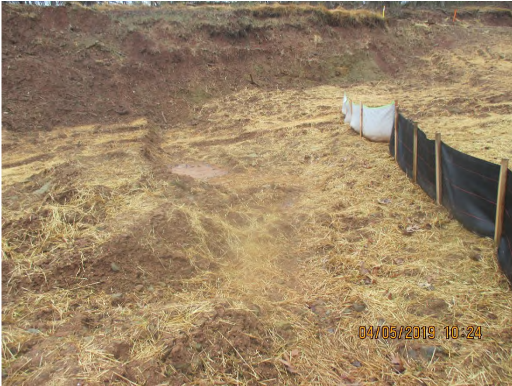
Waterbar near station #6781+55. Ponding present in Waterbar.
