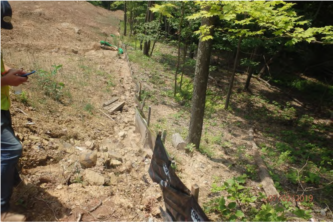
Water bars that do not extend past the installed perimeter controls in the UNT Left Fork of Arnolds Creek watershed showing fill slope erosion along the silt fence trench.
