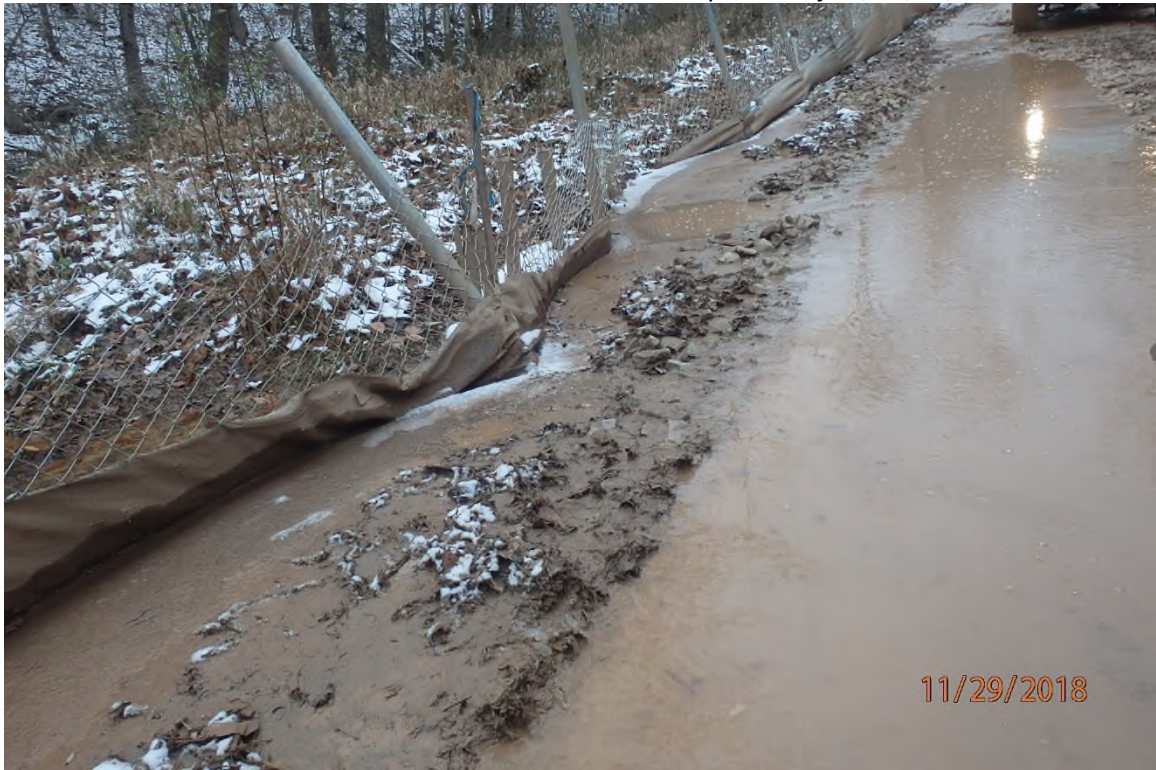
Unmaintained perimeter control on ARDO009.1.
