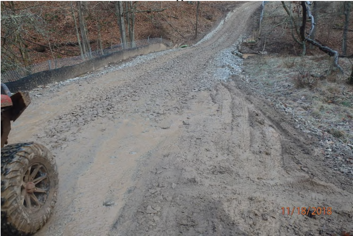
ARDO008.2 showing stormwater flow traveling downslope in ruts to the adjacent receiving stream due to the lack of drainage as indicated in the approved SWPPP.
