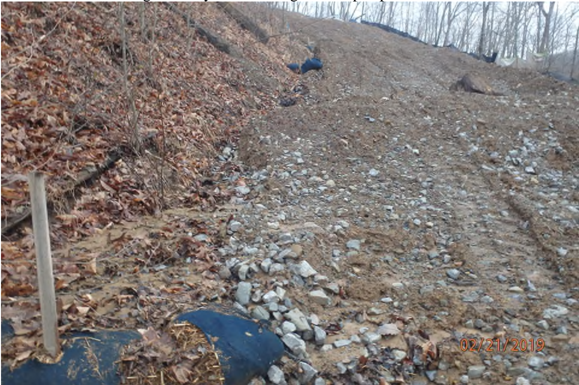
Installed ditch checks and water bars on ARDO002.8 that are overwhelmed by stormwater flow resulting from the lack of installed cross drains/culverts as indicated in the approved SWPPP.
