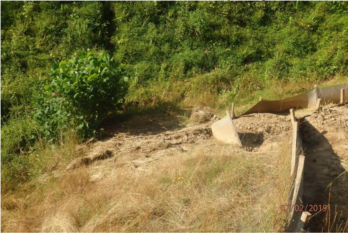
Unmaintained perimeter control in the Sugar Run watershed that is placing sediment into onsite ephemeral UNT Sugar Run.
