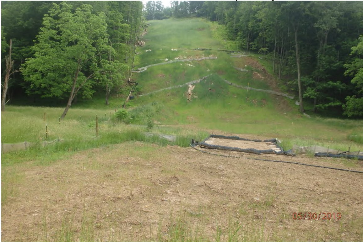
Project area adjacent to 2452+14 showing improperly installed water bars.
