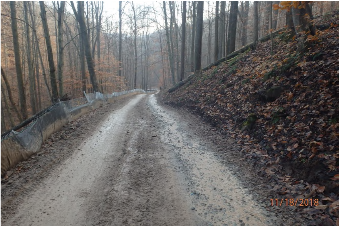
ARDO008.2 showing stormwater flow traveling downslope in ruts due to the lack of drainage as indicated in the approved SWPPP.
