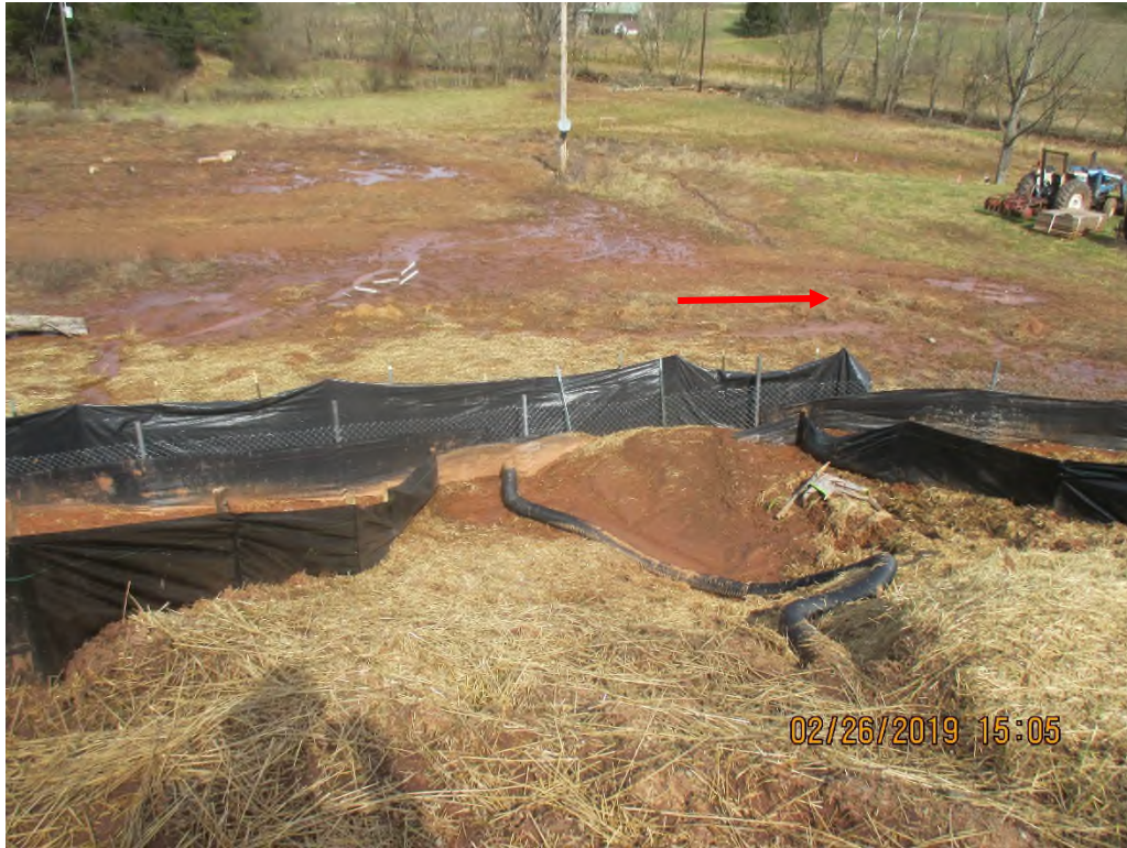
Downslope of station #6702+30. Slope drain outlet terminating into perimeter controls. Culvert installed under additional workspace. No controls installed in this area.
