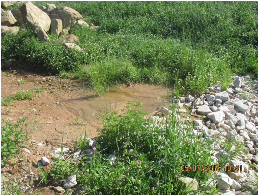
Sediment present above smaller rock in diversion.
