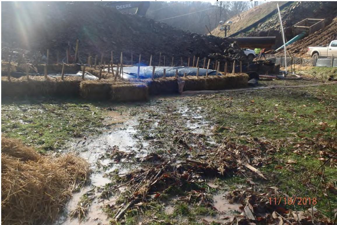
Dewatering bag associated with pipe trench dewatering adjacent to the SDOG055 stream crossing.
