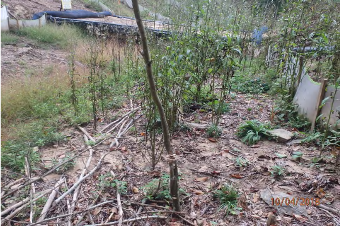
Sediment trail leading to the receiving stream as a result of the previously pictured improperly installed water bars and associated fill slope erosion near SDOI008.
