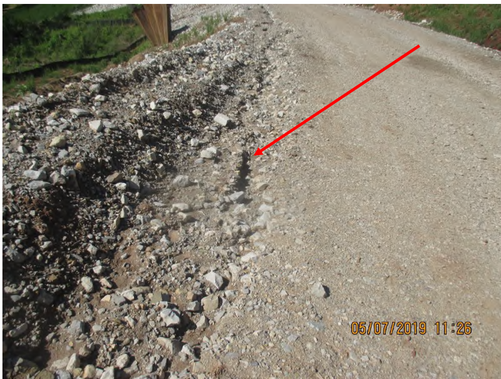
Erosion present on access road above culvert crossing.
