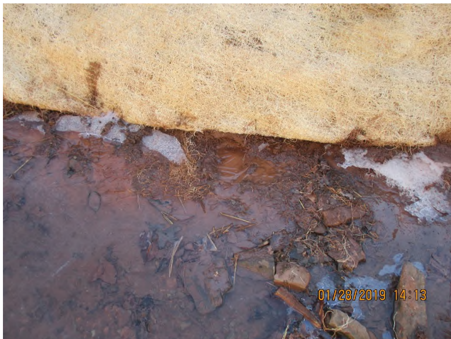
Area where erosion control blankets were added at edge of stream bank.
