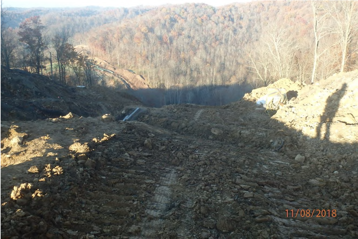
Improperly installed water bars in the Bluestone Creek watershed.
