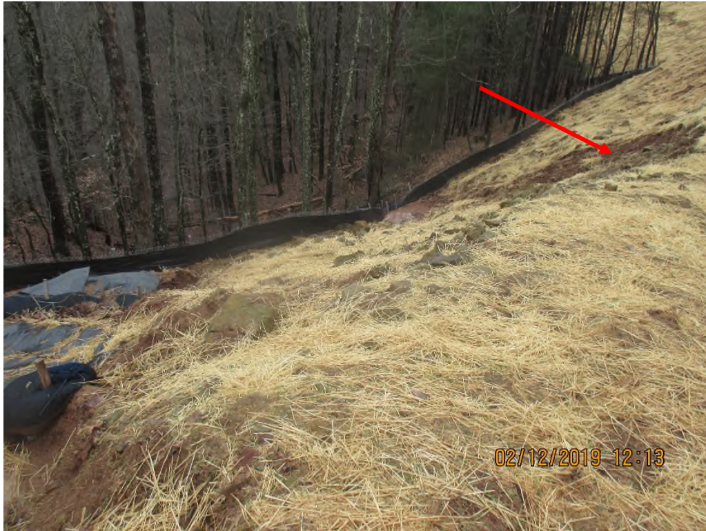
Waterbar terminus leading to perimeter control. Slope eroding above control.
