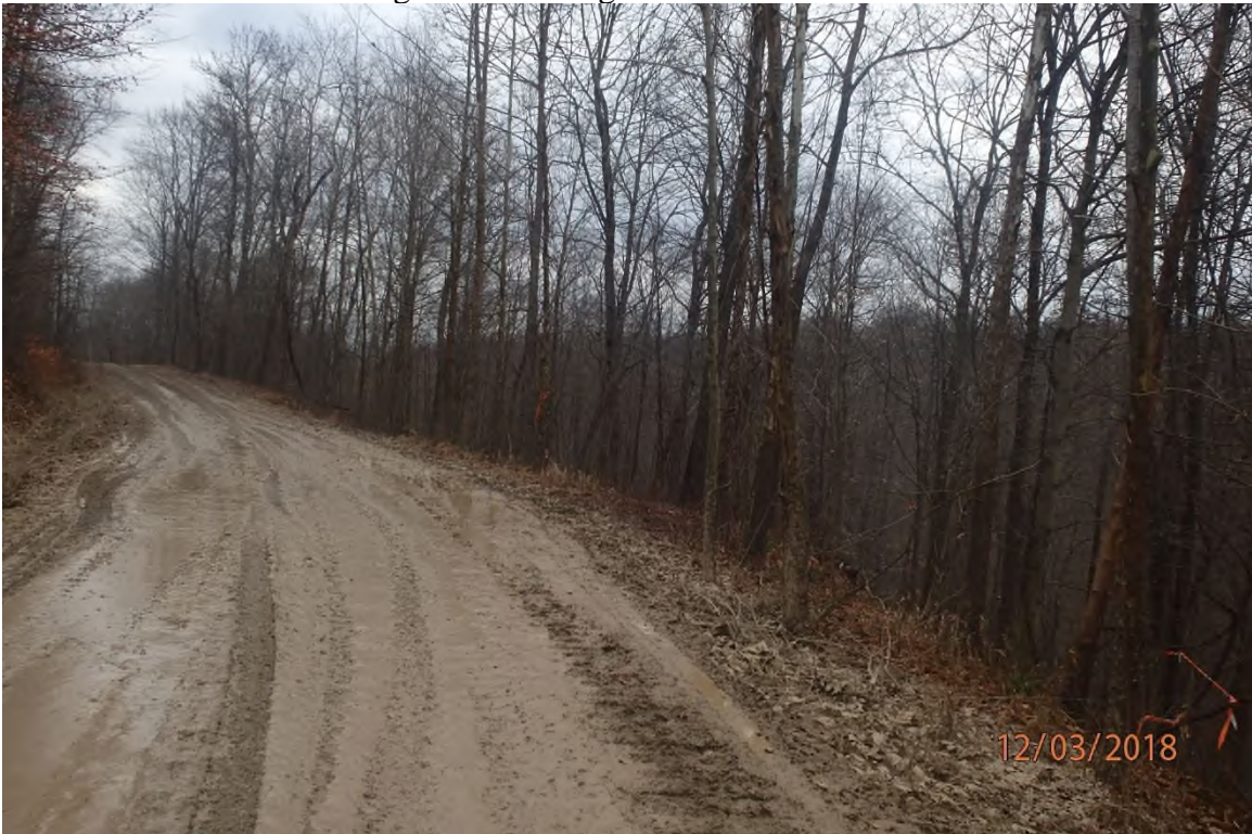
ARDO007.6 showing the lack of a graveled surface and the lack of BMPs.
