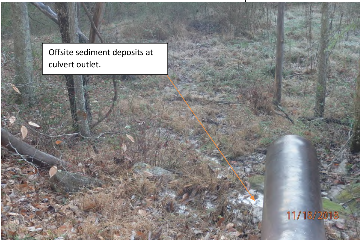
Unmaintained BMP and associated offsite sediment deposits on ARDO008.2.
