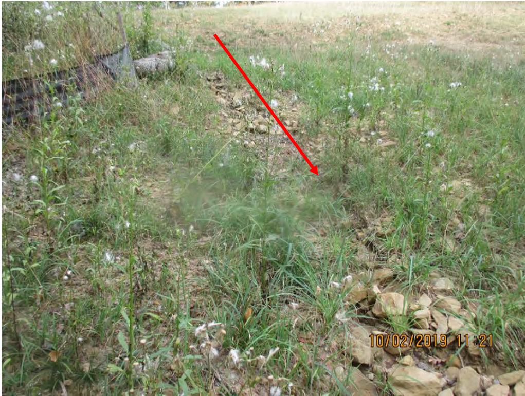
Waterbar terminating into perimeter controls near Station No. 3368+00 causing erosion downslope of controls. Arrow depicts gully erosion on slope.
