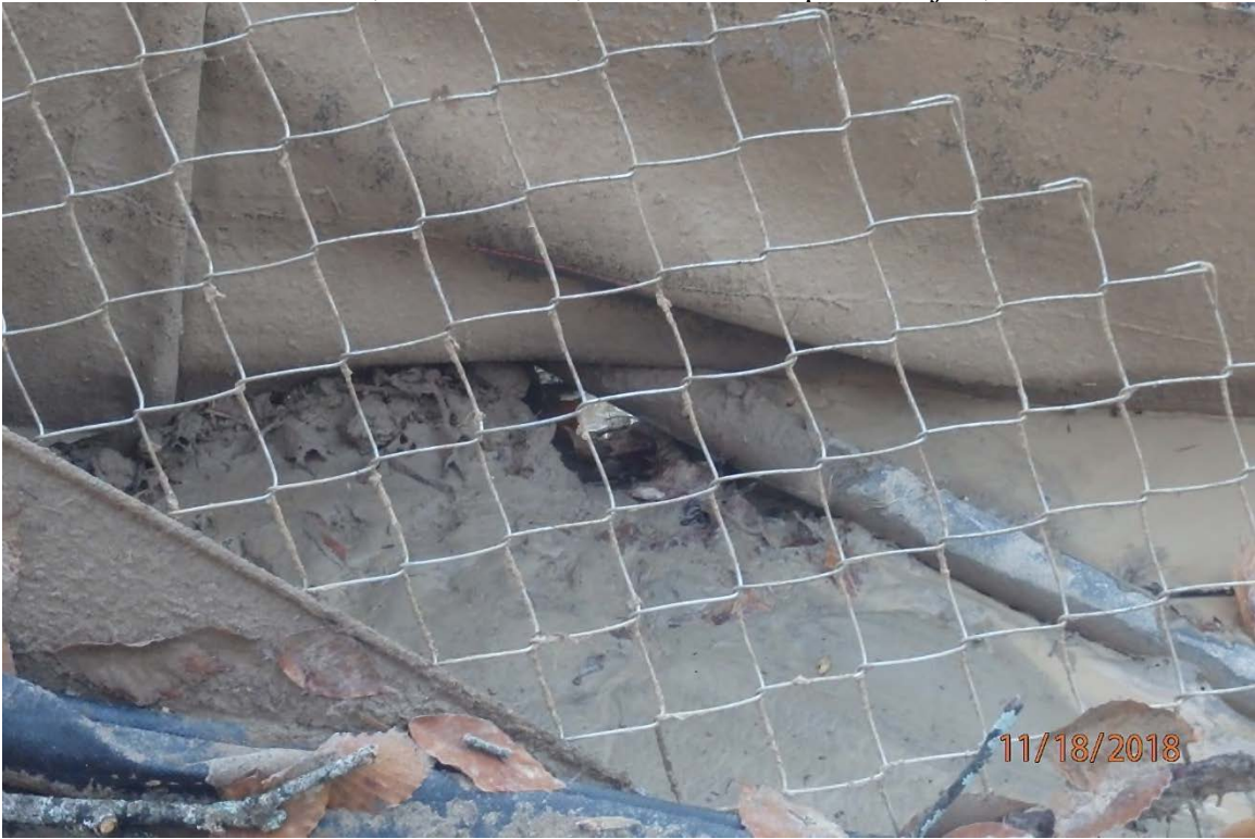
Unmaintained perimeter control and associated offsite sediment deposits on ARDO008.2.
