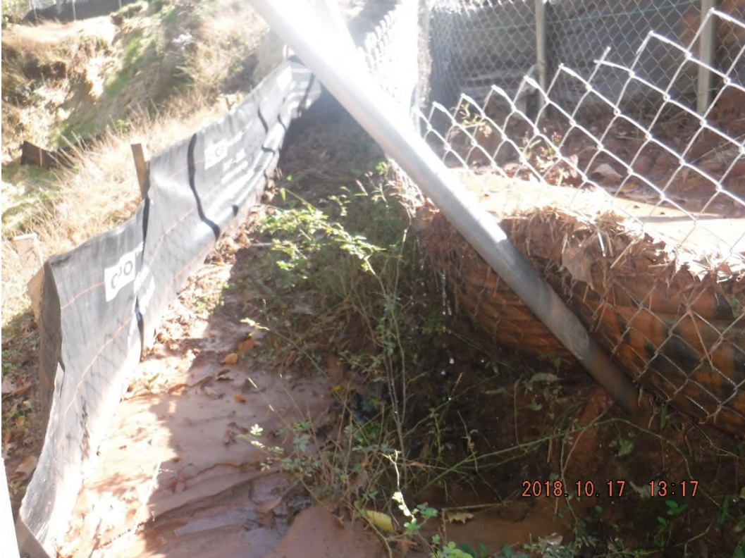
Sediment overtopping silt fence.
