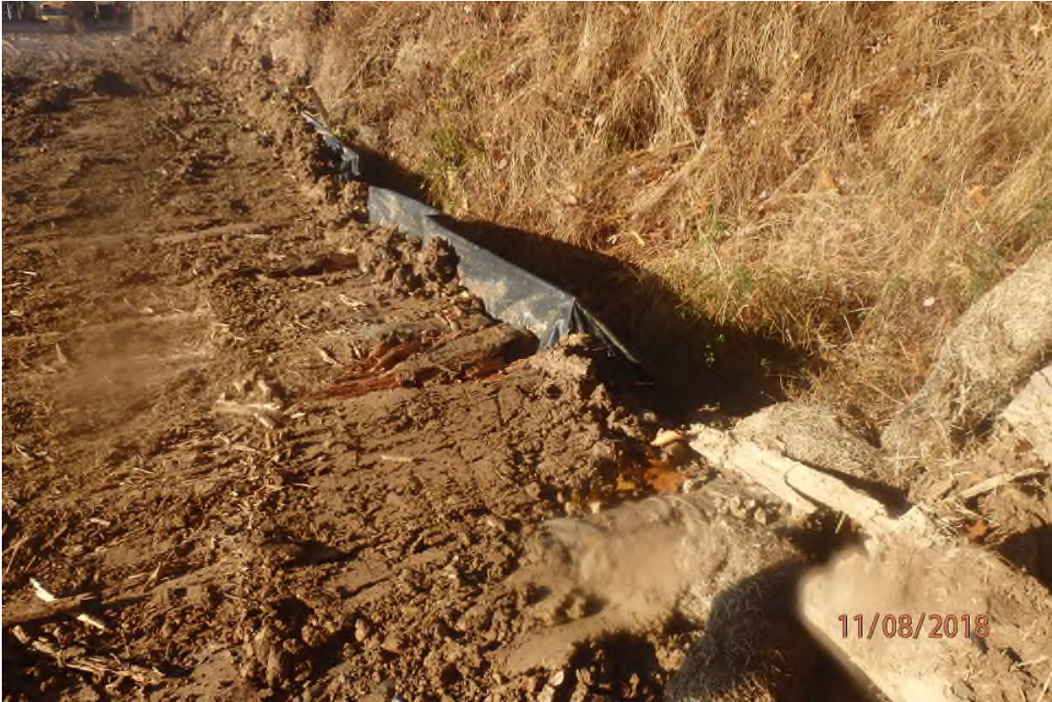
Unmaintained equipment bridge BMP in the Bluestone Creek watershed (SDOG543).
