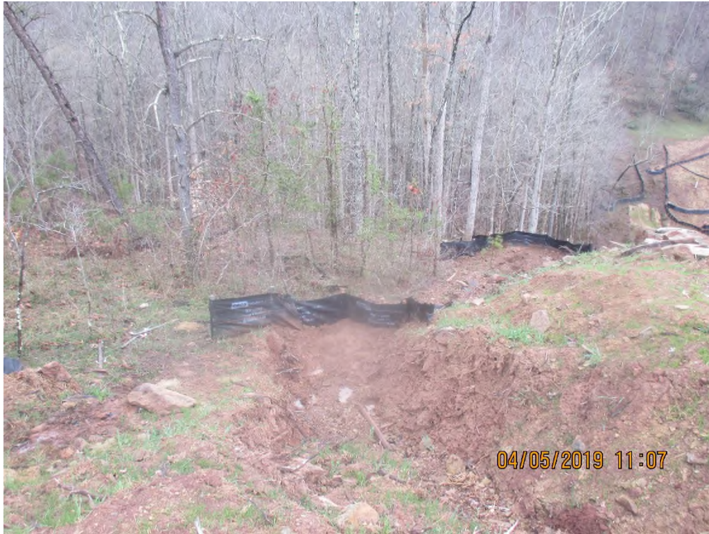
Waterbar terminating onto slope. Downslope of terminus facing controls along perimeter above stream SJAG-316.
