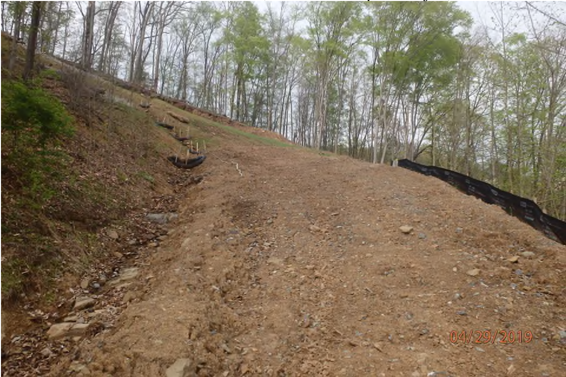
AR -17 showing the need for maintenance to the stabilized road surface and the upslope ditch.
