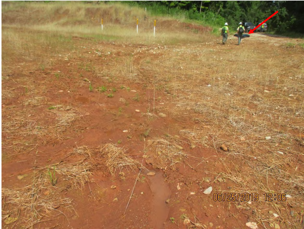
Saturated section of ROW where Access Road ARWI 024 was coming onto MXP ROW at station No. 5372+00. Arrow depicts ditch line on access road that was conveying run-on onto ROW.
