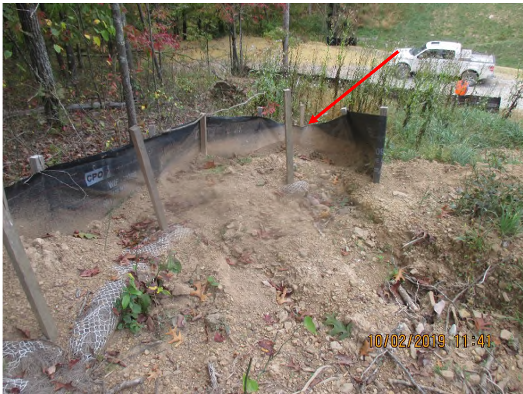
Standing above CR 22/1 facing South. A previous NOV was issued due to failures in this area. Waterbar outlet controls were not maintained, and there was evidence of sediment laden water overtopping controls.
