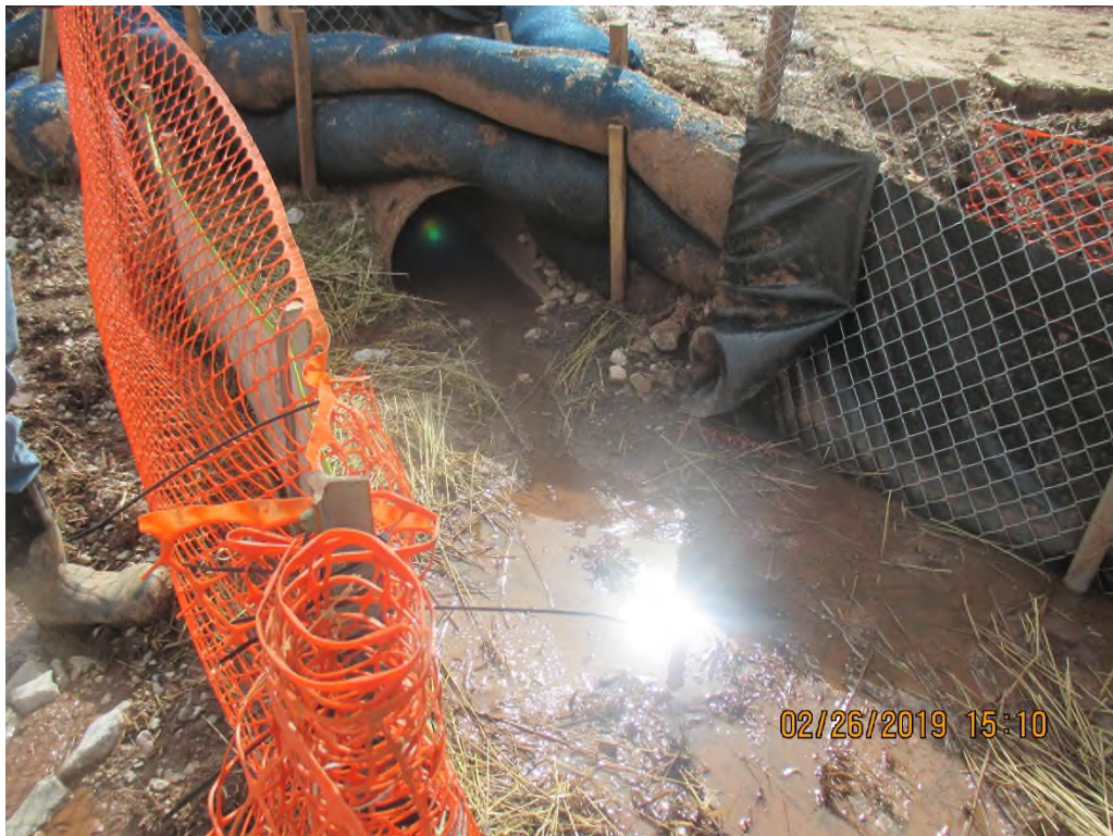
SJAG-346 facing upslope at station #6702+30. Sediment present in stream.
