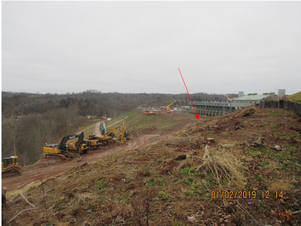
View of South side of project. Slope not protected near compressor station.
