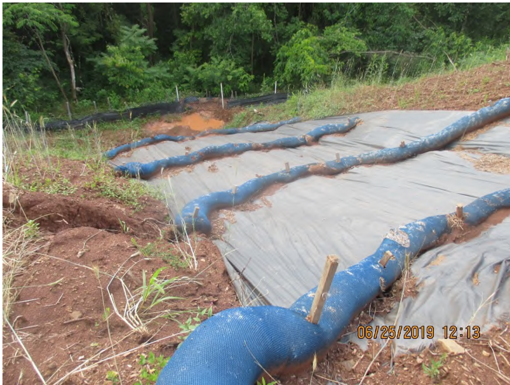
Waterbar outlet controls on slope south of ARWI 024 near station No. 5372+00. Perimeter controls overwhelmed with sediment. Erosion occurring under and next to Geotech fabric.
