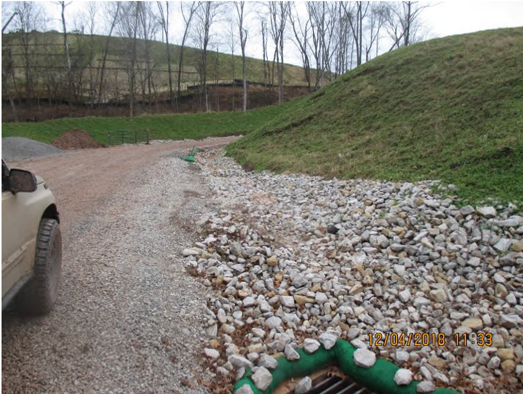
Rock lined ditch terminating at drop inlet adjacent to entrance.
