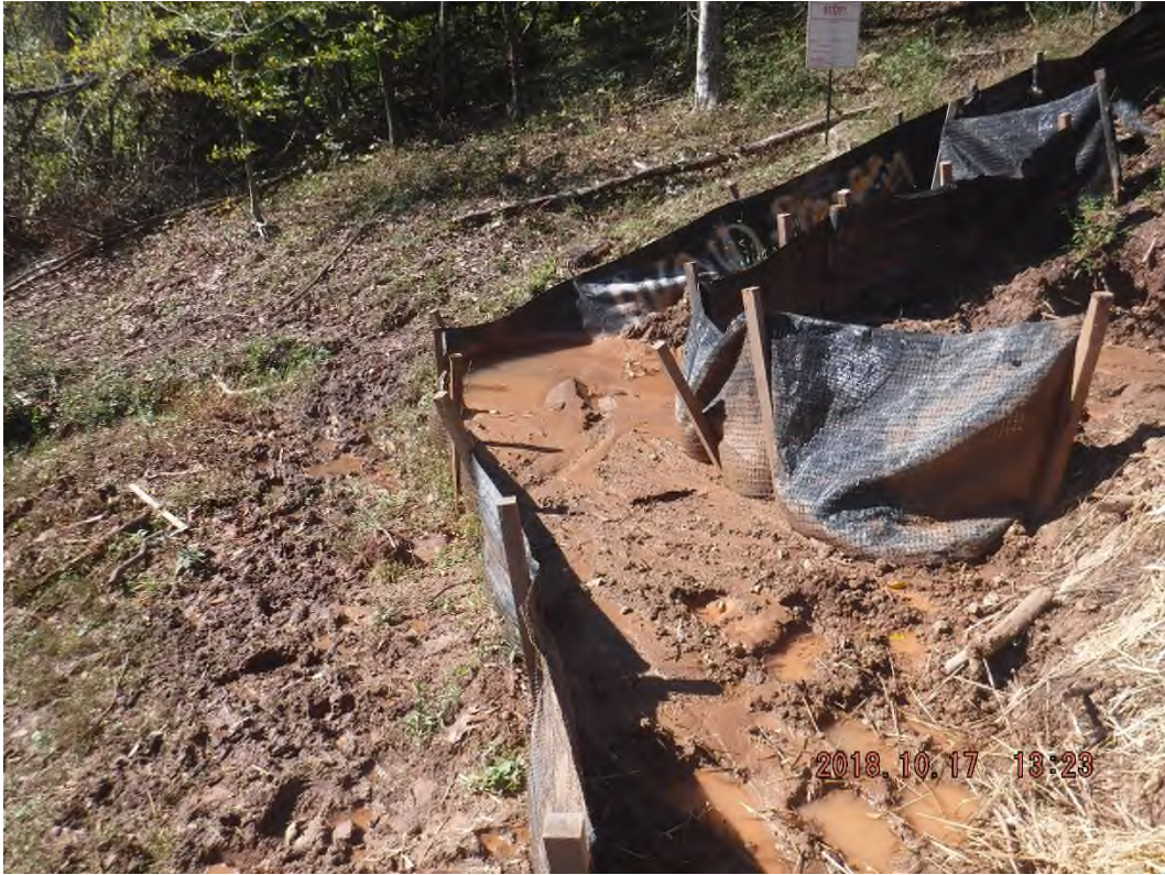
Sediment build-up in silt fence at Station 6705+00.
