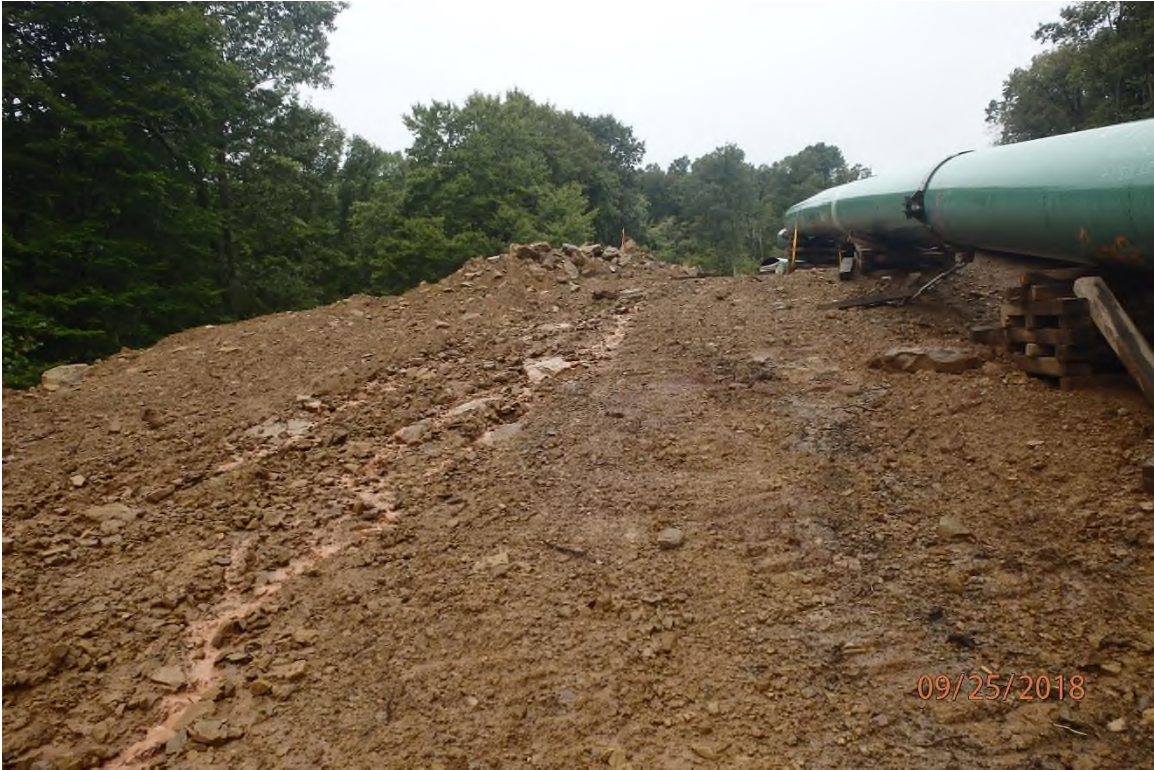
Concentrated flow being directed over fill slope adjacent to ARDO002.8 due to poorly maintained water bars.
