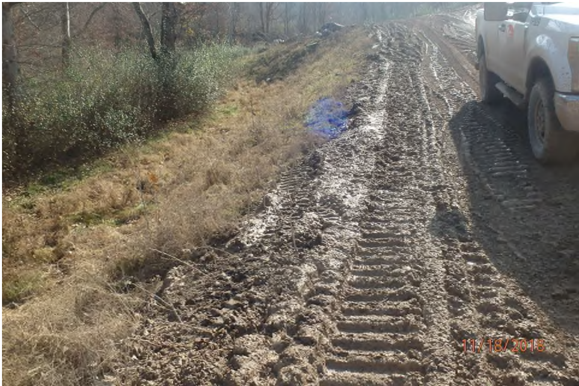
ARDO009.3 showing the lack of a graveled surface and the lack of perimeter controls, even though the road requires construction activity.
