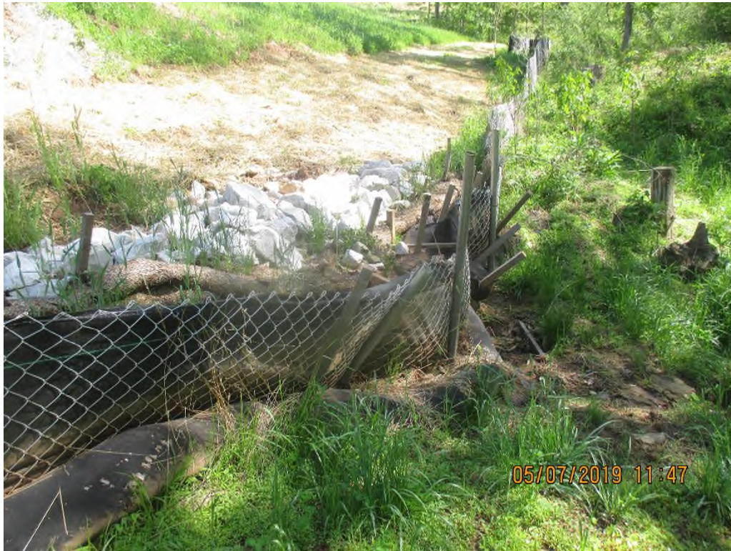
Perimeter controls on southwest slope of project LOD.
