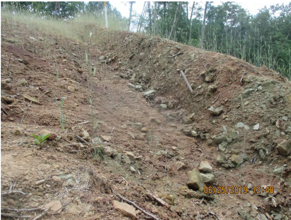
South of Station No. 5396+00. Waterbar with erosion present leading to overwhelmed controls.
