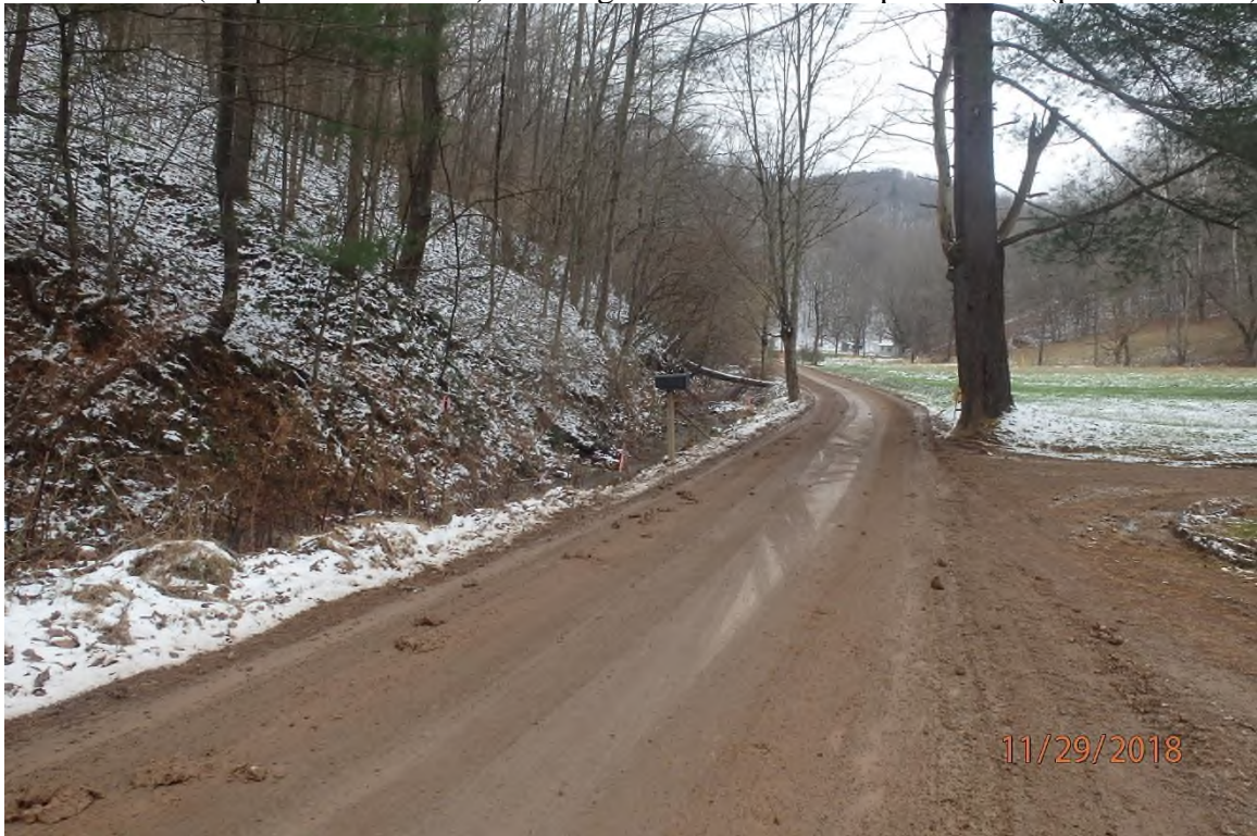
ARDO002.41 (Ralphs Run Access) showing track-out onto the public road (paved surface).
