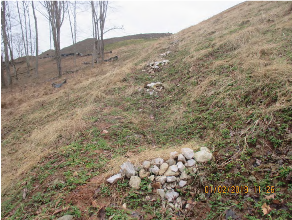
Diversion ditch along south side slope.
