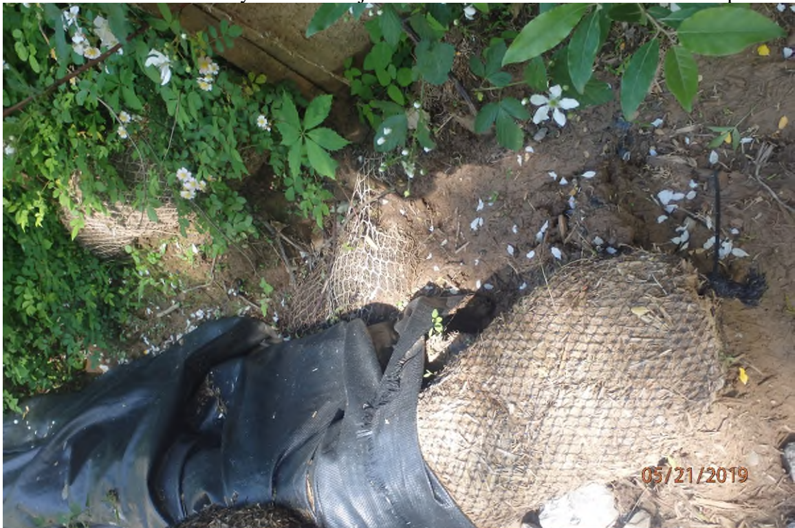
Installed BMP that is in need of maintenance on to ARDO009.1.
