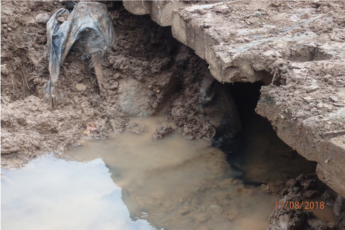
UNT Left Fork of Arnolds Creek (SDOG040) crossing showing a bridge in need of maintenance.
