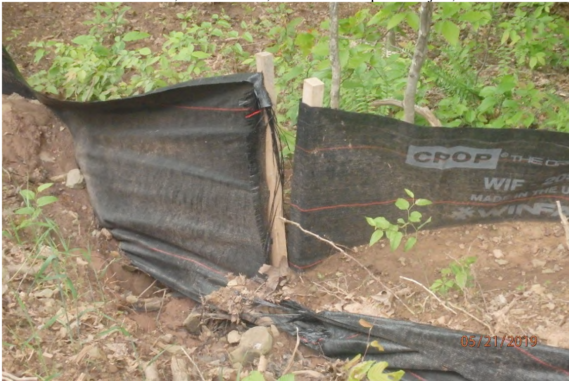
Improperly merged perimeter controls in the S. Fork of Hughes River watershed.
