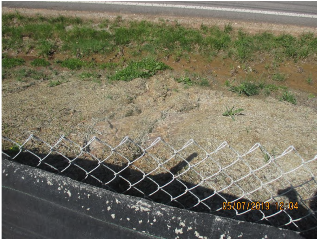
Erosion occurring below unmaintained controls and sediment deposits in Roadside ditch that parallels Route 21.
