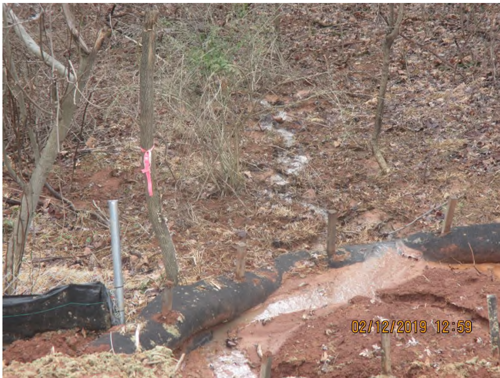
Facing downslope at station 5388+00 at perimeter controls from top of slope. SLW flowing past controls and into ephemeral stream
