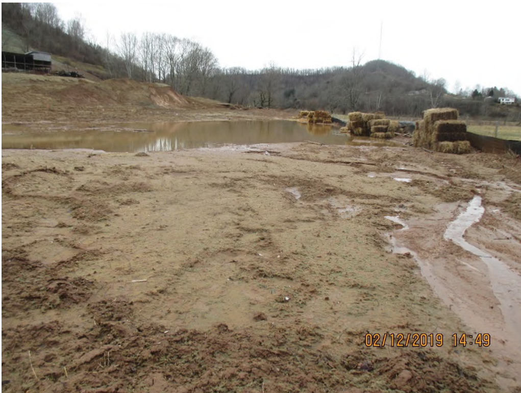
Work space below MXP ROW facing Northeast
