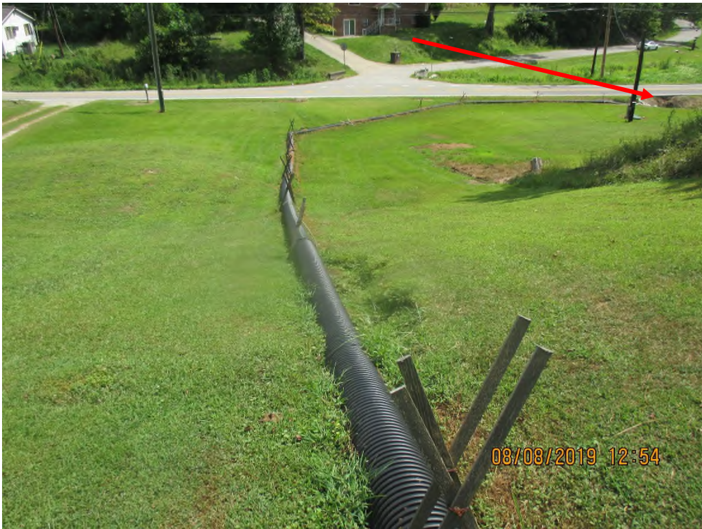
Slope drain conveying across complainants' yard and into roadside ditch. Arrow depicts where slope drain terminated into culvert that conveys under Charles Creek Road.
