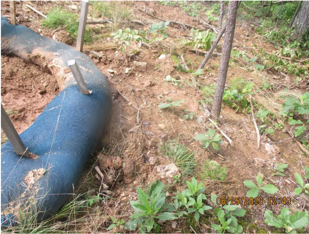
South of Station No. 5396+00. Waterbar outlet controls overwhelmed with sediment deposits past LOD.
