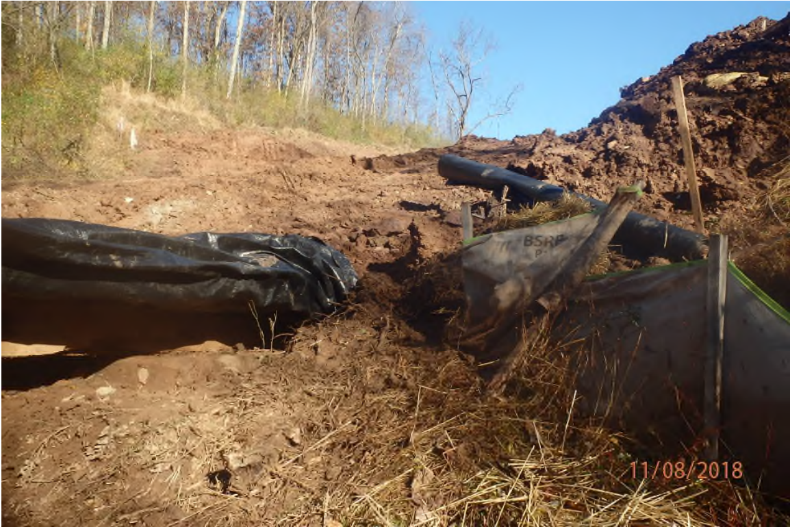
Improperly installed equipment bridge tie in adjacent to wetland UNT Bluestone (WDOG502) crossing.
