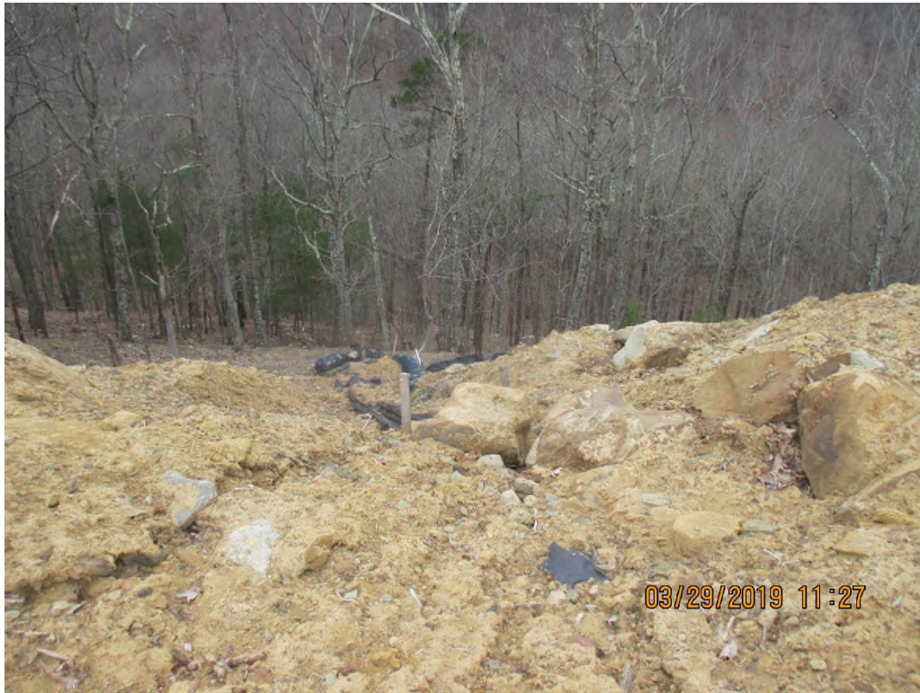
Waterbar terminus with erosion on slope near station #5148+00 facing downslope towards perimeter.
