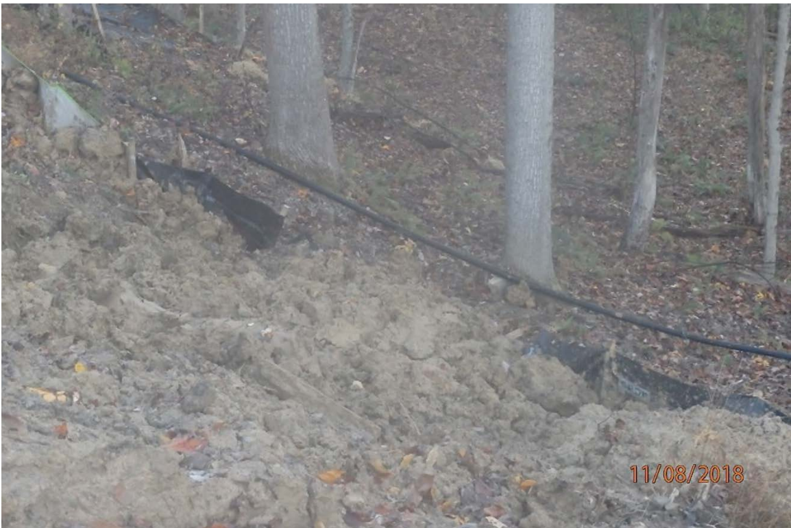
Unmaintained perimeter control and associated offsite sediment deposits in the Bluestone Creek watershed.
