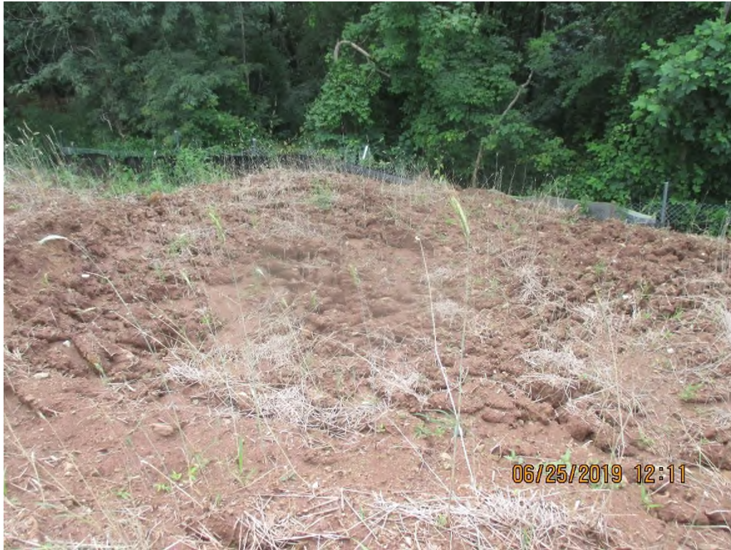
Slip present near station No. 5372+00 south of ARWI 024.
