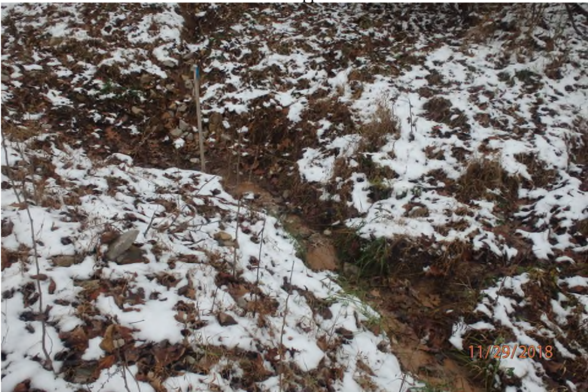
Trail of sediment laden water entering a culvert head just downslope of the area in the picture above on ARDO009.3.
