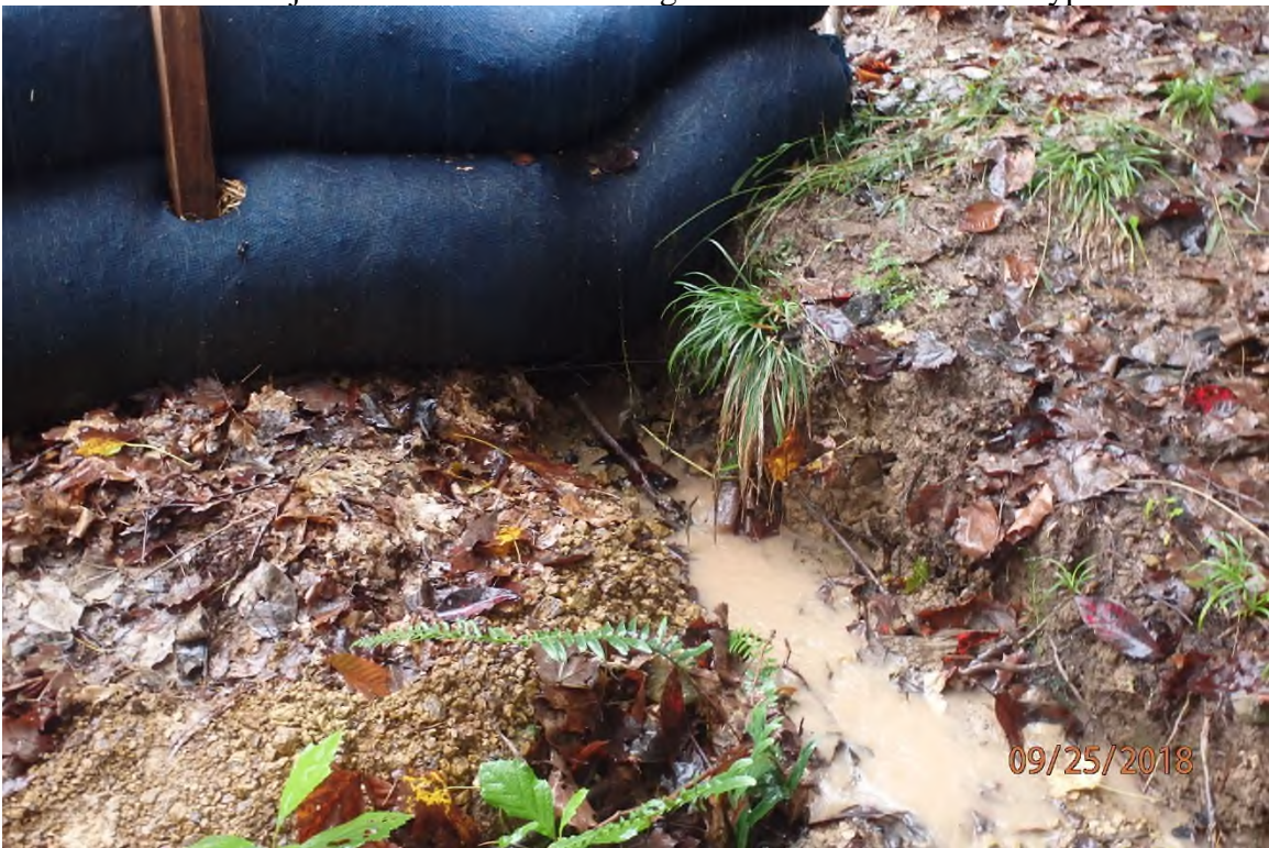
Water bar terminus BMP adjacent to 2275+00 allowing sediment laden water to bypass under the device, resulting in CNA distinctly visible settleable solids in UNT Neds Run ( 39^{\circ} 21.099' X 80^{\circ} 41.670' ).
