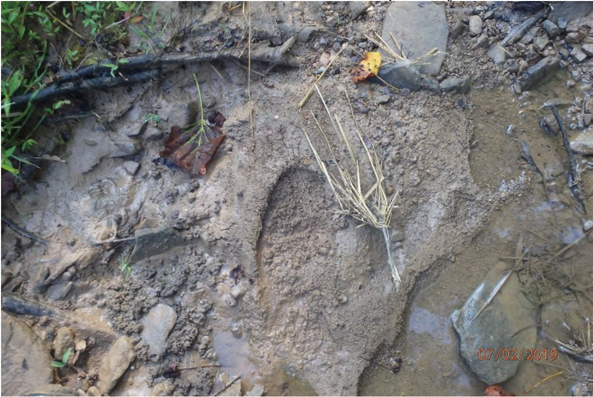
Offsite CNA deposits in UNT Sugar Run (39° 11.075' X 80° 51.108') as a result of the three previously pictured unmaintained perimeter controls.
