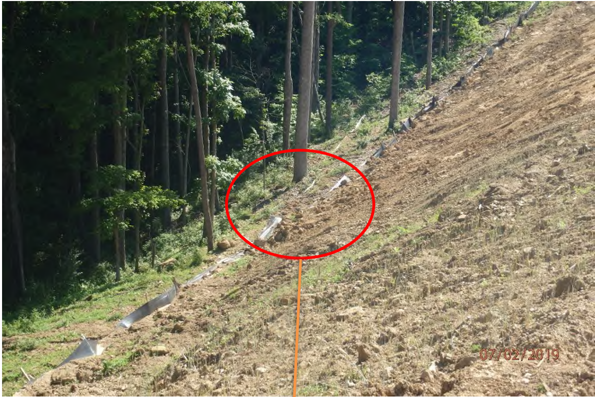
Perimeter control in need of maintenance in the Taylor Drain watershed.
