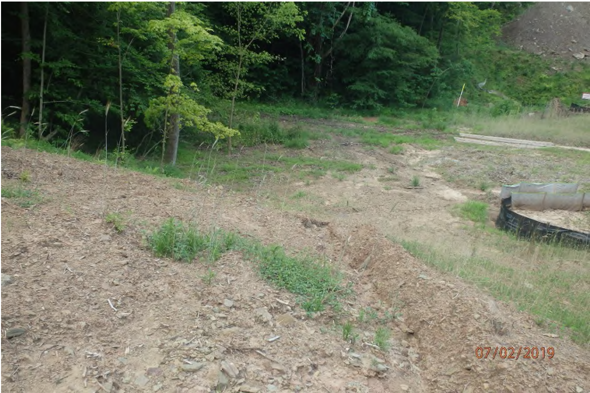
Water bar that lacks the water bar terminus BMP indicated in the approved SWPPP in the UNT Left Fork of Arnolds Creek watershed.
