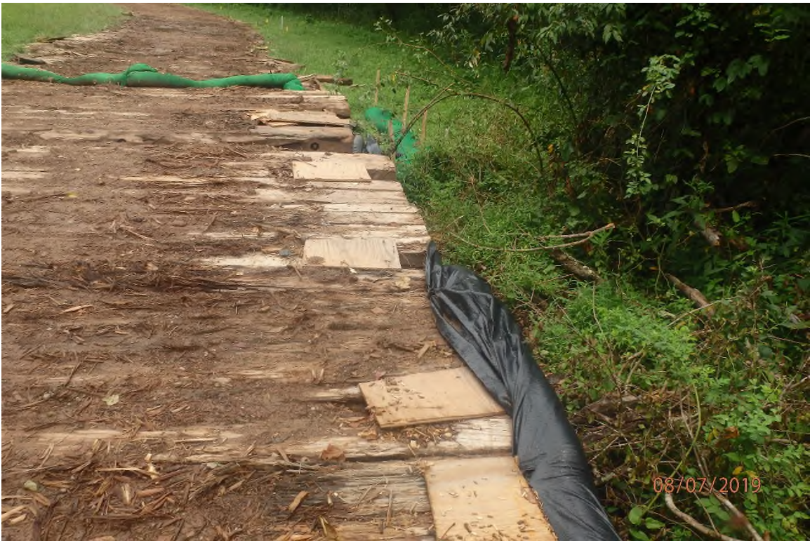
Installed timber mat equipment bridge at UNT Riggins Run (SDOG903) showing the need for maintenance.
