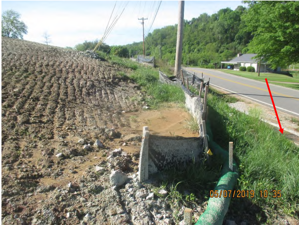
Controls above roadside drain. Sediment being deposited behind controls at base of slope. Arrow depicts roadside drain.
