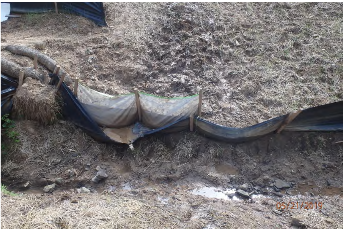
Installed BMP that is overwhelmed adjacent to UNT Taylor Drain as a result of a failure to install water bars.
