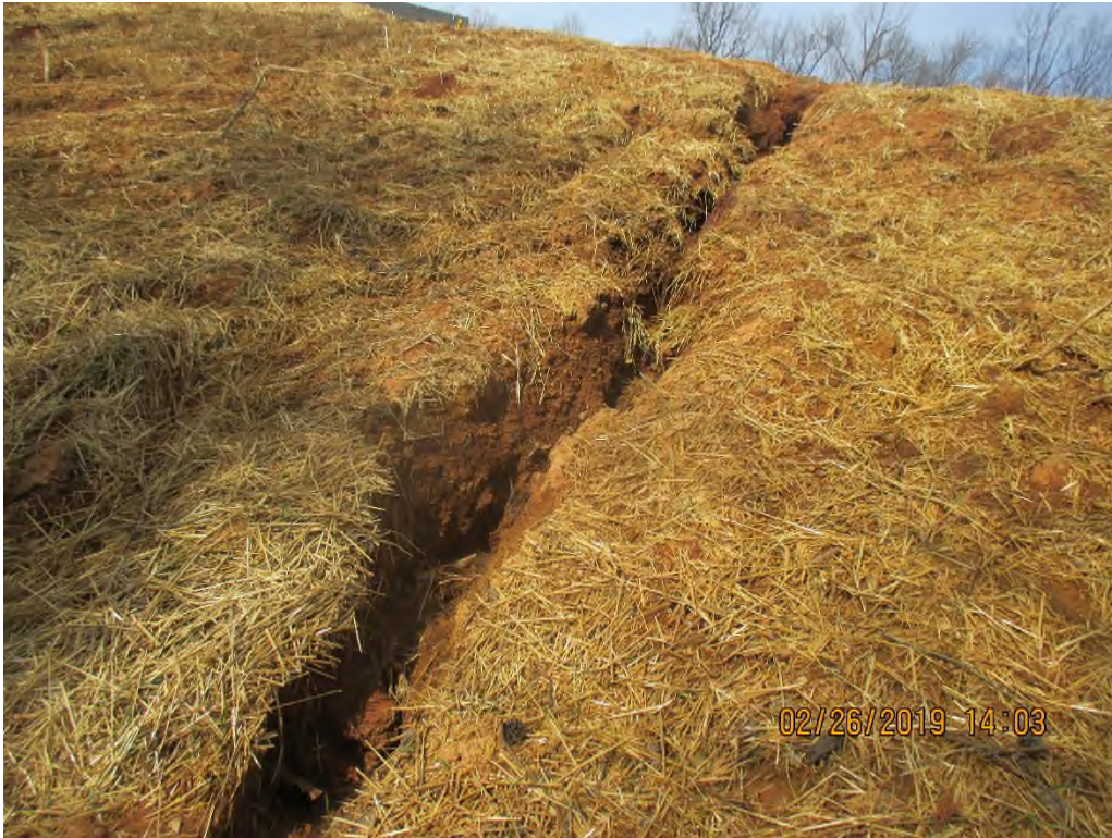
Near station #6620+00 (per SWPPP). Seep intersecting ROW and causing erosion on slope.
