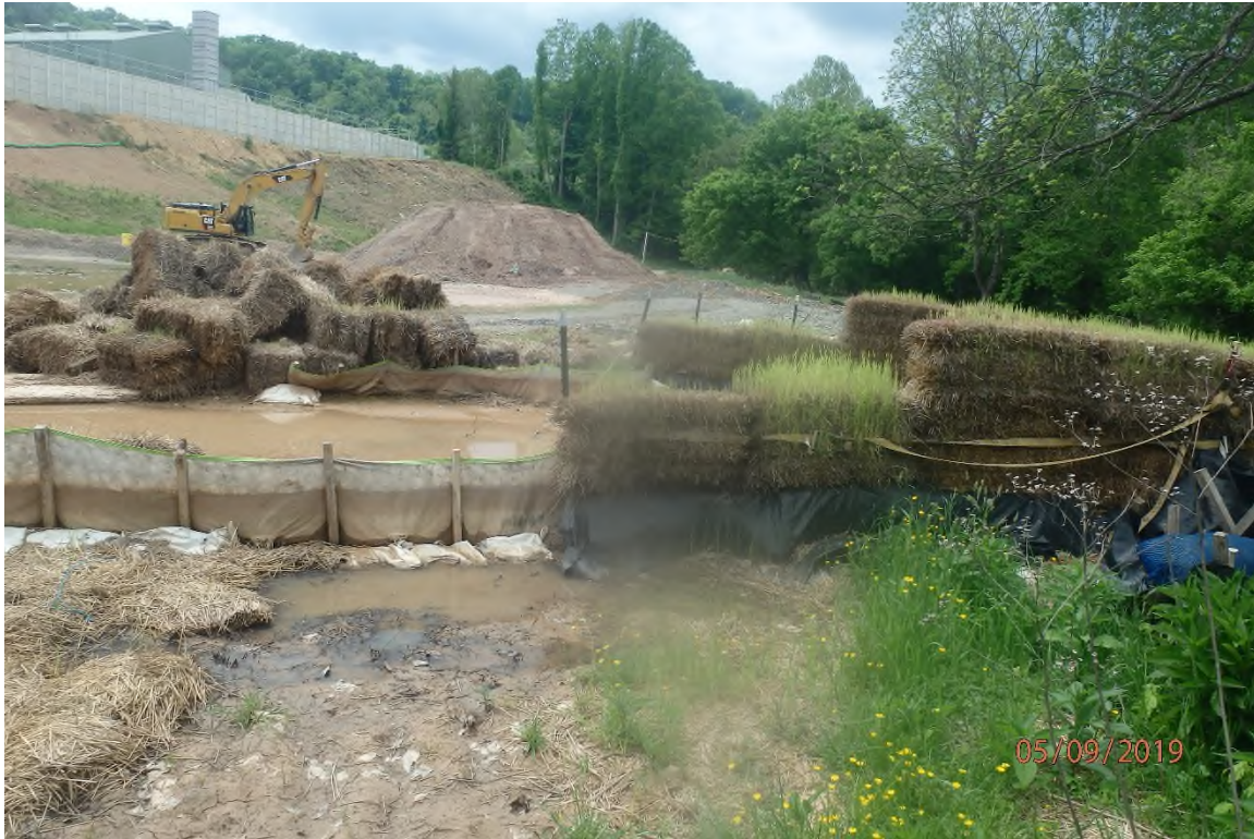
Makeshift treatment structure being utilized to treat stormwater from the sediment basin that is being discharged into an unstable diversion.
