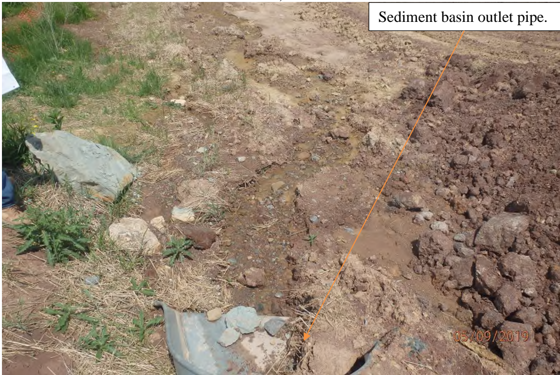
Diversion downslope of the sediment basin outlet pipe showing the lack of a riprap channel and weir.
