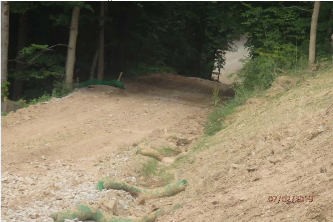
ARDO13.5 showing the need for maintenance to the stabilized surface.
