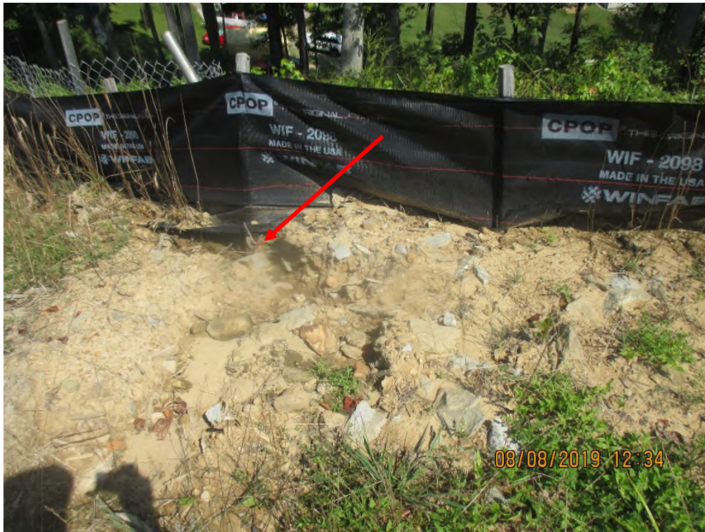
Perimeter control at Waterbar termini downslope of slipped material. Perimeter control overwhelmed and undermined due to concentrated flow.
