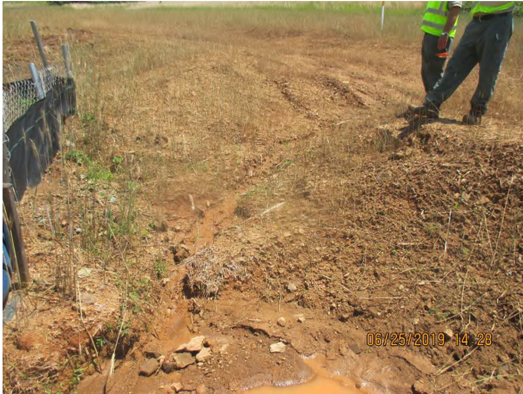
Waterbar terminating into perimeter controls at station No. 5638+46. Erosion present on slope above controls.
