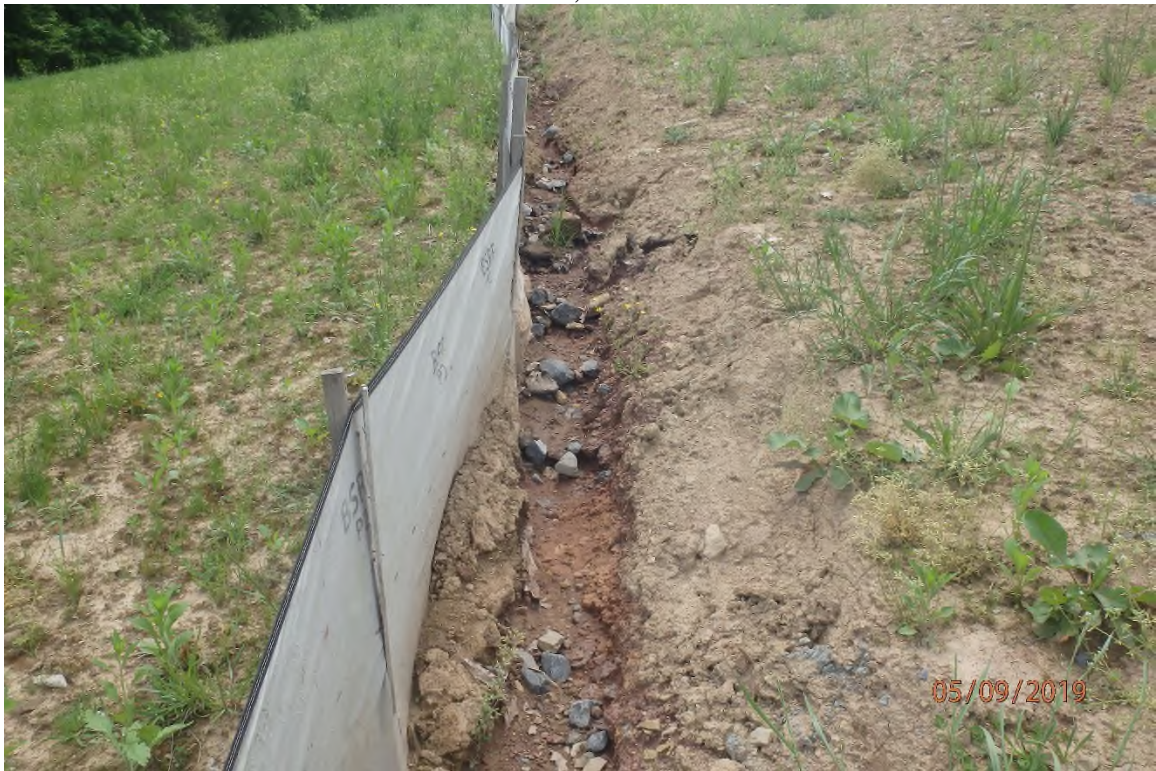
Diversion in need of maintenance adjacent to the fill pad. Perimeter controls improperly installed and in need of maintenance.
