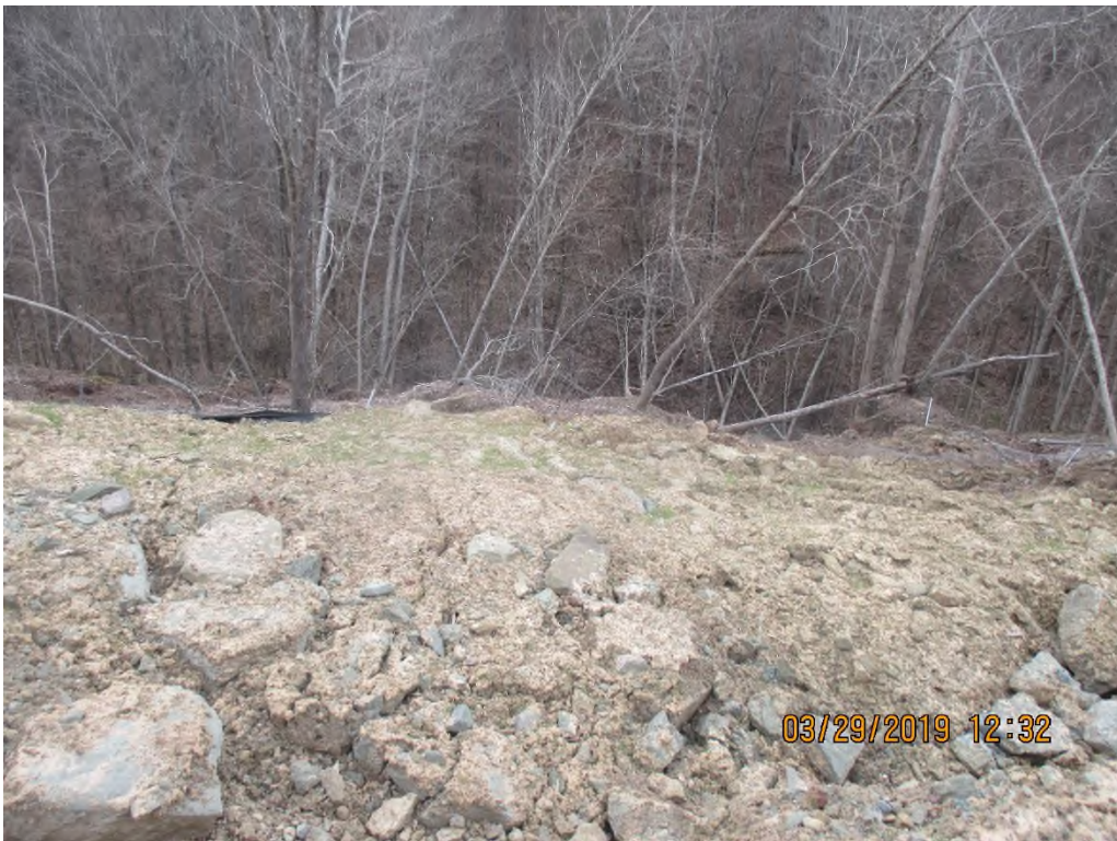
Erosion on fillslope at station #5162+60. Sediment overwhelmed perimeter controls and was deposited past LOD.
