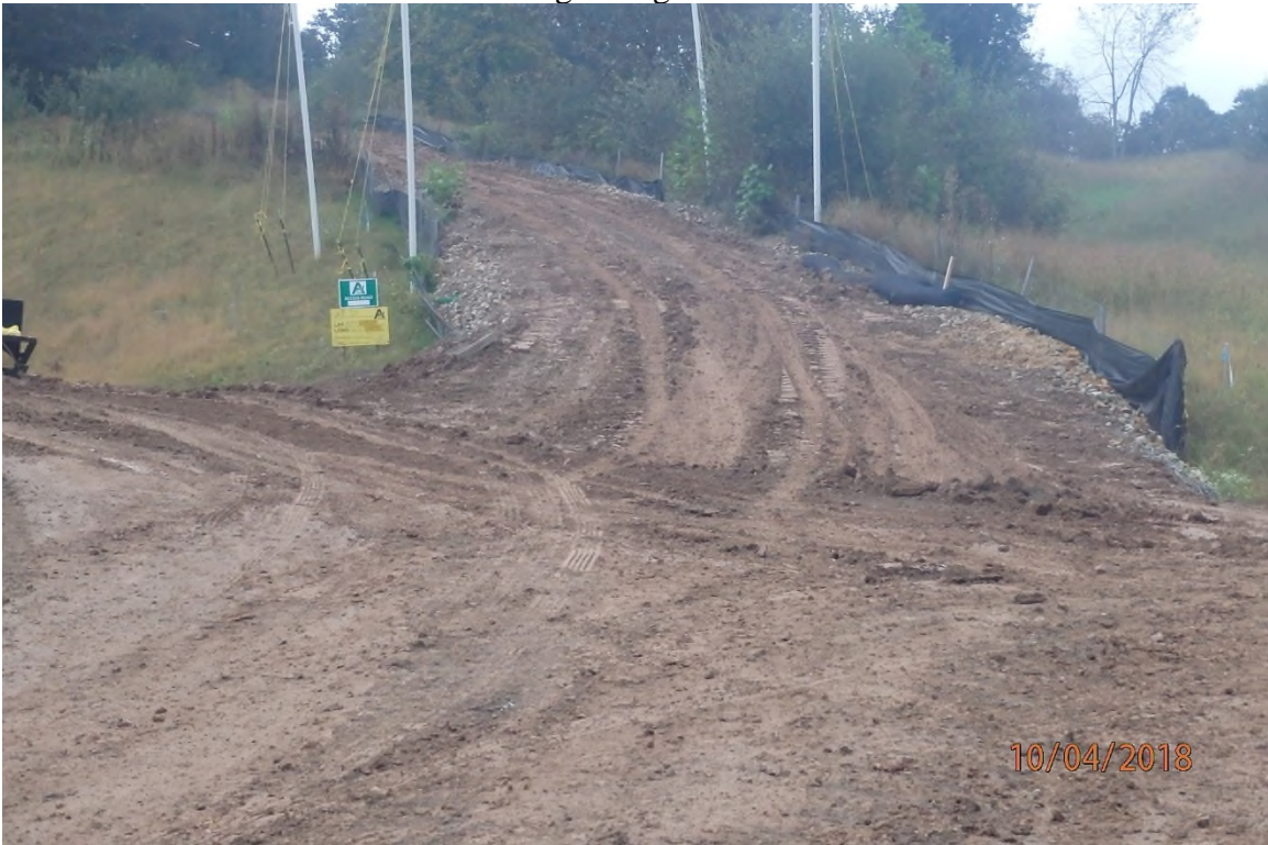
ARDO-001.5 at the intersection of CR 5 showing the lack of a stabilized construction entrance.
