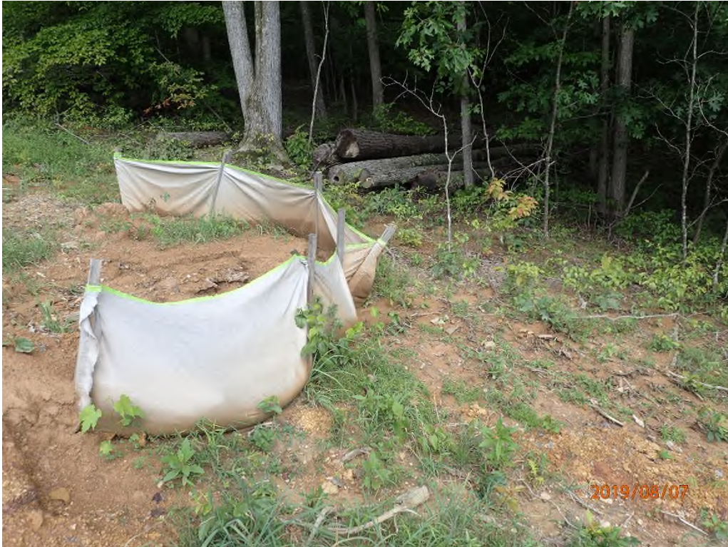
Sump not maintained. Several were noted along the inspected ROW.
