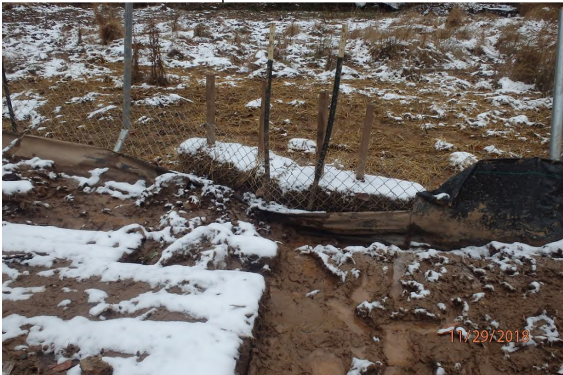
Unmaintained perimeter control on ARDO009.1.
