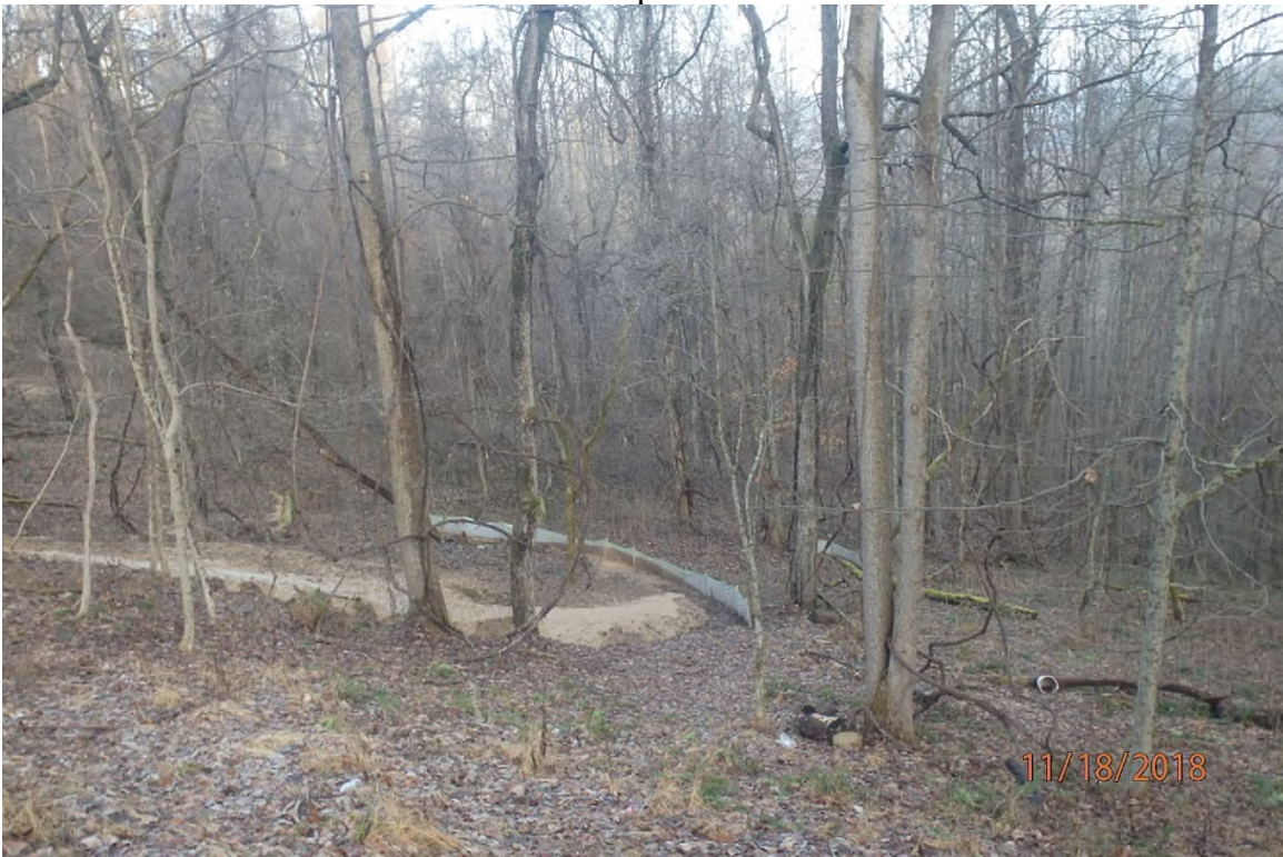
Mud flow and newly installed perimeter control on offsite slip near 2822+00.
