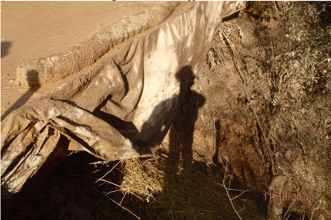
Equipment bridge BMP on the above pictured crossing showing the area of bypass.
