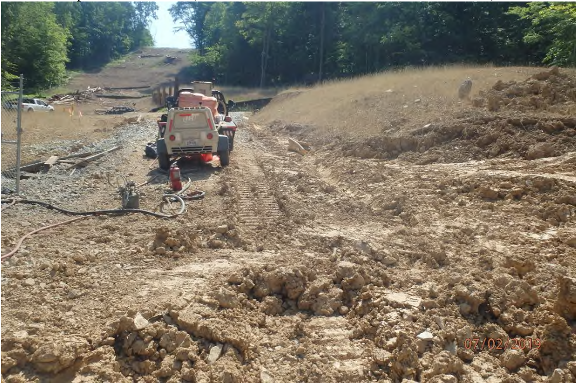
Water bar installed at varying angles in the Taylor Drain watershed.
