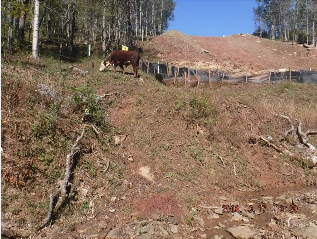
Station 6705+00, showing slope without installed water bars.
