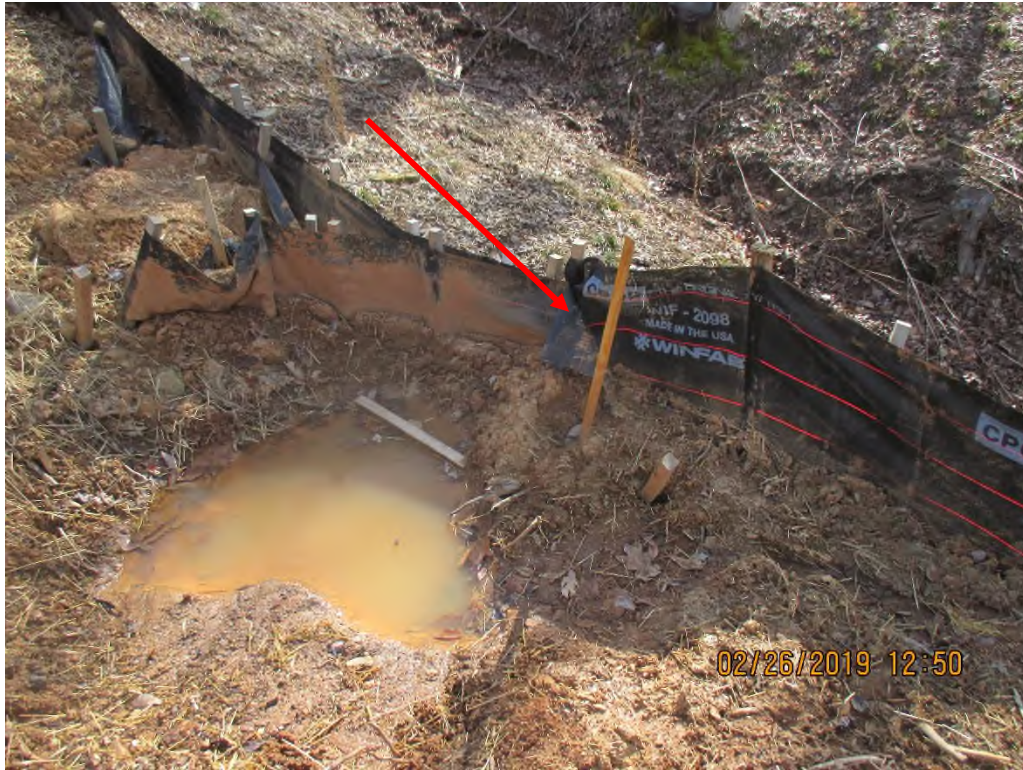
Waterbar outlet above stream SJAD-009. Silt fence not tied into each other.
