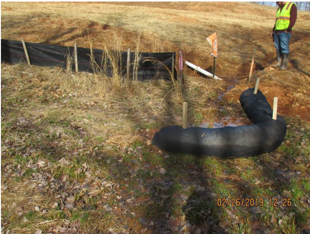
Waterbar outlet with slope drain terminating into control near station #6781+00 and above Stream SJAD-008
