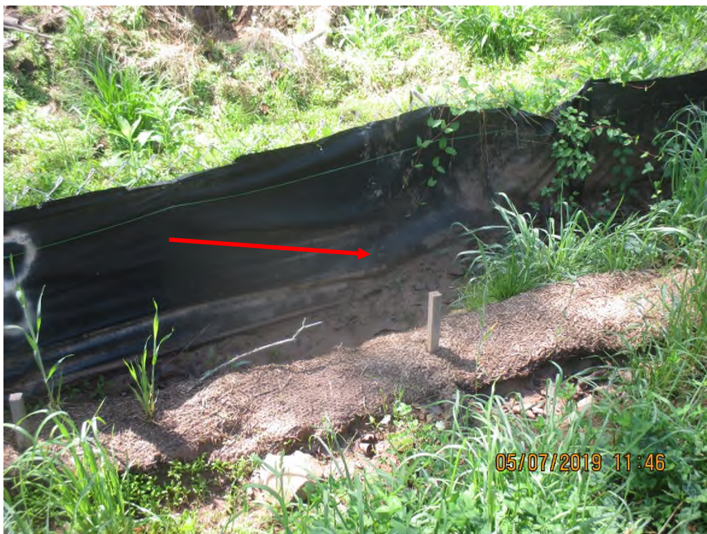
Silt fence on Southwest slope of project perimeter with small hole at stain line on fence.
