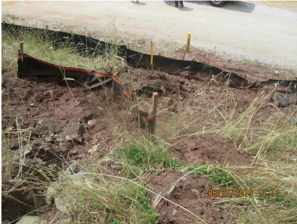
Erosion above and between controls above the Munchausen Road crossing.
