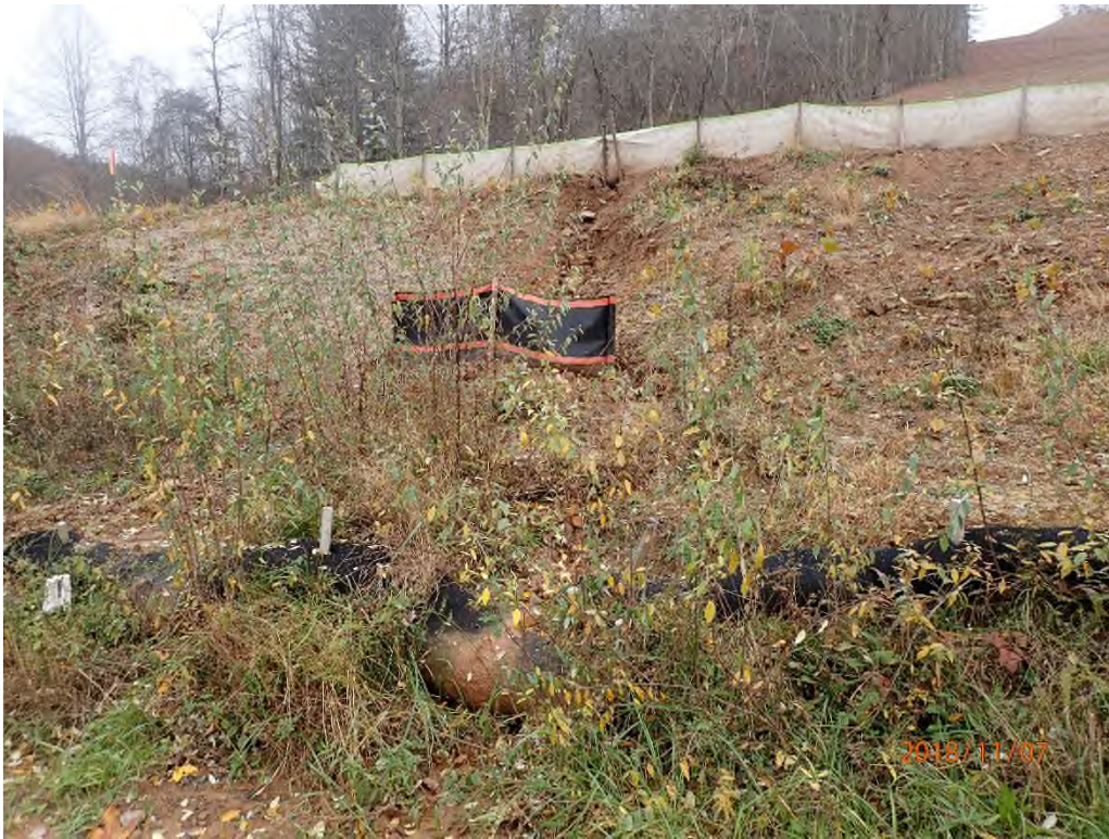
Sediment-laden water leaving the site through perimeter controls in need of maintenance.
