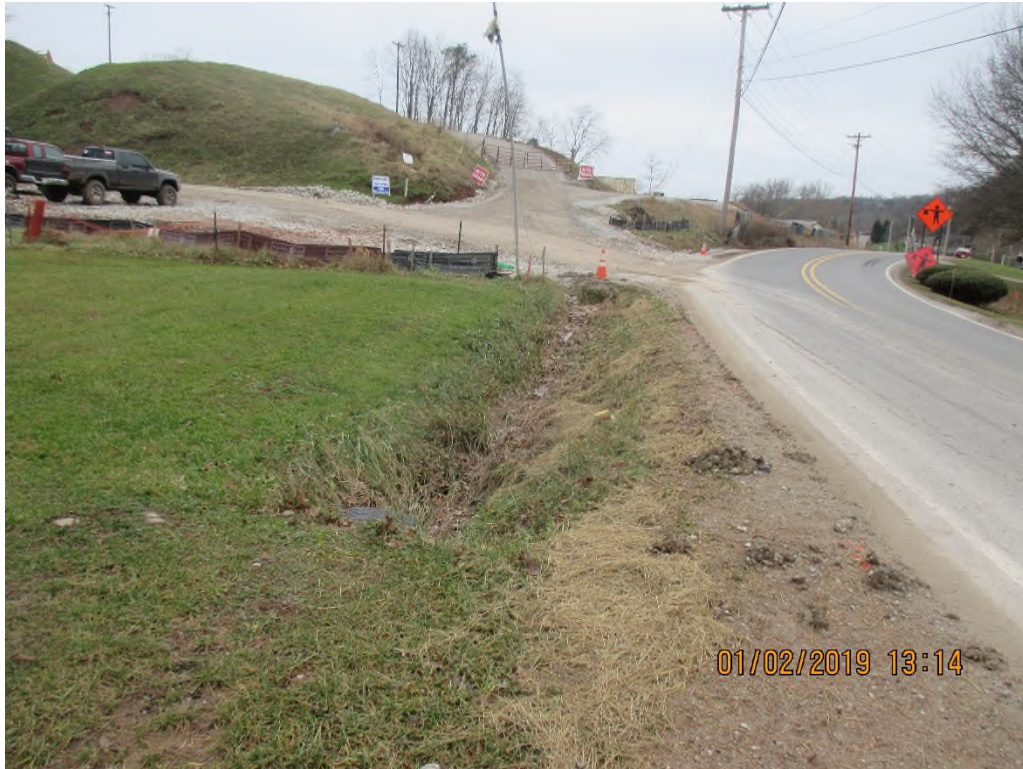
Mt. Olive Compressor station entrance along Route 21.
