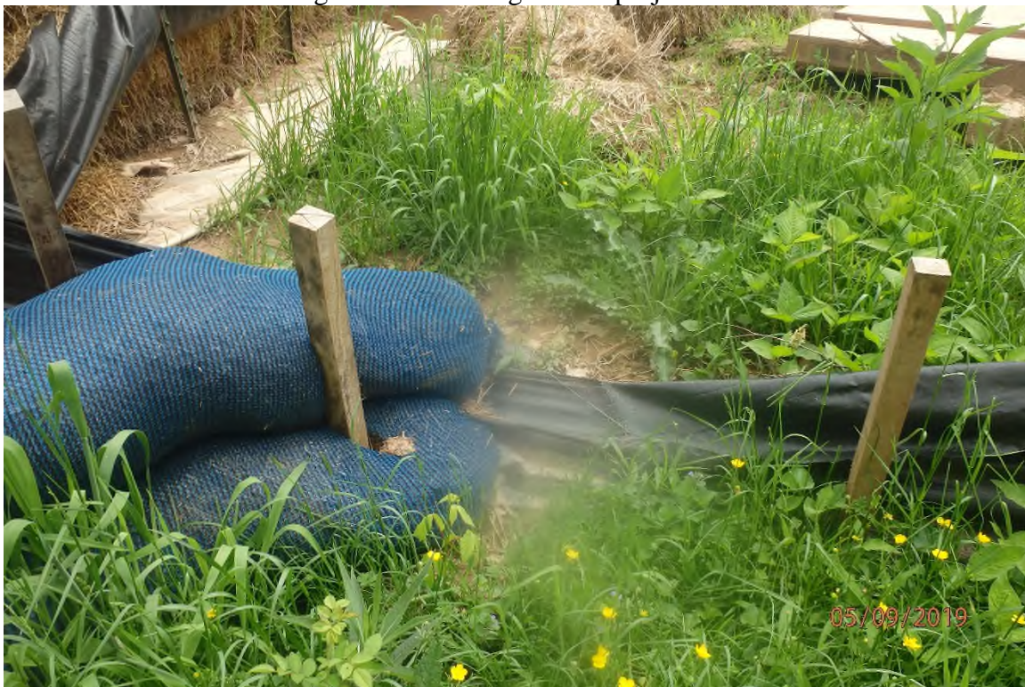
Perimeter control along the northern edge of the project in need of maintenance.
