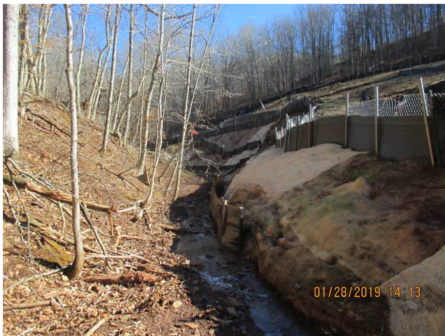
Stream SJAG 316 facing upstream where slips are occurring and impacting stream.
