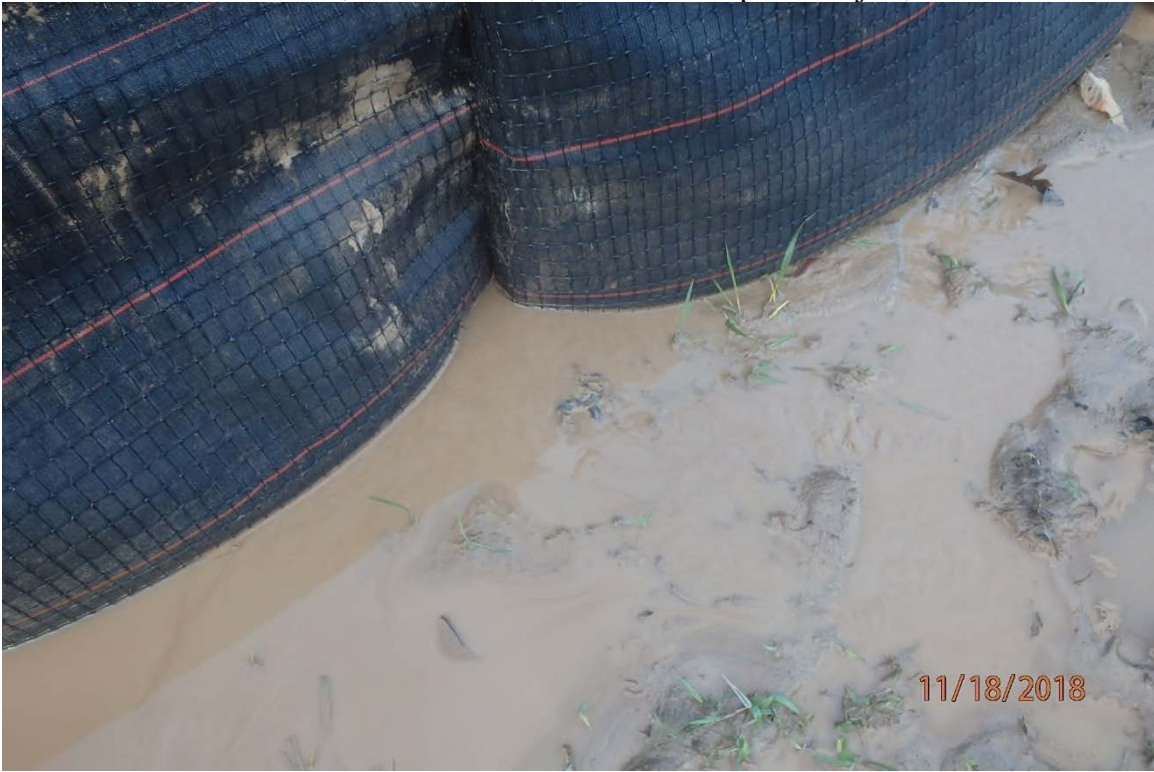
Improperly installed perimeter control on ARDO008.2 allowing sediment laden water to bypass under the installed BMP.
