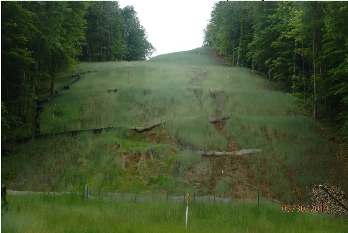
Water bars in the Neds Run watershed that have been temporarily repaired with silt fence and need to be reestablished with equipment.
