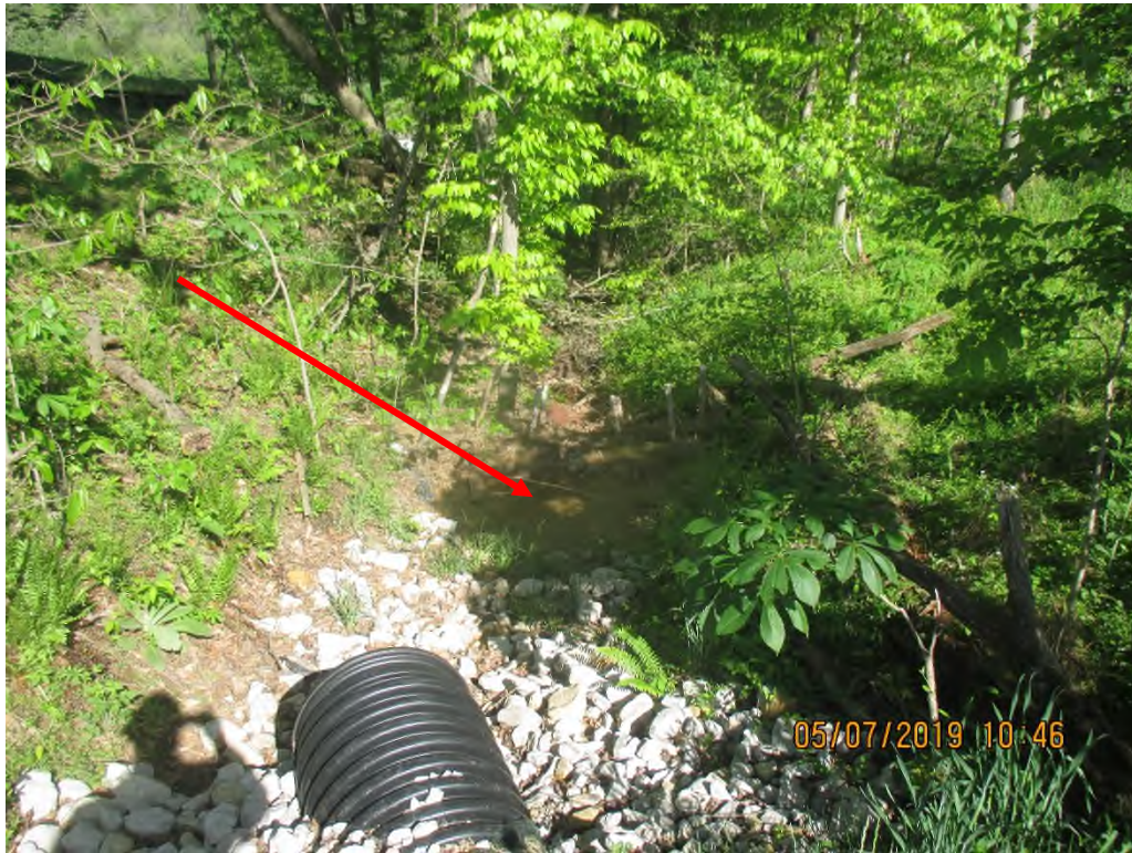
Drop inlet's outlet facing downslope at ephemeral stream leading to UNT of Grasslick Run. Arrow depicts sediment deposits past controls.
