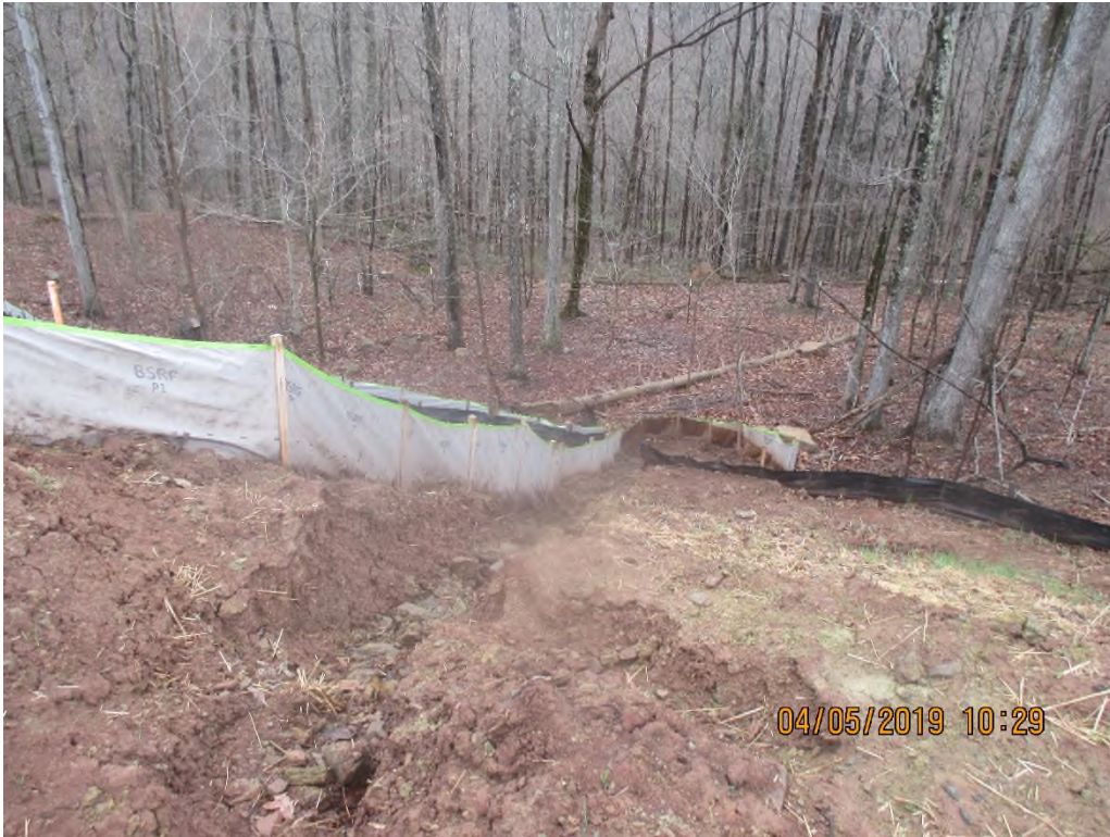
Waterbar outlet near station #6795+40. Waterbar terminating on fill slope causing erosion on slope.
