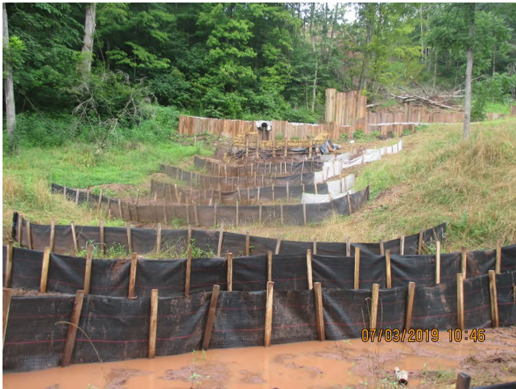
Last silt fence above 18-Mile Creek, upslope at Sulu road and slip.
