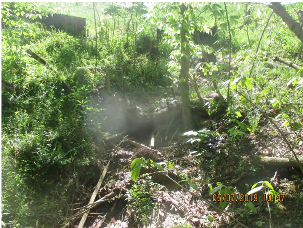
Downslope of controls in ephemeral stream. Controls in need of maintenance and enhancement upslope.
