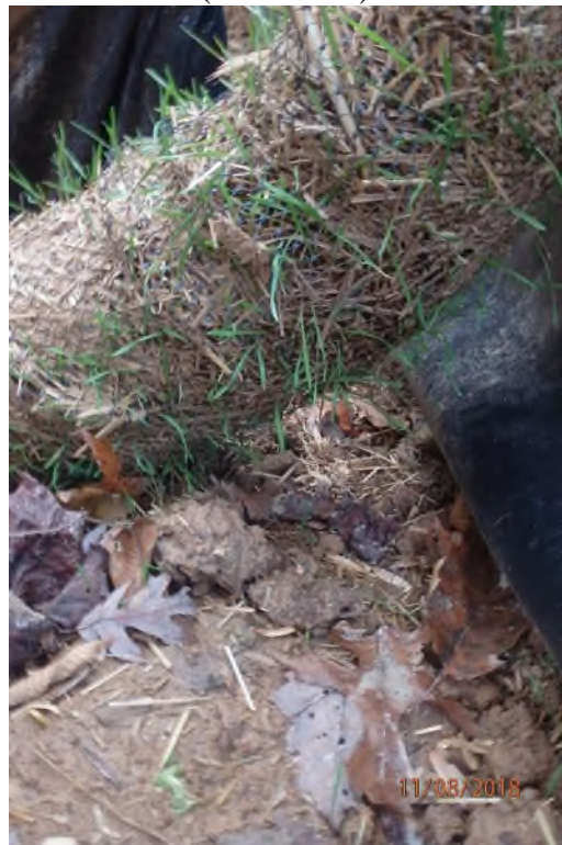
Improperly installed perimeter control equipment bridge tie-in adjacent to UNT Taylor Drain (SDOH012).
