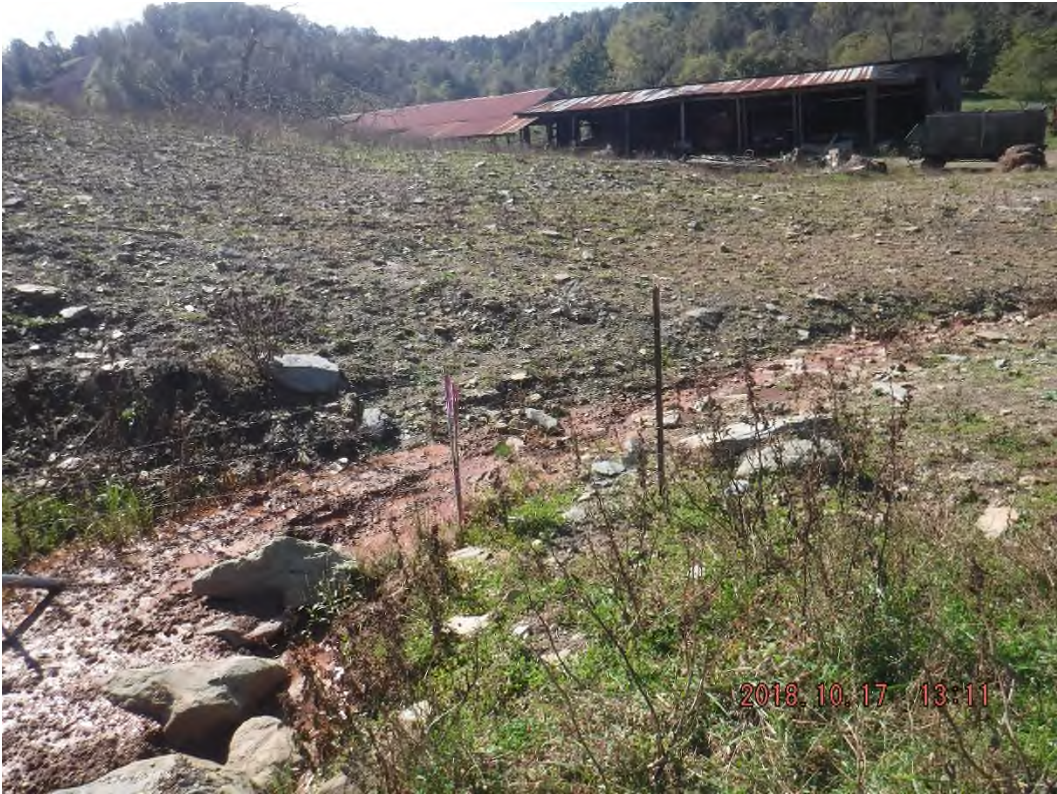
Sediment flow from silt fence.
