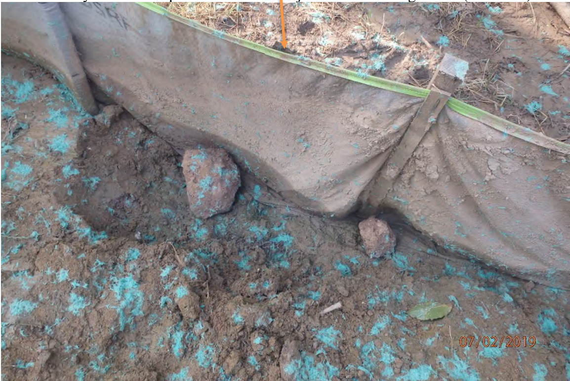
Additional maintenance needed to the above pictured BMP. Dirt clods placed on the silt fence flap and not repaired properly.
