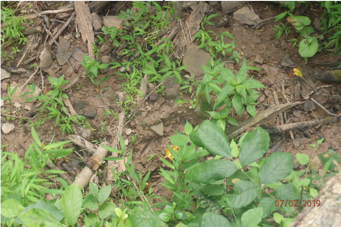
Offsite CNA deposits in UNT Trap Run (SDON829) as a result of the previously pictured deficiencies adjacent to 3214+00.
