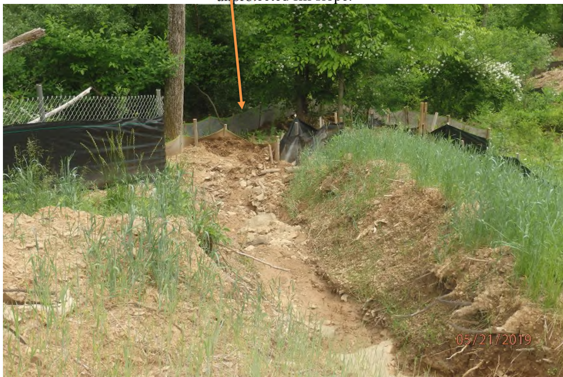
Outlet treatment that is overwhelmed due to stormwater flow from multiple water bars being directed at it. Maintenance of the BMP is poor. The contractor is adding additional layers of BMPs instead of conducting maintenance work. The furthest layer of BMPs is offsite.
