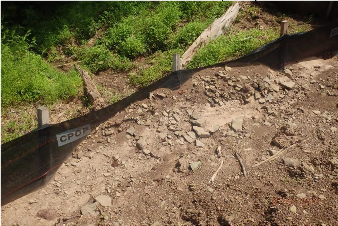
Perimeter controls adjacent to 3214+00 that are inundated with sediment and in need of maintenance as a result of the previously pictured deficiency.
