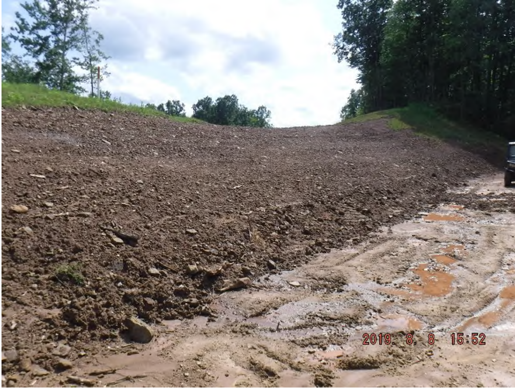
No controls were installed along access road, and seed failed to germinate.
