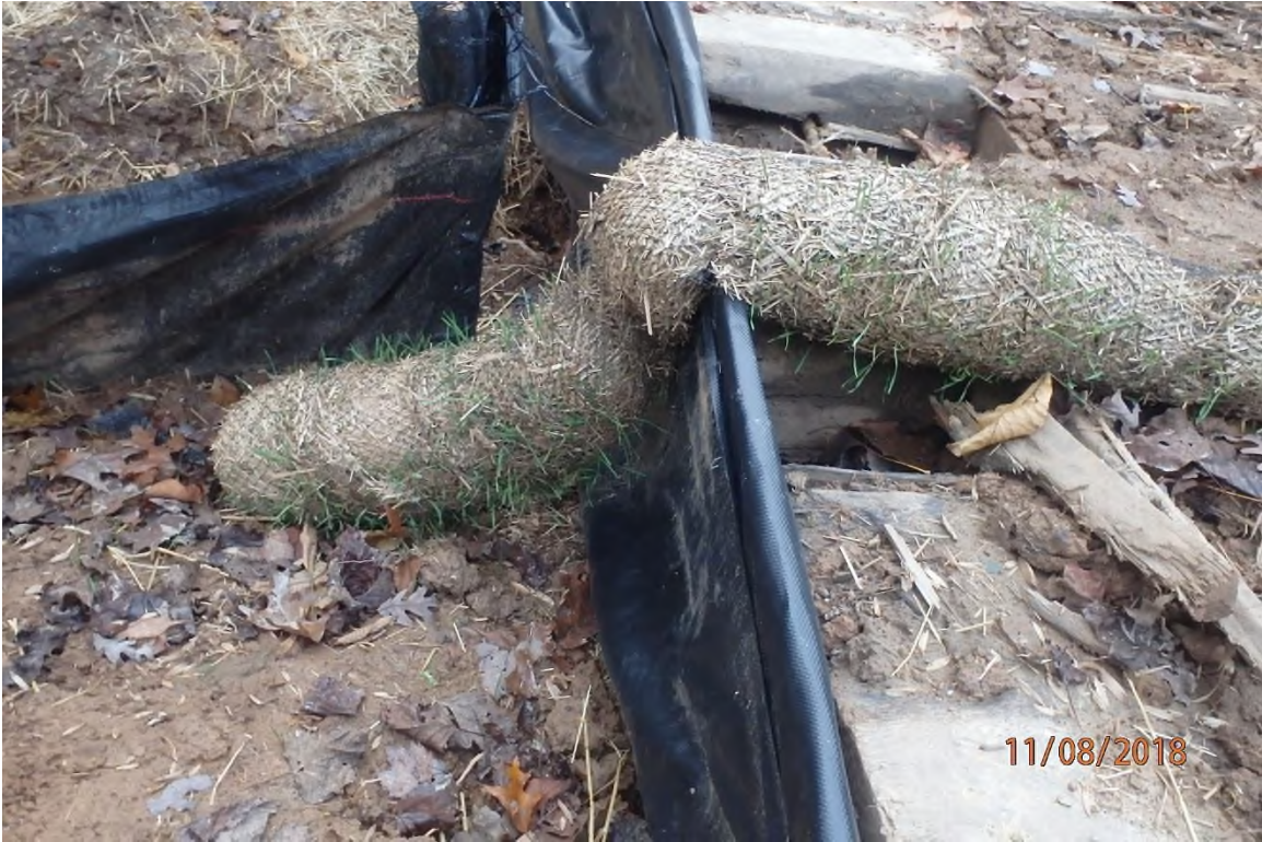
Improperly installed perimeter control equipment bridge tie-in adjacent to UNT Taylor Drain (SDOH012).
