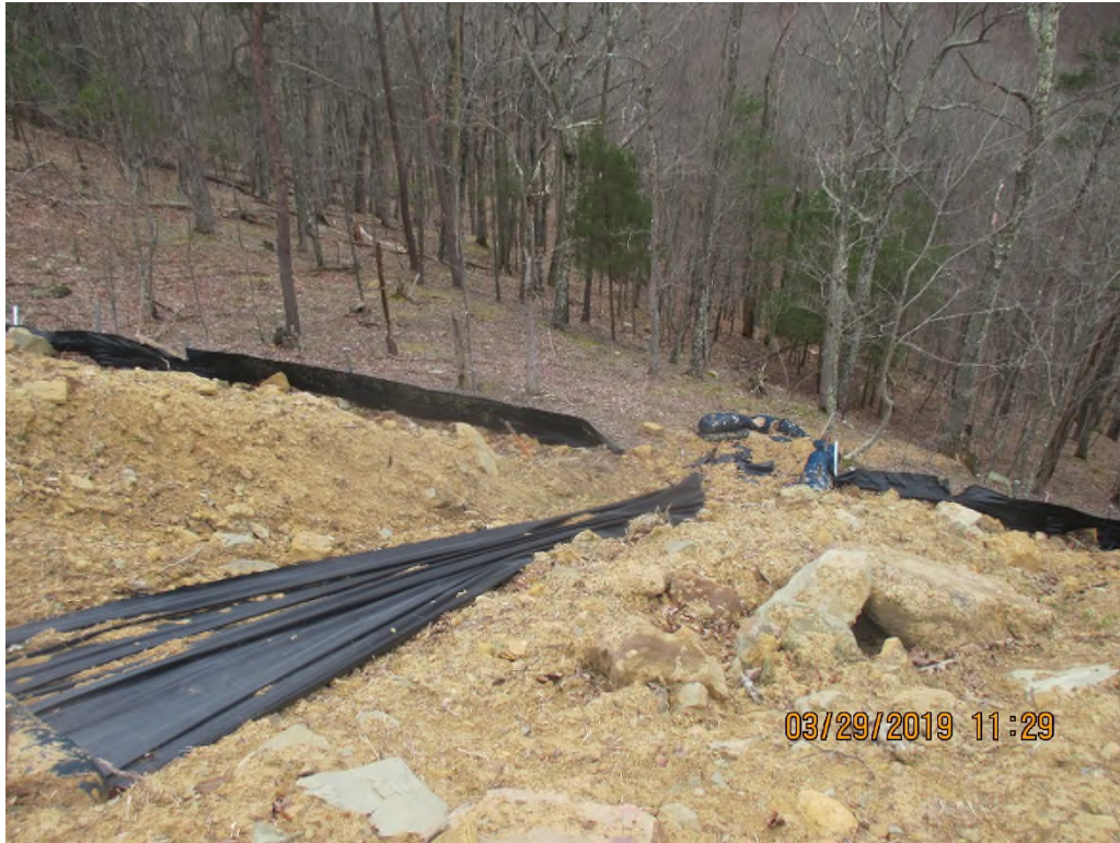
Waterbar outlet near station #5148+00. Erosion occurring on slope around geo mat and perimeter controls being overwhelmed with sediment.
