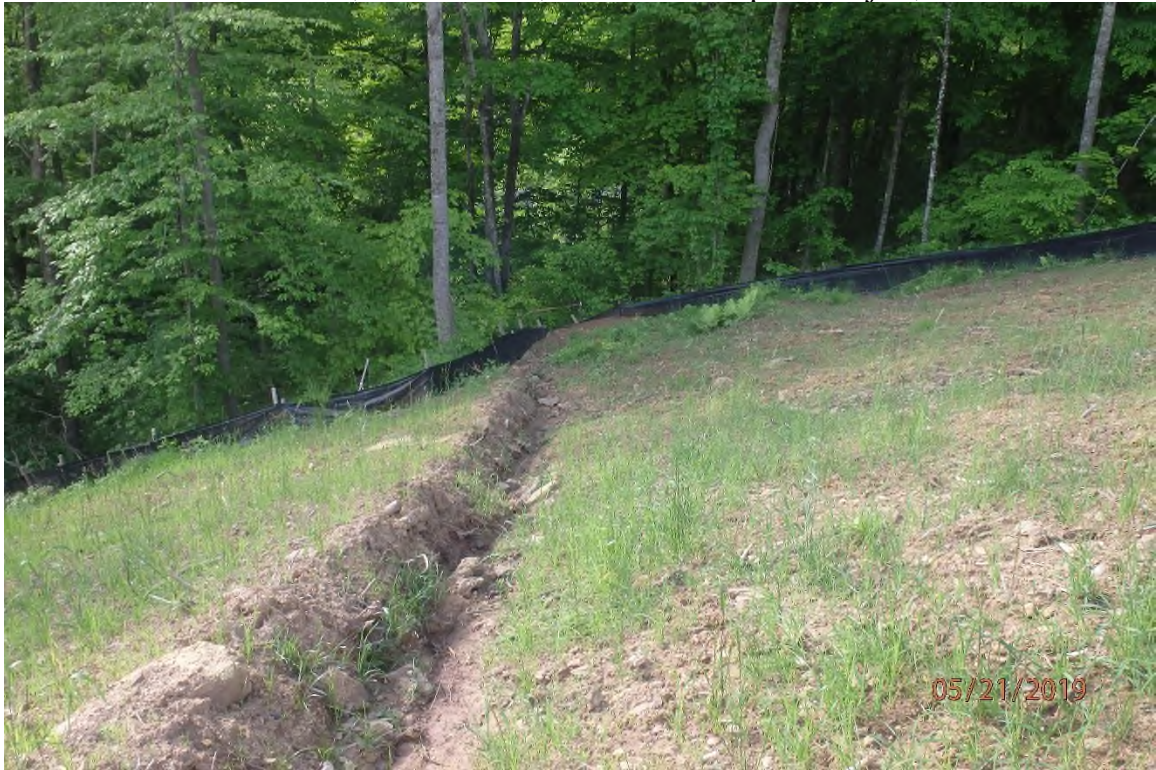
Sheet flow BMP installed in a concentrated flow area in the Sugar Run watershed. Pictured silt fence is not designed for concentrated flow treatment.
