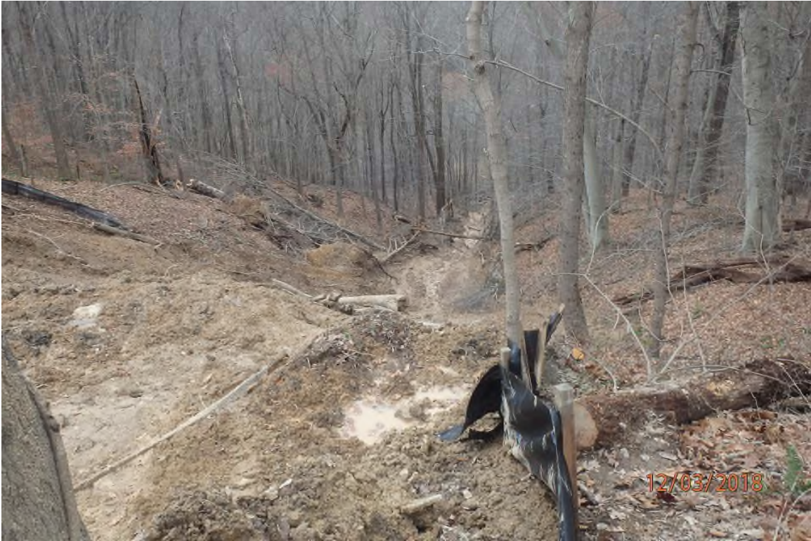
Lower portion of the slip associated with spill report number 09-83236 (A) showing remnants of recently installed silt fence and the lack of installed sheet piling. The pictured mud flow downslope of the slip is in the ephemeral UNT of Meathouse Fork.
