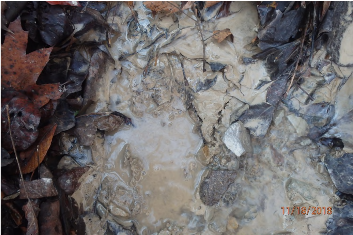
CNA deposits in UNT Georgescamp Run (39° 14.614' X 80° 44.951') on ARDO008.2 due to poor maintenance of installed BMP.
