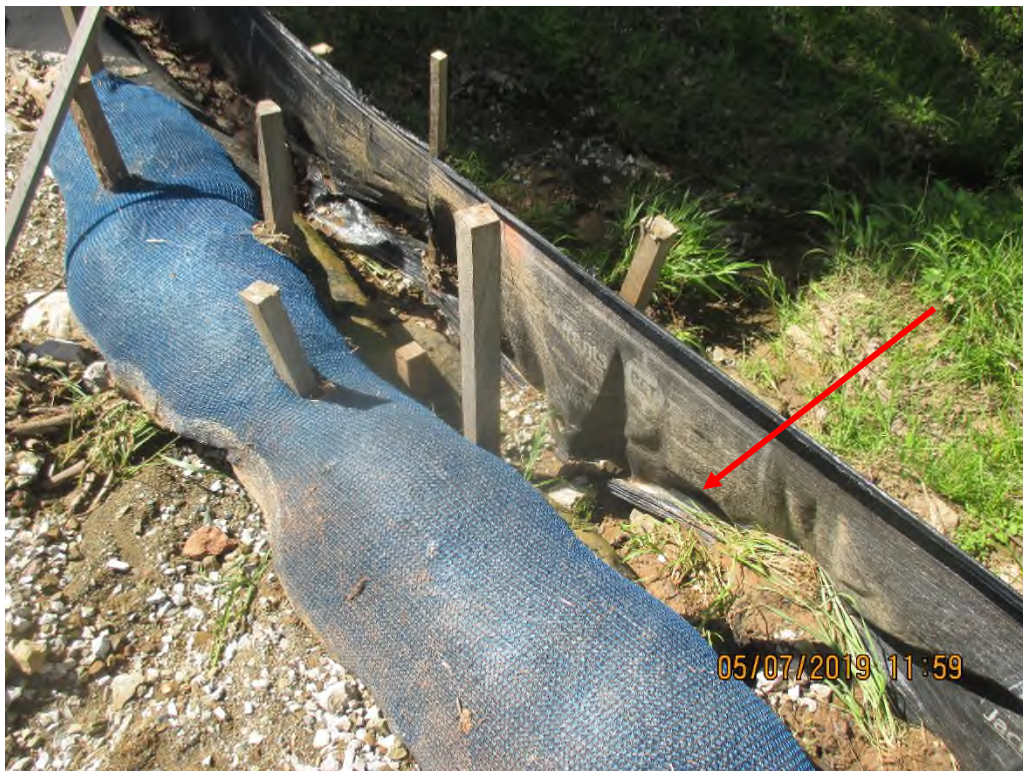
Perimeter controls below erosion on former access road. Arrow depicts silt fence is not trenched-in.
