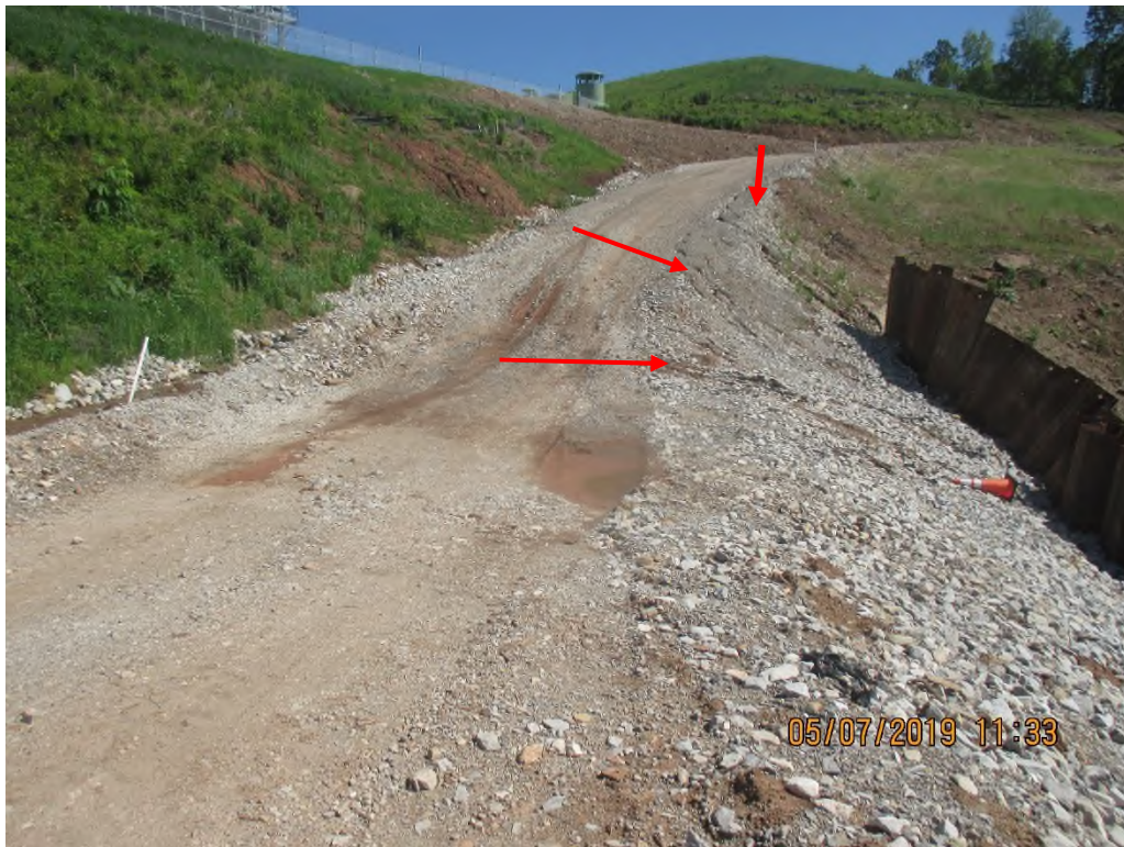
Facing east toward South slope where erosion was observed. Arrow depicts erosion occurring on road.
