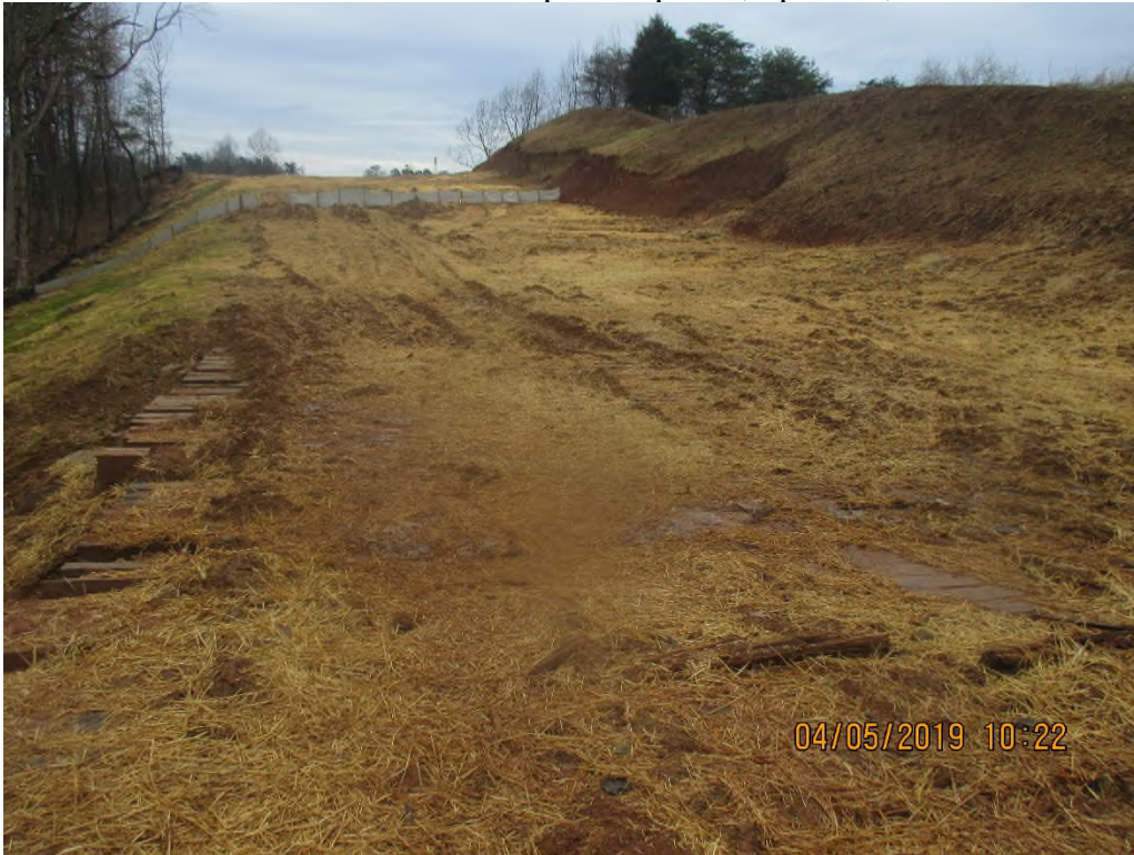
Near station #6781+55 facing South at low spot in ROW where water was accumulating. A pipe slope drain had been installed in this area. However, erosion was occurring on the slope below where timber mats had been installed.
