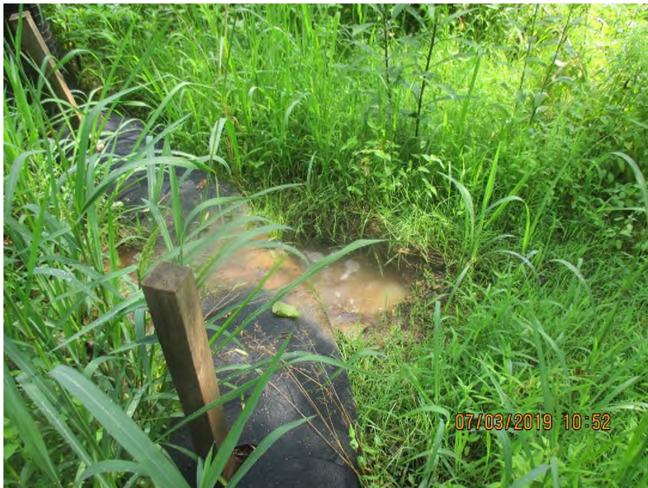
Last control in place above 18-Mile Creek. Sediment laden water was flowing past this control and into dense vegetation.
