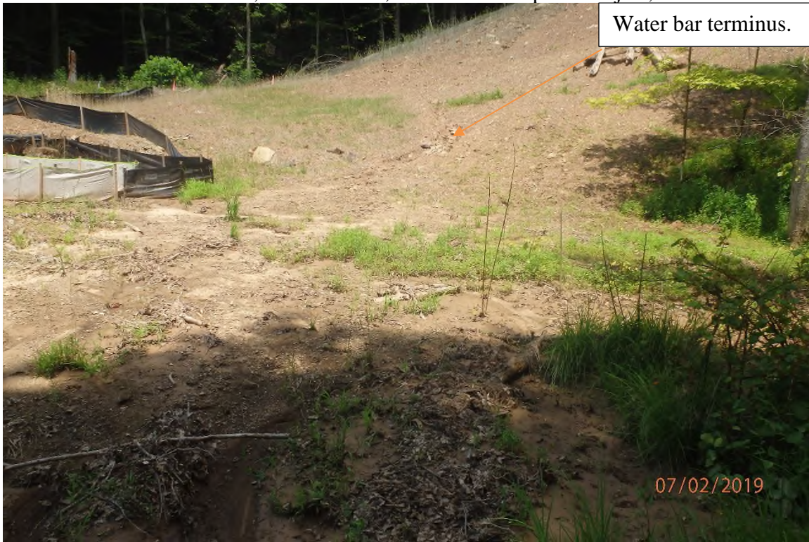
Offsite sediment deposits downslope of the previously pictured water bar that lacks the water bar terminus BMP indicated in the approved SWPPP in the UNT Left Fork of Arnolds Creek watershed.
