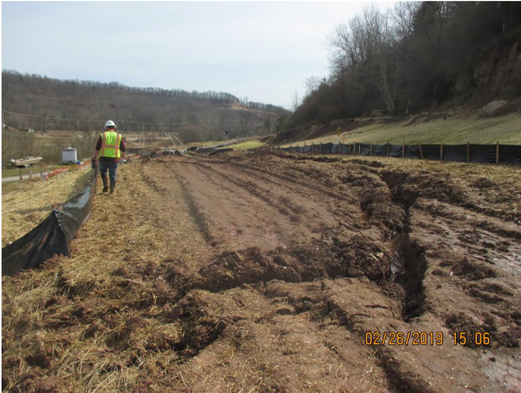
Section of ROW between Ripley regulator station and Rt. 21 with multiple slips on ROW.
