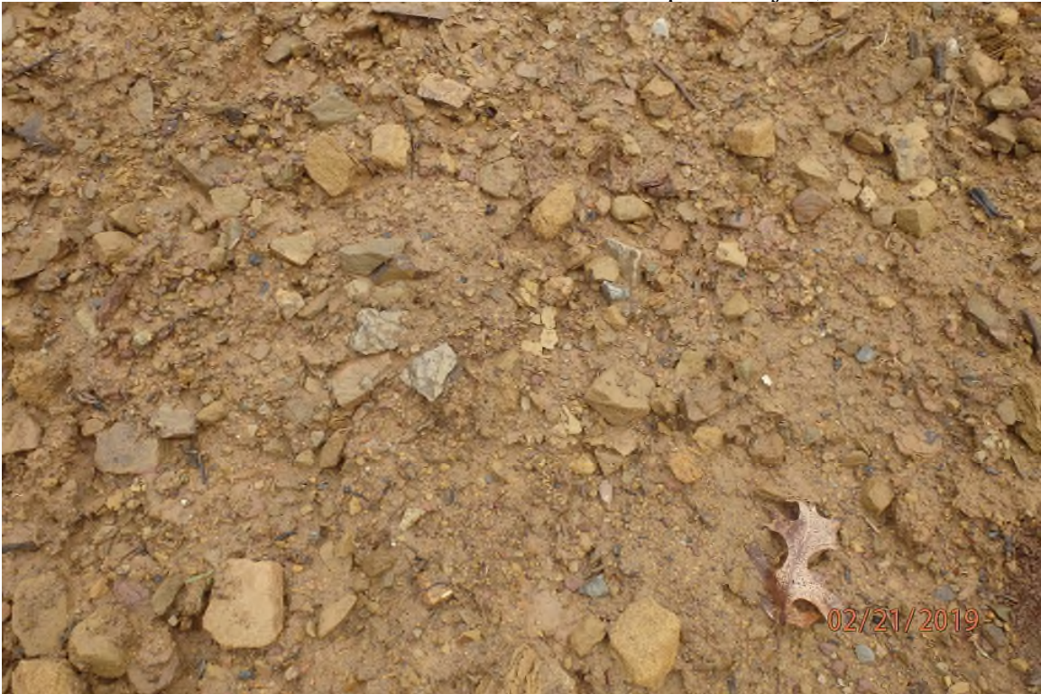
Project area showing the need for maintenance of temporary stabilization.
