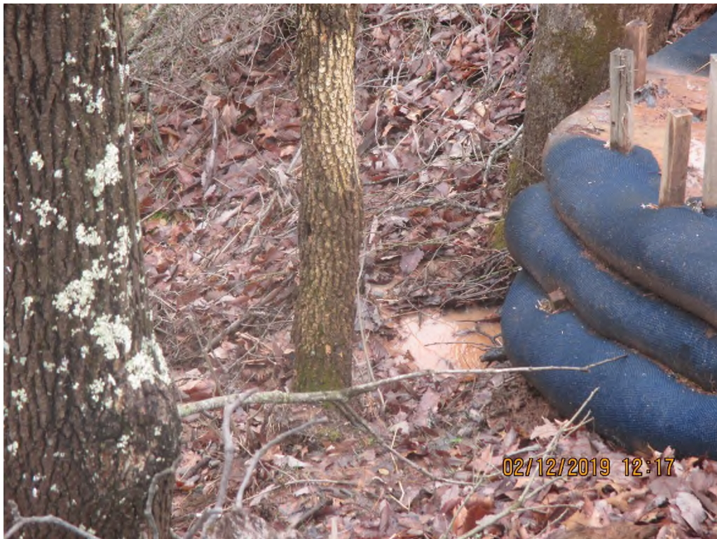
SLW flowing under controls at station number 5359+00 and past LOD
