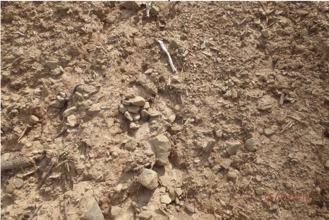
Areas of disturbance that were temporarily stabilized in December that have not germinated and have not been reseeded in the Taylor Drain watershed.
