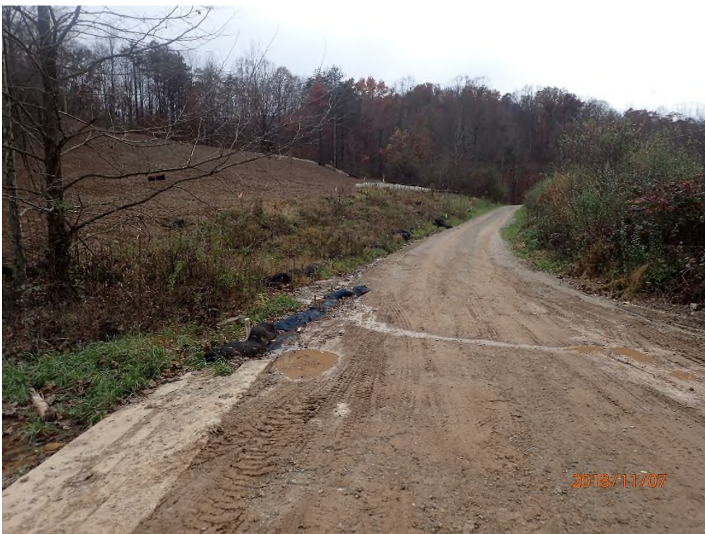
Sediment leaving the project on nearby access road.
