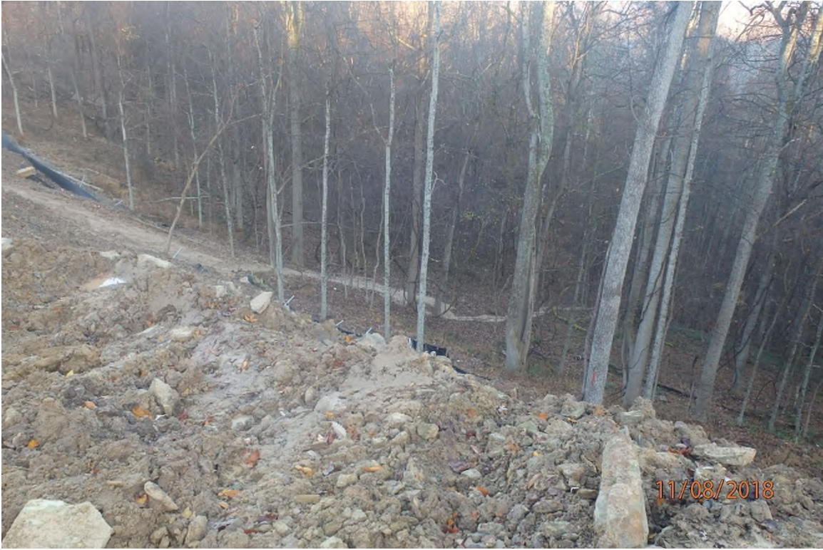
Slip and associated mud flow adjacent to 2822+00.
