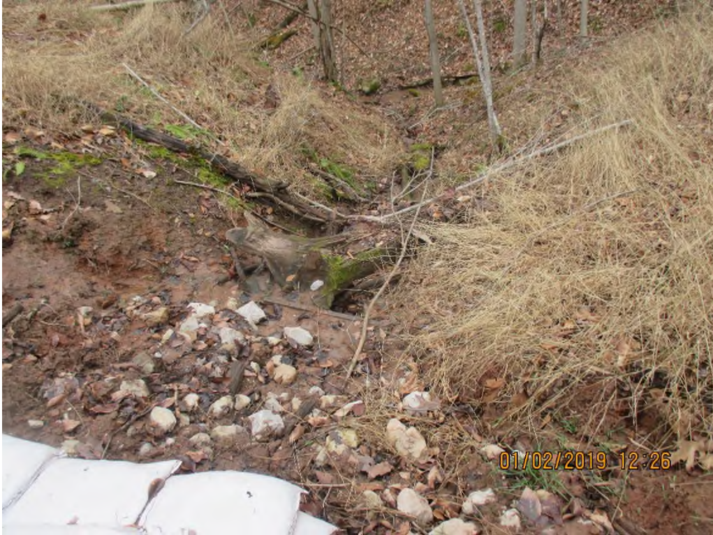
Discharge point at Silt Fence labeled as 24 on North slope that flows into UNT of Grasslick Creek.
