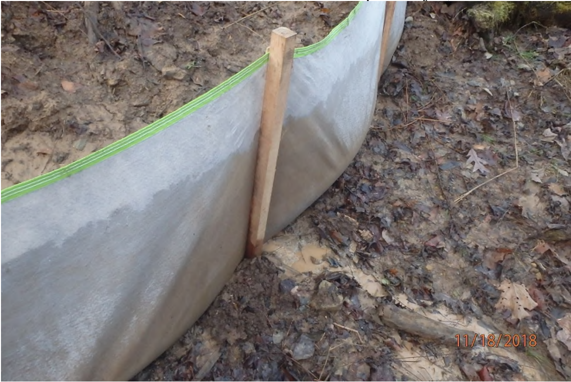
Improperly installed perimeter control allowing sediment laden water to bypass under the device on the offsite slip near 2822+00.
