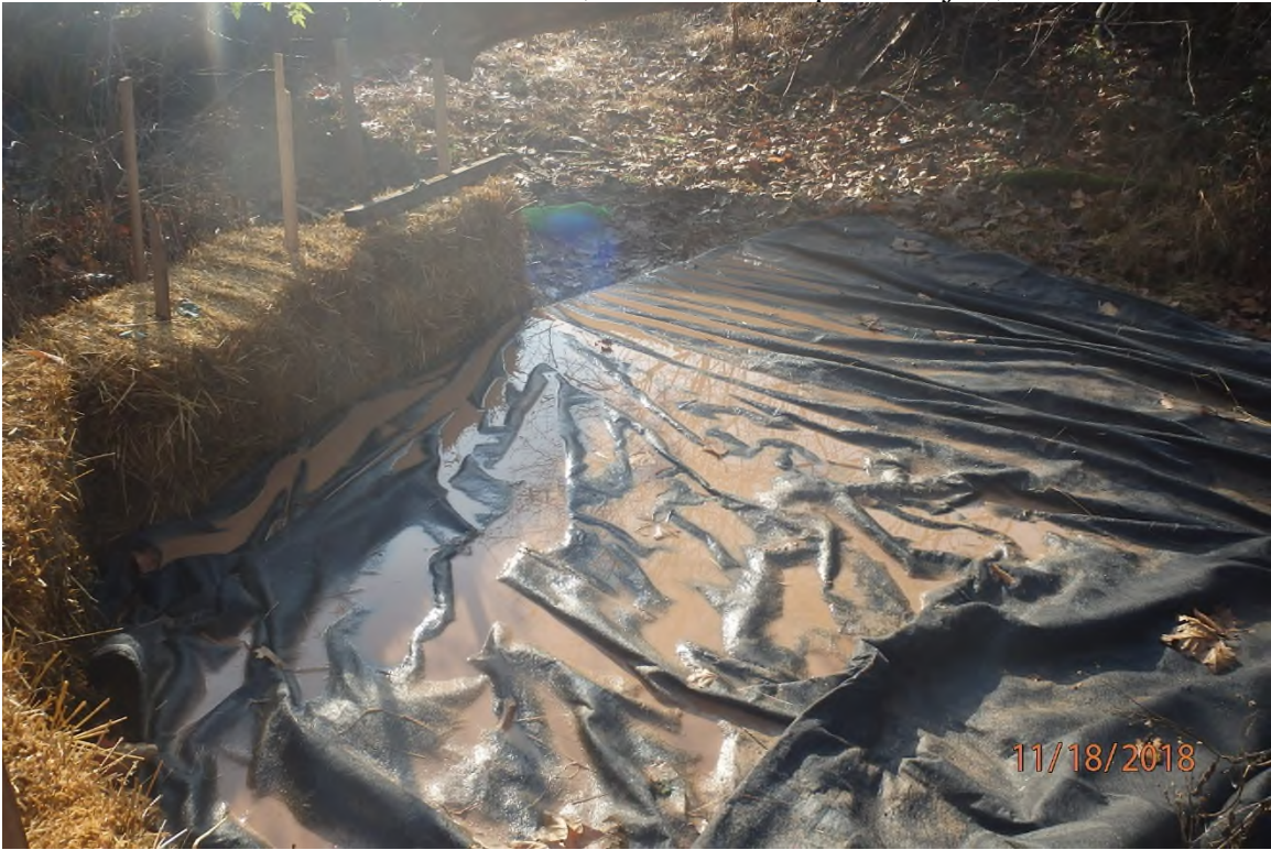
Dewatering bag associated with pipe trench dewatering adjacent to the SDOG048 stream crossing.
