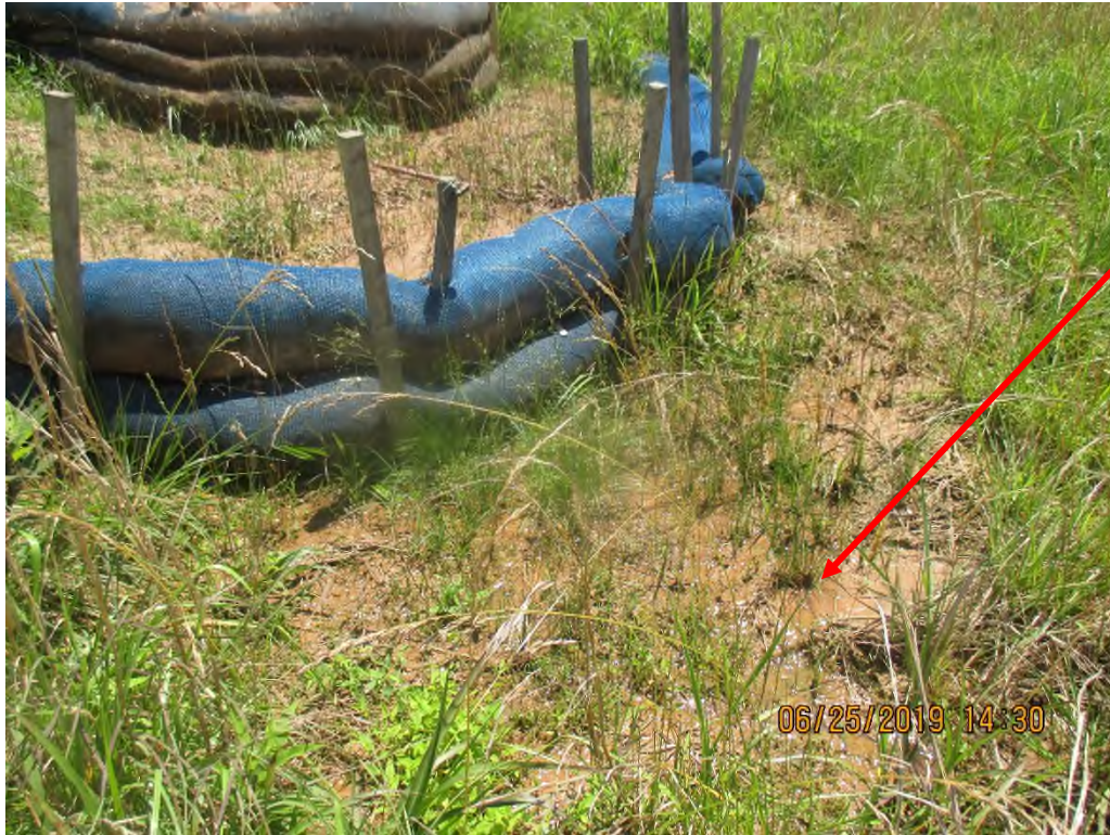
Sediment deposits past controls and LOD at station No. 5638+46. Deposits present above impacted pond.
