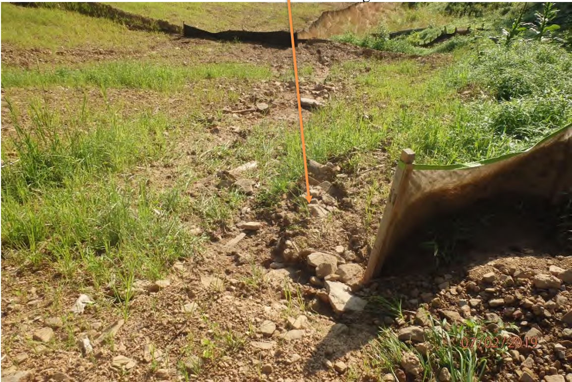
Associated fill slope erosion.
