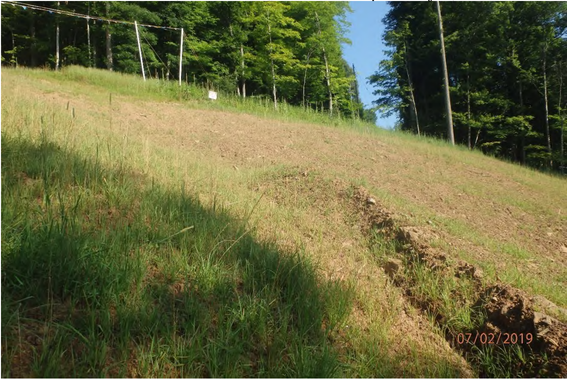
Improperly installed water bar in the Sugar Run watershed. Water bar does not extend across the entire disturbed width of the right of way as indicated in the approved SWPPP.
