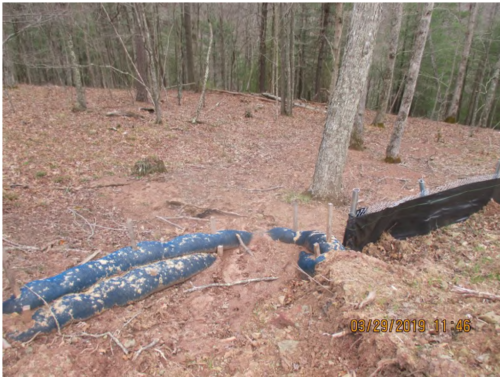
Waterbar terminus above stream SWIF-057 near station #5163+50. Sediment overwhelming controls and being deposited past LOD.
