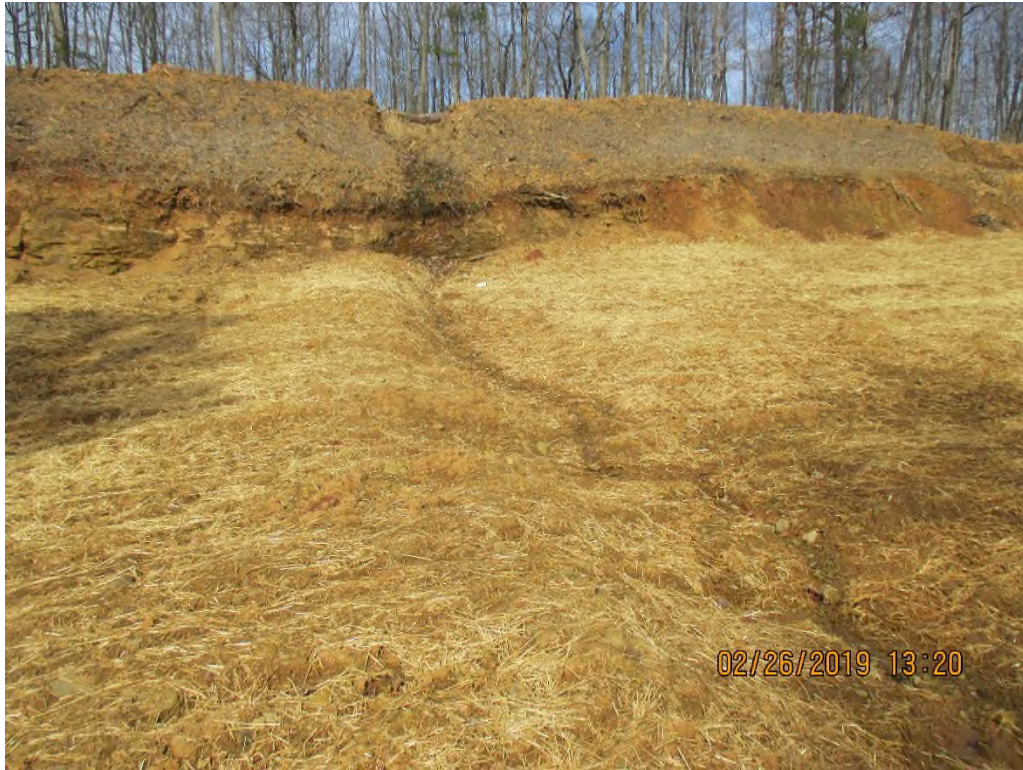
Topsoil pile eroding due to seep, entering waterbar, and causing erosion at station #6760+00
