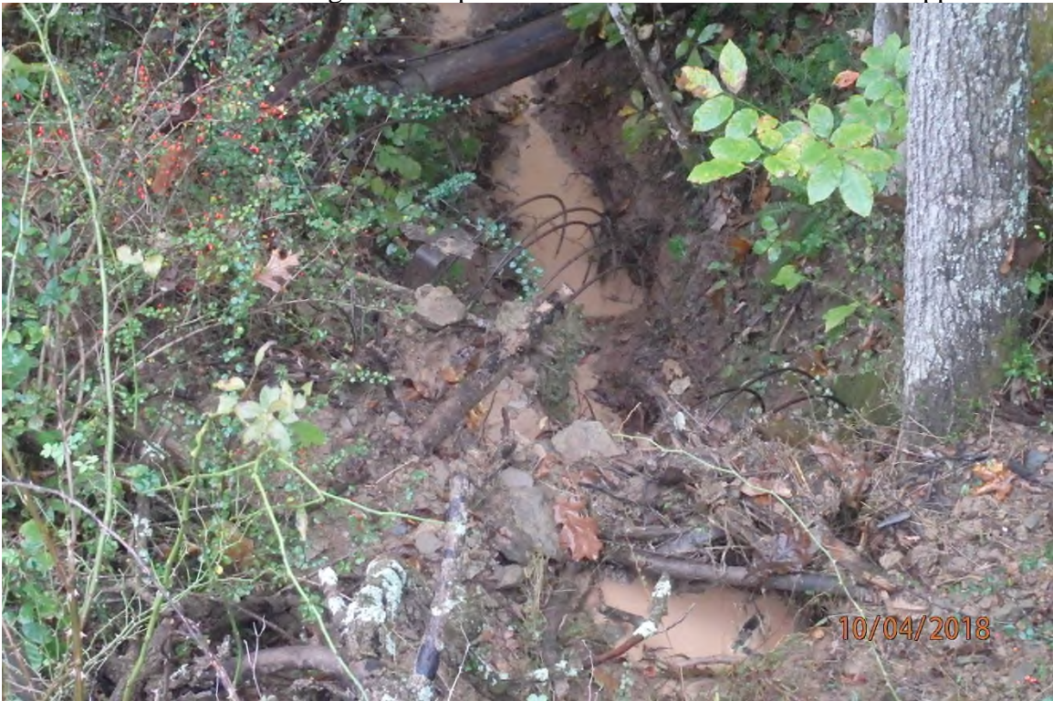
Sediment laden water leaving the site and CNA distinctly visible settleable solids in UNT McElroy Creek (SDOI201).
