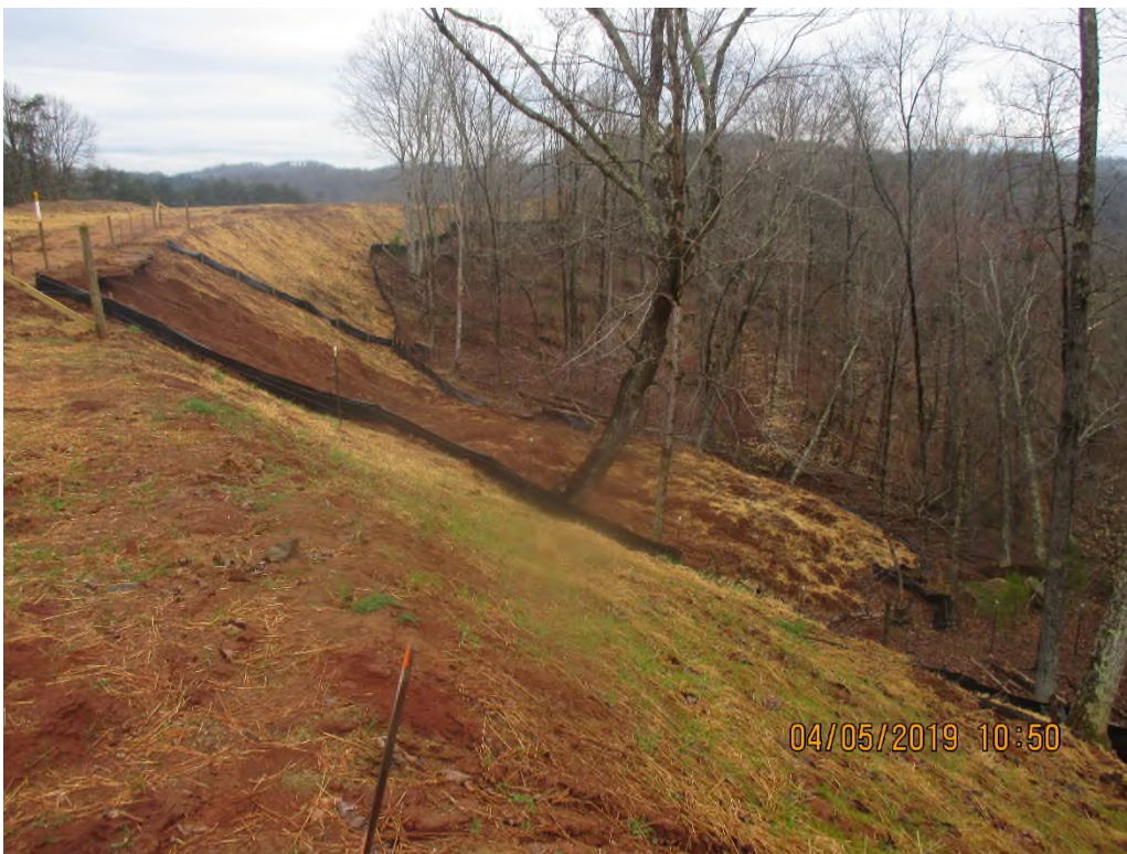
Slip that was reported at station #6810+00.
