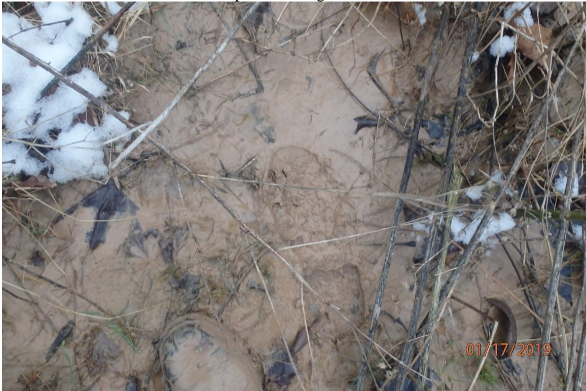
Sediment deposits located outside of the original project area that originate from the rock filtration device due to the lack of an installed sediment basin as indicated in the approved SWPPP.
