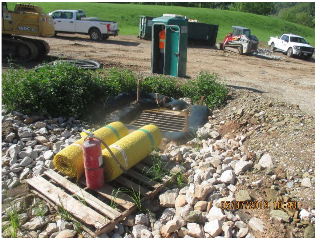
Drop inlet below sediment ponding. Sediment laden water was entering this drop inlet.
