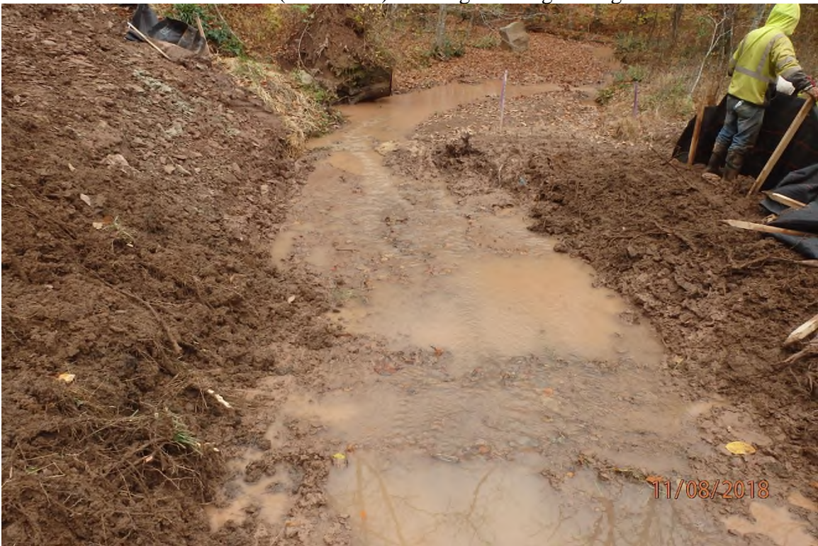
CNA distinctly visible settleable solids in UNT Left Fork of Arnolds Creek (SDOG040) (39°13.294' X 80°46.957').
