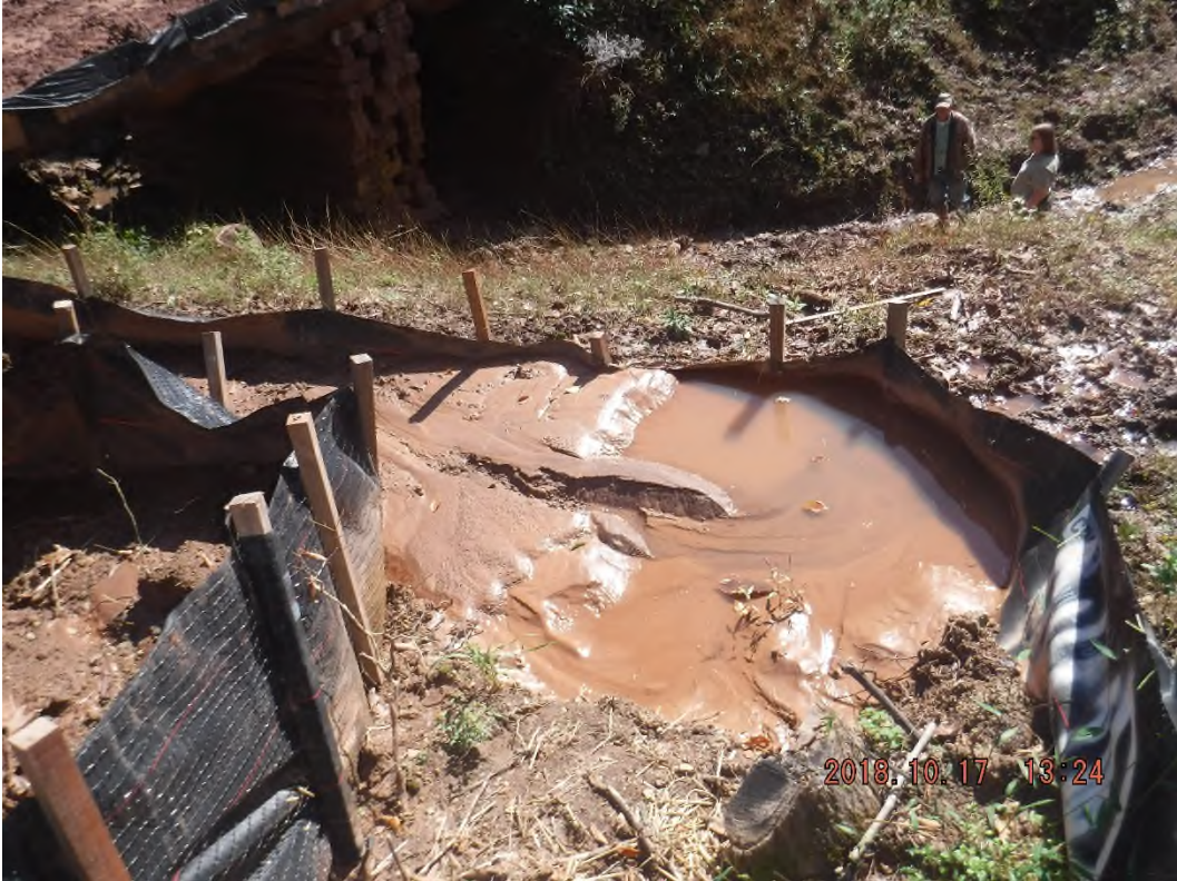
Sediment build-up in silt fence at Station 6705+00.
