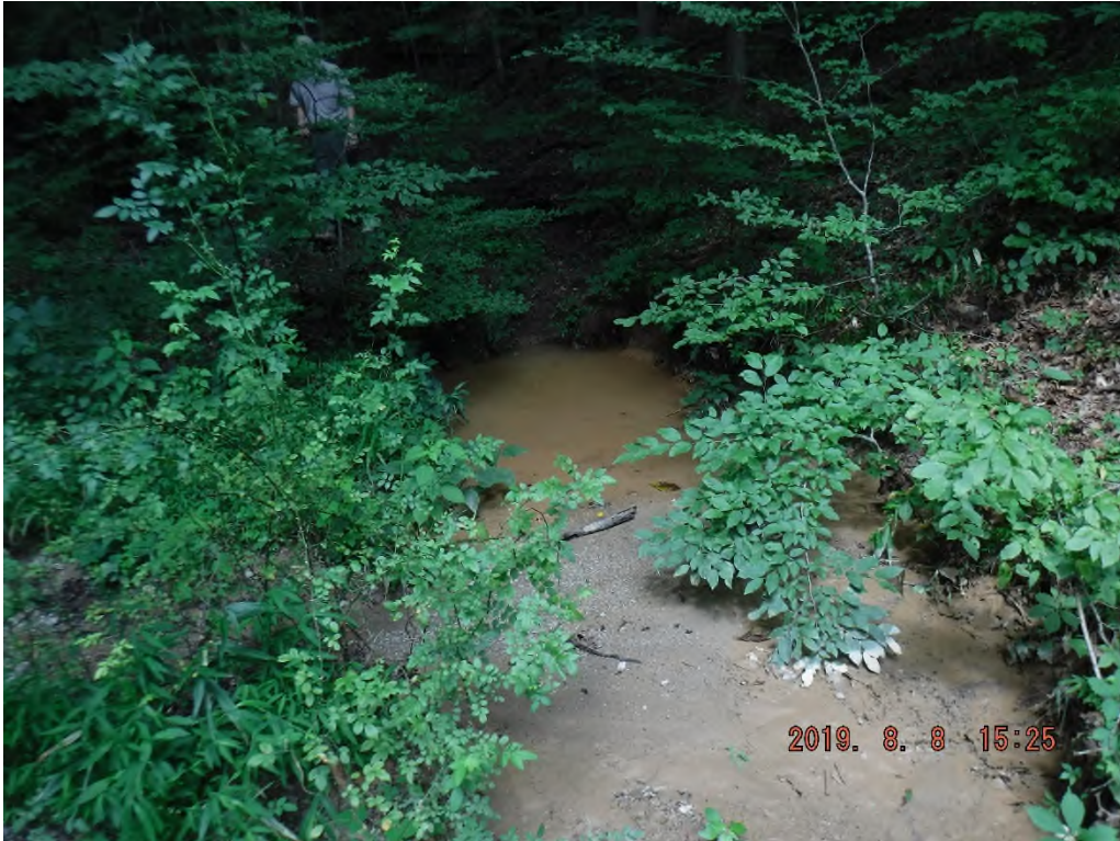
Culvert inlet below ROW on east side filled with sediment from runoff.
