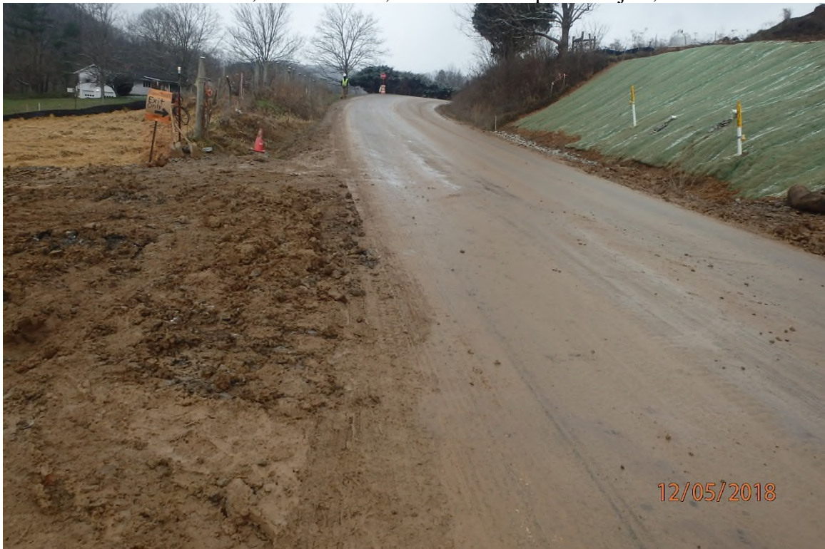
ARDO008 / WV18 crossing accesses showing the lack of a stable construction entrance and the associated track out/slick film of mud that originates from site.
