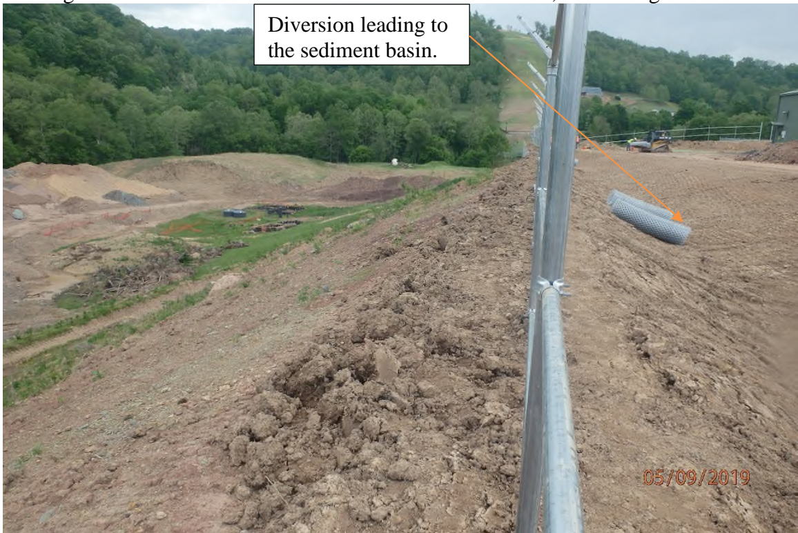
Diversion leading to the sediment basin that has not been stabilized, even though the site is in Phase 3.
