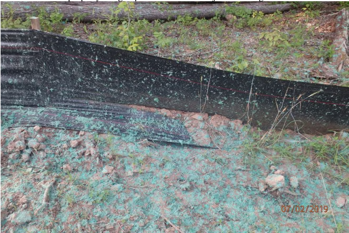
Improperly installed perimeter control in the Sugar Run watershed.
