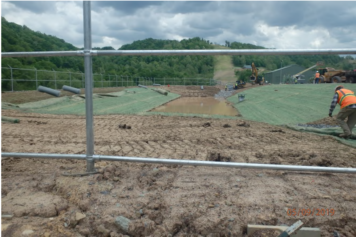
Crews working on stabilization of the area around the sediment basin, even though the site is in Phase 3.
