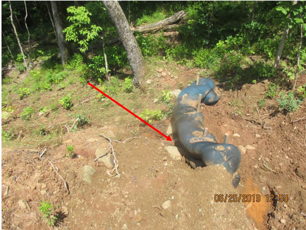
South of Station No. 5396+00. Erosion on slope above Munchausen Road Crossing leading toward waterbar and perimeter controls. Controls in need of maintenance. Arrow depicts where controls are undercut.
