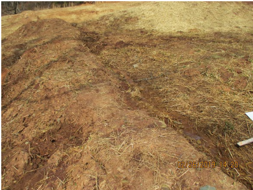
Waterbar at station #6730+05.
