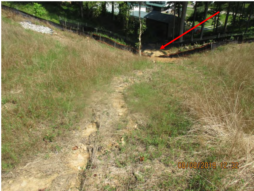
Drainage point between two slopes where erosion was present. Arrow depicts controls overwhelmed with sediment.
