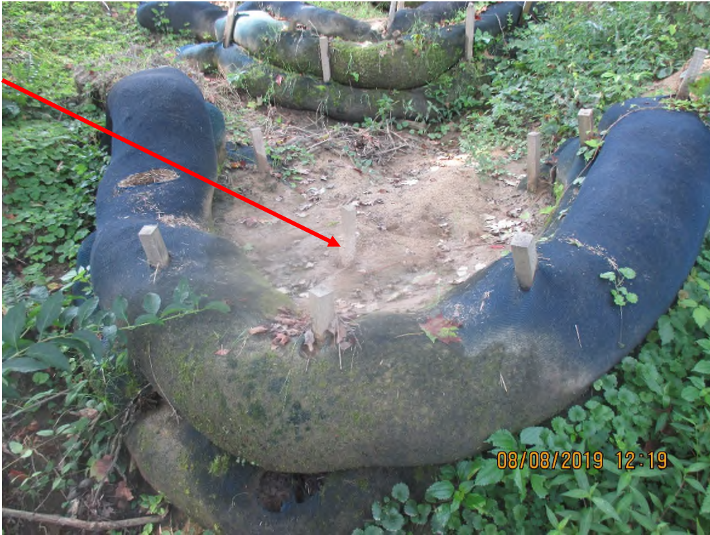
Perimeter controls overwhelmed with sediment and not being maintained.
