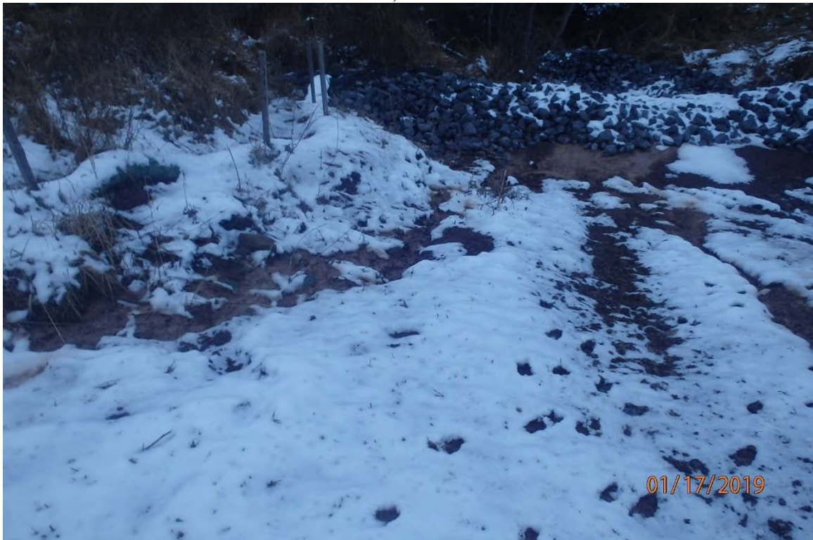
Concentrated flow from the installed truck wash being directed over an unprotected fill slope.
