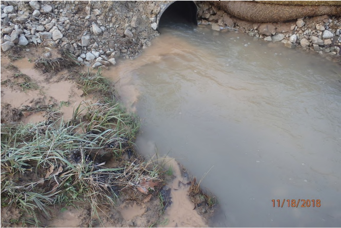
CNA distinctly visible settleable solids in Georgescamp Run (39° 15.092' X 80° 43.970') on ARDO008.2 due to a bypass from an improperly installed perimeter control.
