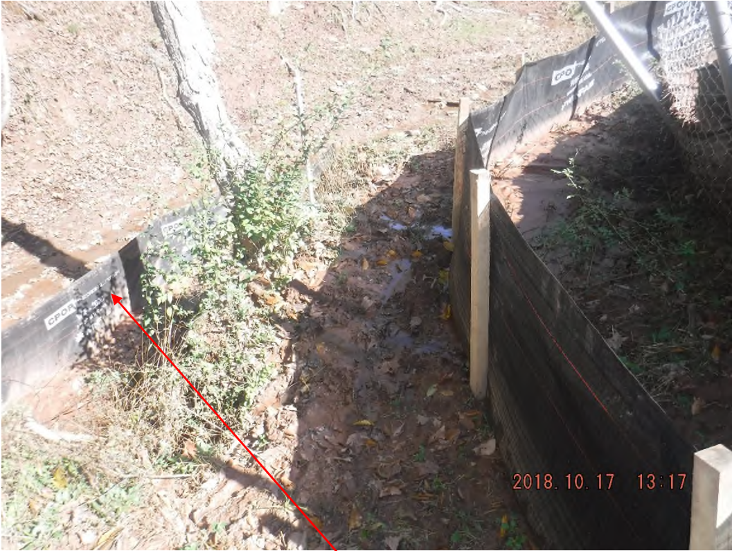
Silt fence that was installed in the stream after a rainfall event.
