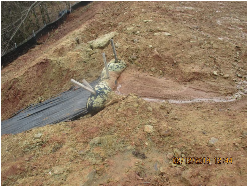
Above mentioned waterbar terminus at top of slope near station #5376+00
