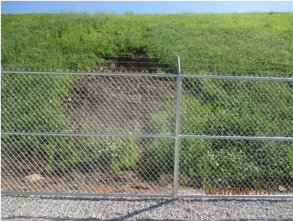
Slip occurring on East side of compressor station above pad.
