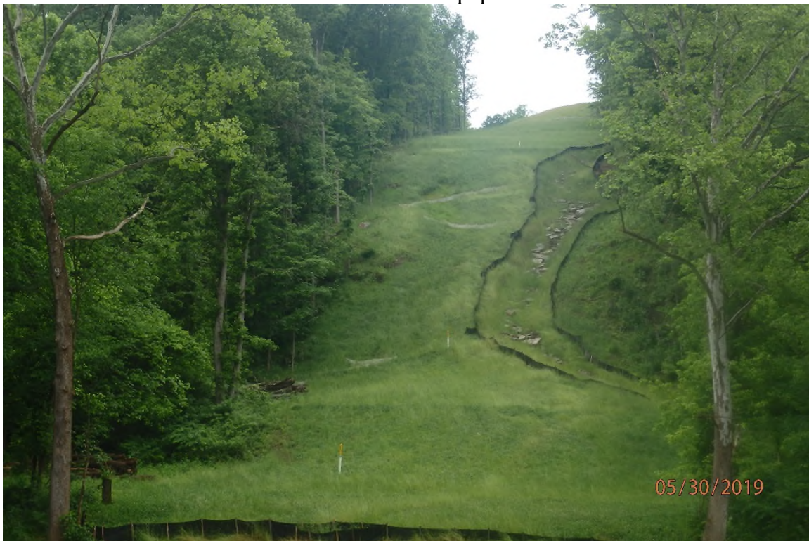
Water bars in the Meathouse Fork watershed that have been temporarily repaired with silt fence and need to be reestablished with equipment.
