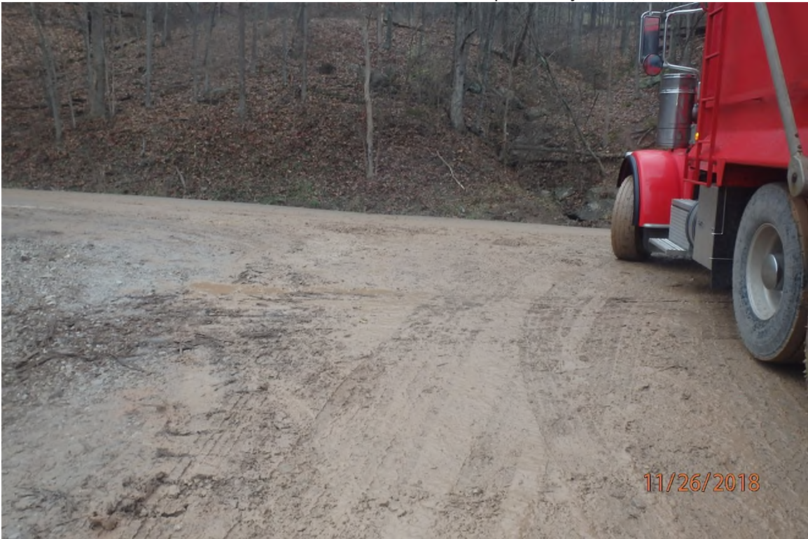
Construction entrance at the WV 23 crossing showing the lack of a stabilized entrance.
