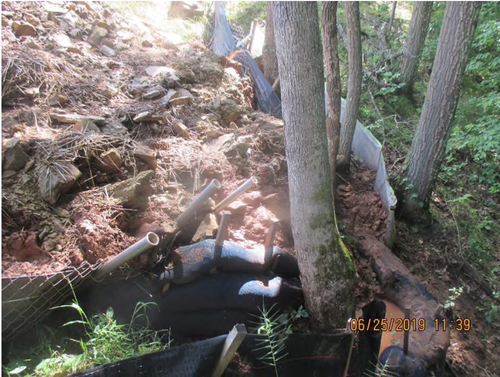
Perimeter controls overwhelmed with sediment downslope of slip area at station No. 5355+67
