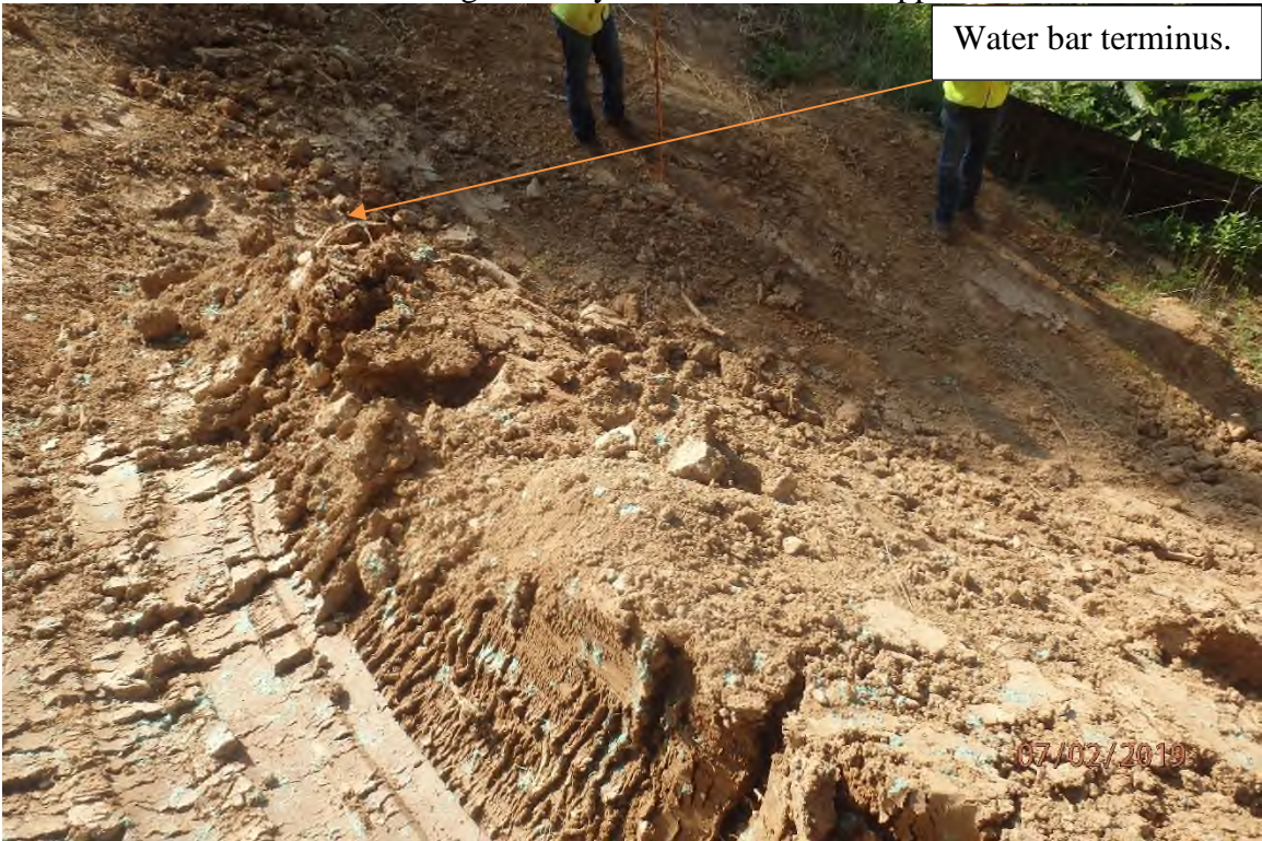
Improperly installed water bar in the Sugar Run watershed. Water bar does not extend across the entire disturbed width of the right of way as indicated in the approved SWPPP and is placing concentrated flow stormwater over an unprotected fill slope.
