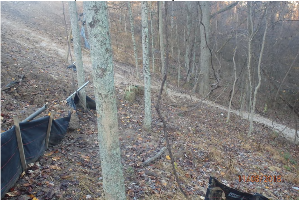
Slip and associated mud flow adjacent to 2822+00.
