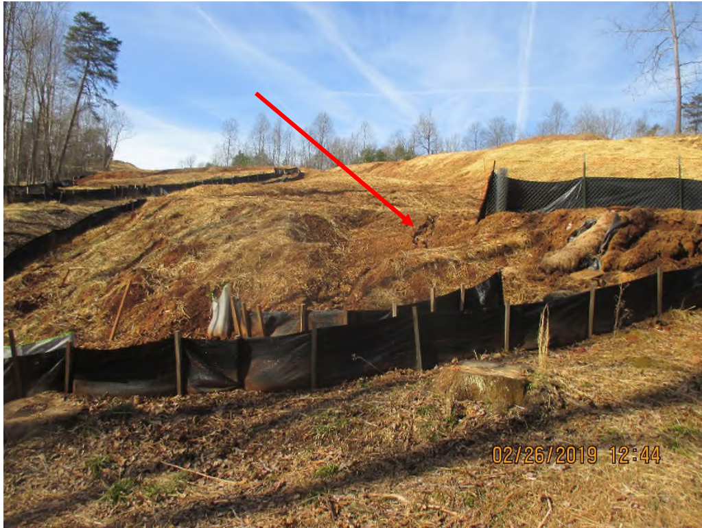
Controls above Stream SJAD-008 near station #6655+00 (per SWPPP). Arrow depicts where erosion is occurring above controls on slope.
