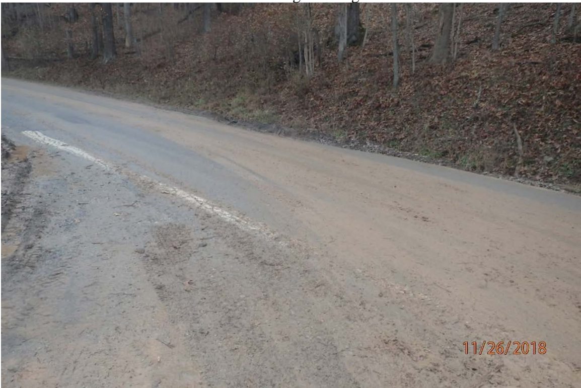
Construction entrance at the WV 23 crossing showing the lack of a stabilized entrance and the associated track out onto the public road.
