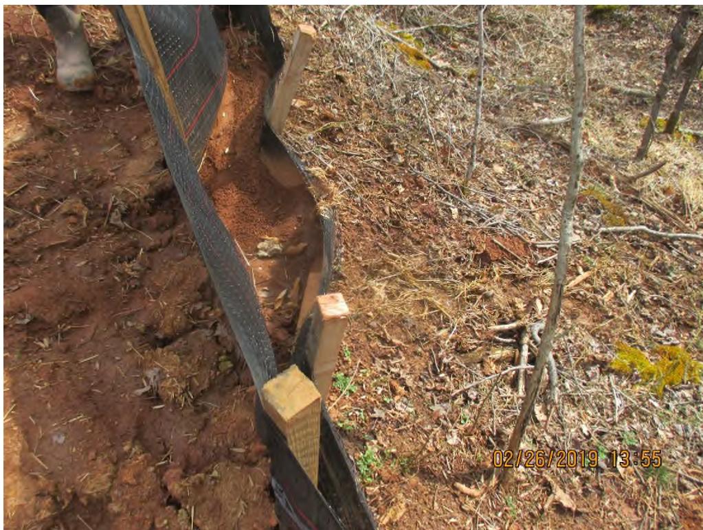
Near station #6742+60. Sediment being deposited against perimeter control and evidence of sediment being deposited past control.
