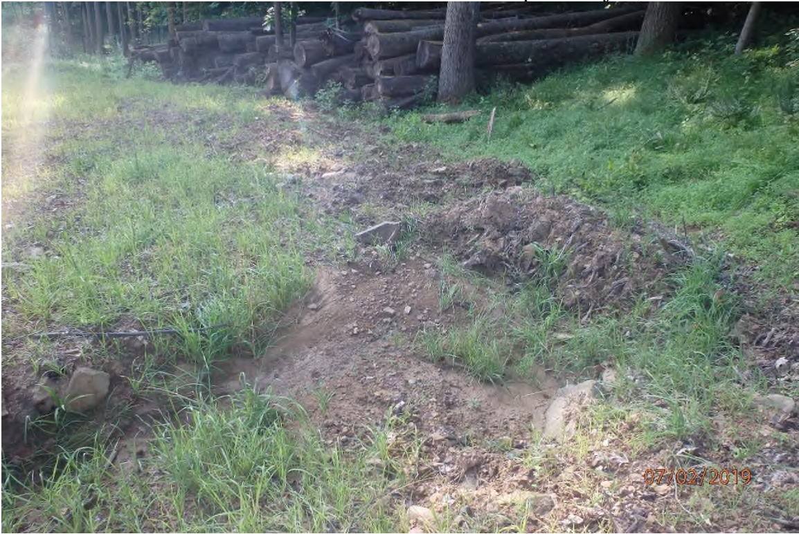
Water bar that lacks the water bar terminus BMP indicated in the approved SWPPP in the Sugar Run watershed.
