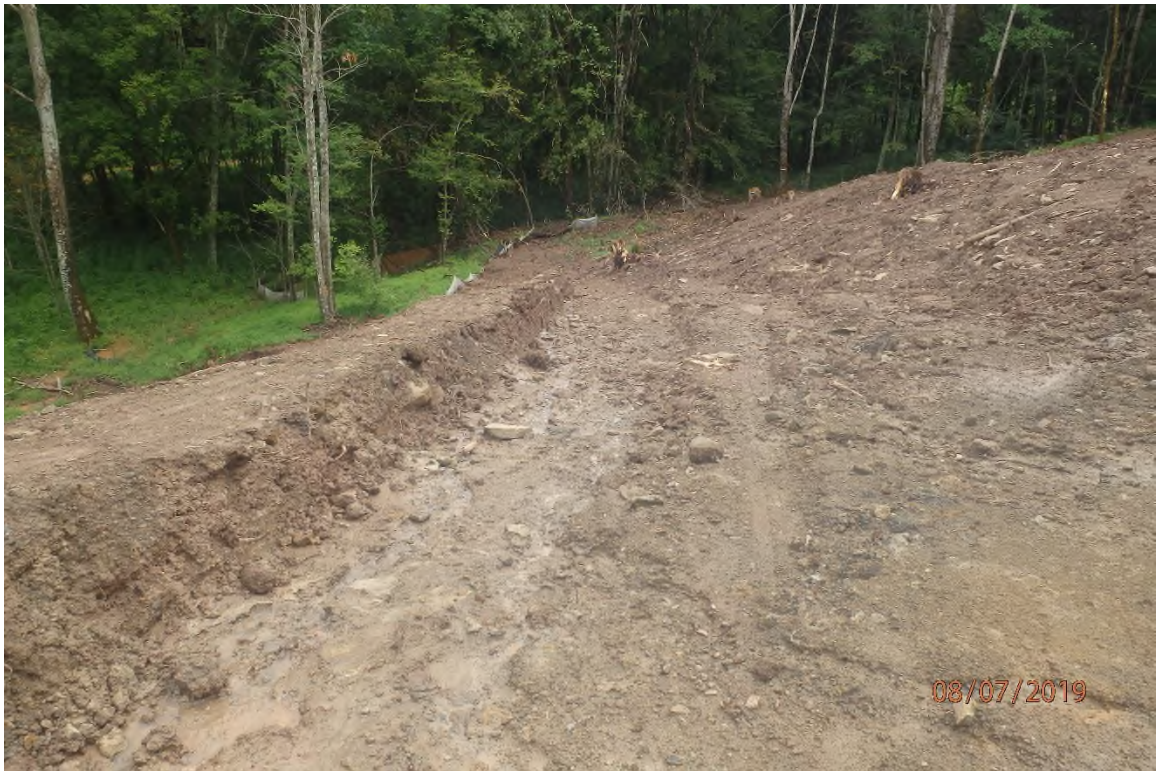
Water bars that were installed at steep angles in the Riggins Run watershed.
