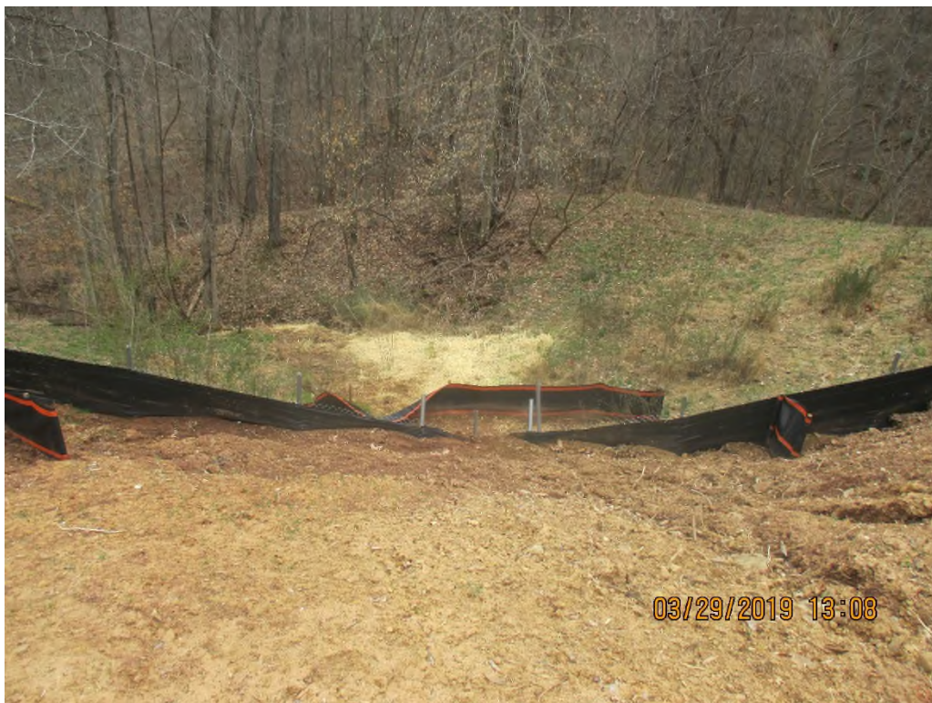
Downslope of controls near station #5180+43. Erosion occurring between and around controls leading to perimeter controls being overwhelmed with sediment.
