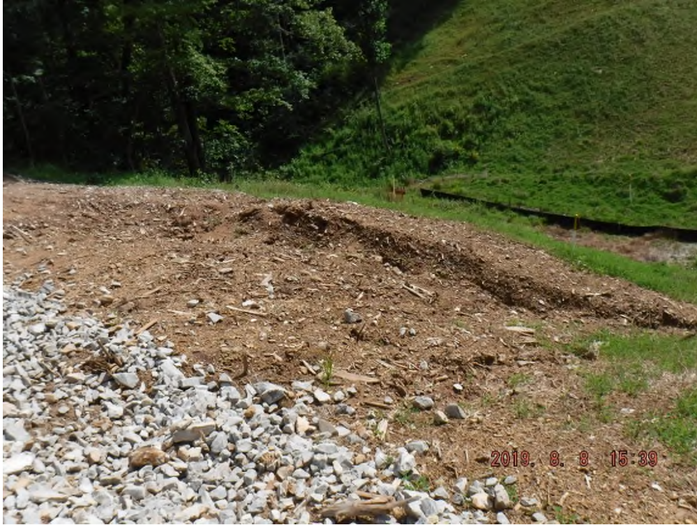
Water bar not installed correctly.
