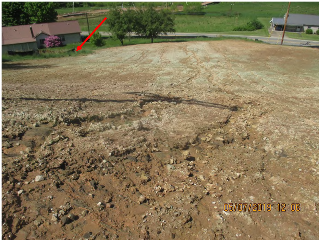
West slope facing perimeter controls and route 21 above slope drain outlet. Erosion present on slope. Arrow depicts slope drain outlet.
