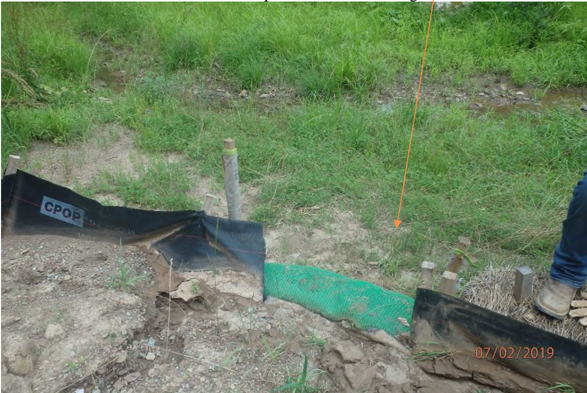
Perimeter control that was recently altered. An inequivalent 8" compost filter sock is being utilized to replace a concentrated flow silt fence in an area where the silt fence had previously failed.
