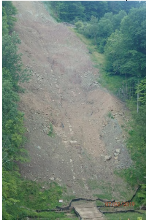
Erosion gullies that run from the top of the slope to the bottom of the slope adjacent to UNT Left Fork of Arnolds Creek (SDOG040) due to poor maintenance of installed water bars. Concentrated flow stormwater is overwhelming the installed perimeter controls at the base of the hill.
