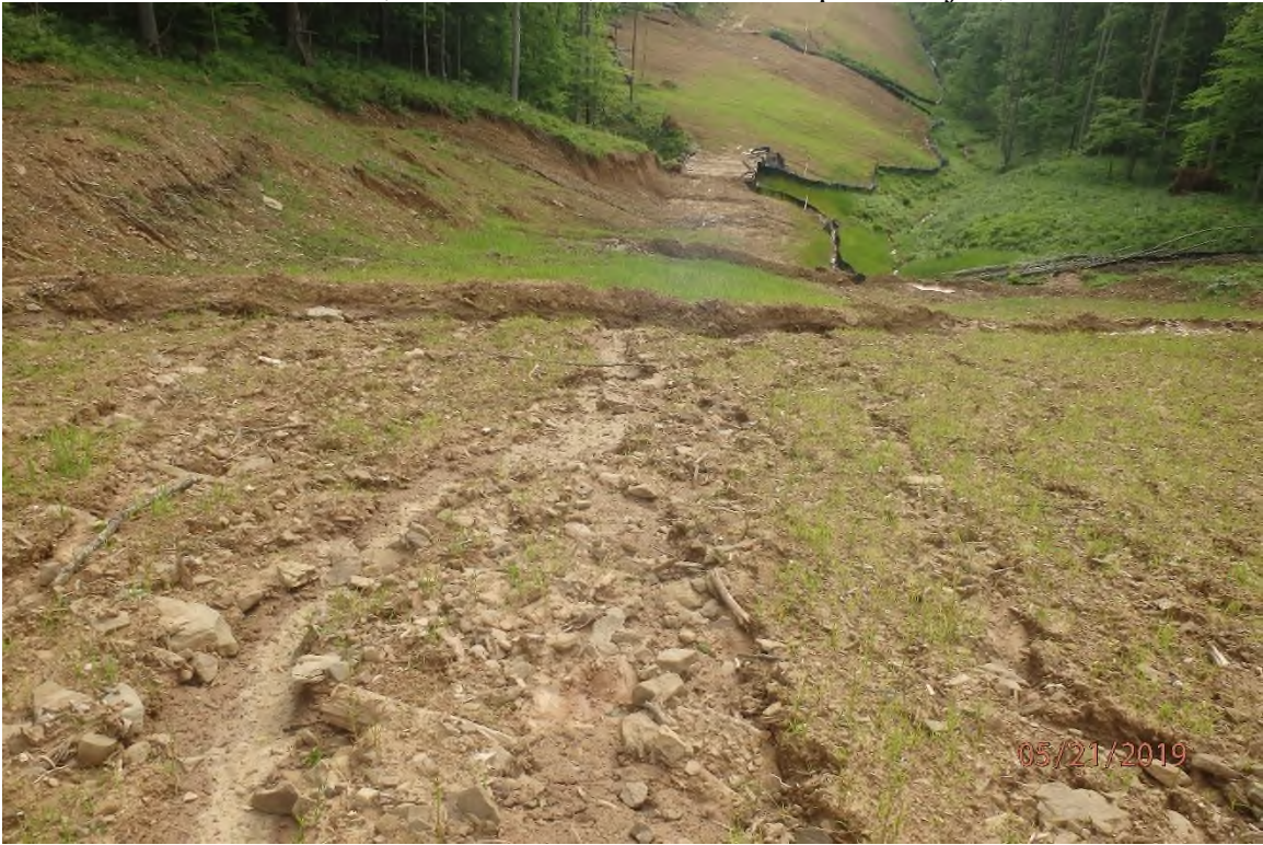
Unmaintained water bars in the UNT Sugar Run watershed.
