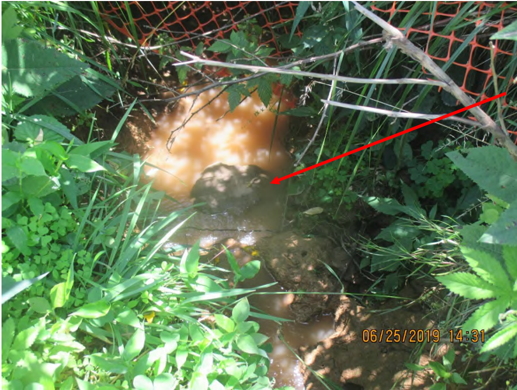
Impacted pond culvert outlet conveying sediment laden water towards Stream SROC 029 at station No. 5638+47. Arrow depicts culvert outlet.
