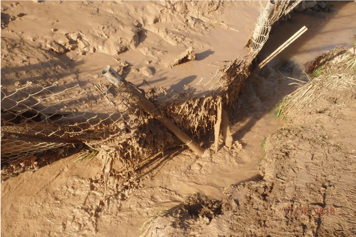
Perimeter control that has been overwhelmed and is causing CNA deposits and a distinctly visible plume in UNT Georgescamp Run (39°15.182' X 80° 44.033').
