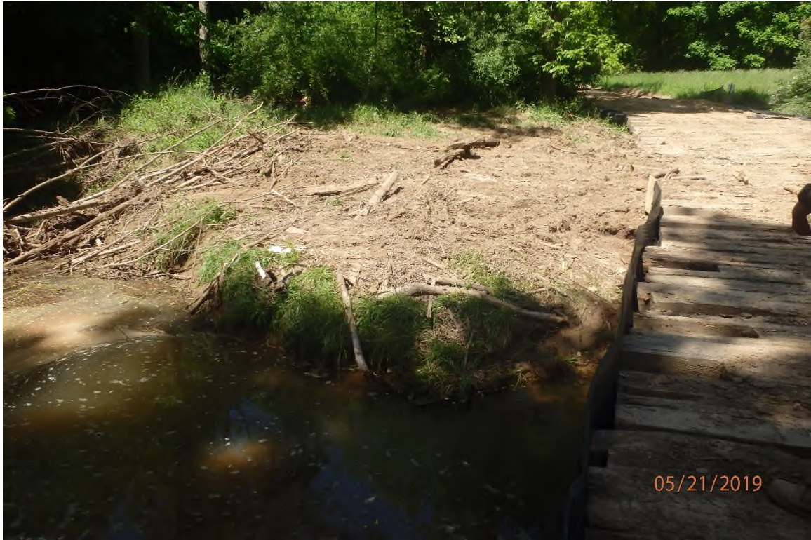
BMP that has been recently removed adjacent to ARDO009.1 and has not been replaced.
