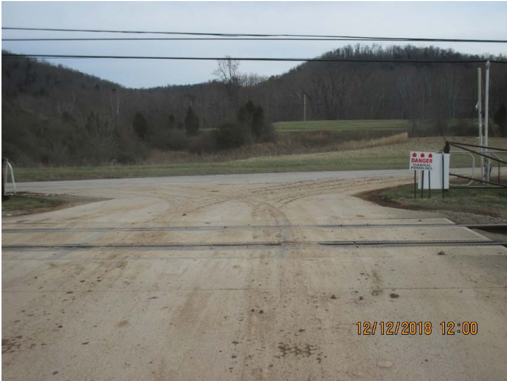
Facing Route 62. Tracking visible in both directions (East and West) along Route 62.
