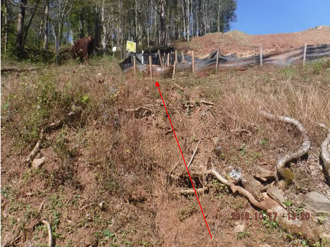
Station 6705+00, showing bulging silt fence.
