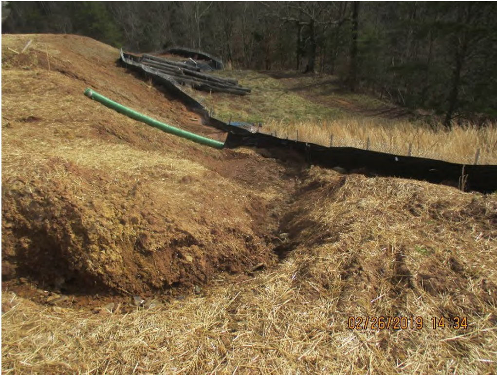
Waterbar terminus with gully erosion present leading toward perimeter controls near station #6727+53
