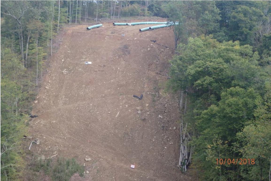
Improperly installed water bars and the associated fill slope erosion near SDOI008.
