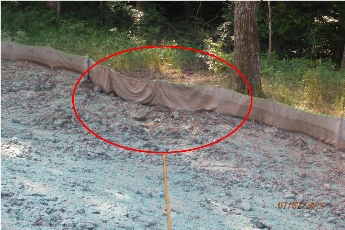
Recently maintained perimeter control adjacent to UNT Sugar Run (SDOH11).
