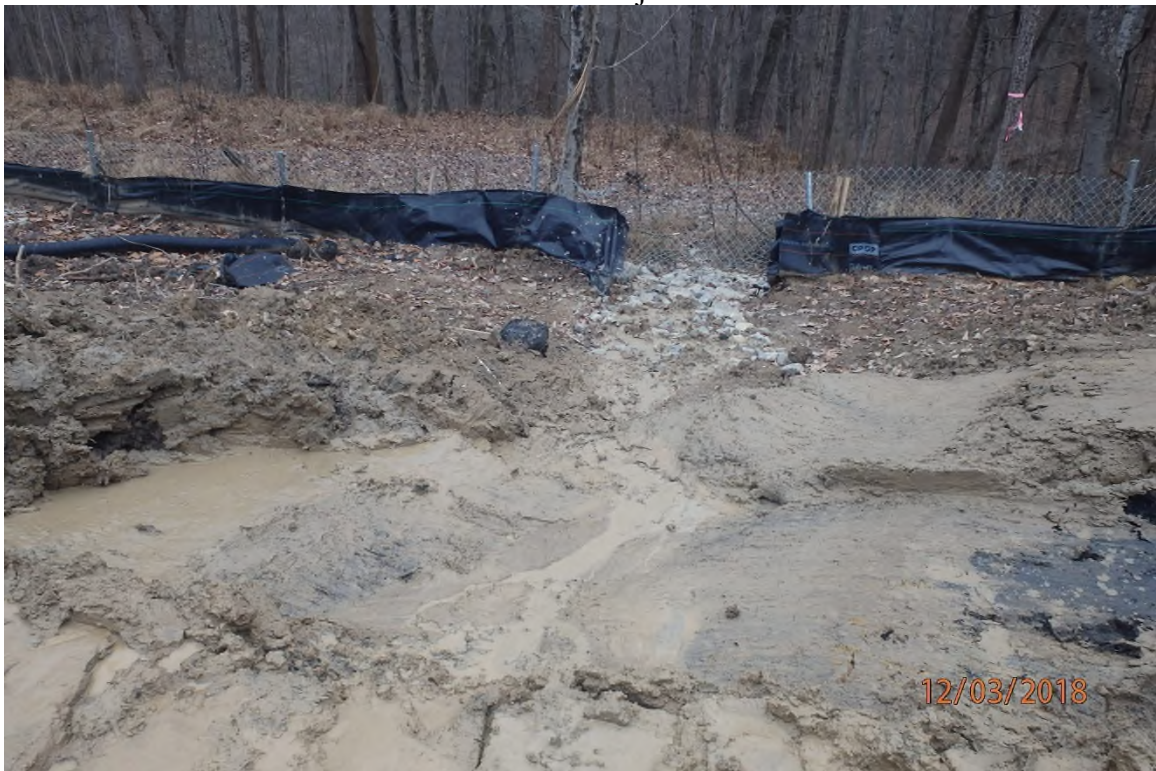
Project area adjacent to 2611+00 showing gaps in the installed perimeter control that allow sediment laden water to leave the site without going through an appropriate device.
