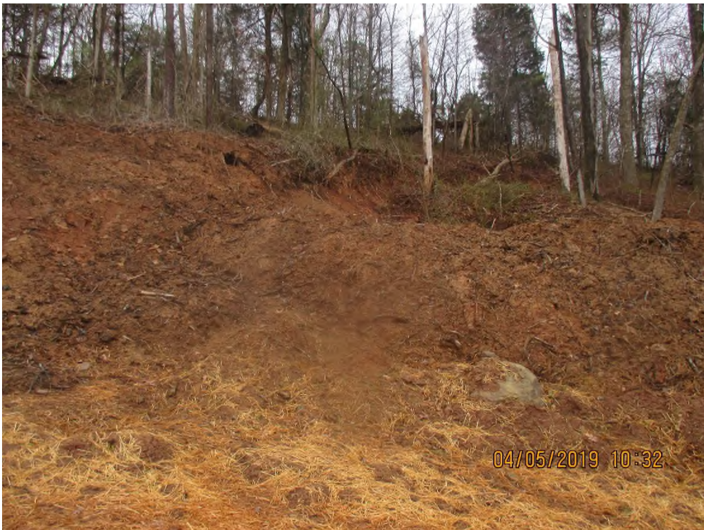
Slip upslope of MXP ROW at station #6792+40 slipping into ROW.
