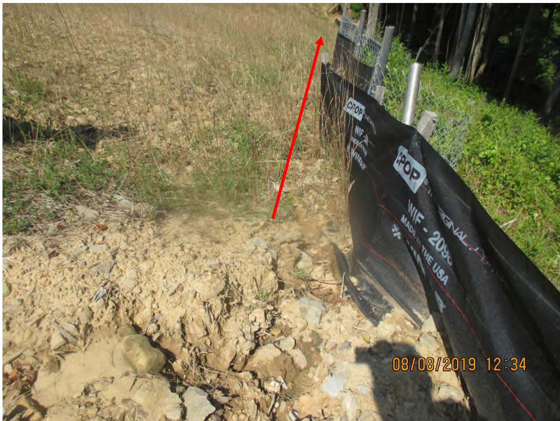
Arrow depicts where erosion was present along perimeter controls flowing towards drainage with overwhelmed outlet controls.
