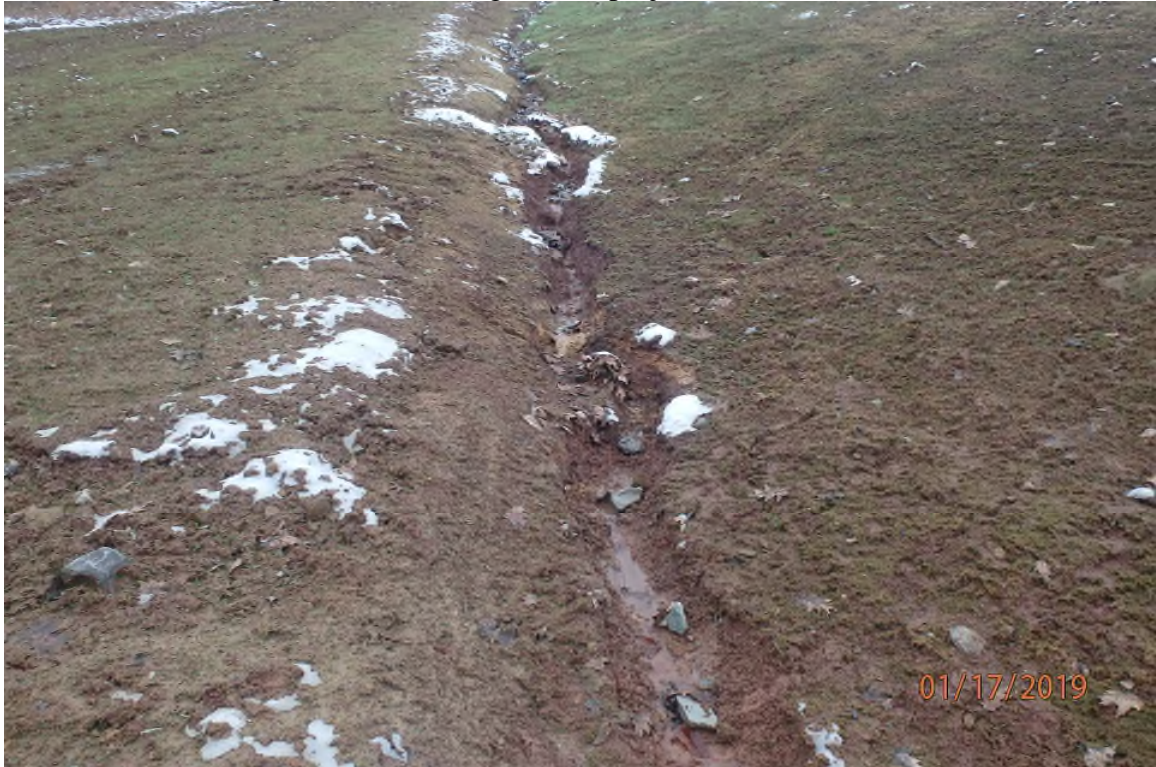
The installed diversion along the southern edge of the project that is eroded and in need of maintenance.
