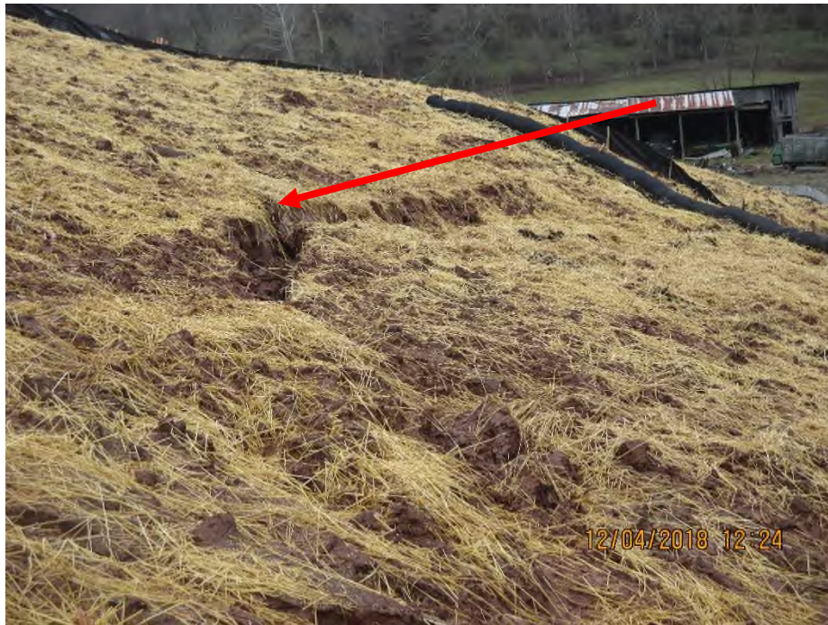
Area where slip was beginning to occur above stream SJAG 316 on 12/04/18.
