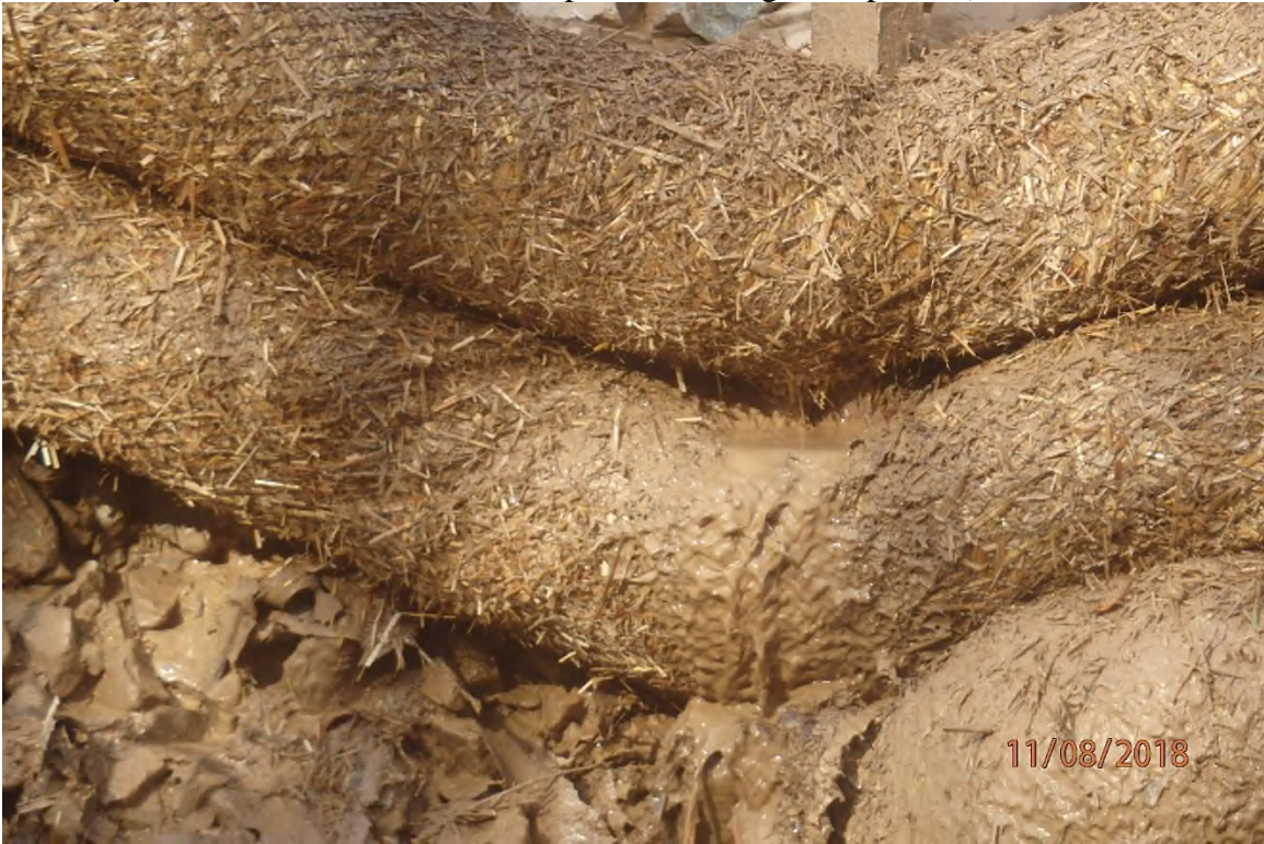
ARDO008.2 showing improperly installed controls that caused CNA.
