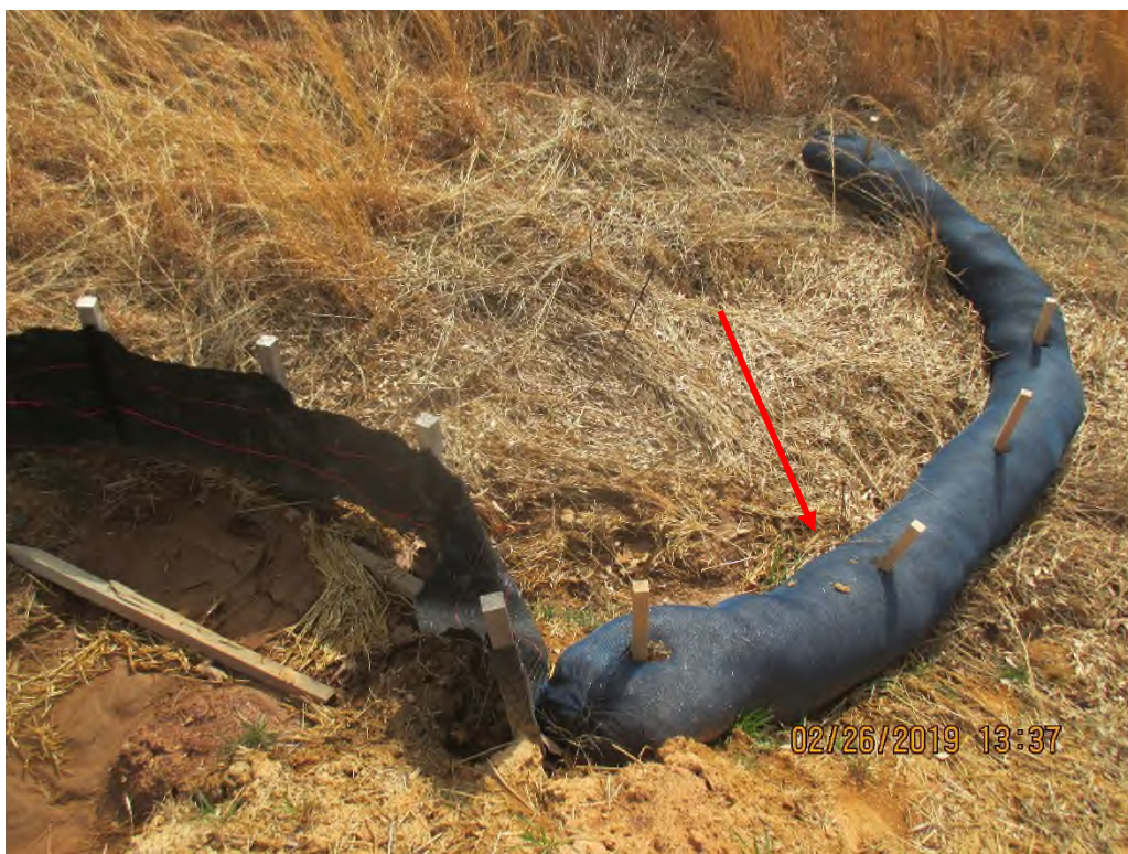
Waterbar outlet at station #6753+94. Arrow depicts where filter sock is undermined with small amount of deposits past control.
