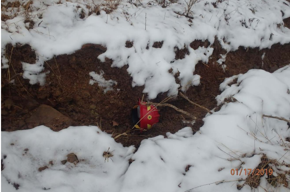
Slope that lacks adequate temporary stabilization in the northwestern portion of the project.
