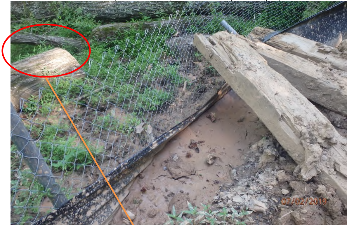
Perimeter control in need of maintenance at ARDO015.12.
