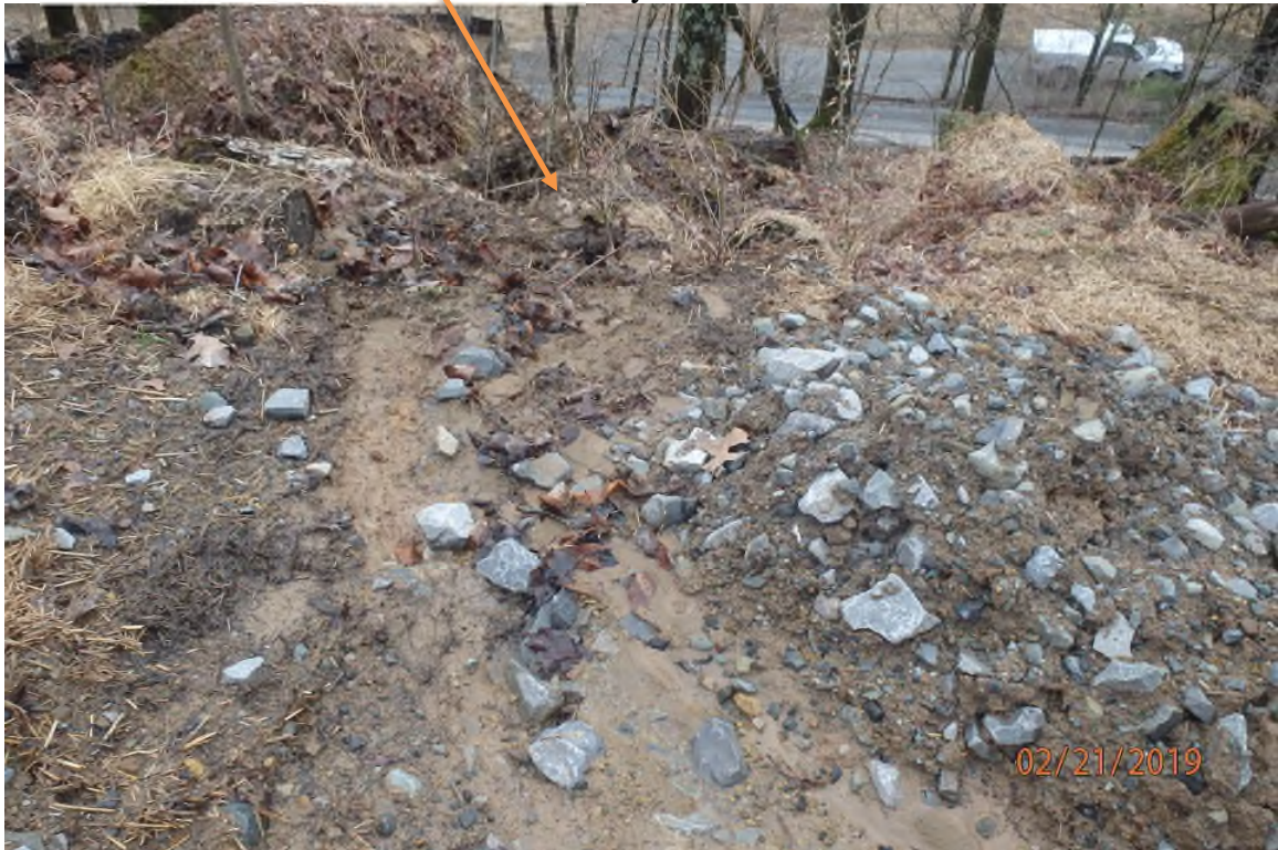
Water bar outlet on ARDO002.8 that lacks a water bar terminus BMP.
