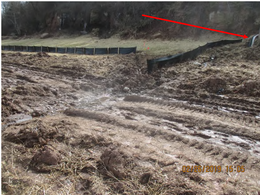
Saturated section of ROW impacting travel lane. Erosion and slips occurring downslope of station #6702+30. Slope drain installed at red arrow.
