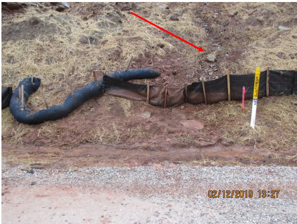
Sediment deposits present along Munchausen Road ditch station #5405+07. Erosion occurring above controls on ROW.
