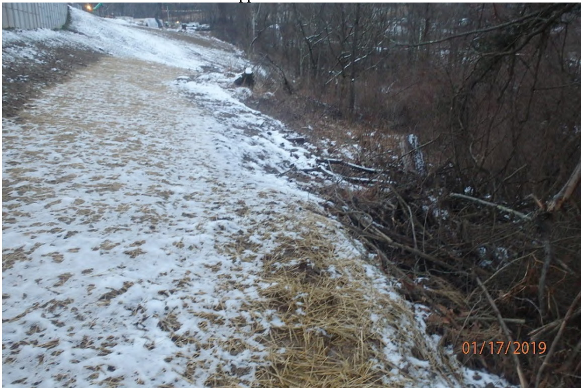
Northwestern perimeter of the project showing the lack of perimeter silt fence that is indicated in the approved SWPPP.
