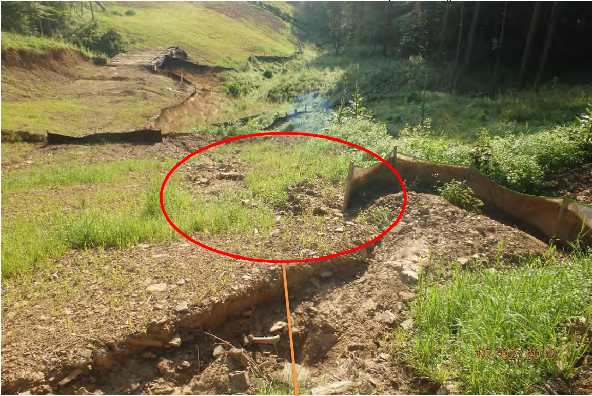
Water bar in need of maintenance in the Sugar Run watershed.
