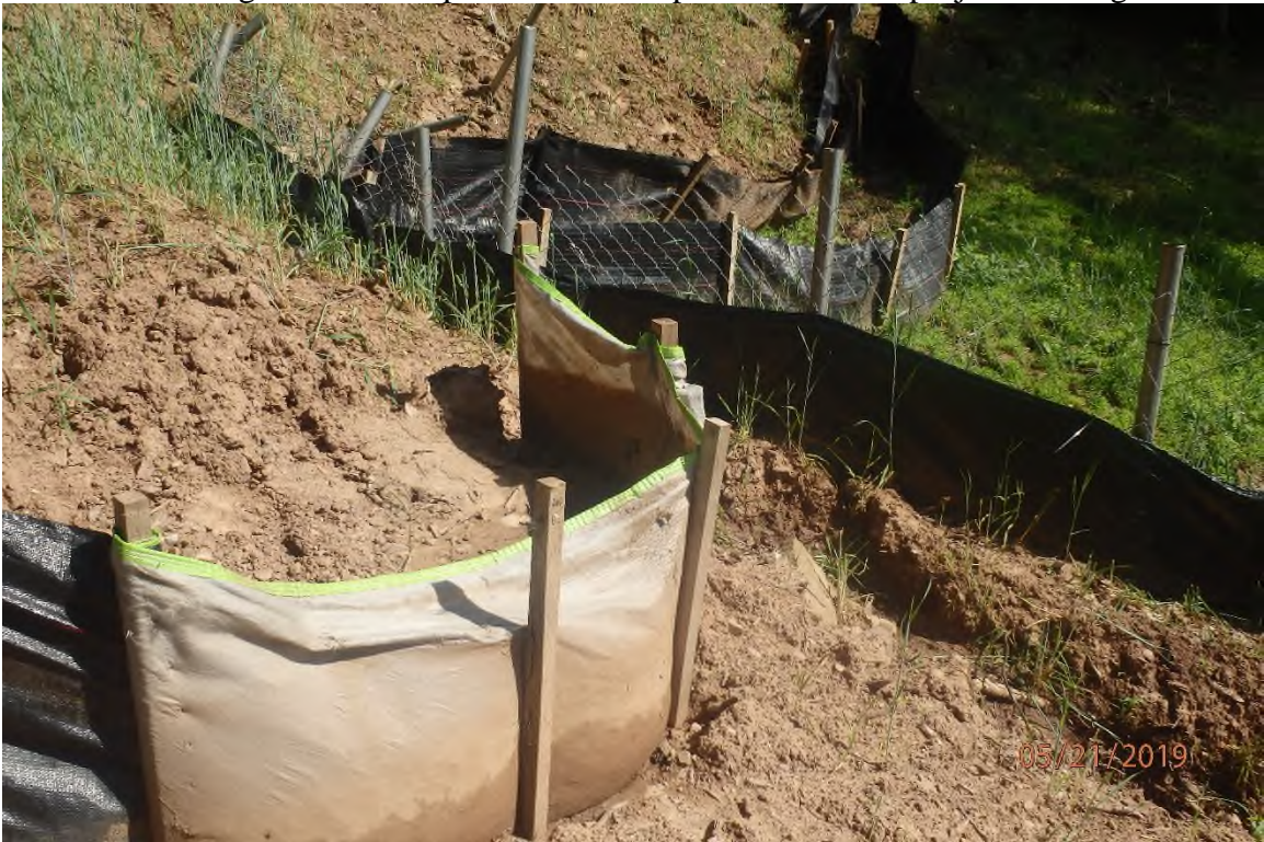
Improperly installed water bar in the Georgescamp Run watershed. Water bar installed at a steep angle and discharges over an unprotected fill slope instead of off project as designed.
