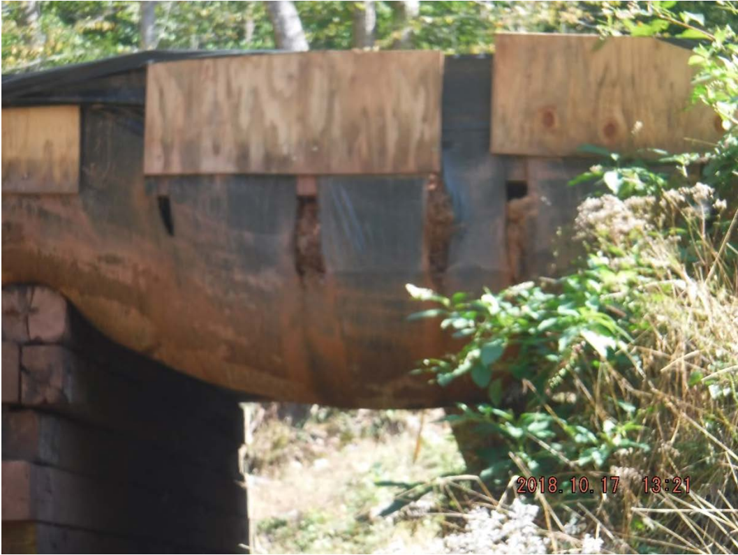
Sediment collected in fabric under timber mat bridge.
