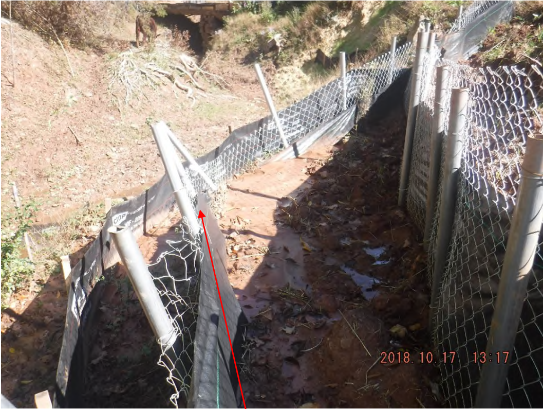
Sediment collected in silt fence.
