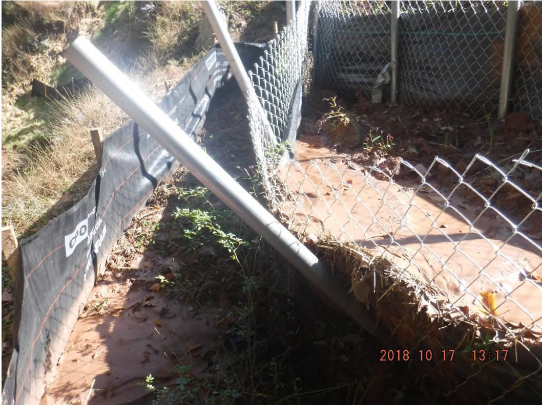
Sediment overtopping silt fence.
