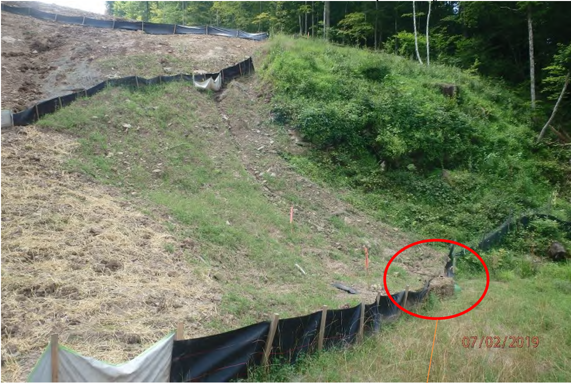
Area of concentrated flow that has caused fill slope erosion. Evidence of a recently altered perimeter control was noted due to the perimeter control being overwhelmed.
