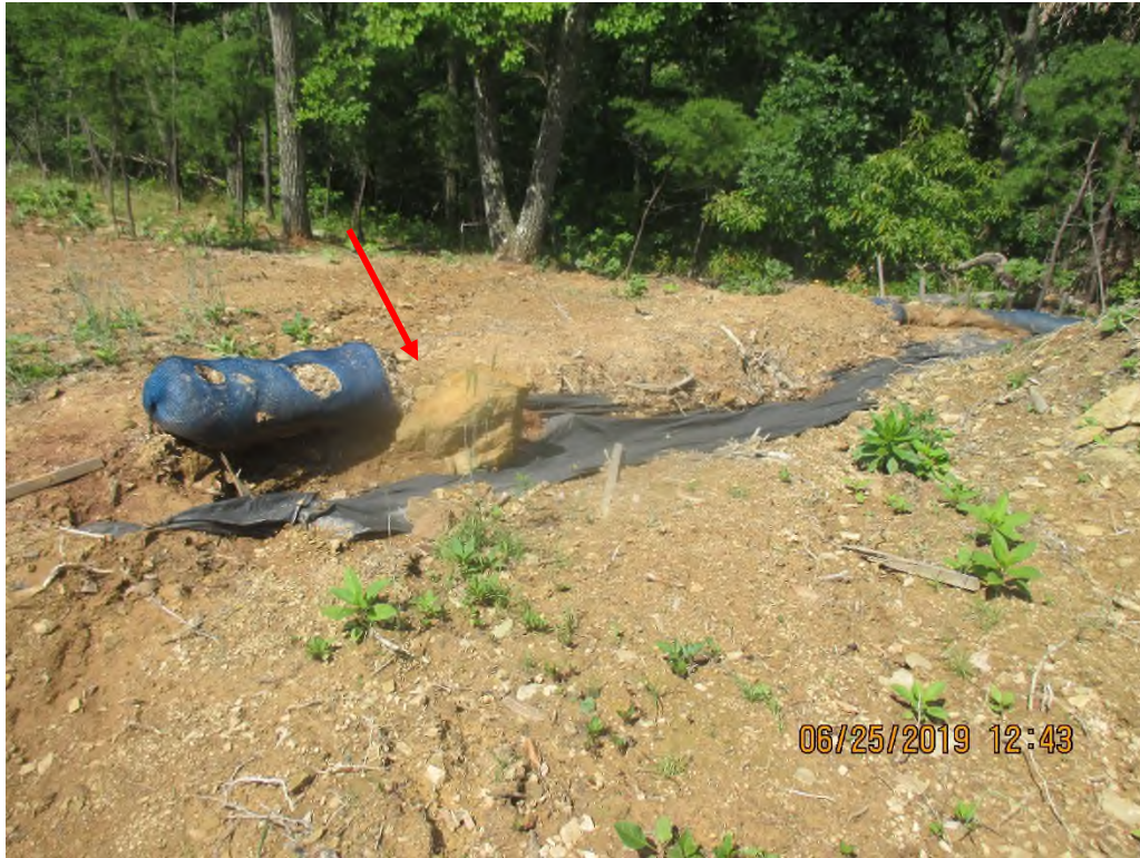
Waterbar terminating onto slope at station No. 5396+00. Arrow depicts where waterbar eroded out and sediment was flowing around controls.
