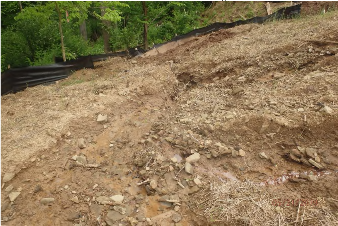
Unmaintained BMP in the UNT S. Fork of the Hughes River watershed.
