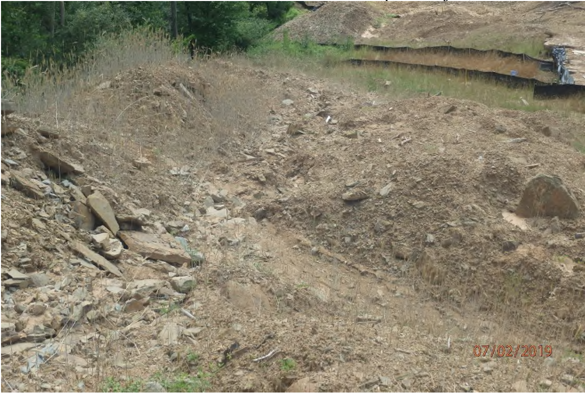
Improperly installed water bar in the Trap Run watershed. Water bar does not extend across the entire disturbed width of the right of way as indicated in the approved SWPPP and is placing concentrated flow stormwater over an unprotected fill slope.
