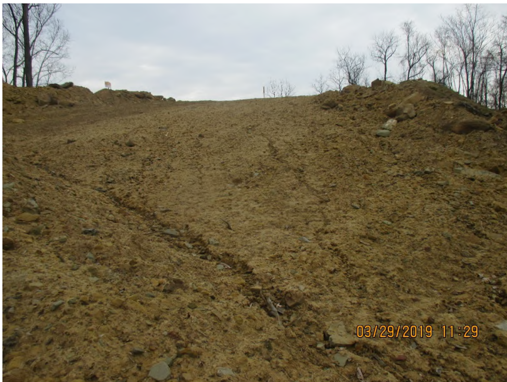
Erosion on slope near station #5148+00 leading to waterbar outlet over slope.
