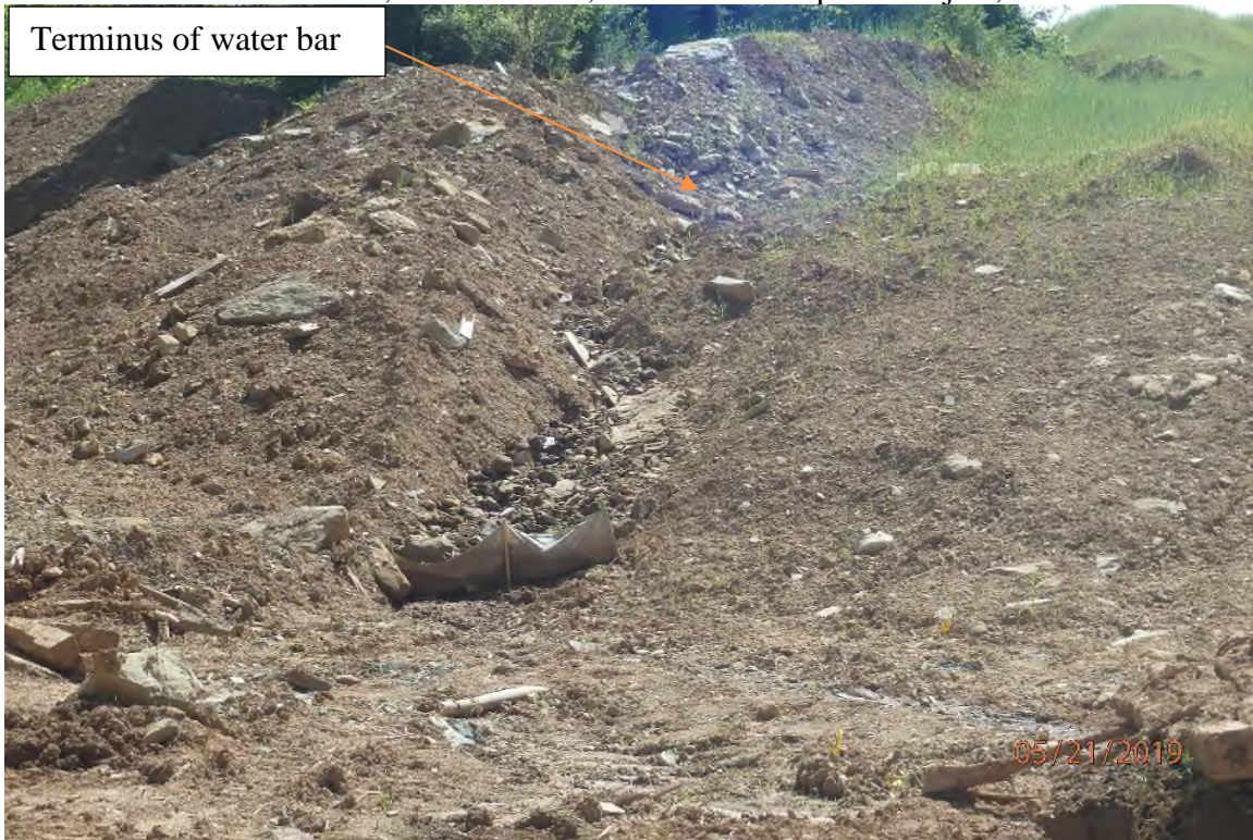
Improperly installed water bar in the Bluestone Creek watershed. Water bar discharges over an unprotected fill slope instead of off project as designed.
