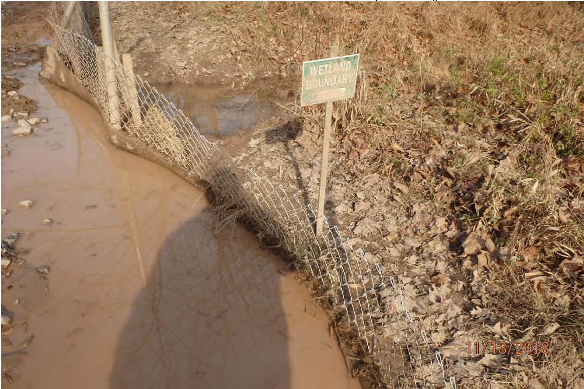
Unmaintained perimeter control and associated offsite sediment deposits on ARDO009.1.
