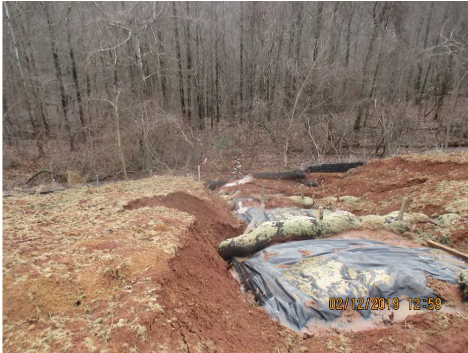
Facing downslope at station 5388+00 at perimeter controls from top of slope
