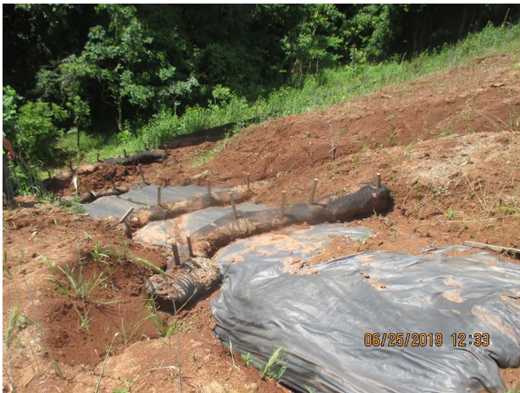
Waterbar outlet controls on slope south of ARWI 024 near station 5396+00. Perimeter controls overwhelmed with sediment. Erosion occurring under and next to Geotech fabric.
