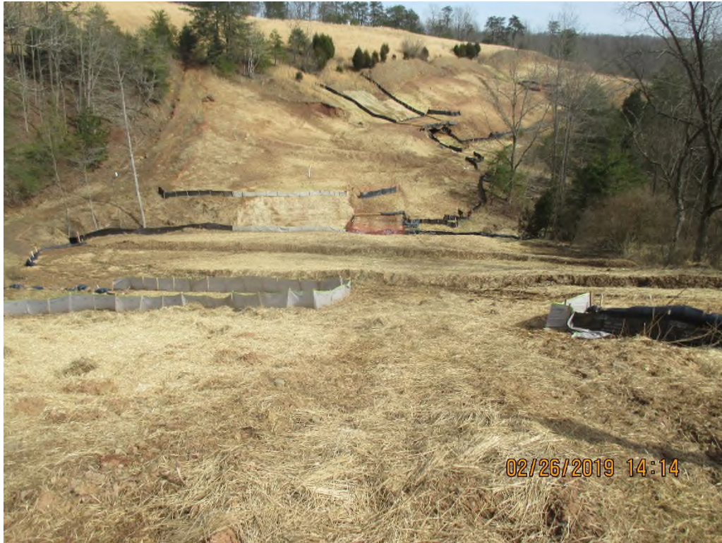
Facing NE toward multiple stream crossings including SJAG-352, 359, and 351 near station #6732+60
