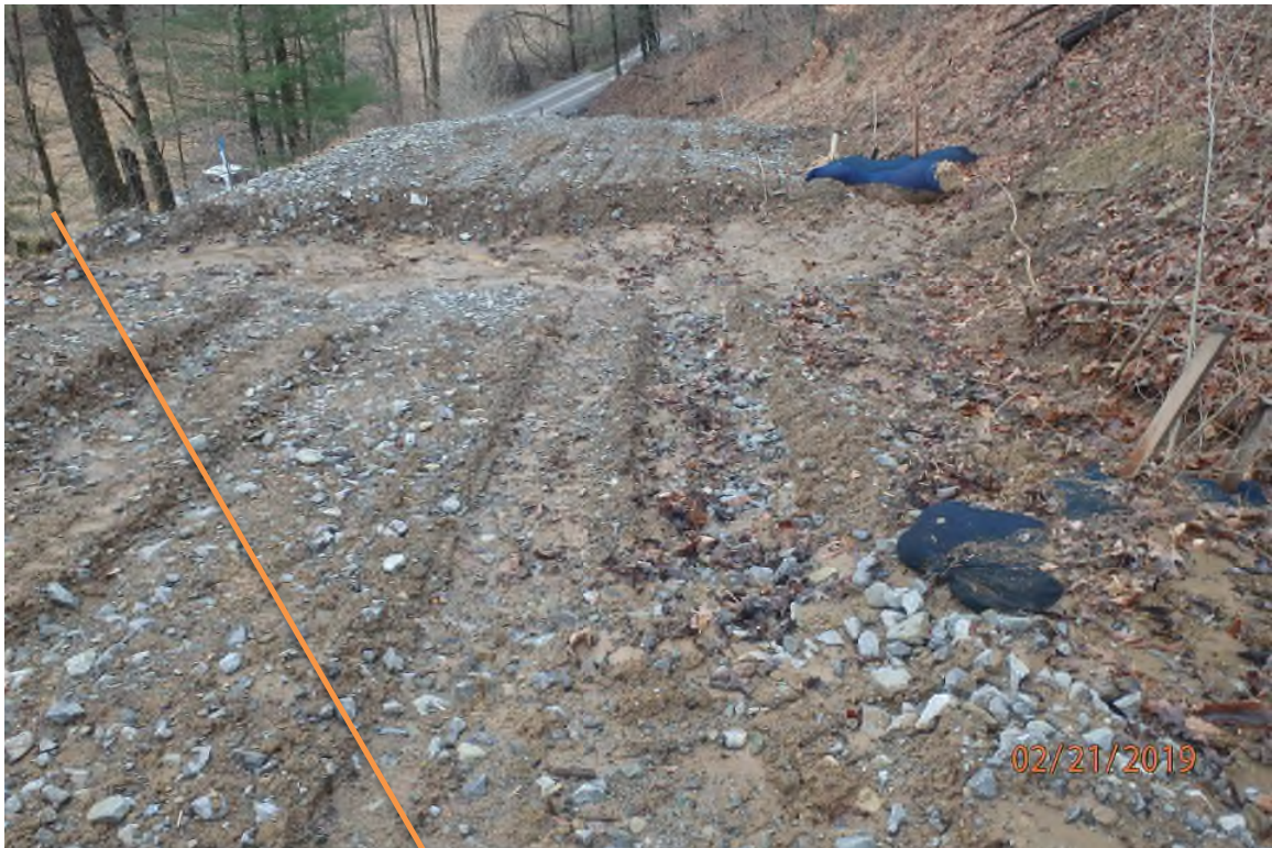
ARDO002.8 - lack of culverts to carry stormwater beneath the road surface.
