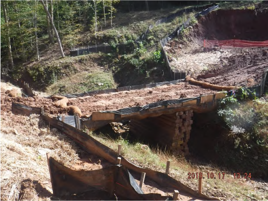
The crossing at Station 6705+00.
