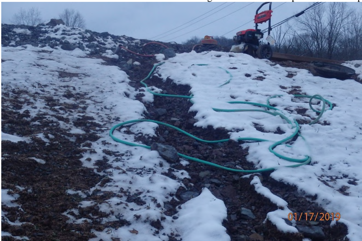
Erosion gullies in the fill slope as a result of concentrated flow originating from the truck wash.
