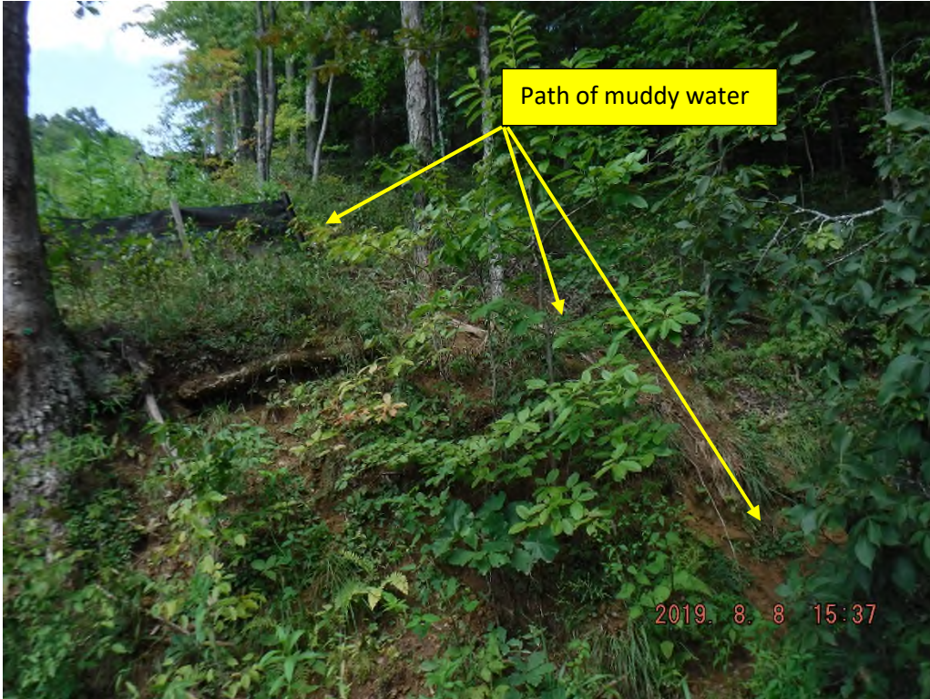
Path of sediment laden water detoured around silt fence resulting in sediment deposits.
