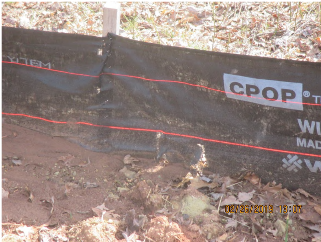
Silt fence at station #6766+60 with holes.
