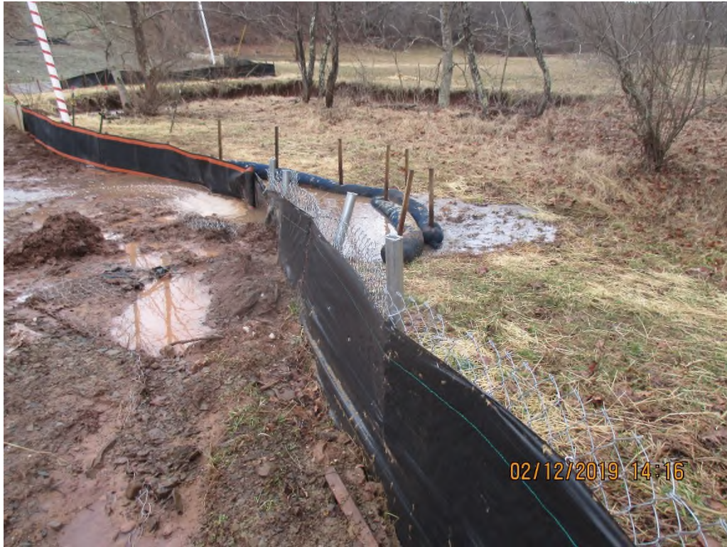
Stutler Road Crossing at station 5453+84 facing south at stream SROC-002
