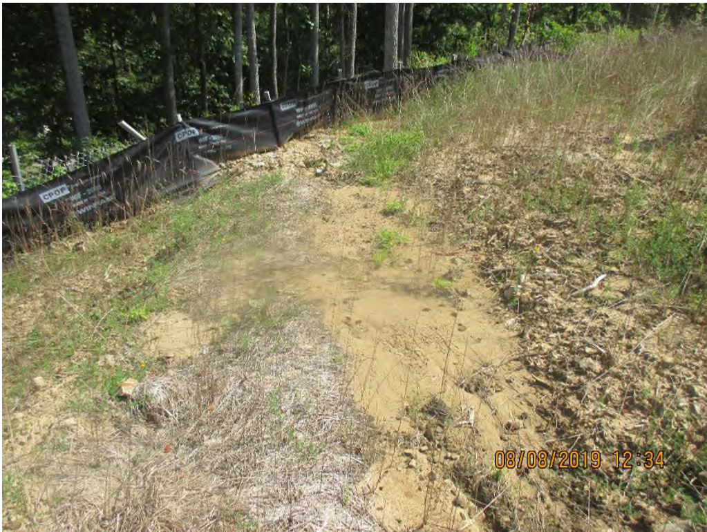
Slipped material accumulating in waterbar at edge of LOD with no outlet control at waterbar terminus near station No. 8772+72.
