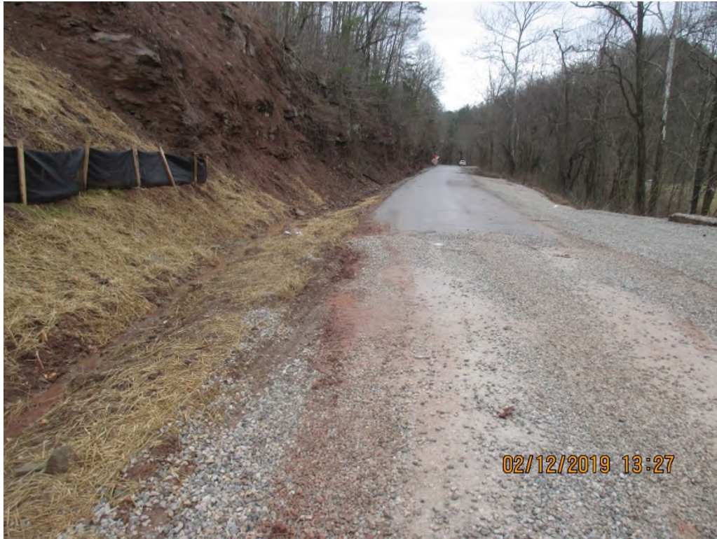
Munchausen Road crossing at station #5407+07 facing East
