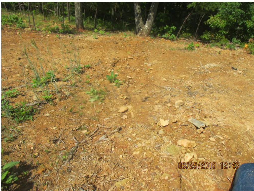
Erosion occurring below where waterbar was eroded. Sediment being deposited past LOD at station No. 5396+00.
