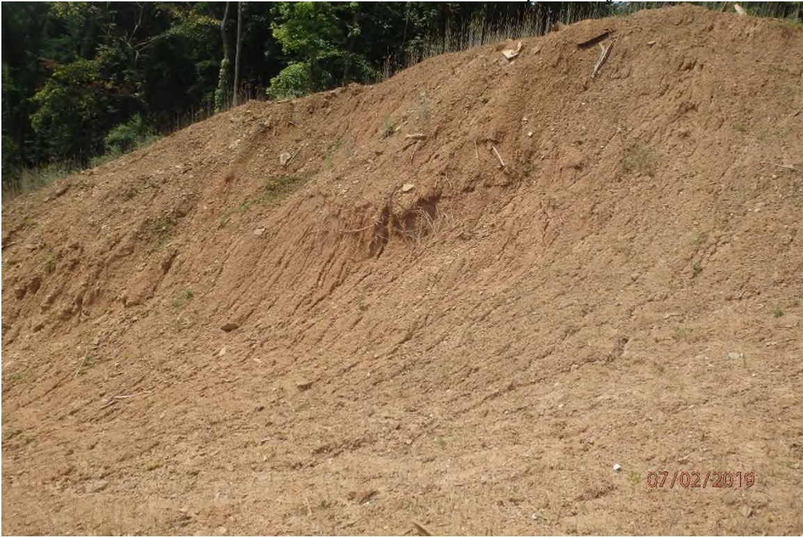
Area in the Trap Run watershed where the applied seed has failed to germinate, and the area was not reseeded.
