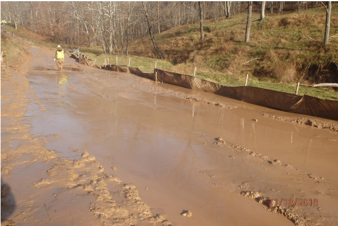
Condition of ARDO008.5 adjacent to the receiving stream.
