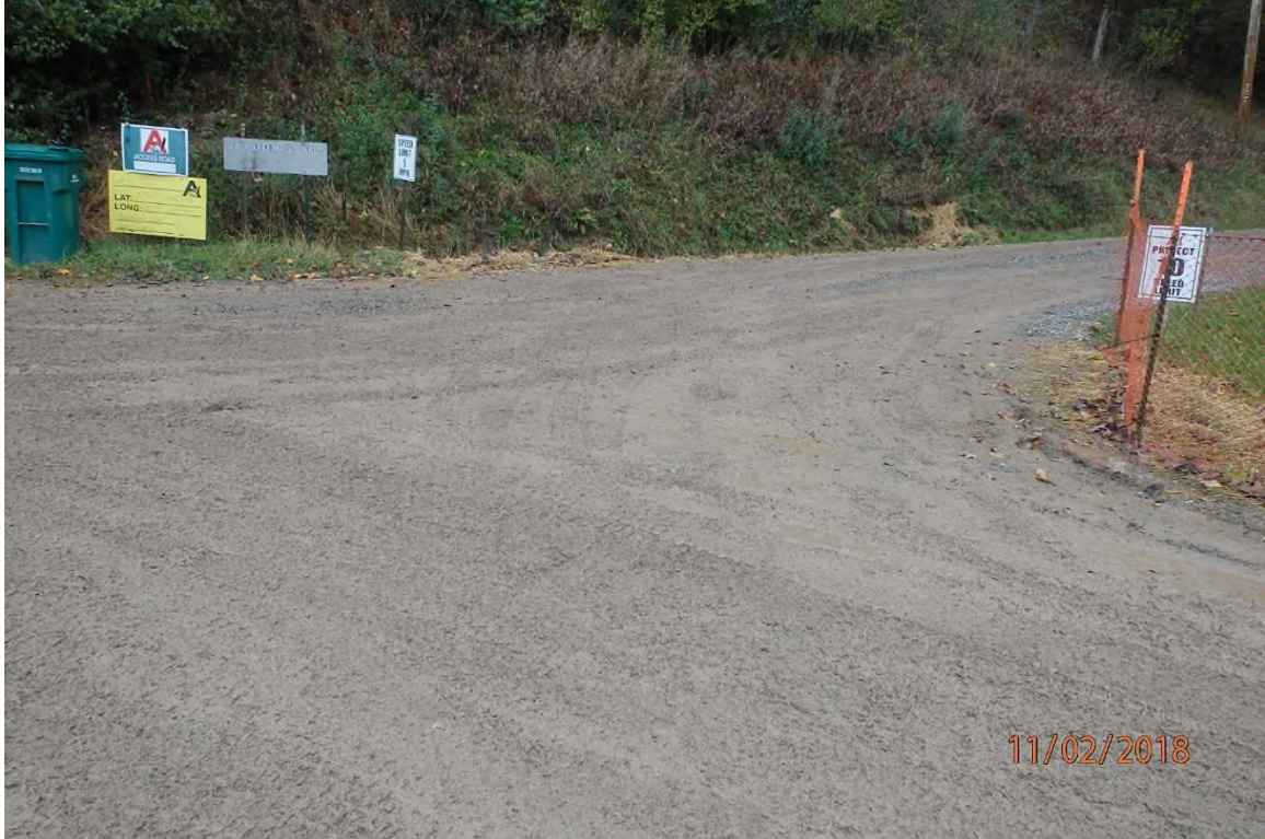
AR – 18 (ARDO002.7) showing an unstable construction entrance.
