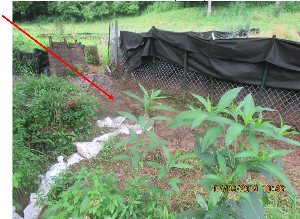
Last silt fence above 18-mile creek. Arrow depicts where sediment laden water was flowing into sandbags.
