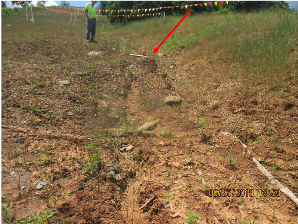
Middle Fork Road Crossing at station No. 5643+50 above stream SRUA 005. Waterbars eroded out where they were tied into topsoil pile.
