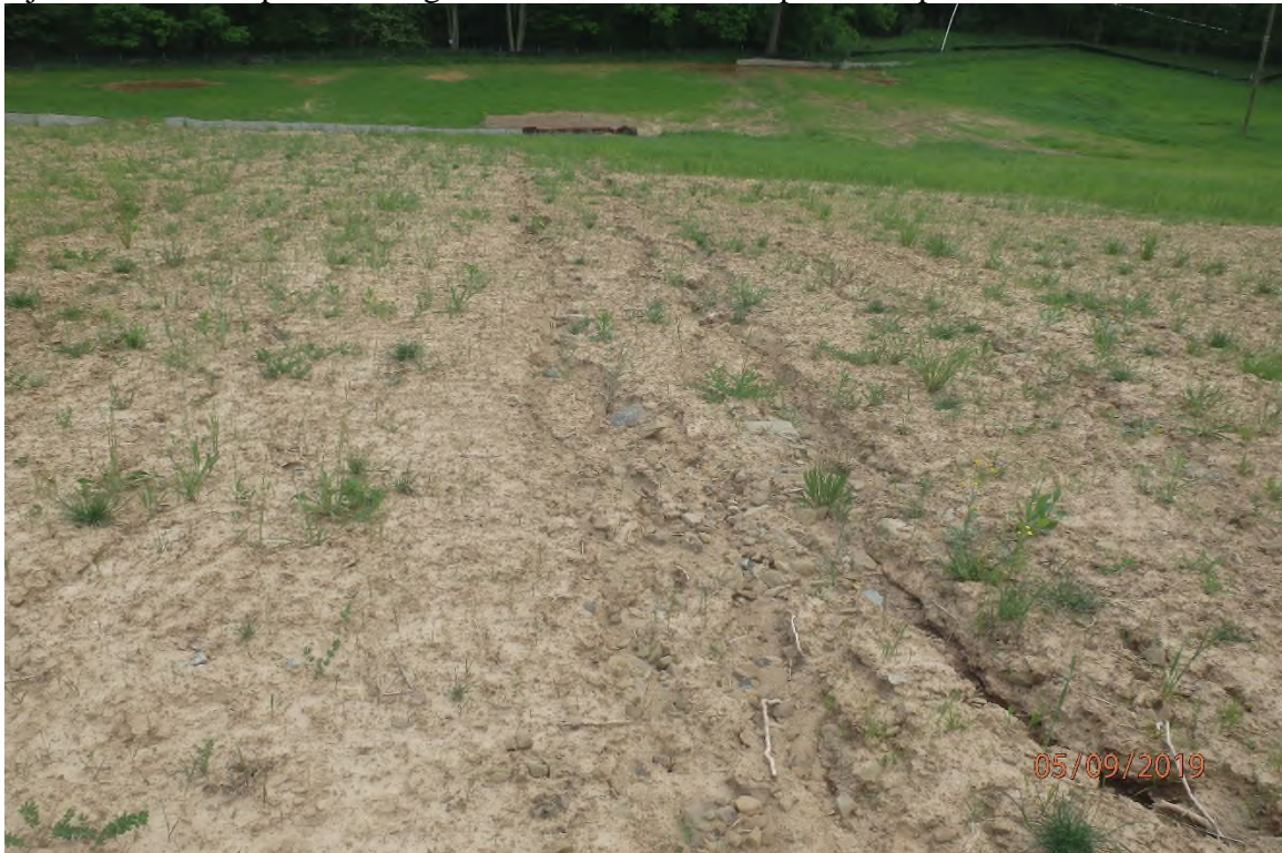
Slope adjacent to the fill pad showing the lack of installed slope interceptors. Fill slope erosion as a result of concentrated flow being directed over an unprotected fill slope. Area in need of reseeding.
