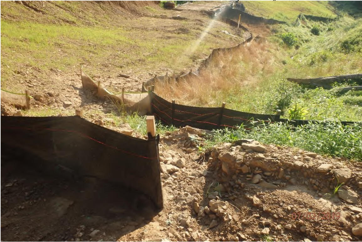
Fill slope erosion downslope of the previously pictured unmaintained water bar.
