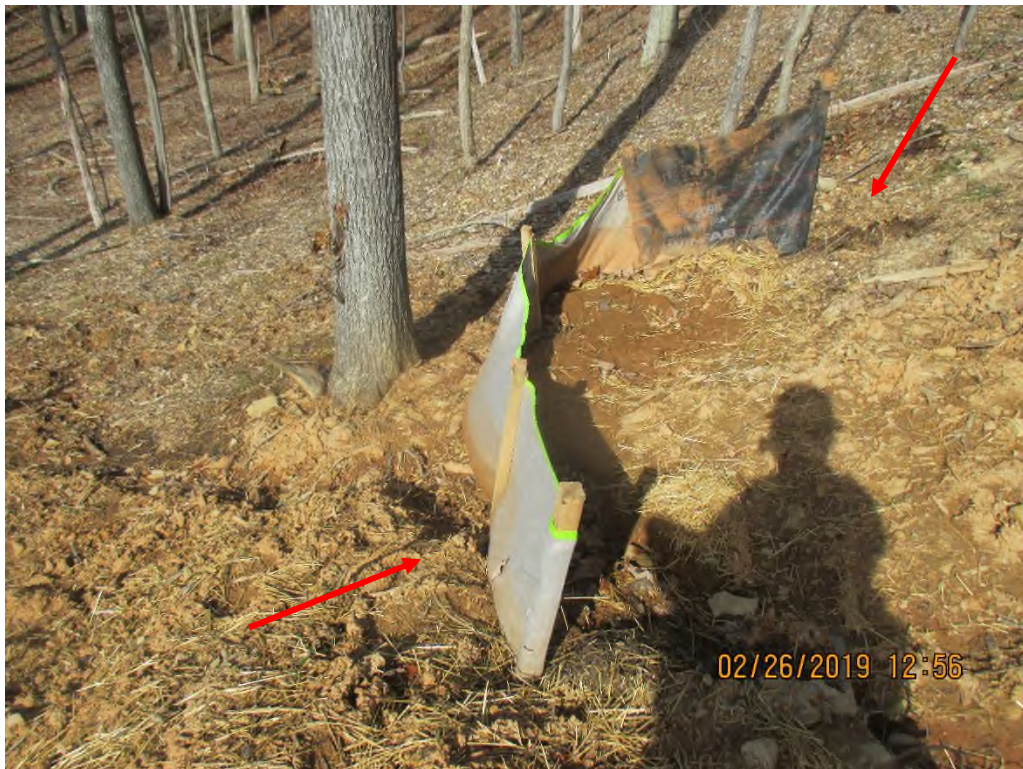
Waterbar outlet above SJAD stream complex at station #6770+75. Silt fence was undermined, and erosion was occurring on downslope side of the control and on the side of the control due to run-off flowing around it.
