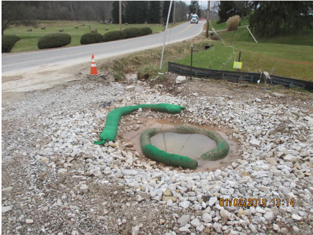
BMPs in place at rock lined ditch terminus.
