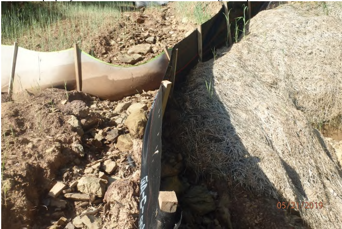
Fill slope erosion and recently repaired perimeter control downslope of the above pictured deficiency.
