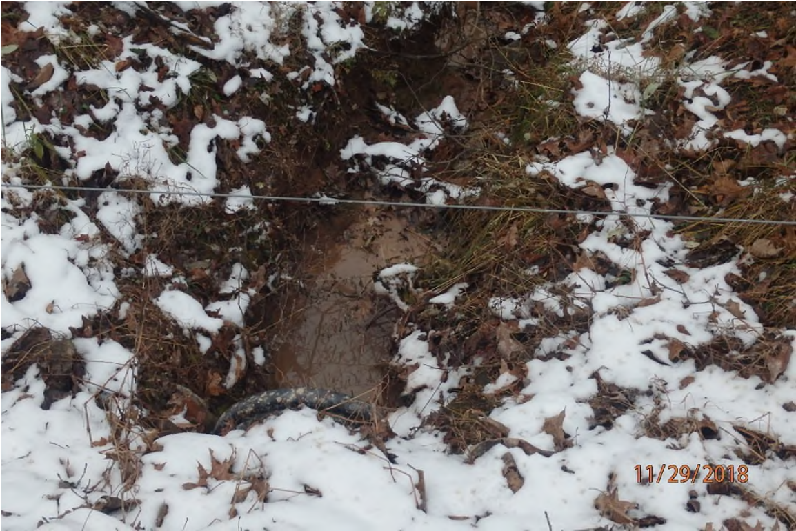
Culvert outlet showing offsite sediment deposits downslope of the previously pictured area on ARDO009.3.
