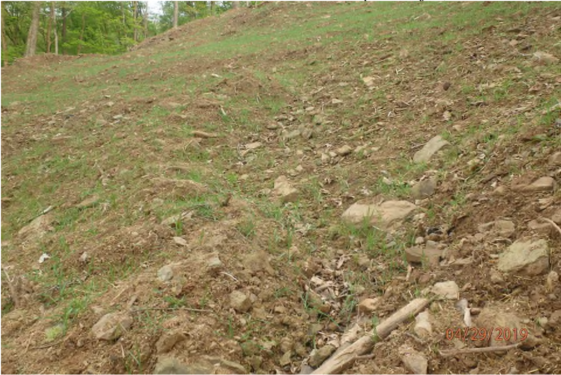
Water bar with varying angles adjacent to 2225+00. A portion of the water bar is installed at an angle greater than 12%.
