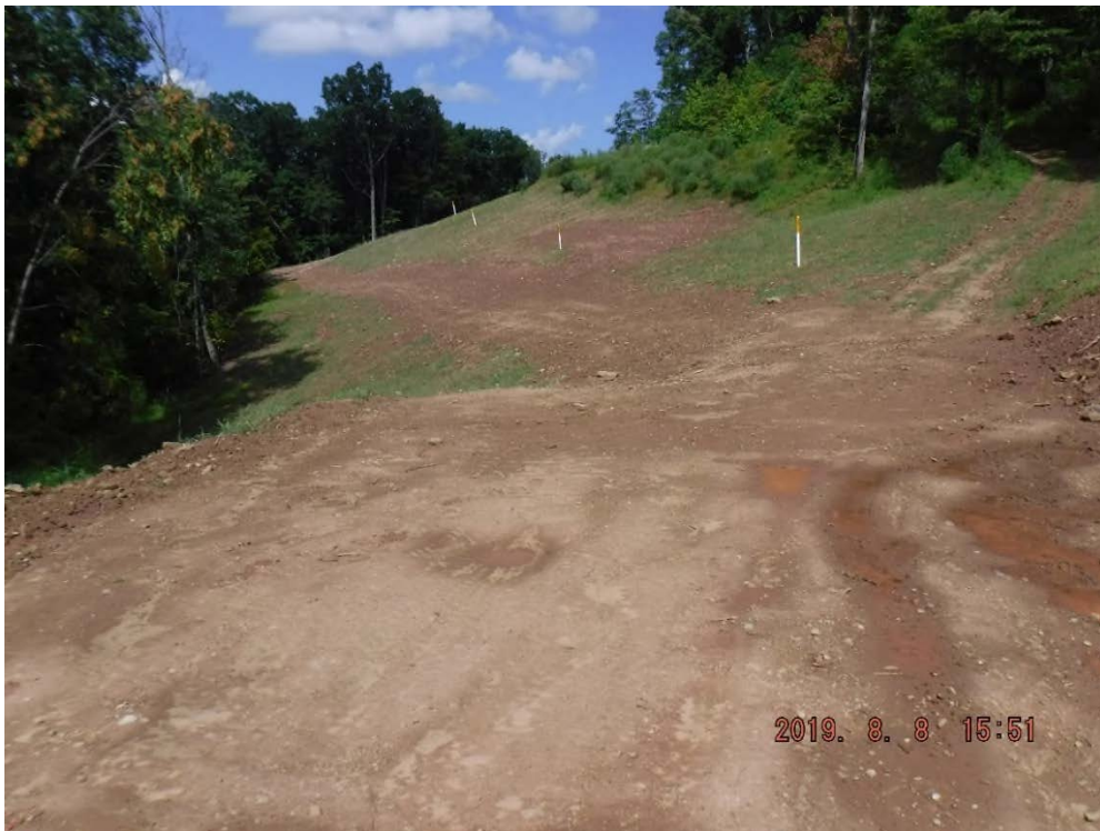
Seed failed to germinate within 30 days.
