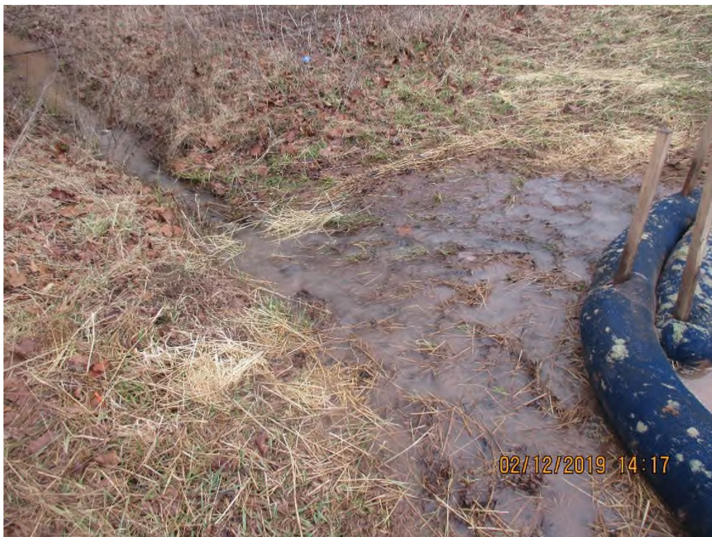
SLW flowing under controls at station #5453+84
