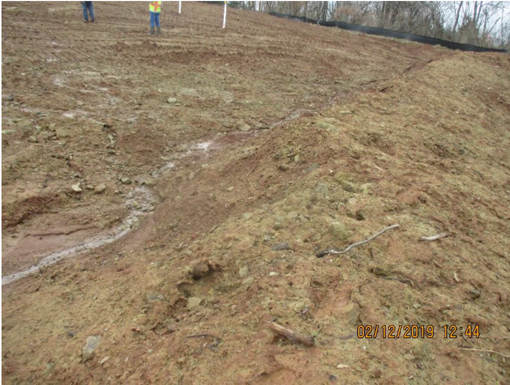
Waterbar near station 5376+00 facing upslope
