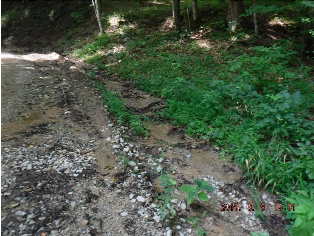
East side ditch filled with sediment from ROW runoff.
