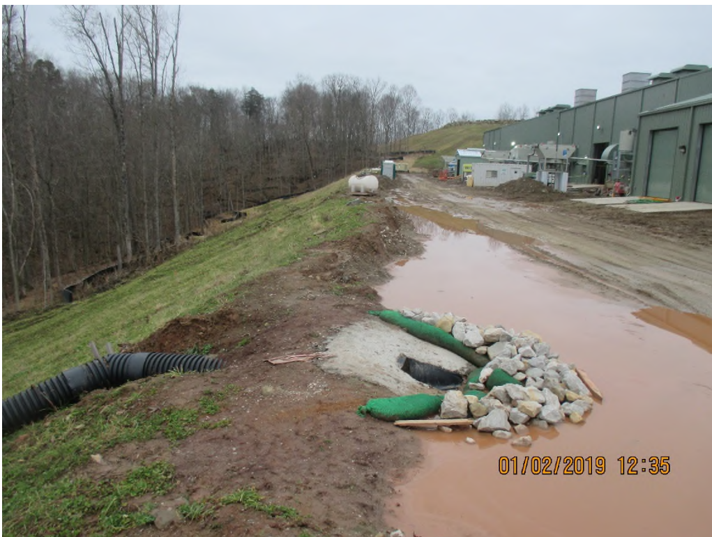
Pipe slope drain on north side of project.
