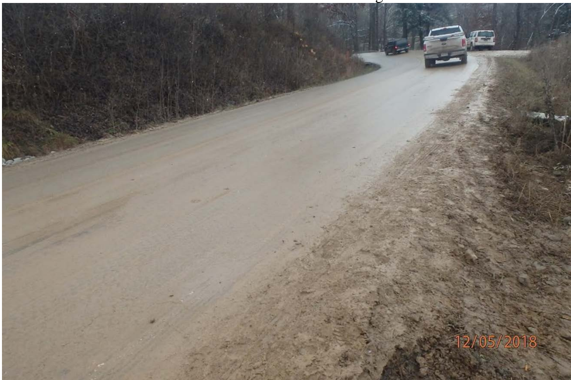
WV 18 showing track out and slick film of mud on the public roadway.
