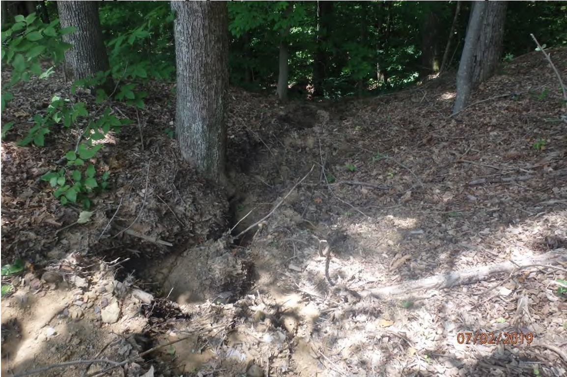
Offsite CNA deposits in UNT Left Fork of Arnolds Creek (SDOG057) (39° 13.355' X 80° 46.851') as a result of the previously pictured improperly installed water bars and unmaintained perimeter controls.
