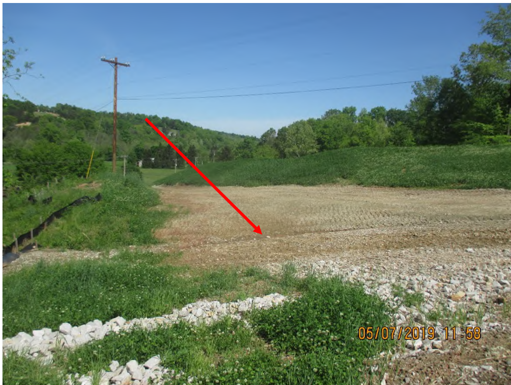
Facing North towards old reggraded construction entrance on West side of project. Arrow depicts erosion occurring on slope.
