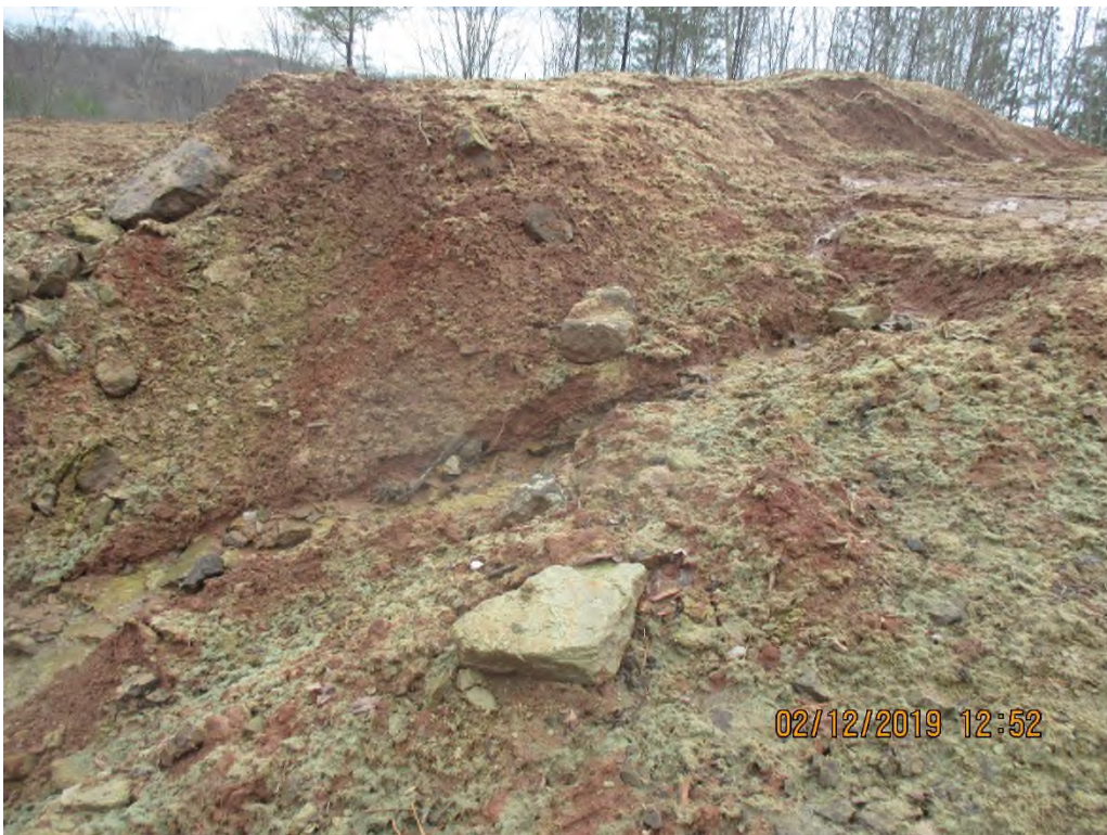
Erosion occurring on slope leading to perimeter control near station 5388+00
