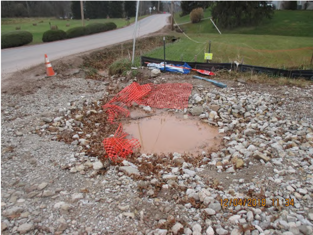
Sediment trap/sump at entrance.
