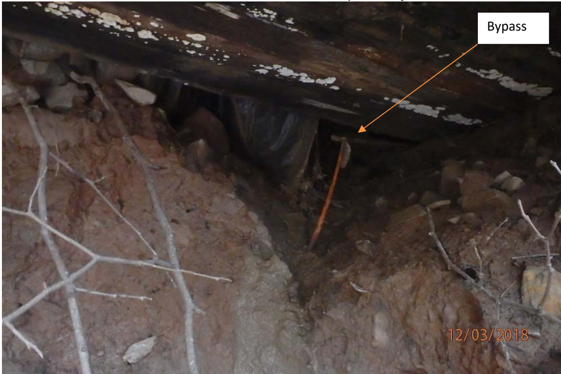
Equipment bridge BMP on ARDO007.6 in need of maintenance showing point of sediment laden water bypass.
