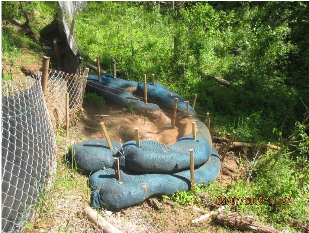
Perimeter outlet controls below armored channel at the base of the South slope.
