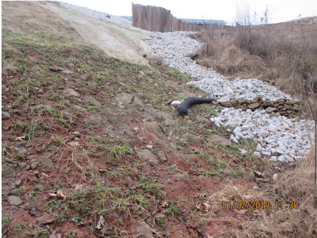
Armored channel on south slope facing station access road.
