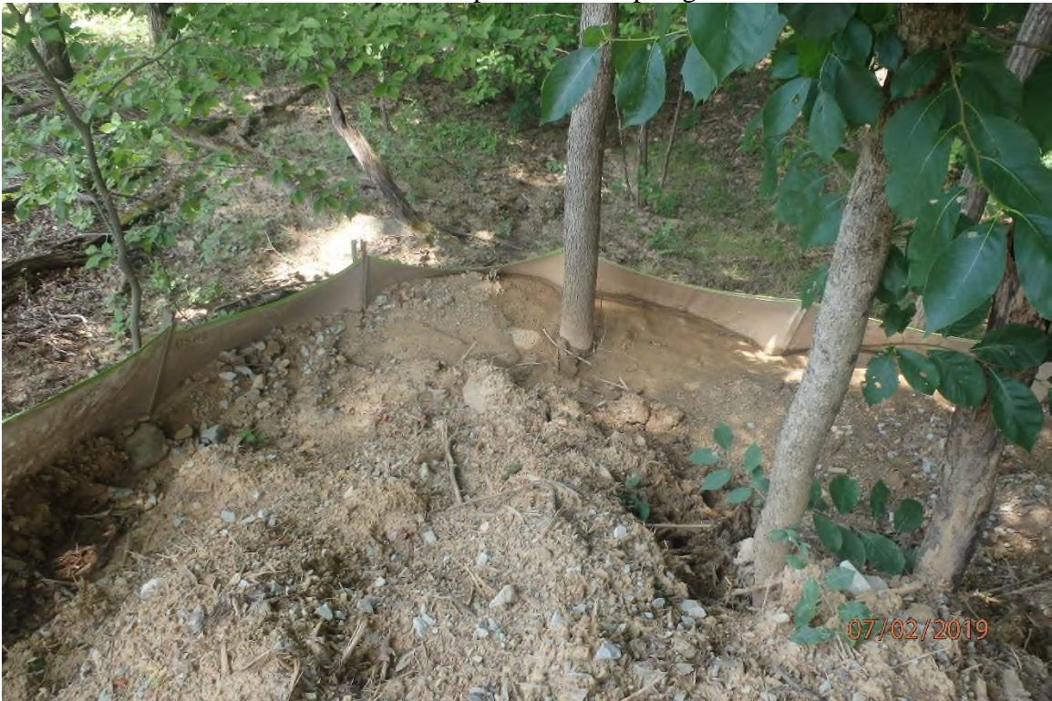
Area adjacent to the above pictured water bar showing offsite sediment deposits associated with a previous mud flow that Columbia Gas attempted to contain with silt fence. The silt fence is in need of maintenance.
