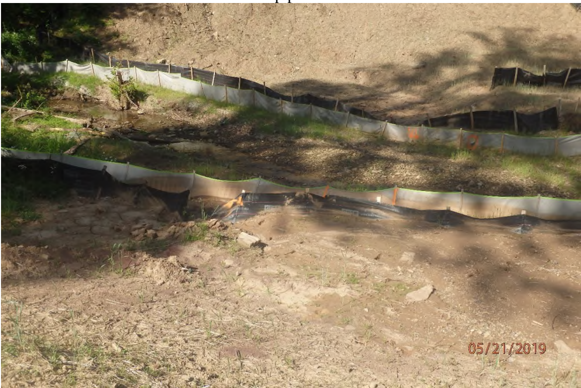
Unmaintained BMP in the Georgescamp Run watershed.
