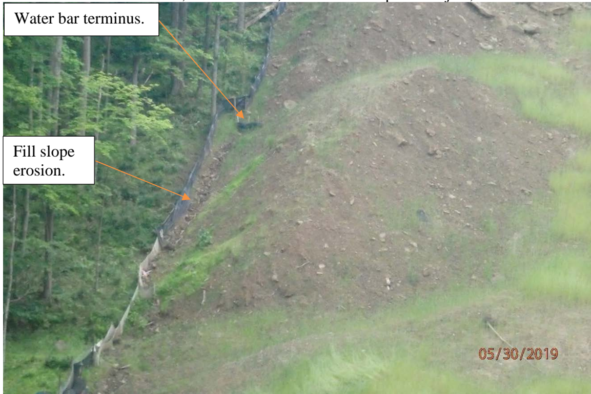
Water bar that terminates inside of the installed perimeter controls in the Wolfepen Run watershed.
