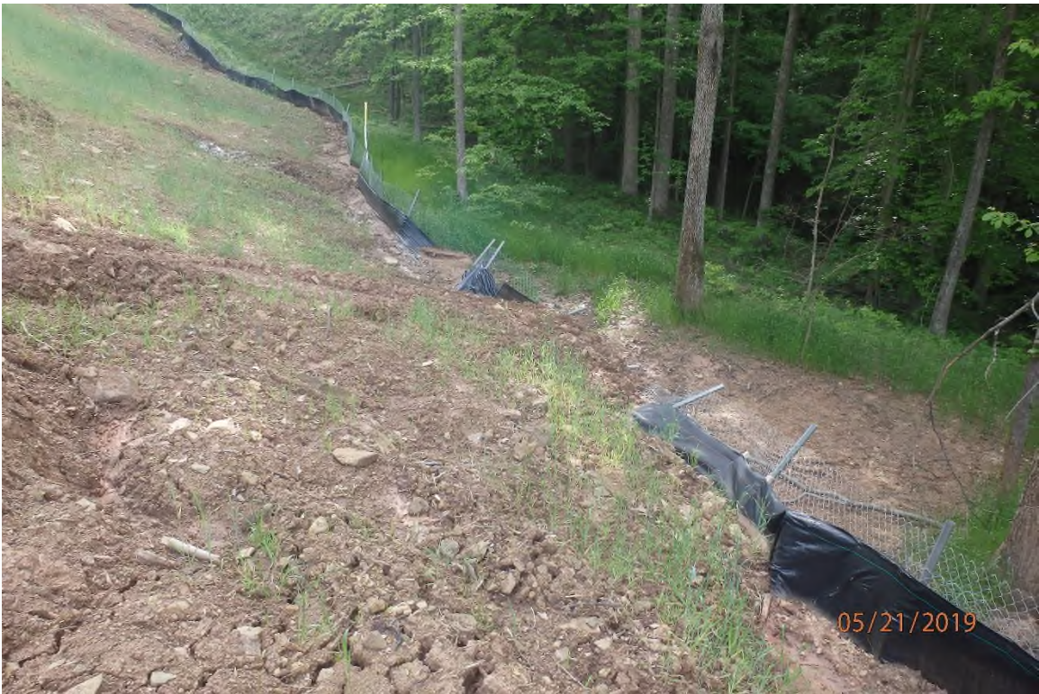
Unmaintained BMP in the Sugar Run watershed.
