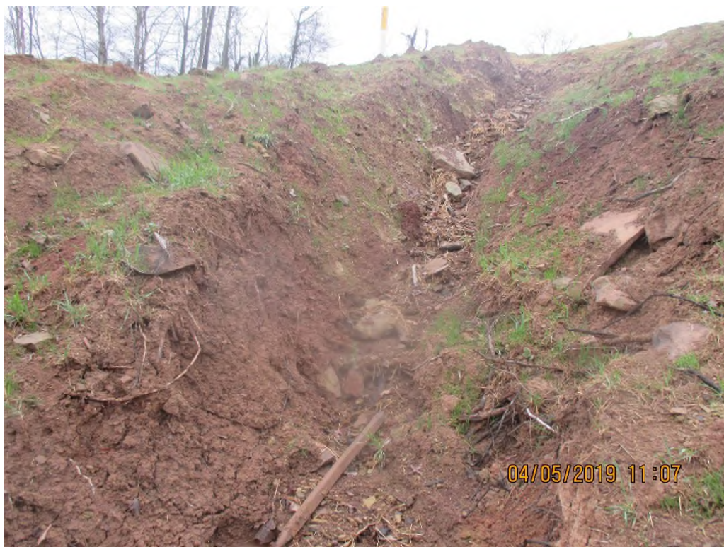
Waterbar terminating onto fill slope above stream SJAG 316. Erosion present in waterbar.
