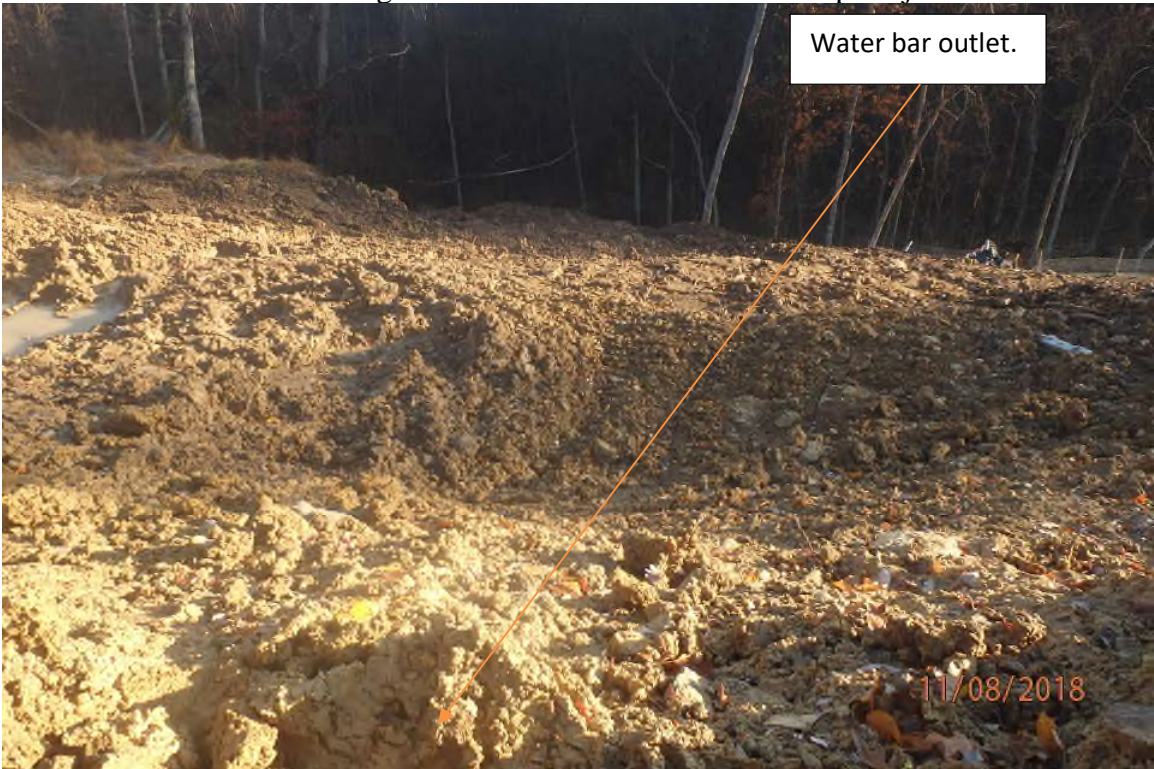
Water bar outlet that discharges concentrated flow over a fill slope adjacent to 2822+00.
