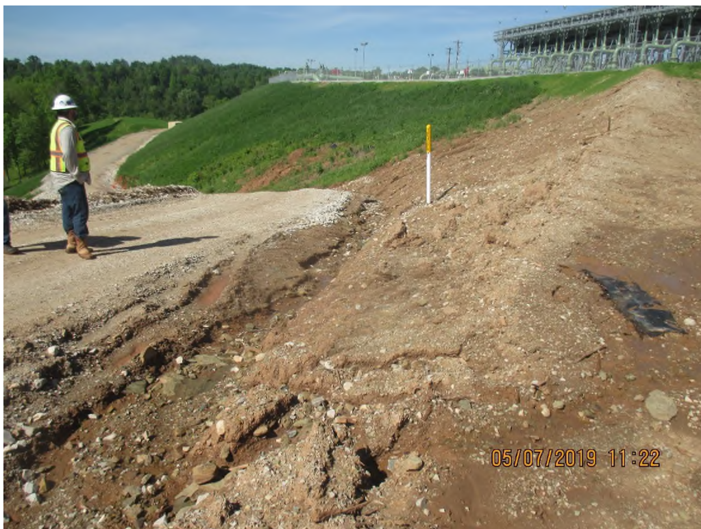
Erosion occurring below swale outlet on South slope.
