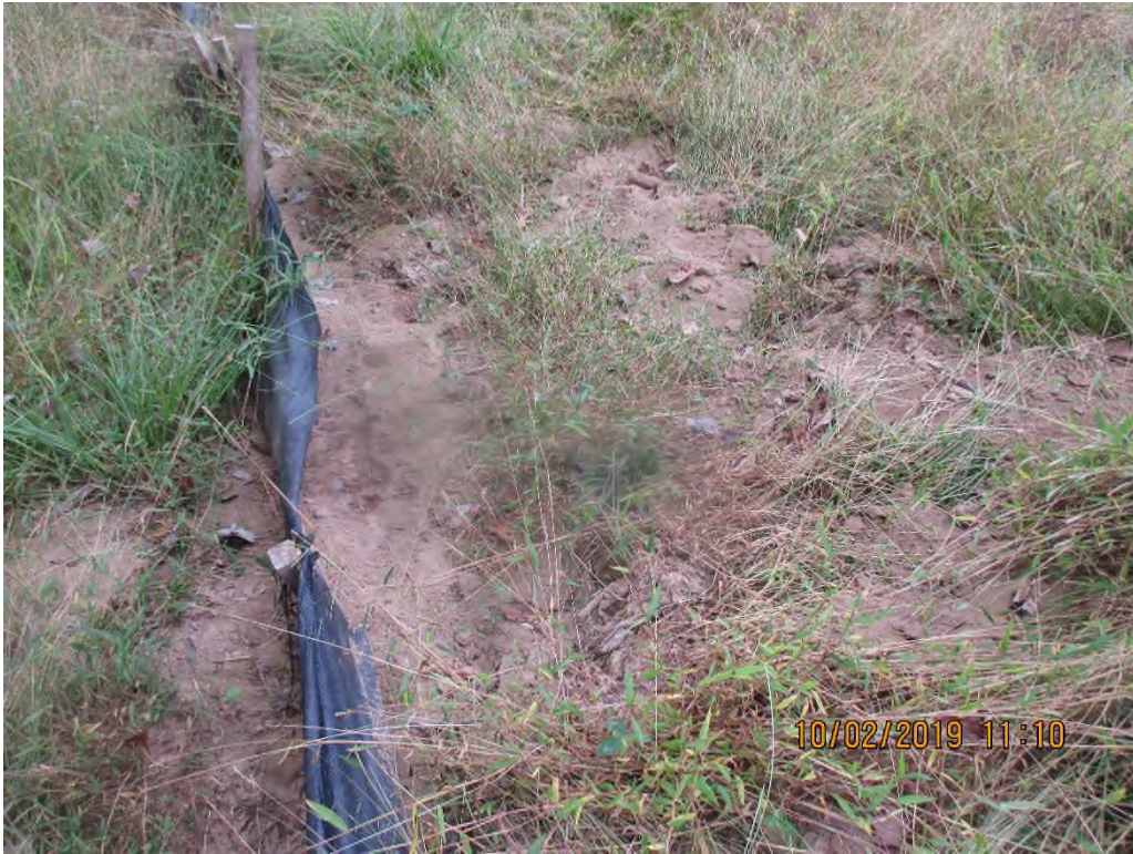
Sediment being deposited behind and past controls near station No. 3368+00.
