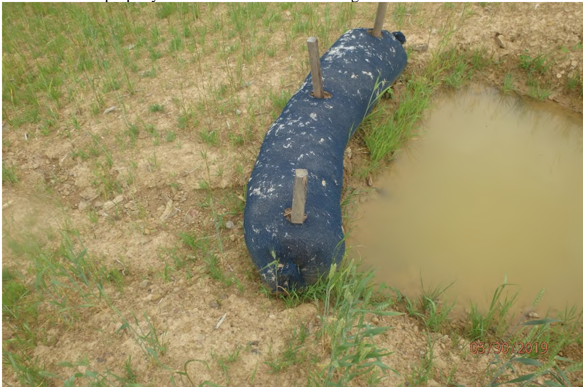
Above pictured water bars showing fill slope erosion downslope of the outlet.
