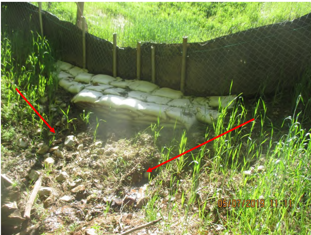
Controls at base of NE slope facing upslope. Controls in need of maintenance due to undermining, causing erosion below controls. Arrow depicts erosion below controls.
