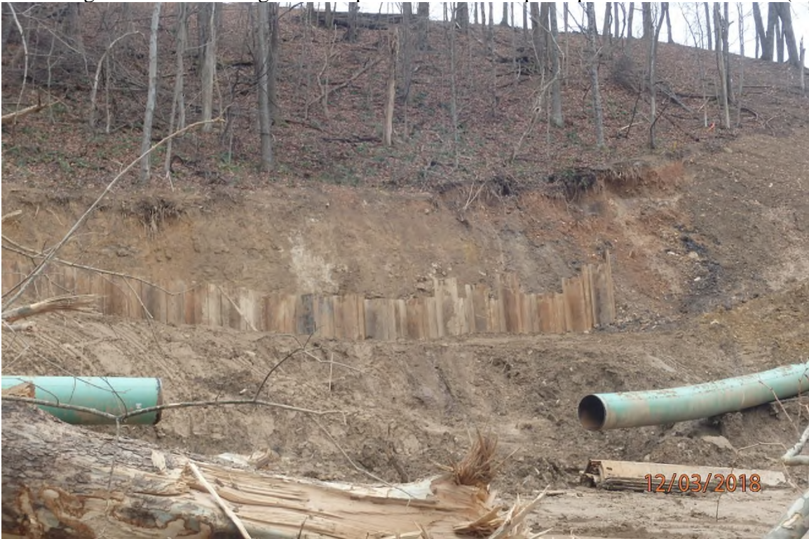
Sheet piling installed upslope of the installed pipe to protect pipe integrity on the slip associated with spill report number 09-83236 (A).
