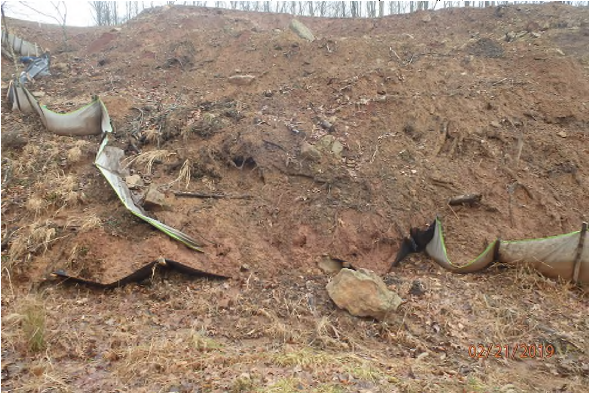
Perimeter control in need of maintenance.
