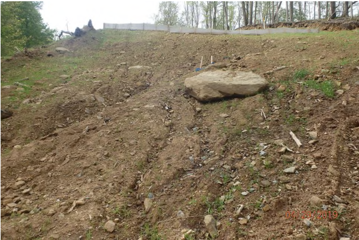
Disturbed areas of the project that are in need of reseeding.
