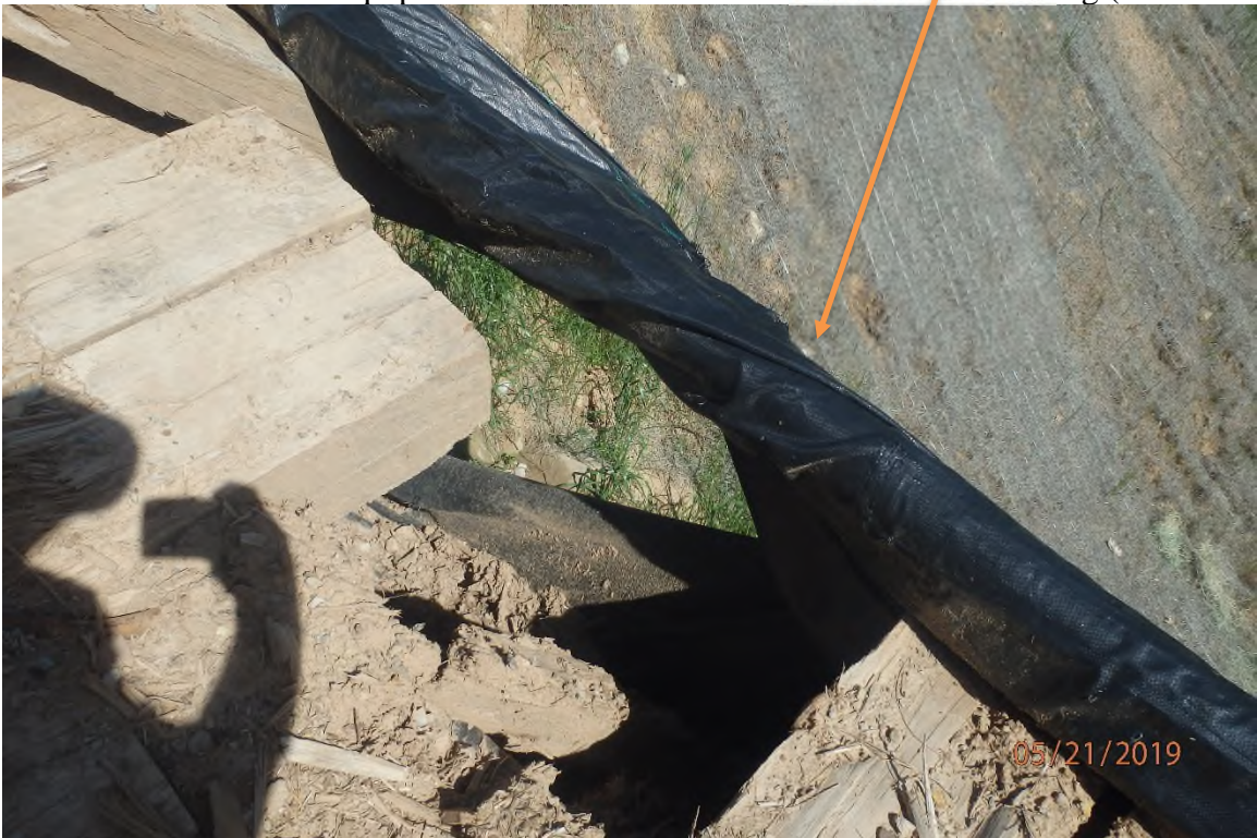
Unmaintained timber mat equipment BMP at the UNT Bluestone Creek crossing (SDOG539).
