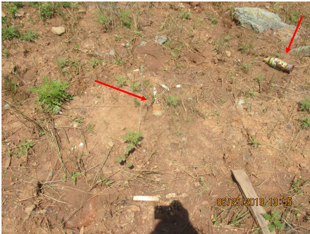
Solid waste present at station No. 5643+50.
