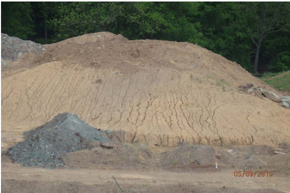
Soil stockpiles have been idle for greater than 21 days and have not been temporarily stabilized.
