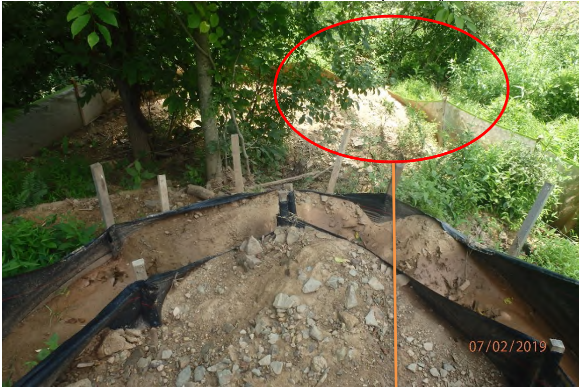
Perimeter controls downslope of the previously pictured deficiency in the Trap Run watershed that has become inundated with sediment as a result of poorly installed water bars.
