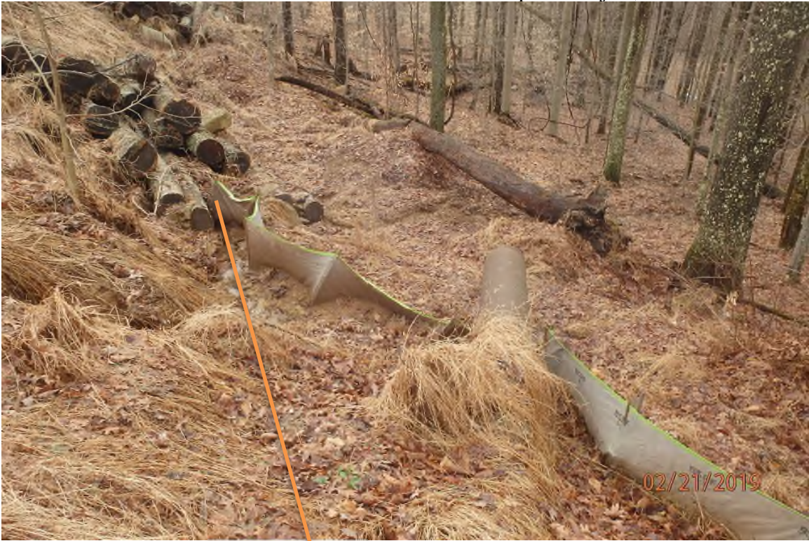
Improperly installed perimeter control adjacent to 2260+00 that allows sediment laden water to bypass the device.
