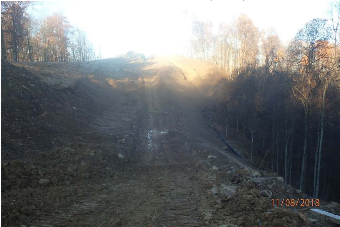
Improperly installed water bars adjacent to 2822+00.
