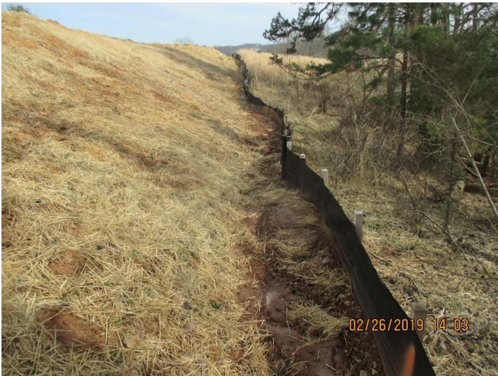
Facing downslope along perimeter control where sediment is backing up against controls due to erosion occurring on slope near station #6620+00 (per SWPPP).
