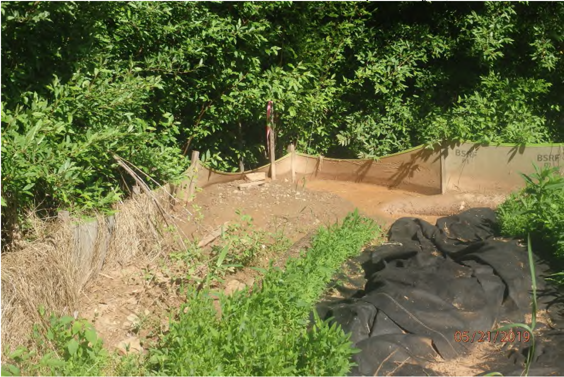
Discarded dewatering bag in the Bluestone Creek watershed.
