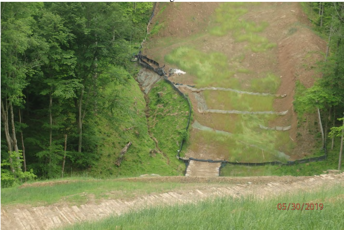
Improperly installed water bars in the Wolfepen Run watershed.
