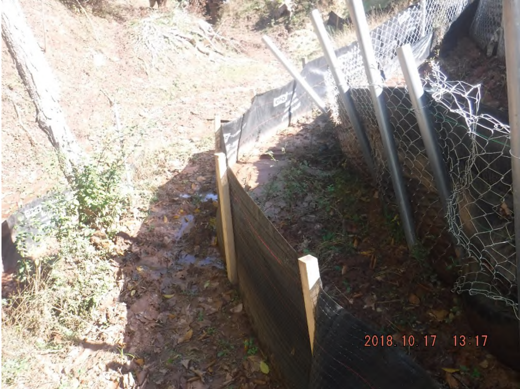
Build-up of sediment collected behind silt fence.
