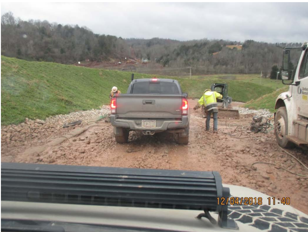
Pressure washing station upslope of entrance and Route 21.
