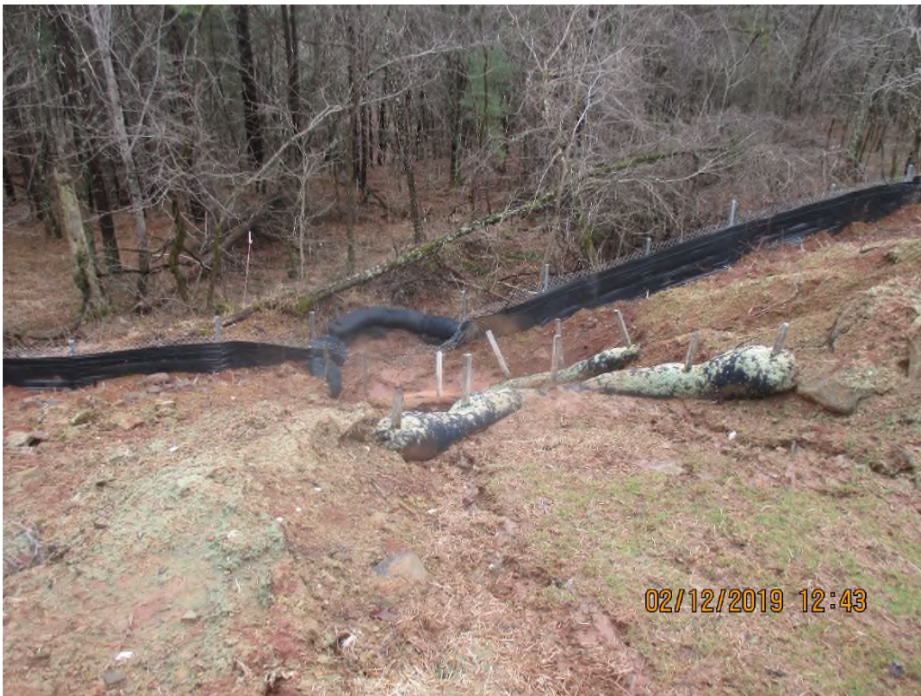
Waterbar outlet near station 5376+00
