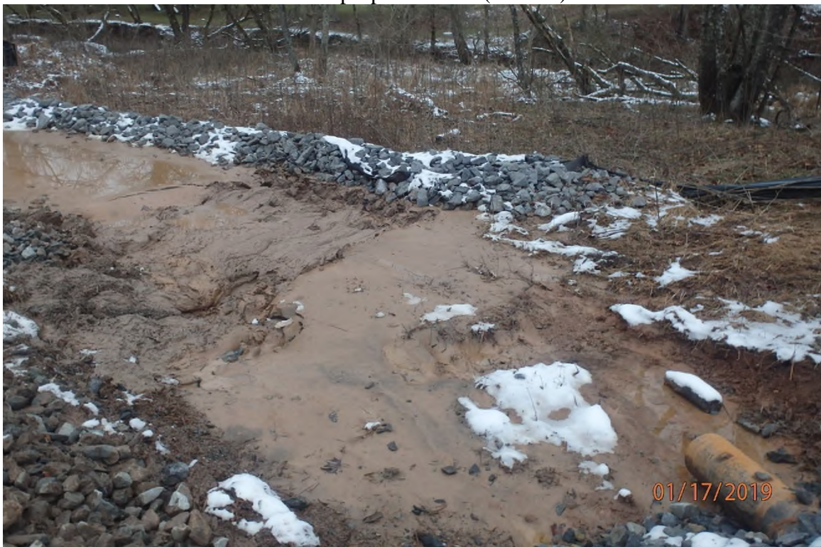
Rock filtration device that is in place. The proposed sediment basin in the approved SWPPP is not in place as designed.
