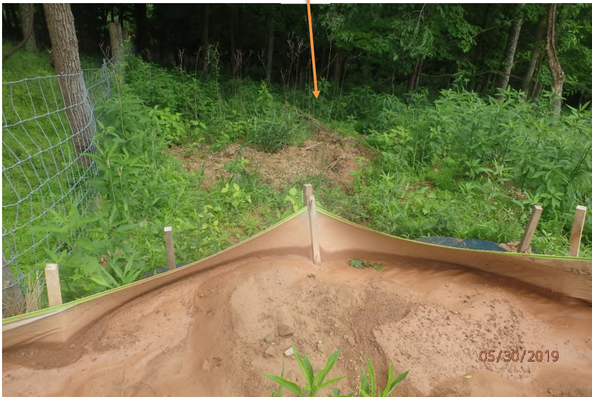
Water bar outlet in need of maintenance and the associated offsite sediment deposits in the UNT Wolfepen Run watershed.
