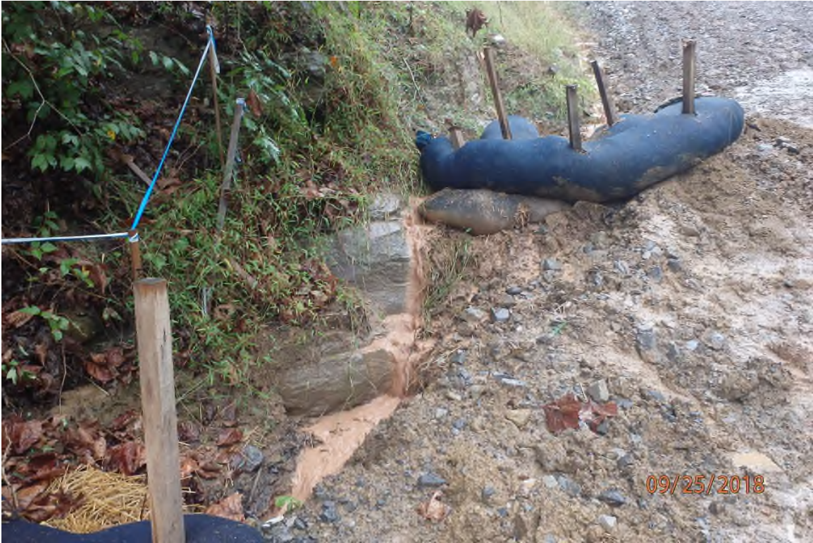
Ditch check along ARDO002.8 that is allowing a sediment laden water bypass.
