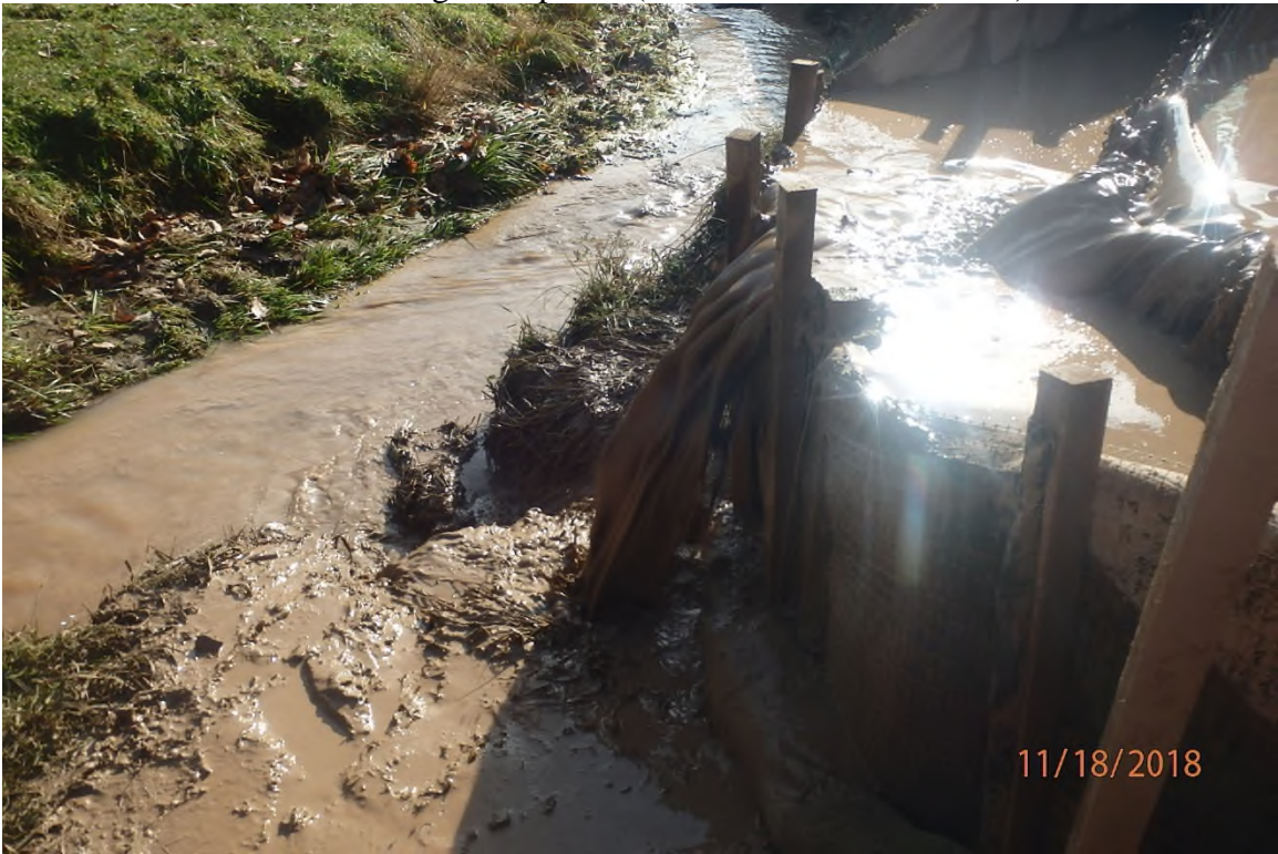
Second perimeter control that has been overwhelmed and is causing CNA deposits and distinctly visible plume in UNT Georgescamp Run (39°15.182' X 80° 44.033').
