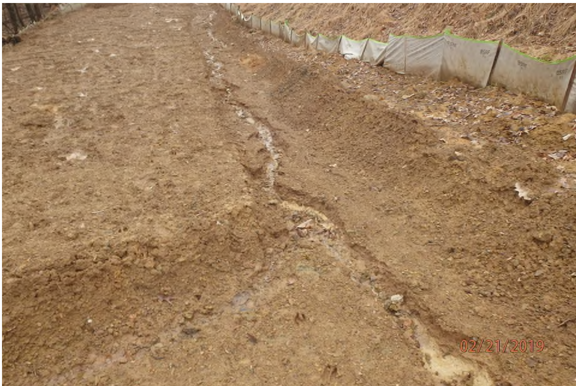
Project area adjacent to 2256+00 showing improperly installed water bars and the associated fill slope erosion.
