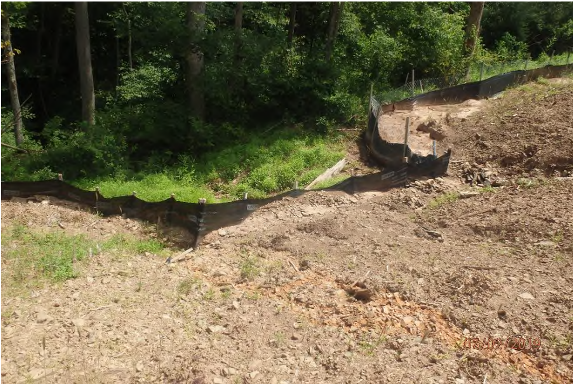
Perimeter controls adjacent to 3214+00 that are inundated with sediment and in need of maintenance as a result of the above pictured deficiency.
