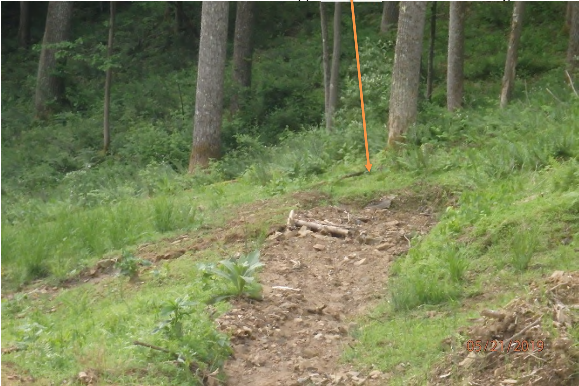
Water bar that lacks the outlet BMP indicated in the approved SWPPP in the UNT Sugar Run watershed.
