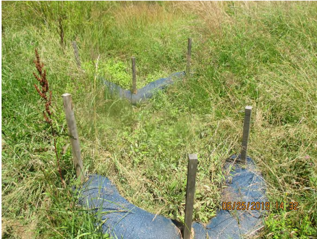
Controls in place on pond edge. Evidence observed that pond overtops banks during high rain events due to staining of grass below these controls. Pond culvert flows under these controls subsurface. Water was running through the culvert.
