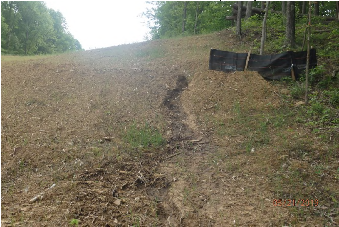
Unmaintained BMP in the Sugar Run watershed and the associated fill slope erosion.
