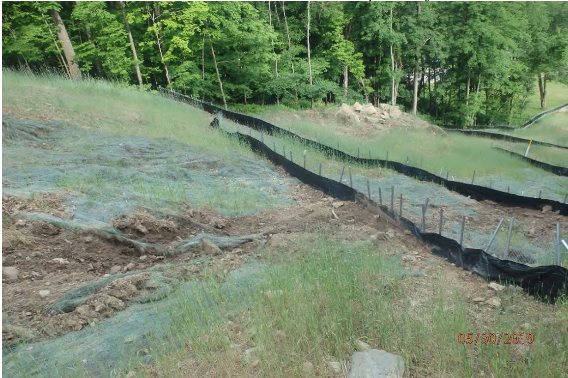
Fill slope erosion below an improperly installed water bar adjacent to 2592+50.
