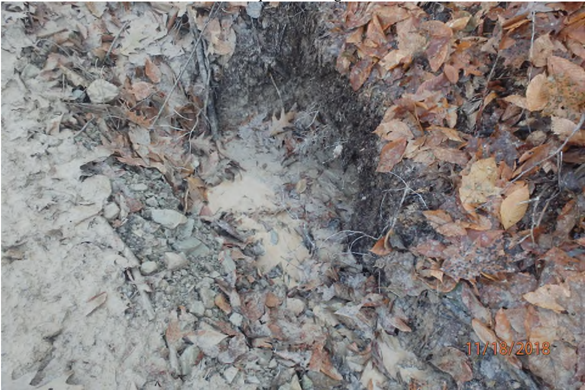
Culvert inlet on ARDO008.2 where the above pictured concentrated flow is directed.
