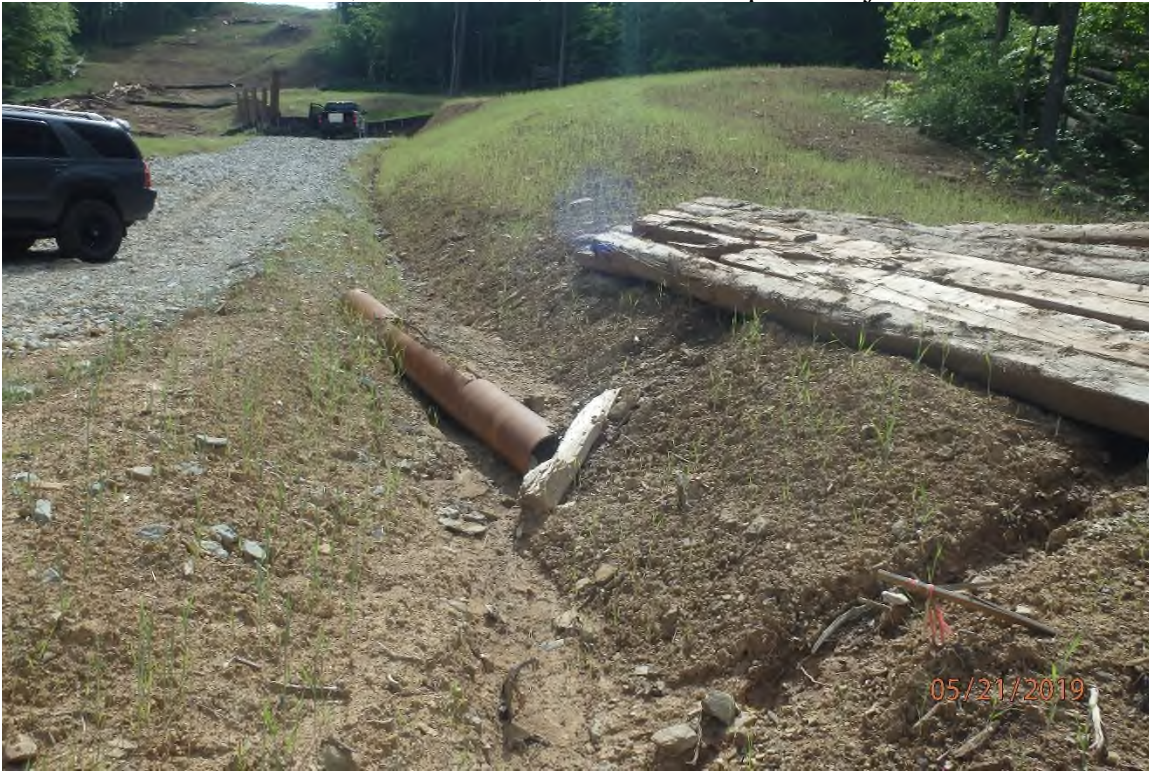
Area where two water bars are indicated in the approved SWPPP in the Taylor drain watershed that are not in place.
