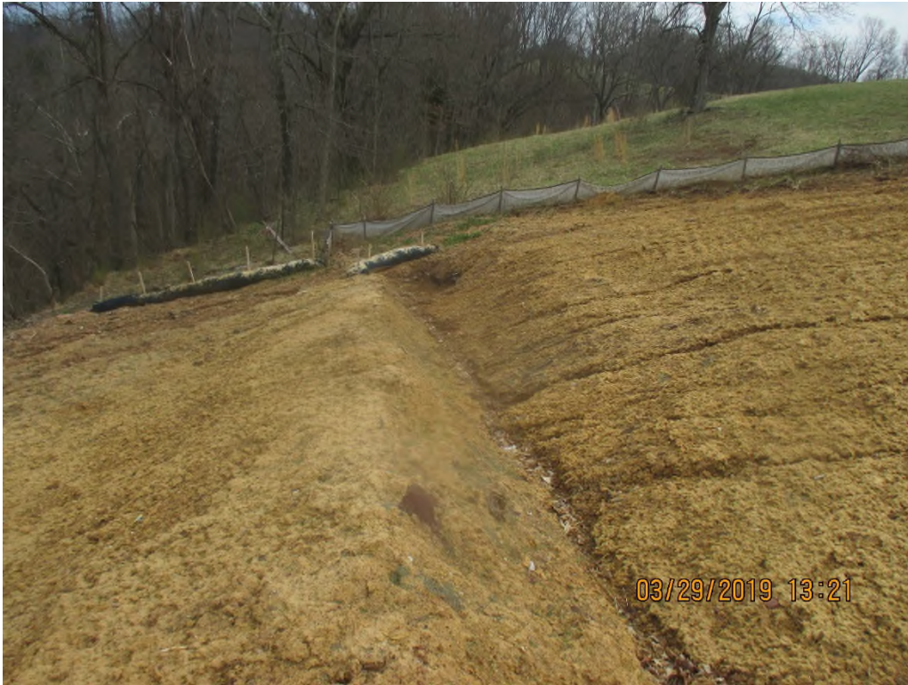
Waterbar near station #5180+43. Erosion occurring in the waterbar.
