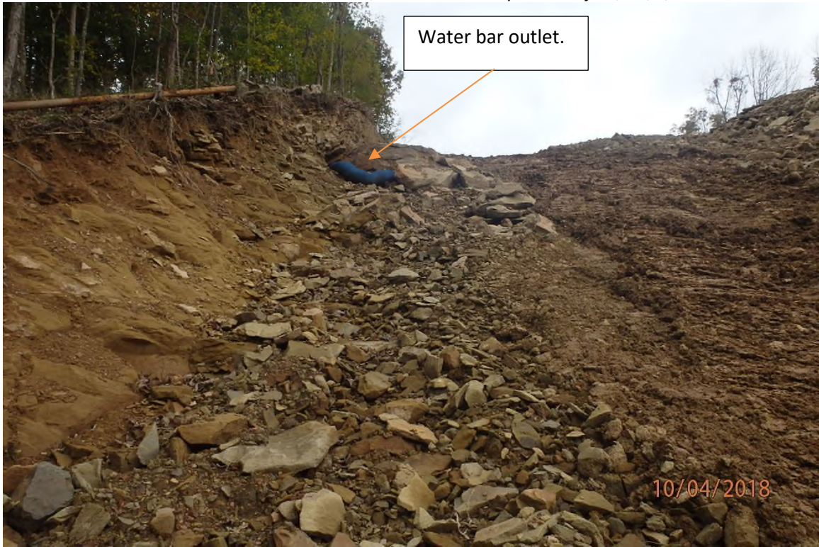
Fill slope erosion as the result of an improperly constructed water bar in the Riggins Run watershed.
