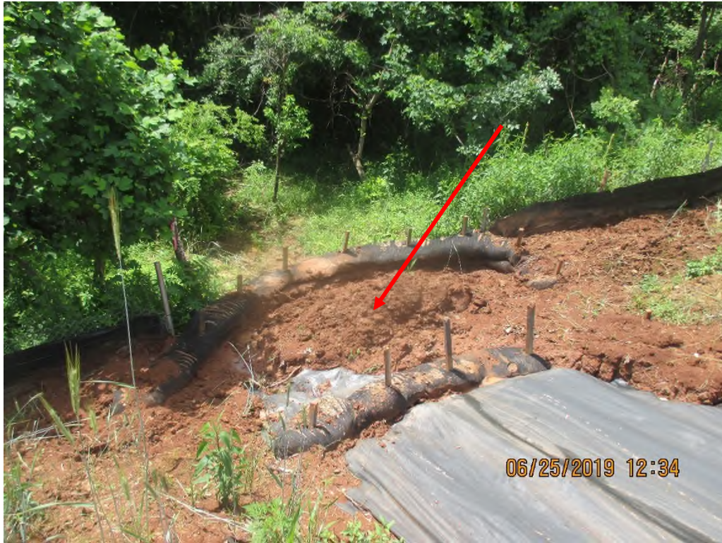
Waterbar outlet controls on slope south of ARWI 024 near station 5372+00. Perimeter controls overwhelmed with sediment. Erosion occurring under and next to Geotech fabric. Sediment removed from behind controls and placed in pile several feet behind controls. Deposits observed past the LOD.
