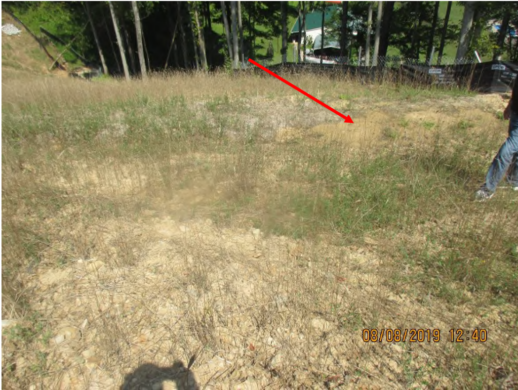
Downslope of slipped material. Sediment being transported into waterbar towards perimeter controls. Arrow depicts sediment accumulation in waterbar.
