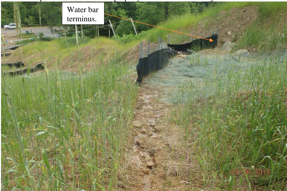
Improperly installed water bar adjacent to 2591+00.
