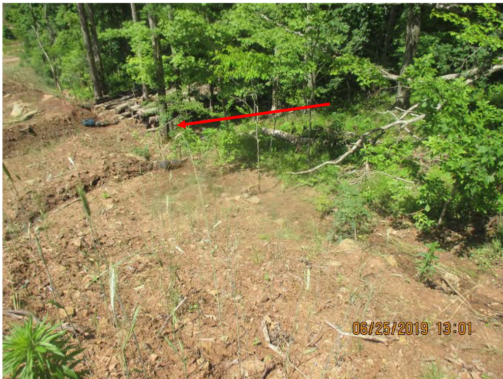
South of Station No. 5396+00. Slope above Munchausen Road Crossing leading toward waterbar and perimeter controls. Sediment being deposited against log piles past LOD.
