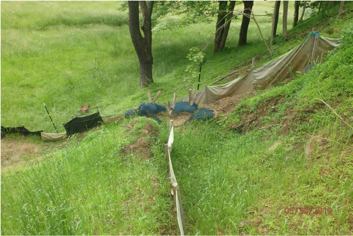
Water bar that terminates inside of the installed perimeter control adjacent to 2452+14.
