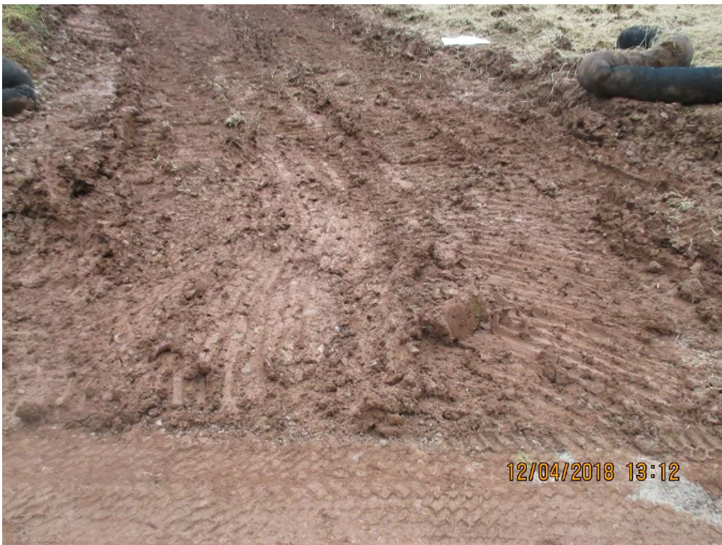
Facing North at MXP ROW entrance at station number 6880+41.
