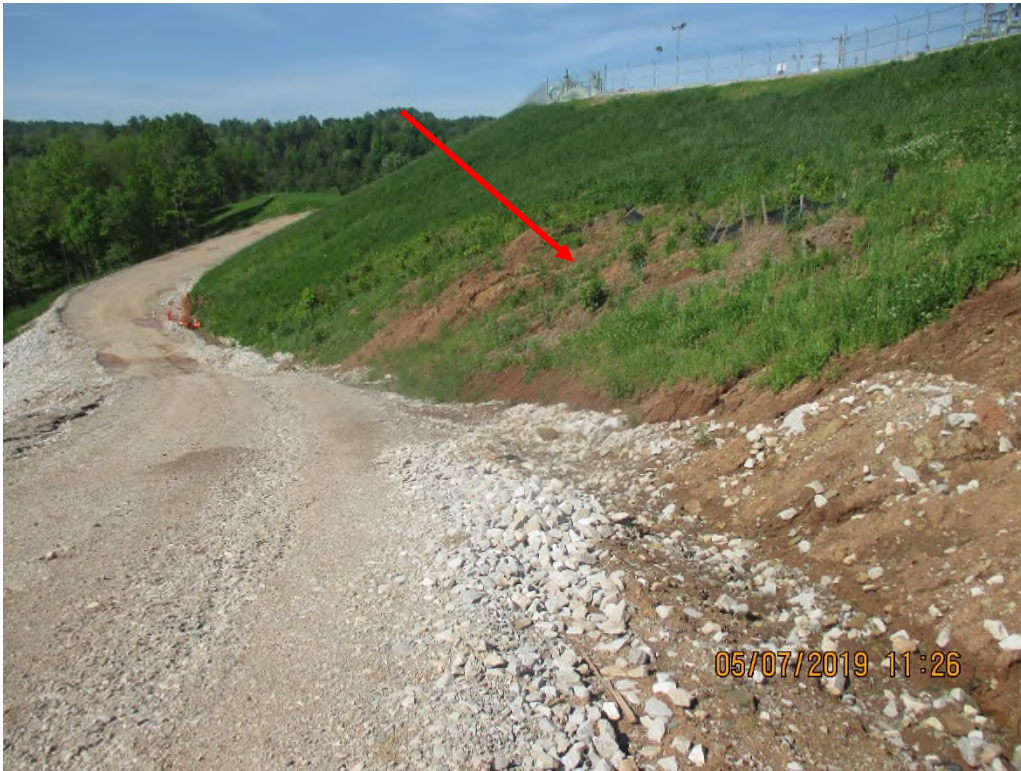
Ditch line along access road below erosion that was taking place along south slope of compressor station pad. Arrow depicts unstabilized portion of slope above ditch and culvert inlet.
