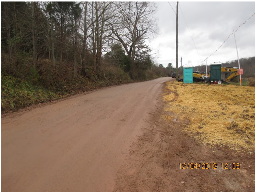
MXP ROW entrance facing South on Shamblin Road.
