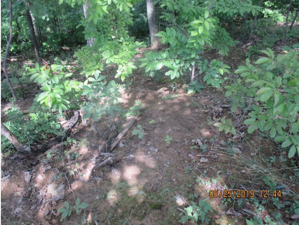
Sediment being deposited past LOD at station No. 5396+00.
