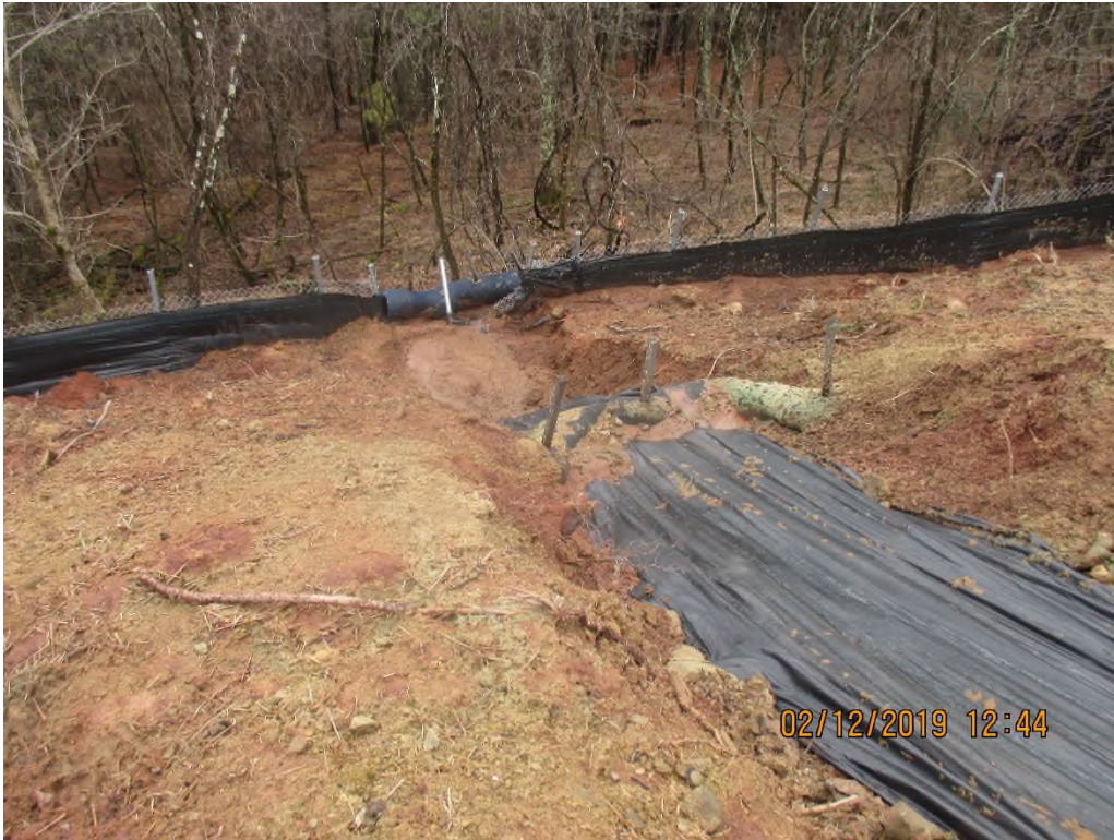
Waterbar outlet at perimeter control. Ephemeral stream impacted with SLW past LOD near station 5376+00
