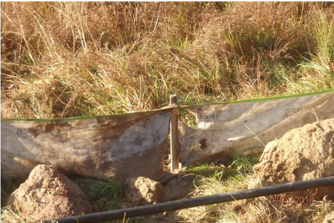
Unmaintained perimeter control in the Bluestone Creek watershed.
