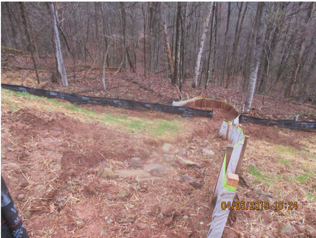
Waterbar terminating on fill slope. Erosion present on fill slope with sediment being deposited behind perimeter controls.
