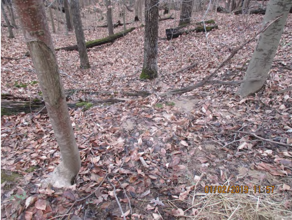
Sediment deposits beyond LOD and BMP along access road.
