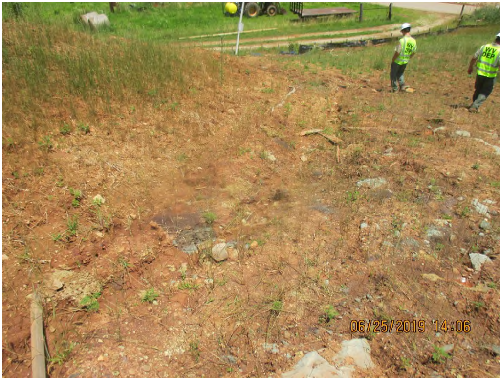
Middle Fork Road Crossing at station No. 5643+50 above stream SRUA 005 facing downslope. Waterbars eroded out where they were tied into topsoil pile.
