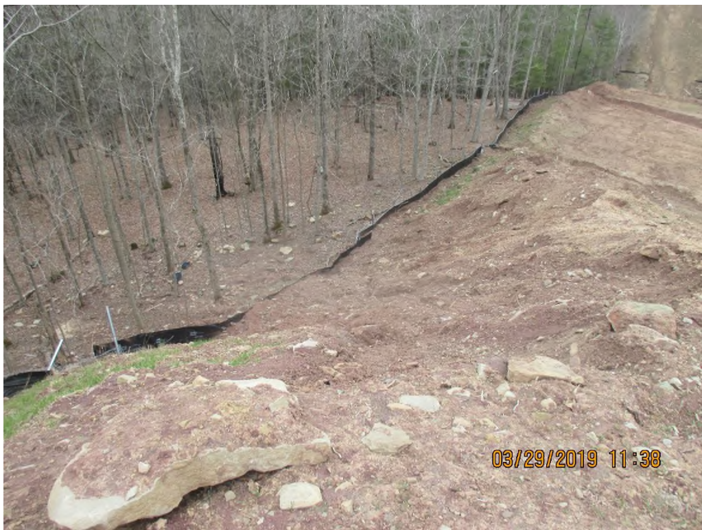
Fill slope eroded above stream SWIF-057. Sediment deposits overwhelming controls and being deposited past LOD near station #5163+50.
