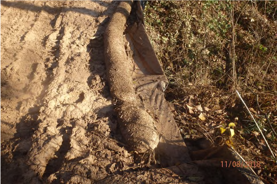
Unmaintained equipment bridge BMP in the Bluestone Creek watershed (SDOG201).
