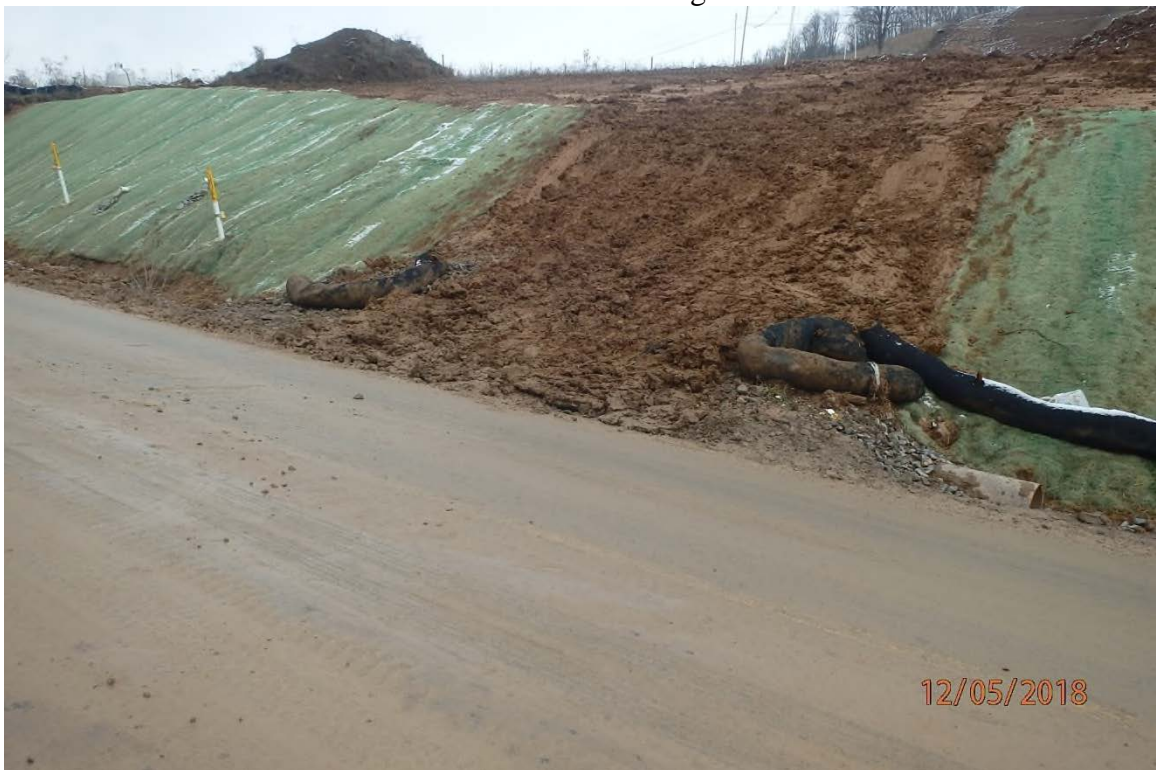
Unstable construction entrance at the WV 18 crossing and the associated track out/slick film of mud that originates from site.
