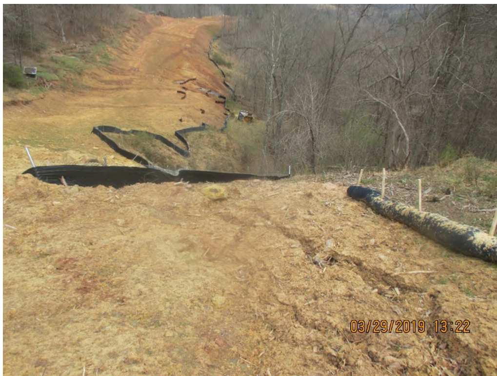
Downslope of waterbar near station #5180+43. Erosion occurring along perimeter.
