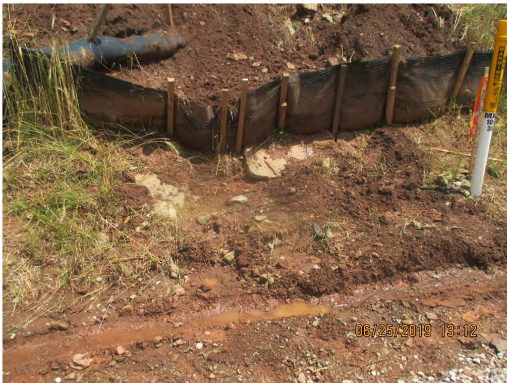
Facing upslope at controls above ditch line that parallels Munchhausen road. Sediment laden water and deposits present in ditch.
