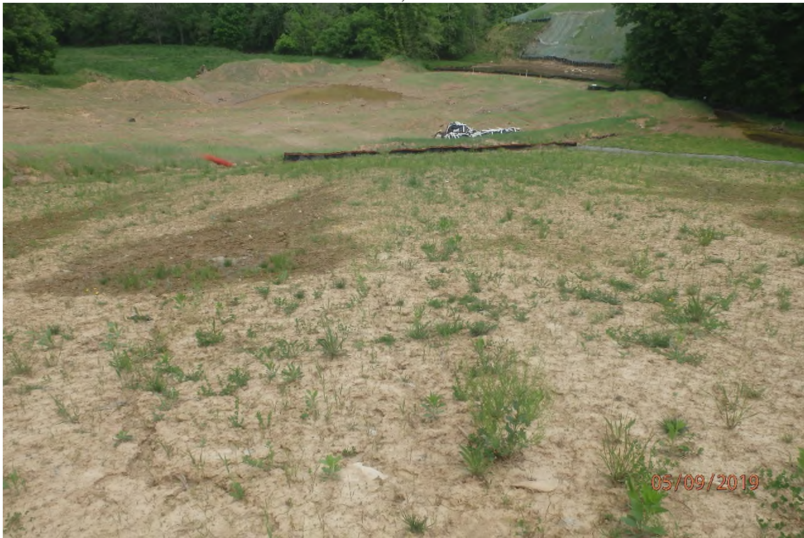
Slope adjacent to the fill pad showing the lack of installed slope interceptors. Area in need of reseeding.
