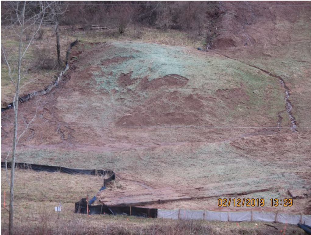
Munchausen Road crossing at station #5407+07 facing south. Erosion present on slopes due to concentrated flow
