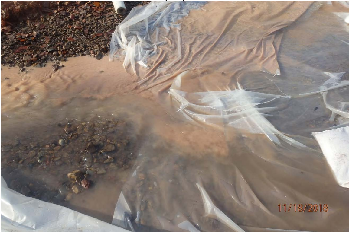
Visible plume in UNT Georgescamp Run (SDOG048) ( 39^{\circ} 15.261' X 80^{\circ} 44.096' ) at outflow of the installed pump-around.
