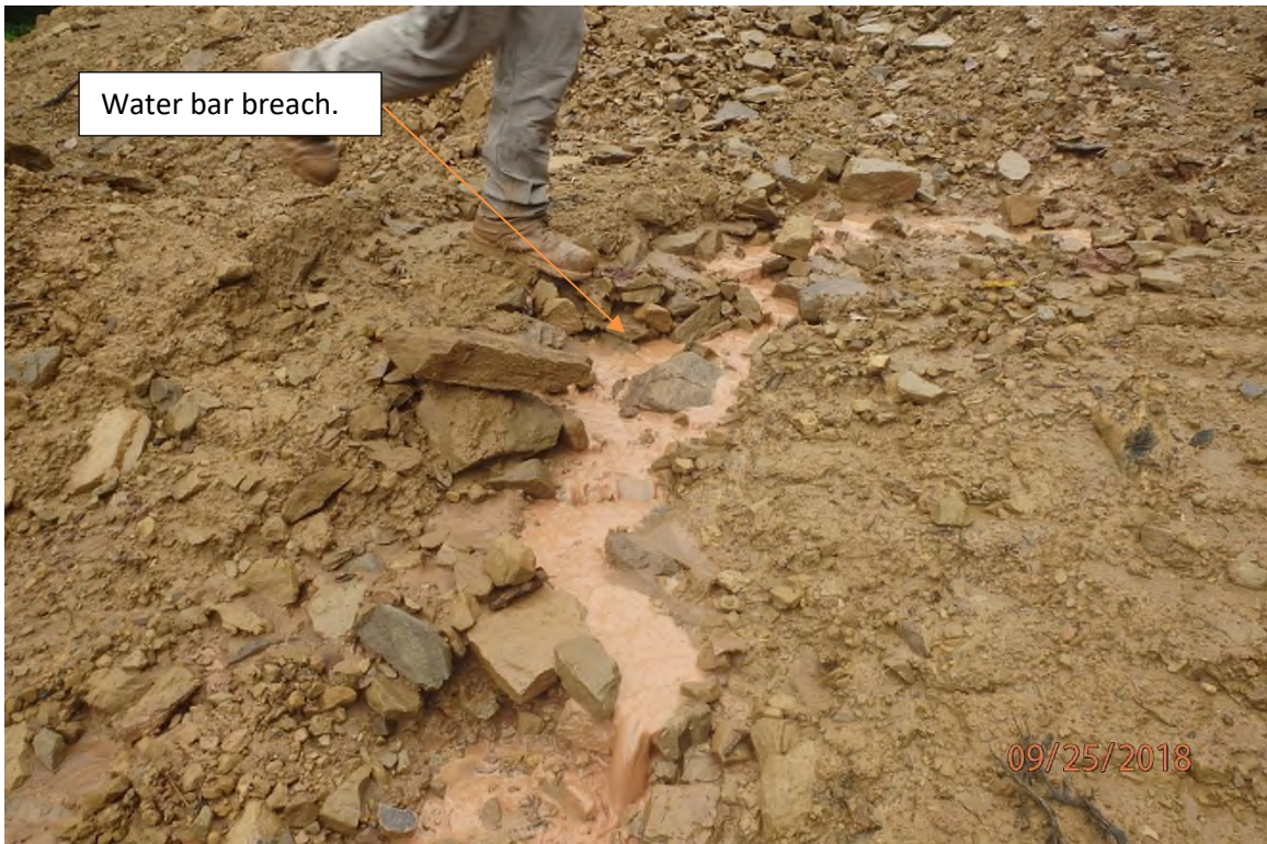
Poorly maintained water bar adjacent to ARDO002.8 that is placing concentrated flow over a fill slope.
