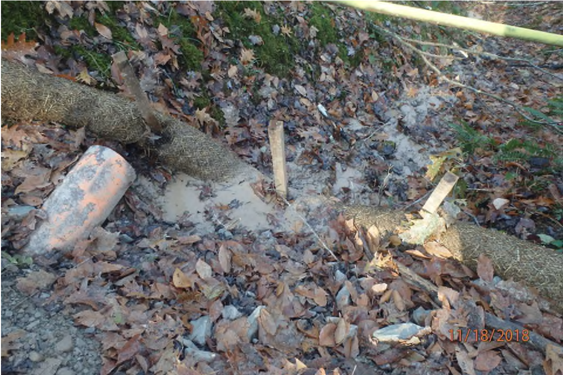
Outlet of the above pictured culvert outlet on ARDO008.2 showing sediment laden water bypassing the installed BMP that is in need of maintenance.
