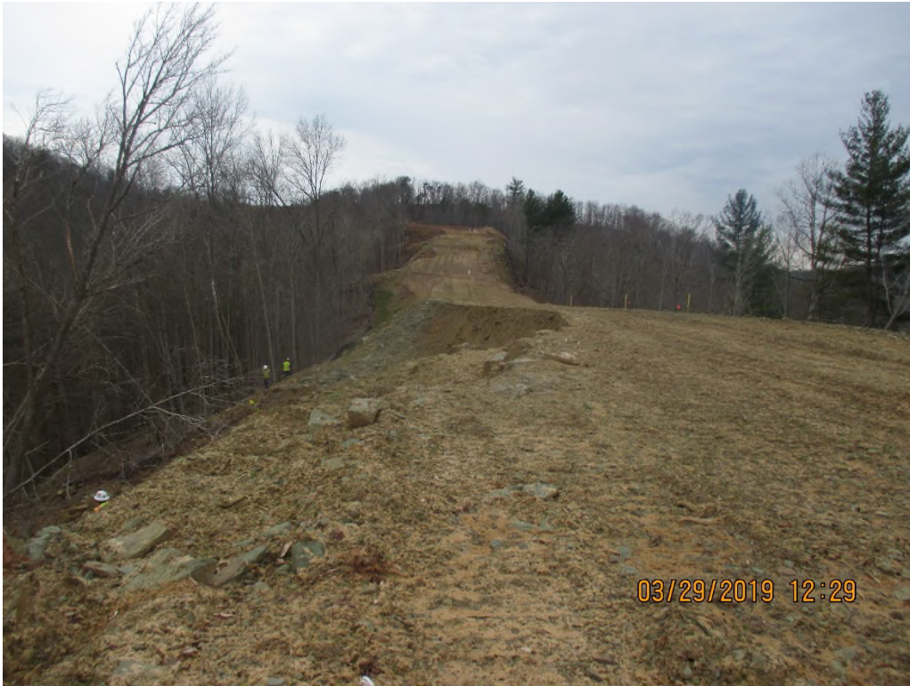
Station #5163+50 facing South at section of Row that slipped into Stream SWIF-057
