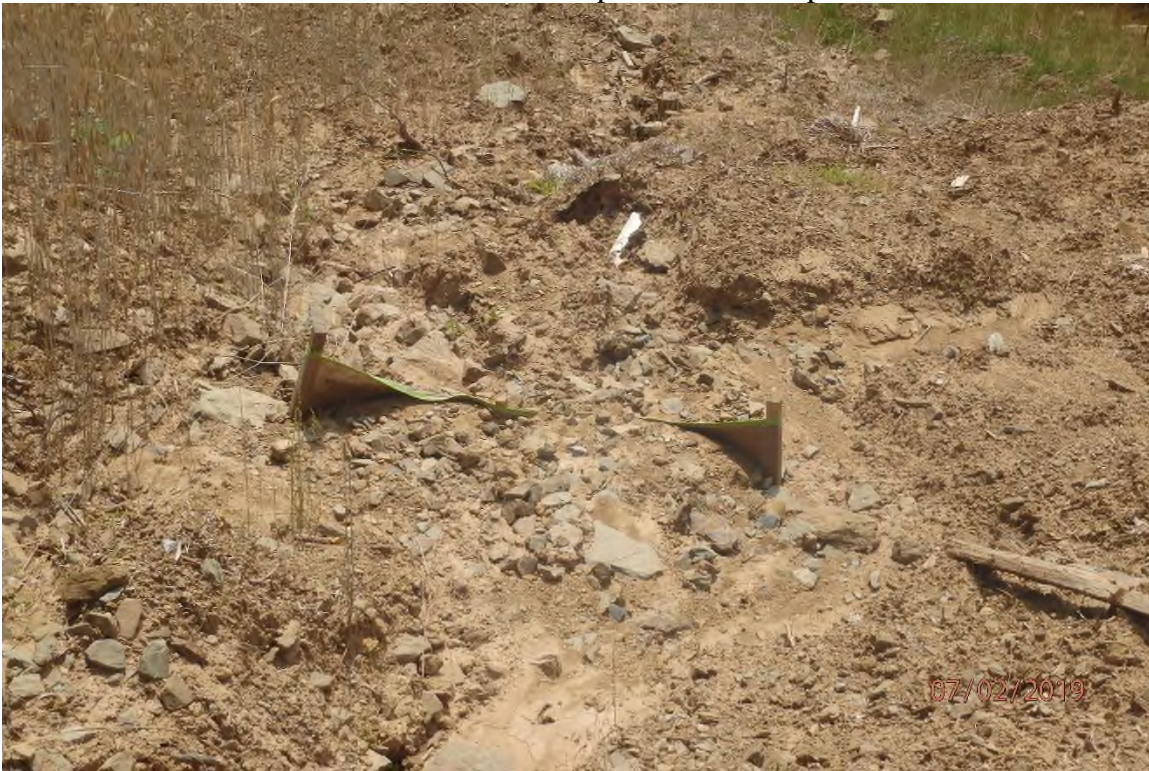
Fill slope erosion downslope of the above pictured deficiency. Silt fence ditch check in the erosion gully has become inundated with sediment.
