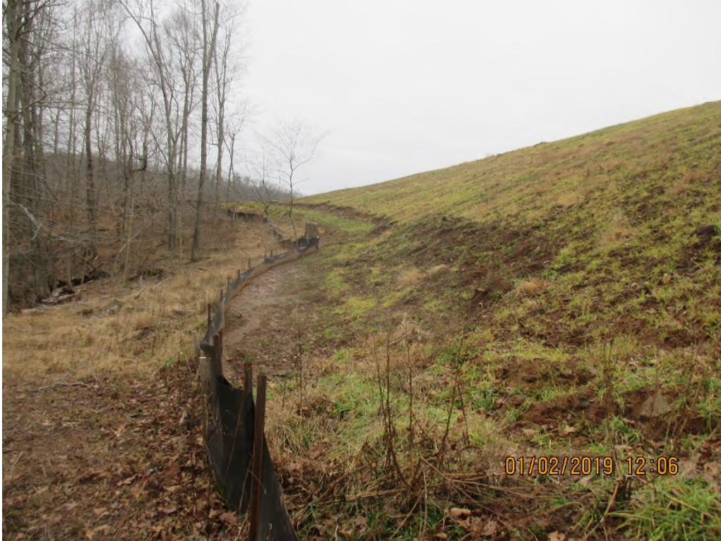
North west slope. Slope is eroding above silt fence.
