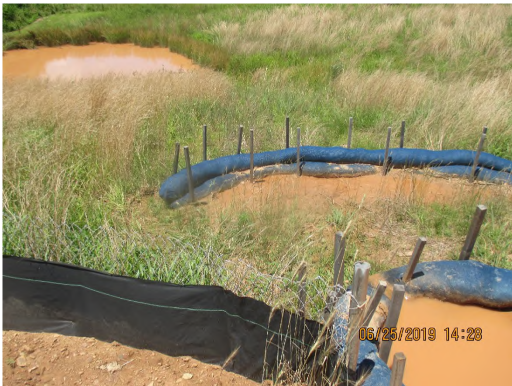
Perimeter controls at station No. 5638+46. Impacted pond downslope of controls.
