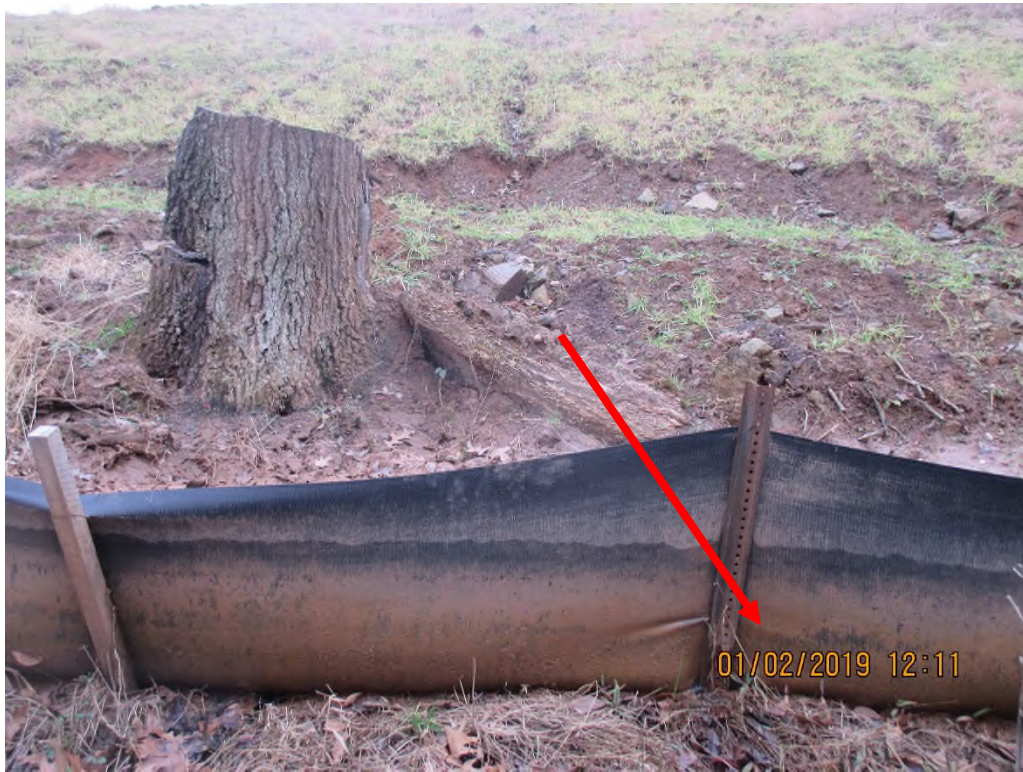
Silt fence with hole.
