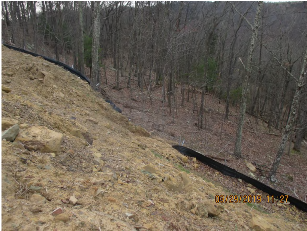
Perimeter controls being overwhelmed with sediment near station #5148+00.
