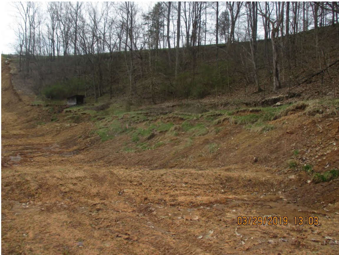
Section of adjacent land that slipped into ROW and within LOD near station #5180+43
