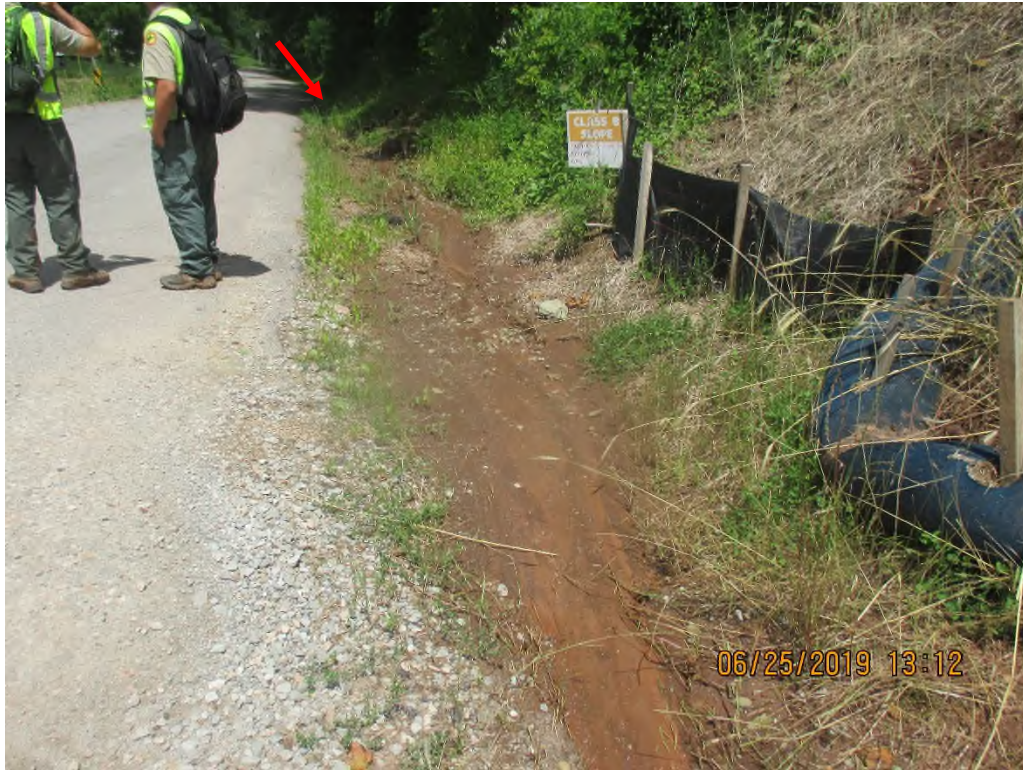
Munchausen Road crossing and ditch with sediment deposits. Ditch conveys to culvert that conveys under road to grass field outside of permitted workspace and LOD. Arrow depicts culvert approximate location.
