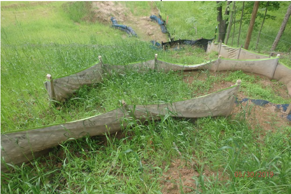
Fill slope erosion downslope of the above pictured water bar.
