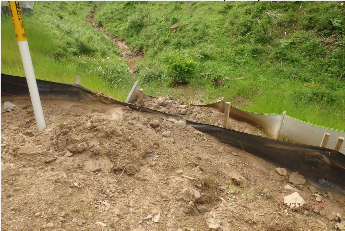
Unmaintained BMP in the UNT Sugar Run watershed.
