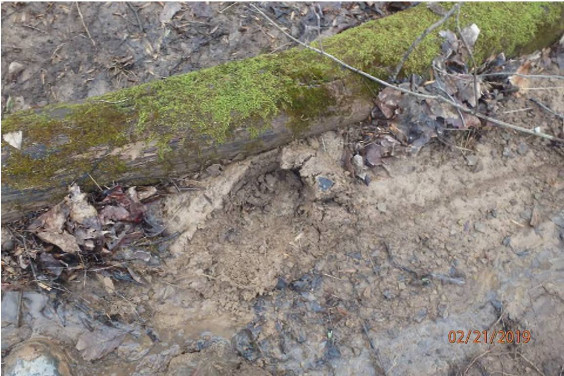
Offsite sediment deposits downslope of the above pictured BMP.
