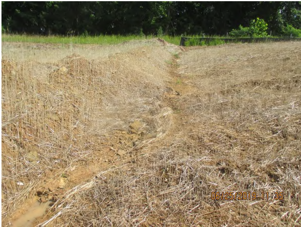
Upslope at station No. 5355+67. Erosion present in waterbar.
