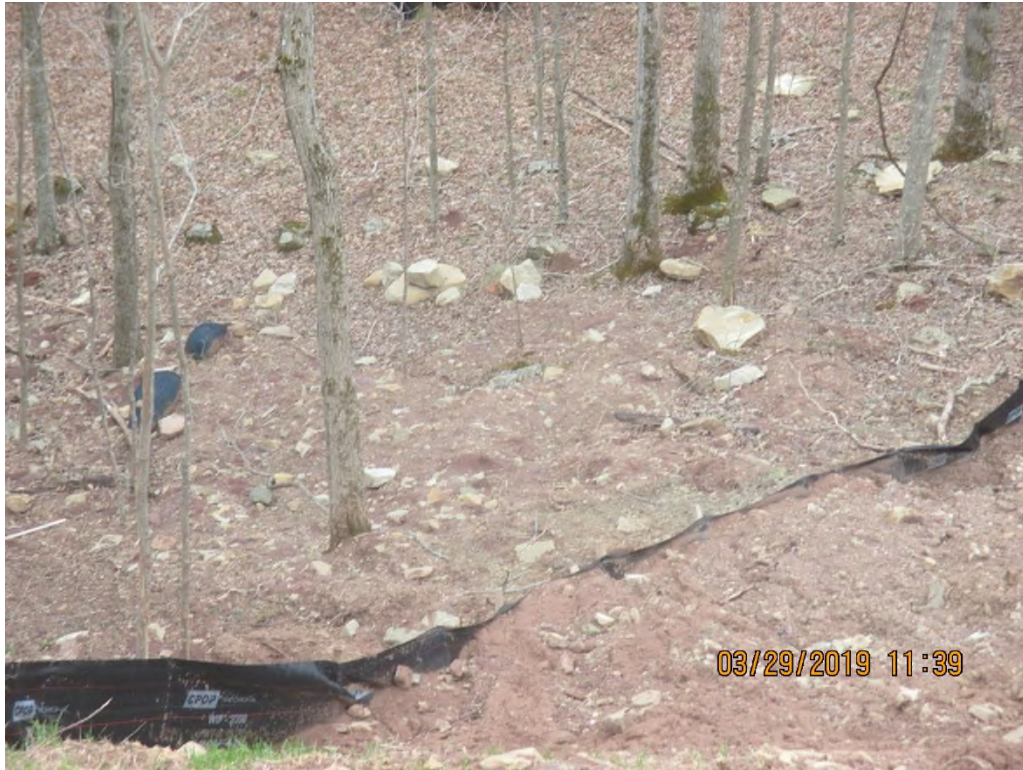
Sediment overwhelming controls and being deposited past LOD near station #5163+50
