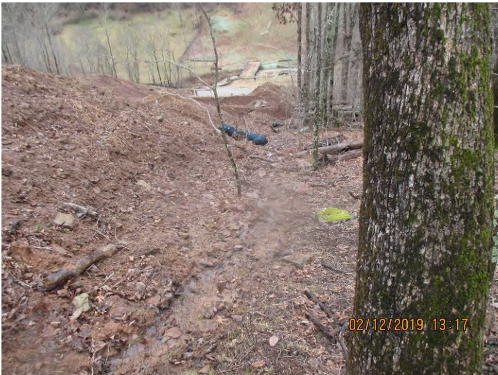
Runoff from waterbar outlet running downslope towards log pile off LOD
