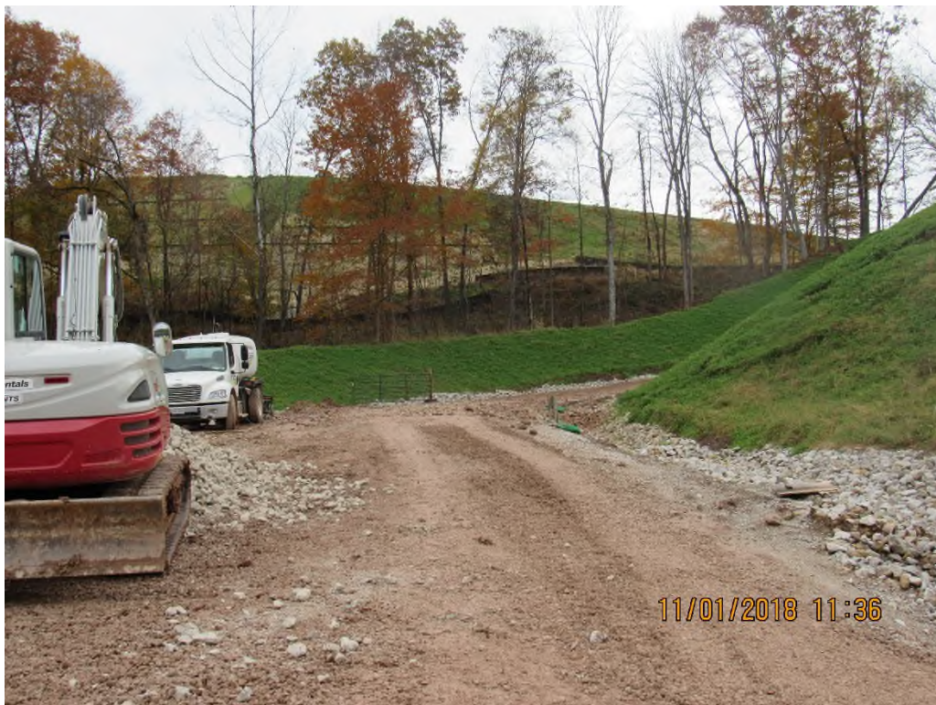
View of the "exit" road that passes through wash station.
