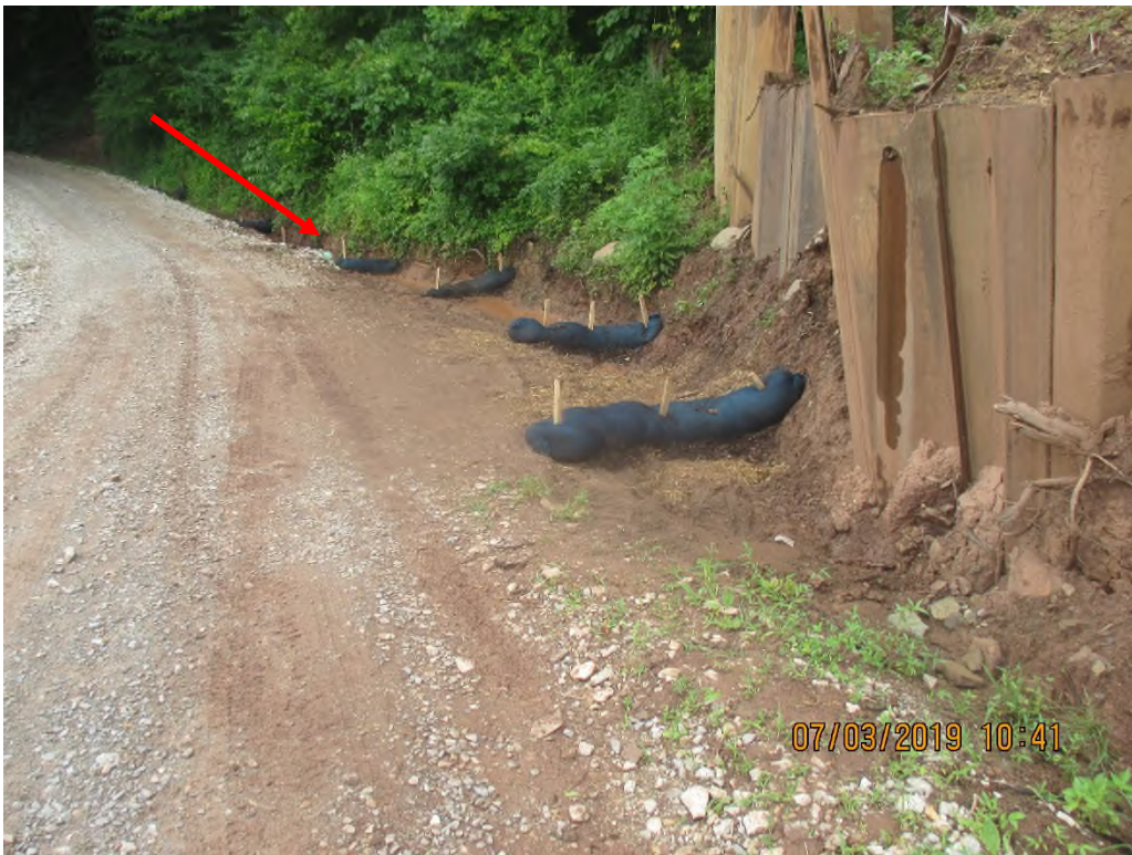
Facing toward ditch line along Sulu road below slip. Arrow depicts culvert inlet.
