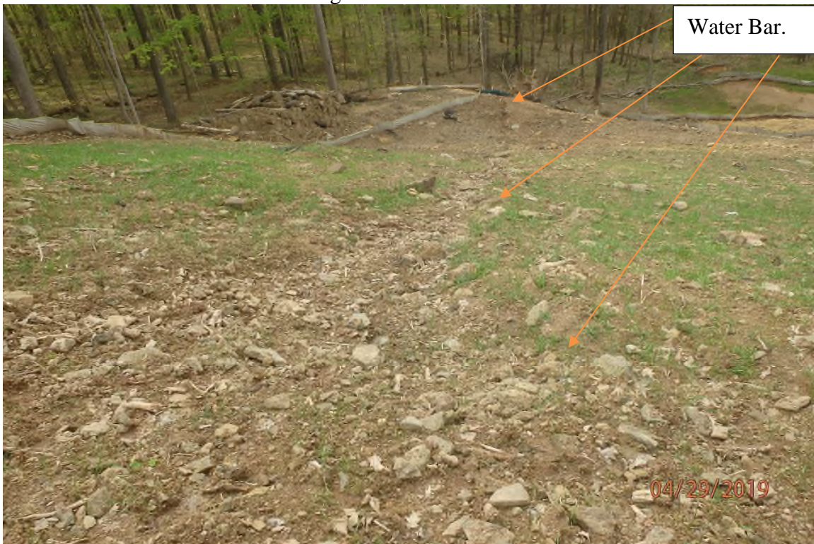
Water bar adjacent to 2225+00 installed at an angle greater than 12%.
