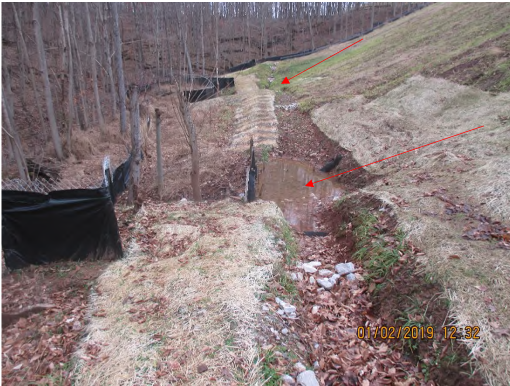
North slope of project where several discharge points (silt fences labeled as 23 and 24) are located along diversionary berm.
