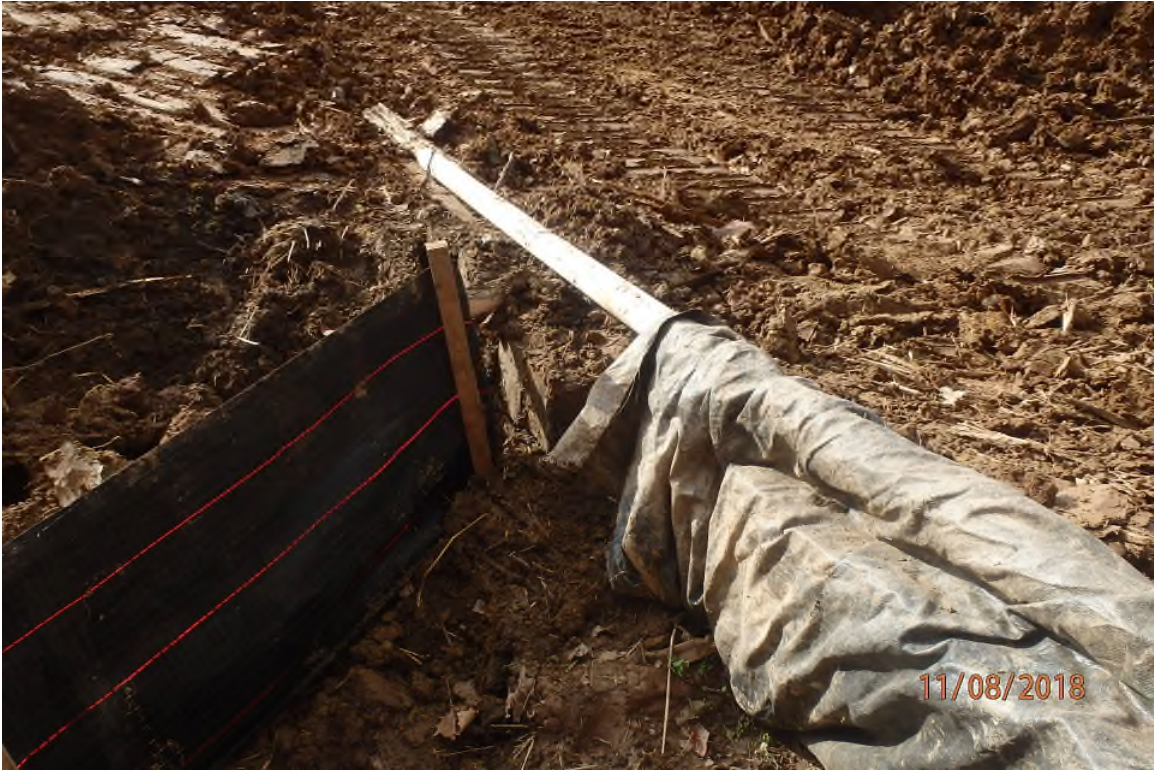
Unmaintained equipment bridge BMP in the Bluestone Creek watershed (SDOG0048).
