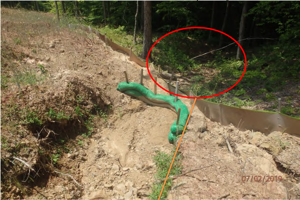
Low area adjacent to UNT Left Fork of Arnolds Creek (SDOG057) where stormwater from a large area is directed due to improperly installed water bars that don't discharge stormwater offsite in small quantities as designed. BMPs are inundated with sediment and in need of maintenance as a result.
