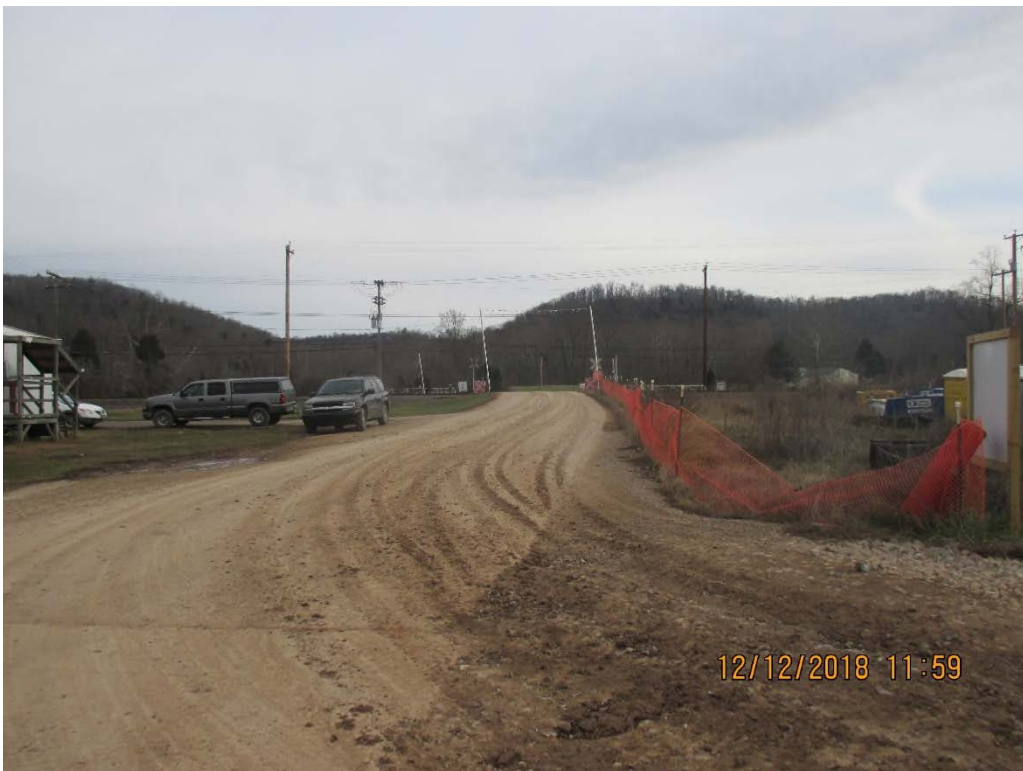
Tracking occurring onto access road, facing North towards Route 62.
