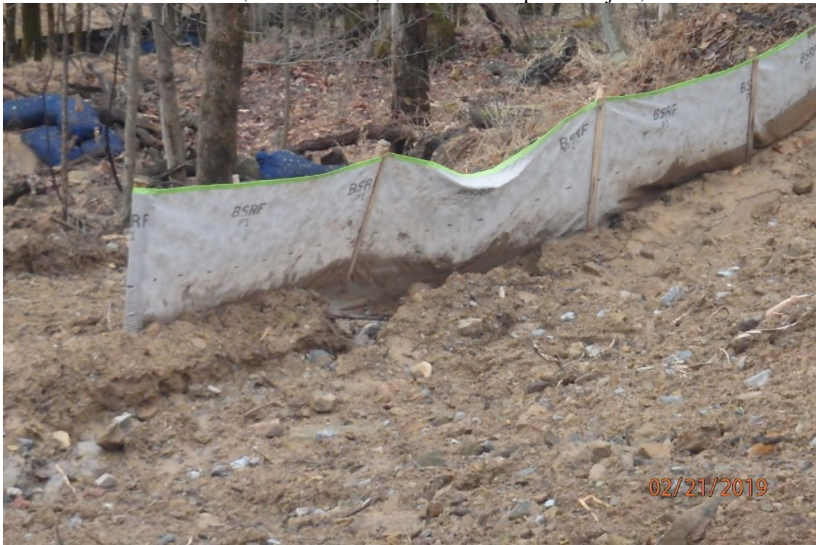
Perimeter control in need of maintenance.
