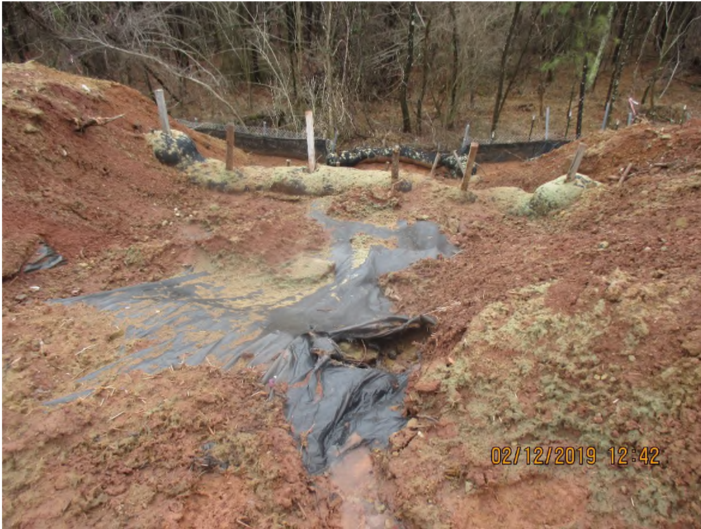
Waterbar outlet near station 5376+00
