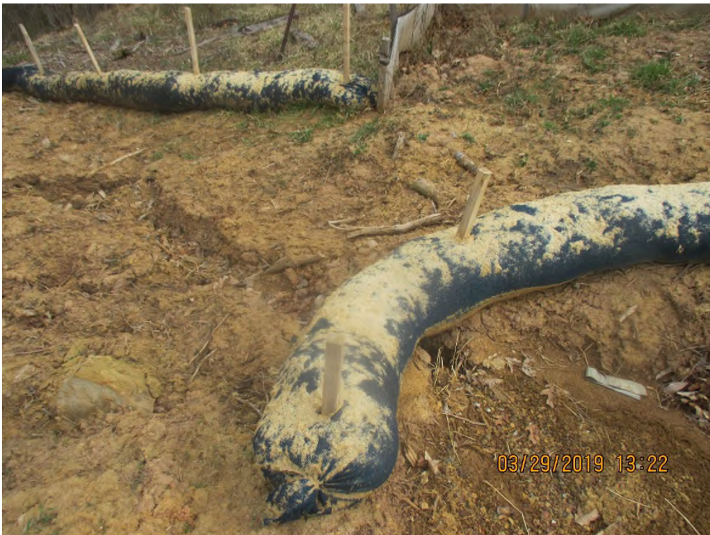
Waterbar terminus near station #5180+43. CFS is being undercut and erosion is occurring downslope of the control along the perimeter.
