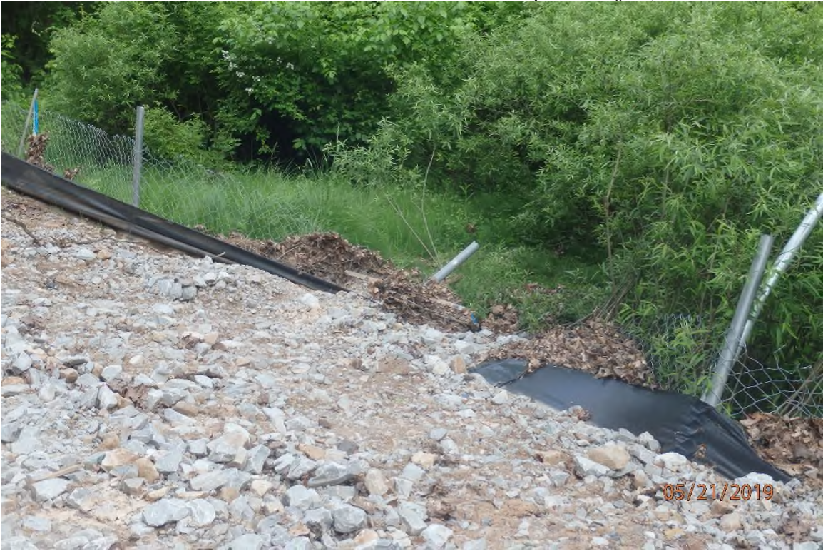
Unmaintained BMP on ARDO016.
