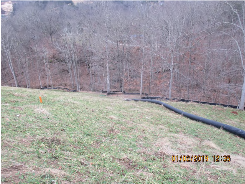
Slope drain terminus at silt fence labeled as 30.
