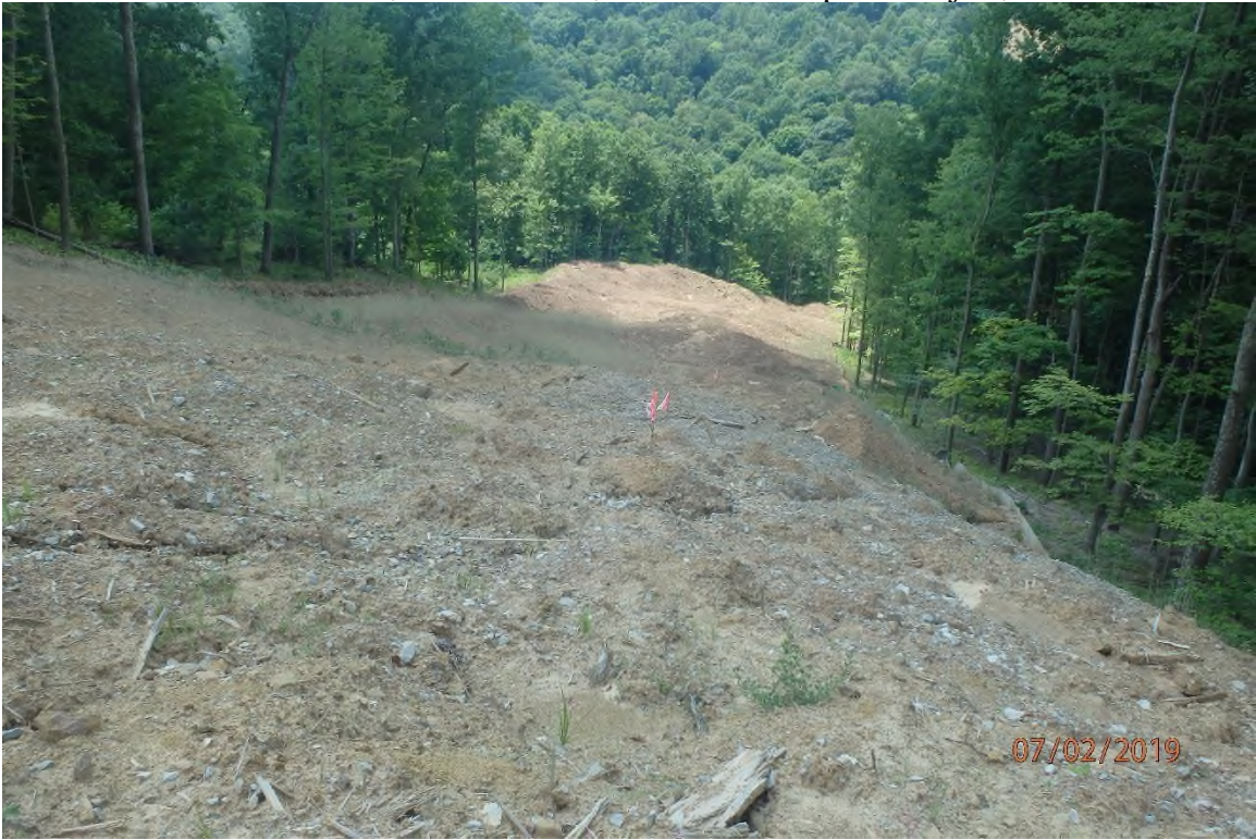
Improperly installed water bar in the UNT Left Fork of Arnolds Creek watershed. Water bar is installed at a shallow depth and a steep angle.
