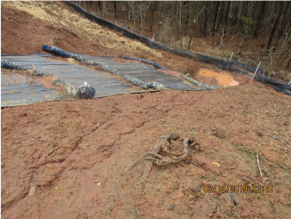
Waterbar outlet near station 5376+00
