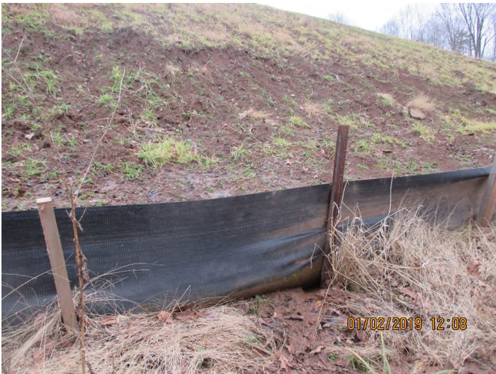
Silt fence being undermined where sediment has concentrated behind fence.
