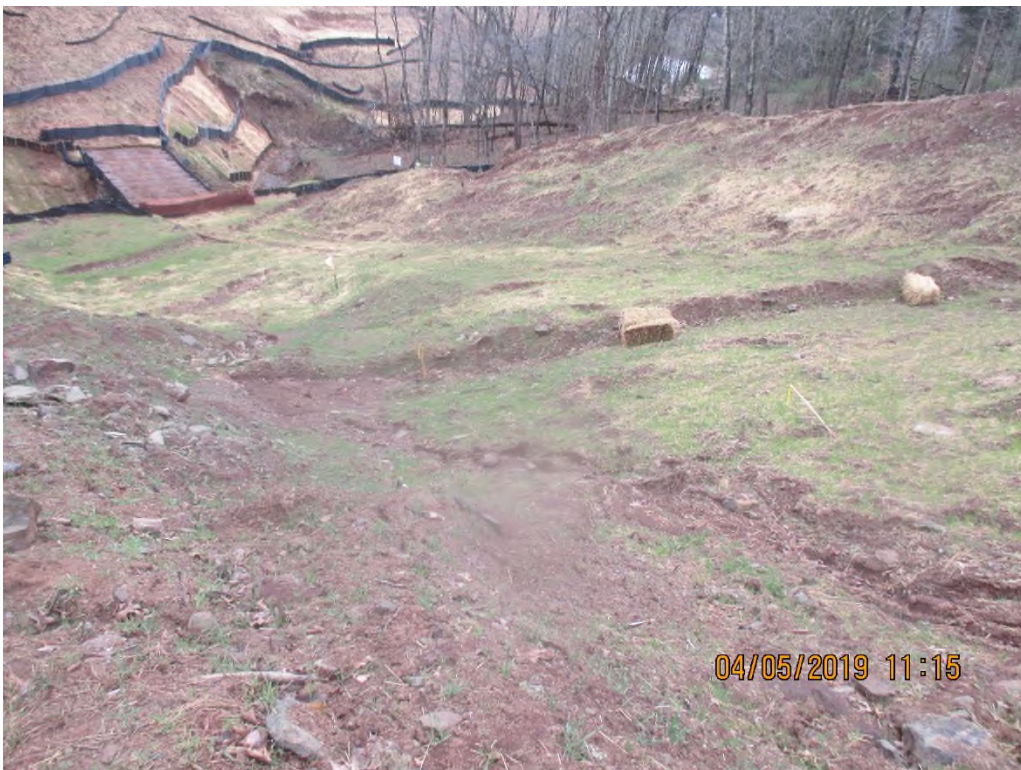
Erosion occurring on ROW between the waterbars above stream SJAG-316. These waterbars were terminating into the topsoil pile and not being diverted off the ROW.
