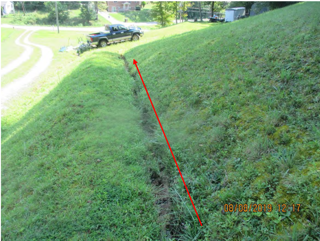
Ditch line conveying across complainants' yard towards Charles Creek Road.
