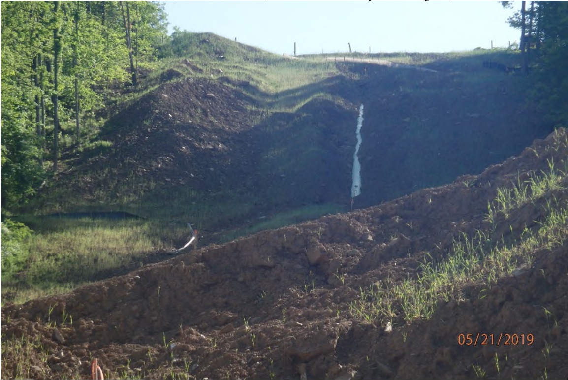
Unmaintained water bars in the Georgescamp Run watershed that have led to the exposure of the installed pipe.
