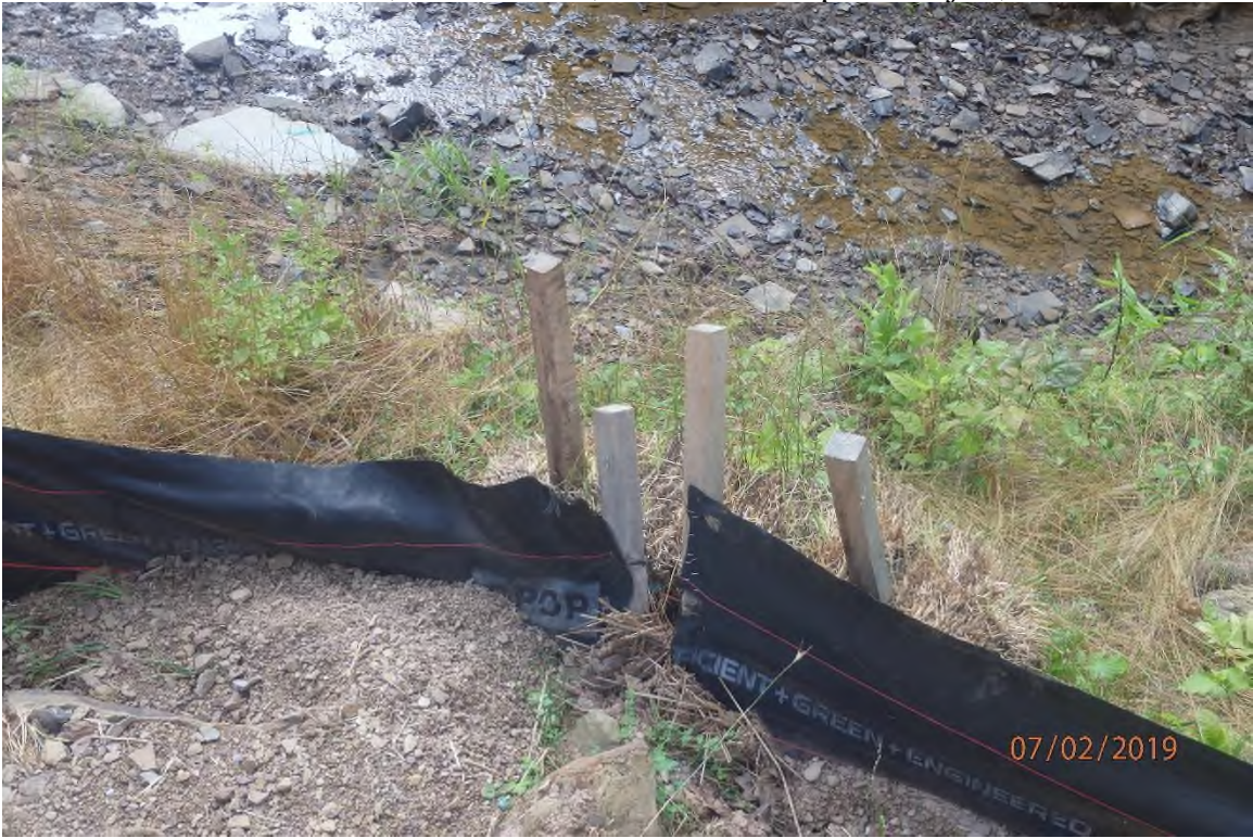
Improperly merged perimeter control adjacent to Sugar Run.
