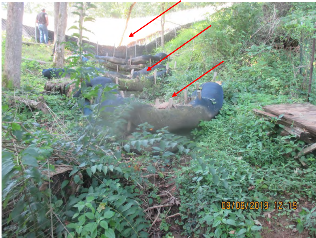
Perimeter Controls that were overwhelmed with sediment.
