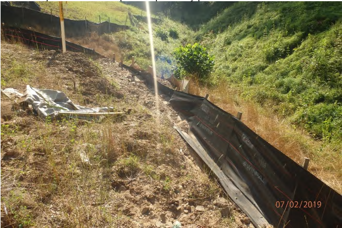
Installed perimeter control downslope of the above pictured fill slope erosion that has been overwhelmed and is placing sediment into ephemeral UNT Sugar Run (onsite stream pictured).
