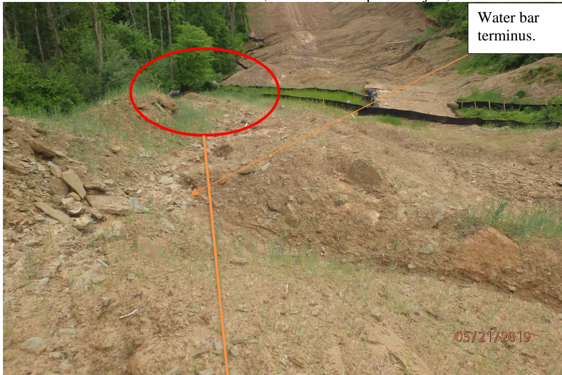
Improperly installed water bar in the S. Fork of Hughes River watershed. Water bar discharges over an unprotected fill slope.
