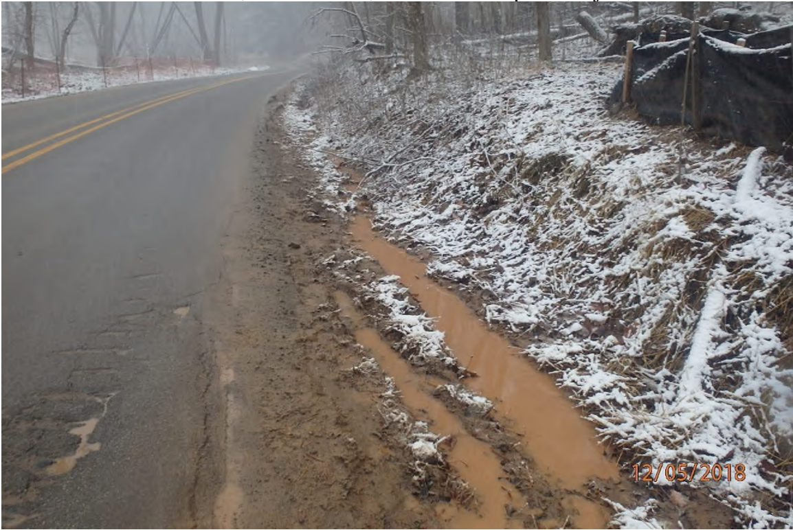
Sediment laden water that originates from the site (ARDO002.9) in DOH conveyance.
