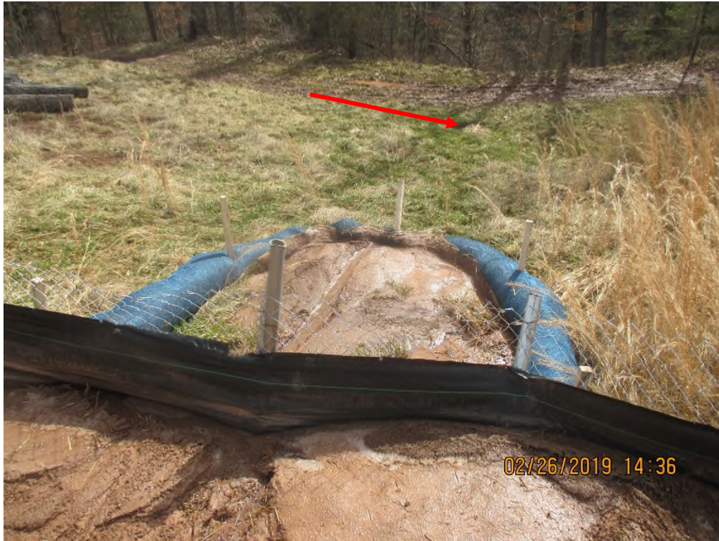
Perimeter controls near station #6727+53. Sediment deposits present and water flowing into culvert depicted by arrow.
