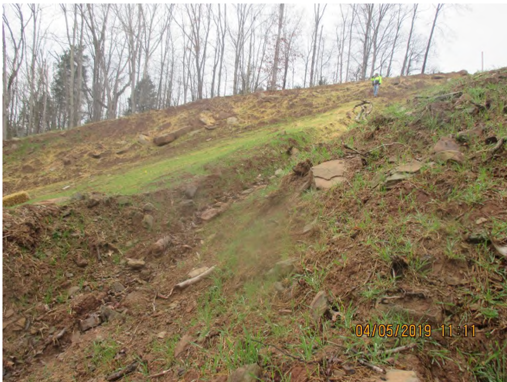
Waterbar above stream SJAG-316 terminating into topsoil pile.
