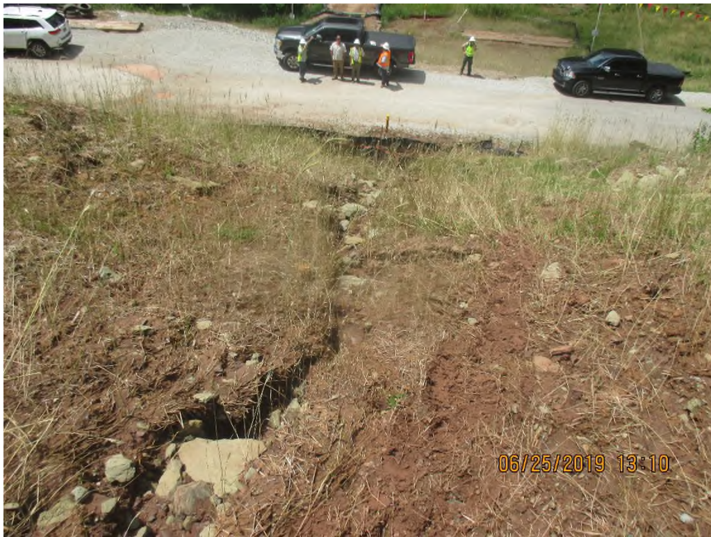
Erosion on slope above Munchausen Road crossing.
