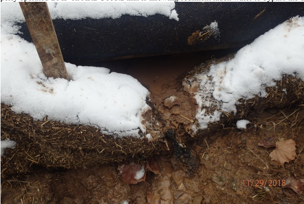
Improperly operated BMP on ARDO008.2 that is allowing sediment laden water to bypass the device.
