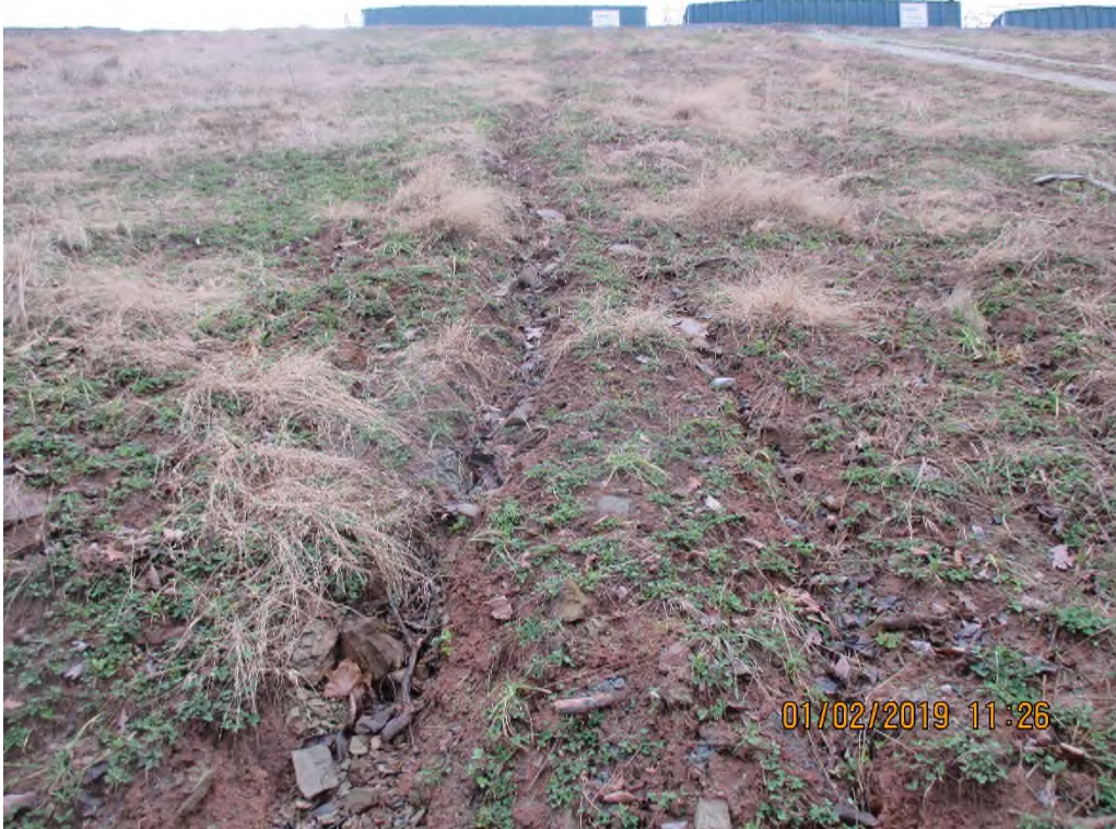
Facing toward compressor station. Erosion rills occurring along south slope.
