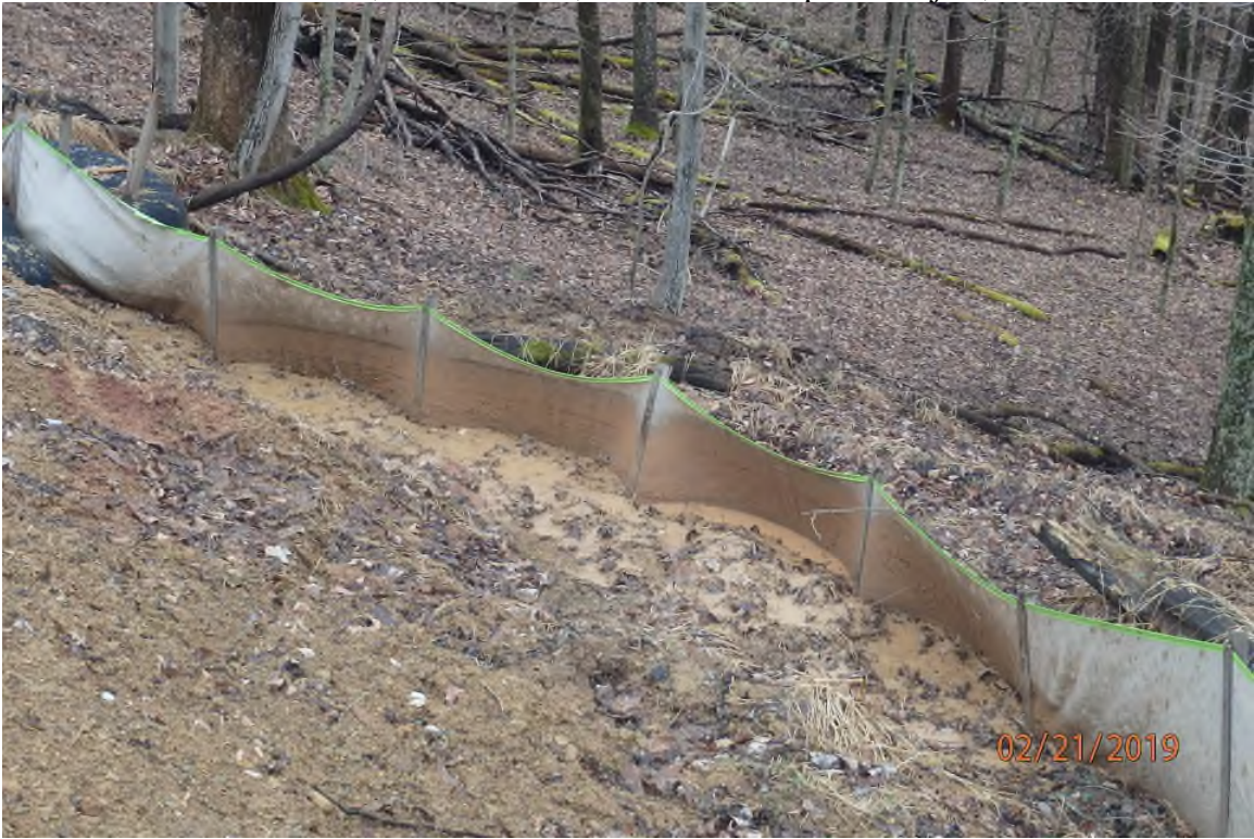
Installed perimeter control adjacent to 2256+00 that has been overwhelmed due to improperly installed water bars.
