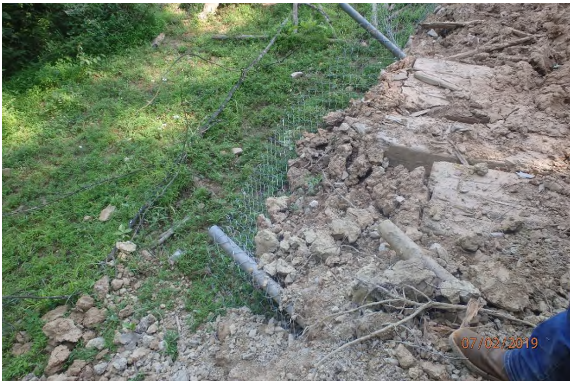
Perimeter control in need of maintenance at ARDO015.12.
