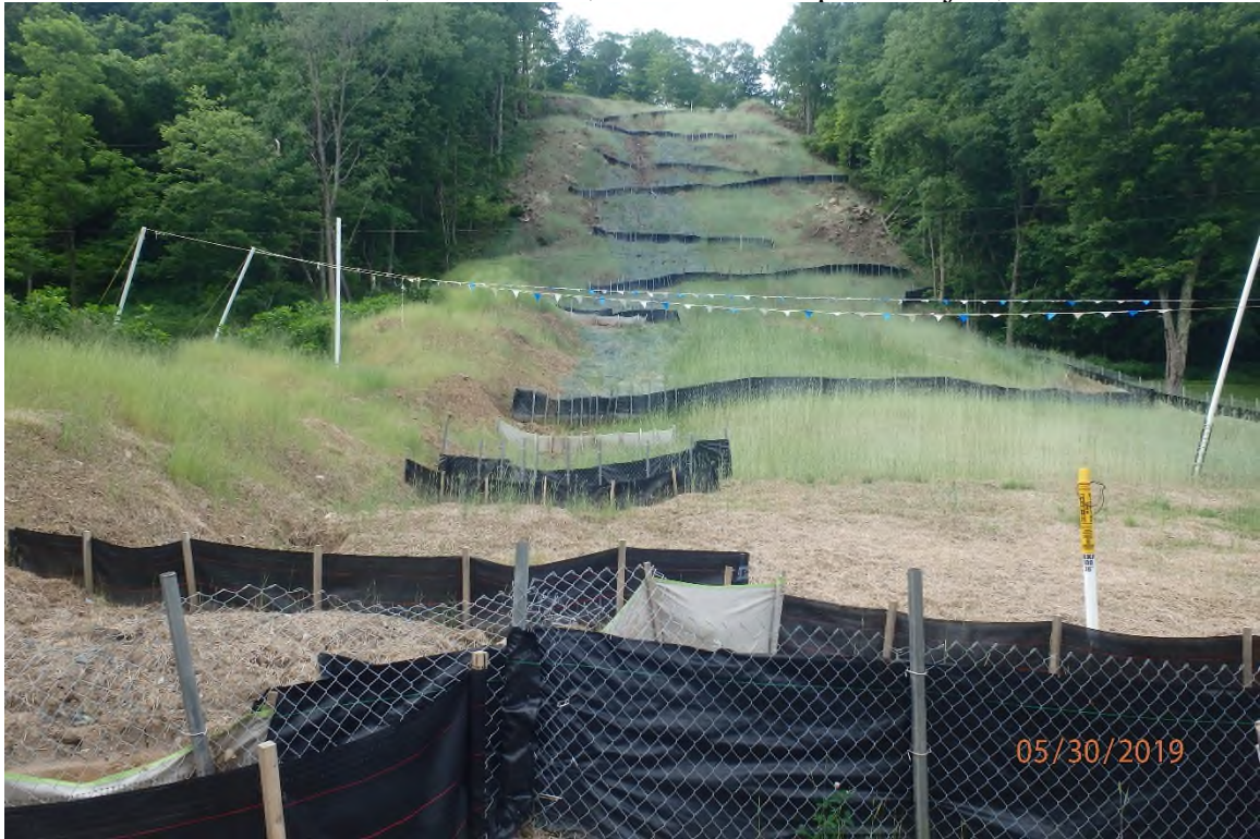
Overview of area of improperly installed water bars from 2590+00 to 2595+00.
