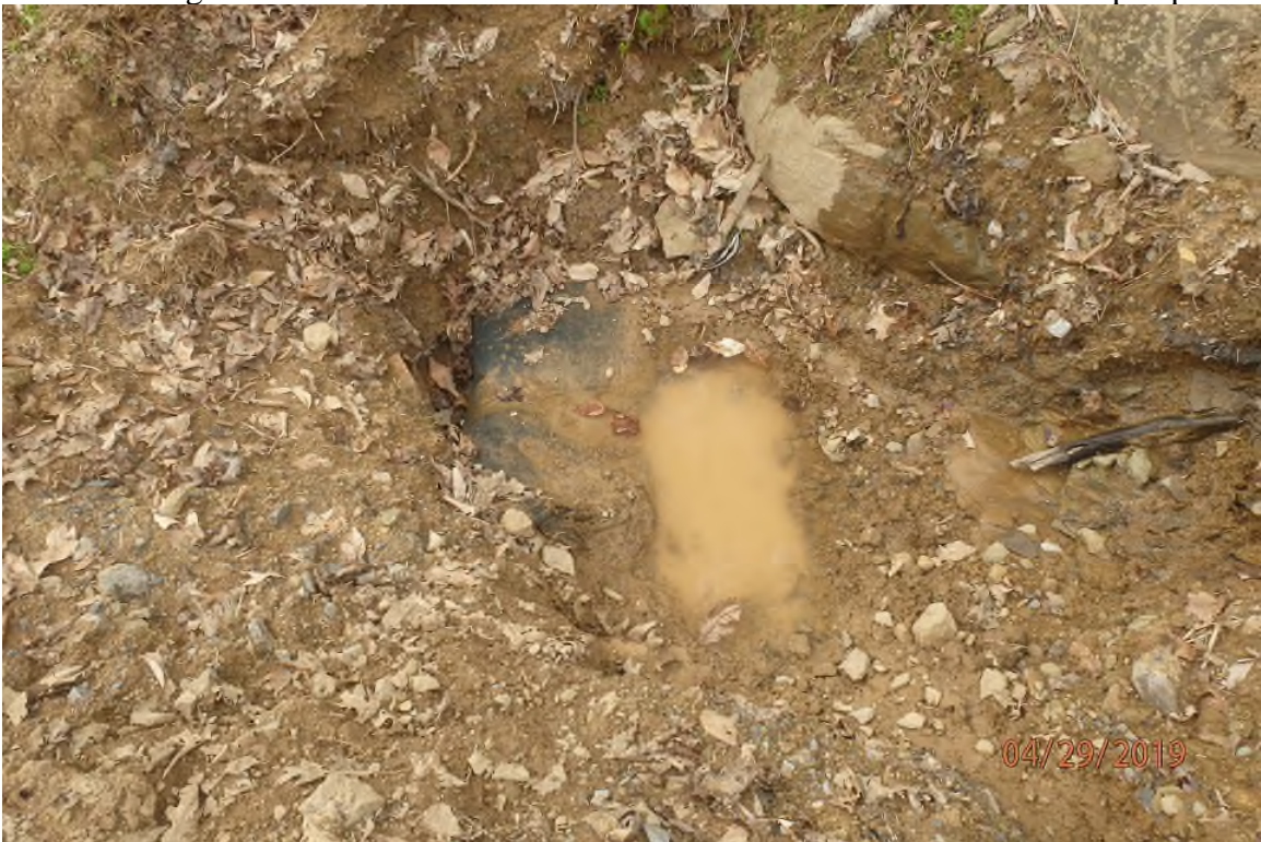
AR - 17 showing the need for maintenance to the ditch check upslope of the interceptor culvert.
