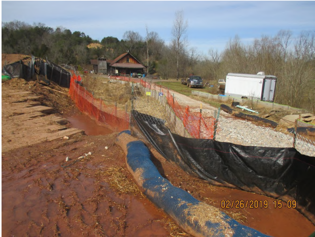
SJAG-346 facing downslope at station #6702+30
