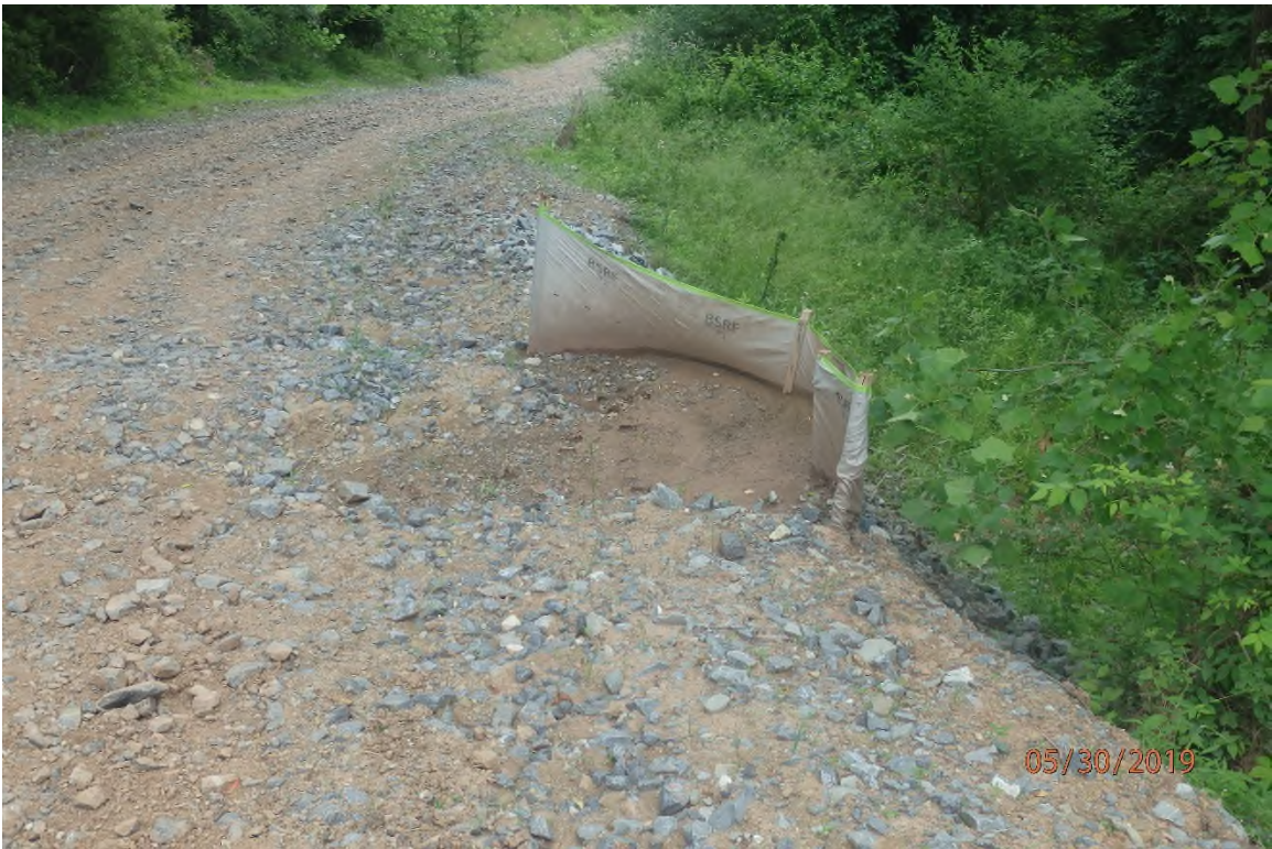
Access road ARDO004 showing the need for maintenance and stabilization.
