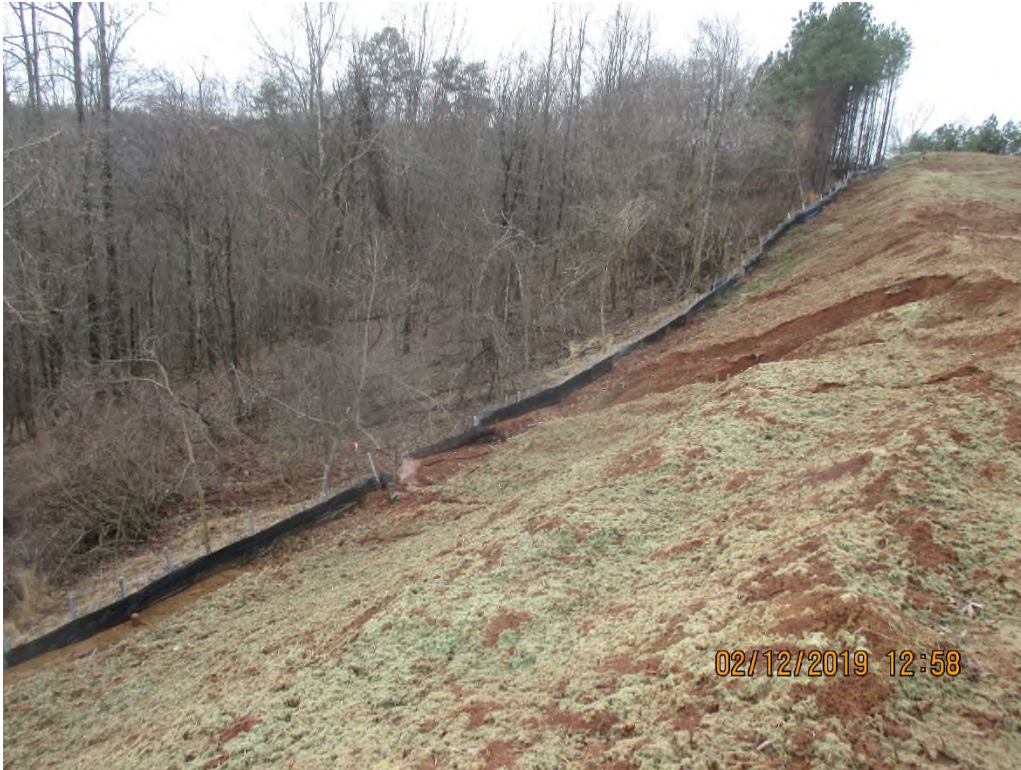
Facing South at station 5388+00 downslope at perimeter controls and top of slope
