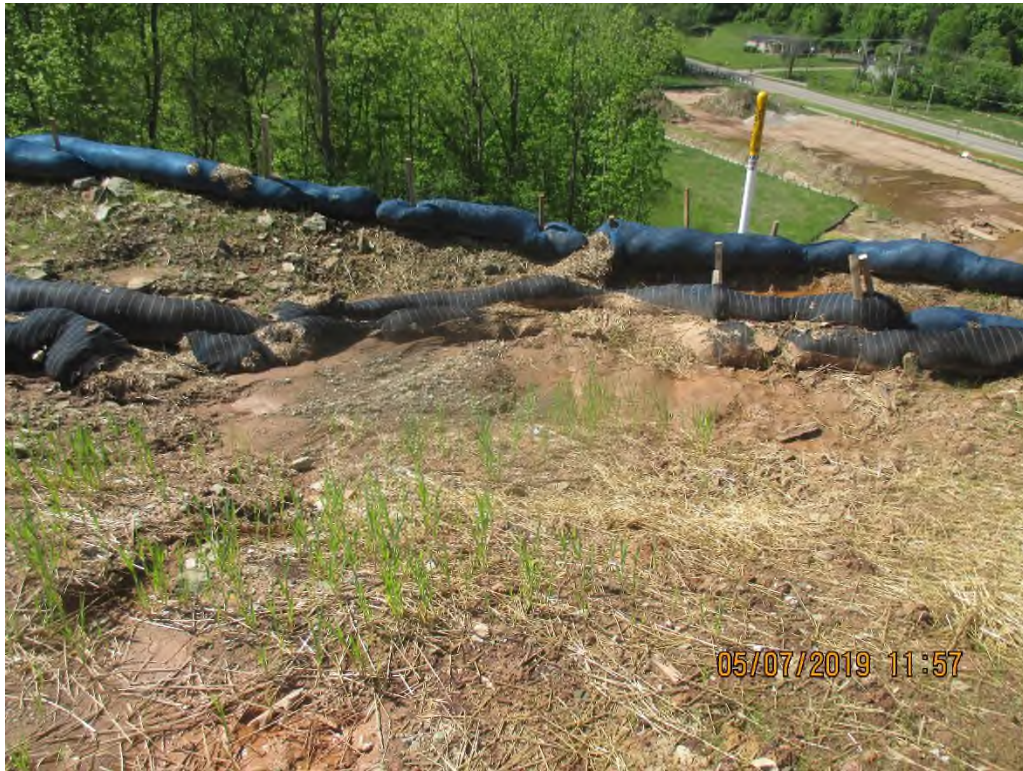
Controls on West side of unstabilized slope facing MXP Spread 7 and Route 21.
