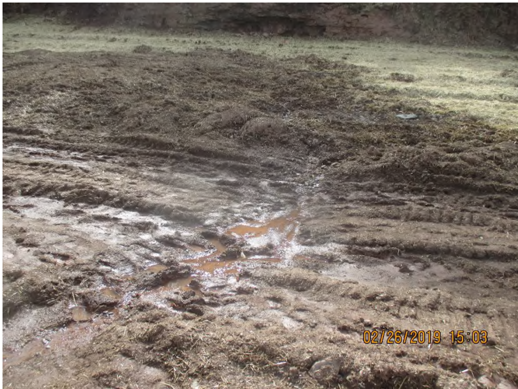
Saturated section of ROW near station #6720+60 leading to erosion downslope of travel lane.
