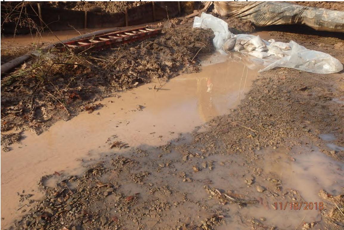
CNA distinctly visible settleable solids in UNT Georgescamp Run (SDOG048) (39° 15.261' X 80° 44.096) as a result of the above pictured dewatering.
