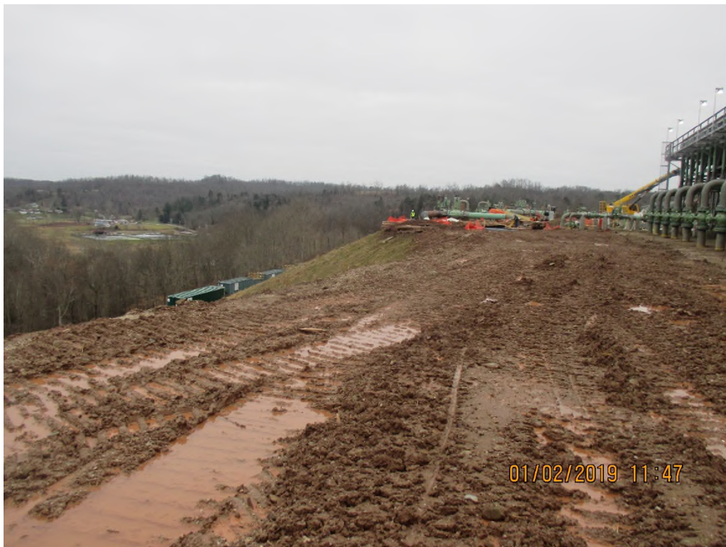
Top of slope facing section of slope not stabilized.
