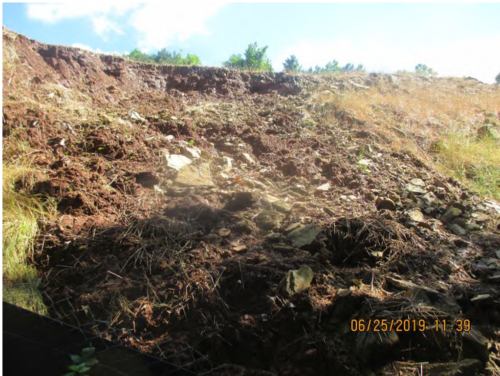
Facing upslope at station No. 5355+67 where slip was occurring and depositing sediment against and over perimeter controls.
