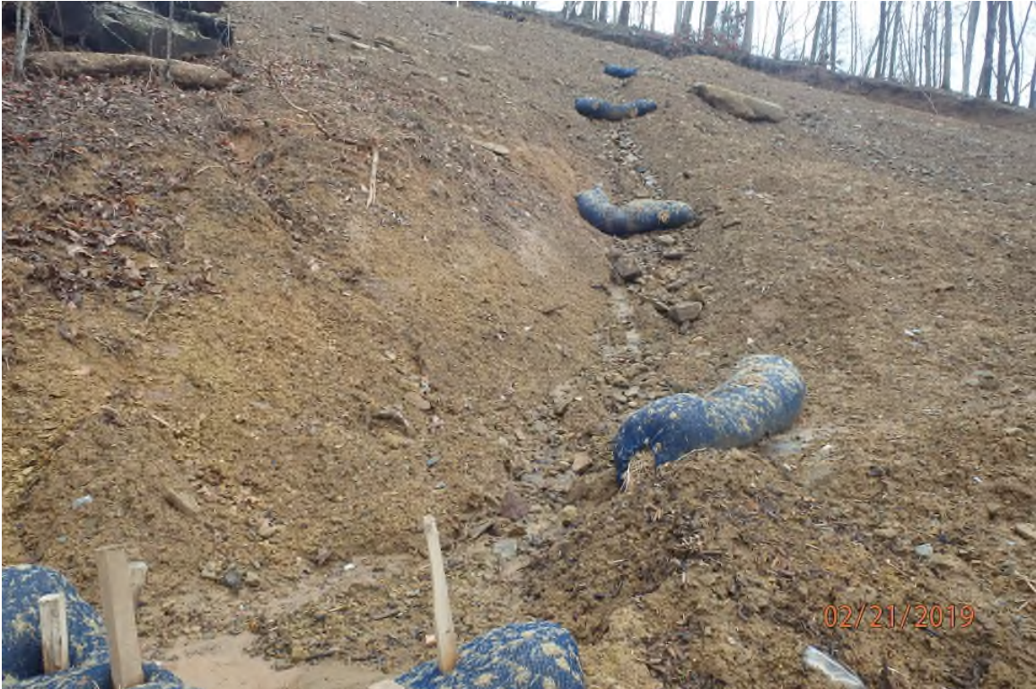
Water bar on right of way that discharges into upslope ditch of ARDO002.8
