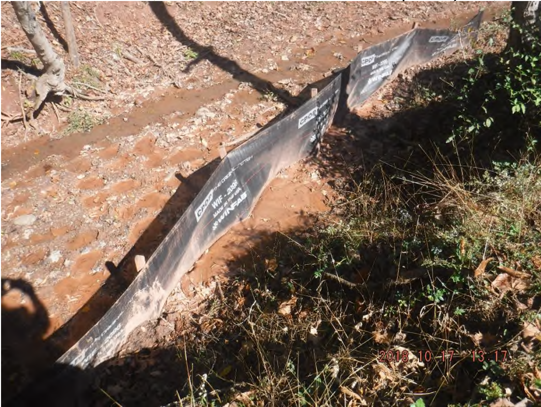
Sediment collected behind the in-stream silt fence.
