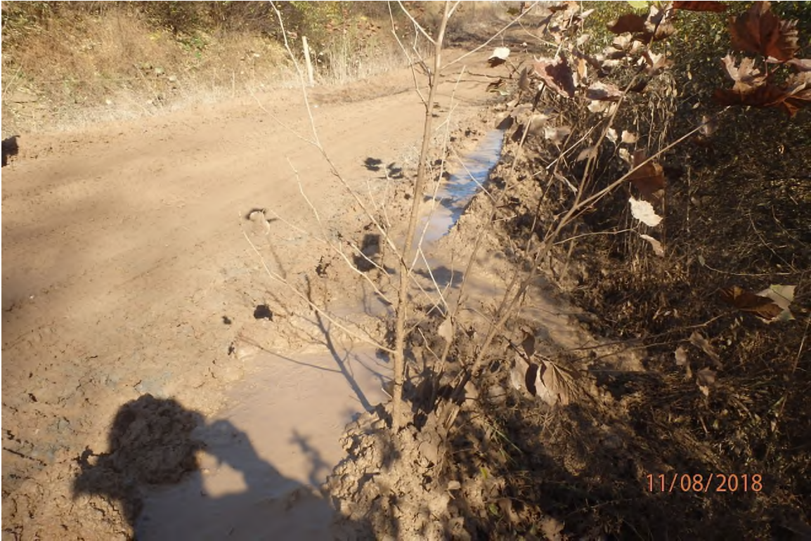
Existing access (ARDO9.3) that requires construction activity with no BMPs in place.
