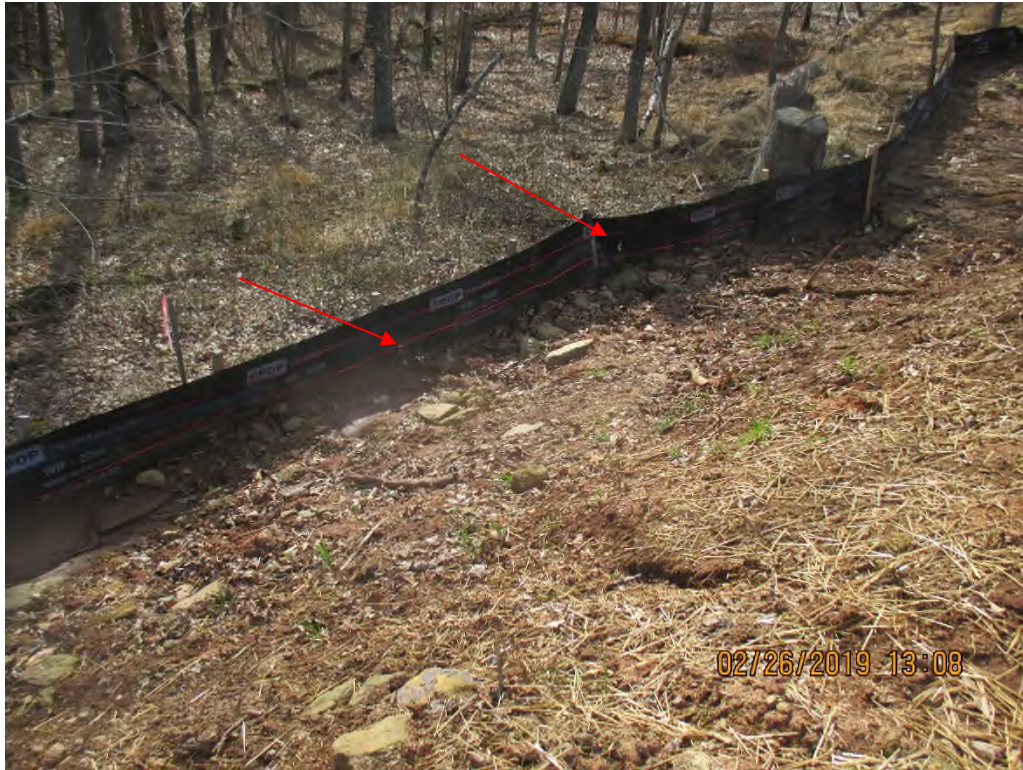
Silt fence with multiple holes near station 6766+60
