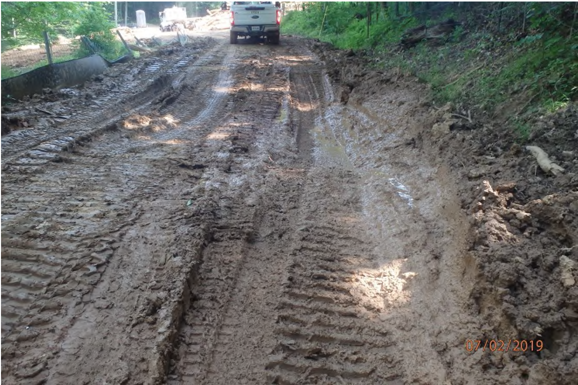
ARDO015.12 - lack of installed upslope ditching and the associated cross drains as well as lack of a graveled surface as indicated in the approved SWPPP.
