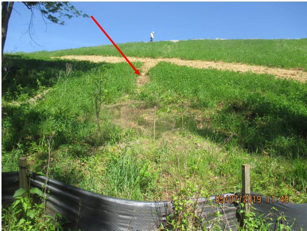
Southwest slope above LOD facing perimeter controls. Scouring present on slope above controls.
