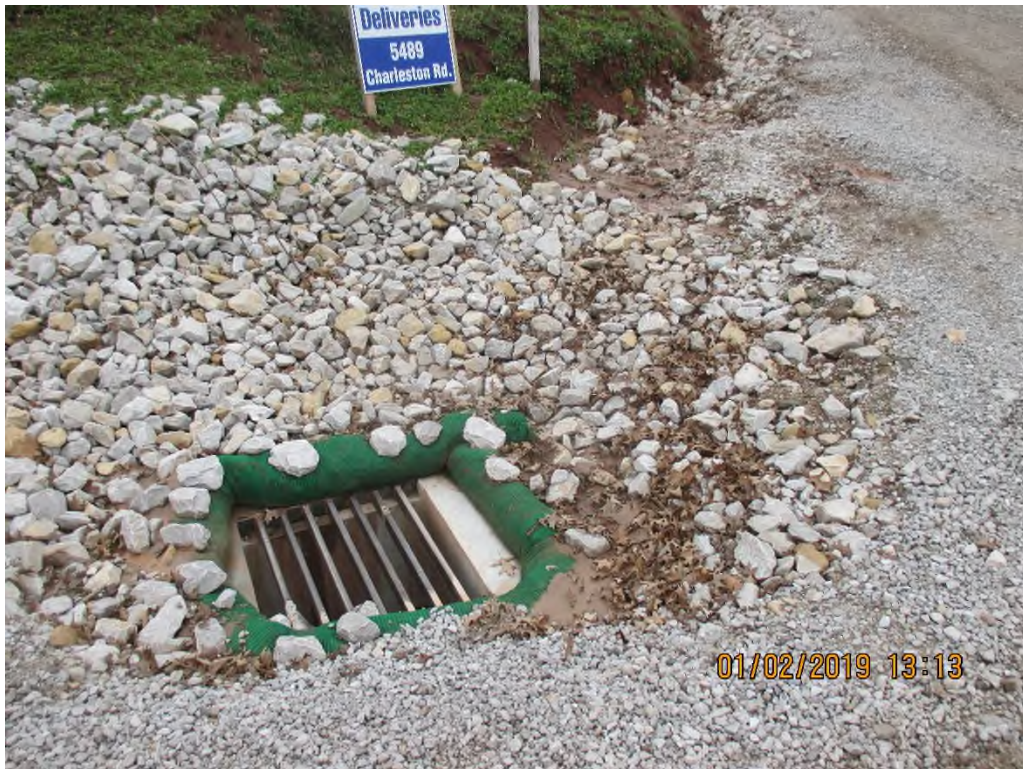
South side of access road rock lined ditch terminus.
