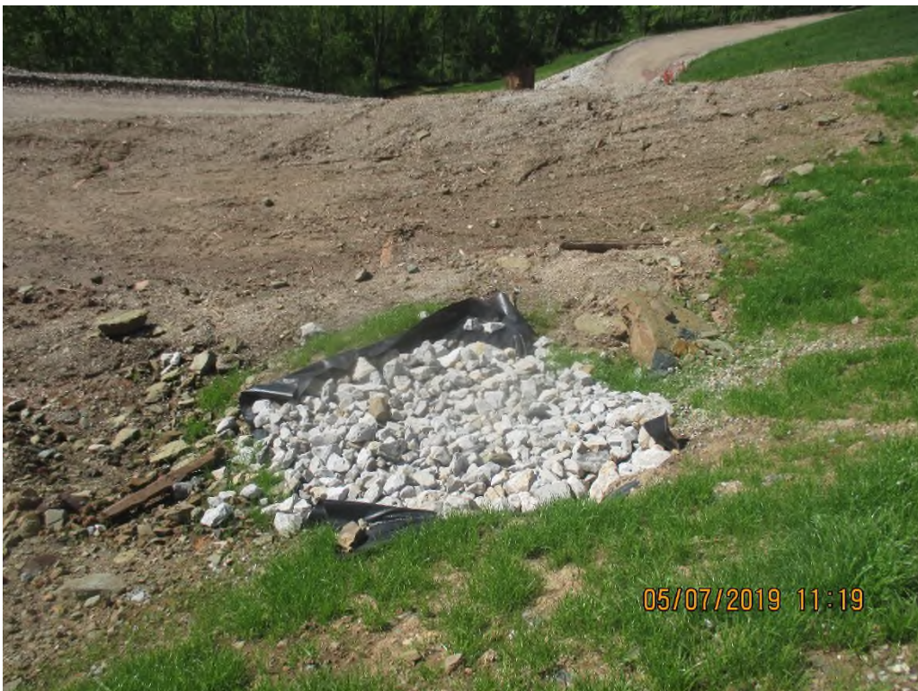
Diversion swale outlet terminating on rock armored pad. However, no controls to protect fill slope below this to the access road were in place.
