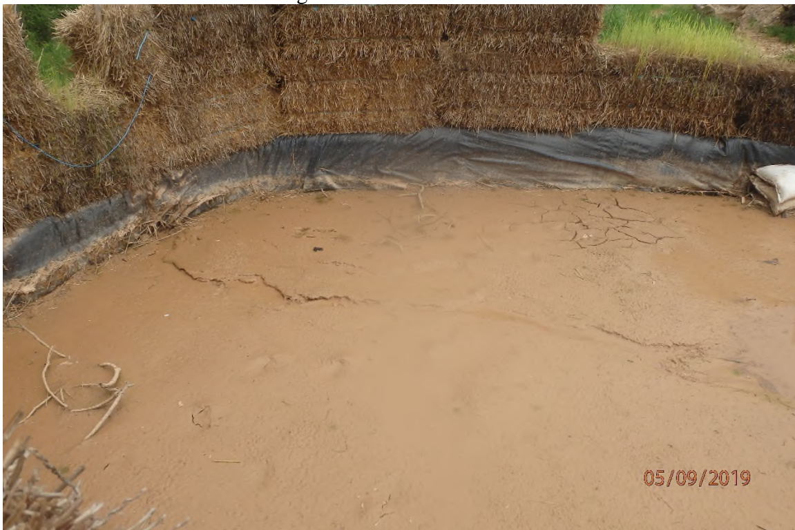
Makeshift treatment structure being utilized to treat stormwater from the sediment basin that is being discharged into an unstable diversion. Structure is inundated with sediment and in need of maintenance.
