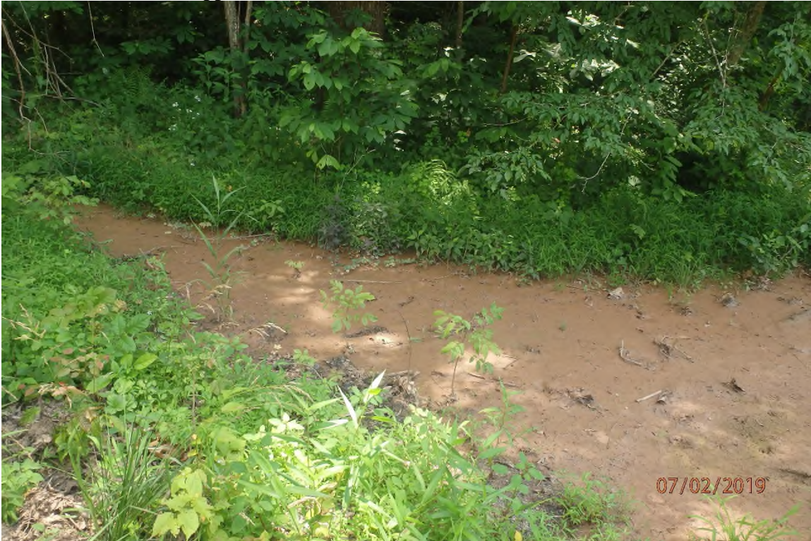
Offsite sediment deposits downslope of the previously pictured water bar that lacks the water bar terminus BMP indicated in the approved SWPPP in the UNT Left Fork of Arnolds Creek watershed.
