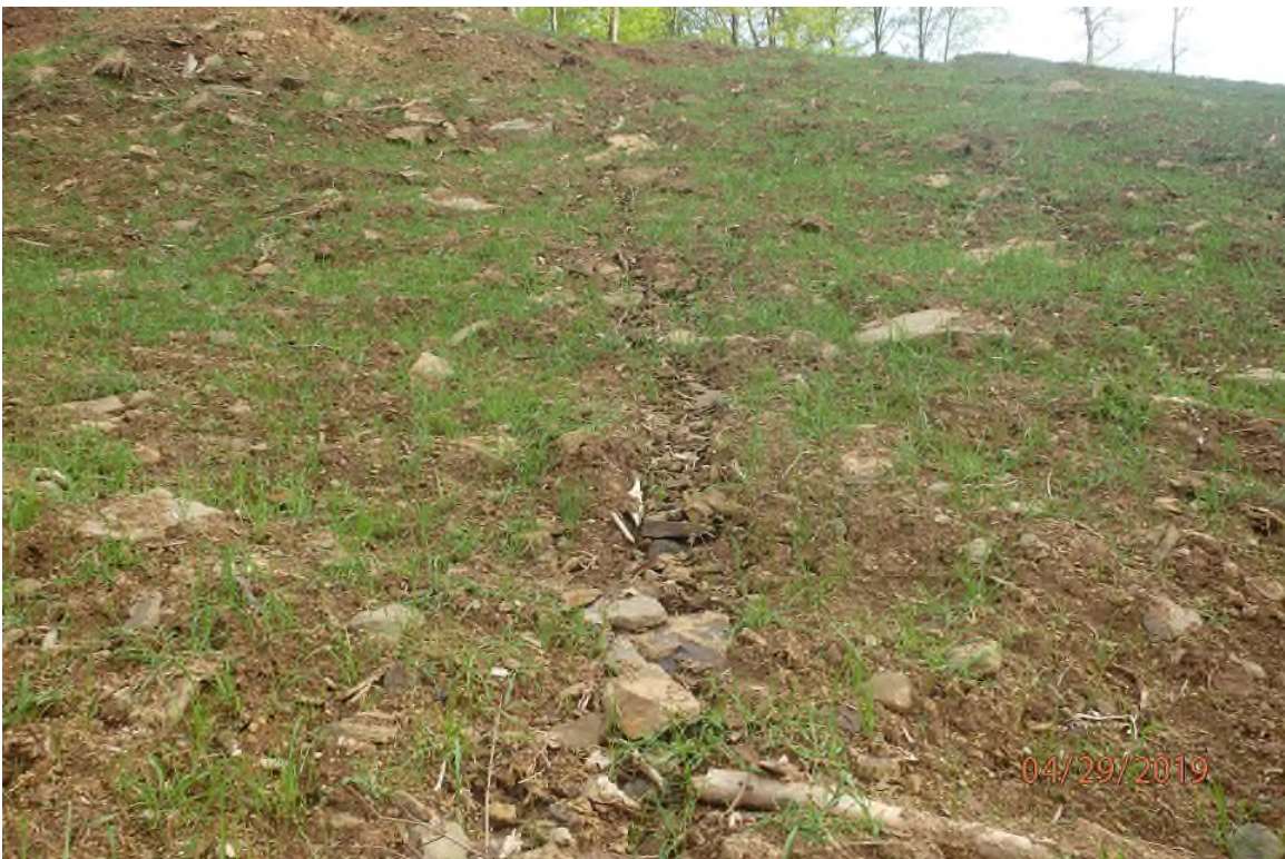
Erosion gully downslope of the above pictured water bar adjacent to 2226+50.
