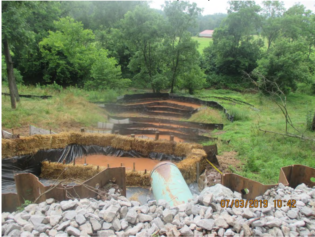
Culvert outlet downslope of Sulu Road leading to multiple controls upslope of 18-Mile creek.
