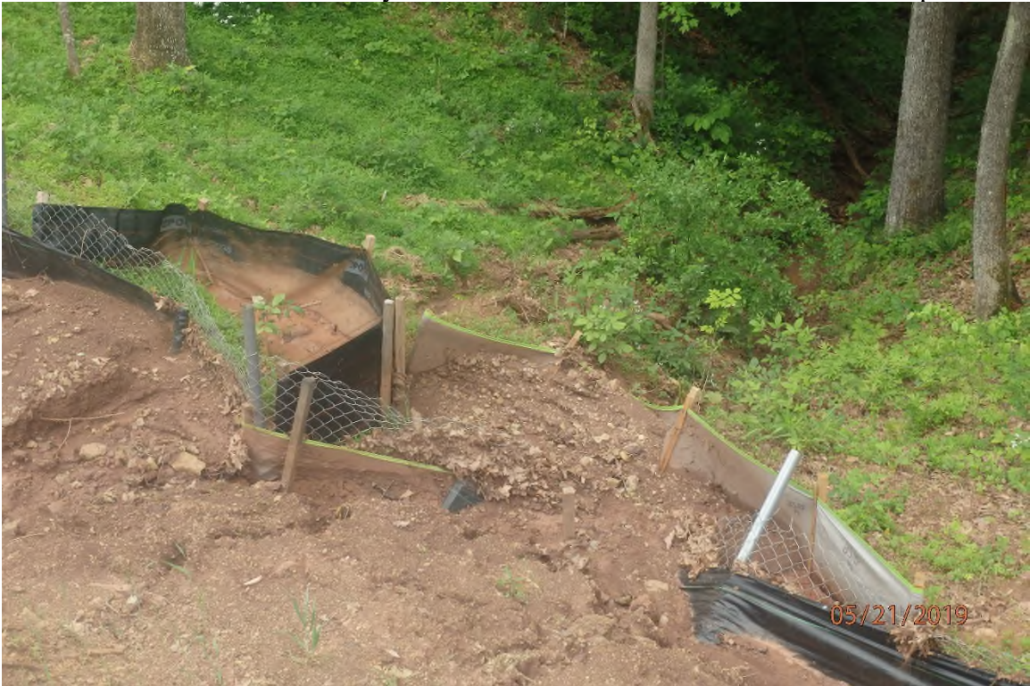
Unmaintained BMP in the Jims Run watershed.
