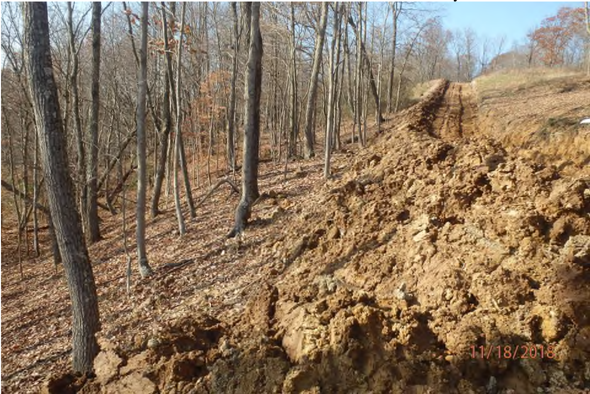
ARDO008.4 showing the lack of a graveled surface and the lack of perimeter controls, even though the road shows evidence of recent construction activity.
