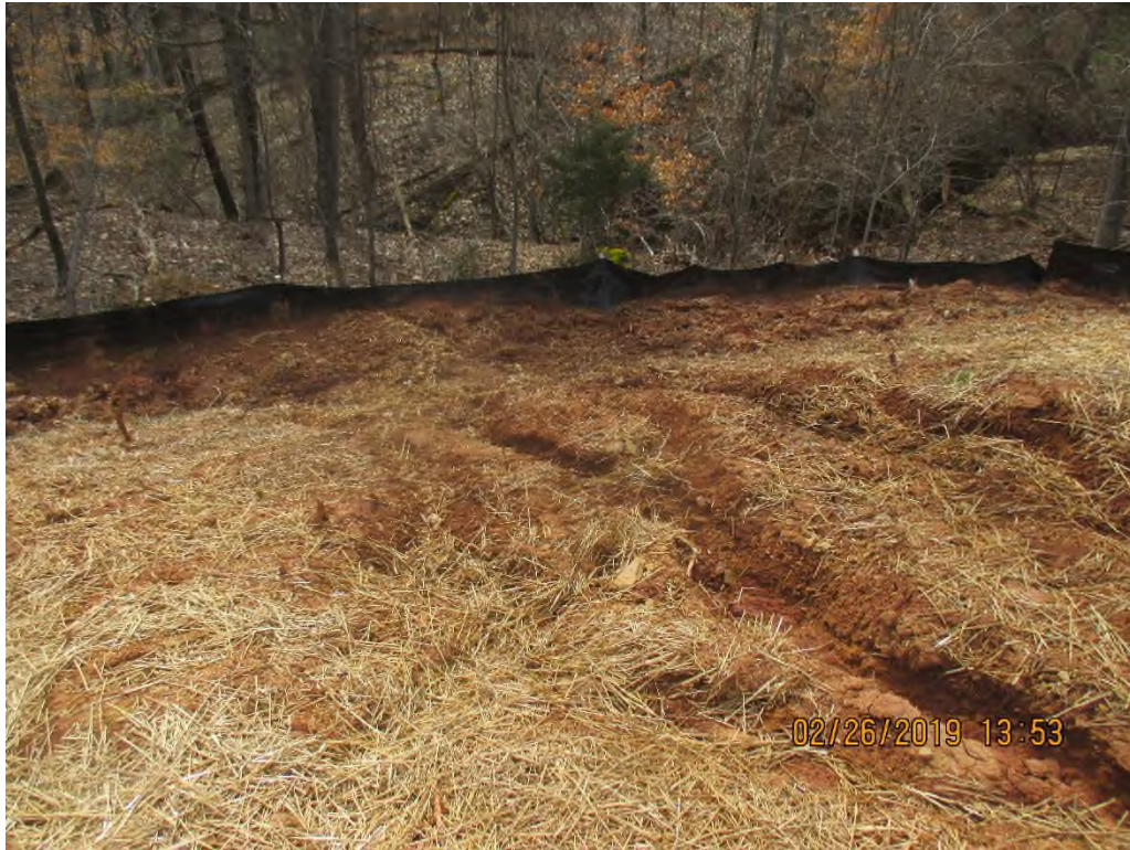
Run-on from adjacent field flowing across ROW, creating rill/gully erosion on slope near station #6742+60 and sediment being deposited against perimeter control.
