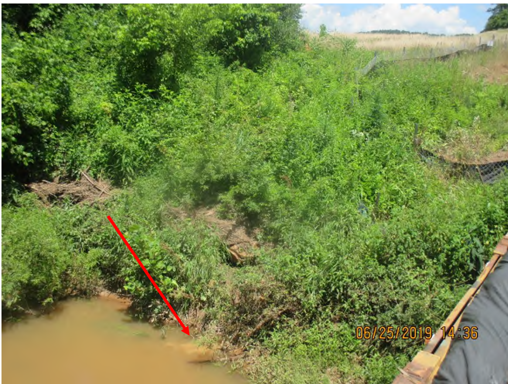
Stream SROC 029 crossing facing North near station No. 5638+47. Arrow depicts distinct sediment plume observed on day of inspection.
