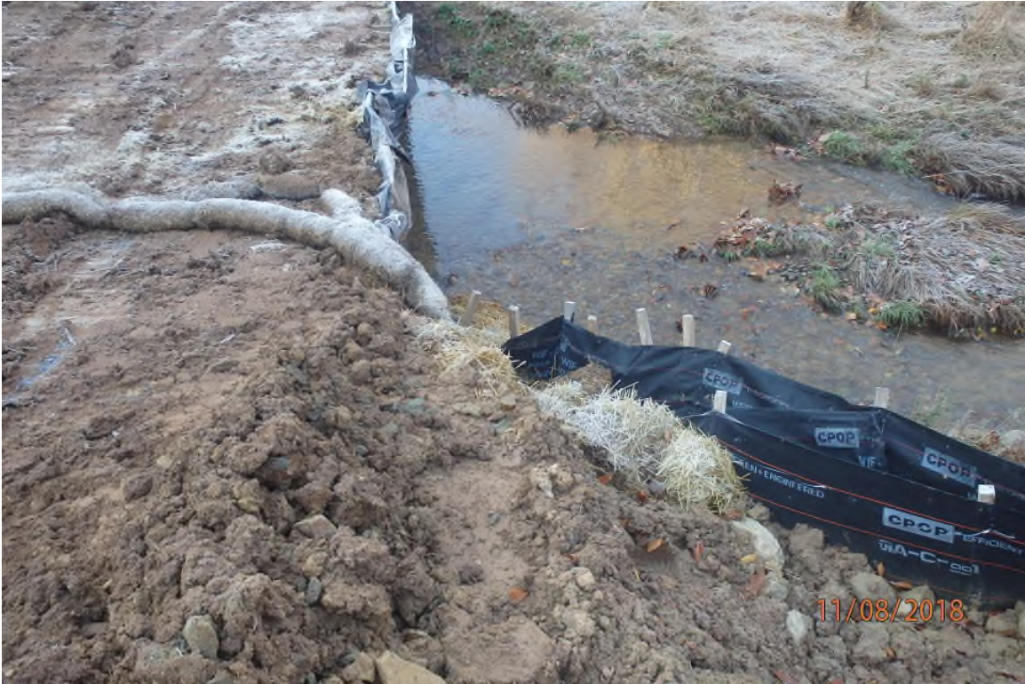
Unmaintained equipment bridge BMP in the Bluestone Creek watershed (SDOG537).
