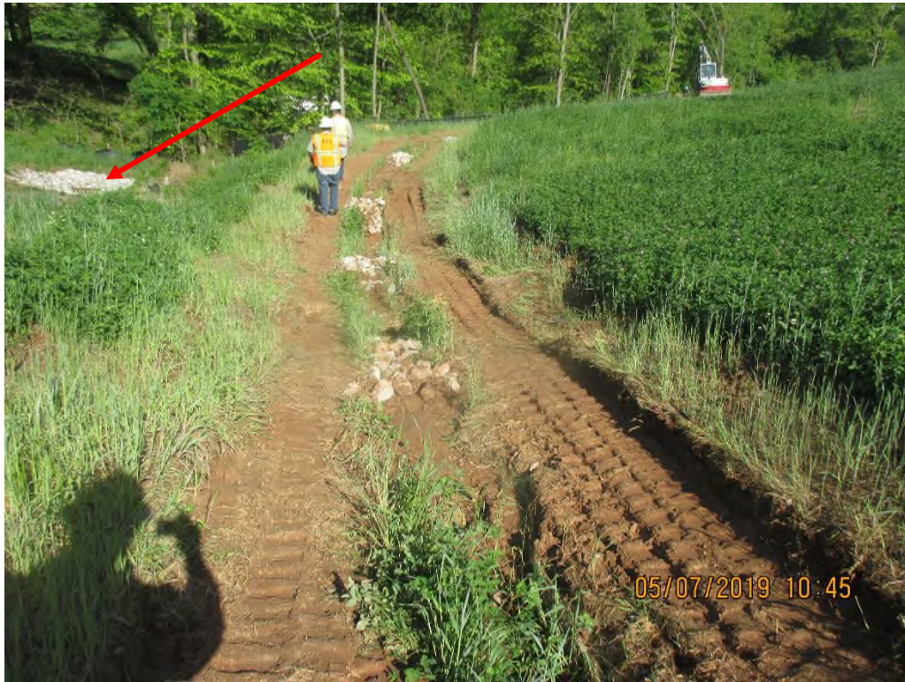
Access road to bottom of West side slope. Rock checks present in middle of road. Drop inlet in place downslope of this road. Sediment was being conveyed into this inlet and was present in the ephemeral stream within the LOD. Arrow depicts drop inlet below this road.
