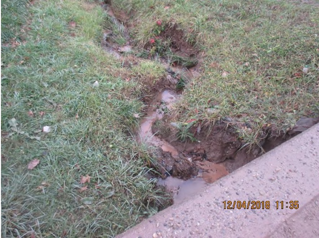
West Side of Route 21 at culvert crossing, flowing towards Grasslick Run.
