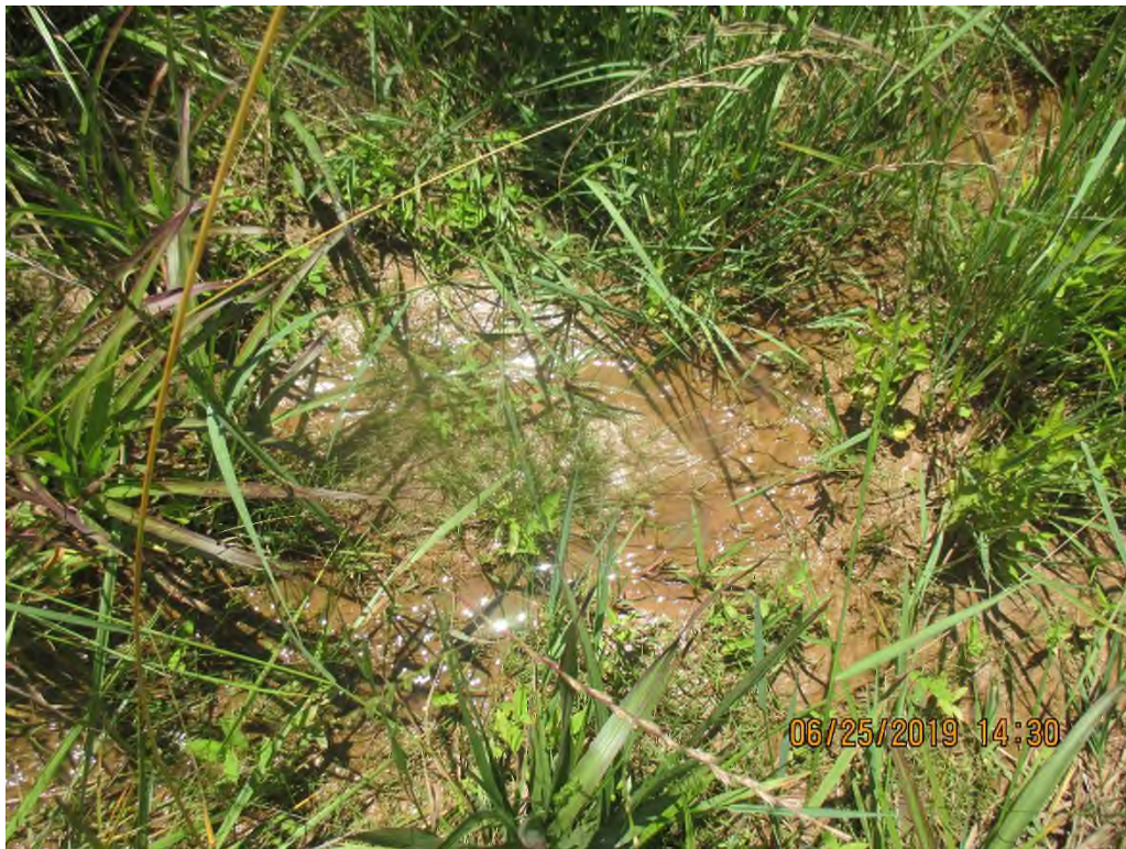
Sediment laden water and deposits being transported towards impacted pond at station No. 5638+46.
