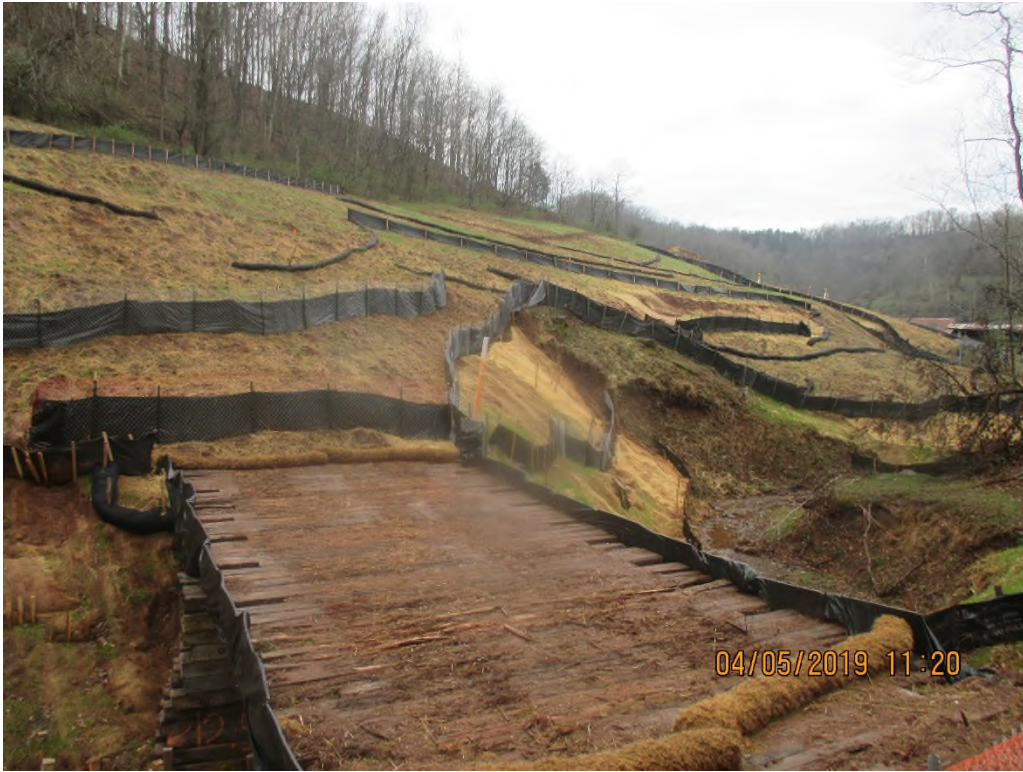
Stream SJAG-316 crossing where multiple slips have been reported.
