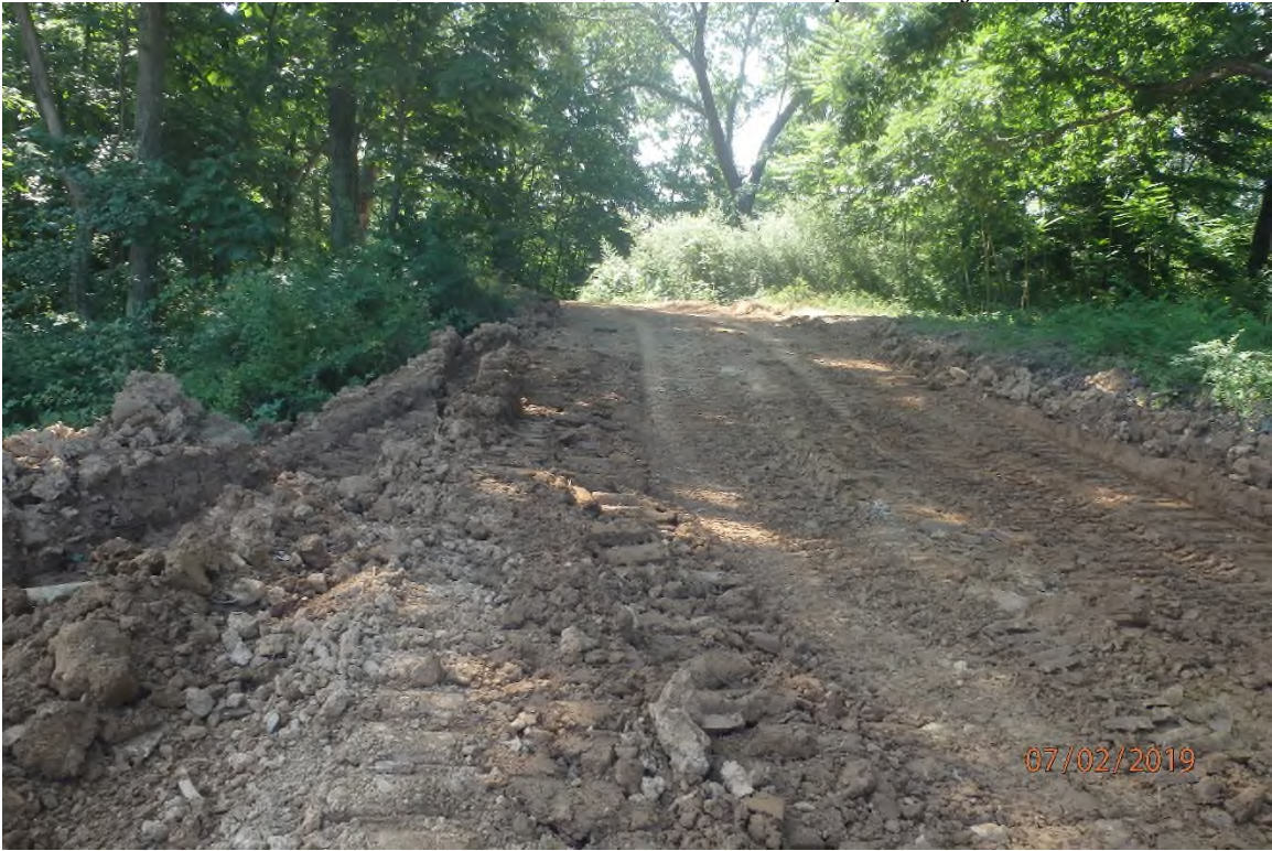
ARDO015.12 - lack of installed BMPs and lack of a graveled surface as indicated in the approved SWPPP.
