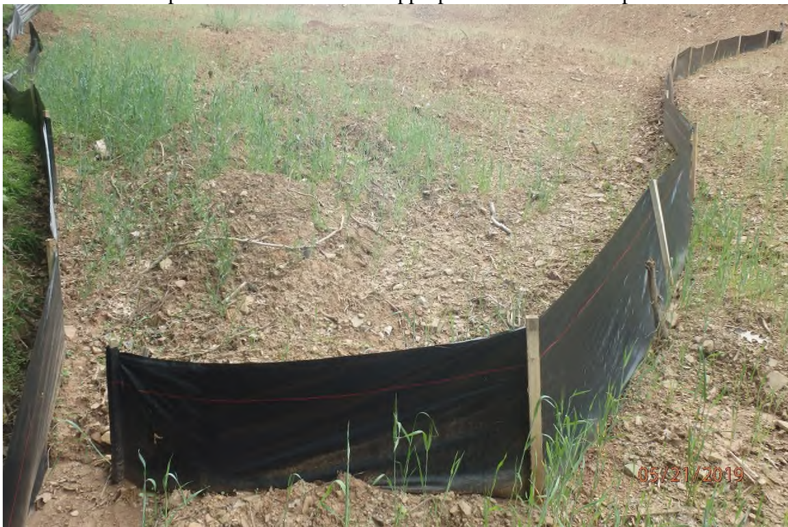
Improperly installed water bar in the Taylor Drain watershed. Water bar outlet discharges inside of the installed perimeter control and an appropriate outlet was not provided.
