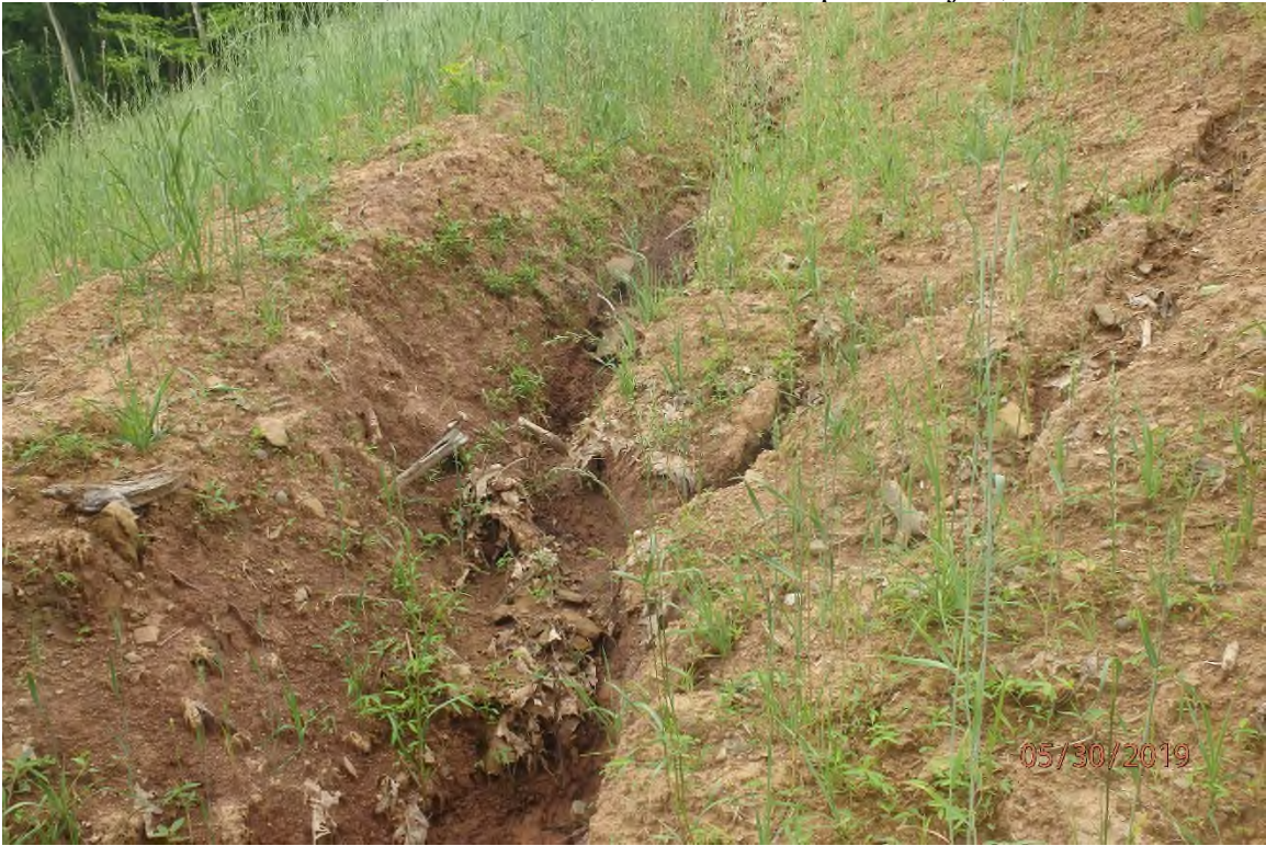
Water bar erosion in the Wolfepen Run watershed as a result of the BMP being constructed at a steep angle.
