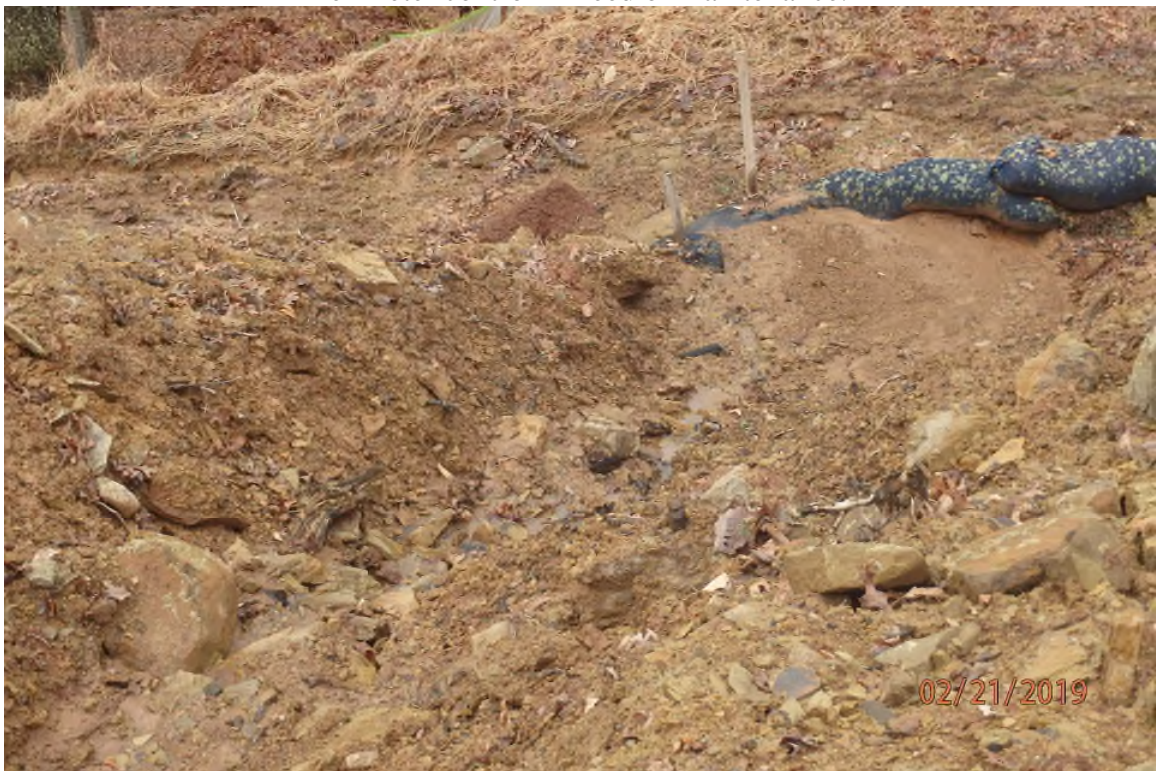
Water bar terminus BMP in need of maintenance.
