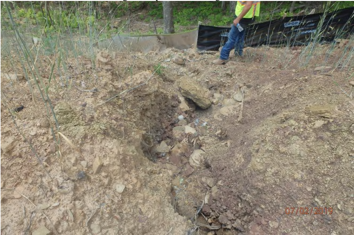
Water bar that does not extend past the installed perimeter controls in the UNT Left Fork of Arnolds Creek watershed.
