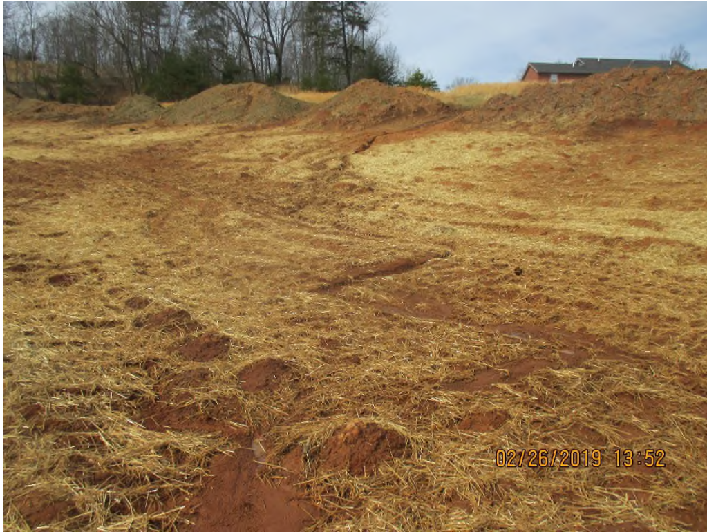
Run-on from adjacent field flowing across ROW and creating rill erosion near station#6742+60.
