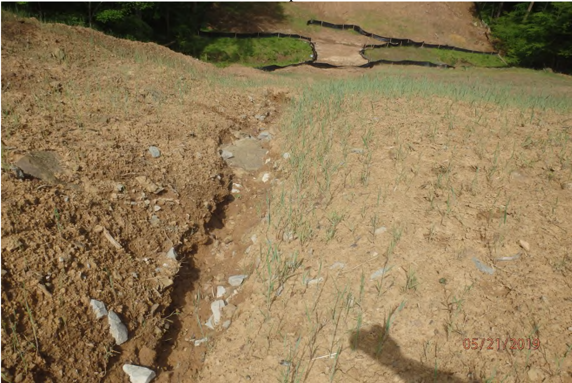
Associated fill slope erosion downslope of the above pictured area lacking water bars that are indicated in the approved SWPPP.
