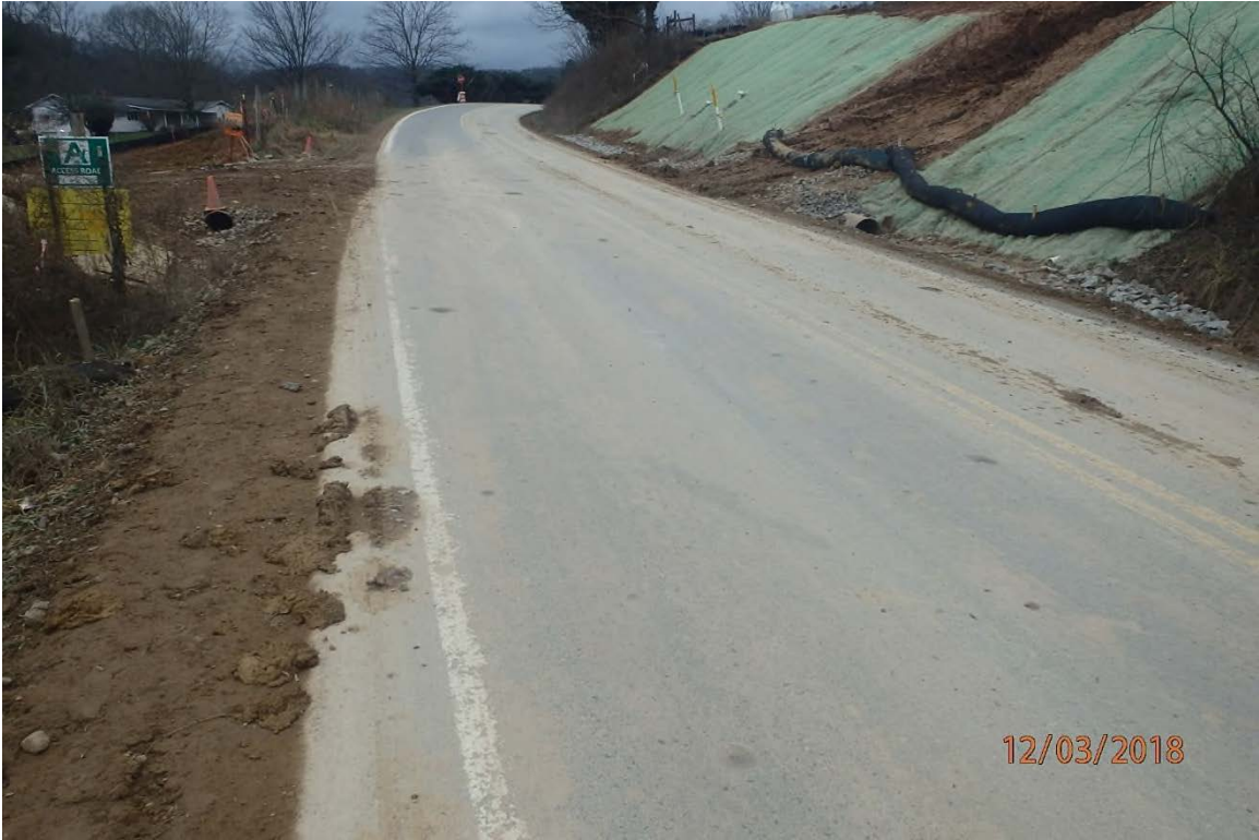
ARDO008/WV 18 crossing showing the lack of a stable construction entrance and the associated track-out onto the public roadway.
