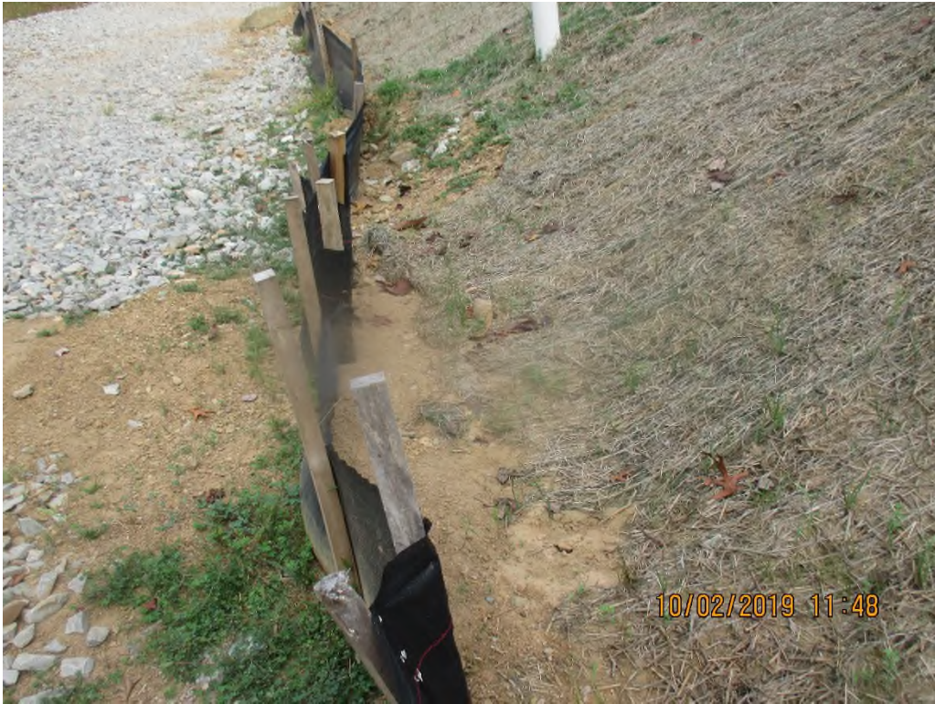
Perimeter controls along CR 22/1 with sediment deposits behind and past controls. Hole present in silt fence.
