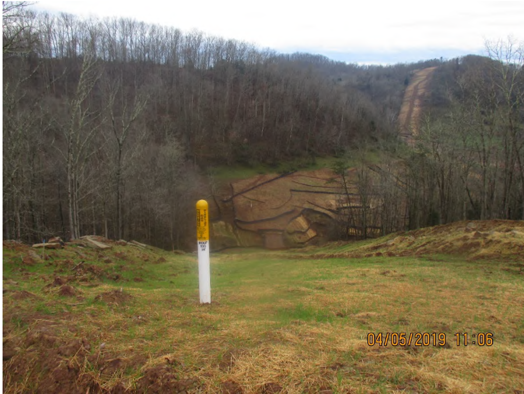
Facing towards SJAG 316 and the Shamblin Run Road crossing where multiple slips have occurred on ROW.
