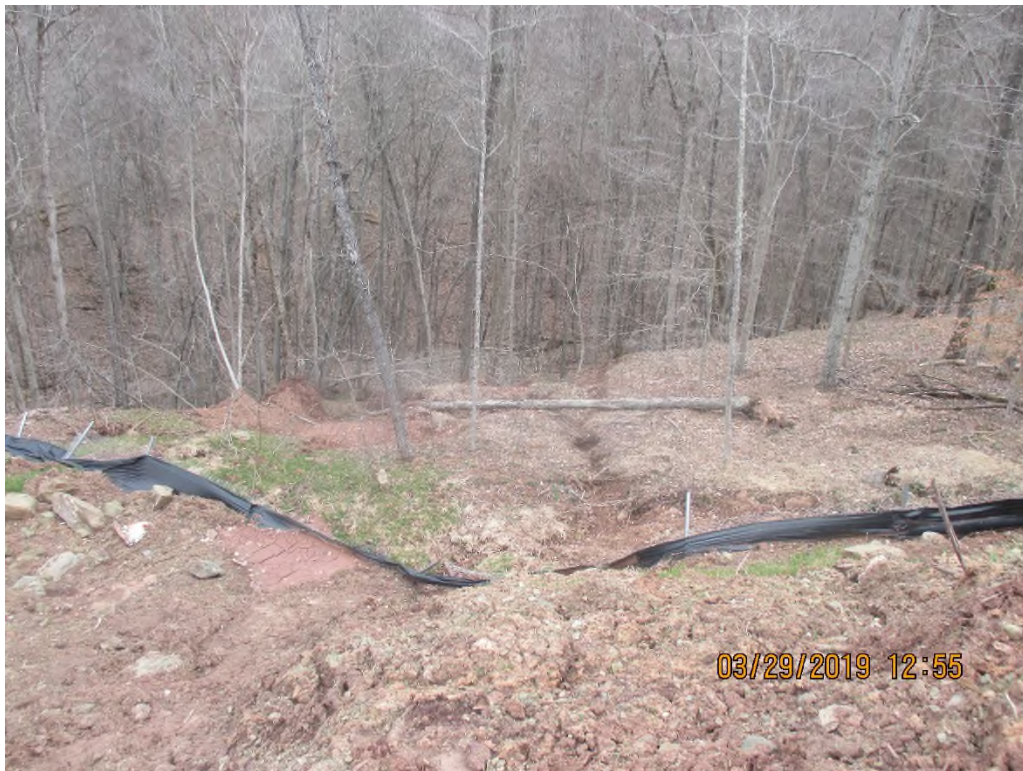
Slip at station #5171+34 facing South. Sediment deposited past LOD
