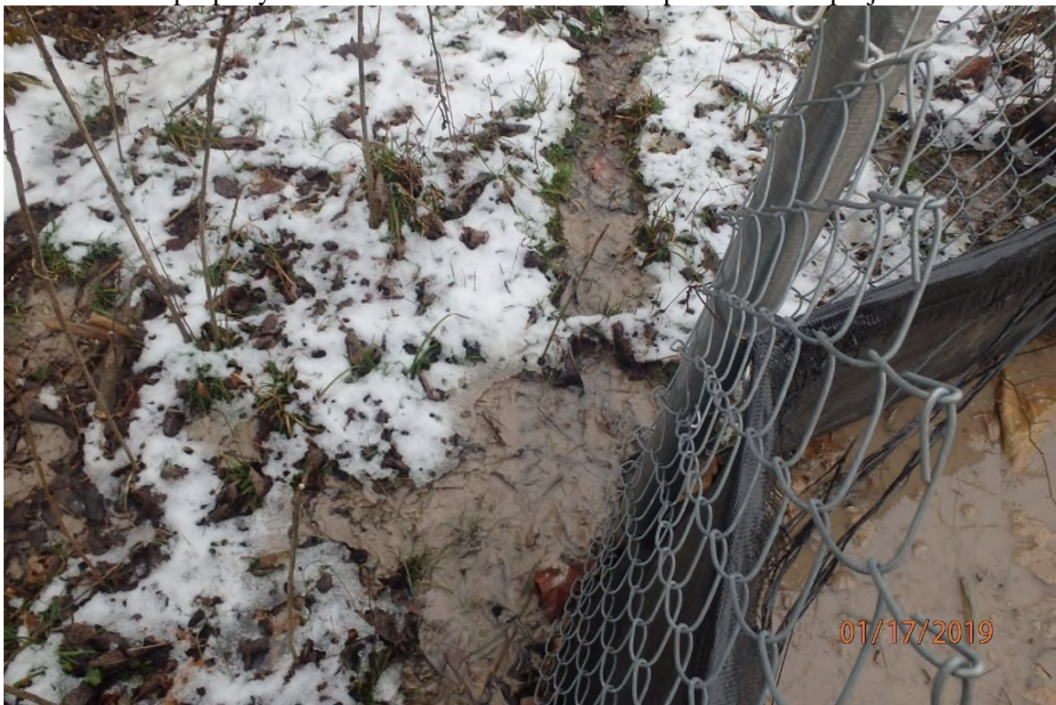
Small amount of offsite sediment deposits as a result of the above pictured deficiency.
