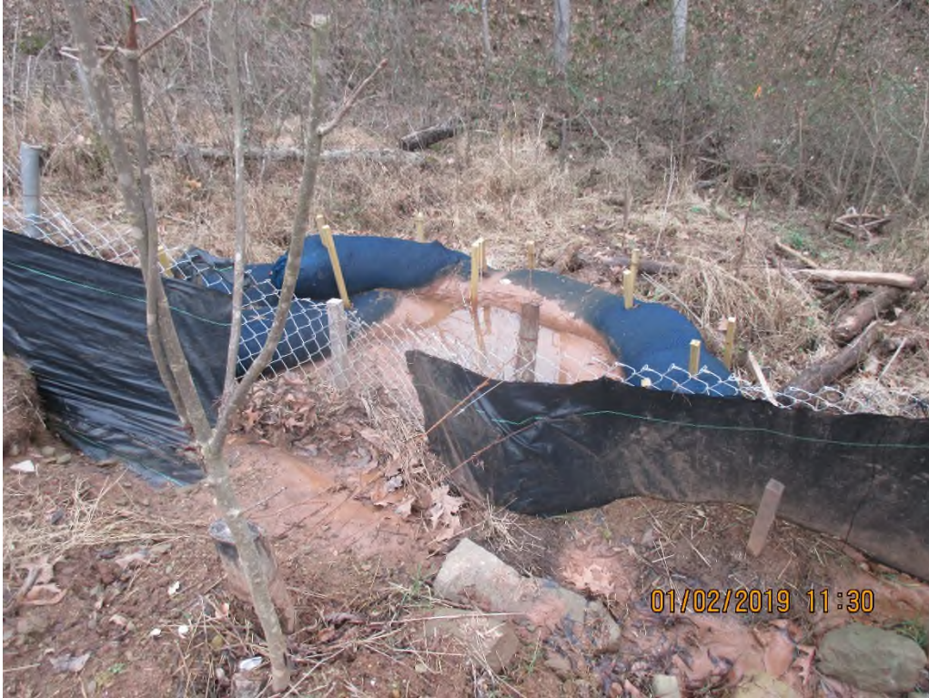
Southern slope armored channel terminus with evidence of concentrated flows and BMP being overwhelmed during rain events.
