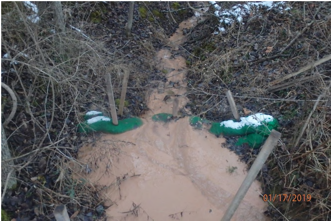
Installed BMPs showing the need for maintenance.
