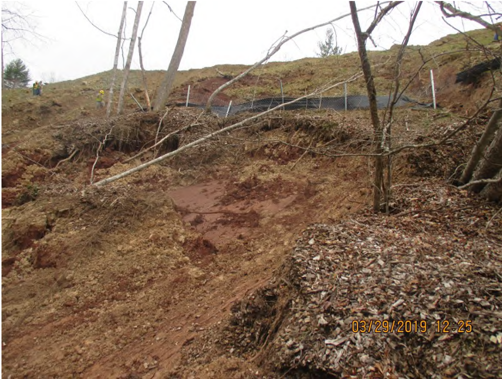
Facing upslope at section of ROW that slipped into stream SWIF-057
