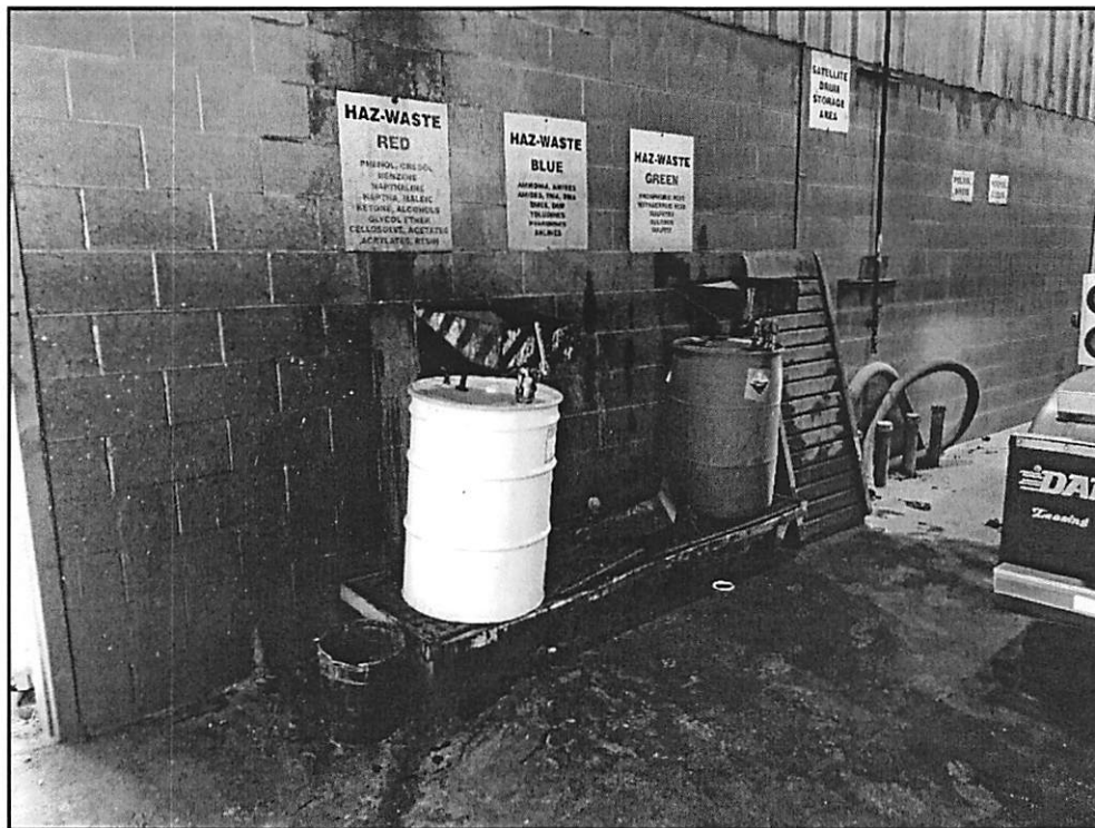
10/3/2019 - Satellite accumulation area in Bay 1. Spillage on the floor. Secondary containment pallet full of spillage and rinsate.
