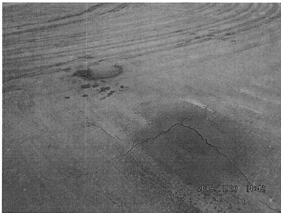
11.20.2019 – Evidence of a spill event.
