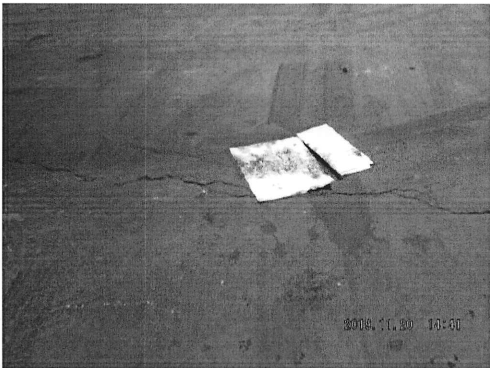
11.20.2019 – Evidence of spill without adequate removal of materials.
