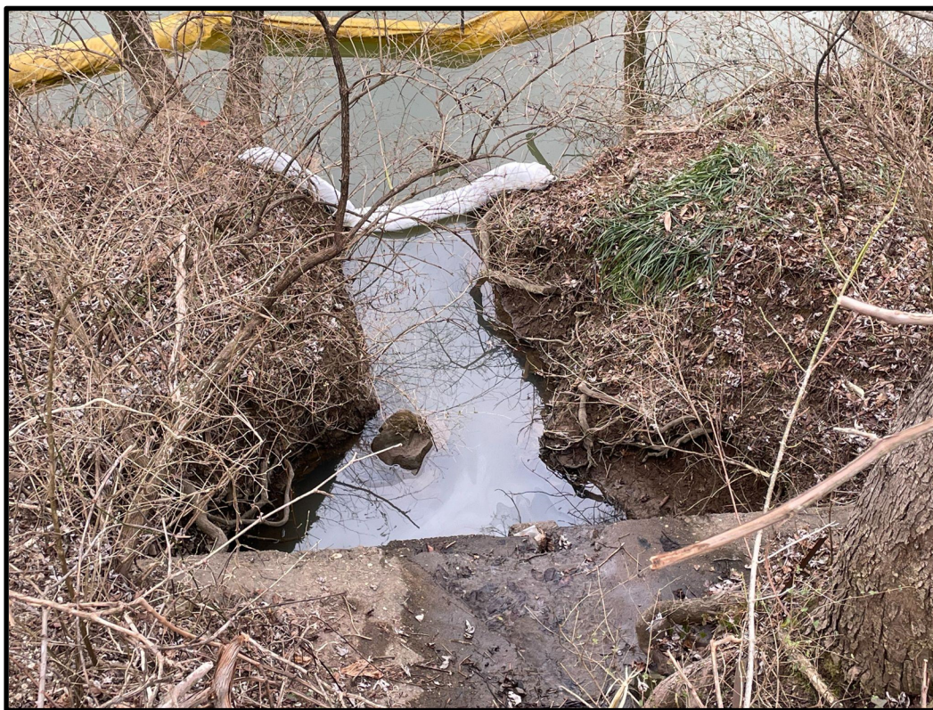
January 30, 2025 - Sheen of gasoline on the water discharging from stormwater outlet into Twelvepole Creek.
