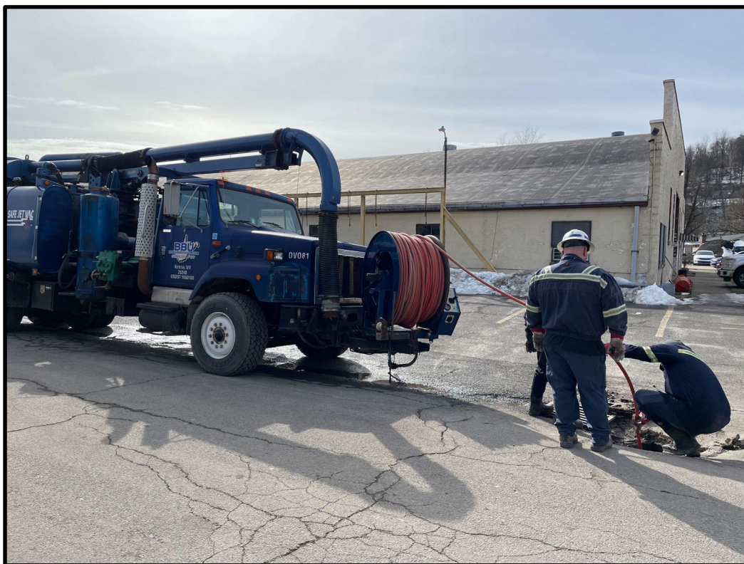
January 30, 2025 - BBU Services of WV flushing out storm drain beside the WVDOH garage.
