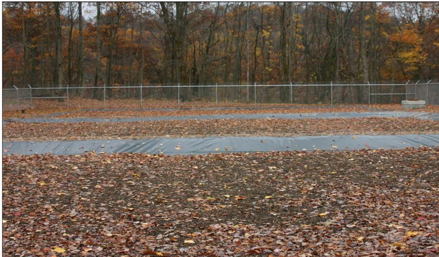
The wastewater treatment system's three wetland cells are located on top of a mountain adjacent to the community of Ashland. From here, water will flow down to a drainfield.
