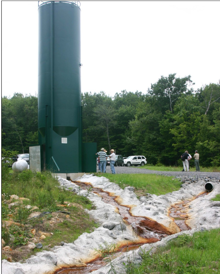
The Little Creek doser near Mount Storm in Grant County is one of three dosers that will treat Abram Creek's acid-laden waters. The doser was activated by state and local officials during an August ceremony.
