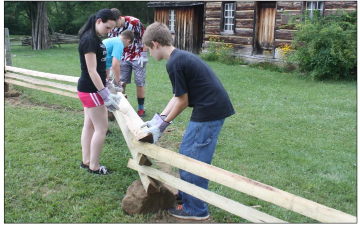
One of the projects at Junior Conservation Camp was to repair the split rail fence at Cedar Lakes' historic Heritage House.
