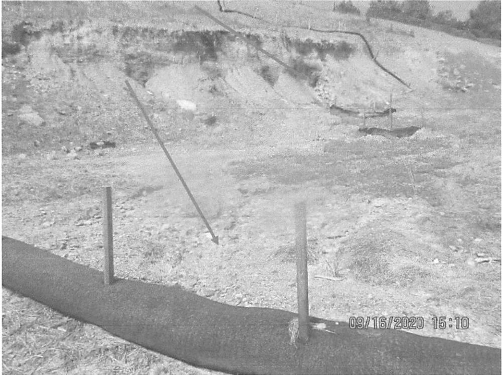
Standing at Access Road 159.01 facing upslope at Station No. 6450+76. Erosion present on cut slope and above controls (red arrow).
