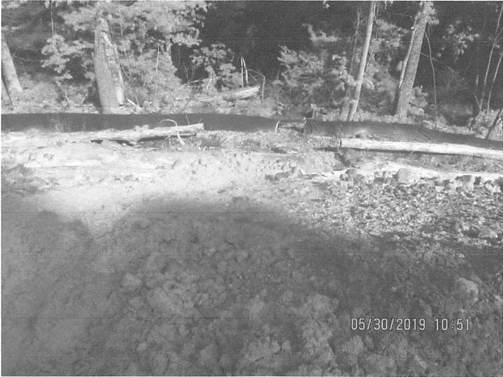
Waterbar outlet terminating onto slope at station 6485+10. Erosion present on slope above perimeter controls.
