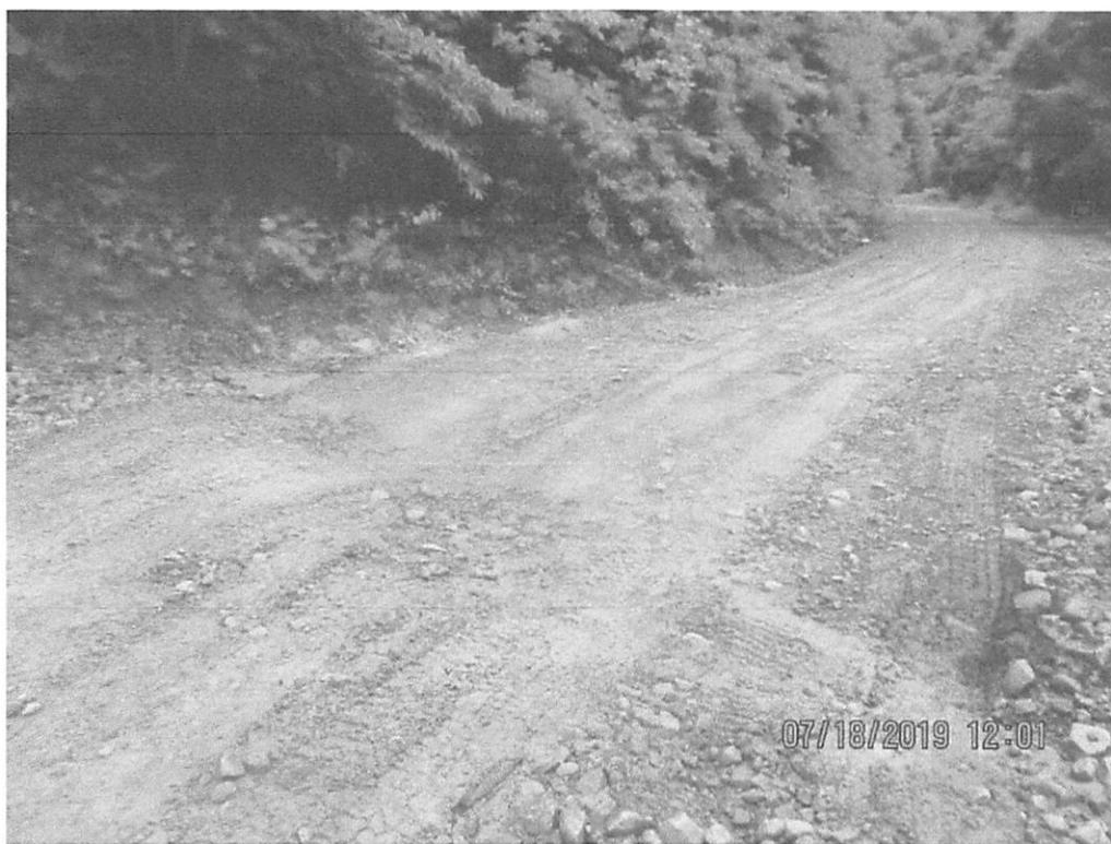
Waterbar installed on Access Road MVP-WB-119. Ditch line had rock checks present. Sediment deposits overwhelmed perimeter controls downslope of waterbar.
