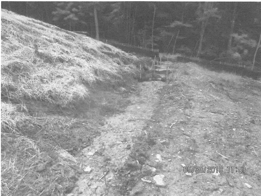
Waterbar with CFS checks installed and scouring topsoil pile below Deepwell road crossing at Station 6508+30.
