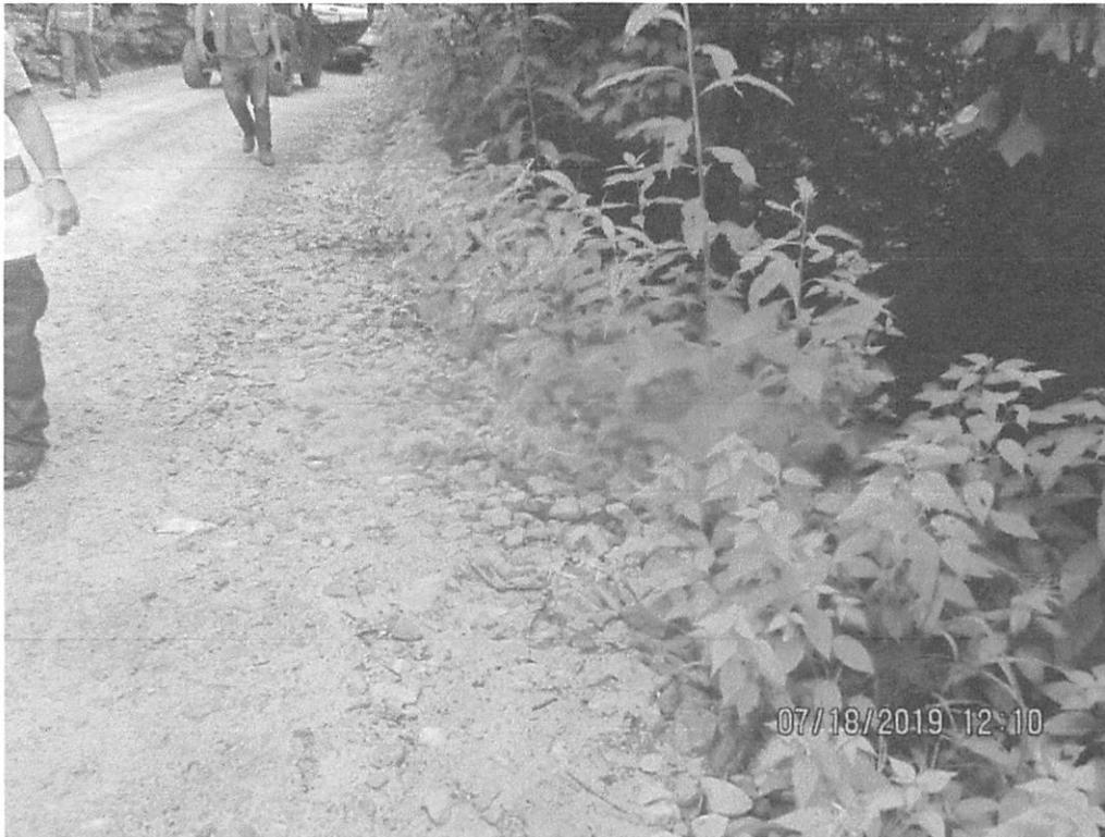
Section of MVP-WB-119 with no perimeter controls installed. Sediment deposits were observed past the LOD.
