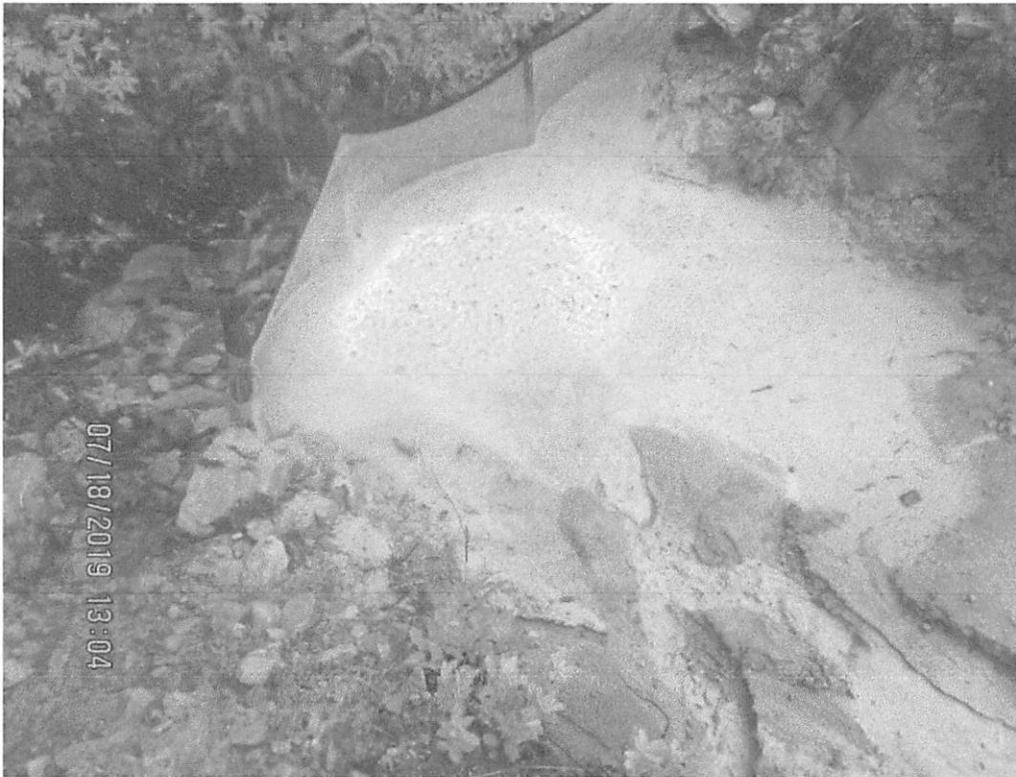
Above station 4539+00 during rain event. Sump full of sediment and in need of maintenance. Sediment-laden water undercutting silt fence and flowing past LOD.
