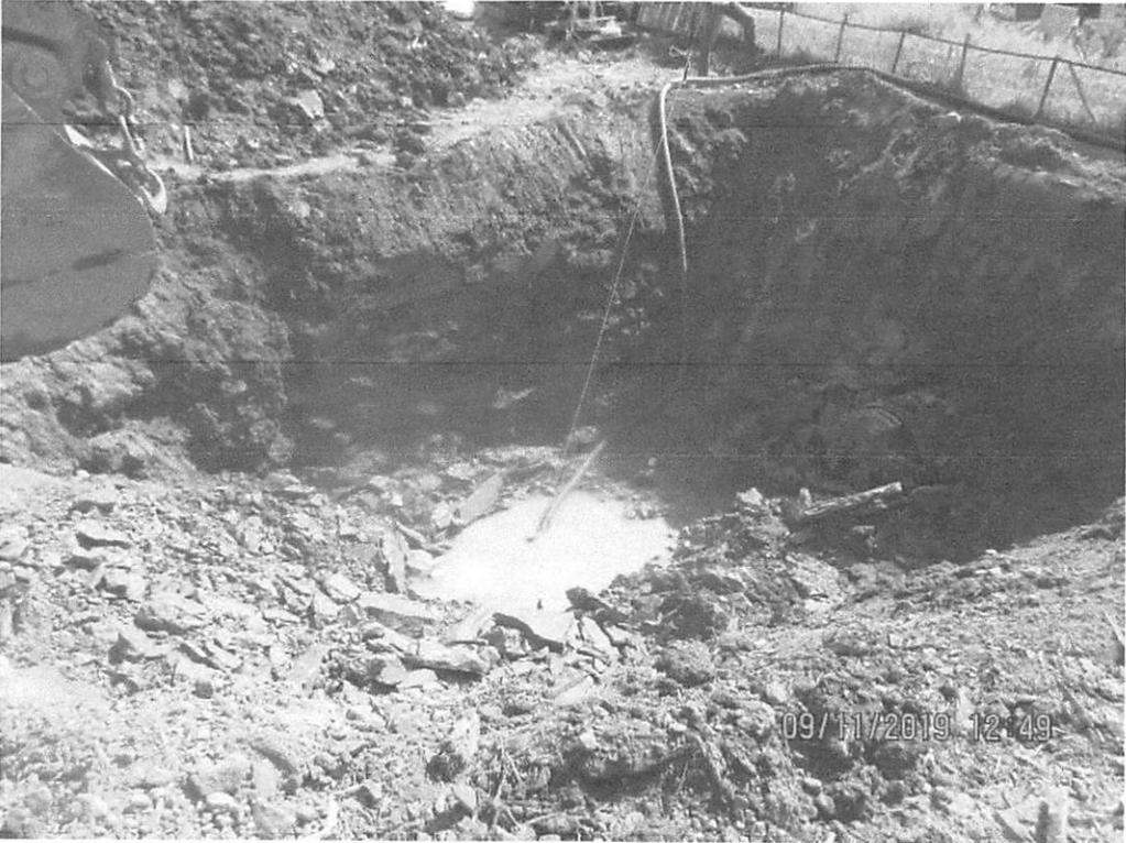
Open bore pit at the Goose Run (Stream S-B75) crossing at station 645+35.
