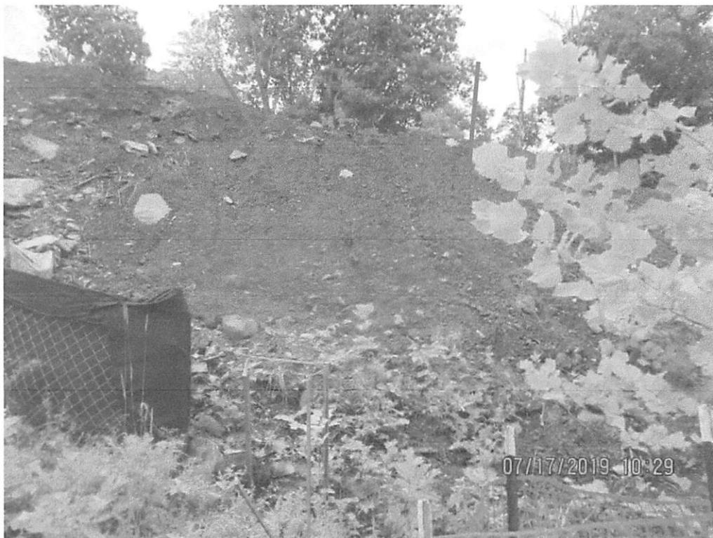
Fill slope erosion occurring at station 3159+46 facing edge of MVP LOD. Sediment deposits observed past the LOD.
