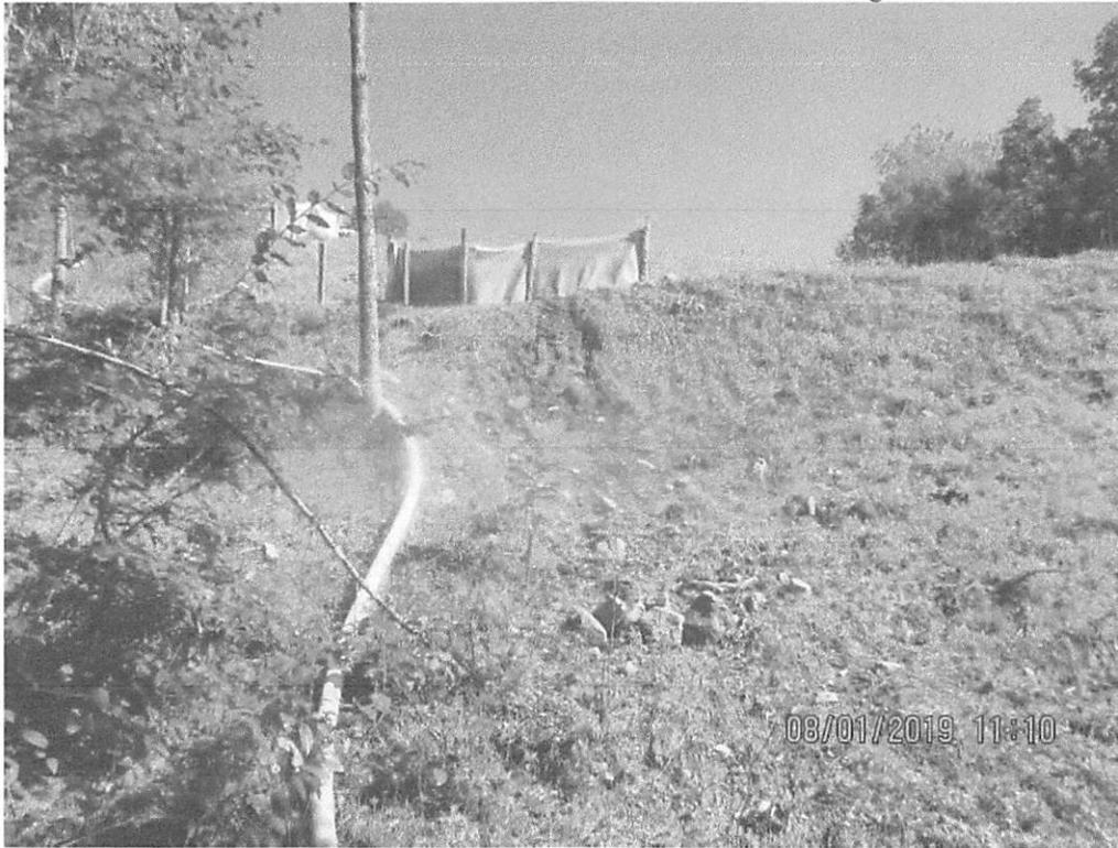
Waterbar that was overwhelmed with run-off causing undermining of controls leading to erosion downslope of controls South of BR-099 near station 3897+75.
