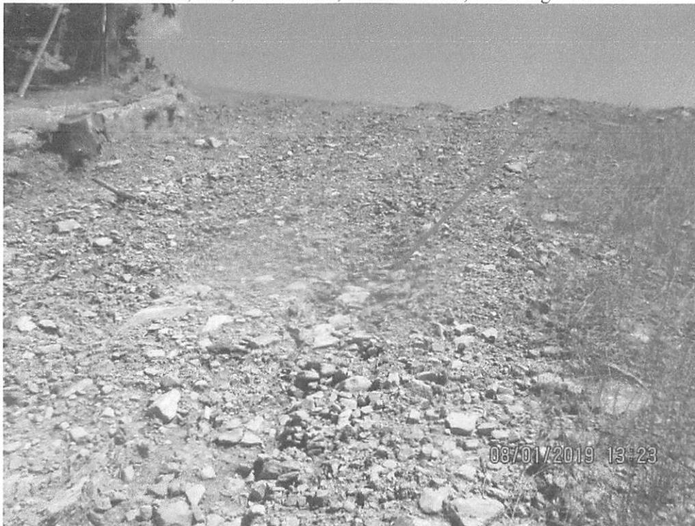
Travel lane on slope near station 3831+00. Erosion present in travel lane, resulting in waterbar being overwhelmed with sediment and not functioning as designed.
