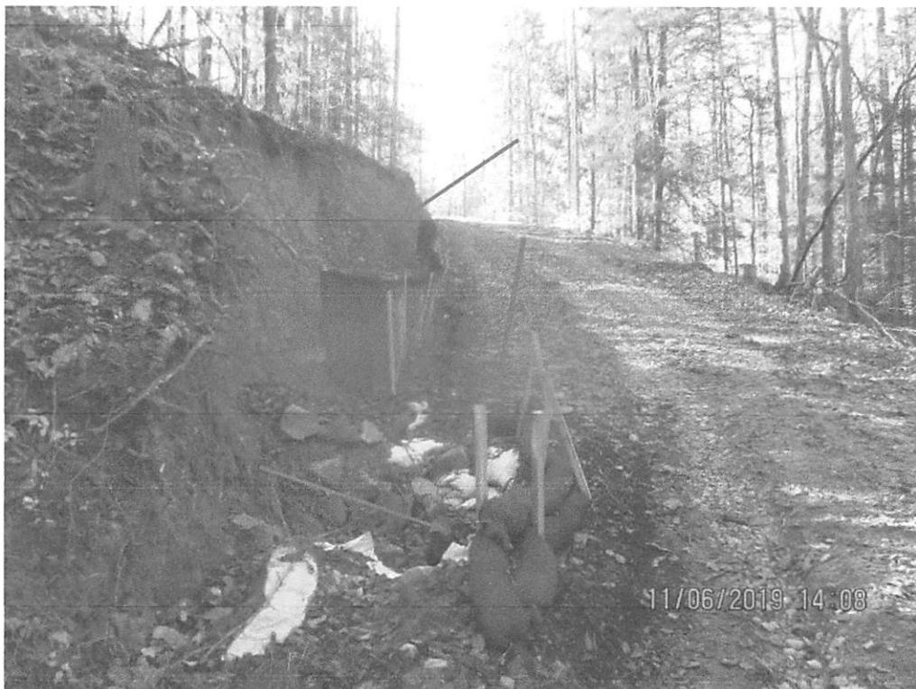
Access Road 114 above Stream S-S2. Red Arrow depicts slip. Orange arrows depict slope drain and small sump with culvert inlet conveying under AR-114.
