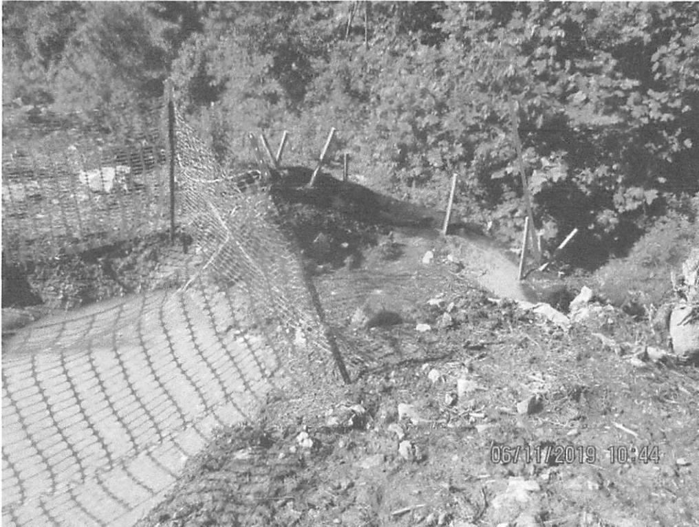
Above Station 7604+41. Controls below waterbar and sump had sediment due to erosion. Perimeter controls being overwhelmed with sediment.
