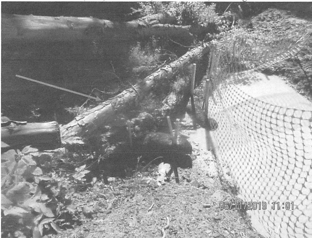
Above Lower Krosier Road crossing. Sediment and SLW overwhelming sump and perimeter controls near station 7604+41. Sediment deposits and SLW past controls and LOD.
