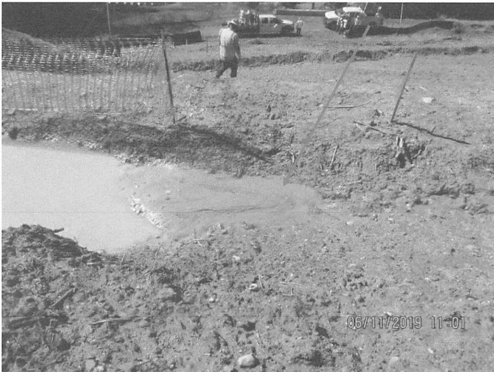
Above Lower Krosier Road crossing. Erosion present in waterbar causing sediment to be deposited in sump. Sump in need of maintenance.
