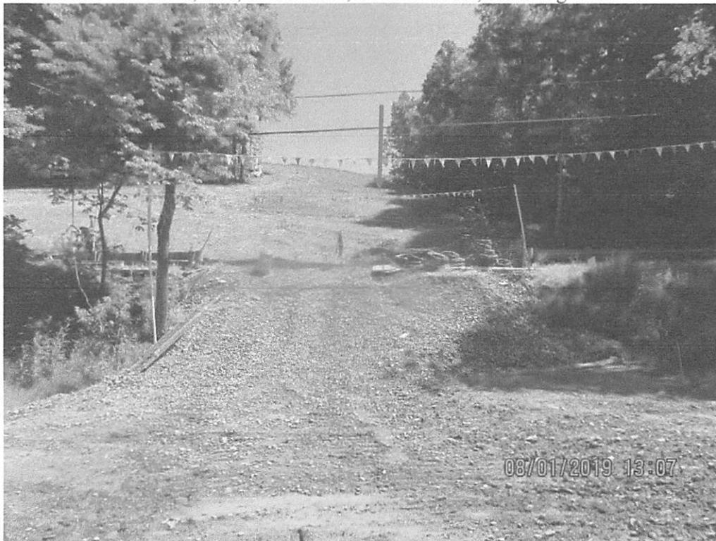
Above stream S-J70 and below US 19/Hwy 4 crossing near station 3829+00. Arrow depicts slope with lack of temporary stabilization.
