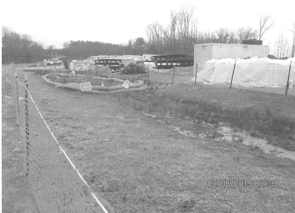
Facing toward wetland in drainage ditch. Sediment-laden water (SLW) present in ditch and wetland.
