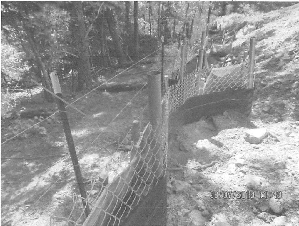
Perimeter controls below dewatering structure at station 8955+00. Arrow depicts where sediment deposits were observed.
