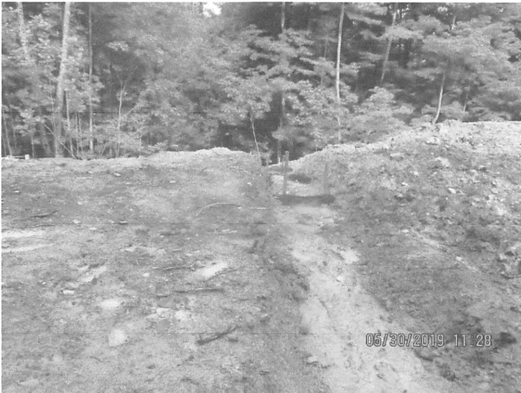
Seep running onto ROW via waterbar above Stream S-N13. Diversion not stabilized near station 6940+00.
