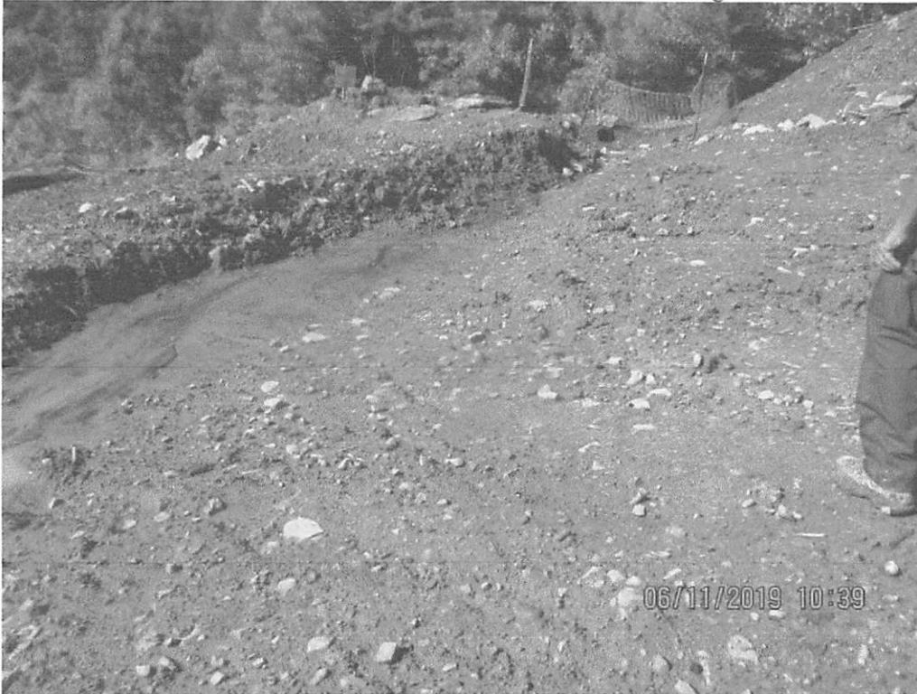
Below upper Krosier Road crossing near station 7576+01 facing toward waterbar outlet. Erosion present on slope due to seep running onto ROW causing sediment to be deposited in waterbar.
