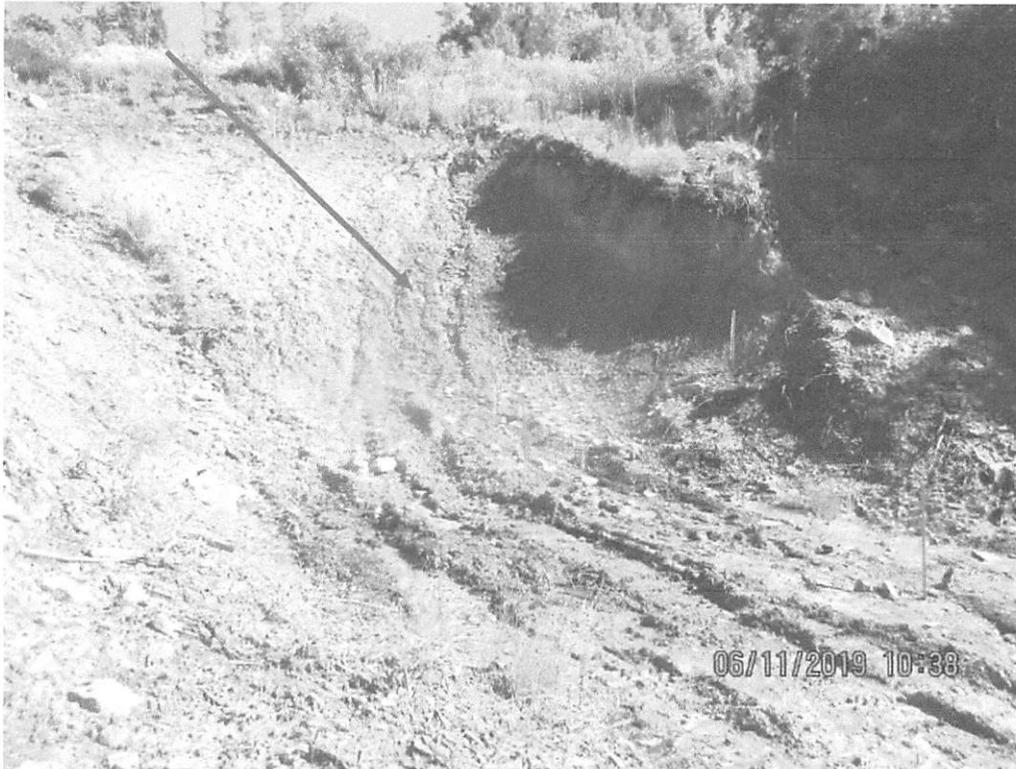
Below upper Krosier Road crossing near station 7576+01 facing North. Erosion present on slope due to seep running onto ROW.
