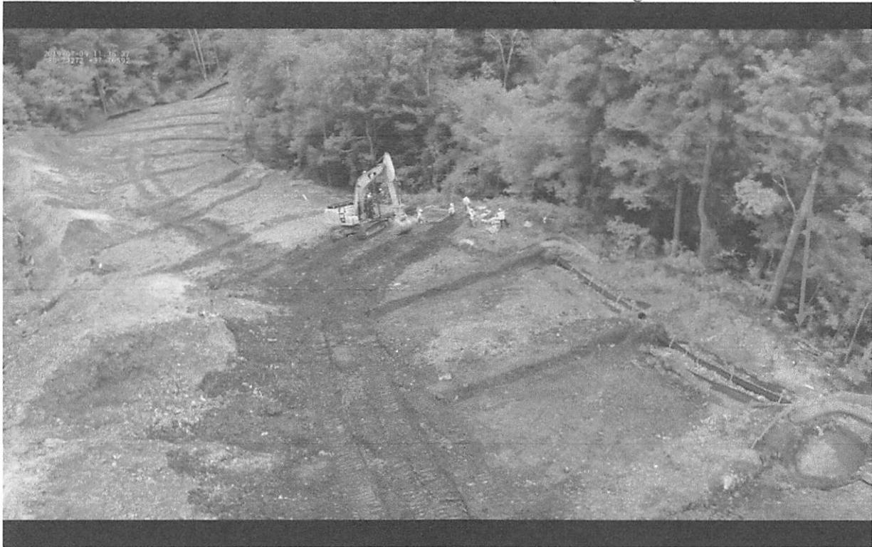
Overview of upper portion of slope near station 8634+00. Arrow depicts cut original cut that created a “wall” effect not allowing for proper waterbar outlets to be installed per the SWPPP.
