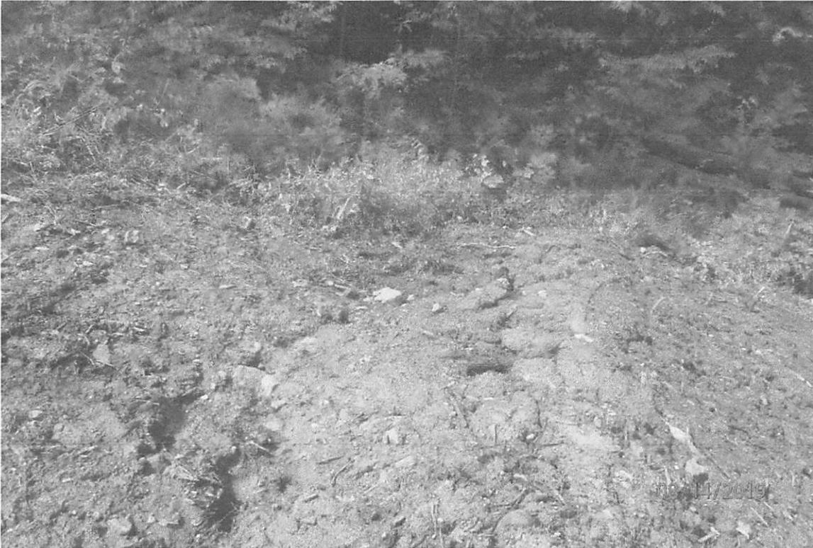
Water bar in inspected area 5 showing the lack of a water bar terminus BMP that is indicated in the approved SWPPP.
