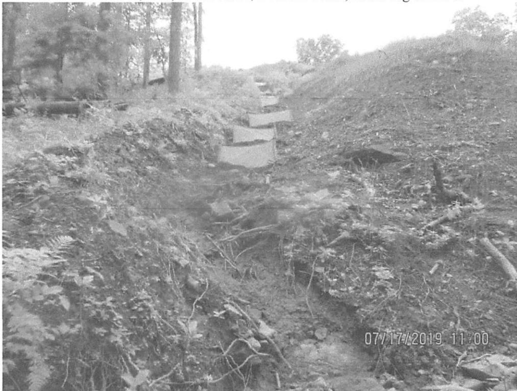
Diversion berm with erosion present above stream S-H154 at station 3147+11. Silt fence installed on steep slope where channelized/concentrated flow was occurring.
