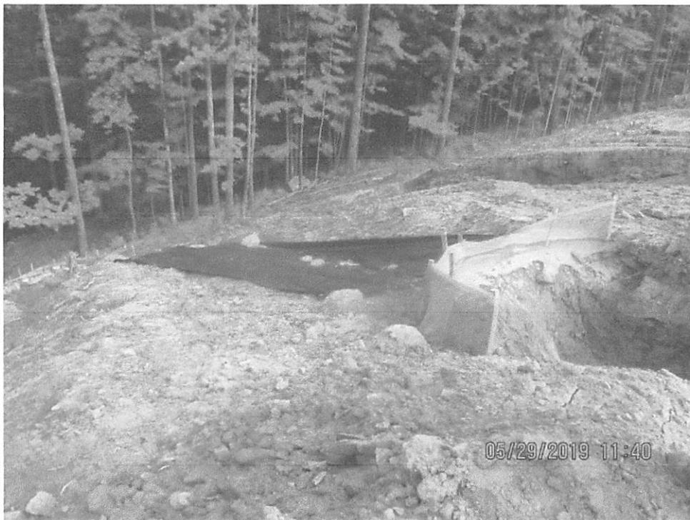
Waterbar outlet downslope of station 4027+00. Waterbar terminating on slope. Fabric installed below control on slope above perimeter outlet.
