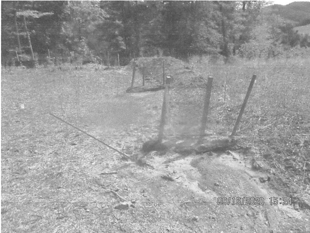
Near Station 6450+76 facing downslope toward erosion in waterbar (red arrow). Sediment was being deposited in waterbar, and runoff was flowing around unmaintained controls.
