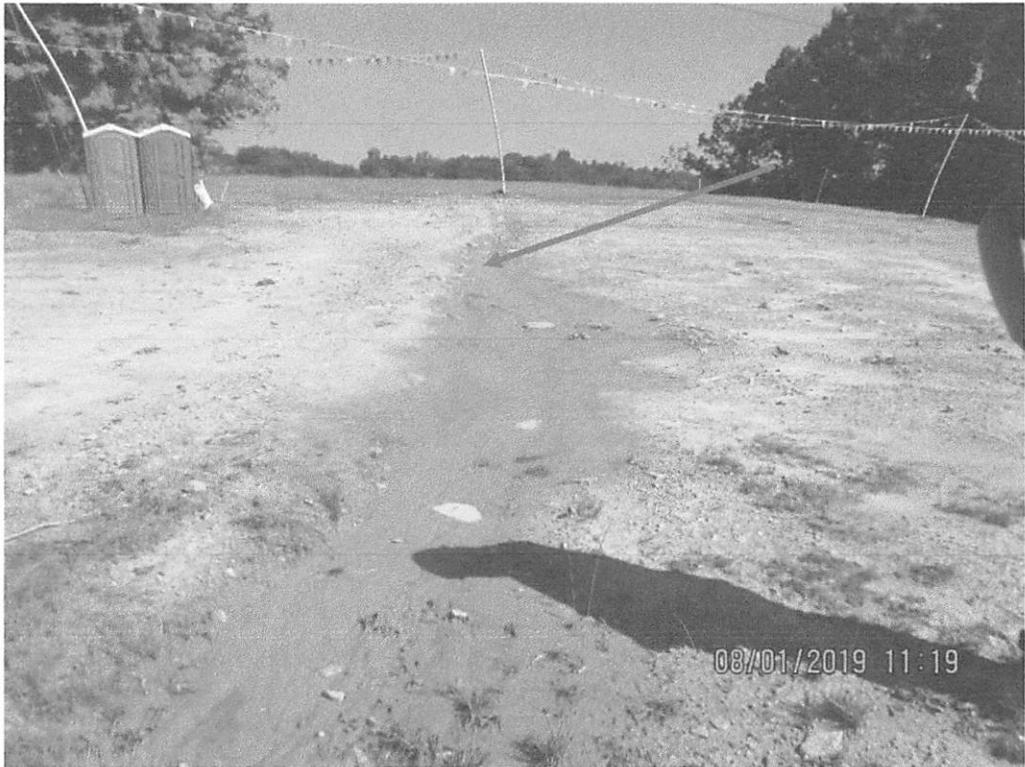
Facing North where Access Road MVP-BR-099 intersects ROW near station 3897+75. Arrow depicts where run-off was overtopping the diversion berm and flowing downslope.
