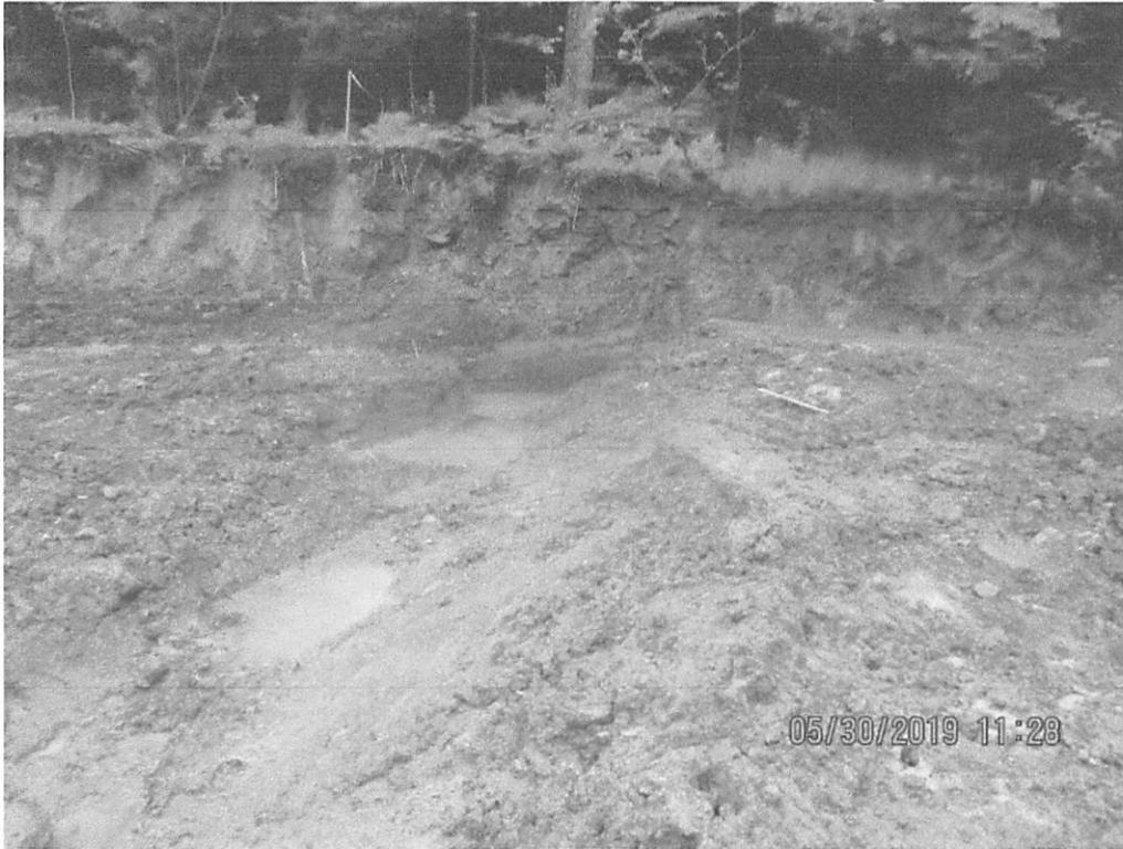
Seep running onto ROW above Stream S-N13. Diversion not stabilized near station 6940+00.
