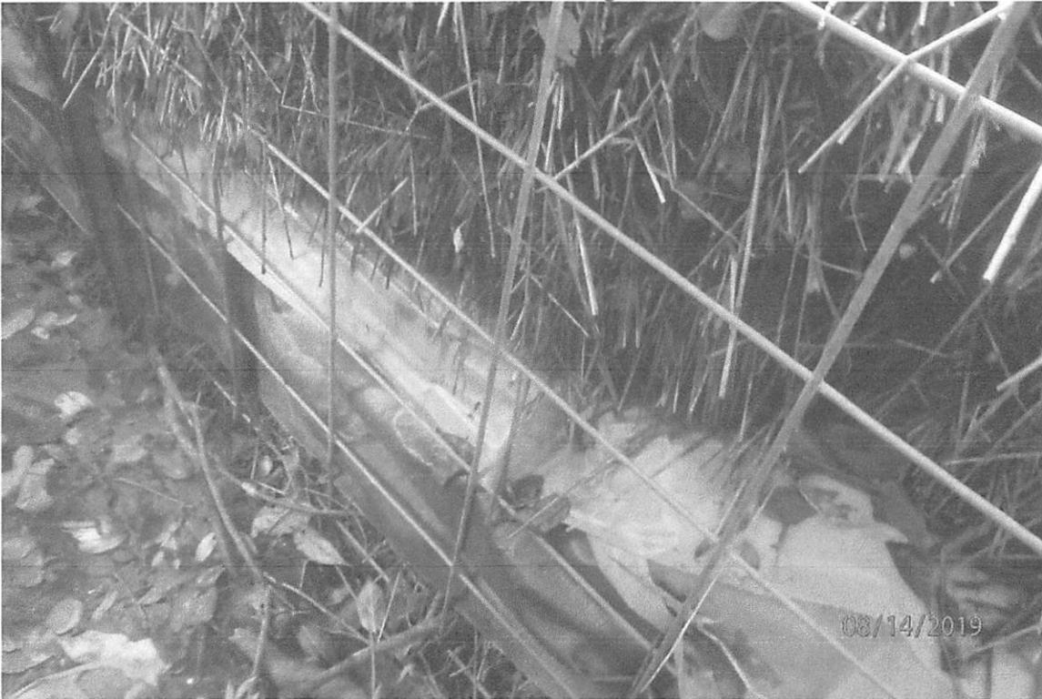
Dewatering structure with impermeable plastic installed, causing it to not function as designed in inspected area 8.
