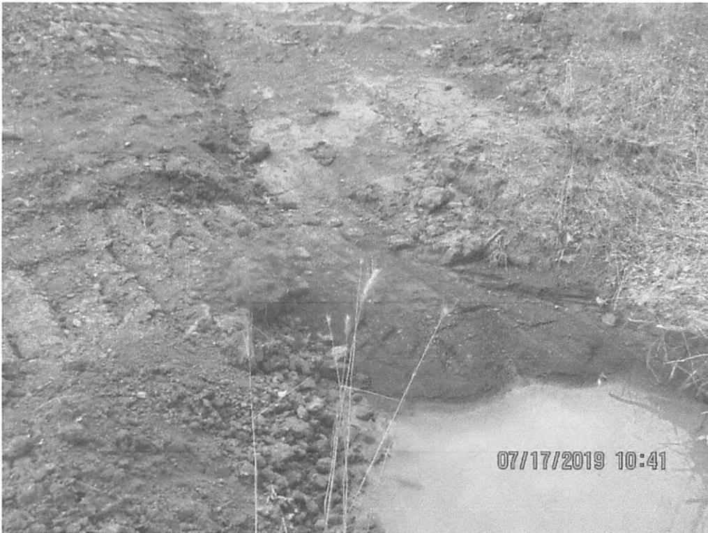
Sump at waterbar terminus near station 3151+47. Sediment deposits present past LOD due to lack of sump maintenance.
