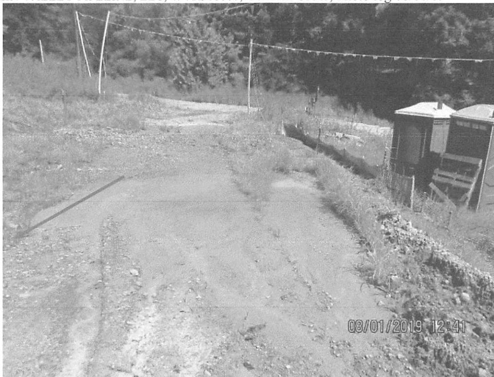
Above Access Road MVP-BR-097 and Falls Run (Stream S-J70) facing North. Run-on entering LOD and causing sediment to overwhelm controls. Arrow depicts where run-on was coming onto Access Road.
