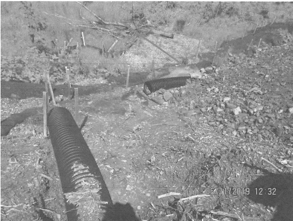
at station 7636+00 at waterbar outlet and slope drain. Slope drain was being undercut. Sediment was overwhelming perimeter control. Sediment deposits observed past controls and LOD.
