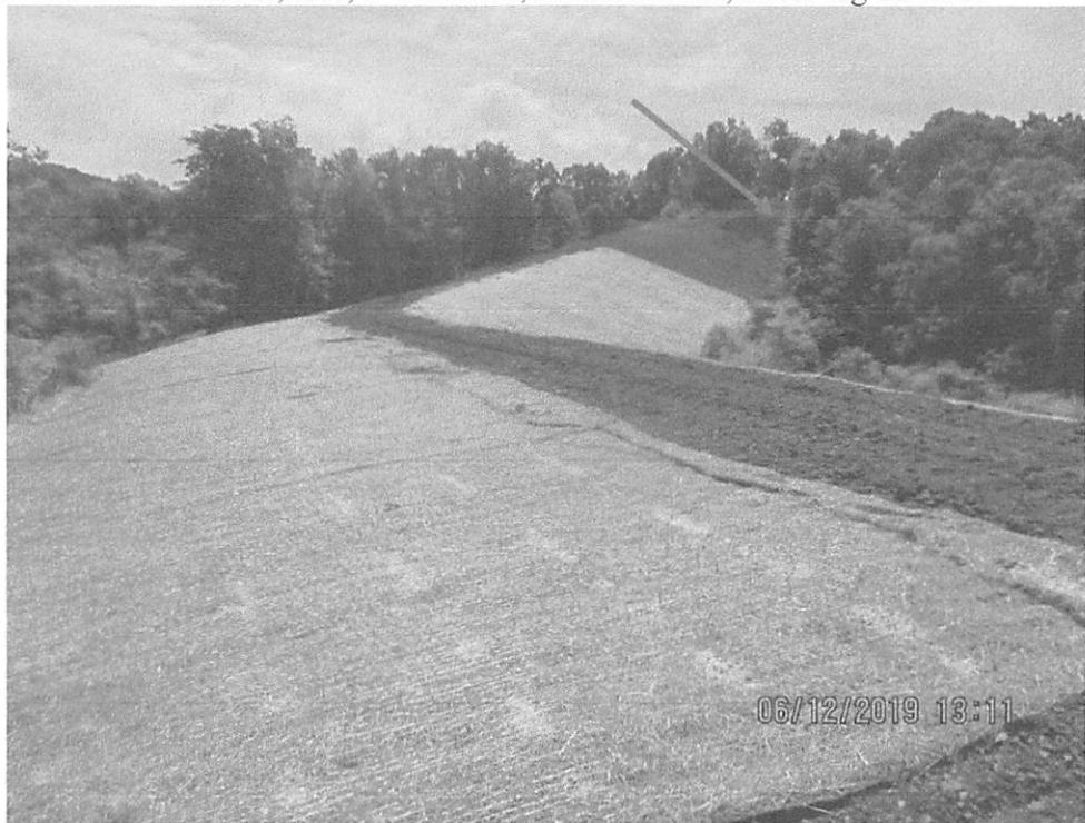
Upslope of Dargo silt fence. Facing South toward AR-221. Arrow depicts where dozer work was ongoing during inspection and controls needed maintenance.
