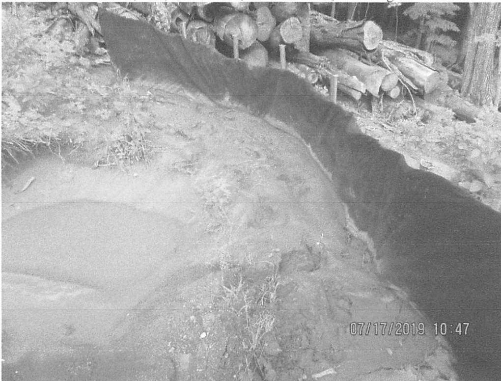
Waterbar terminus and sump at station 3149+00. Sump full of sediment and sediment deposits past LOD.
