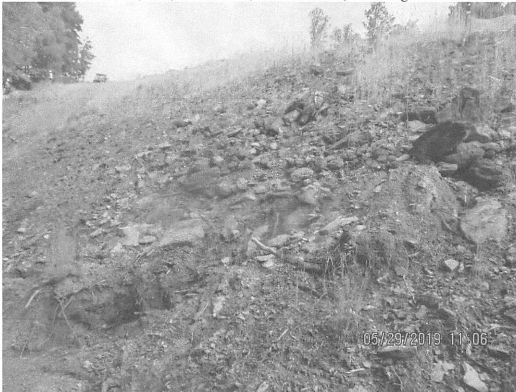
Fill slope with erosion present above diversion berm Outlet 3.
