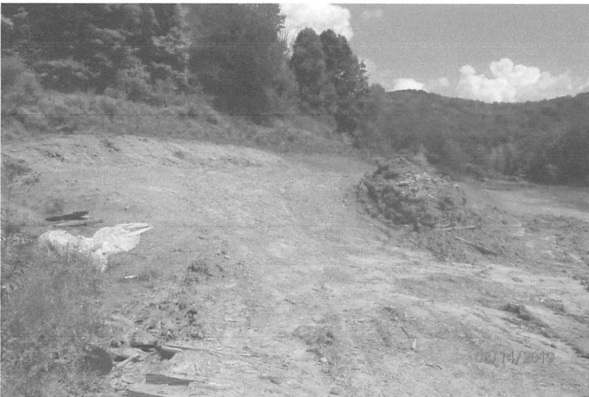
Area of disturbance associated with an extra workspace in inspected area 8 showing the lack of temporary stabilization, even though the site has been idle for a long period of time.
