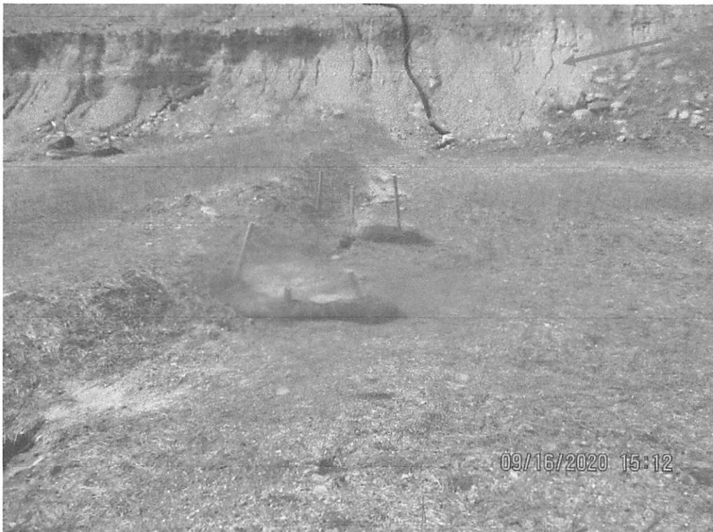
Erosion occurring on cut slope (red arrow) below slope drain outlet at Station No. 6450+76. Erosion present in waterbar. Area not reseeded.
