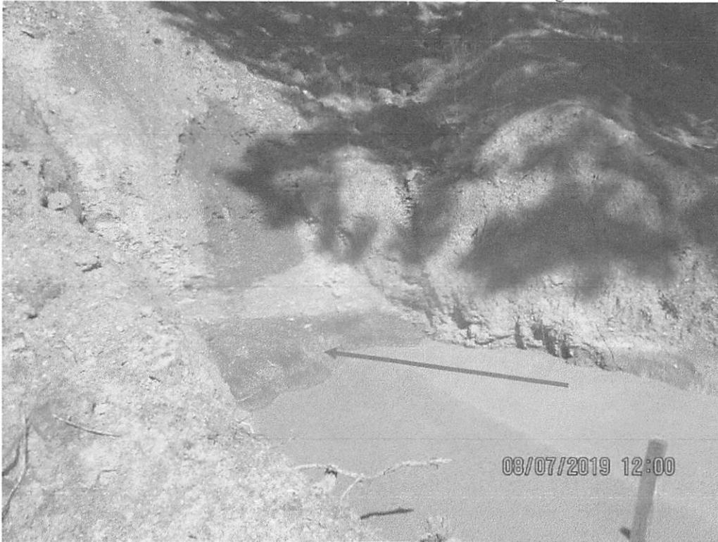
Near station 8955+00. Sump below waterbar terminating onto fill slope. Sump overwhelmed with sediment.
