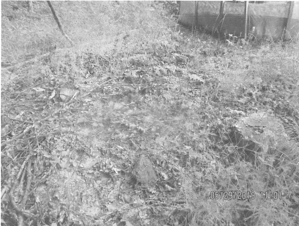
below diversion berm Outlet 2 near 4031+00. Scouring of vegetation below control.
