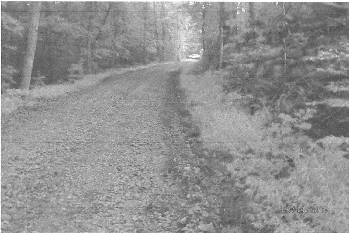
Access road MVP-BR-092.01 showing the area where concentrated flow stormwater is flowing from the top of the slope to the base of the hill due to poor maintenance on the installed culvert. The diversion lacks installed BMPs.
