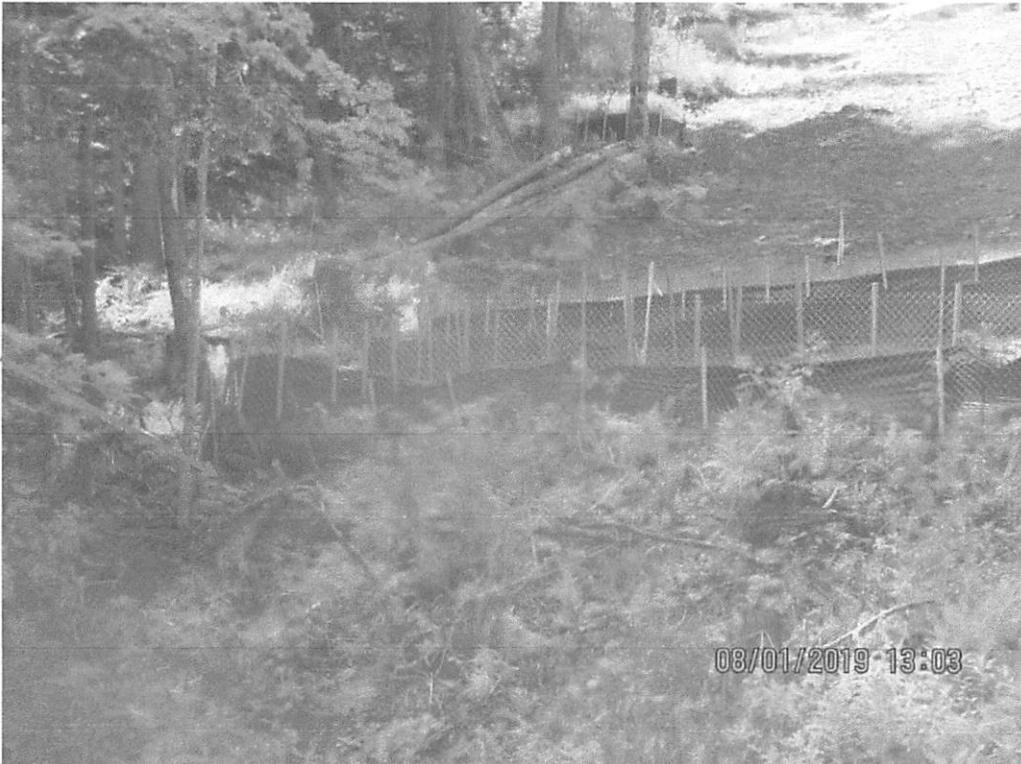
Controls above the South side of Falls Run (Stream S-J70) and US 19/Hwy 4 ROW crossing. Scouring present below controls.
