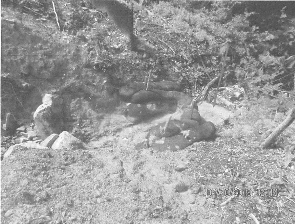
Downslope of slope drain outlet below seep coming onto ROW at Station 6510+40. SLW and sediment overwhelming controls.
