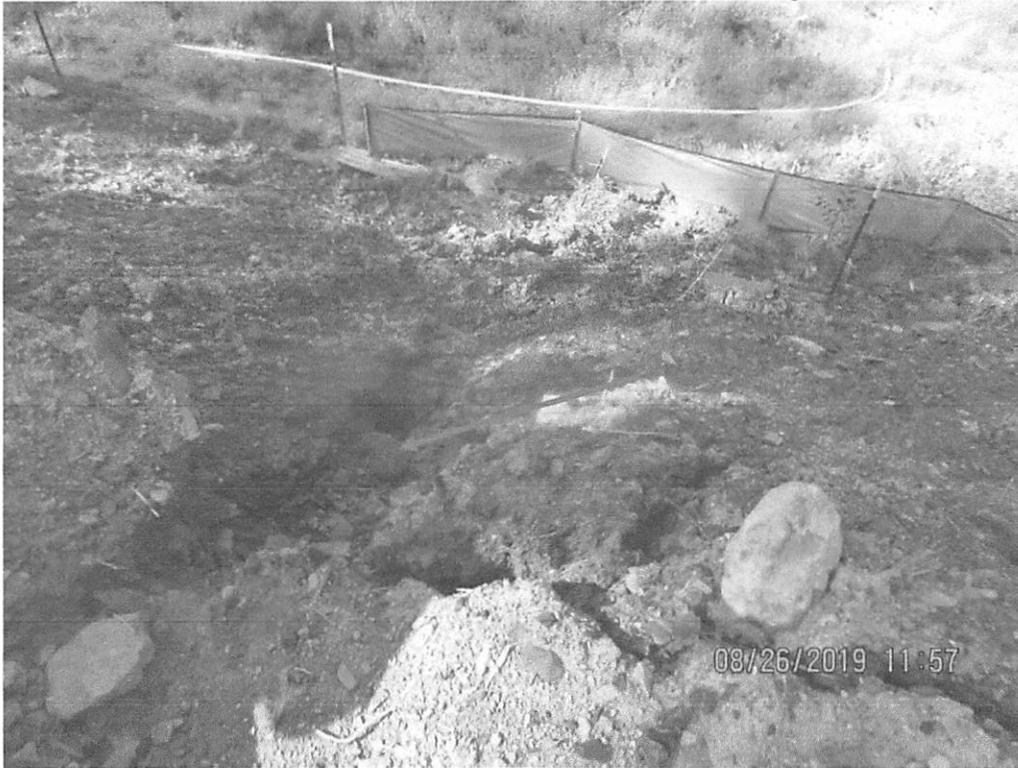
Near station 1833+00. Erosion occurring on slope resulting in sediment deposits being present past the LOD.
