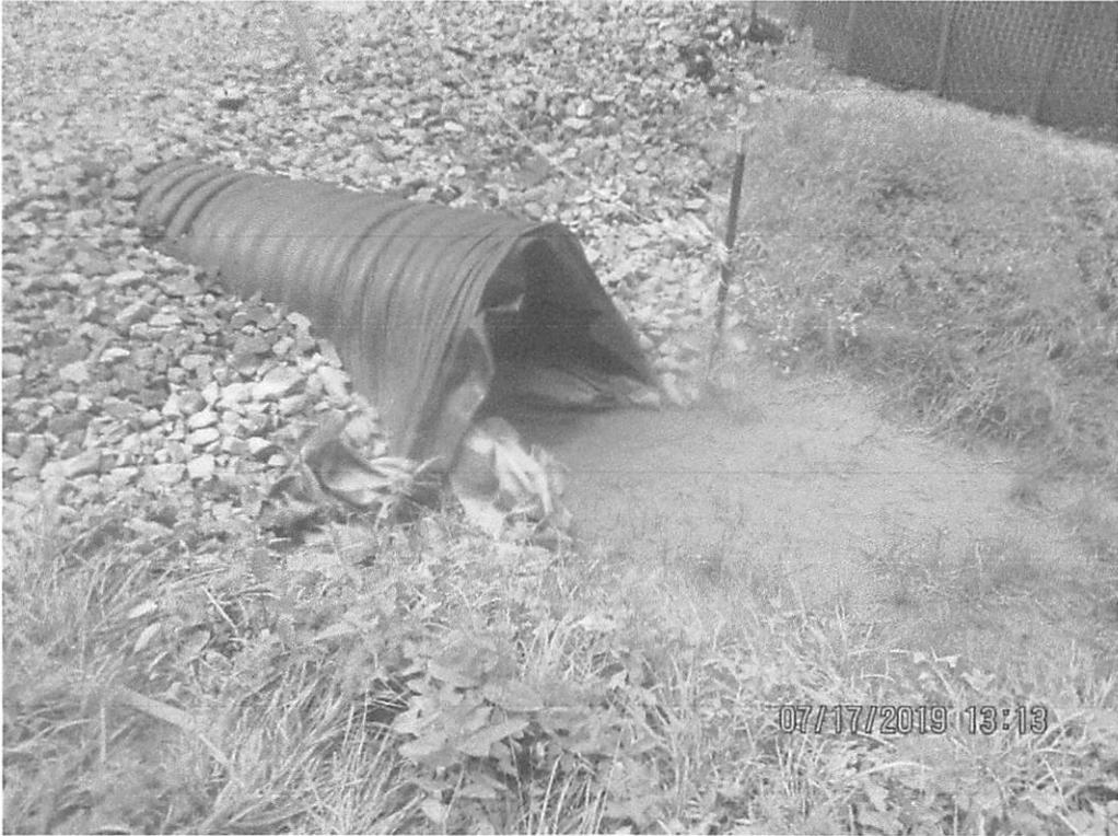
Sediment deposits and sediment-laden water present in ditch that conveys under ROW construction entrance, connects to elbow, conveys under CR23, and outlets on South side of road above Stream S-UV12.
