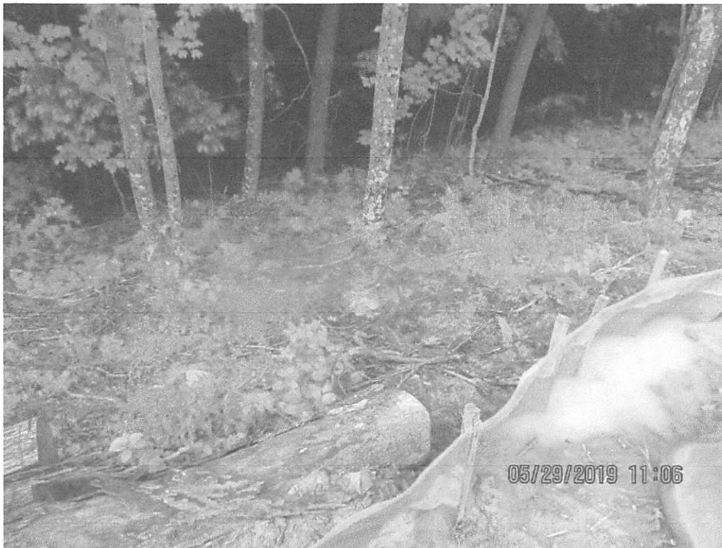
Downslope of diversion berm Outlet 3 controls. Scouring of vegetation with sediment deposits present past LOD.
