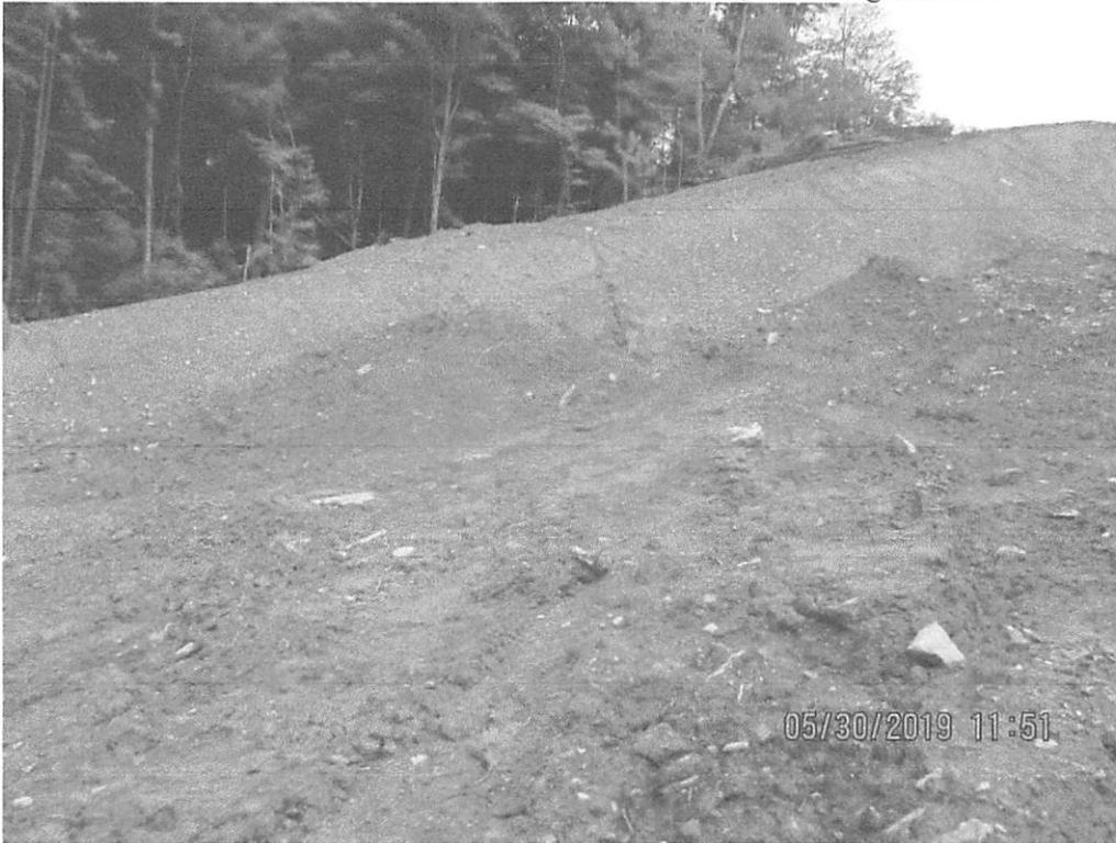
Facing upslope at Deepwell road construction entrance near station 6504+20. Erosion present on fill slope and ROW leading to waterbar.
