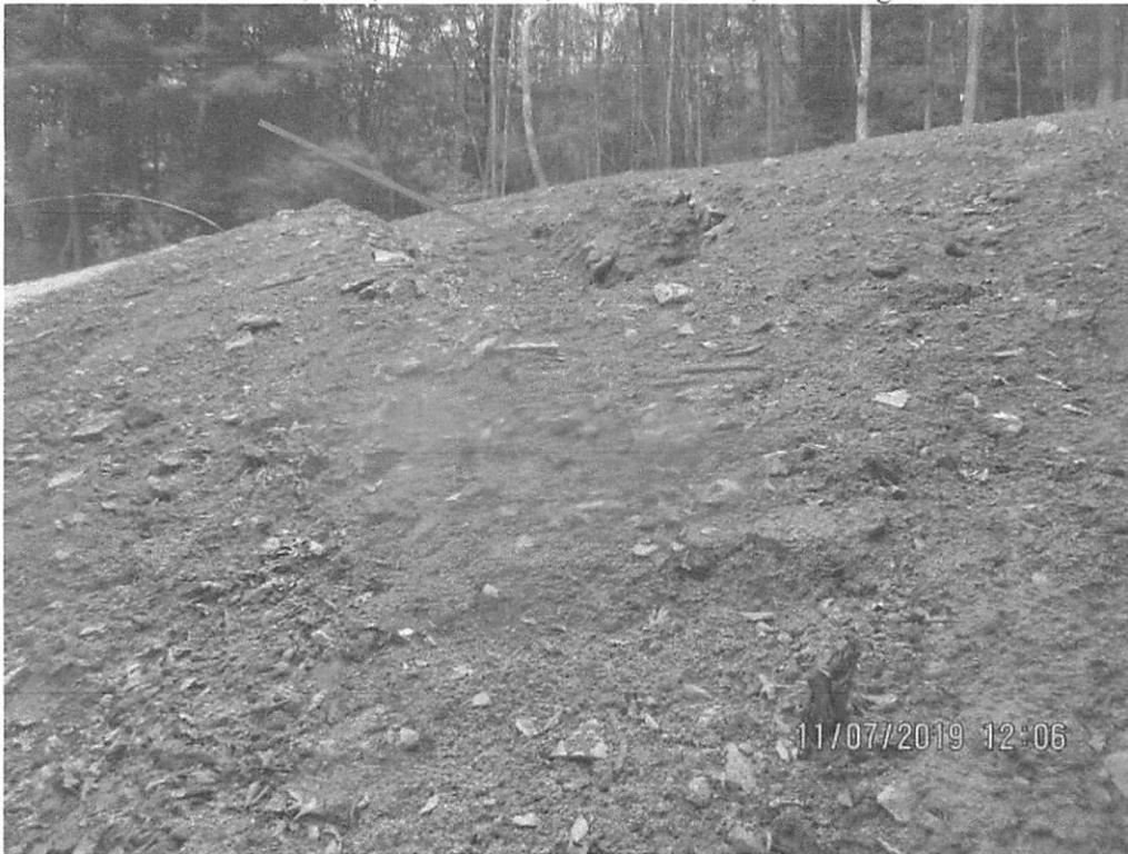
Waterbar terminating onto ROW above slipped section of ROW near Station 3946+00 with no outlet control present. Arrow indicates sump at waterbar terminus.
