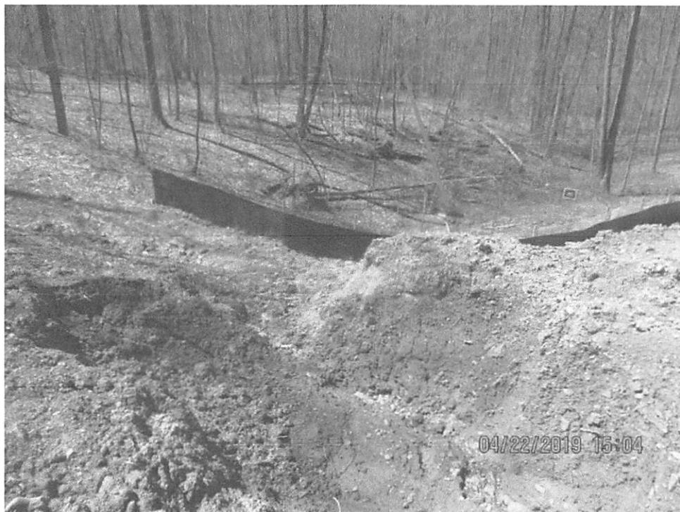
Stream S-T35(A) facing downslope waterbar terminus at Station 8633+71. Waterbar appeared to be directed toward stream. Controls were buried in sediment where erosion was present. Super silt fence was added after clean-up occurred. Sediment deposits were present in stream.
