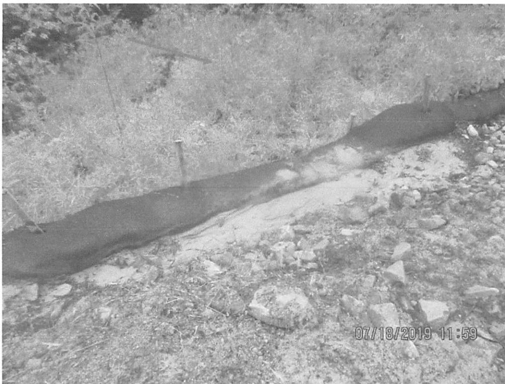
Perimeter controls along MVP-WB-119 overwhelmed with sediment with sediment deposits past the LOD. Arrow depicts sediment deposits.
