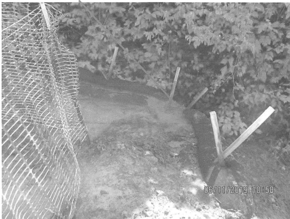
Above Lower Krosier Road crossing. Erosion present on ROW above waterbar. Sediment being deposited in waterbar and sump, overwhelming sump and perimeter controls near station 7604+41.
