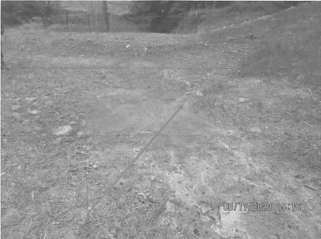
Erosion occurring on fill slope that is downslope from run-on being conveyed onto ROW at Station No. 6613+00.
