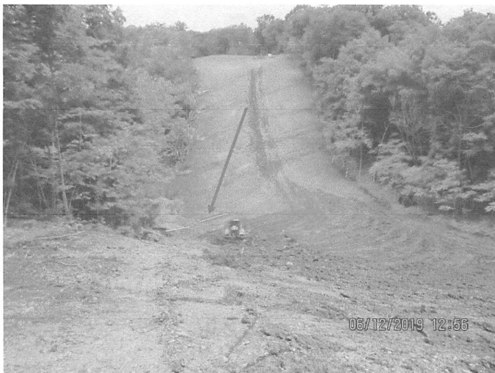
South Side slope facing downslope (North) at Dargo Silt fence. Red Arrow depicts where slope drain terminated onto ROW.
