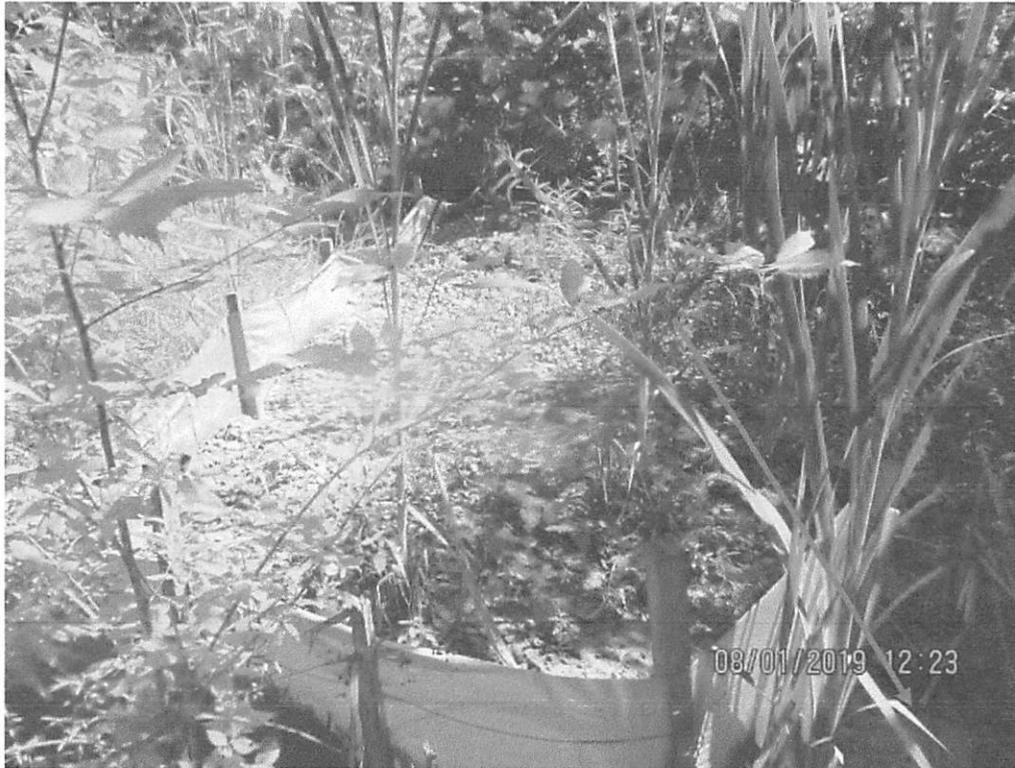
Controls located below washed out section of AR-095 and above stream S-J74 and Wetland W-J42. Arrow depicts where controls were overwhelmed and sediment-laden water had flowed past controls.
