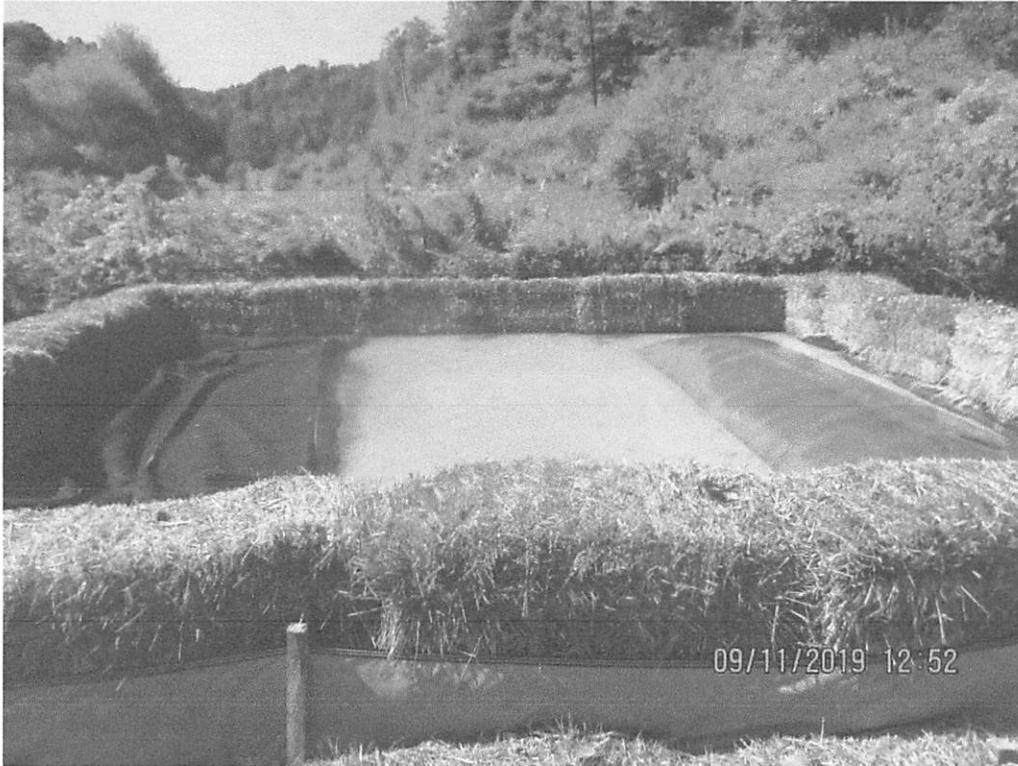
Dewatering structure for Goose Run (Stream S-B75) bore near station 645+35. Dewatering structure full of sediment-laden water.
