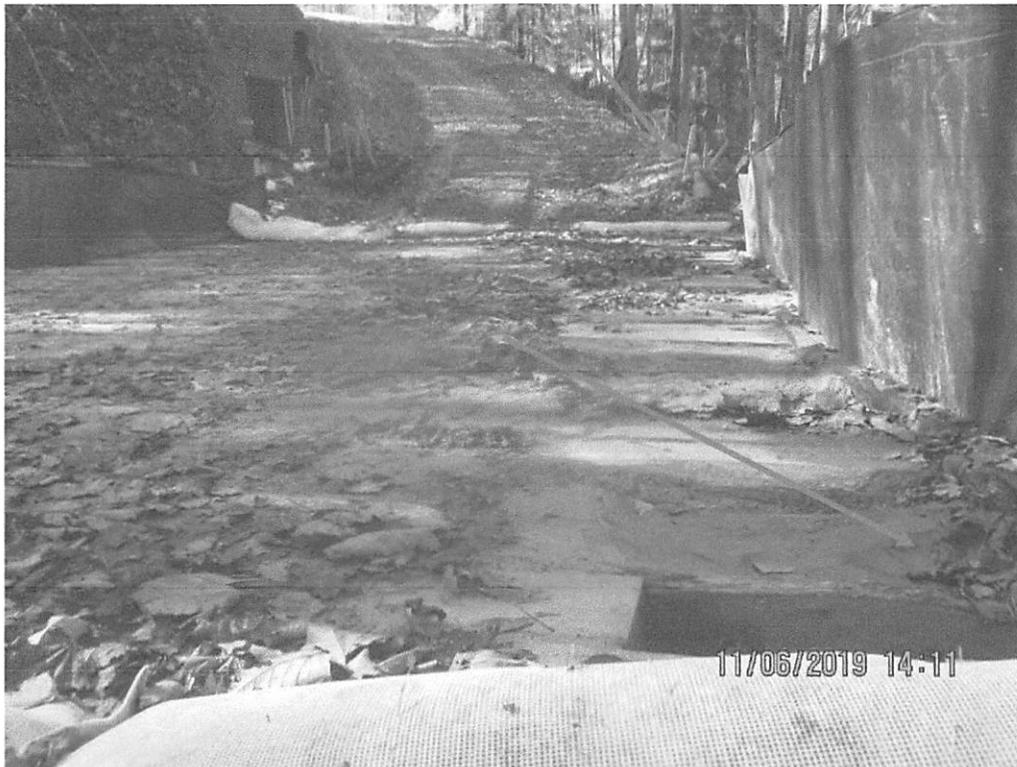
Facing upslope on Stream S-S2 bridge crossing. Arrow depicts where erosion was present on road resulting in controls being overwhelmed and sediment being deposited on bridge and past LOD.
