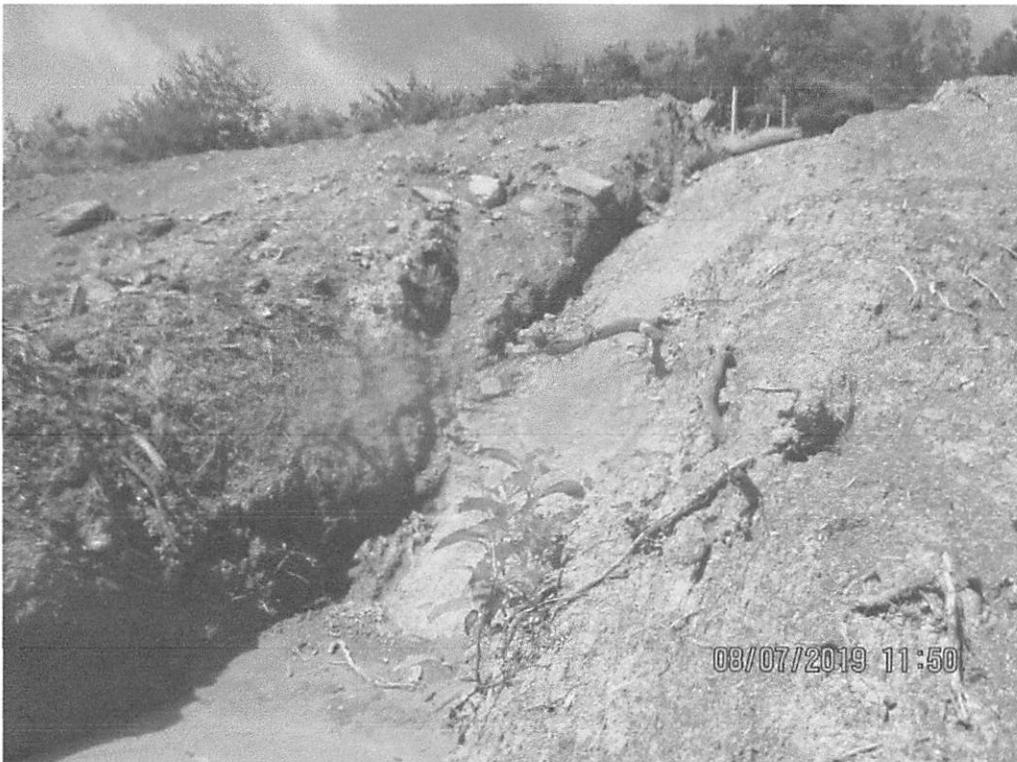
Waterbar terminating onto slope near station 8955+00. Erosion present on slope. Sump overwhelmed with sediment.
