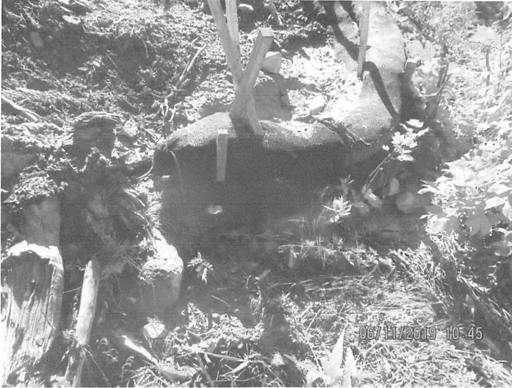
Downslope of waterbar outlet near 7604+41. Perimeter controls in need of maintenance. Sediment deposited behind perimeter controls. Sediment deposits observed past controls and LOD.
