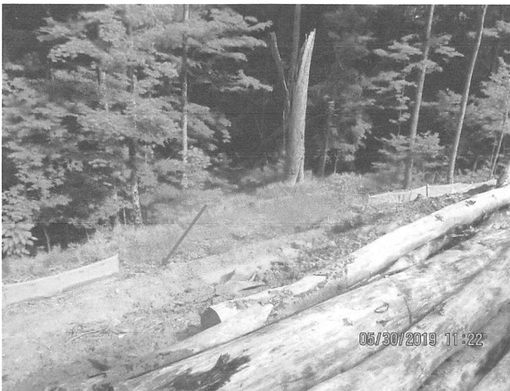
Station 6497+50. Perimeter controls not installed per SWPPP. Diversion berm installed, however, arrow depicts section where sediment was being deposited against controls which were not tied-in to berm.
