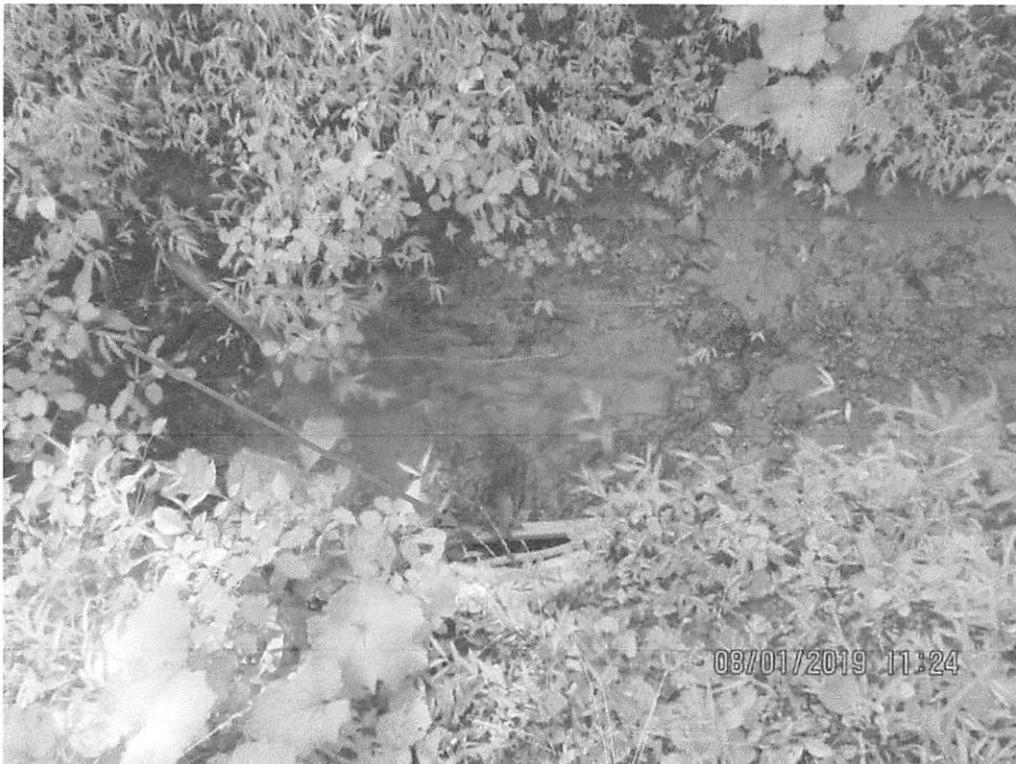
Sediment deposits observed along CR 24 downslope of Access Road MVP-BR-099 near station 3897+75. Arrow depicts culvert location that conveys under CR 24. Culvert inlet also demarcates where delineated stream S-K35 begins.
