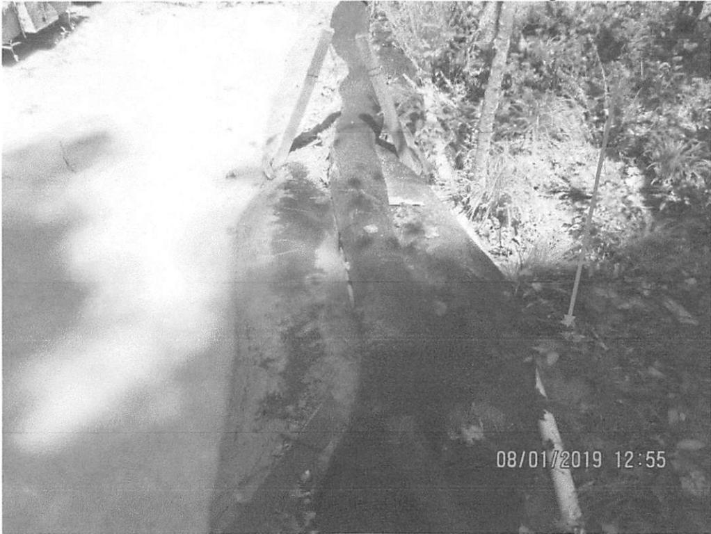
Perimeter controls below timber mat bridge on edge of LOD with sediment deposits past the LOD below MVP-BR-097.
