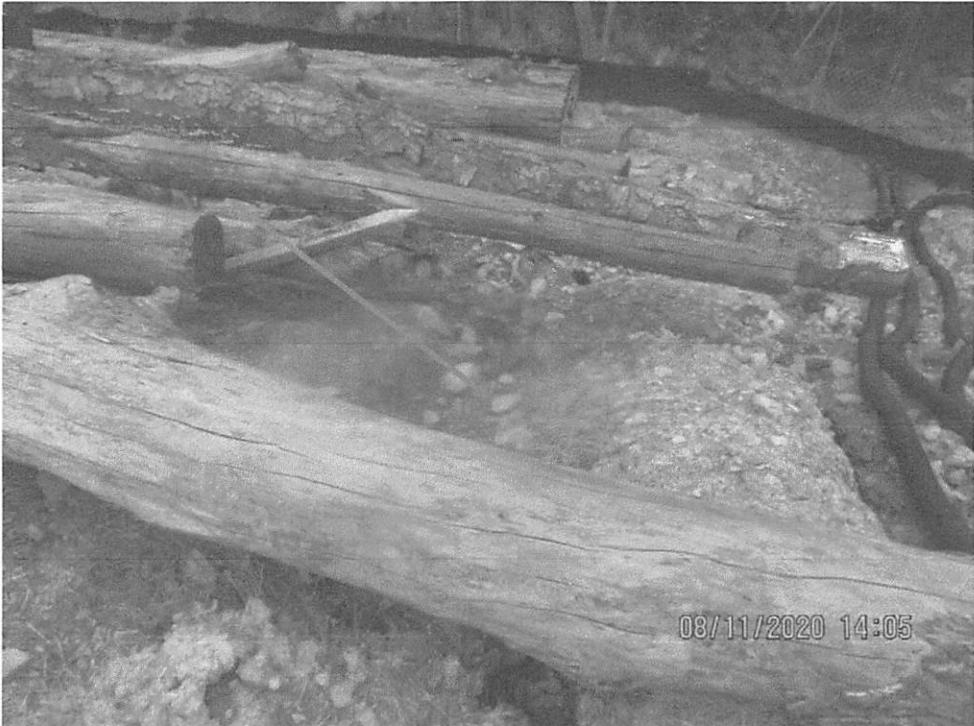
Erosion present (red arrow) next to log pile and slope drains that were recently installed near Station No. 6485+50.
