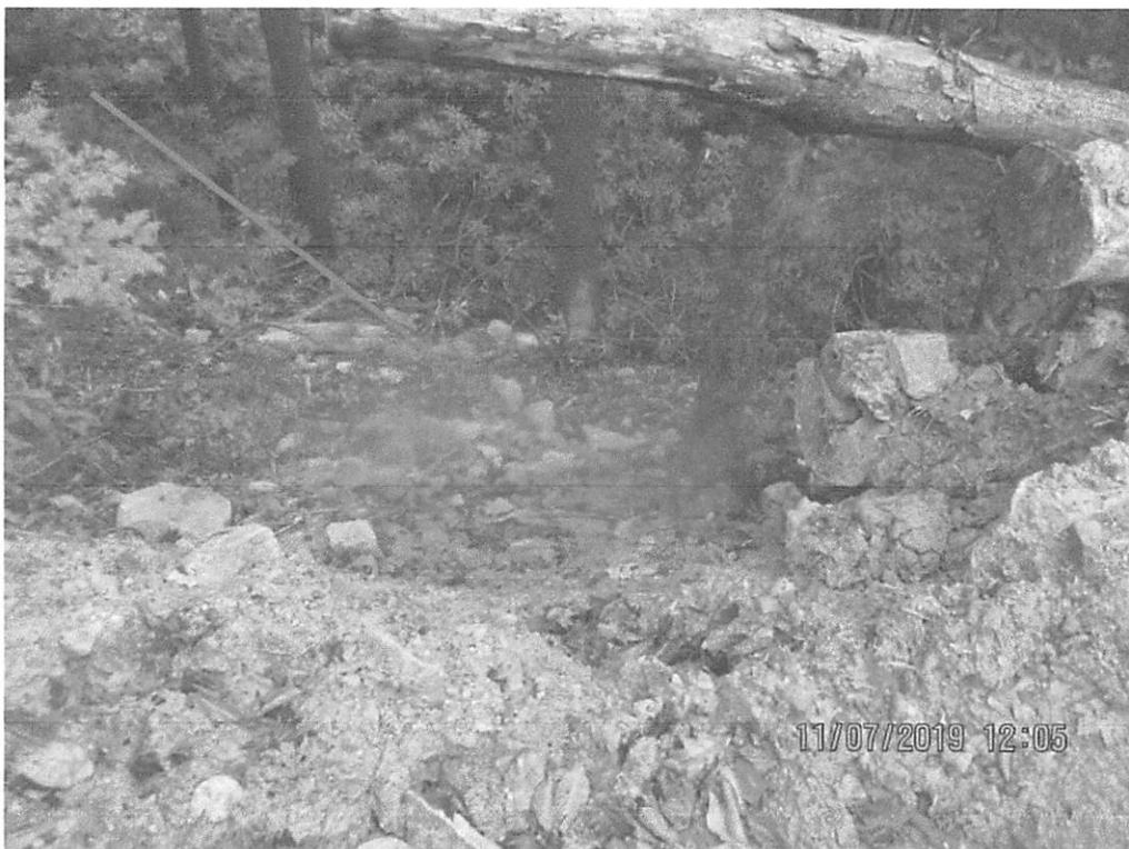
Section of ROW above Elliott Run where material/debris was slipping upstream of larger slip impacting Elliott Run near station 3946+00. No perimeter controls were in place at the time of inspection. Large rocks observed in stream above larger slip.
