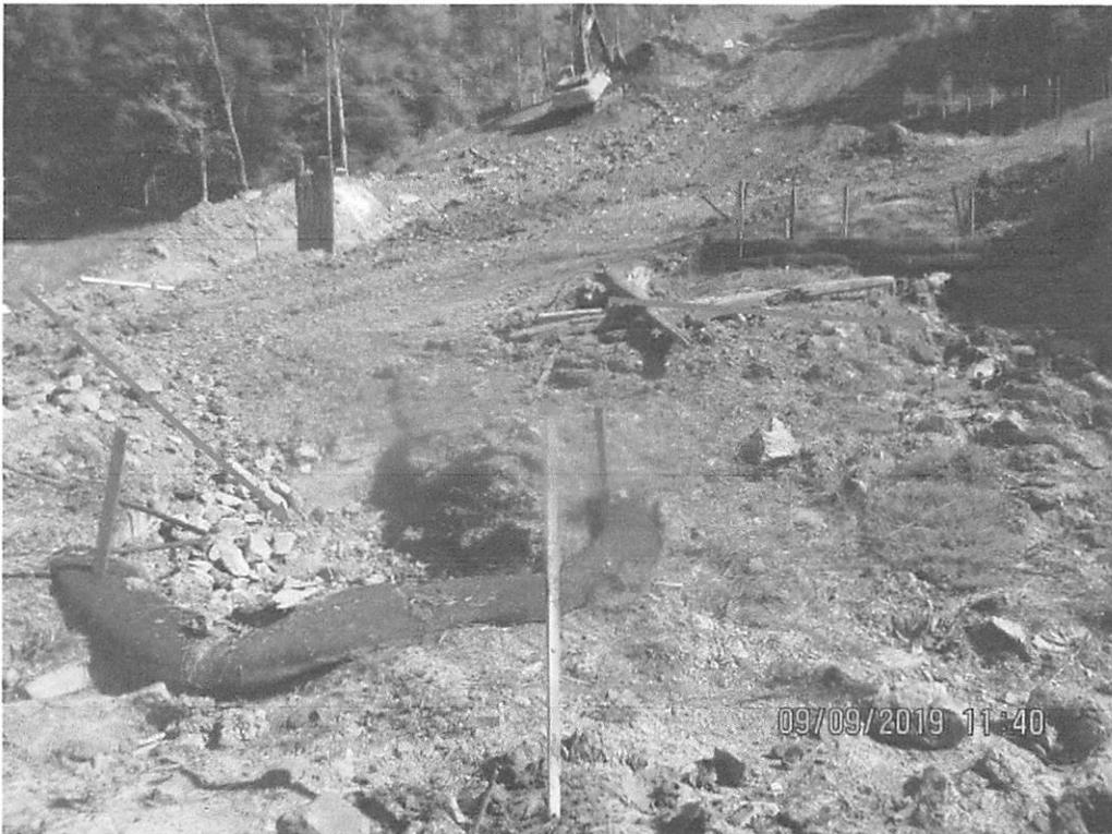
At station 3089+00 facing North. Arrow depicts sump not being maintained and erosion on slope below controls.
