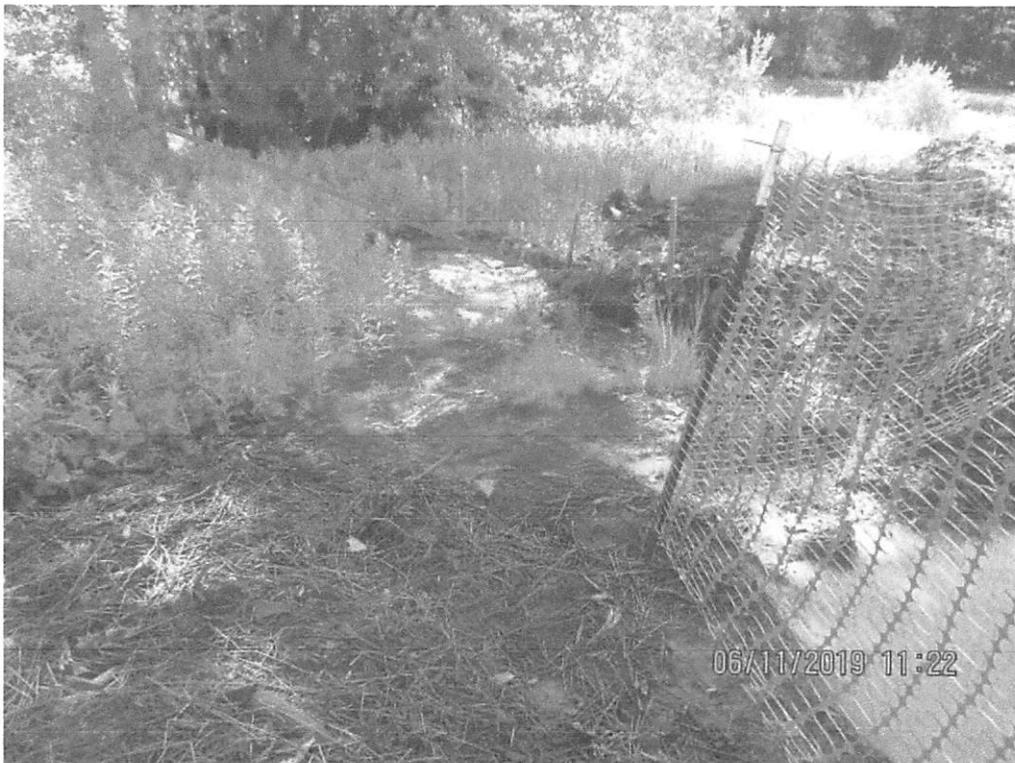
Facing South (Downslope) at station 7609+50. Waterbar outlet controls overwhelmed with SLW and deposits.
