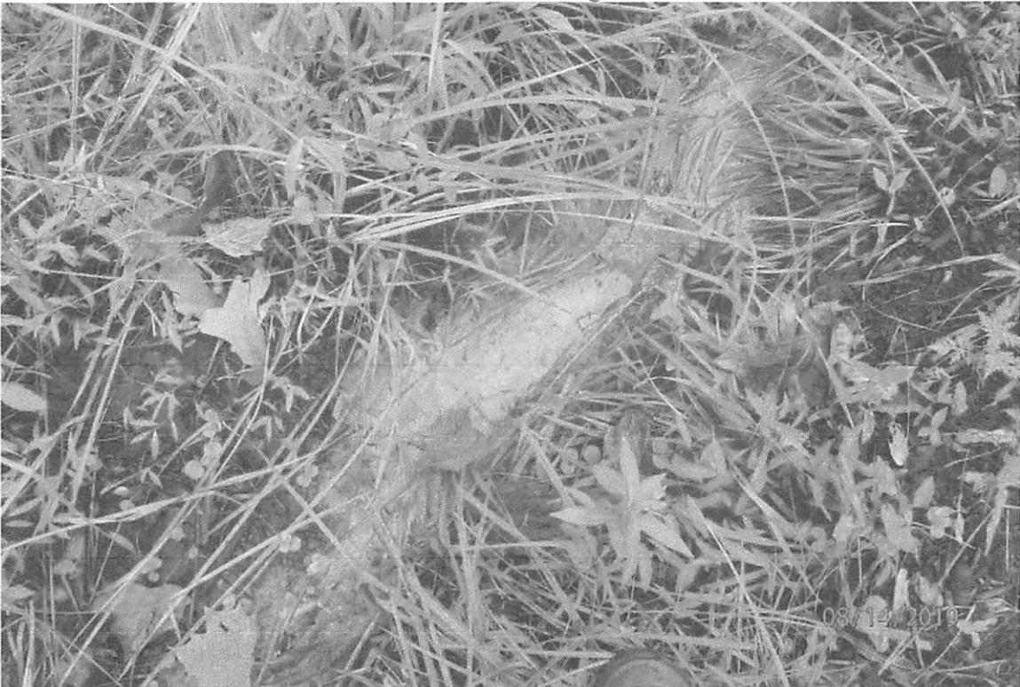
Offsite sediment deposits adjacent to inspected area 3, showing where a dewatering structure was placed offsite and caused offsite deposits.
