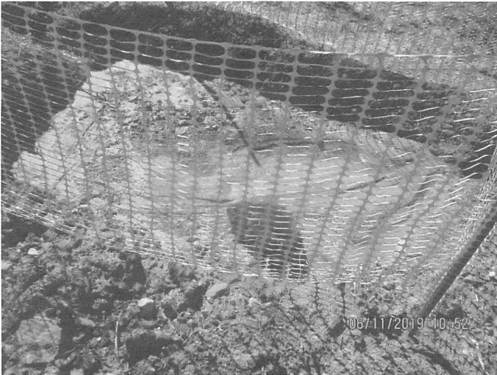
Above station 7604+41. Waterbar had sediment from erosion, causing sump to be full of sediment.
