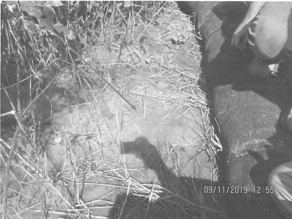
Sediment-laden water flowing under controls and into vegetation above Stream S-B75 (Goose Run) near station 645+35.
