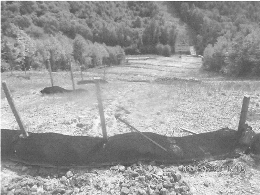
Standing at Access Road 159.01 facing downslope from Station No. 6657+00. Erosion present on slope (red arrow) with deposits in the waterbar channel.
