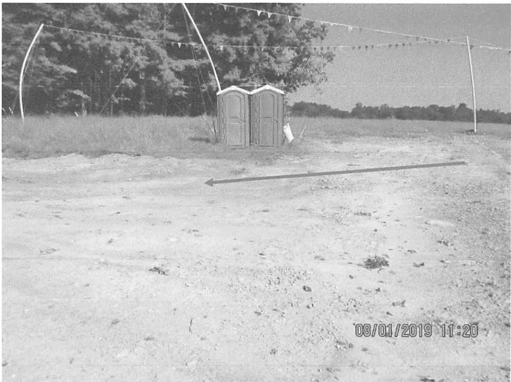
Downslope of diversion berm near station 3897+75. Arrow depicts where sheet flow due to run-off was occurring.
