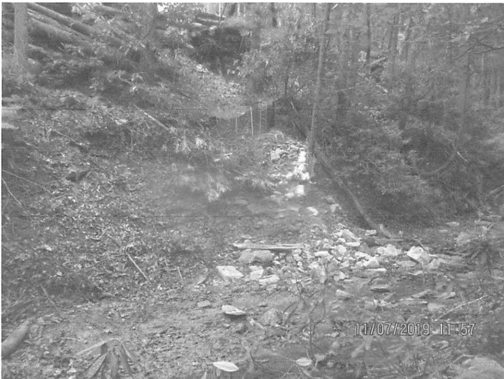
Slip that impacted Elliott Run near Station 3946+00 and was not reported to WVDEP spill reporting hotline. Super silt fence installed near the edge of LOD.
