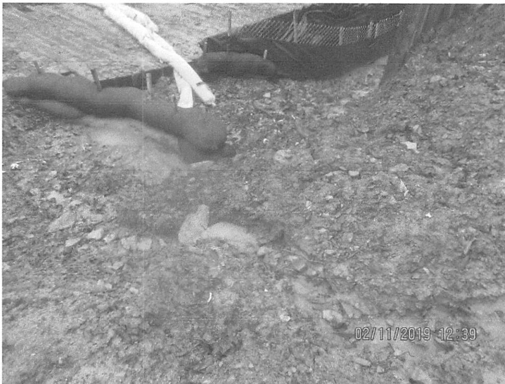
Erosion occurring due to runoff from ROW and being diverted to Wetland W-IJ-55
