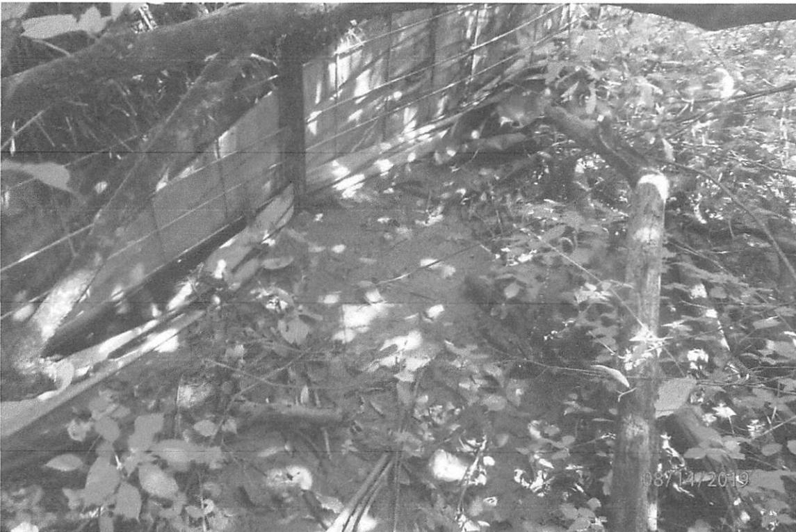
Dewatering structure with impermeable plastic installed causing it to not function as designed in inspected area 8. Offsite sediment deposits pictured.
