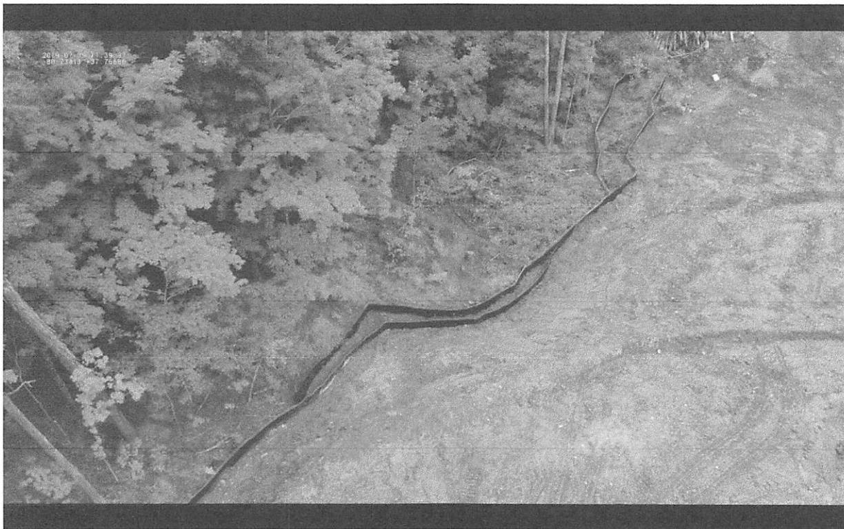
Stream S-T35A at station 8634+00 at the West side of the LOD. Arrow depicts additional super silt fence installed after impacts. Sediment deposits in stream.
