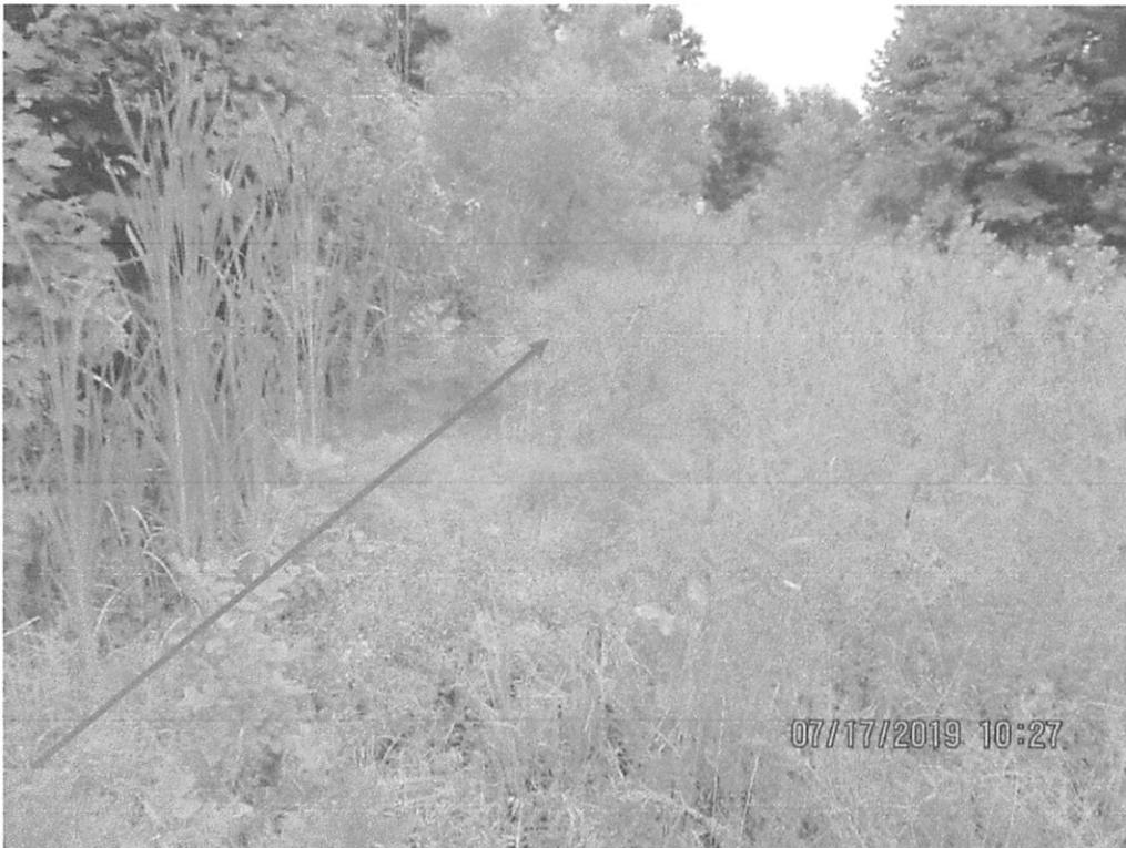
Area where sediment deposits were observed due to fill slope erosion at station 3159+46. Arrow depicts ditch line where deposits were present.
