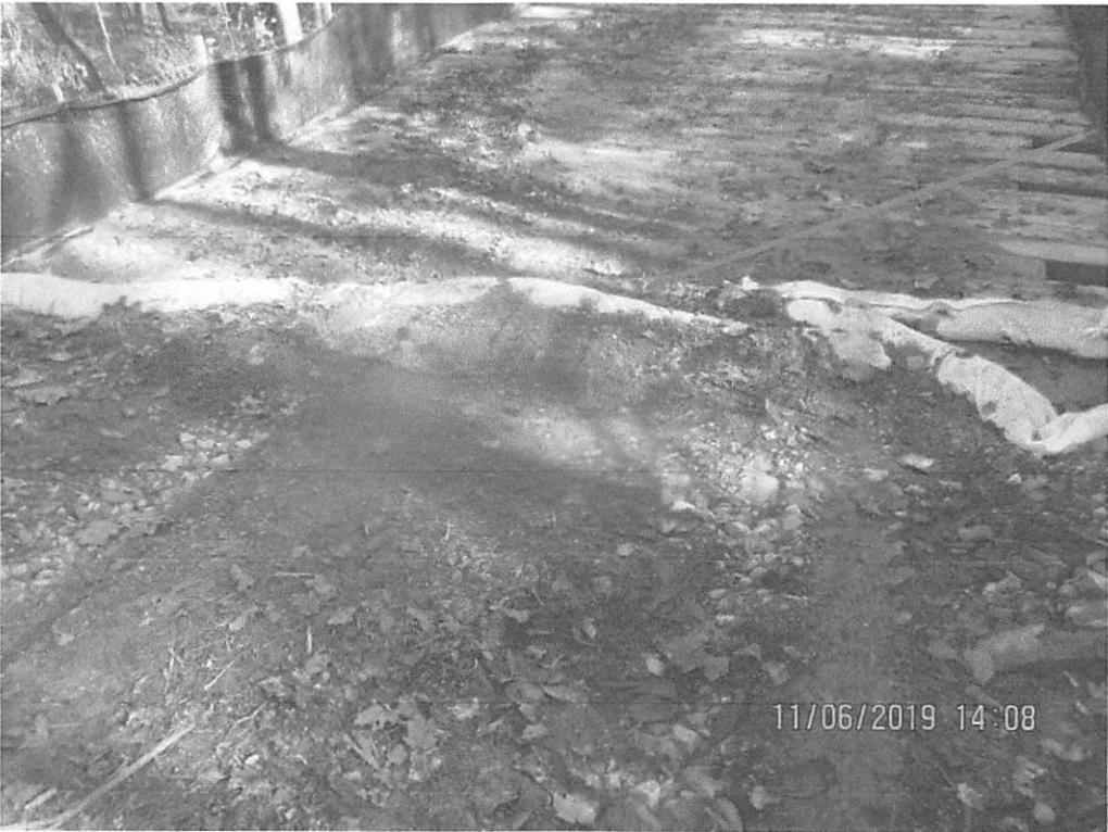
Stream S-S2 near station 4364+00. CFS at edge of bridge crossing flattened with sediment deposits built up behind it.
