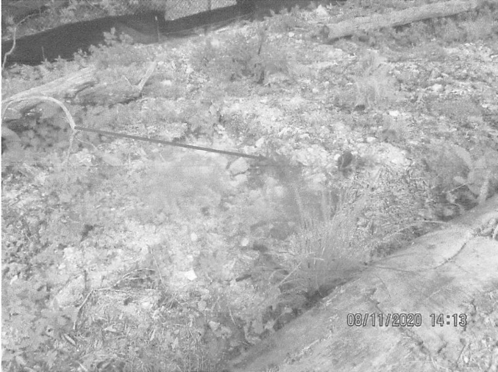
Erosion on fill slope below log pile (red arrow) near Station No. 6485+50.
