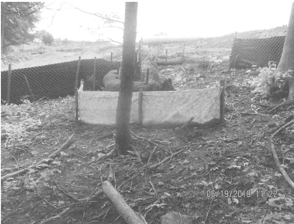
Waterbar outlet with enhanced secondary controls added at Station 6587+00.
