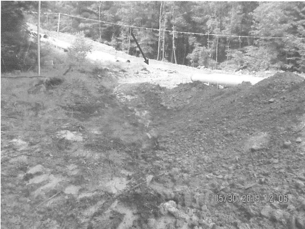
Sediment deposits and SLW traveling downslope at station 6510+40. Seep was present in cut next to topsoil pile. Channel was not stabilized and conveyed to a sump with a slope drain that crosses ROW. Arrow depicts seep. Black arrow shows sump with slope drain inlet.
