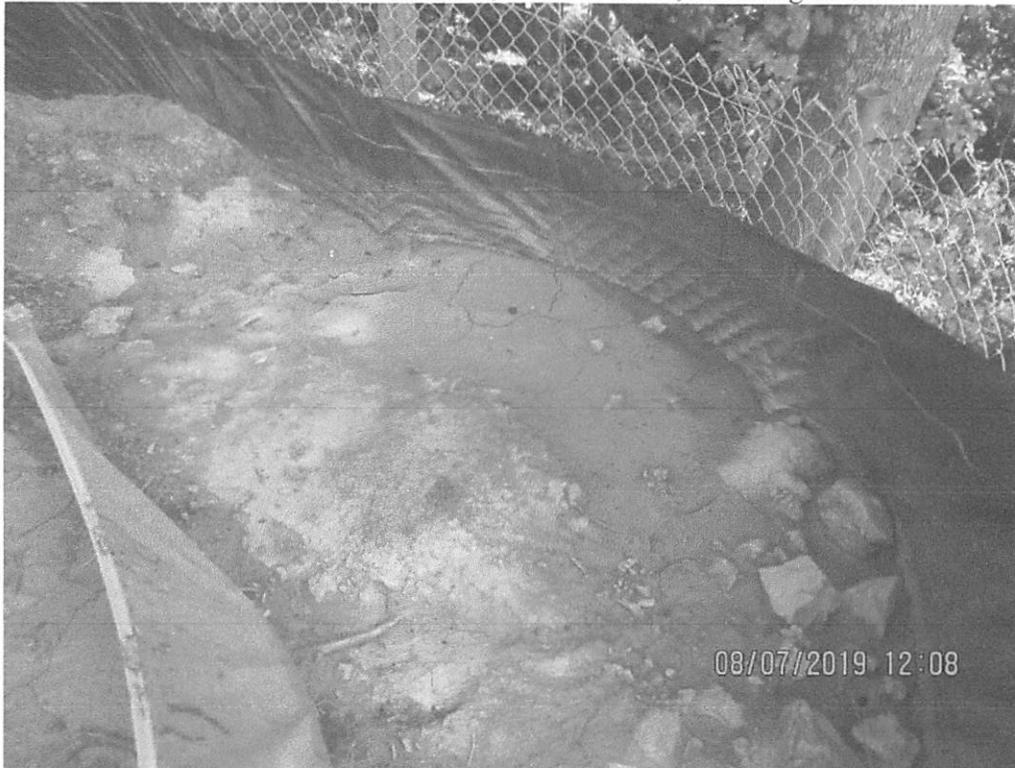
Further downslope near station 8951+00. Controls below waterbar termini with no outlet control terminating onto fill slope and above LOD. Controls needed maintained.
