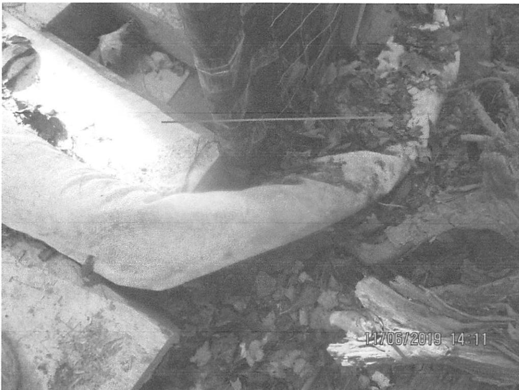
Downslope section of bridge where sediment-laden water was flowing around and past controls near station 4364+00.
