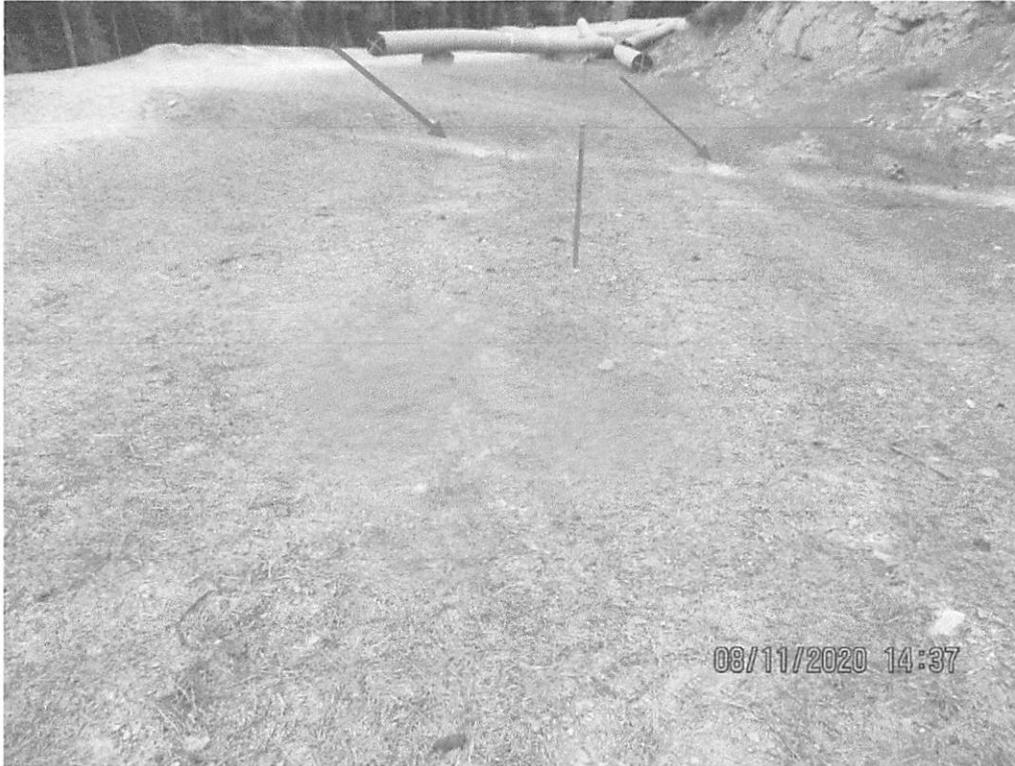
Near Station No. 6485+50 facing North. Sheet flow transporting sediment toward waterbar with sediment deposits (red arrows) in waterbar. Lack of 70 percent vegetative coverage.
