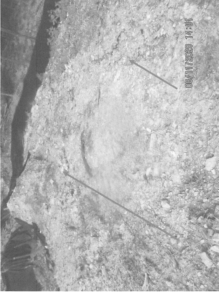
Erosion on fill slope near Station No. 6485+50. Lack of 70 percent vegetative cover and slope was not reseeded.
