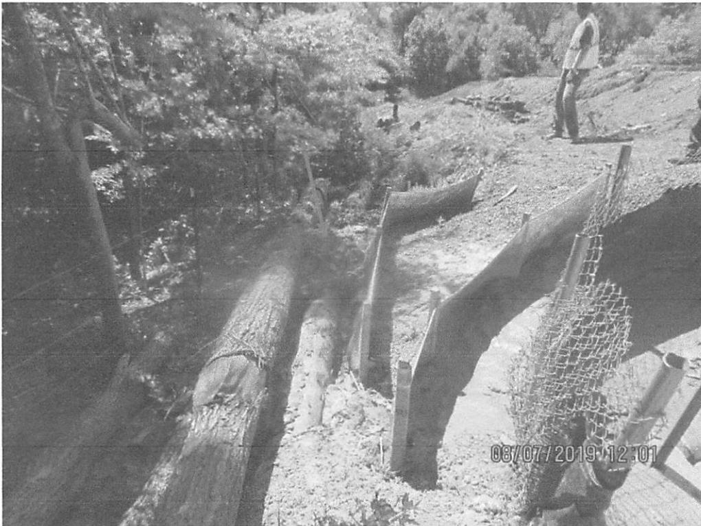
Near station 8955+00. Perimeter controls below waterbar terminating onto fill slope and sump that was full of sediment. Perimeter controls overwhelmed and sediment deposits present past log pile.
