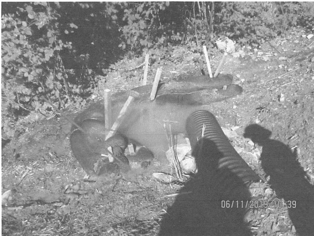
Below upper Krosier Road crossing near station 7576+01 facing downslope below waterbar outlet. Arrow depicts where run-off was flowing around controls and causing erosion downslope of controls.
