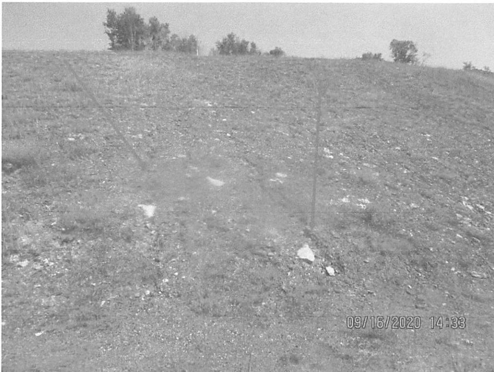
Rill erosion occurring on slope above AR-160.1 at Station No. 6698+00.
