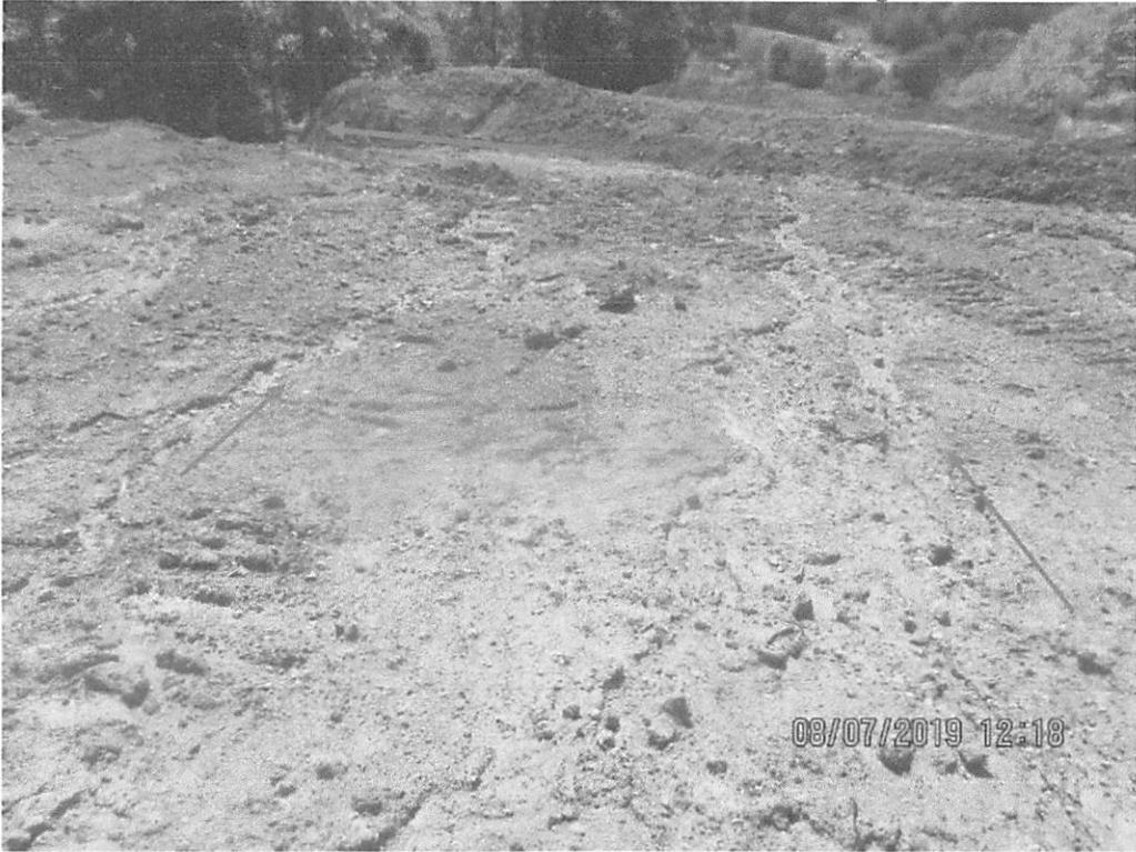
At top of steep slope facing South toward Boom Hollow Road at station 8951+00. Arrow depicts erosion on slope and waterbar with no outlet control.
