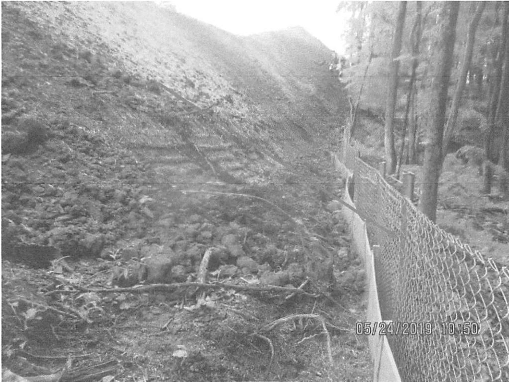
Near station 8419+00 facing South. Arrow depicts where material has slipped into P1 silt fence.
