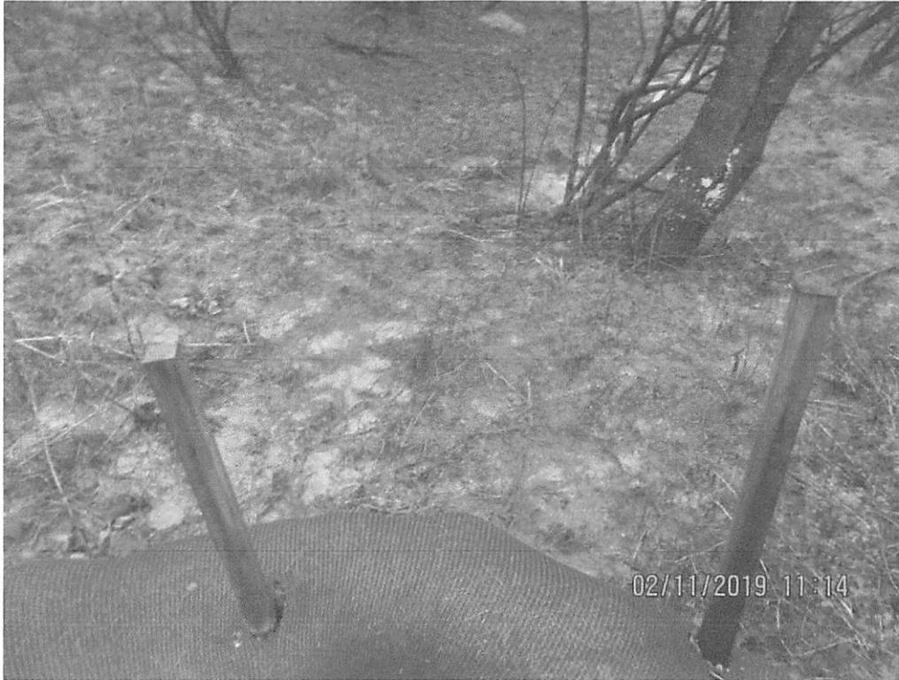
Evidence of sediment being deposited past LOD near station 6017+50
