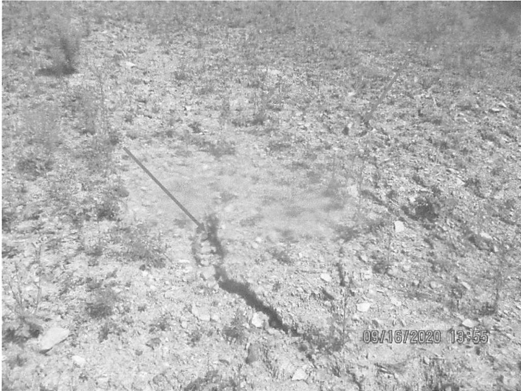
Rill erosion occurring between waterbars downslope near Station No. 6703+00.
