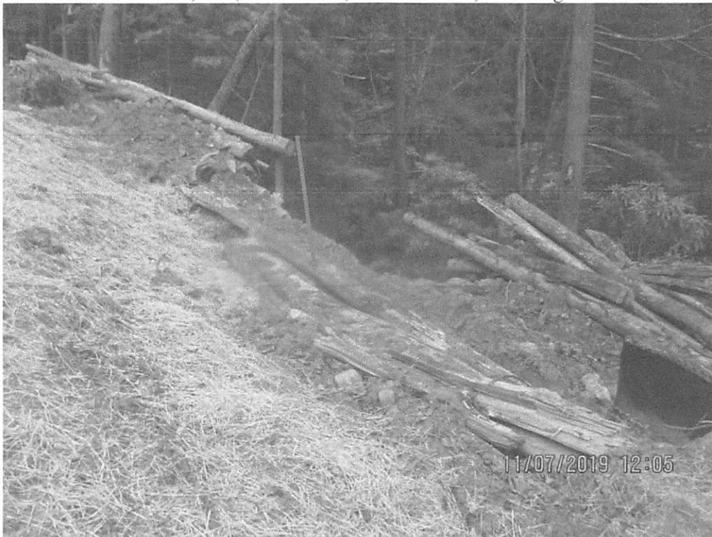
Section of ROW above Elliott Run where slip occurred near station 3946+00. Logs being used as perimeter controls (red arrow).
