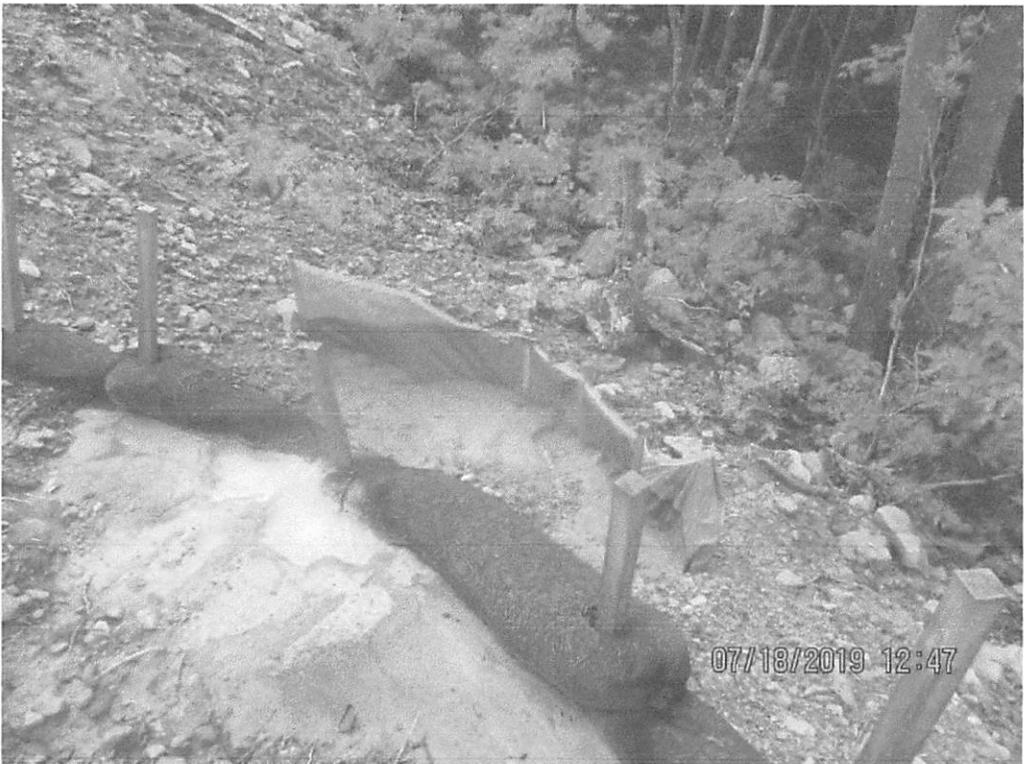
Waterbar outlet on opposite side of ROW at station 4559+96. Controls undercut and sediment deposits observed past controls and LOD.
