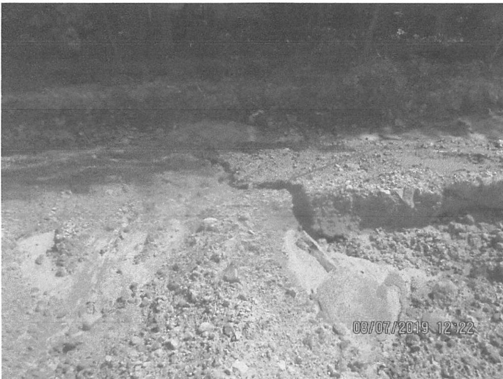
Fill slope near station 8946+00. Erosion present on fill slope resulting in sediment overwhelming perimeter controls.
