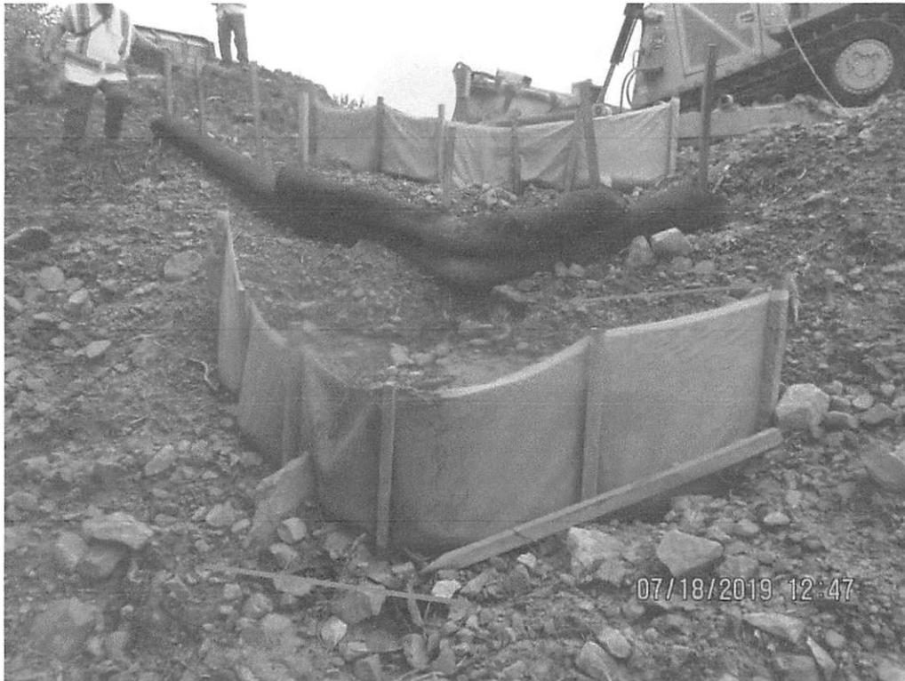
Waterbar outlet on opposite side of ROW at station 4559+96. Controls undercut and sediment deposits observed past controls and LOD. Arrow depicts undercut controls.
