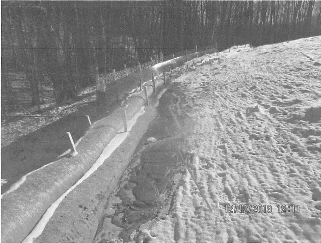
Sediment deposits present behind controls due to upslope erosion at station 8433+50.
