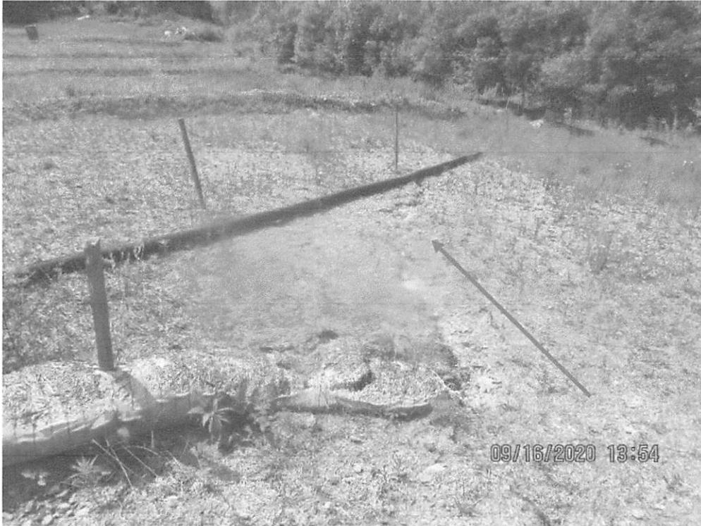
Further downslope from Station No. 6698+00 where trench drain was out-letting onto fill slope and causing erosion (red arrow).
