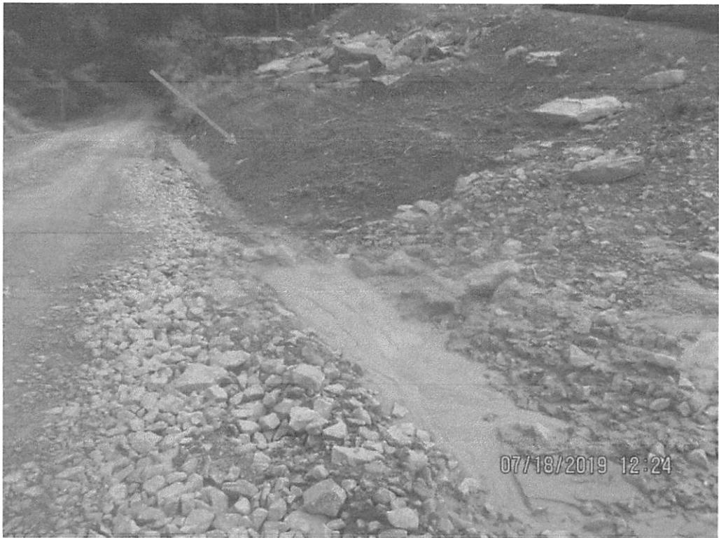
At station 4559+96 facing Access Road MVP-WB-119. Sediment deposits present in roadside ditch.
