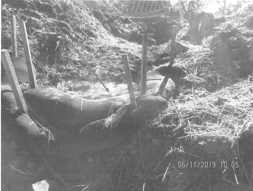
200 ft upslope of Krosier road crossing. Waterbar outlet in need of maintenance. Controls overwhelmed with sediment. Deposits present past LOD.
