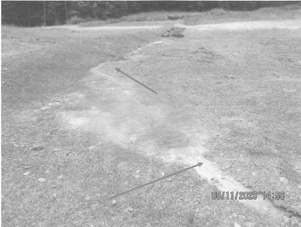
Facing Southwest at the Route 39 crossing. Red arrow depicts where concentrated flow of runoff was forming erosion rills on the slope and in the water bar. Less than 70 percent vegetative cover.
