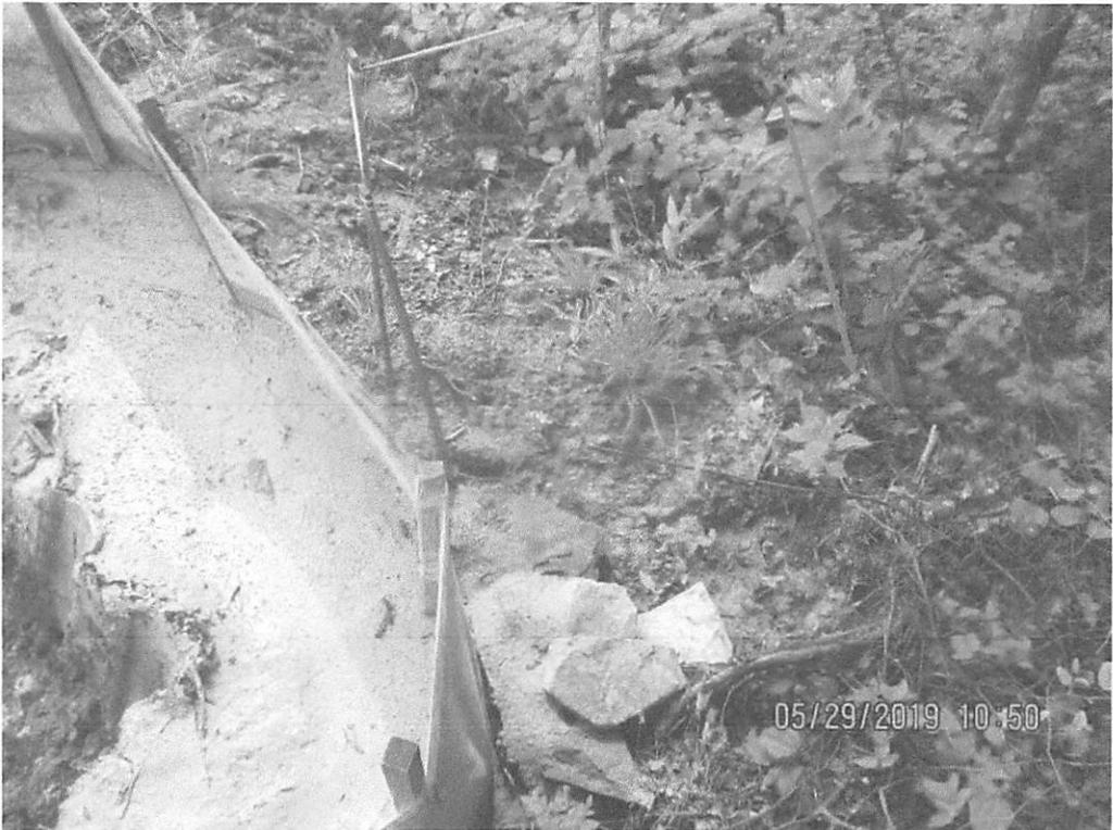
Waterbar outlet above fill slope at station 4031+00 facing downslope. Sediment deposits past LOD.
