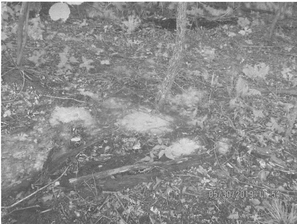
Sediment deposits observed past LOD and controls below waterbar and topsoil pile at station 6508+30.
