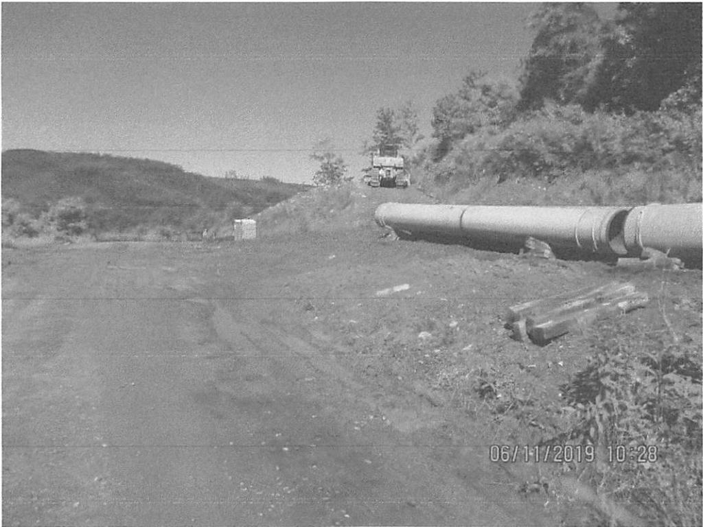
on Krosier road facing east at additional workspace and ROW crossing. Mud and sediment present on road. Run-off flowing toward culvert inlet along Krosier road. Arrow depicts culvert inlet location.
