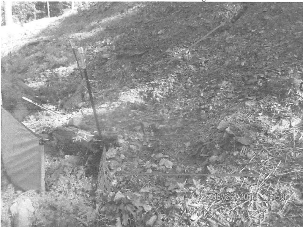
Near Station 1833+00. Erosion occurring on slope leading to sediment deposits being present past the LOD.
