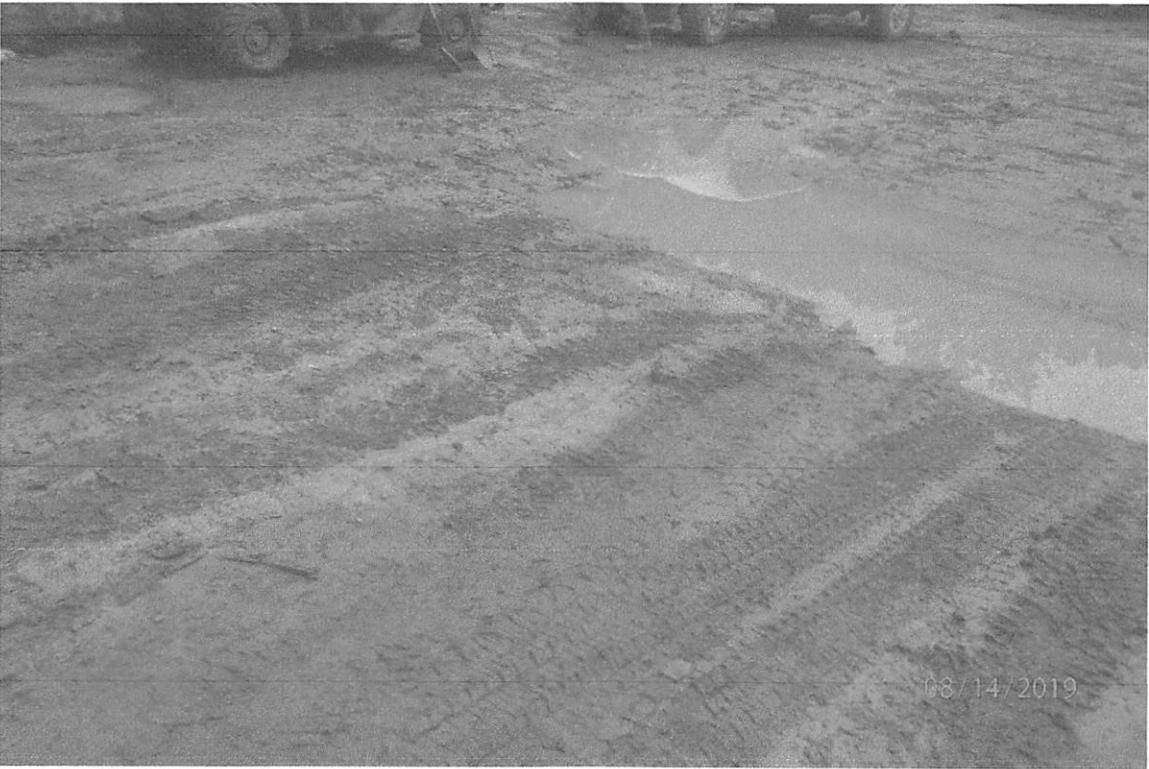
Access road MVP-BR-89.01 showing the need for maintenance to the installed rock construction entrance.
