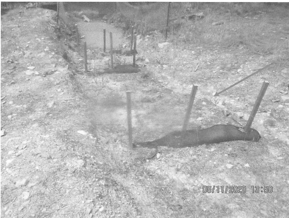
Controls in waterbar on fill slope needed maintenance. Runoff was causing erosion within waterbar and flowing around controls (red arrow).
