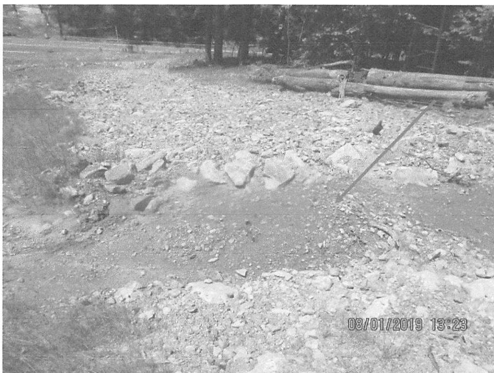
Near station 3831+00. Erosion present in travel lane resulting in waterbar being overwhelmed with sediment and not functioning as designed. Arrow depicts sediment deposited behind Waterbar.
