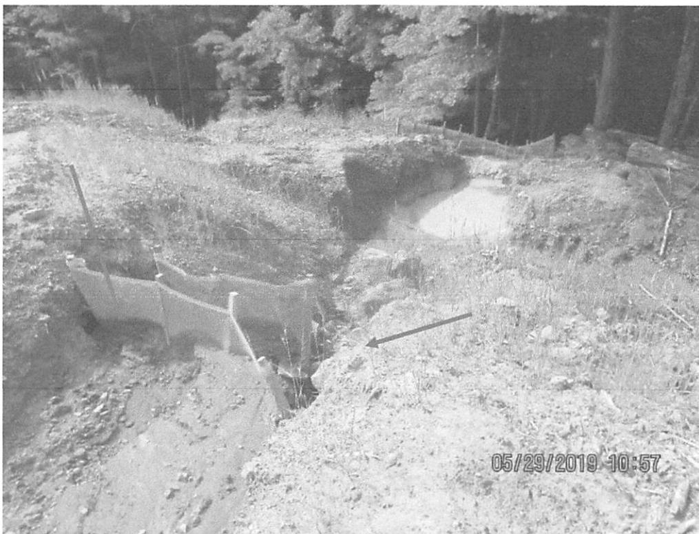
Waterbar outlet and diversion berm outlet at station 4031+00. Sediment was being deposited behind controls. Arrow depicts where runoff was flowing around controls.
