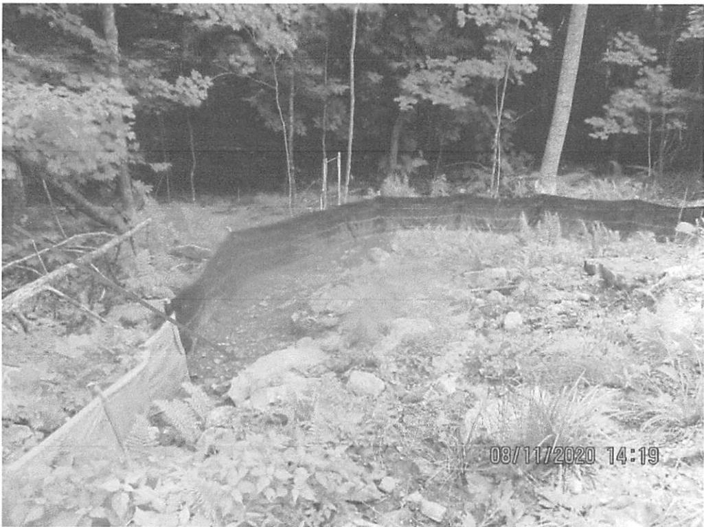
Downslope of the slope drain outlet at Station No. 6490+00. Sediment deposits behind controls due to erosion occurring upslope.
