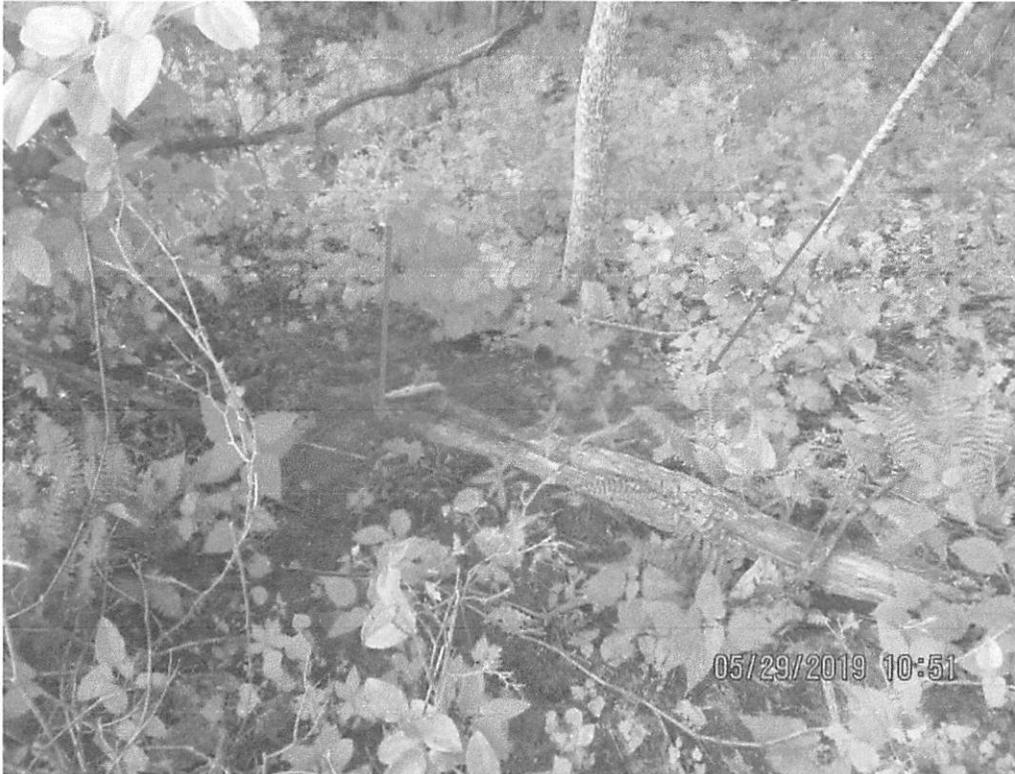
Waterbar outlet above fill slope at station 4031+00 facing downslope. Sediment deposits past LOD. Scouring from concentrated flow.
