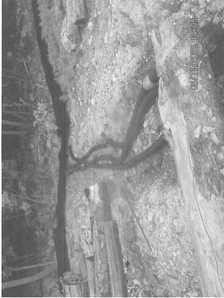
Slope below slope drain install. Erosion present (red arrow) where slope drains were installed and next to the log piles.
