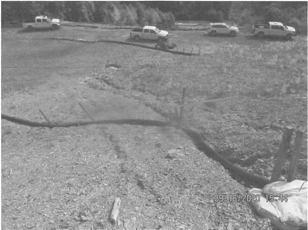
Standing at Station No. 6450+76 at slope drain. Run-off causing erosion on cut slope (red arrow).
