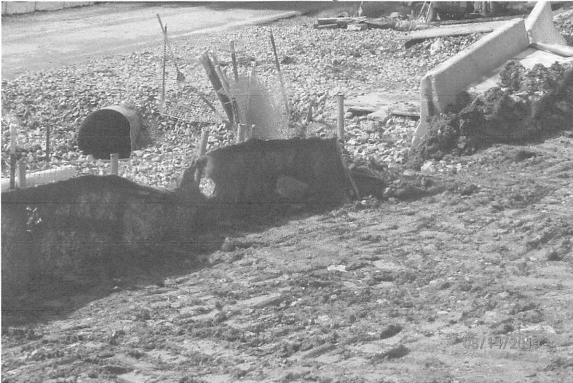
Perimeter controls in need of maintenance in inspected area 3.
