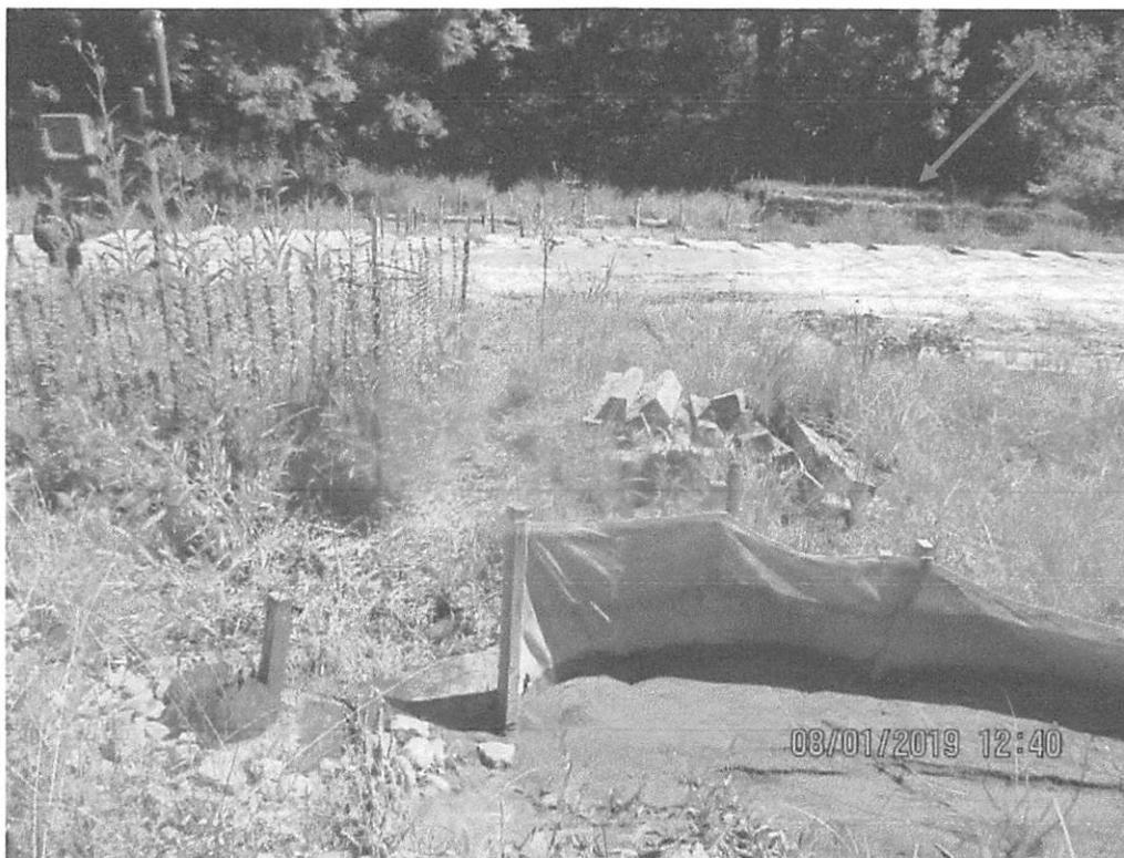
Facing Access Road MVP-BR-097. Controls overwhelmed with sediment due to run-on causing erosion. Controls had not been maintained. Arrow depicts dewatering structure.
