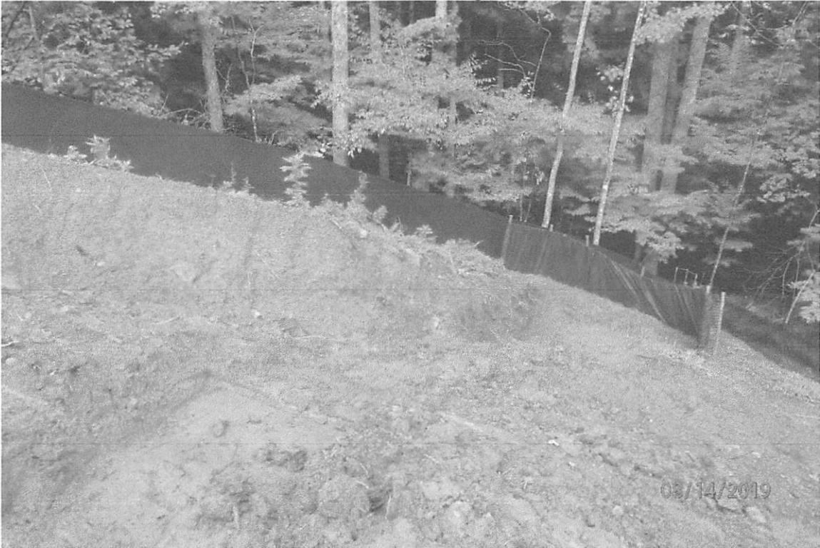
Water bar in inspected area 1 installed at a steep angle and discharging prior to the installed perimeter controls.
