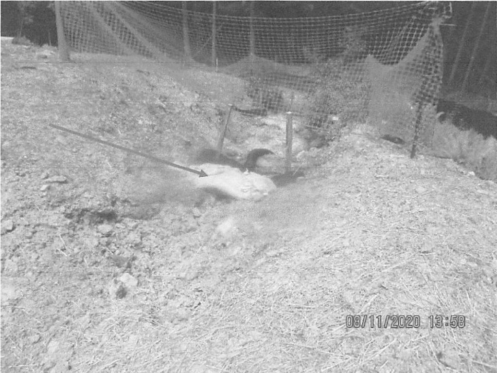
Waterbar outlet terminating onto fill slope. Red arrow depicts recently installed slope drain at top of slope. No sump present at top of slope.
