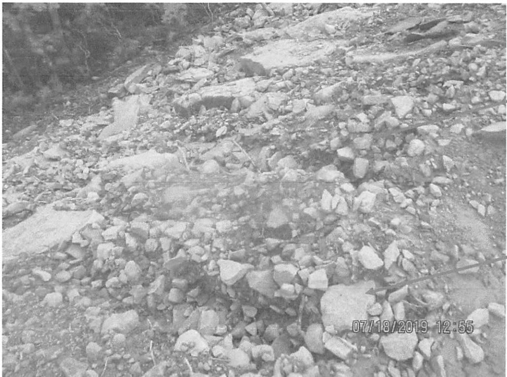
Near station 4559+96, erosion present on fill slope. Arrows depict erosion.
