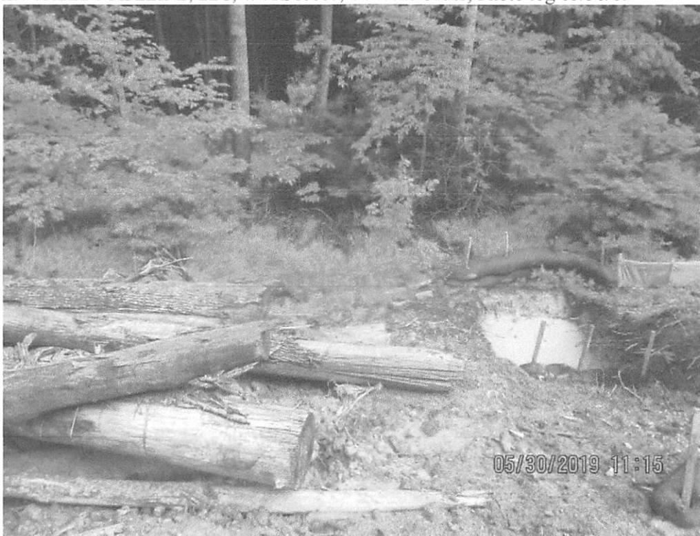
Same area near station 6945+00. Perimeter controls not extended per SWPPP into outlet controls.
