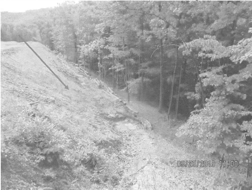
Near station 4031+00 facing downslope at diversion berm Outlet 2. Arrow depicts erosion on fill slope.
