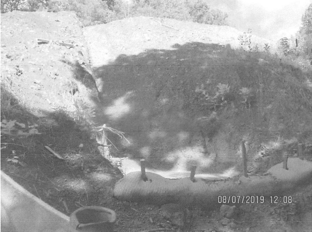
Controls below waterbar termini with no outlet control, terminating onto fill slope and above LOD near station 8951+00.
