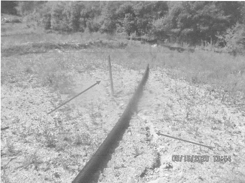
Erosion present on slope below pipe trench drain outlet and slope drain.
