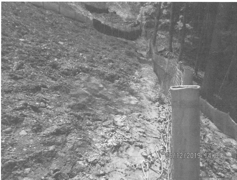
Controls below where dozer work was taking place. Sediment deposits observed below these controls at station 9780+00.
