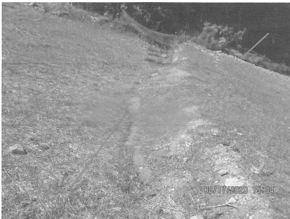
Station No. 6613+00 downslope toward waterbar that failed. 70 percent vegetative coverage not present. Erosion present in waterbar and at outlet (red arrows).
