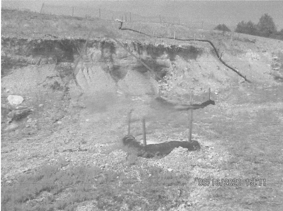
Erosion occurring on cut slope (red arrow) below slope drain outlet at Station No. 6450+76.
