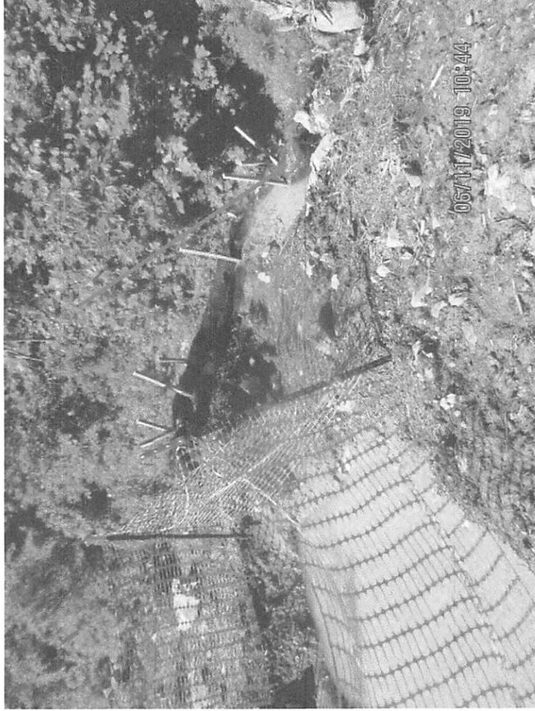
Waterbar outlet near 7604+41. Sump and perimeter controls in need of maintenance. Sediment deposited behind perimeter controls.
