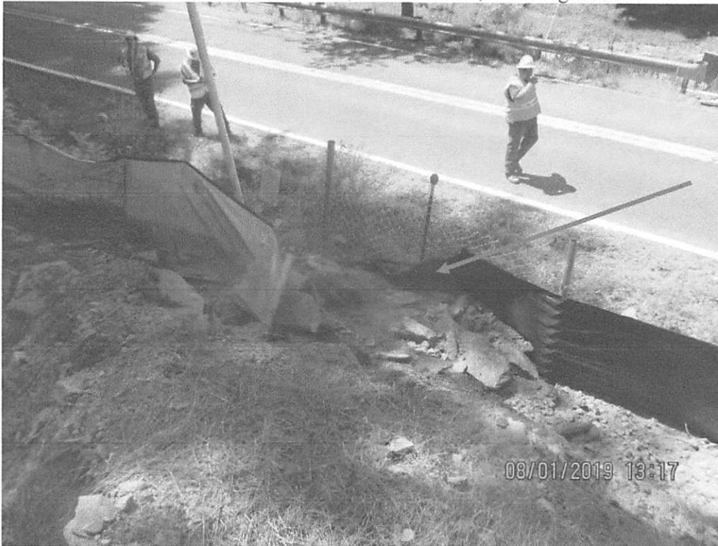
Perimeter controls at base of slope above US 19/Hwy 4 crossing. Controls overwhelmed with sediment, causing control failure above roadside ditch.
