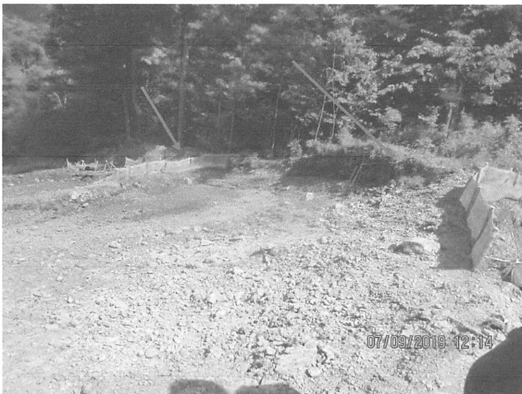
Above Stream S-T35A near station 8634+00 facing toward the East side of the LOD. Arrows depict the original cut to grade ROW that created a wall, preventing proper waterbar outlet installation.
