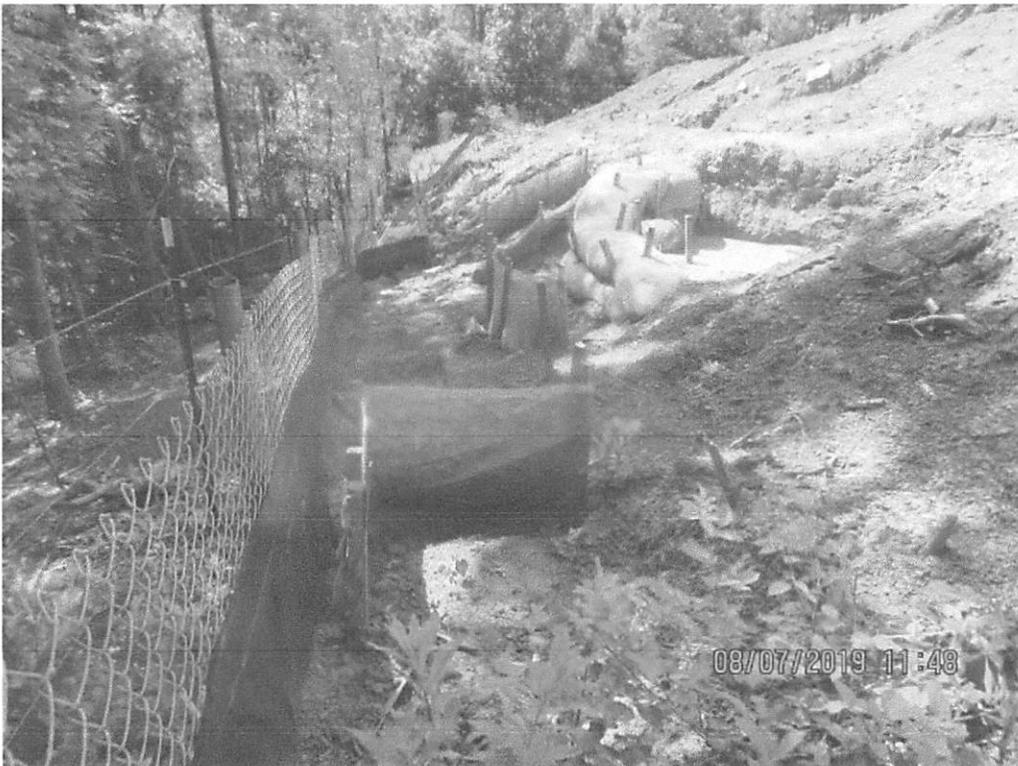
Perimeter controls below dewatering structure at station 8955+00. Arrow depicts where controls were overwhelmed with sediment.
