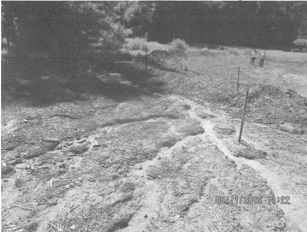
Facing South (Downslope) at station 7609+50. Waterbar receiving sediment due to erosion on slope. Controls overwhelmed with SLW and sediment.
