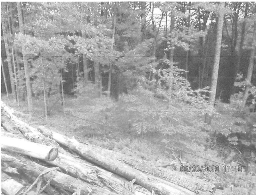
No perimeter control installed per SWPPP on downslope side of fill slope at station 6945+00.
