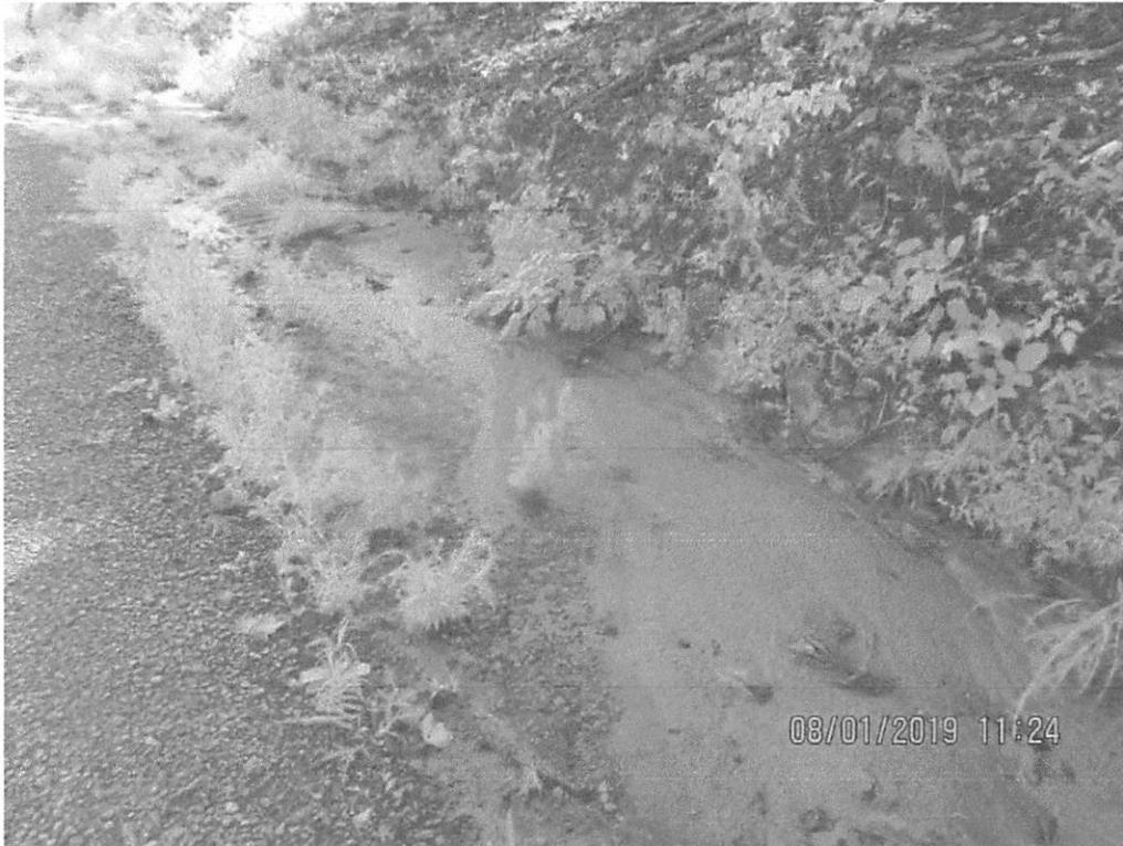
Sediment deposits observed along CR 24 downslope of Access Road MVP-BR-99 near station 3897+75.
