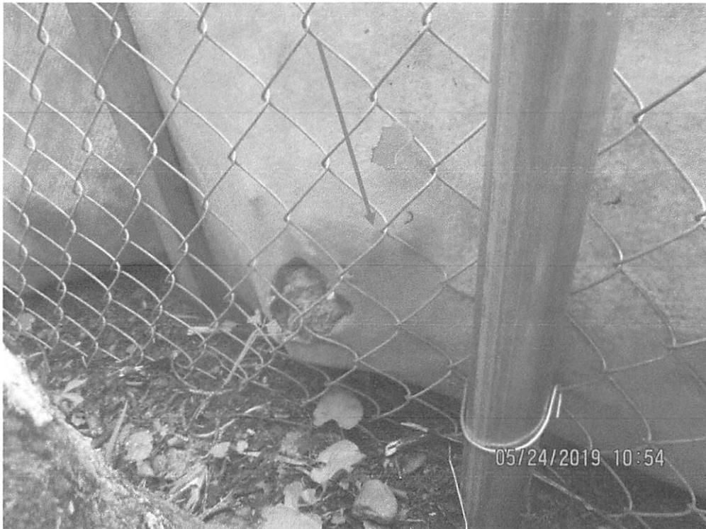
Near station 8410+00. Hole in P1 silt fence due to material slipping into controls.
