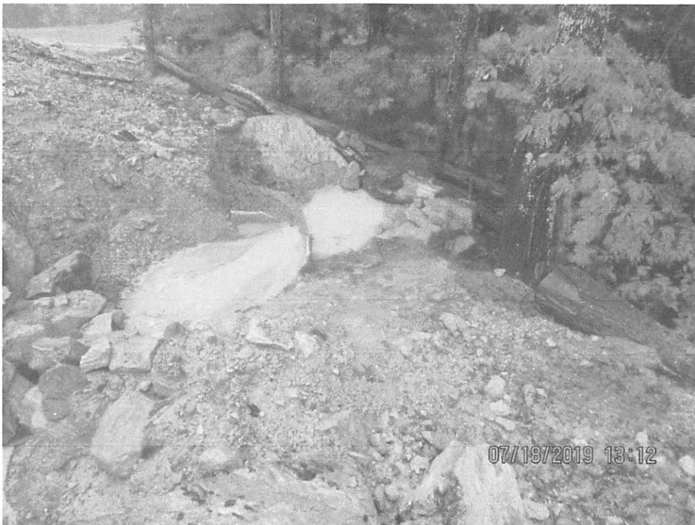
Waterbar terminating onto fill slope at station 4539+00. Large rocks installed as checks in eroded channel. SLW was flowing under and through these checks, overwhelming controls.
