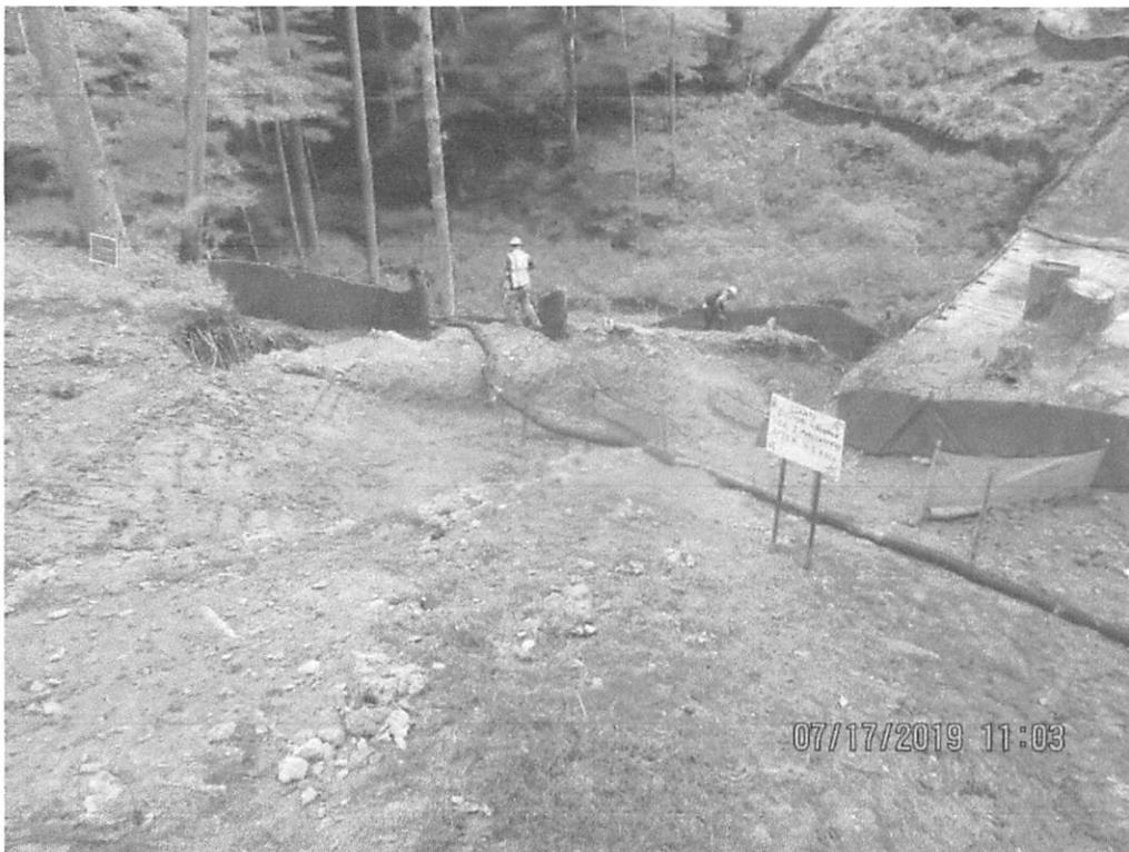
Slope drain conveying across ROW and terminating past LOD and controls. Control failures occurred in this location and impacted stream S-H153.
