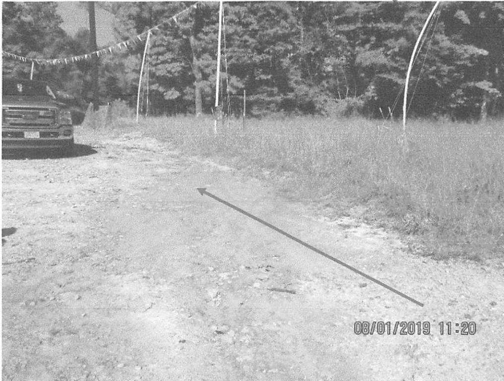
Below diversion berm and facing CR 24 and MVP-BR-099. Arrow depicts direction of sheet flow and sediment transportation downslope toward CR24.
