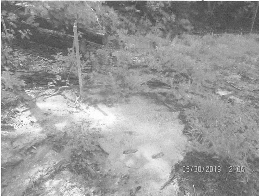
Sediment deposits downslope of waterbar outlet at station 6510+40.
