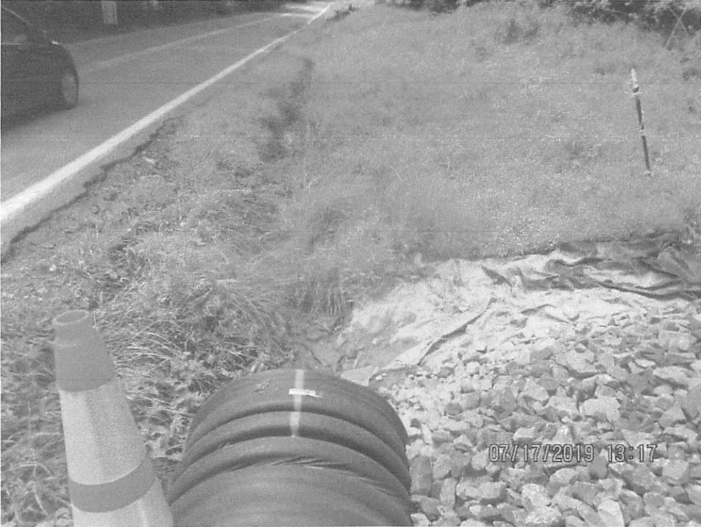
Culvert outlet that conveys under ROW construction entrance. Sediment deposits and SLW present in ditch.
