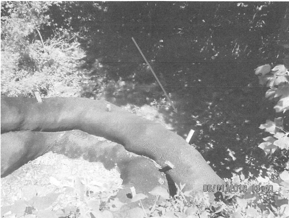
Controls below culvert outlet and bridge crossing with AR-182.5. Sediment deposits and SLW observed past these controls and LOD. Arrow depicts deposits.
