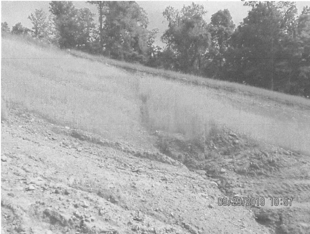
Facing toward cut in slope/ROW at station 4031+00. Waterbar had erosion.
