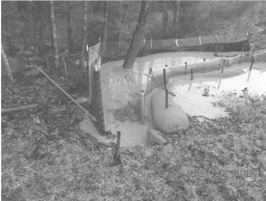
Controls downstream of culvert. SLW going around controls.
