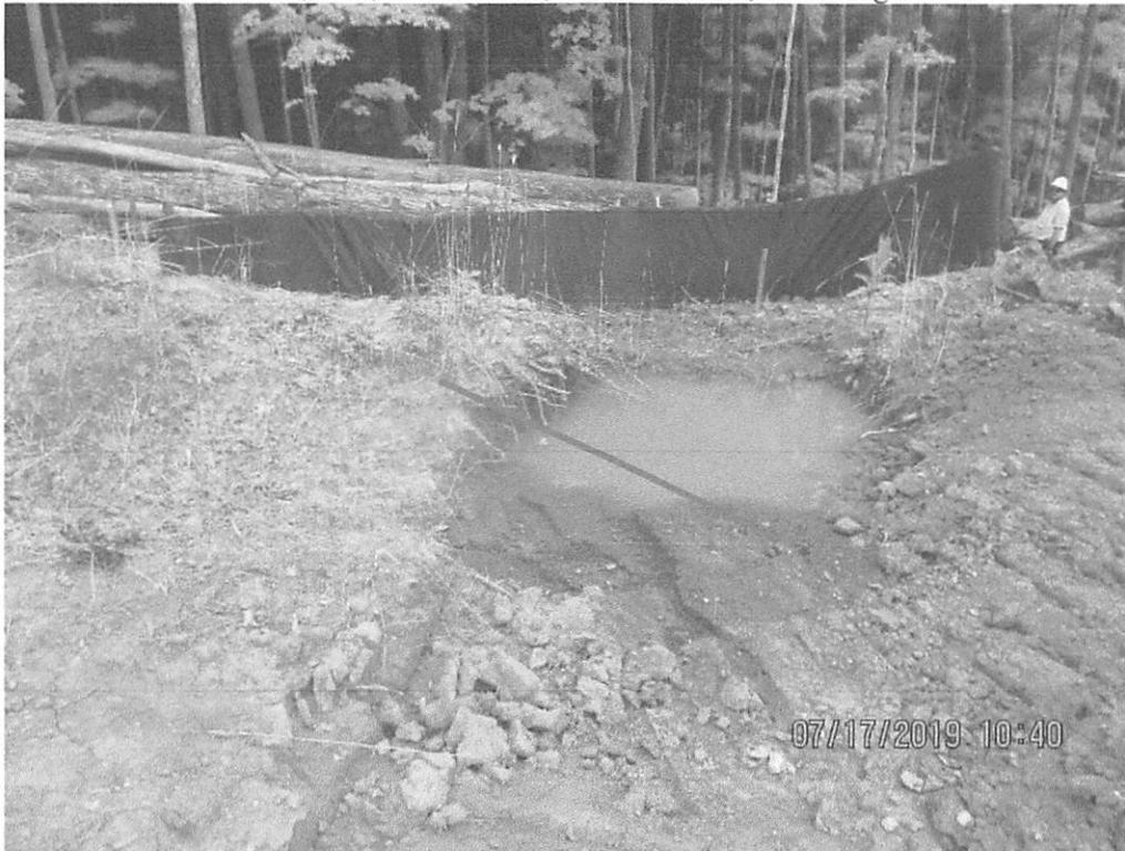
Sump at waterbar terminus near station 3151+47. Sediment deposits present past LOD due to lack of sump maintenance. Sump becoming overwhelmed with sediment.
