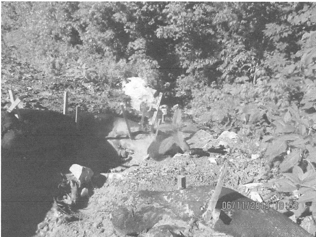
Above Station 7604+41. Perimeter controls overwhelmed with sediment. Sediment deposits present past LOD.
