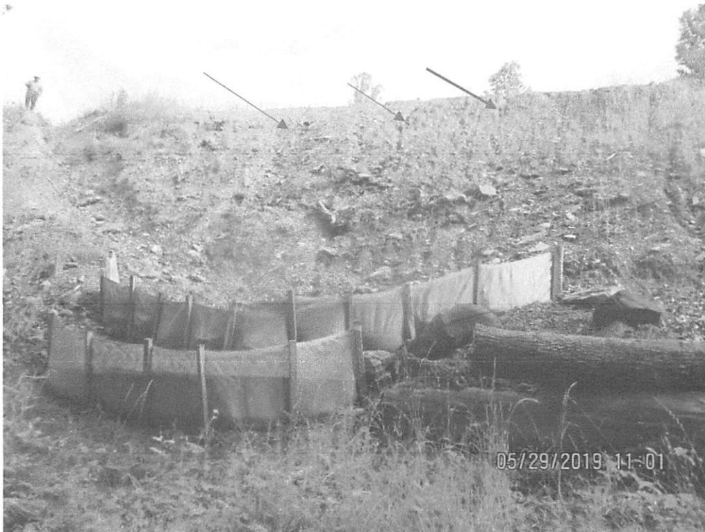
Facing upslope near station 4031+00 at diversion berm Outlet 2. Waterbar was terminating onto slope with no controls. Arrow depicts erosion on slope.
