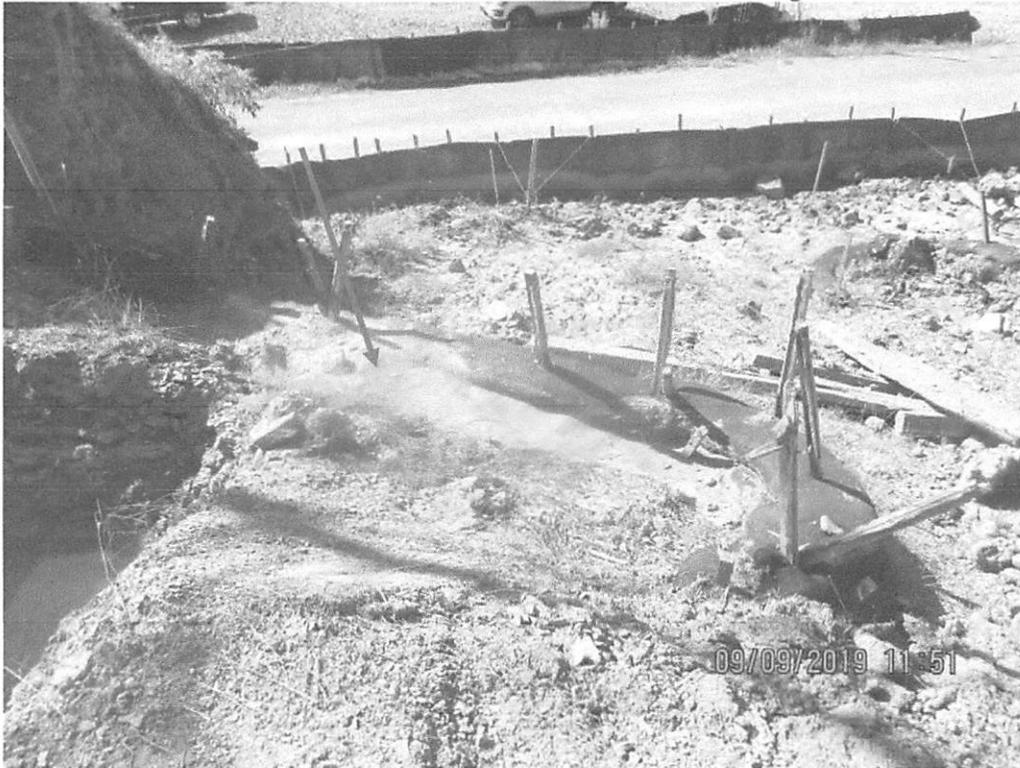
Controls upslope of CR21 and roadside ditch. Arrow depicts where sediment was overwhelming waterbar outlet controls.
