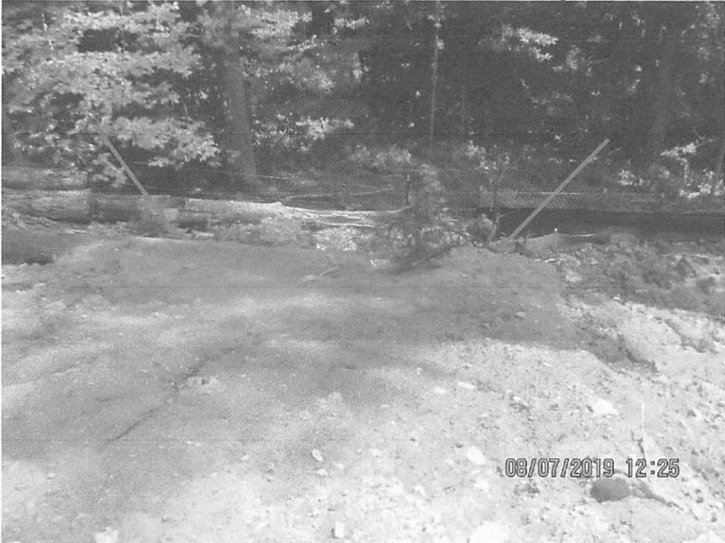
Fill slope near station 8946+00. Erosion present on fill slope resulting in sediment overwhelming perimeter controls. Arrows depict overwhelmed controls.
