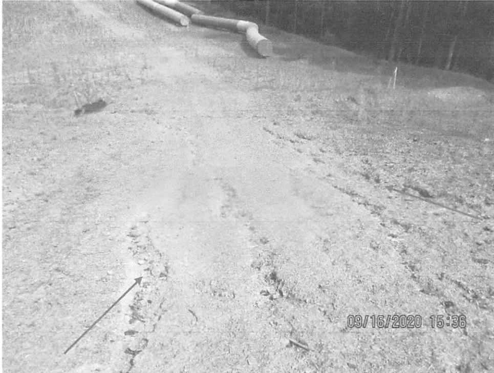
Erosion on slope between waterbars near station No. 6450+76 (red arrows). Area had not been reseeded.
