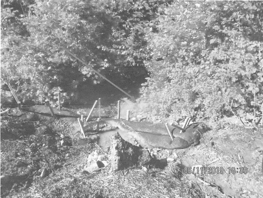
at station 7576+01 downslope of waterbar with sediment deposits due to run-on from seep. Controls overwhelmed with sediment. Erosion on slope, SLW, and deposits observed past LOD and controls.
