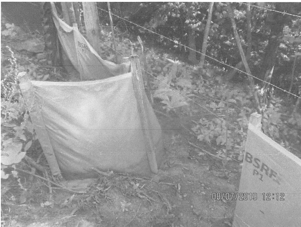
Further downslope near station 8951+00. Perimeter Controls below waterbar termini with no outlet control terminating onto fill slope and above LOD. Sediment deposits observed past the LOD.
