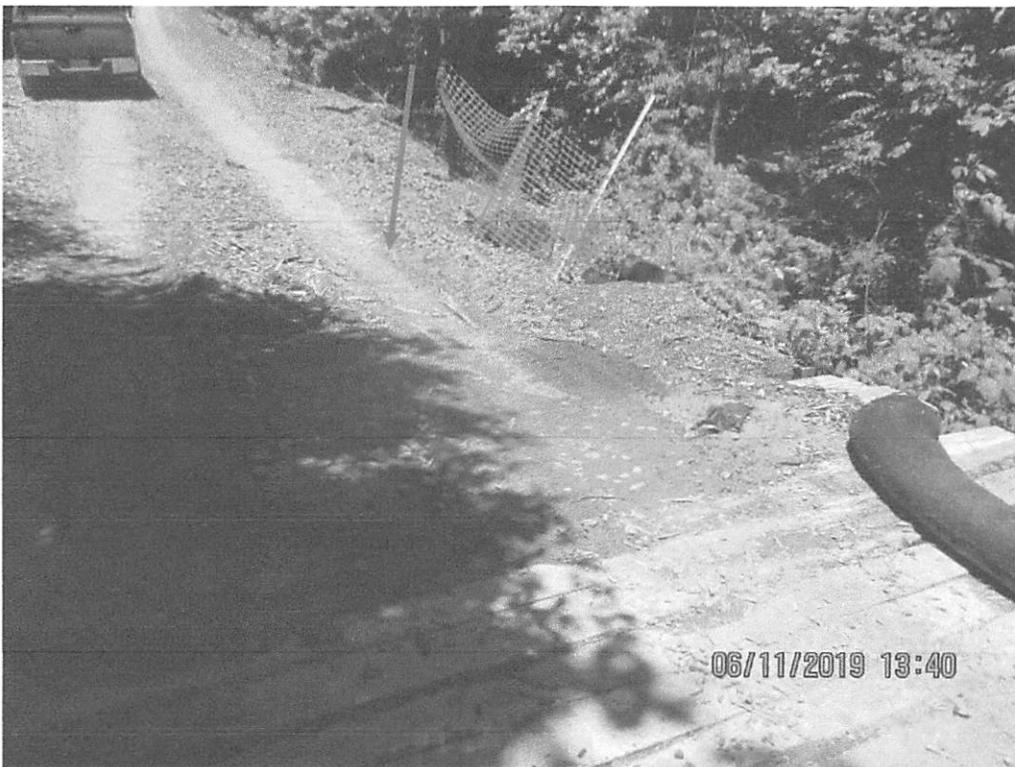
Facing up grade on Access Road 192.5 at wetland crossing W-V6. SWPPP detailed waterbar above this crossing. waterbar had been eroded and was barely distinguishable. Arrow depicts where waterbar was installed and terminated on road bank (slope).
