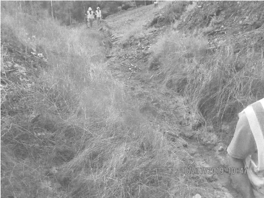
Waterbar with erosion at station 3149+00.
