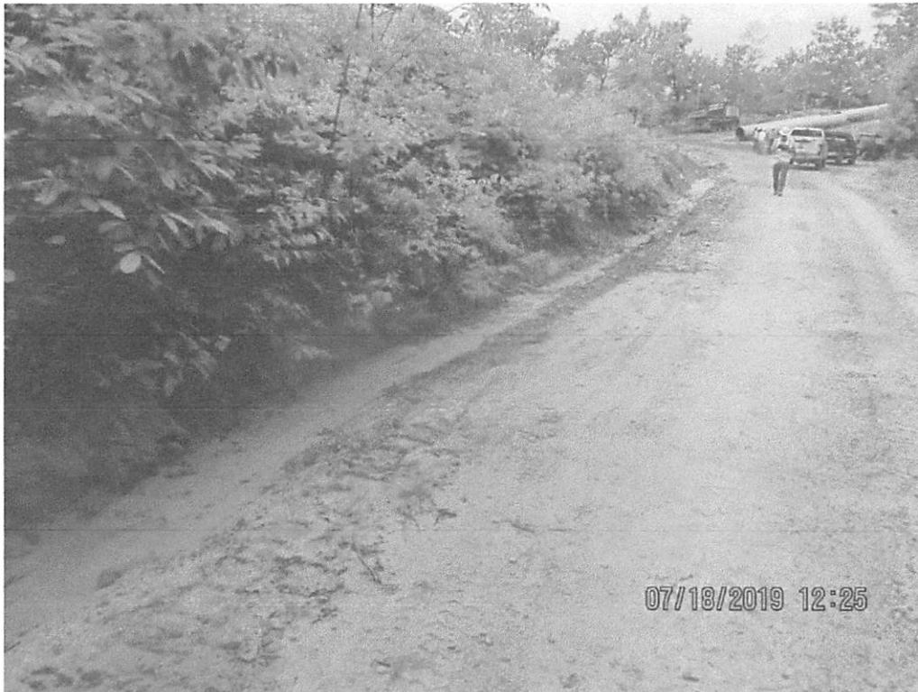
Downslope from station 4559+96 from Access Road MVP-WB-119 facing toward MVP ROW. Sediment deposits present in roadside ditch.
