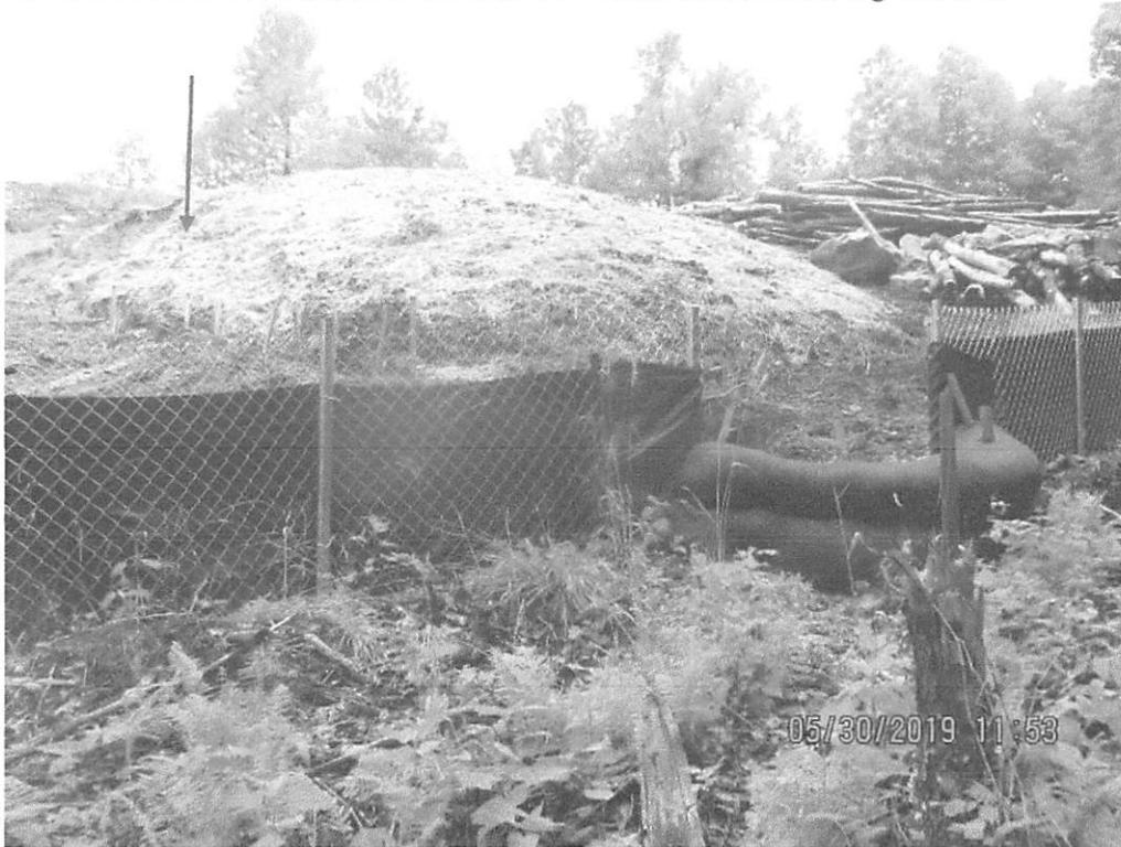
Facing upslope at waterbar and topsoil pile at station 6508+30. Arrow depicts topsoil pile that is slipping into waterbar.
