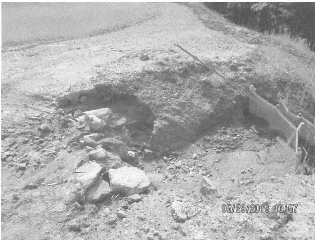
Waterbar outlet at station 4031+00. Arrow depicts where runoff was flowing around control and causing increased erosion.
