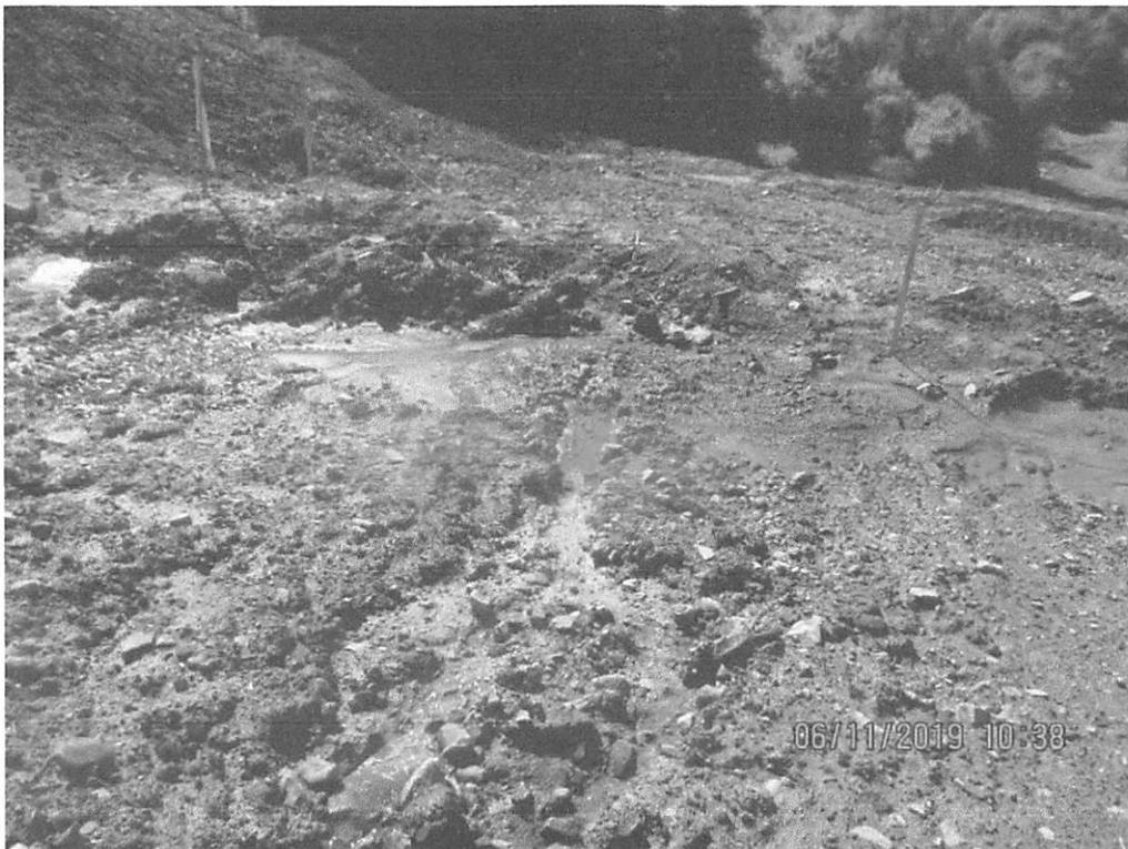
Below upper Krosier Road crossing near station 7576+01 facing South at waterbar. Erosion present on slope due to seep running onto ROW. Sediment deposited in waterbar.
