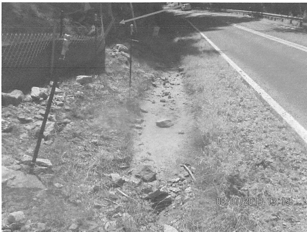
Sediment present in ditch that parallels US 19/Hwy 4 due to control failure. Arrow depicts control failure at base of slope.
