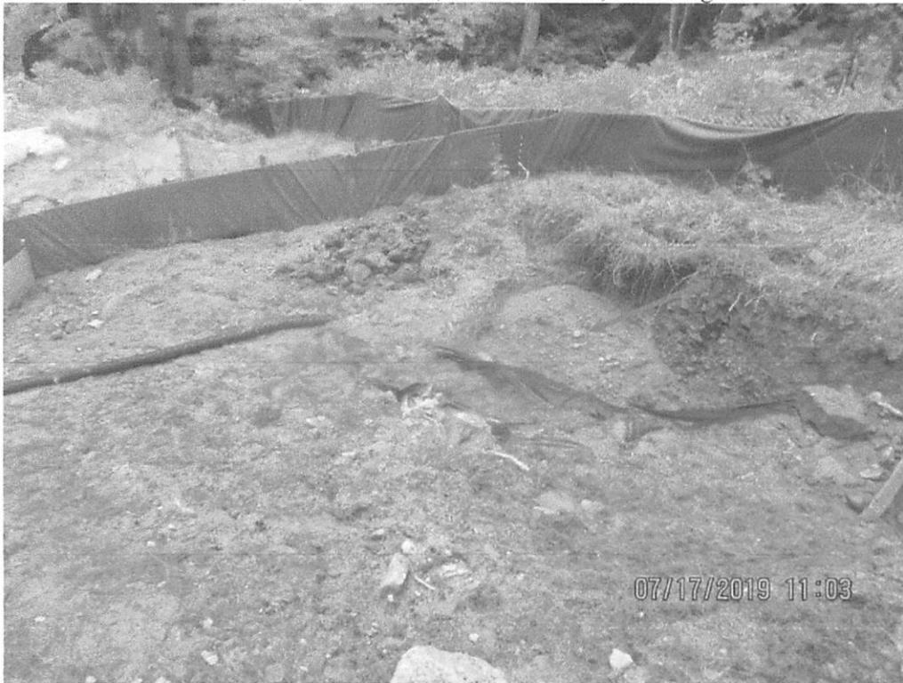
Sump at base of slope where diversion berm terminates above Stream S-H153. Slope drain installed in sump overwhelmed with sediment which was conveyed past the LOD. Arrow depicts slope drain inlet approximate location.
