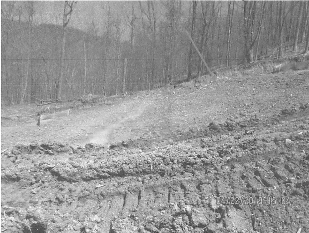
Facing toward cut slope and where waterbars terminated onto ROW. Arrow depicts where waterbars were terminating into cut slope at Station 8633+71.
