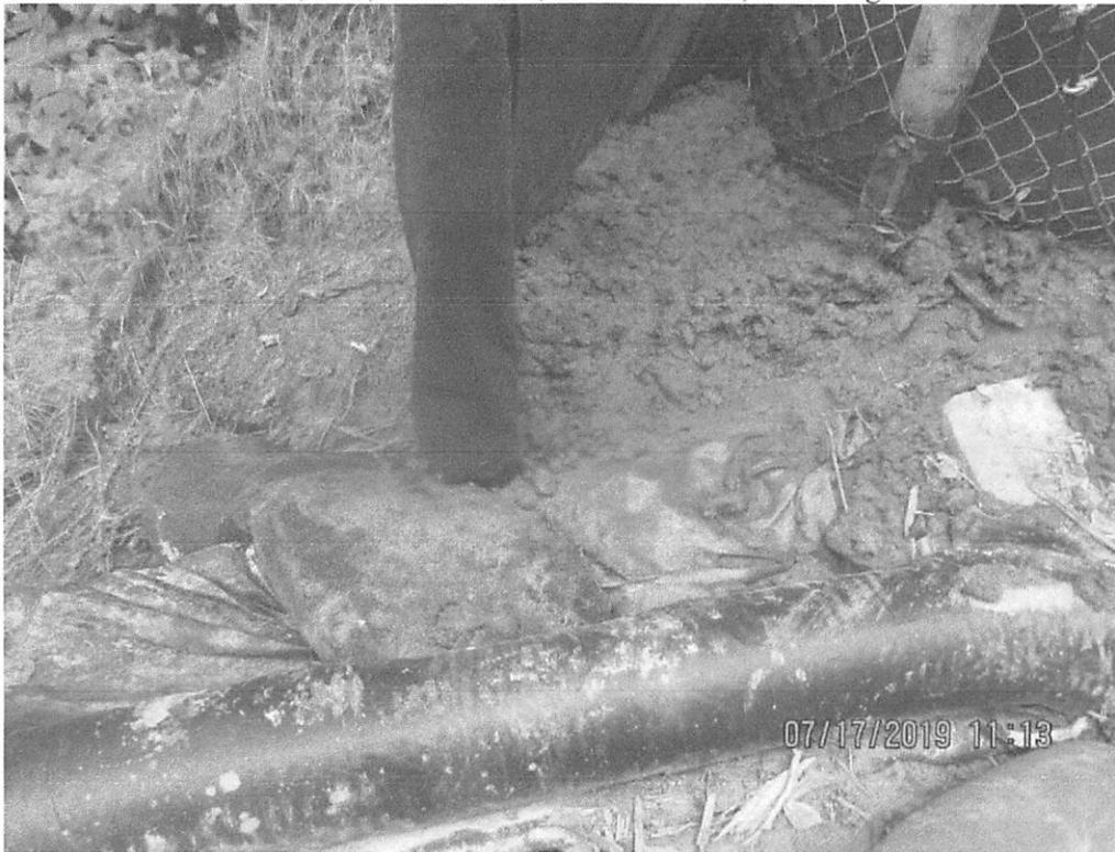
Controls at bridge that crosses Stream S-H153. Controls were overwhelmed with sediment.
