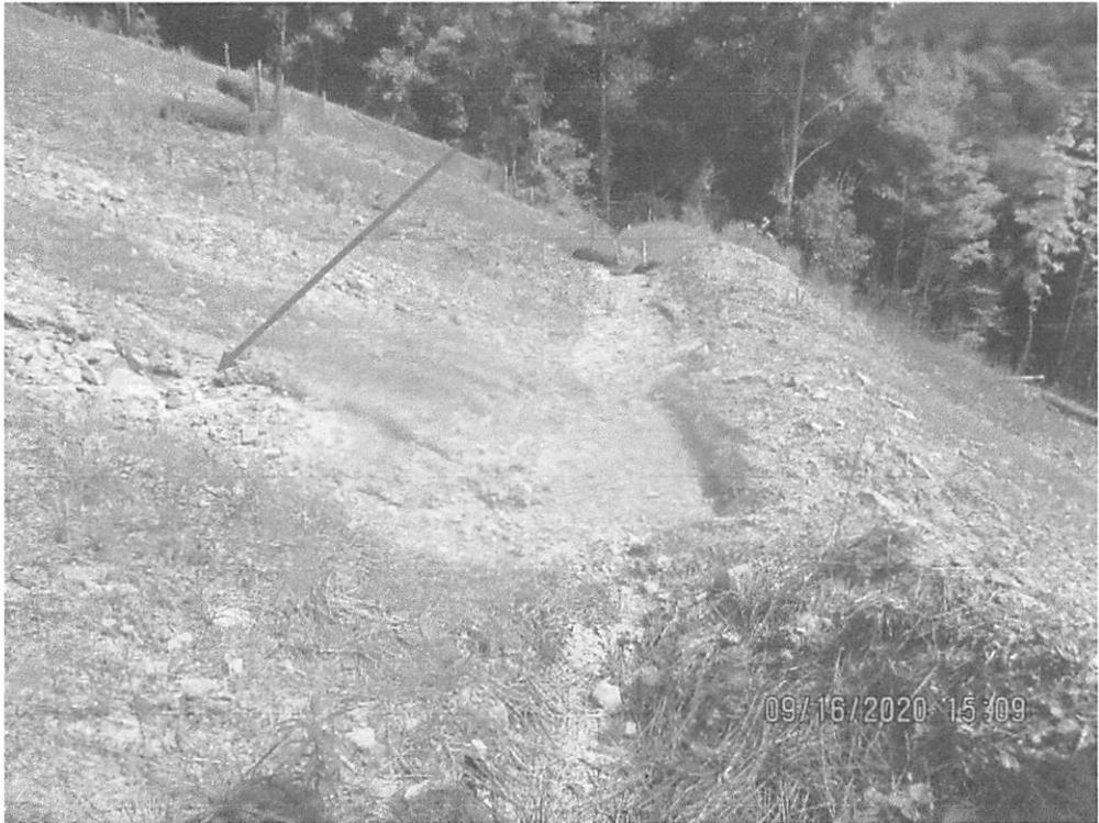
Standing downslope from Access Road 159.01 facing east near station No. 6657+00. Erosion present on slope, depositing sediment into waterbar and controls (red arrow).
