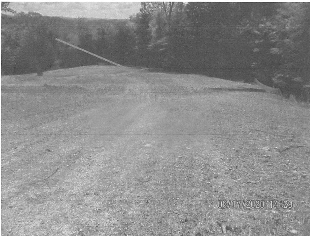
Facing downslope (South) near Station No. 6617+00. Less than 70 percent vegetative coverage. Erosion present in waterbar.
