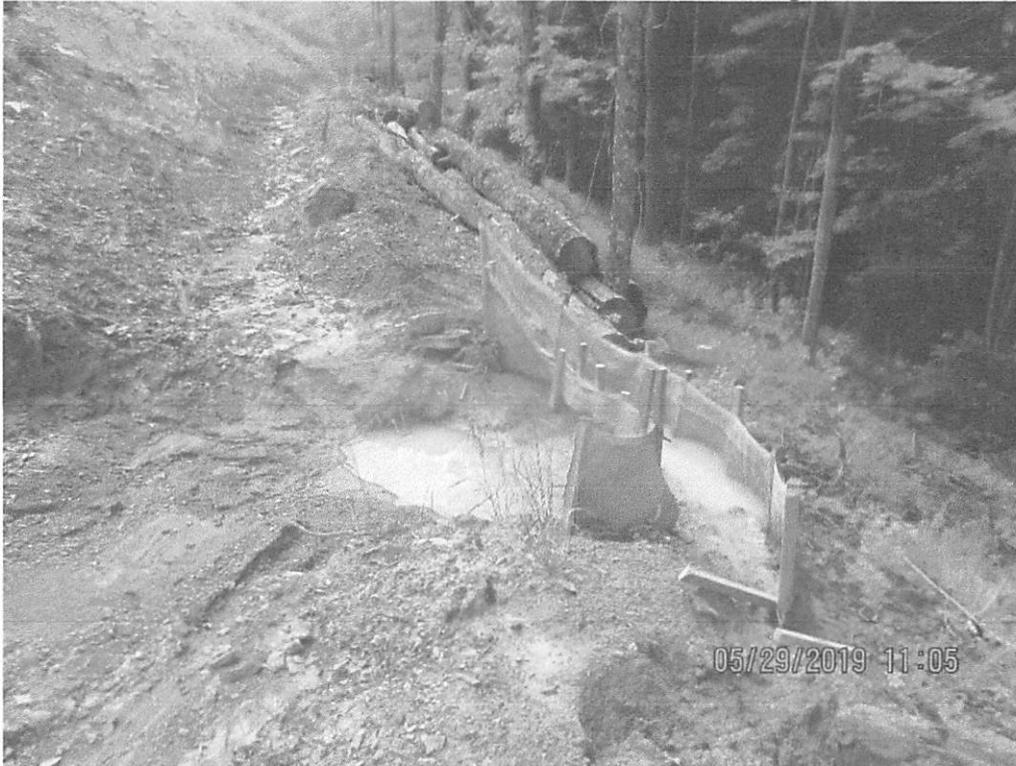
Diversion berm Outlet 3. Sediment being deposited behind controls.
