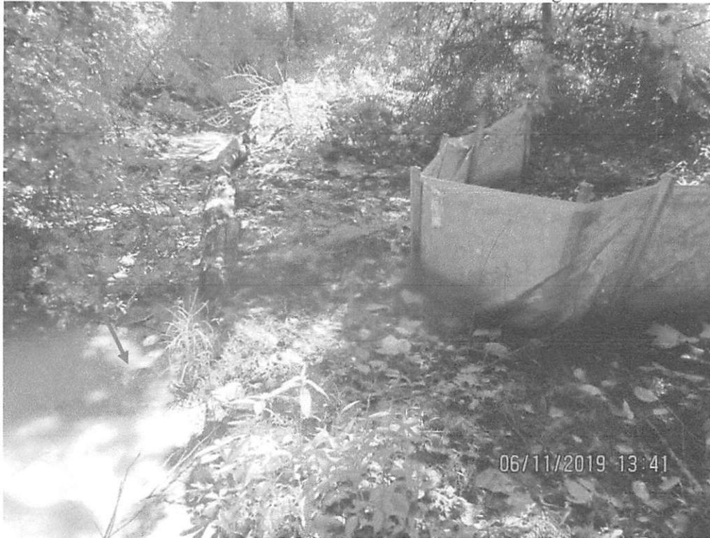
Further downslope of culvert outlet and bridge crossing with AR-182.5, below second culvert outlet where P1 silt fence was installed. Sediment deposits and SLW present past LOD. Arrows depict outlet controls and where SLW and deposits were observed.
