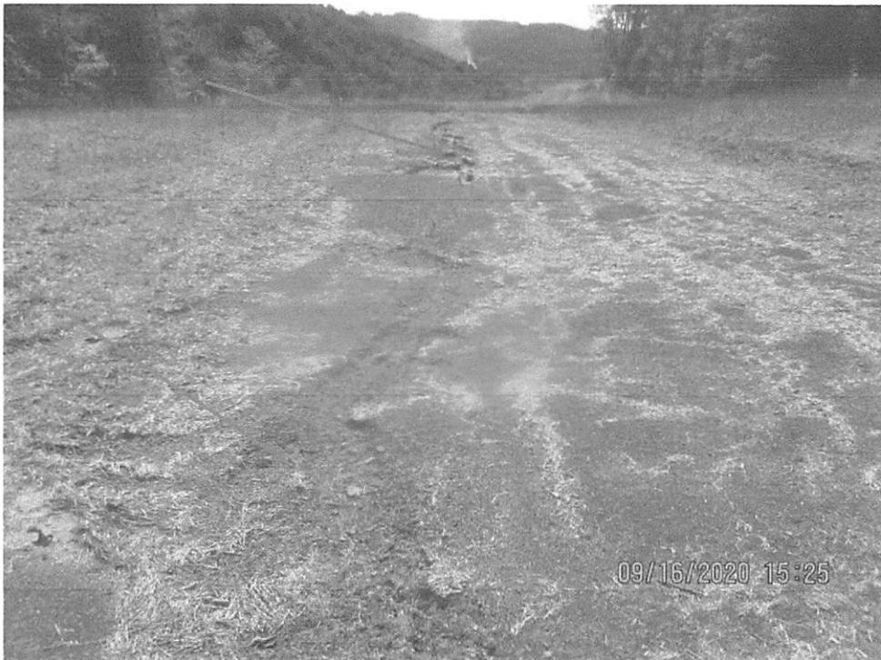
Section of ROW upslope from 6450+76 that was not reseeded since Fall 2019. Red arrow shows erosion occurring due to increased sheet flow.
