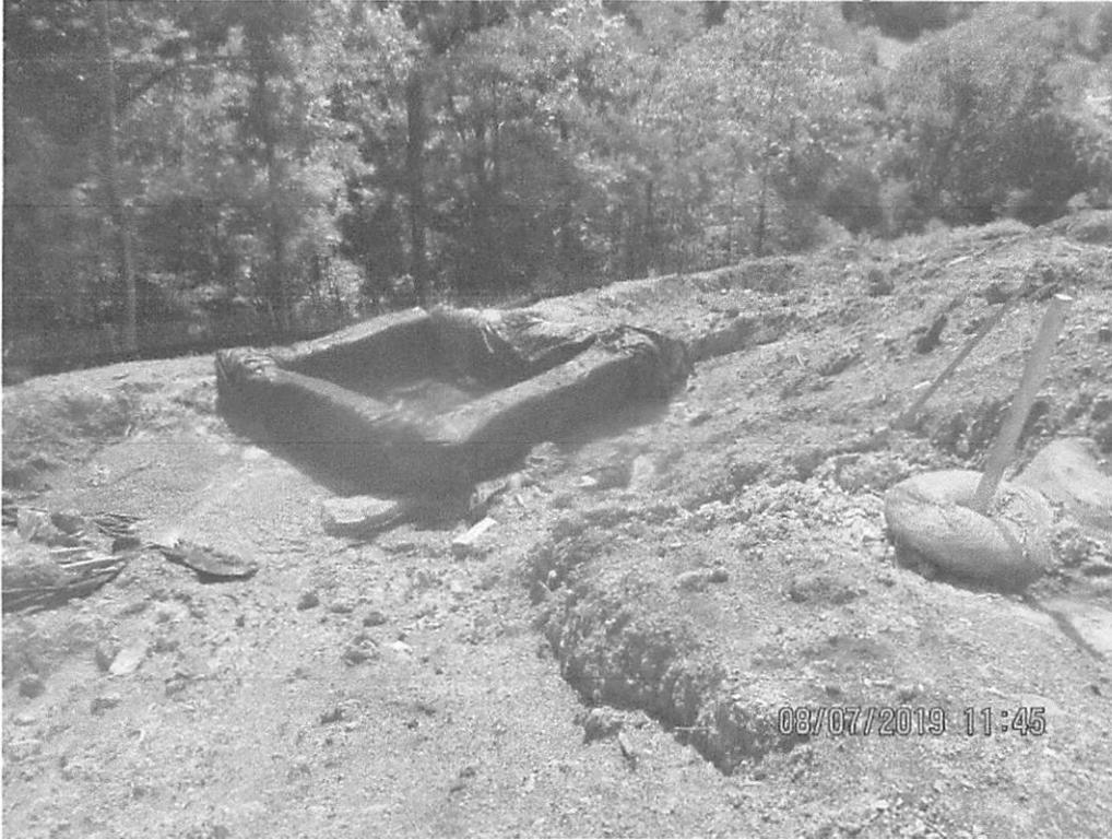
Dewatering structure present on slope and below waterbar terminus near station 8955+00. Erosion present on slope.
