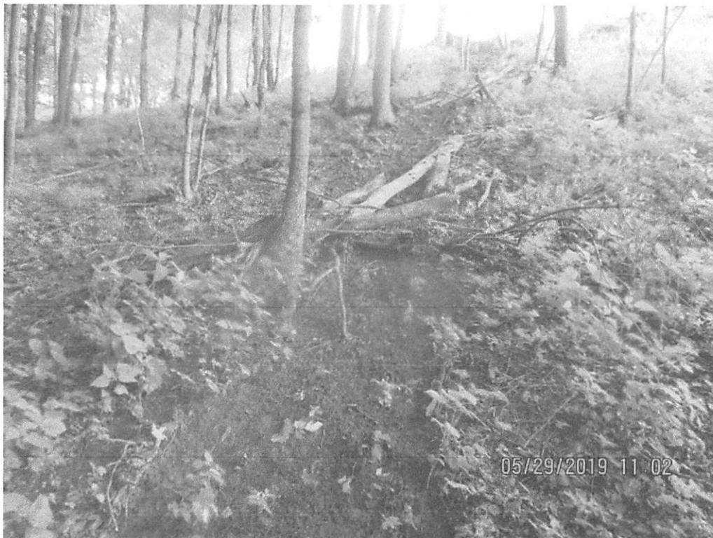
further downslope below diversion berm Outlet 2 near 4031+00. Scouring of vegetation below control.
