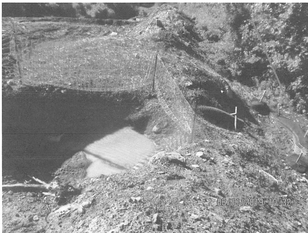
Downslope of Krosier Road Crossing near station 7576+01. Waterbar outlet perimeter controls in need of maintenance. SLW and deposits were present past controls and LOD. Arrow depicts sediment backed up behind controls causing SLW to overtop the control.
