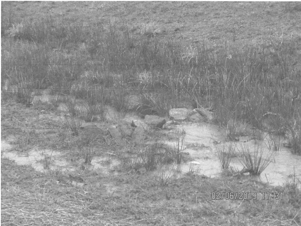
Rock check in ditch with SLW present, draining toward culvert.
