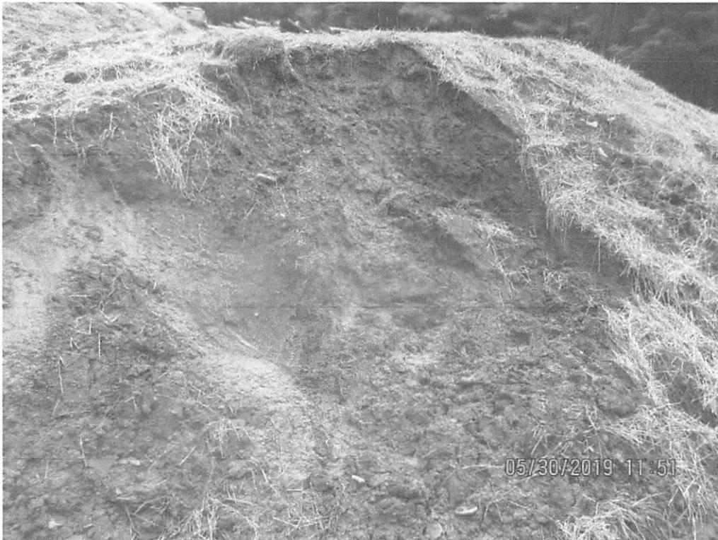
Topsoil pile slipping into waterbar at station 6508+40.
