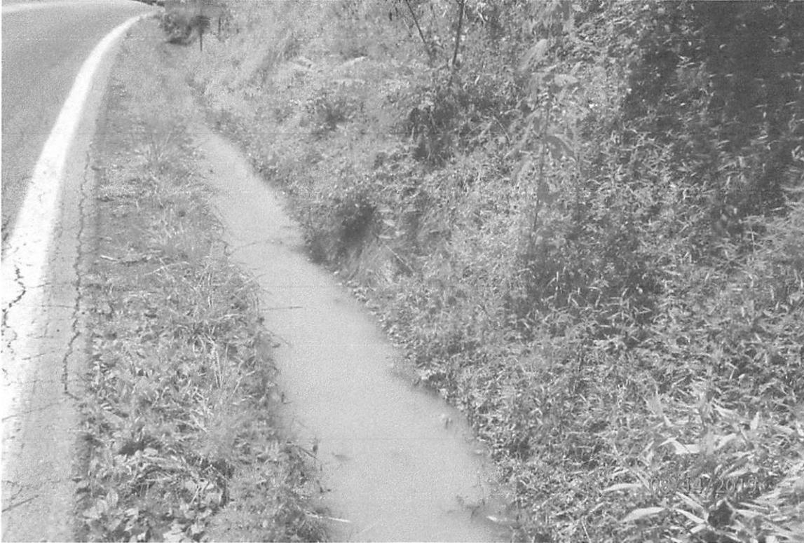
Offsite sediment-laden water in DOH conveyance that leads from the previously pictured dewatering operation with the unmaintained perimeter control.
