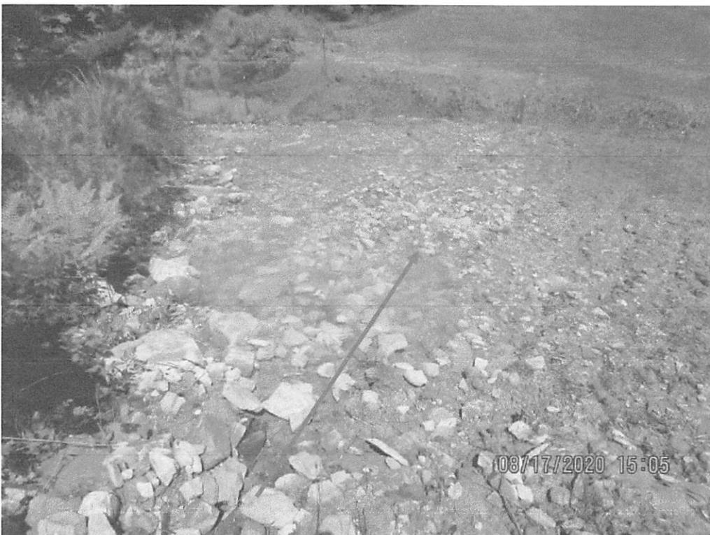
Facing downslope at the fill slope where the waterbar failed and was causing erosion at Station No. 6613+00.
