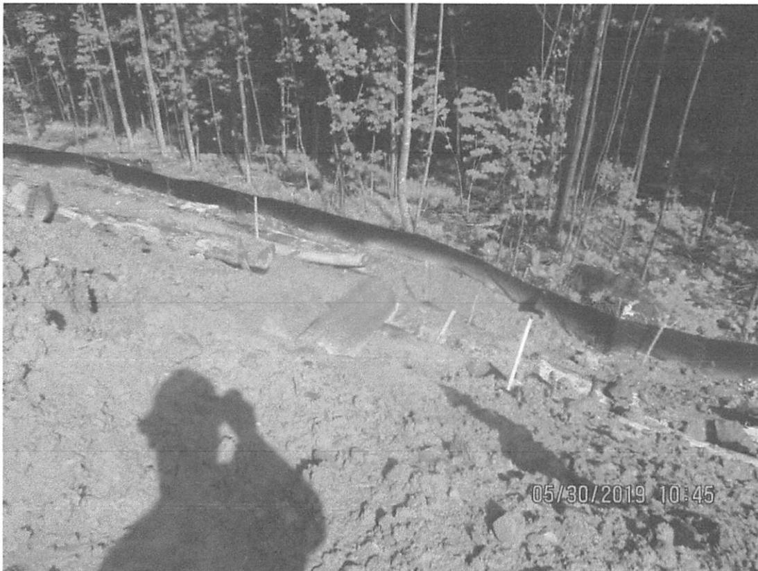
Pipe outlet below seep. Diversion not stabilized and no rip rap apron installed as required per SWPPP near station 6485+10. The inlet had been cut due to trench being dug.
