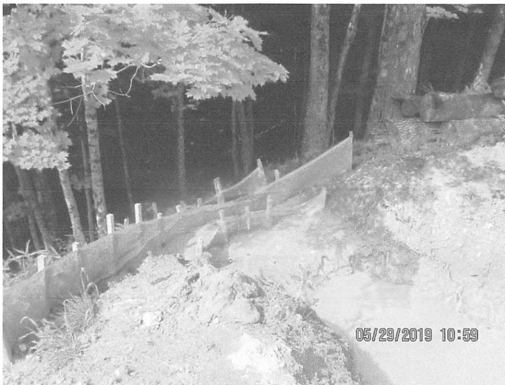
Diversion berm Outlet 1 at station 4031+00. Controls in need of maintenance.
