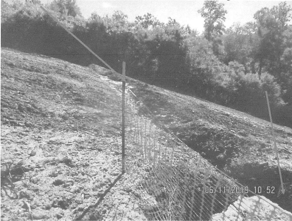
Above Station 7604+41. Waterbar with sediment deposits due to erosion upslope. Sump was full of sediment and needed maintained. Arrow depicts sediment in waterbar and sump.
