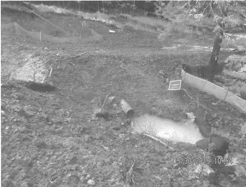
Drain outlet above Stream S-EE1. Clean water diversion not stabilized above or below inlet/outlet. Clean water was being conveyed approximately 15 ft across disturbed soil to a sump where the inlet was located. The topsoil pile around the inlet was eroding into the sump. Arrow depicts inlet.
