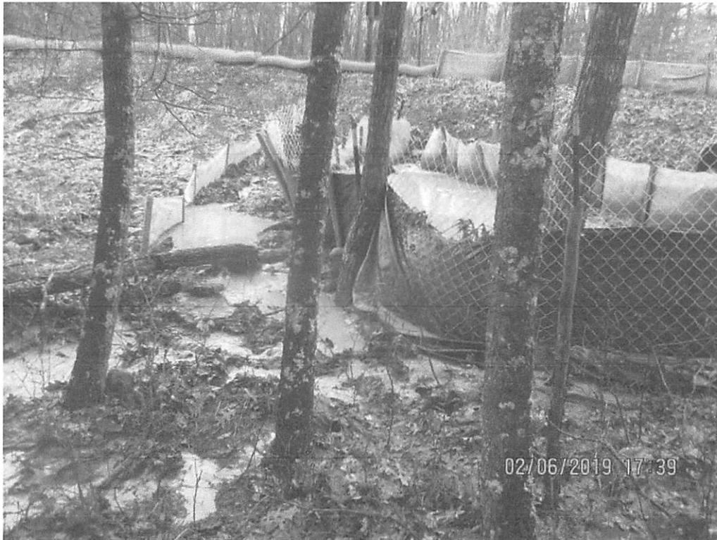
SLW flowing past controls and downslope to UNT of Brammer Branch. Back side of silt fence fallen over.
