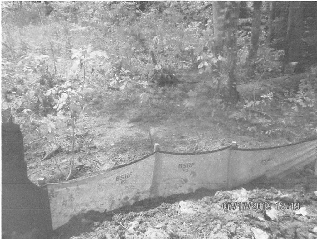
Controls below culvert outlets at station 3192+50. Sediment had been removed from behind controls and new controls had been installed. Sediment-laden water had left the site.
