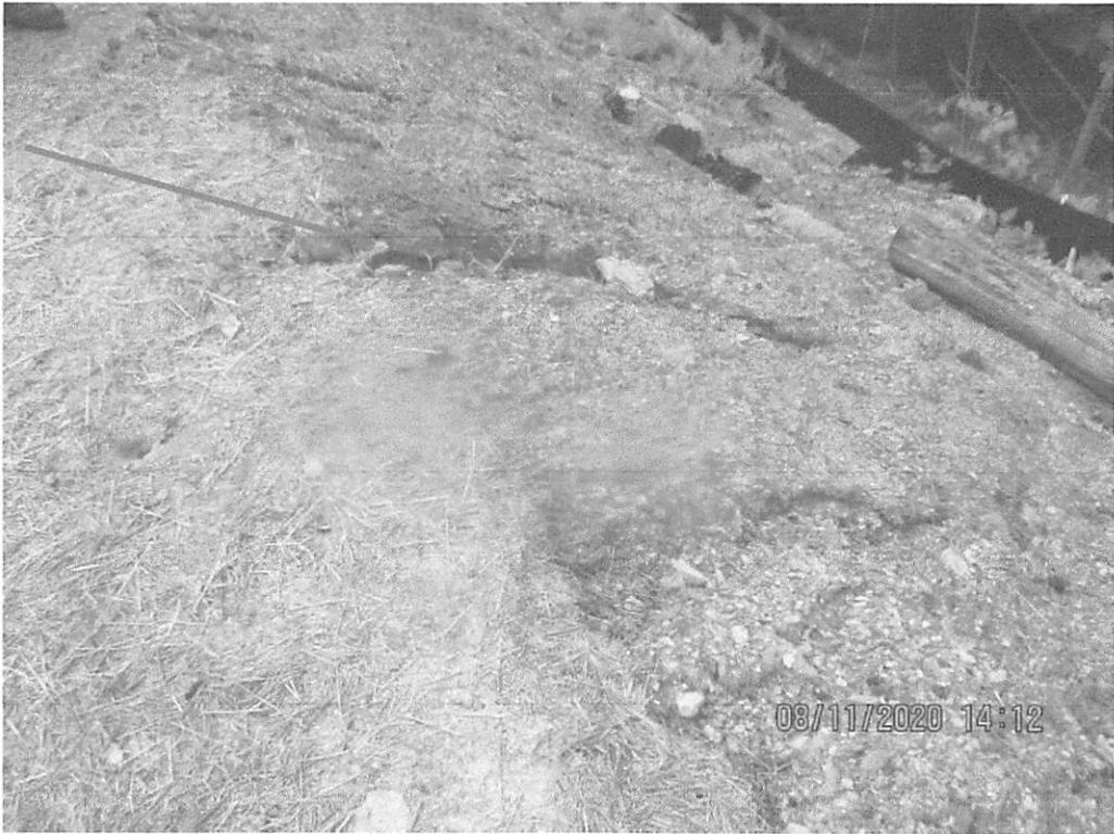
Fill slope erosion above log piles near Station No. 6485+50.
