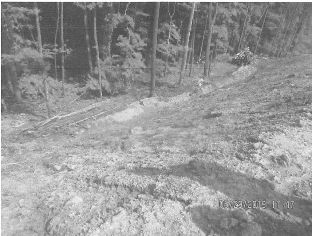
Erosion present on slope near Station 4017+00. Perimeter controls overwhelmed with sediment.
