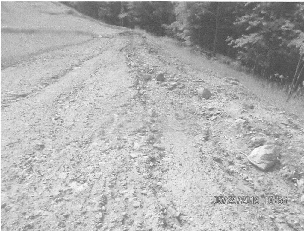
Near station 4031+00 facing downslope. Erosion on ROW where grass had not germinated in travel lane.
