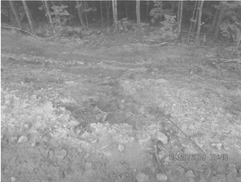
near station 4027+00 facing downslope. Erosion present on fill slope. Perimeter control being overwhelmed with sediment, resulting in sediment-laden water being present past controls. According to representative, logging disturbance had taken place.
