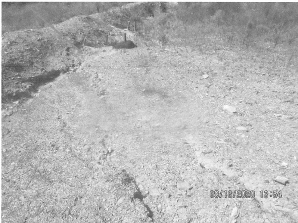
Facing downslope near station No. 6698+00. Erosion occurring between waterbars on slope and in waterbars. Controls lacking maintenance within waterbar (red arrow).
