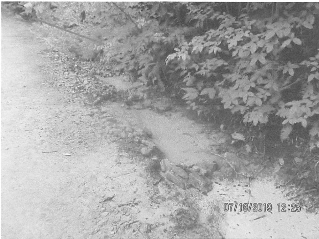
Downslope of station 4559+96 on Access Road MVP-WB-119. Sediment deposits present in roadside ditch and conveying to culvert inlet. Arrow depicts approximate location of culvert inlet.
