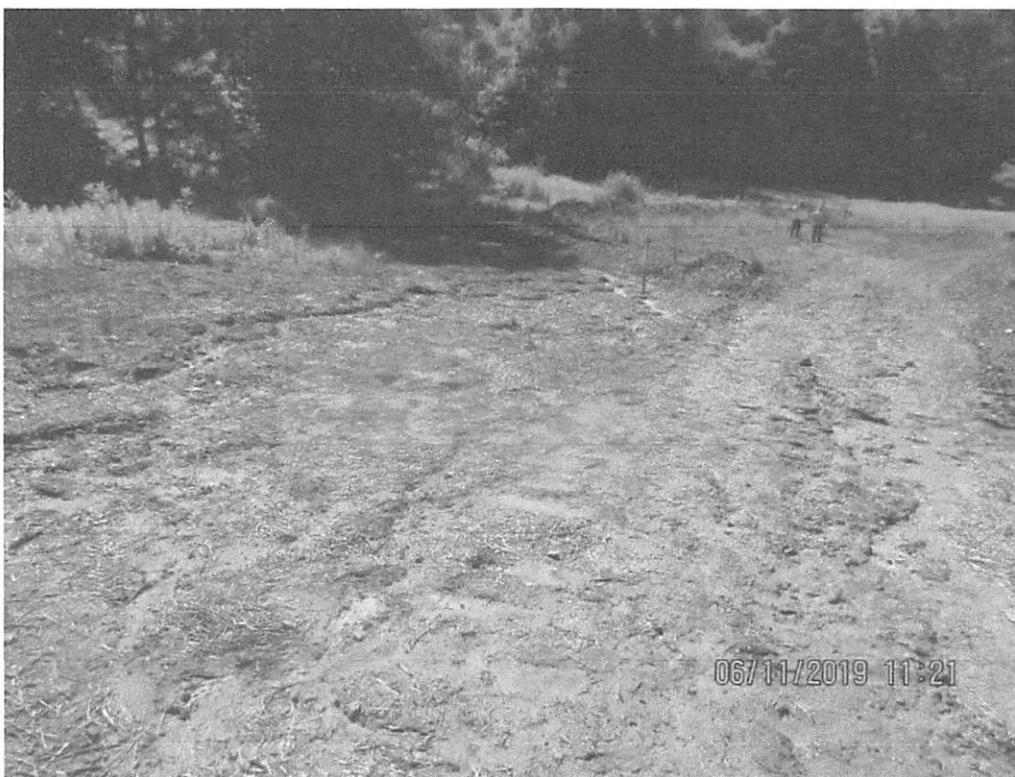
Facing South (Downslope) at station 7609+50. Waterbar receiving sediment due to erosion on slope.
