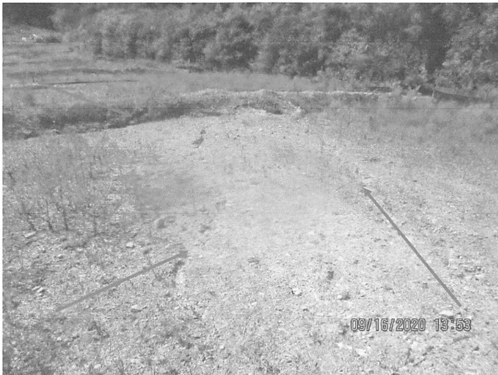
Facing downslope near station No. 6698+00. Erosion occurring between waterbars on slope (red arrow) and in waterbars.
