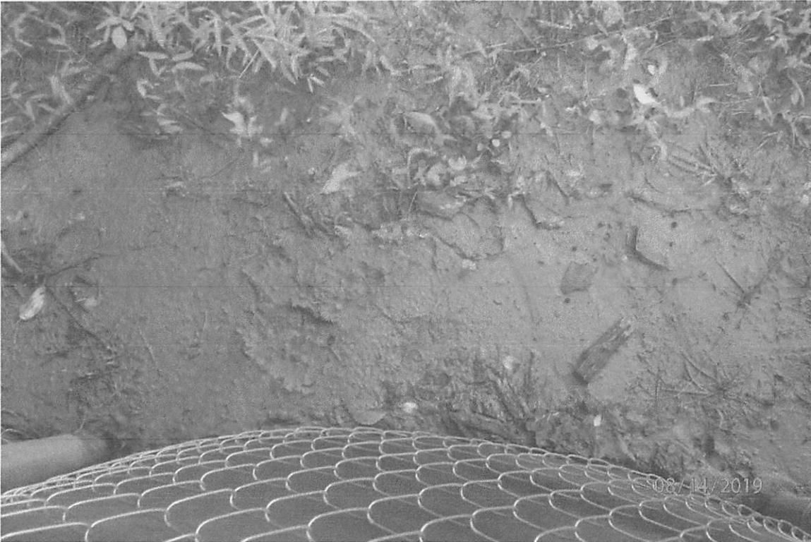
Sediment-laden water that has bypassed under the installed perimeter control in inspected area 3 as a result of failure to properly operate and maintain the installed BMP. Offsite sediment deposits pictured.
