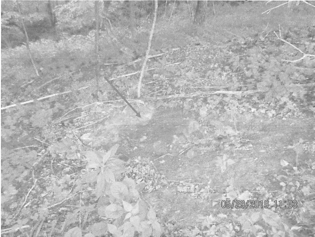
Below diversion berm Outlet 2 near 4031+00. Scouring of vegetation present below control. Sediment deposits were observed approximately 150 ft downslope of controls.
