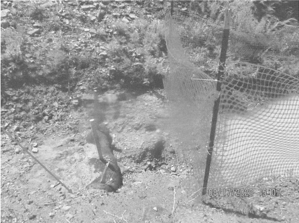
Sediment deposited into waterbar was overwhelming controls below. Waterbar failure and erosion occurring on fill slope at Station No. 6613+00.
