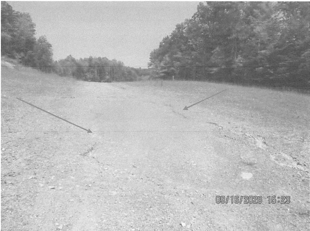
Near Station 6450+76 facing upslope toward erosion on slope (red arrow).
