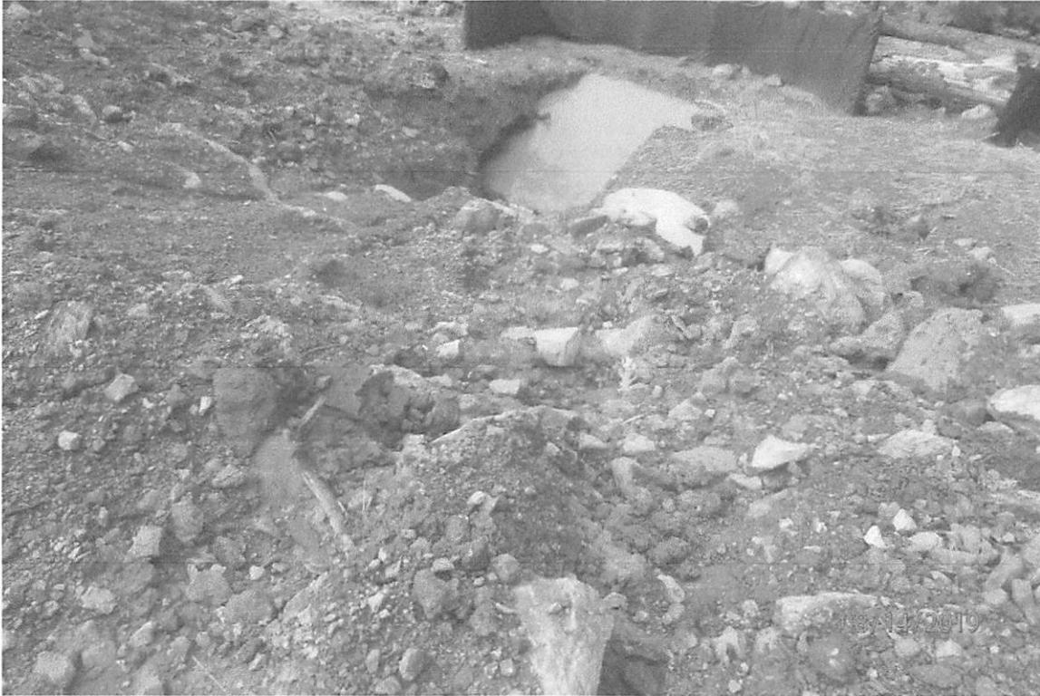
Water bar in inspected area 2 discharging over a steep slope with no fill slope protection in place.
