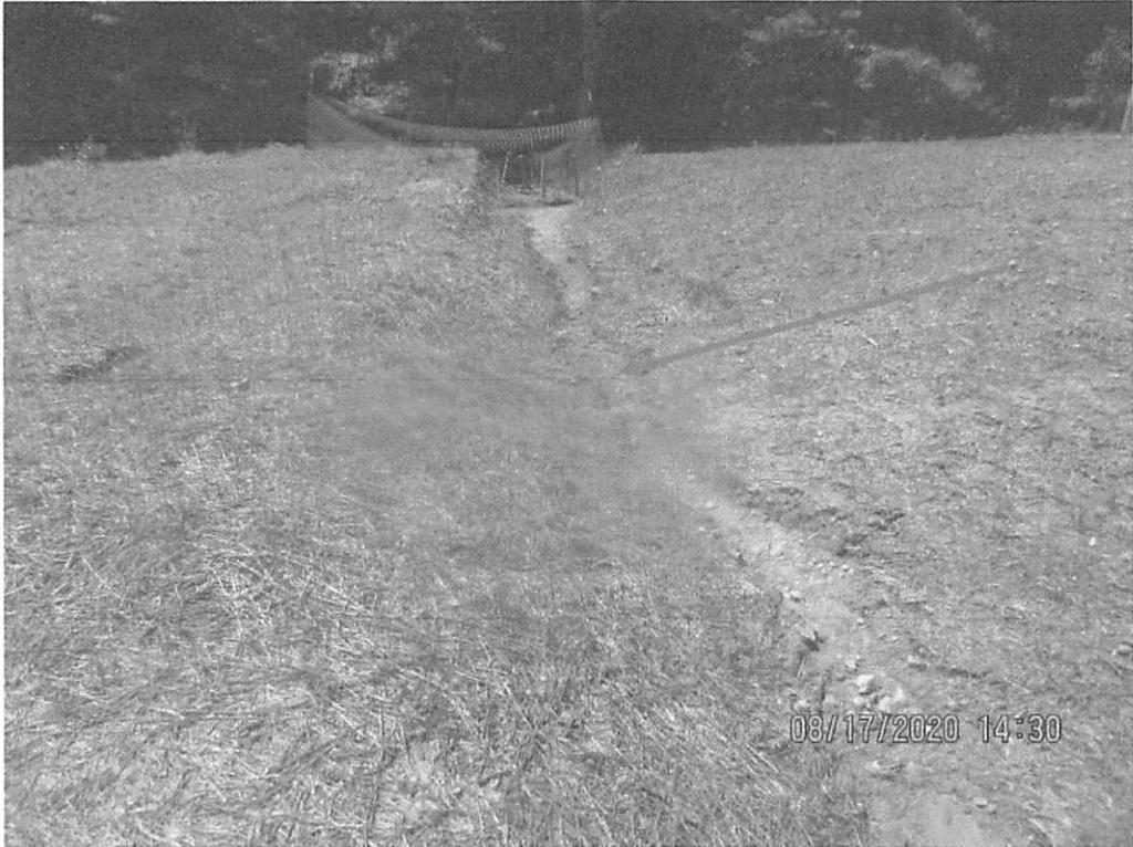
Facing downslope (South) near Station No. 6617+00. Less than 70 percent vegetative coverage. Erosion present in waterbar.
