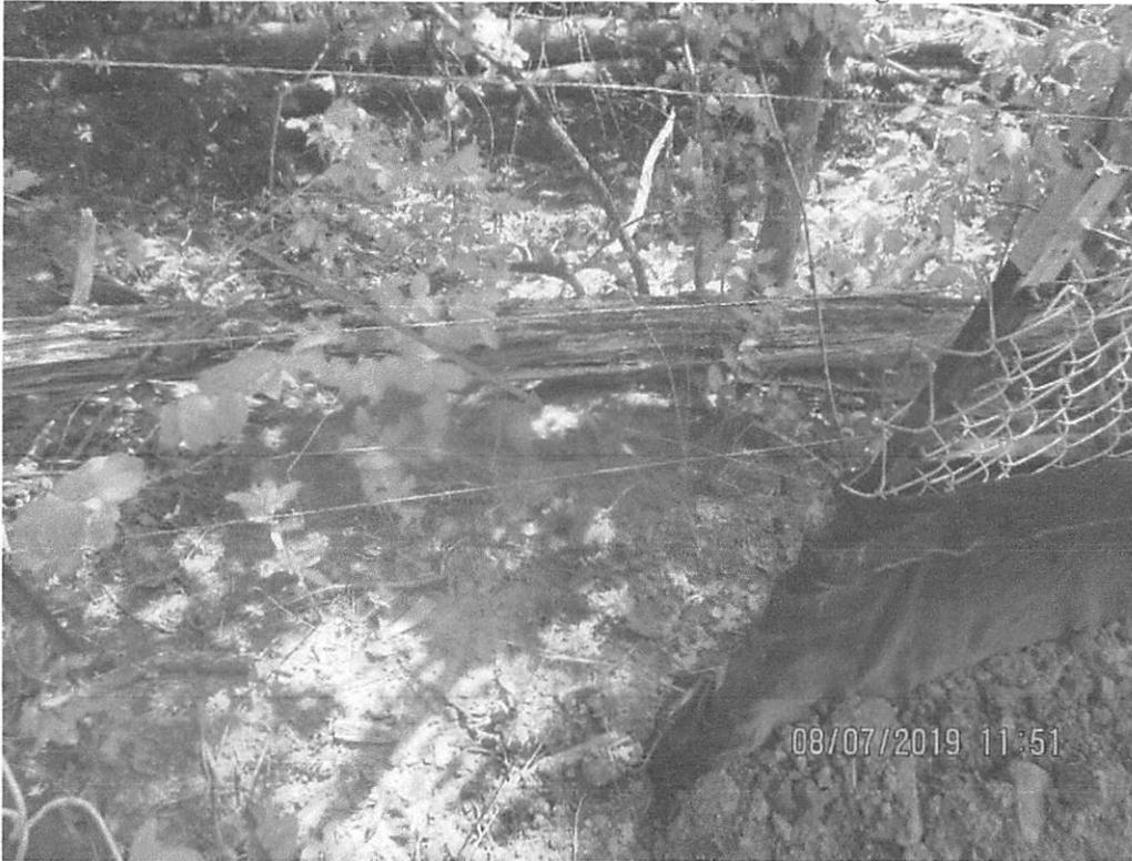
Sediment deposits past the LOD near station 8955+00, downslope of waterbar terminating onto ROW.
