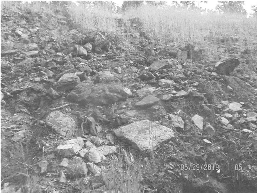
Fill slope with erosion present above diversion berm Outlet 3 near station 4031+00.
