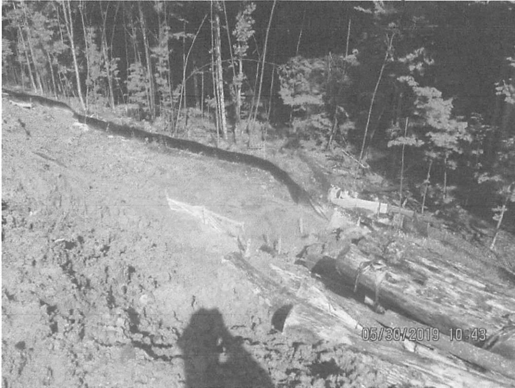
Slope below waterbar terminus. Perimeter controls becoming overwhelmed with sediment.
