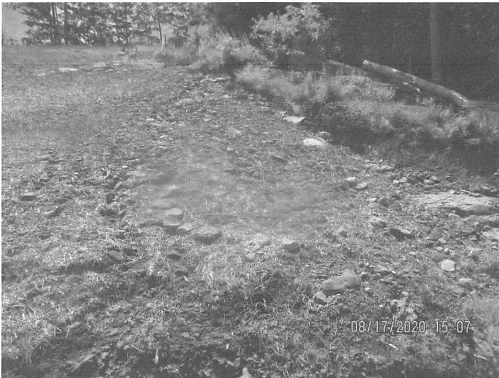
Facing upslope at waterbar that had failed, was terminating onto the fill slope, and was causing erosion at Station No. 6613+00.
