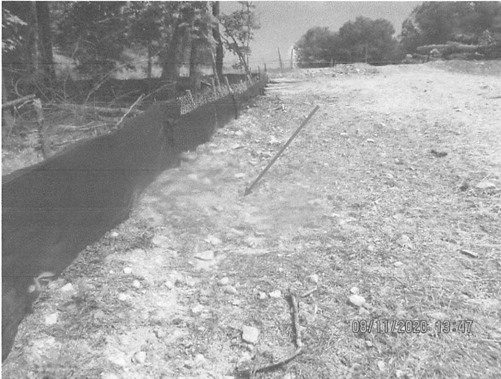
Facing North above Stream S-N10. Perimeter controls were recently replaced. However, erosion was present along controls lacking j-hooks.
