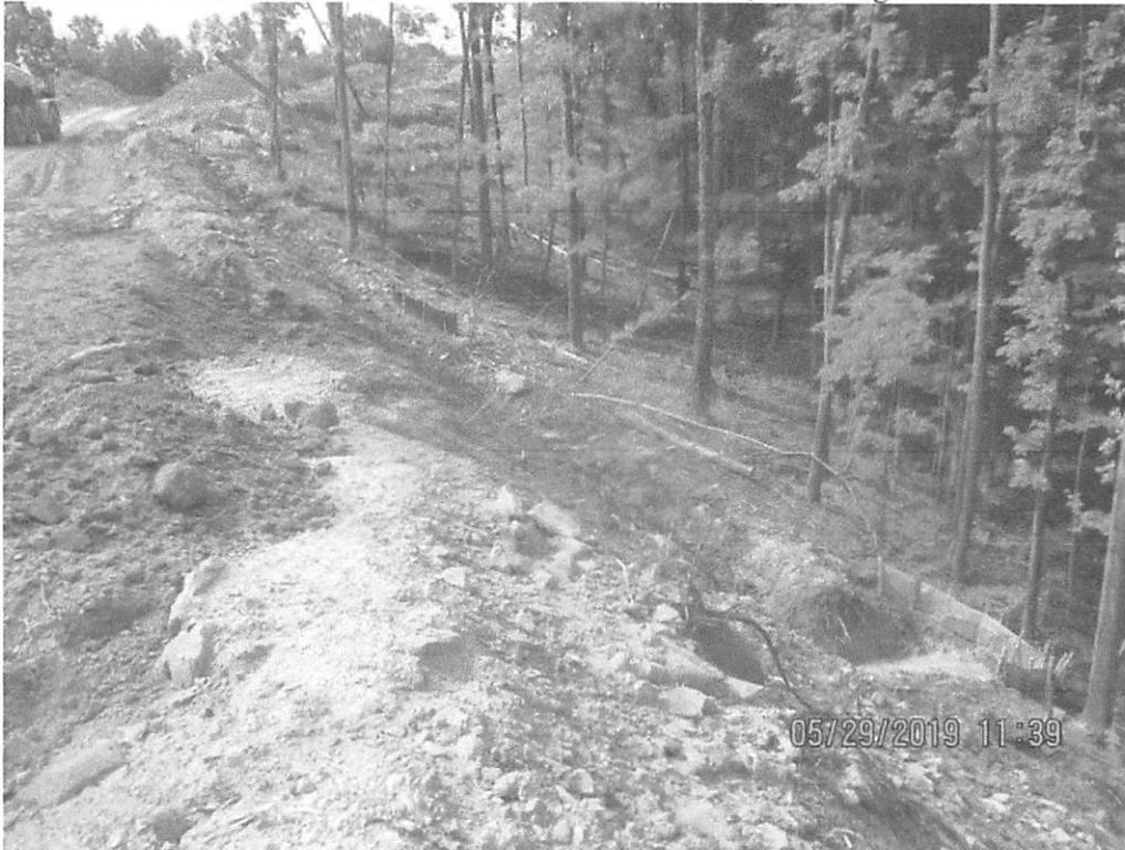
Facing upslope near station 4027+00. Arrow depicts waterbar and sediment deposits. Diversion berm installed as perimeter control with multiple outlets.
