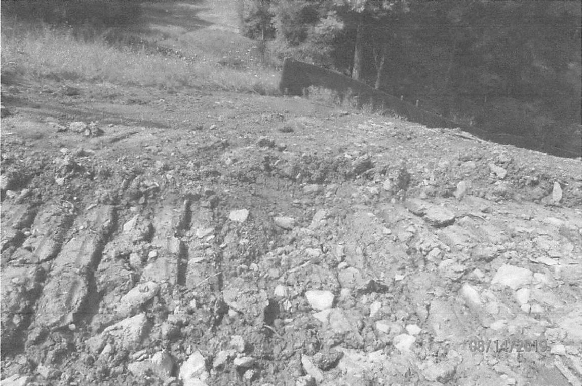
Water bars in inspected area 5 installed at a steep angle and discharging prior to the installed perimeter controls.
