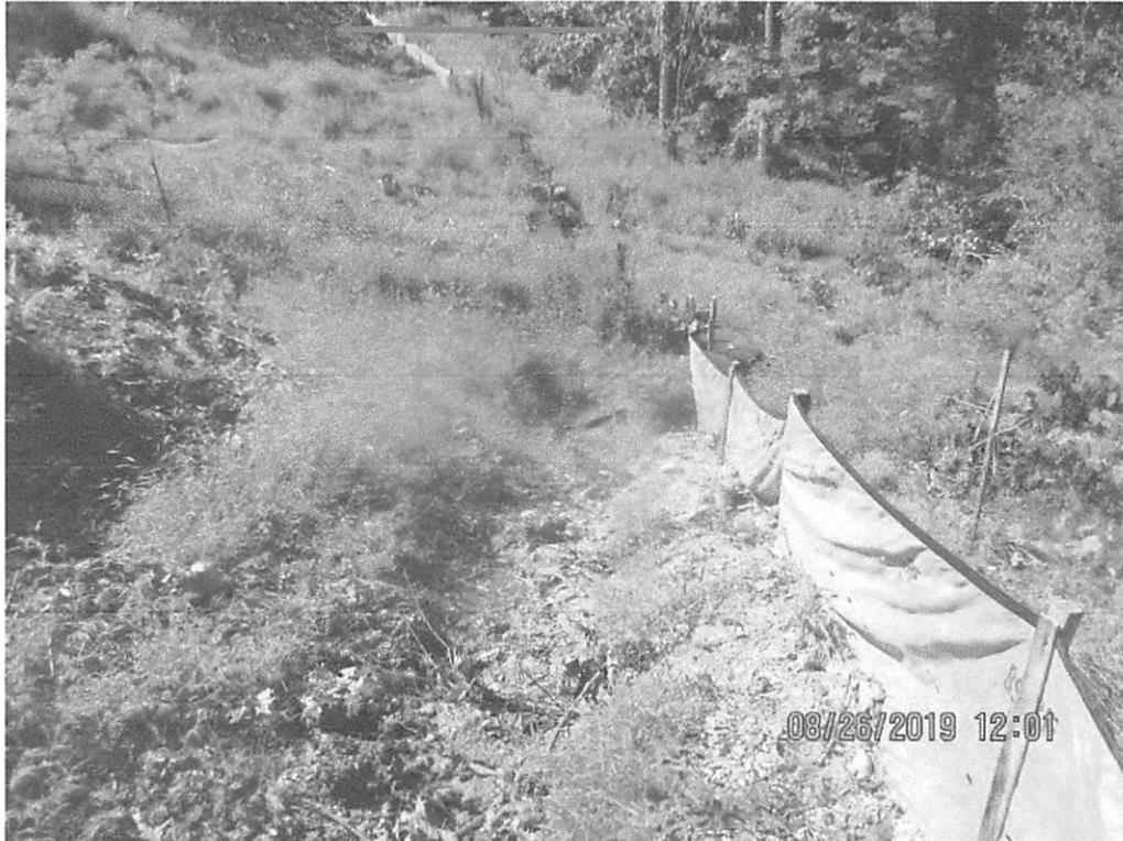
Near Station 1833+00. Perimeter controls overwhelmed due to erosion on slope. Arrow depicts where erosion was occurring.
