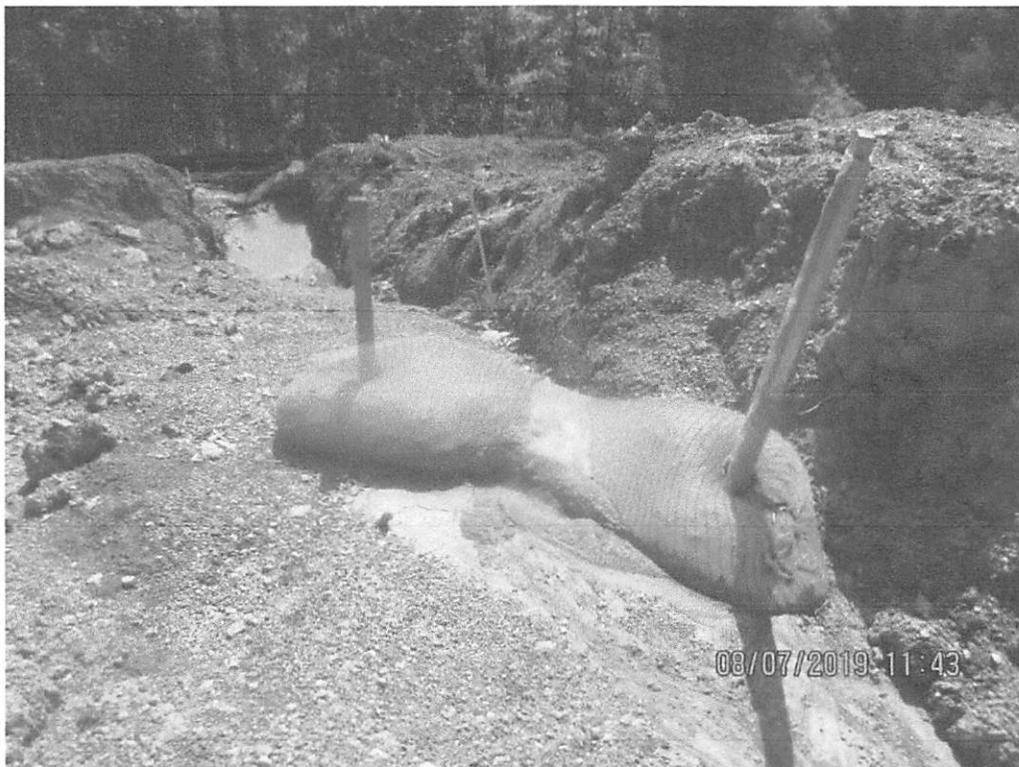
Waterbar terminus near station 8955+00. Erosion present on slope below waterbar terminus.
