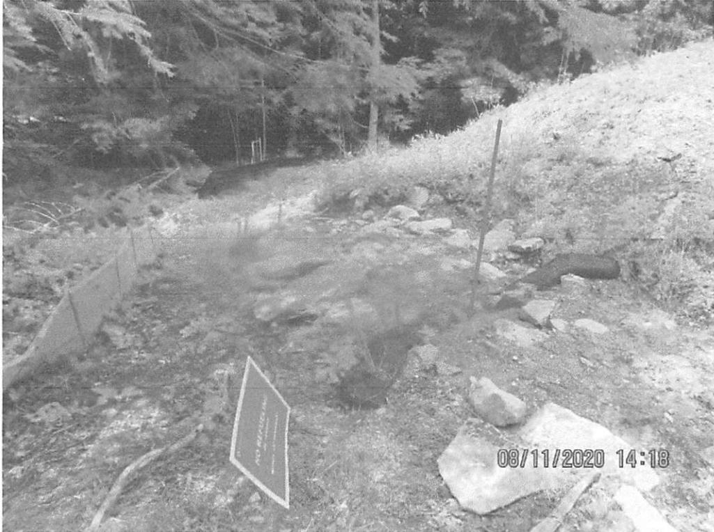
Downslope of slope drain outlet at Station No. 6490+00. Sediment deposits behind controls.
