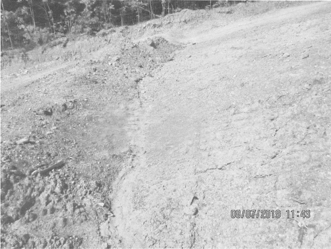
Erosion present in waterbar near station 8955+00 facing upslope.
