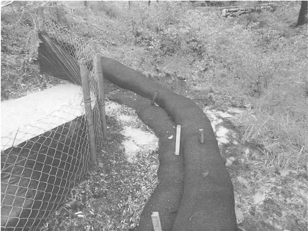
Controls below Stout Run Road were not effective at controlling sediment runoff
