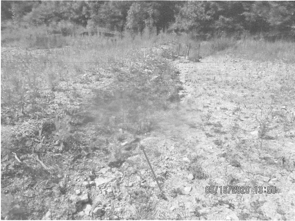
Waterbar with erosion present near Station No. 6703+00, controls in waterbar lacking maintenance.
