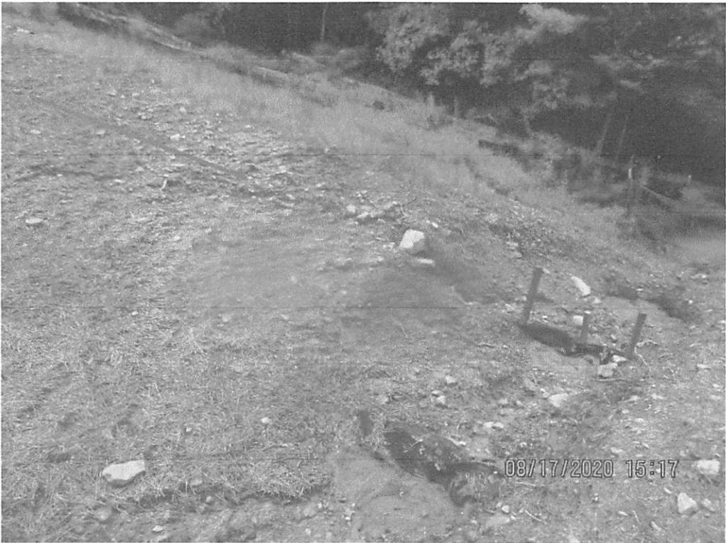
Waterbar downslope of Station No. 6613+00 with erosion present due to concentrated flows. Controls lacking maintenance and/or enhancement. Red arrow depicts erosion on fill slope above waterbar.
