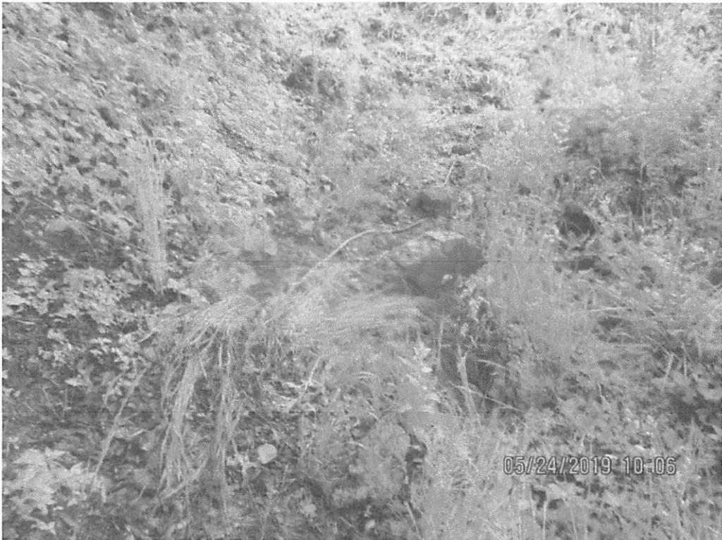
Facing toward MVP LOD near station 8387+96. Material had slipped from pile off ROW past LOD. No perimeter controls in place.
