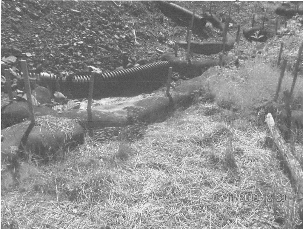
at station 7636+00 at waterbar outlet and slope drain. Slope drain was being undercut. Sediment was overwhelming perimeter control. Control in need of maintenance.
