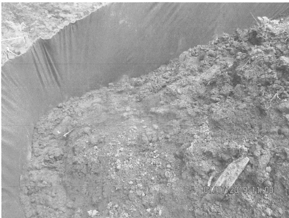
Controls at base of diversion berm. Sediment deposits had been removed from behind controls and new fabric installed over super silt fence at station 3147+11.
