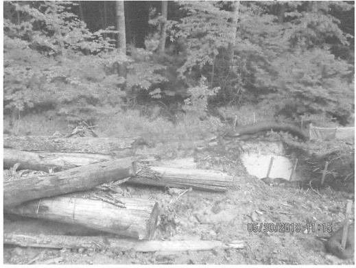
Same area near station 6945+00. Perimeter controls not extended per SWPPP into outlet controls.
