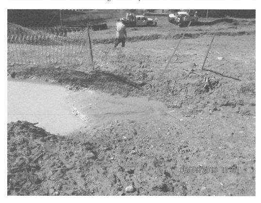
Above Lower Krosier Road crossing. Erosion present in waterbar causing sediment to be deposited in sump. Sump in need of maintenance.
