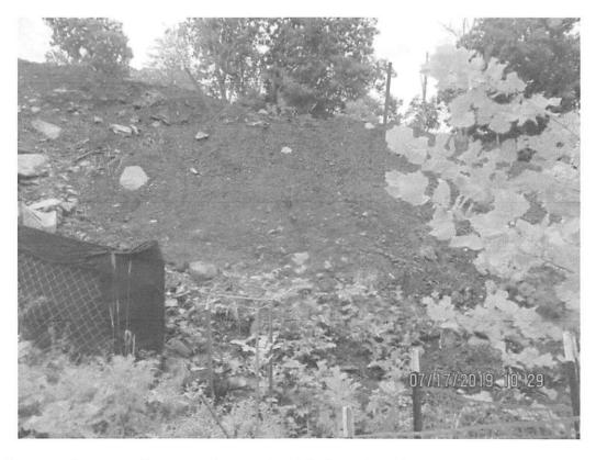
Fill slope erosion occurring at station 3159+46 facing edge of MVP LOD. Sediment deposits observed past the LOD.
