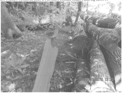
Downslope of waterbar terminating onto ROW at station 3831+00. Arrow depicts where perimeter controls were undercut from run-off and sediment deposits were observed past the LOD.
