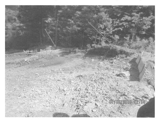
Above Stream S-T35A near station 8634+00 facing toward the East side of the LOD. Arrows depict the original cut to grade ROW that created a wall, preventing proper waterbar outlet installation.
