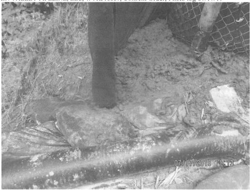
Controls at bridge that crosses Stream S-H153. Controls were overwhelmed with sediment.
