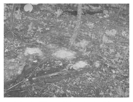
Sediment deposits observed past LOD and controls below waterbar and topsoil pile at station 6508+30.
