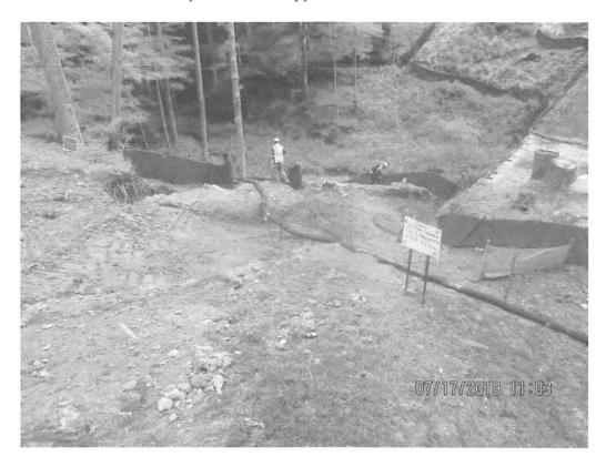
Slope drain conveying across ROW and terminating past LOD and controls. Control failures occurred in this location and impacted stream S-H153.
