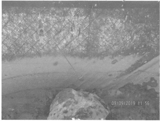
Super silt fence below unmaintained controls at station 3089+00. Hole present in silt fence below where sediment stain line was observed.
