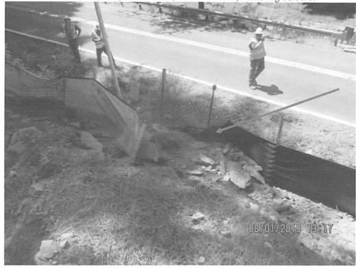
Perimeter controls at base of slope above US 19/Hwy 4 crossing. Controls overwhelmed with sediment, causing control failure above roadside ditch.
