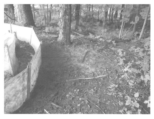
Facing downslope toward Stream S-N10. Scouring of vegetation and sediment deposits were observed below these controls.
