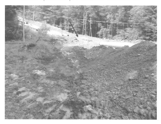
Sediment deposits and SLW traveling downslope at station 6510+40. Seep was present in cut next to topsoil pile. Channel was not stabilized and conveyed to a sump with a slope drain that crosses ROW. Arrow depicts seep. Black arrow shows sump with slope drain inlet.
