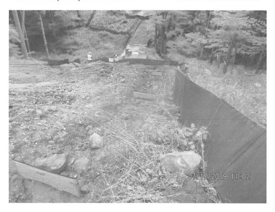
Facing downslope at station 3146+00 toward stream S-H153. Diversion berm installed on slope leading to sump above stream.
