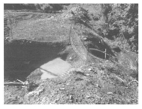
Downslope of Krosier Road Crossing near station 7576+01. Waterbar outlet perimeter controls in need of maintenance. SLW and deposits were present past controls and LOD. Arrow depicts sediment backed up behind controls causing SLW to overtop the control.
