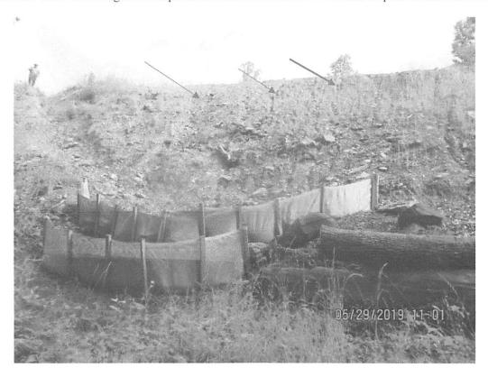
Facing upslope near station 4031+00 at diversion berm Outlet 2. Waterbar was terminating onto slope with no controls. Arrow depicts erosion on slope.
