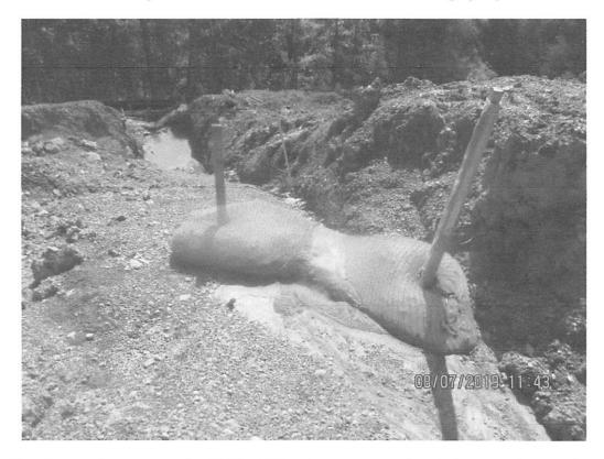
Waterbar terminus near station 8955+00. Erosion present on slope below waterbar terminus.
