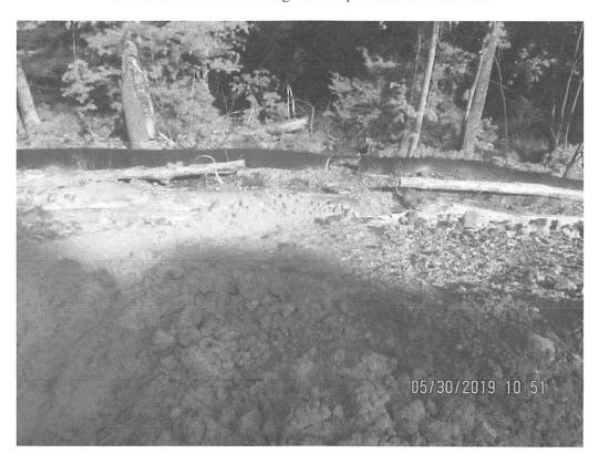
Waterbar outlet terminating onto slope at station 6485+10. Erosion present on slope above perimeter controls.
