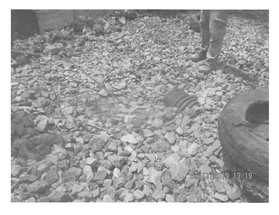
Above Stream S-UV12. Culvert outlets where sediment-laden water was conveyed that overtopped controls.
