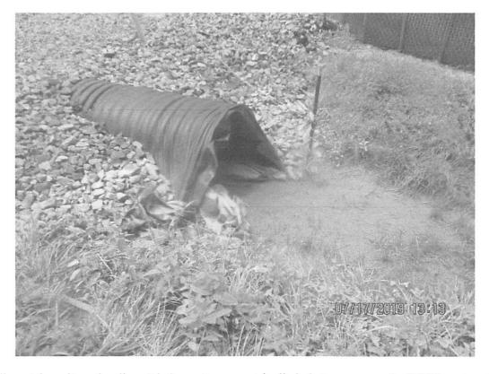
Sediment deposits and sediment-laden water present in ditch that conveys under ROW construction entrance, connects to elbow, conveys under CR23, and outlets on South side of road above Stream S-UV12.
