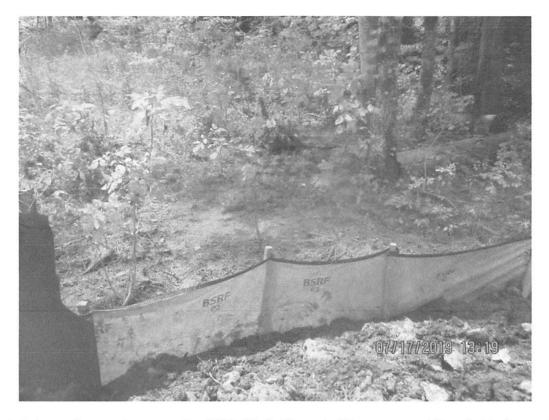
Controls below culvert outlets at station 3192+50. Sediment had been removed from behind controls and new controls had been installed. Sediment-laden water had left the site.
