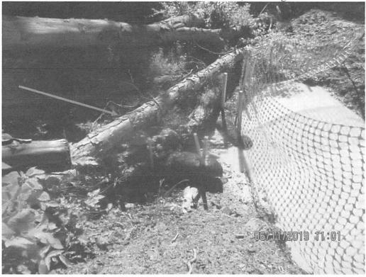
Above Lower Krosier Road crossing. Sediment and SLW overwhelming sump and perimeter controls near station 7604+41. Sediment deposits and SLW past controls and LOD.
