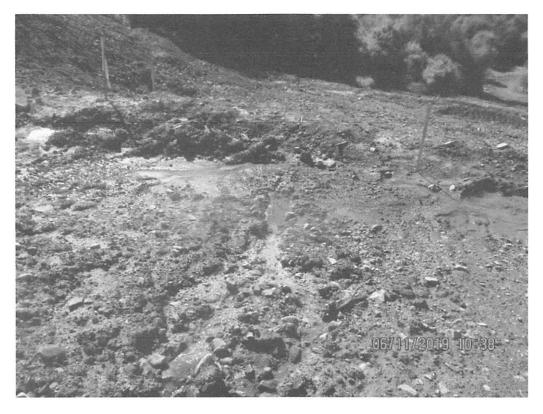
Below upper Krosier Road crossing near station 7576+01 facing South at waterbar. Erosion present on slope due to seep running onto ROW. Sediment deposited in waterbar.
