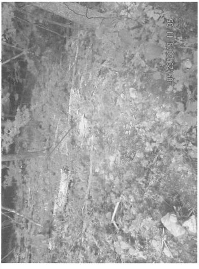
Sediment deposits present past LOD at station 4027+00 facing downslope of perimeter outlet.
