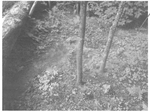
Sediment deposits past controls and LOD at station 3136+00. Log piles placed behind controls.
