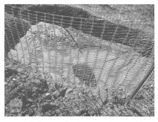
Above station 7604+41. Waterbar had sediment from erosion, causing sump to be full of sediment.
