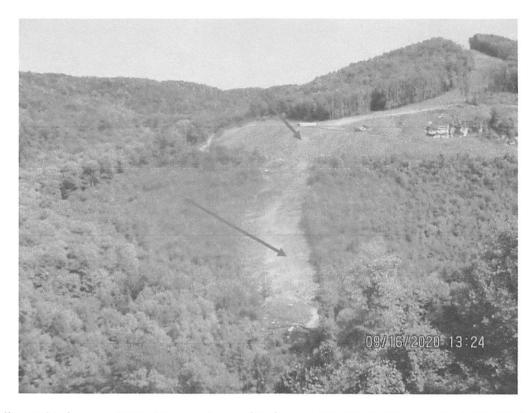
Standing at Station No. 6715+00 toward opposite slope at AR-160.01 (Station No. 6698+00 through 6707+00). Erosion observed on slope (red arrows).
