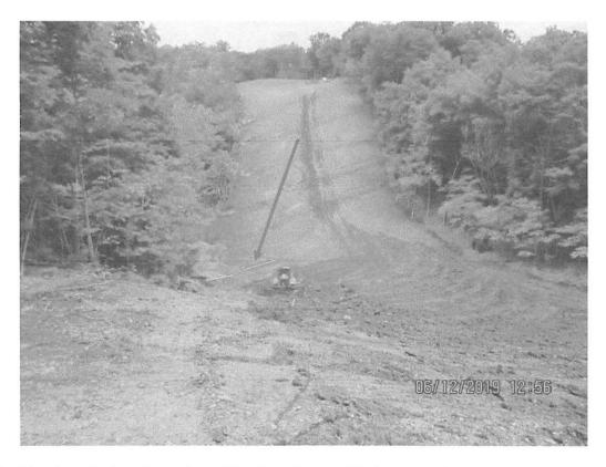
South Side slope facing downslope (North) at Dargo Silt fence. Red Arrow depicts where slope drain terminated onto ROW.
