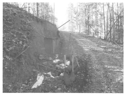
Access Road 114 above Stream S-S2. Red Arrow depicts slip. Orange arrows depict slope drain and small sump with culvert inlet conveying under AR-114.
