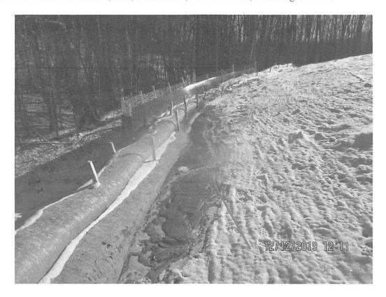
Sediment deposits present behind controls due to upslope erosion at station 8433+50.
