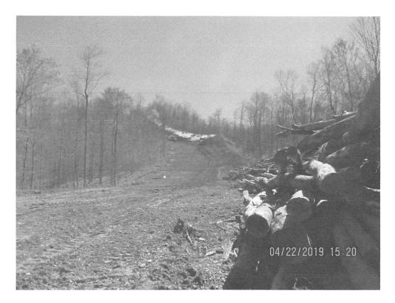
Facing South toward slope with waterbar failure near station 8628+00.
