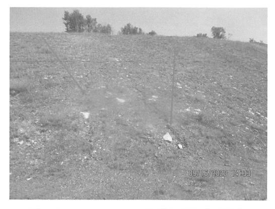
Rill erosion occurring on slope above AR-160.1 at Station No. 6698+00.
