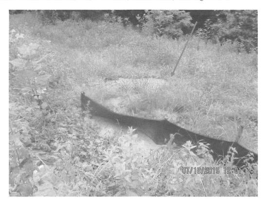
Downslope of waterbar outlet terminating on slope. Controls overwhelmed with sediment and deposits were present past the LOD and Controls. Arrow depicts sediment deposits.
