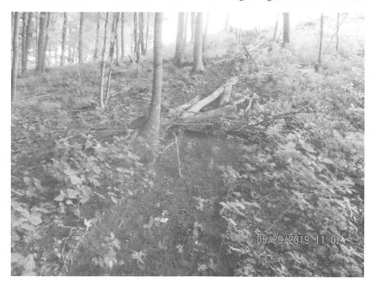
further downslope below diversion berm Outlet 2 near 4031+00. Scouring of vegetation below control.
