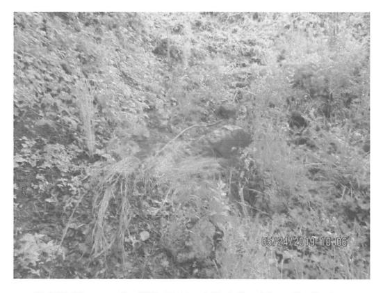
Facing toward MVP LOD near station 8387+96. Material had slipped from pile off ROW past LOD. No perimeter controls in place.
