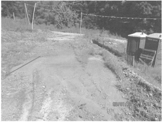
Above Access Road MVP-BR-097 and Falls Run (Stream S-J70) facing North. Run-on entering LOD and causing sediment to overwhelm controls. Arrow depicts where run-on was coming onto Access Road.
