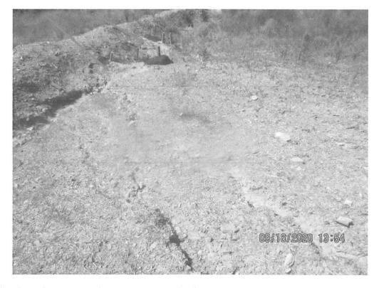
Facing downslope near station No. 6698+00. Erosion occurring between waterbars on slope and in waterbars. Controls lacking maintenance within waterbar (red arrow).
