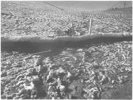
Section of ROW at station 8433+50 that was not tracked-in properly, causing enhanced erosion upslope of controls. Arrow depicts where CFS was undermined due to concentrated flows and area of ROW not tracked-in properly.
