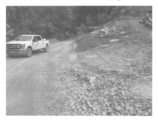
At station 4559+96 facing Access Road MVP-WB-119. Sediment deposits present in roadside ditch.
