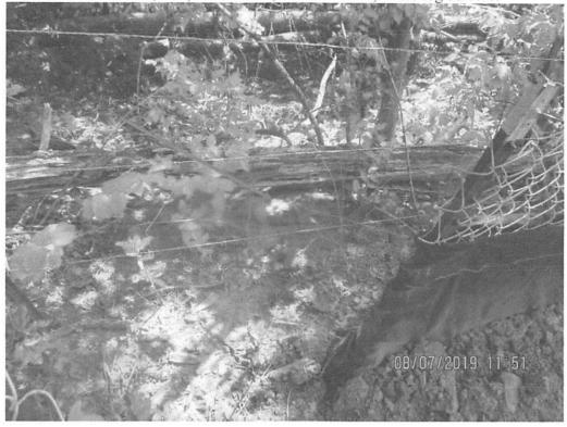
Sediment deposits past the LOD near station 8955+00, downslope of waterbar terminating onto ROW.
