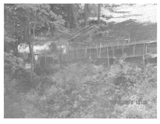
Controls above the South side of Falls Run (Stream S-J70) and US 19/Hwy 4 ROW crossing. Scouring present below controls.
