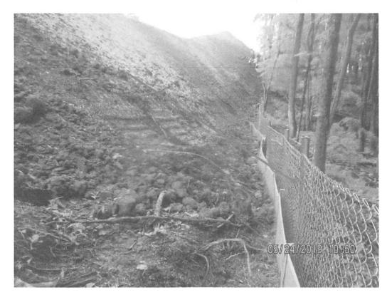
Near station 8419+00 facing South. Arrow depicts where material has slipped into P1 silt fence.
