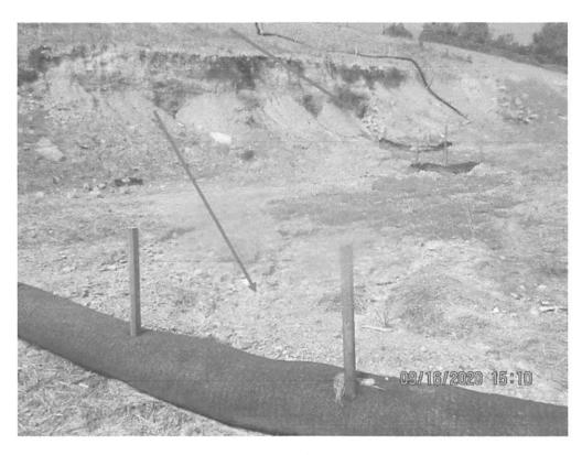
Standing at Access Road 159.01 facing upslope at Station No. 6450+76. Erosion present on cut slope and above controls (red arrow).
