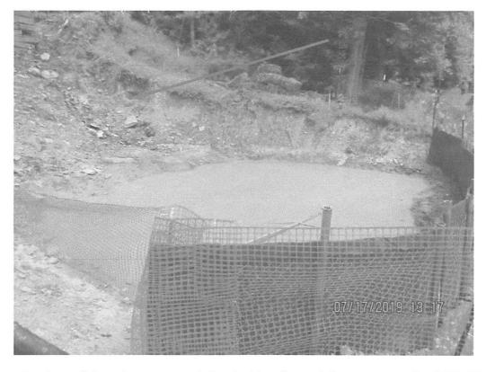
Open trench at base of slope that was overwhelmed with sediment-laden water at station 3192+50. Arrow depicts erosion present on slope above open trench/sump.
