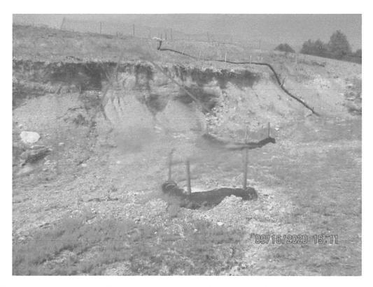
Erosion occurring on cut slope (red arrow) below slope drain outlet at Station No. 6450+76.
