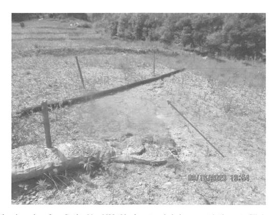
Further downslope from Station No. 6698+00 where trench drain was out-letting onto fill slope and causing erosion (red arrow).
