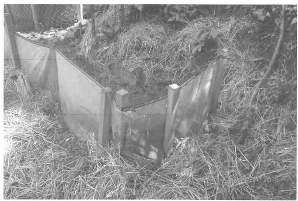
Recently maintained perimeter control utilized to treat stormwater from six water bars upslope of the pictured BMP.
