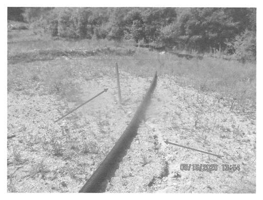
Erosion present on slope below pipe trench drain outlet and slope drain.
