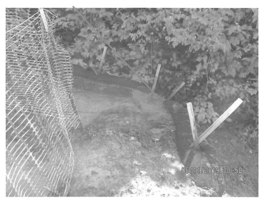
Above Lower Krosier Road crossing. Erosion present on ROW above waterbar. Sediment being deposited in waterbar and sump, overwhelming sump and perimeter controls near station 7604+41.
