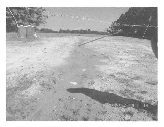
Facing North where Access Road MVP-BR-099 intersects ROW near station 3897+75. Arrow depicts where run-off was overtopping the diversion berm and flowing downslope.
