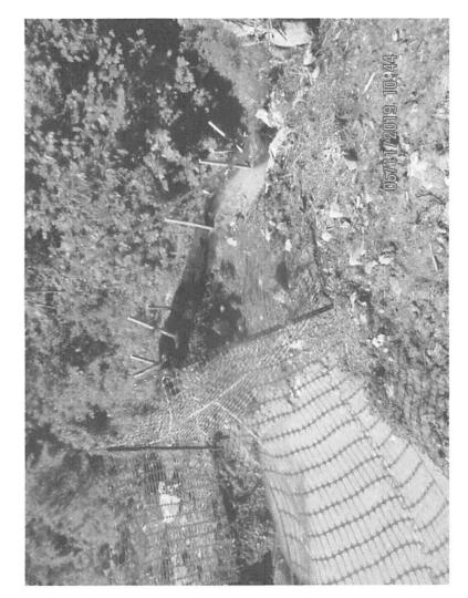
Waterbar outlet near 7604+41. Sump and perimeter controls in need of maintenance. Sediment deposited behind perimeter controls.
