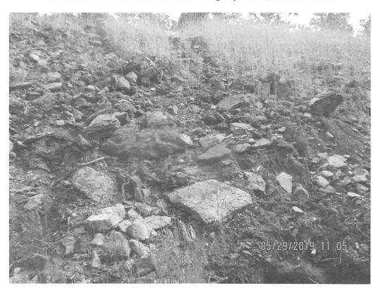
Fill slope with erosion present above diversion berm Outlet 3 near station 4031+00.
