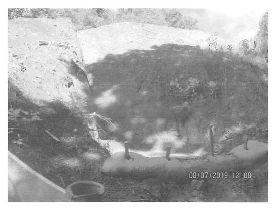
Controls below waterbar termini with no outlet control, terminating onto fill slope and above LOD near station 8951+00.
