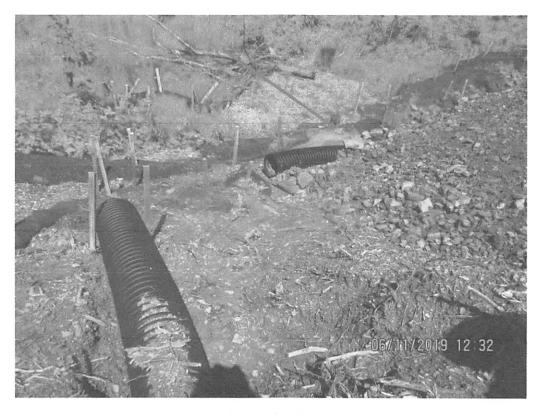
at station 7636+00 at waterbar outlet and slope drain. Slope drain was being undercut. Sediment was overwhelming perimeter control. Sediment deposits observed past controls and LOD.
