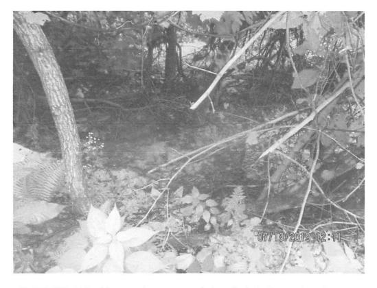
Section of MVP-WB-119 with no perimeter controls installed. Sediment deposits were observed past the LOD throughout the vegetated area downslope of the road.
