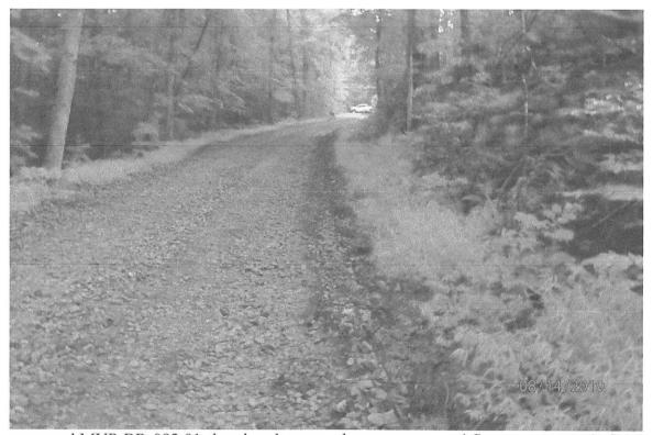
Access road MVP-BR-092.01 showing the area where concentrated flow stormwater is flowing from the top of the slope to the base of the hill due to poor maintenance on the installed culvert.
