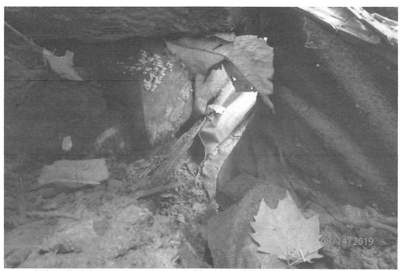
Improperly installed timber mat equipment bridge at the Oil Creek (inspected area 3) crossing, showing an area where sediment-laden water can bypass treatment.
