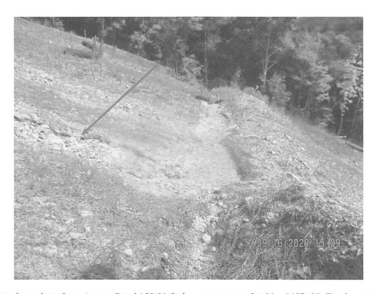
Standing downslope from Access Road 159.01 facing east near station No. 6657+00. Erosion present on slope, depositing sediment into waterbar and controls (red arrow).
