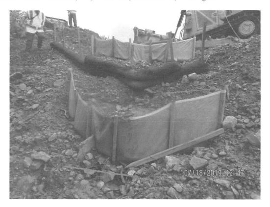
Waterbar outlet on opposite side of ROW at station 4559+96. Controls undercut and sediment deposits observed past controls and LOD. Arrow depicts undercut controls.
