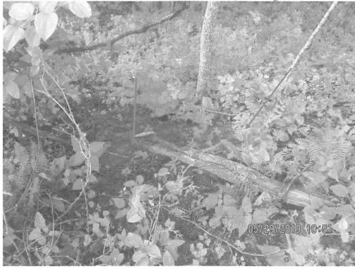
Waterbar outlet above fill slope at station 4031+00 facing downslope. Sediment deposits past LOD. Scouring from concentrated flow.
