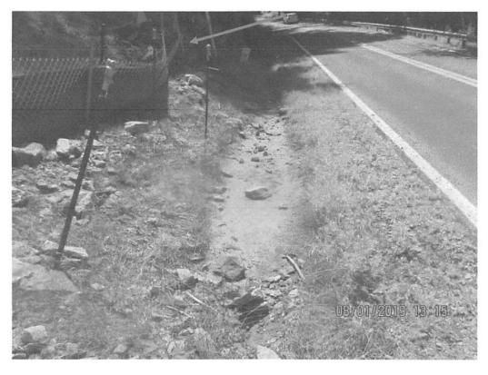
Sediment present in ditch that parallels US 19/Hwy 4 due to control failure. Arrow depicts control failure at base of slope.
