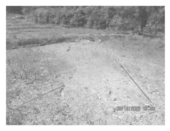
Facing downslope near station No. 6698+00. Erosion occurring between waterbars on slope (red arrow) and in waterbars.
