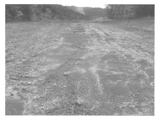
Section of ROW upslope from 6450+76 that was not reseeded since Fall 2019. Red arrow shows erosion occurring due to increased sheet flow.
