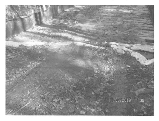
Stream S-S2 near station 4364+00. CFS at edge of bridge crossing flattened with sediment deposits built up behind it.
