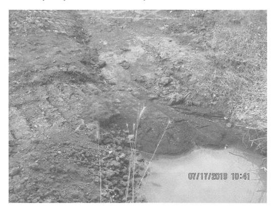
Sump at waterbar terminus near station 3151+47. Sediment deposits present past LOD due to lack of sump maintenance.
