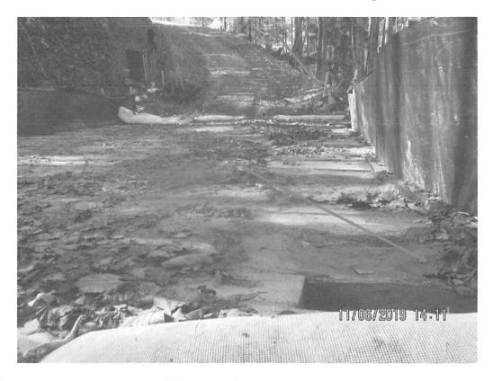
Facing upslope on Stream S-S2 bridge crossing. Arrow depicts where erosion was present on road resulting in controls being overwhelmed and sediment being deposited on bridge and past LOD.
