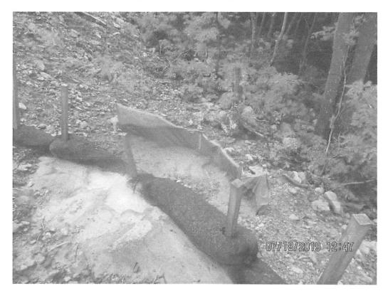
Waterbar outlet on opposite side of ROW at station 4559+96. Controls undercut and sediment deposits observed past controls and LOD.
