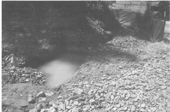
Improperly installed water bars in inspected area 8 that are discharging into a diversion, with stormwater from the diversion being directed at two pieces of installed perimeter controls.
