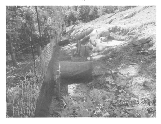
Perimeter controls below dewatering structure at station 8955+00. Arrow depicts where controls were overwhelmed with sediment.
