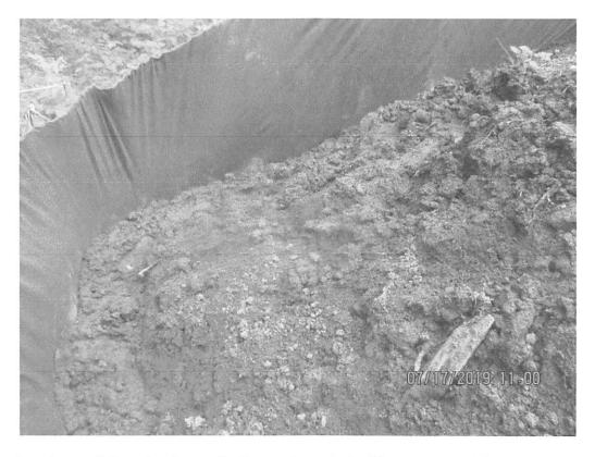
Controls at base of diversion berm. Sediment deposits had been removed from behind controls and new fabric installed over super silt fence at station 3147+11.
