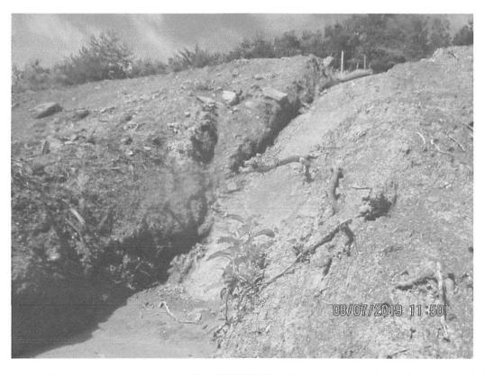
Waterbar terminating onto slope near station 8955+00. Erosion present on slope. Sump overwhelmed with sediment.
