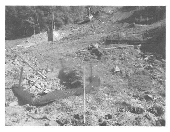
At station 3089+00 facing North. Arrow depicts sump not being maintained and erosion on slope below controls.
