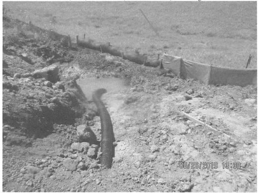
Slope drain extending from waterbar outlet terminating into sump above perimeter controls. Arrow depicts where sediment deposits were observed past controls above Wetland W-K48 at station 1730+00.
