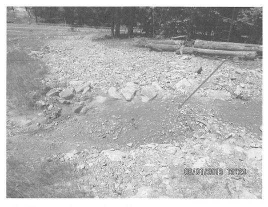
Near station 3831+00. Erosion present in travel lane resulting in waterbar being overwhelmed with sediment and not functioning as designed. Arrow depicts sediment deposited behind Waterbar.
