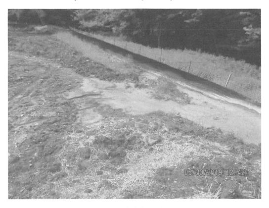
Erosion (Red Arrow) and Sediment/SLW overwhelming perimeter controls at ATWS-22-7A at station 6514+60. Sediment deposits observed past controls and LOD.
