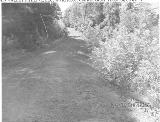
MVP-BR-095 facing upslope above US 19/Hwy 4. Arrow depicts where road was eroded out, overwhelming downslope controls.
