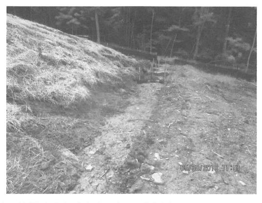
Waterbar with CFS checks installed and scouring topsoil pile below Deepwell road crossing at Station 6508+30.
