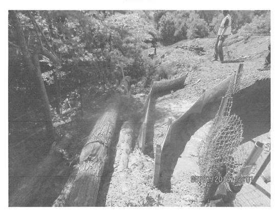
Near station 8955+00. Perimeter controls below waterbar terminating onto fill slope and sump that was full of sediment. Perimeter controls overwhelmed and sediment deposits present past log pile.
