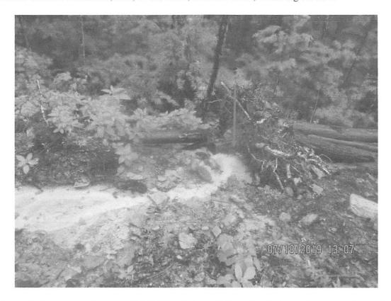
Sediment-laden water flowing off ROW and through log pile during rain event. No perimeter controls were present at the base of the slope. Arrow depicts were SLW was flowing through log pile.
