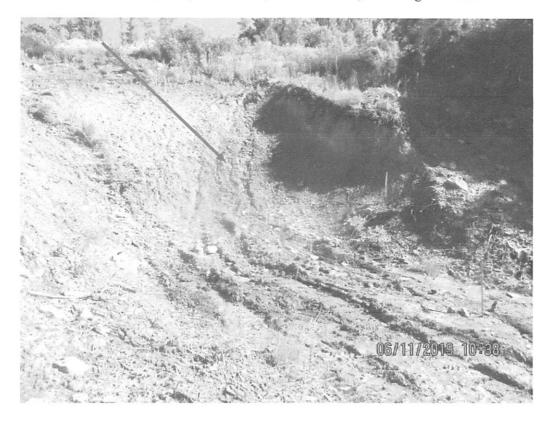
Below upper Krosier Road crossing near station 7576+01 facing North. Erosion present on slope due to seep running onto ROW.
