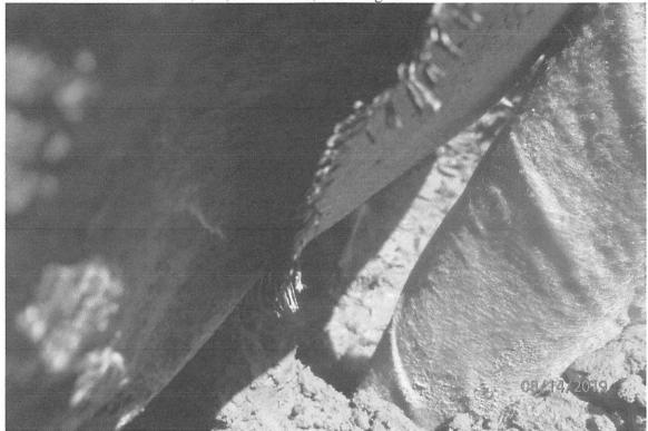
Improperly installed timber mat equipment bridge at the Cove Run (S-K-45) (inspected area 8) crossing, showing an area where sediment-laden water can bypass treatment.
