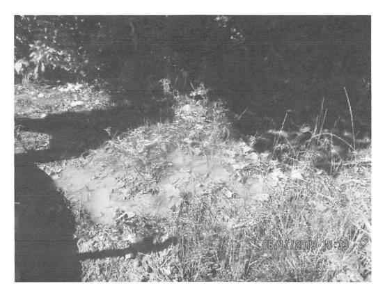
Downslope of Krosier Road Crossing near station 7576+01. SLW and deposits were present past controls and LOD.
