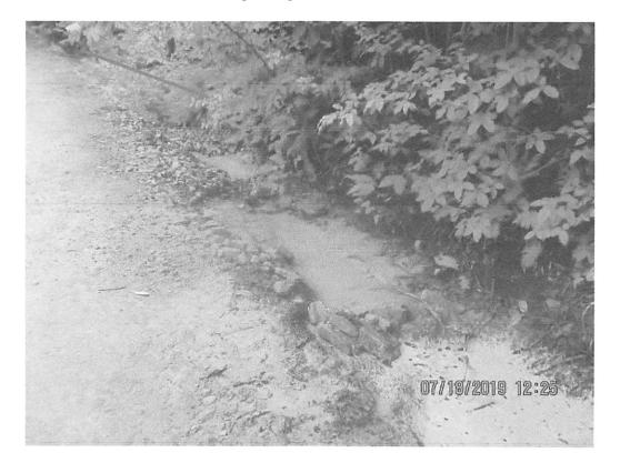
Downslope of station 4559+96 on Access Road MVP-WB-119. Sediment deposits present in roadside ditch and conveying to culvert inlet. Arrow depicts approximate location of culvert inlet.
