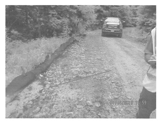
Facing perimeter controls along access road MVP-WB-119. Controls were overwhelmed with sediment.
