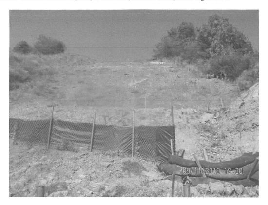
South slope at station 645+00 above the Big Elk Creek crossing. Winter stabilization no longer adequate, and reseeding/re-stabilization had not occurred.
