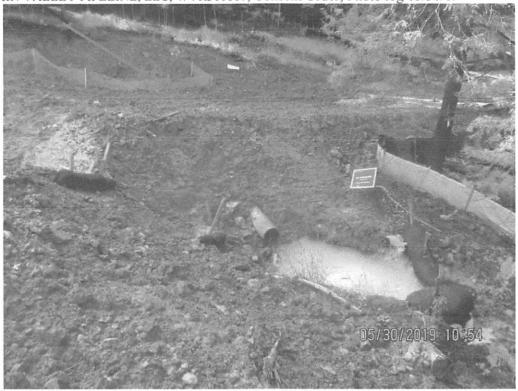
Drain outlet above Stream S-EE1. Clean water diversion not stabilized above or below inlet/outlet. Clean water was being conveyed approximately 15 ft across disturbed soil to a sump where the inlet was located. The topsoil pile around the inlet was eroding into the sump. Arrow depicts inlet.
