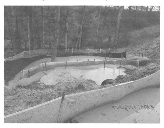
Culvert outflow into multiple controls with SLW present.
