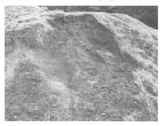
Topsoil pile slipping into waterbar at station 6508+40.
