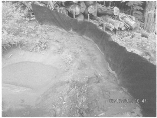
Waterbar terminus and sump at station 3149+00. Sump full of sediment and sediment deposits past LOD.
