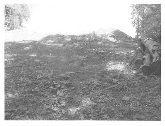
Slope above US 19/Hwy 4 and station 3831+00 not stabilized. Waterbars terminating onto ROW and not at edge of LOD. Arrow depicts erosion occurring below waterbar on slope.
