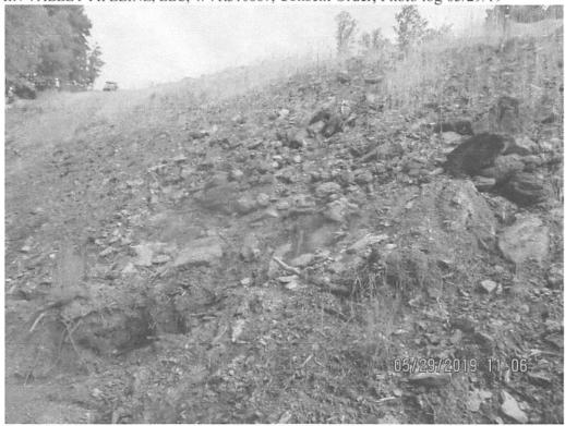
Fill slope with erosion present above diversion berm Outlet 3.
