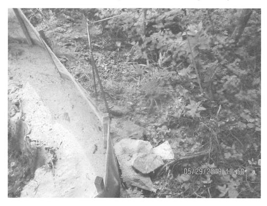
Waterbar outlet above fill slope at station 4031+00 facing downslope. Sediment deposits past LOD.
