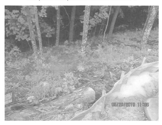
Downslope of diversion berm Outlet 3 controls. Scouring of vegetation with sediment deposits present past LOD.
