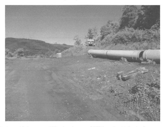
on Krosier road facing east at additional workspace and ROW crossing. Mud and sediment present on road. Run-off flowing toward culvert inlet along Krosier road. Arrow depicts culvert inlet location.
