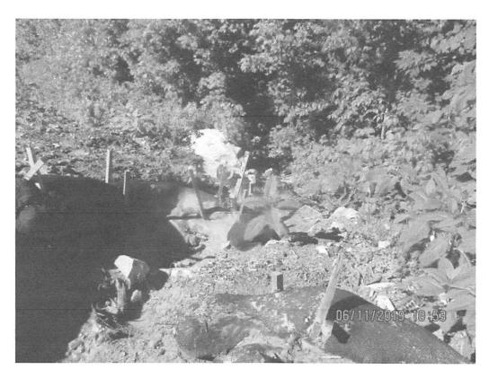
Above Station 7604+41. Perimeter controls overwhelmed with sediment. Sediment deposits present past LOD.
