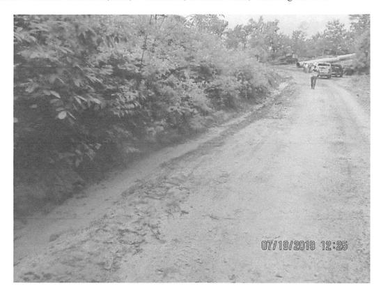
Downslope from station 4559+96 from Access Road MVP-WB-119 facing toward MVP ROW. Sediment deposits present in roadside ditch.
