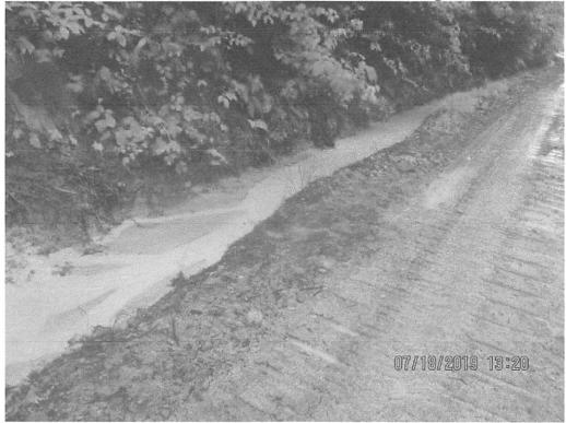
Downslope of failed controls post rain event along Access Road MVP-WB-119. SLW was entering/cascading into the ditch that conveys back downslope toward ROW crossing with access road.
