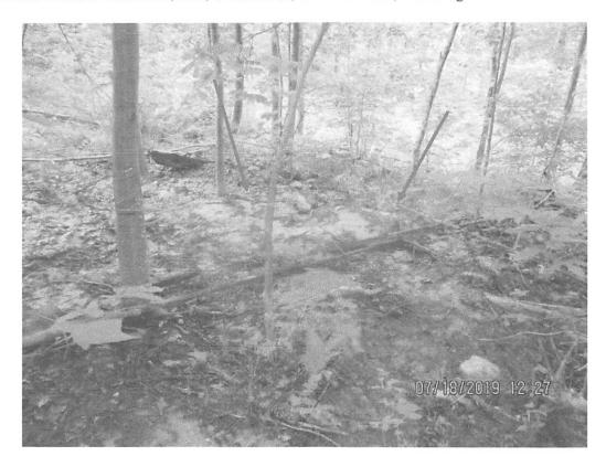
Downslope of culvert outlet. Significant sediment deposits present past controls and LOD. Arrows depicts examples of deposits observed.
