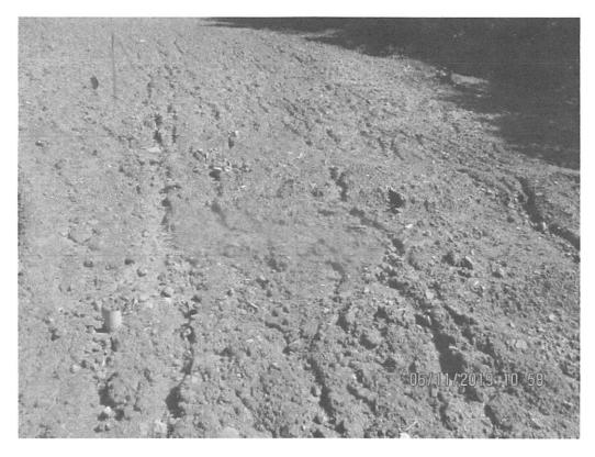
Above Lower Krosier Road crossing. Erosion present on ROW above Waterbar. Facing upslope near station 7604+41.
