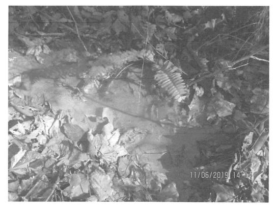
Example of sediment deposits observed in the conveyance between S-S2 crossing and Oddlick Creek near station 4364+00.
