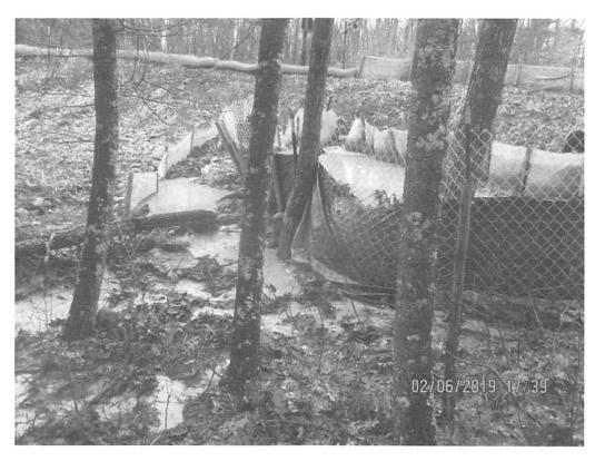
SLW flowing past controls and downslope to UNT of Brammer Branch. Back side of silt fence fallen over.
