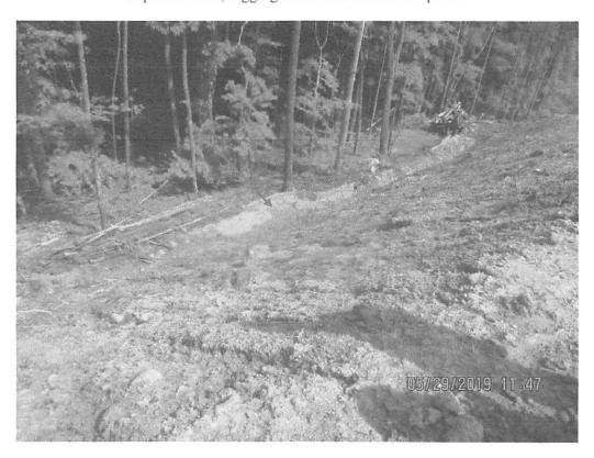
Erosion present on slope near Station 4017+00. Perimeter controls overwhelmed with sediment.
