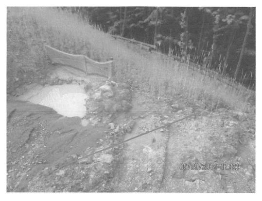
Waterbar outlet above diversion berm Outlet 3. Sump full of sediment and concentrated flow on slope was observed due to controls not functioning as designed. Arrow depicts flow.
