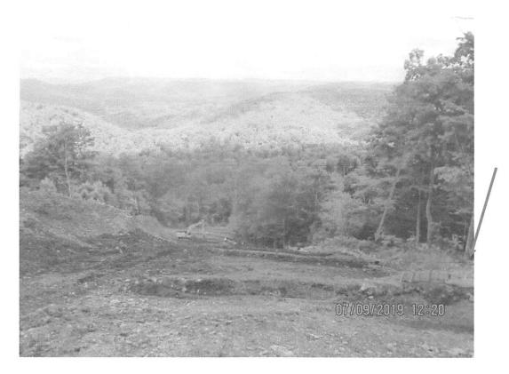
Overview of Lick Creek basin facing North above Station 8634+00 on upper section of slope. Arrow depicts cut into natural grade that continues down to lower portion of slope.
