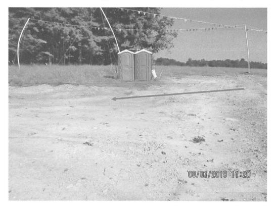
Downslope of diversion berm near station 3897+75. Arrow depicts where sheet flow due to run-off was occurring.
