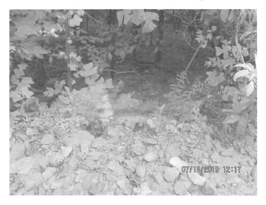
Section along Access road MVP-WB-119 where rock washed out past LOD. No controls present on downslope edge of road. Sediment deposits observed past LOD.
