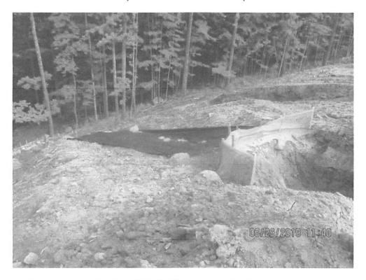
Waterbar outlet downslope of station 4027+00. Waterbar terminating on slope. Fabric installed below control on slope above perimeter outlet.
