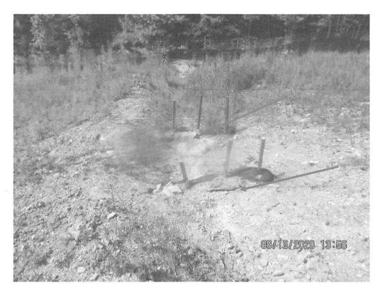
Waterbar with erosion near Station No. 6703+00, controls in waterbar lacking maintenance (red arrow).
