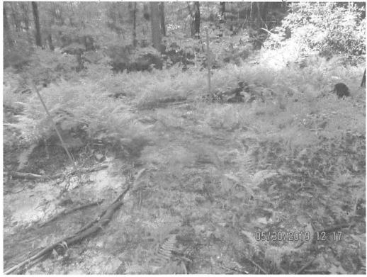
SLW and sediment deposits observed past controls and LOD near station 6510+40 approximately 200 ft past LOD and downslope of sump outlet.
