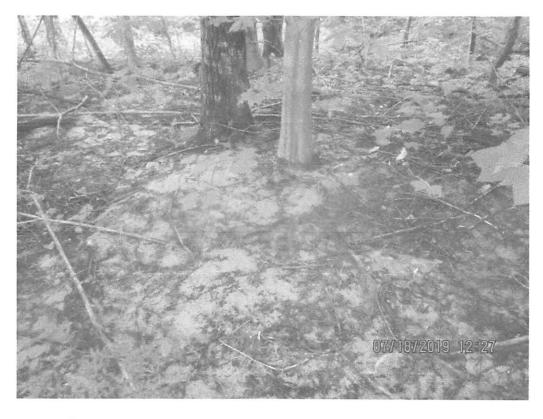
Downslope of culvert outlet. Significant sediment deposits present past controls and LOD.
