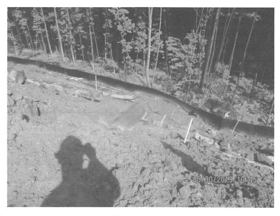
Pipe outlet below seep. Diversion not stabilized and no rip rap apron installed as required per SWPPP near station 6485+10. The inlet had been cut due to trench being dug.
