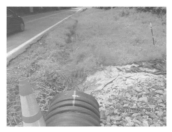
Culvert outlet that conveys under ROW construction entrance. Sediment deposits and SLW present in ditch.
