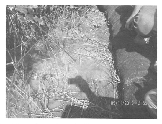
Sediment-laden water flowing under controls and into vegetation above Stream S-B75 (Goose Run) near station 645+35.
