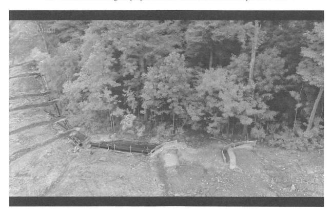
Lower portion of slope with flume pipe system. Arrow depicts where single outlet received concentrated flow from run-off. Impacts occurred to East side of LOD.
