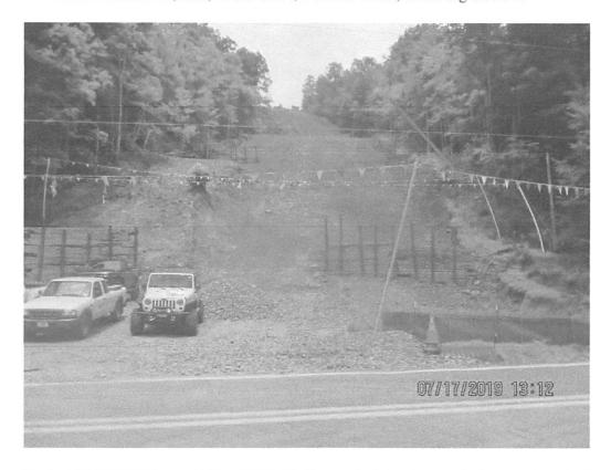
Facing North at MVP ROW near station 3192+50. Arrow depicts where waterbar was terminating onto ROW and failed causing pipe trench to become overwhelmed with sediment-laden water.
