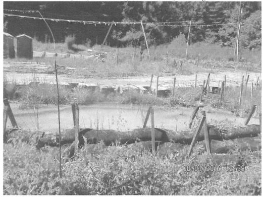
Facing upslope at MVP-BR-097. Arrow depicts where run-on was coming onto site. Sandbags had been installed to divert run-on away from site but had failed due to concentrated flow upslope of LOD.
