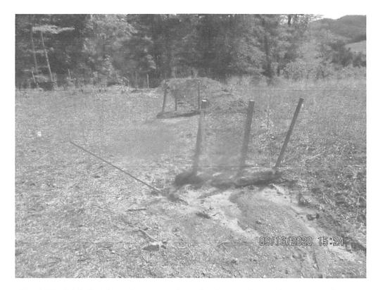
Near Station 6450+76 facing downslope toward erosion in waterbar (red arrow). Sediment was being deposited in waterbar, and runoff was flowing around unmaintained controls.
