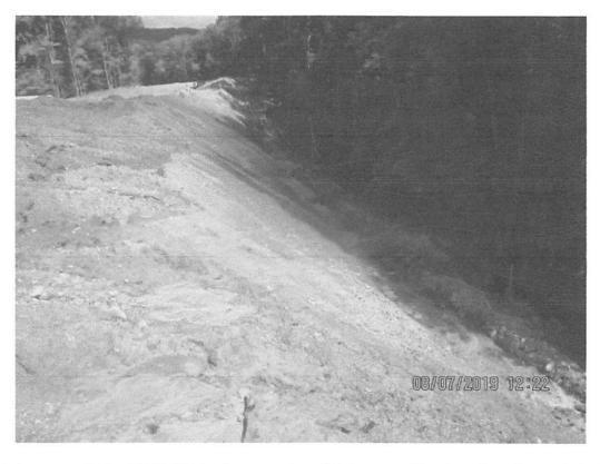
Fill slope near station 8946+00. Erosion present on fill slope resulting in sediment overwhelming perimeter controls.
