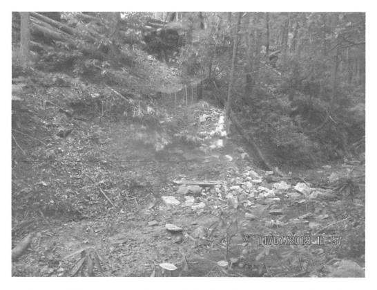
Slip that impacted Elliott Run near Station 3946+00 and was not reported to WVDEP spill reporting hotline. Super silt fence installed near the edge of LOD.
