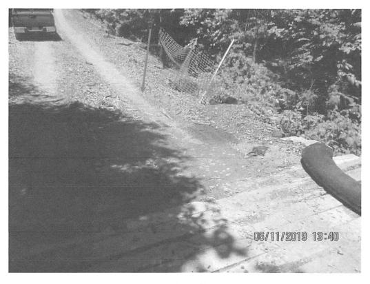
Facing up grade on Access Road 192.5 at wetland crossing W-V6. SWPPP detailed waterbar above this crossing. waterbar had been eroded and was barely distinguishable. Arrow depicts where waterbar was installed and terminated on road bank (slope).
