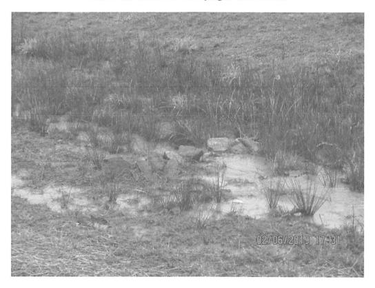
Rock check in ditch with SLW present, draining toward culvert.
