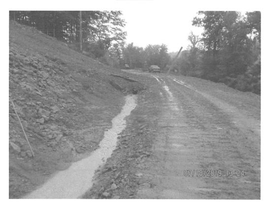
Downslope from where SLW was entering ditch. Arrow depicts culvert that conveys under ROW crossing. No controls present upslope of ditch below station 4539+00.
