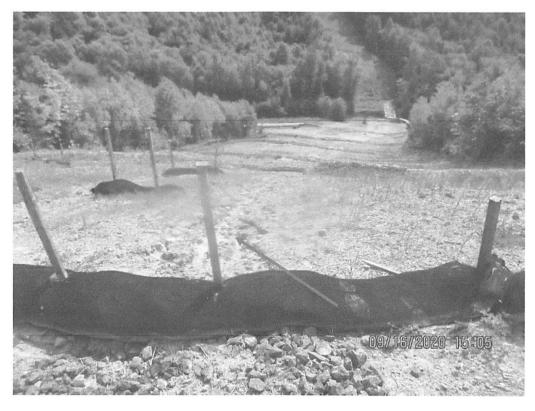
Standing at Access Road 159.01 facing downslope from Station No. 6657+00. Erosion present on slope (red arrow) with deposits in the waterbar channel.
