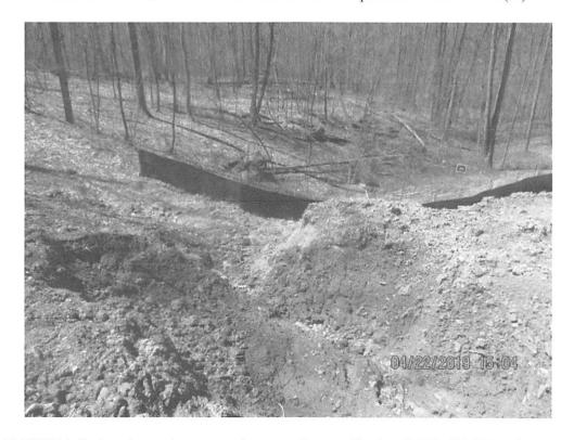
Stream S-T35(A) facing downslope waterbar terminus at Station 8633+71. Waterbar appeared to be directed toward stream. Controls were buried in sediment where erosion was present. Super silt fence was added after clean-up occurred. Sediment deposits were present in stream.
