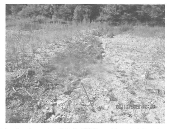
Waterbar with erosion present near Station No. 6703+00, controls in waterbar lacking maintenance.
