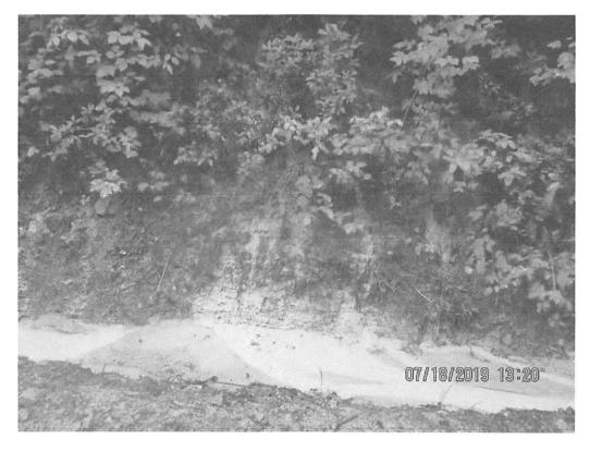
Downslope of failed controls post rain event along Access Road MVP-WB-119. SLW was entering/cascading into the ditch that conveys back downslope toward ROW crossing with access road.
