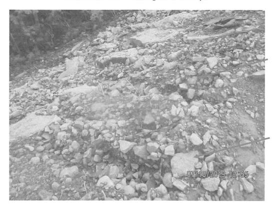
Near station 4559+96, erosion present on fill slope. Arrows depict erosion.
