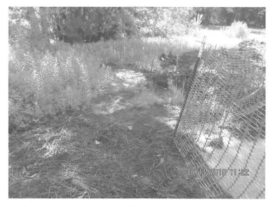
Facing South (Downslope) at station 7609+50. Waterbar outlet controls overwhelmed with SLW and deposits.
