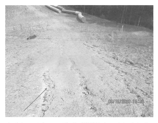
Erosion on slope between waterbars near station No. 6450+76 (red arrows). Area had not been reseeded.
