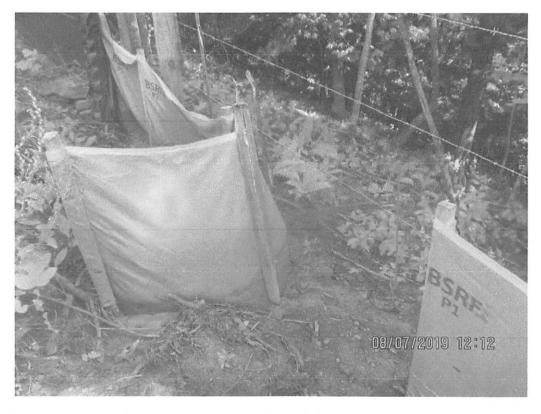
Further downslope near statio 8951+00. Perimeter Controls below waterbar termini with no outlet control terminating onto fill slope and above LOD. Sediment deposits observed past the LOD.
