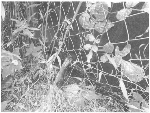
Silt fence is damaged near Stout Run bridge
