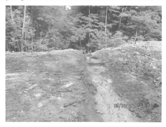
Seep running onto ROW via waterbar above Stream S-N13. Diversion not stabilized near station 6940+00.
