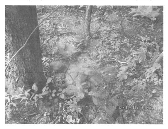
Sediment deposits past the LOD and controls at station 6474+16.
