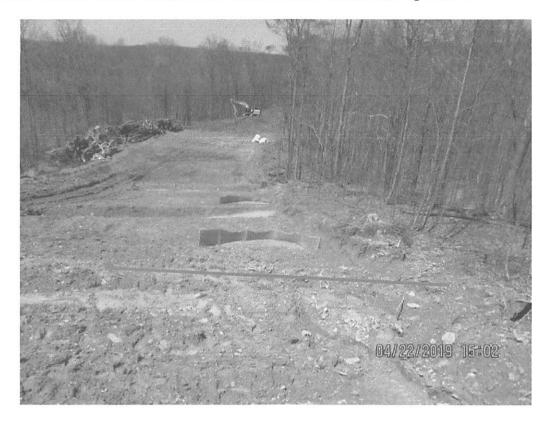
Waterbars terminating onto ROW at station 8633+71 facing North/Downslope. Arrow depicts waterbar overwhelmed with sediment that impacted stream S-T35(A).
