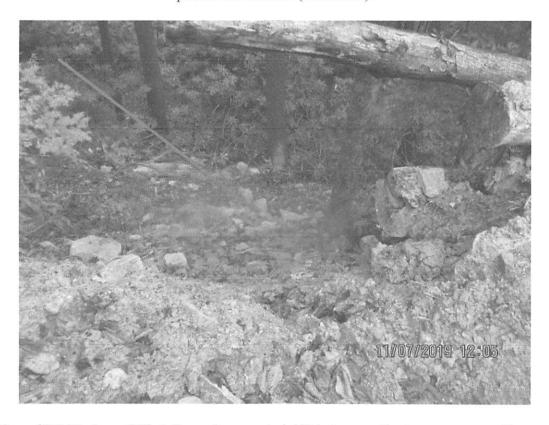
Section of ROW above Elliott Run where material/debris was slipping upstream of larger slip impacting Elliott Run near station 3946+00. No perimeter controls were in place at the time of inspection. Large rocks observed in stream above larger slip.
