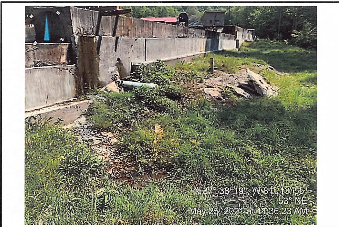
5/25/2021 – Evidence of process water escaping raceway on southside of the structure.
