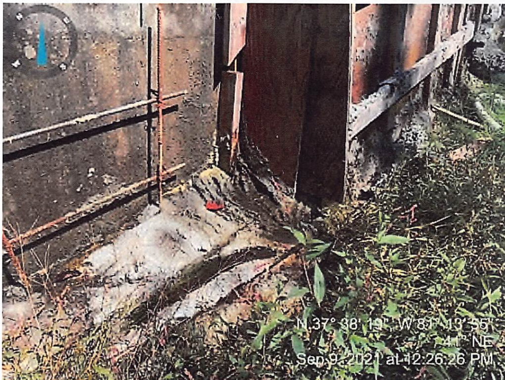
9/9/2021 – Process water leak from southside of raceway.
