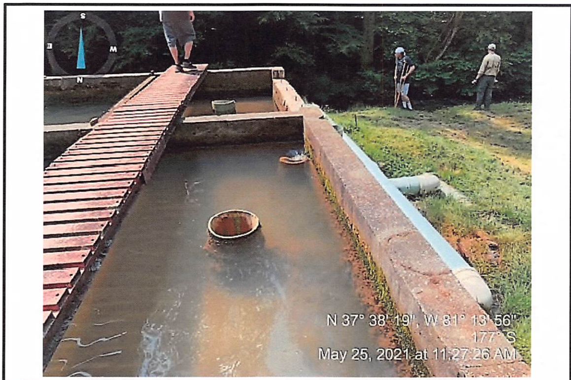
5/25/2021 – Effluent pipe for Outlet 001, as well as overflow pipe for excess discharge.
