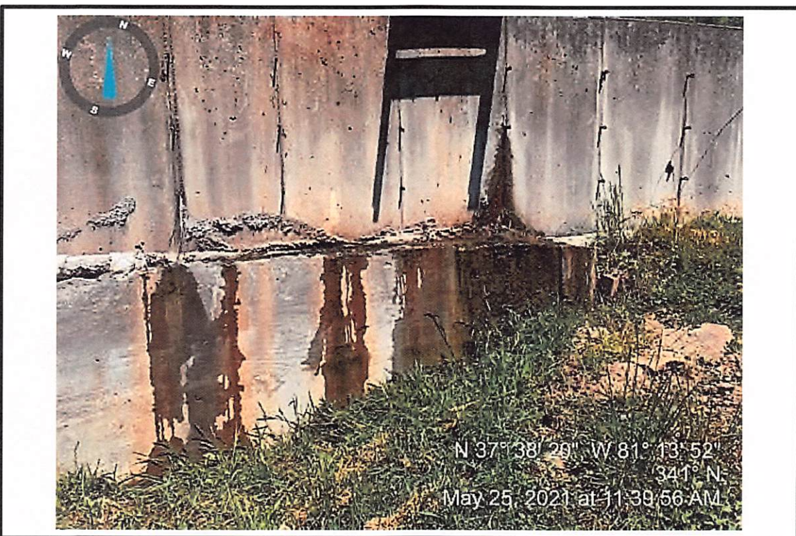
5/25/2021 – Closer view of leaks from the raceway.
