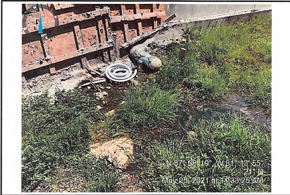
5/25/2021 – Closer view of raceway wall leak.
