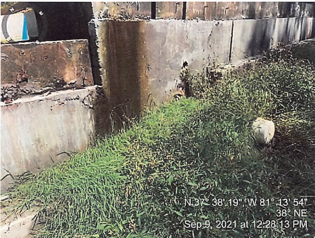
9/9/2021 – Evidence of process water escaping raceway on southside of the structure.
