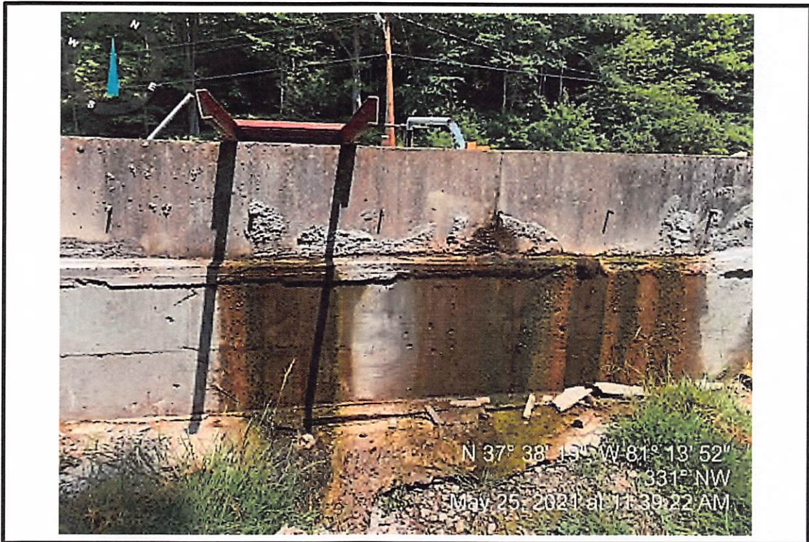
5/25/2021 – More evidence of process water escaping the raceway structure.
