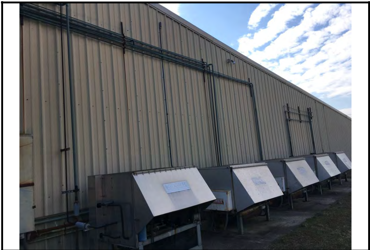
Photo No. 6 Five compressors used for cooling cold rooms. Photo taken 03/06/2017.
