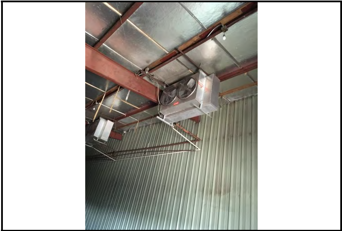
Photo No. 5 Overhead cooling units for cold room. Photo taken 03/06/2017.
