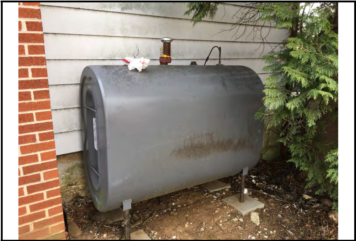
Photo No. 15 175 gallon heating oil above ground storage tank (AST) at residence. Photo taken 03/06/2017.
