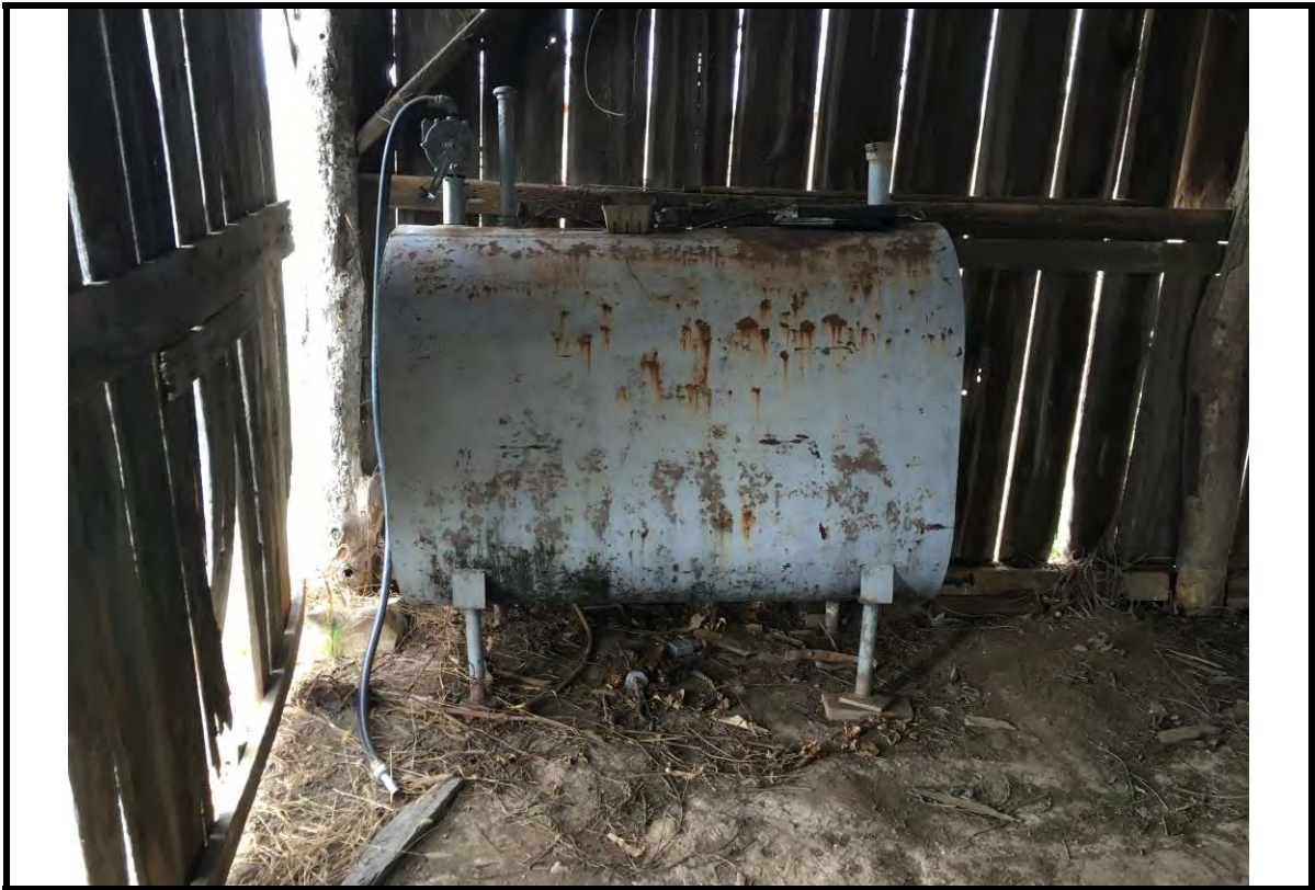
Photo No. 19 AST in dirt-floor barn used for gasoline. Photo taken 03/06/2017.
