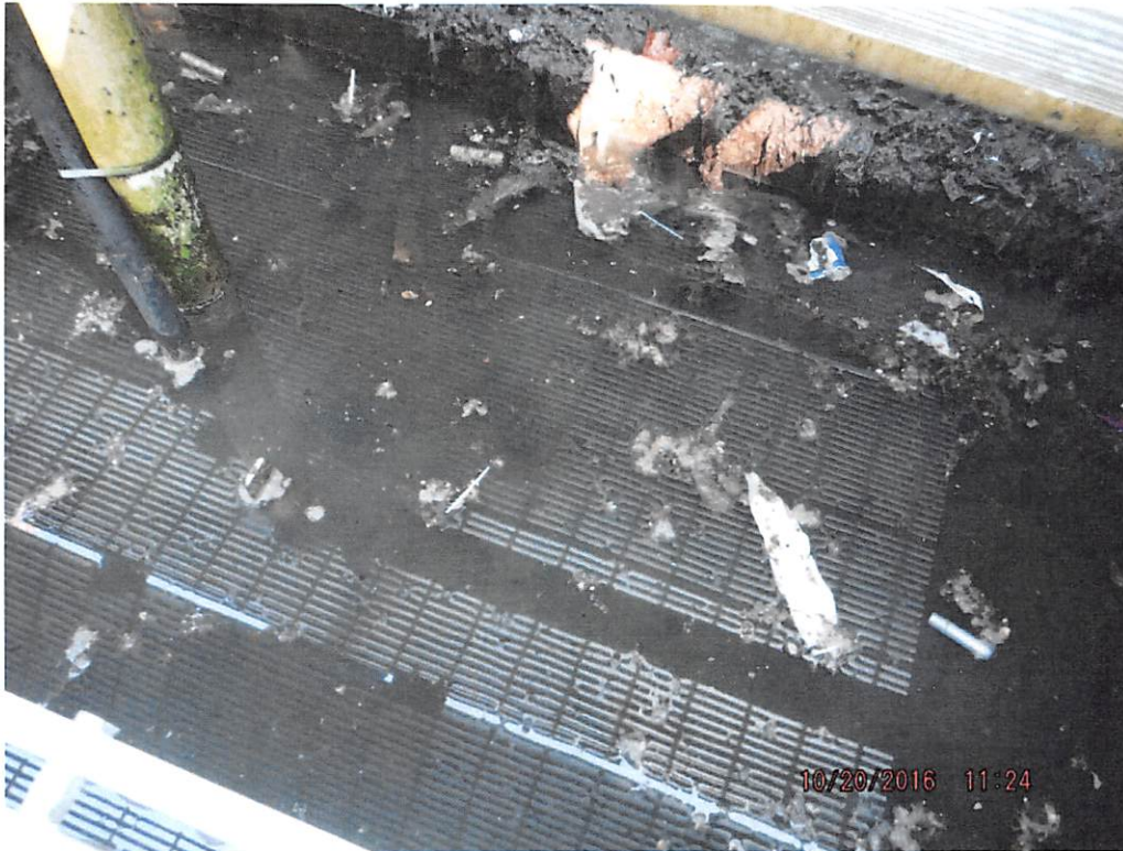
Photo # DSCF8988 – Floatable solids and scum buildup in clarifier No. One (1)
