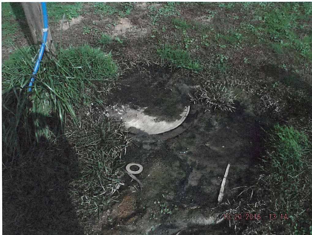
Photo # DSCF9025 – Sanitary Sewer Overflow from a vacuum pit located along Alley Addition
