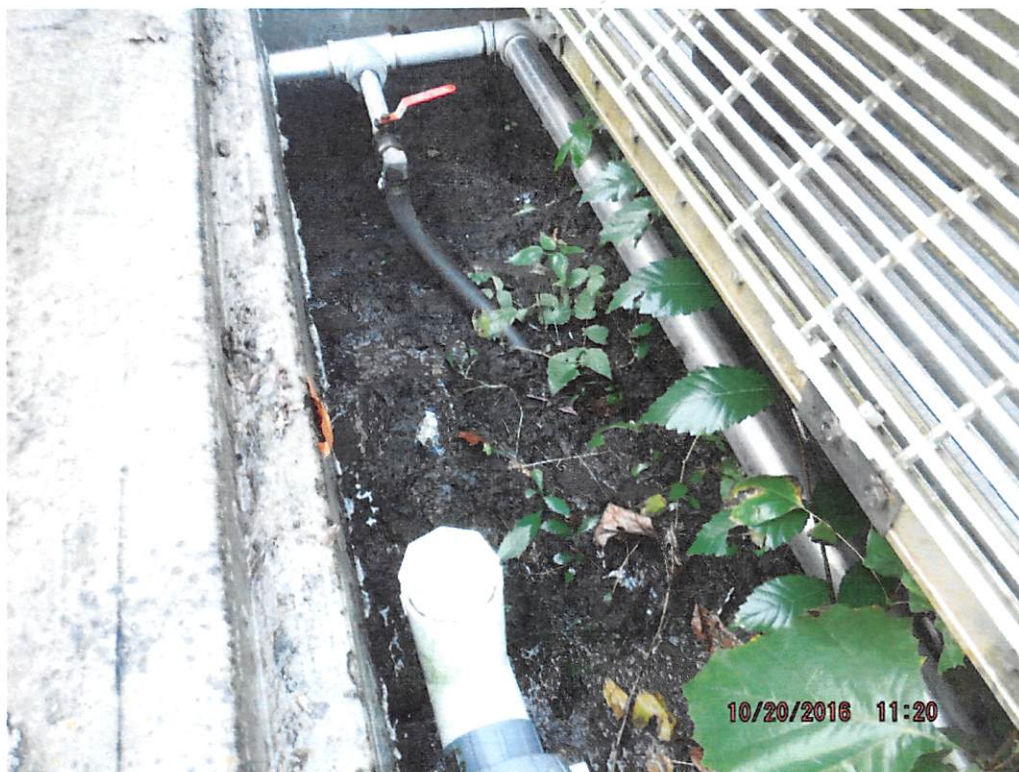
Photo # 8987 – Solids buildup/vegetation growth behind the scum baffle of clarifier No. Two (2)
