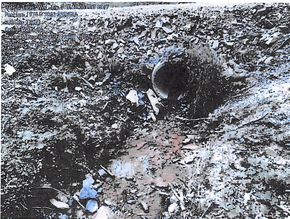
Culvert outlet from project road with sediment laden deposits in UT of Maple Run. 06/07/17
