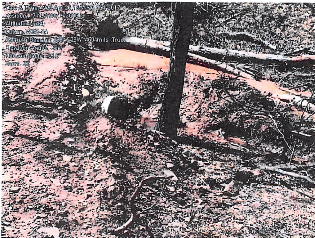
Inlet of culvert with clear water upstream of project road. Note: sediment laden water pooling near culvert inlet. 04/26/17
