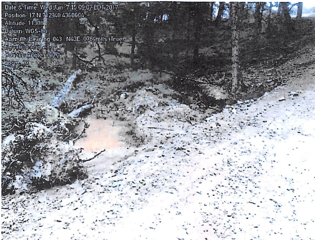
Inlet of culvert upstream of the project road. Note: sediment laden water pooling near culvert inlet. 06/07/17
