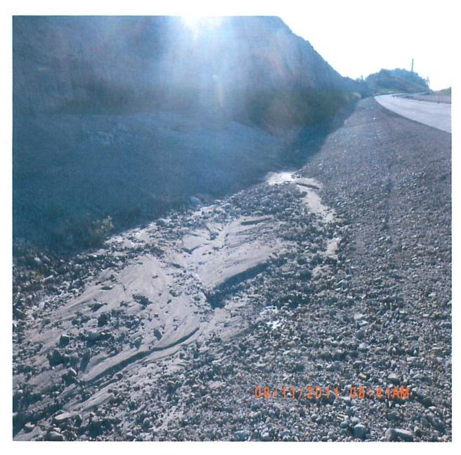
Location of drop inlet that is buried. Runoff bypassing this inlet and flowing to Outlet 016,
