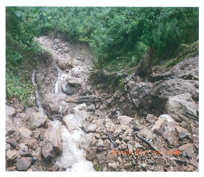
View looking down the unnamed tributary of Spice Branch, from the location shown in the above photo. The sheer cliff can be seen where the AEP access road crossed the tributary and collapsed. The severe erosion and scouring can be seen down this tributary.
