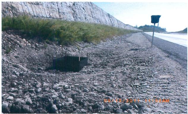
Several drop inlets in the side ditch leading uphill of Outlet 016 have been uncovered and proper protections installed.
