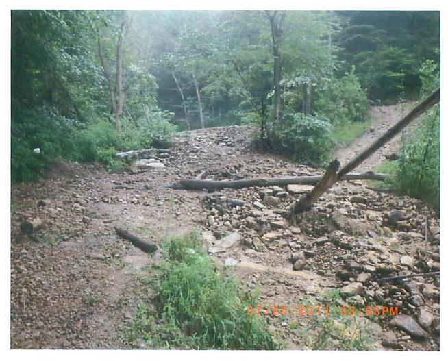
Large amount of material shown completely blocking Spice Branch. Material is approximately 10-12 feet tall and 30-40 yards in length. The remnants of the AEP access road that crosses
