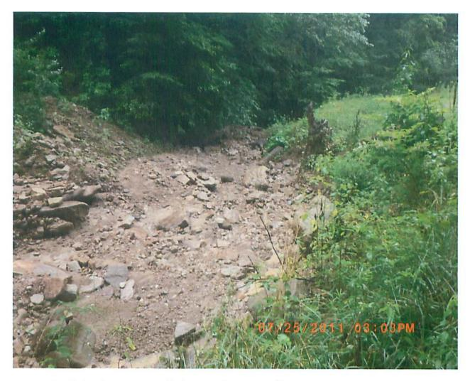
View facing downstream at the bottom of the deposit/blockage. No flow in Spice Branch. Large amount of deposits downstream for several hundred yards.
