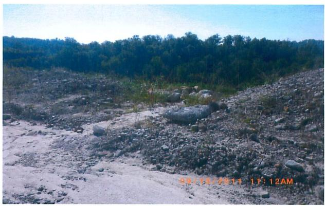
Breach in the berm across from Sta. 1968+00 needs repaired.
