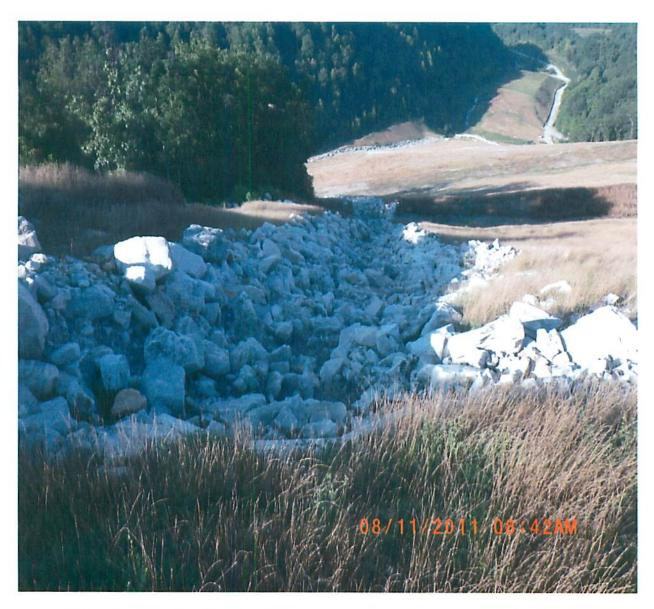
DRG on the east side of Fill #4, with the concrete wingwall shown on the edge of the grass line, which is where the median and side ditch drainage is supposed to discharge.
