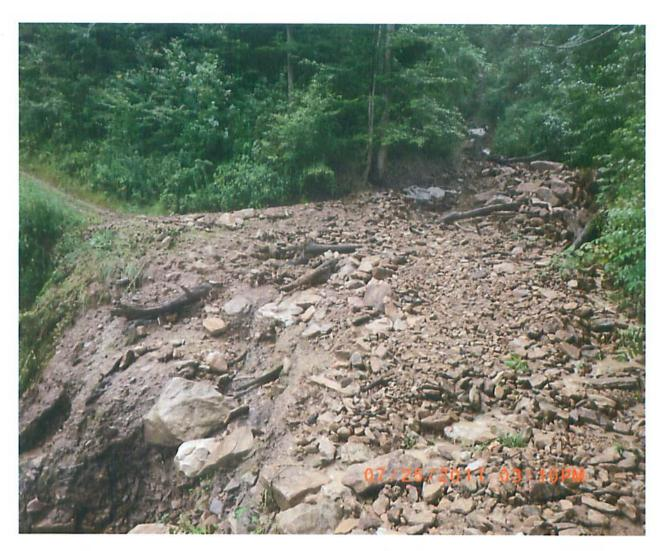
View looking upstream on the unnamed tributary to Spice Branch, approximately 100-150 yards upstream of its confluence with Spice Branch. What's left of the existing AEP access road can be seen in the upper left. The bottom left portion of the photo shows where the road has collapsed, leaving an approximately 20ft sheer cliff in the unnamed tributary of Spice Branch.
