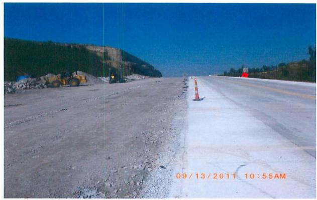
Median drop inlets continue to be buried from the Horsepen connector end to a point near the new high school.
