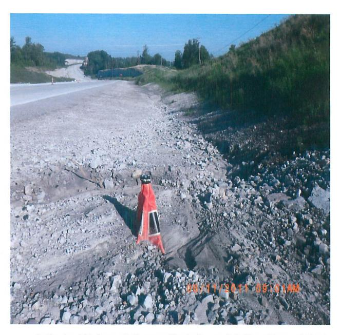
Another drop inlet, shown with the orange DI protection over it, that has not been maintained.
