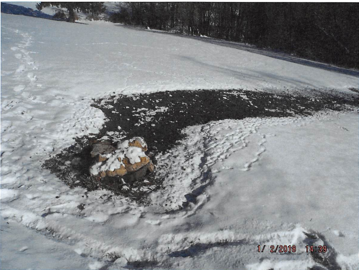
DSCF5009 Sanitary sewer overflow
